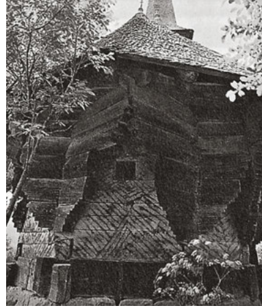
323 The crossing of the bracket timbers was sometimes carried out in an almost overpowering form. – Poarta Salajului, Salaj, Romania
