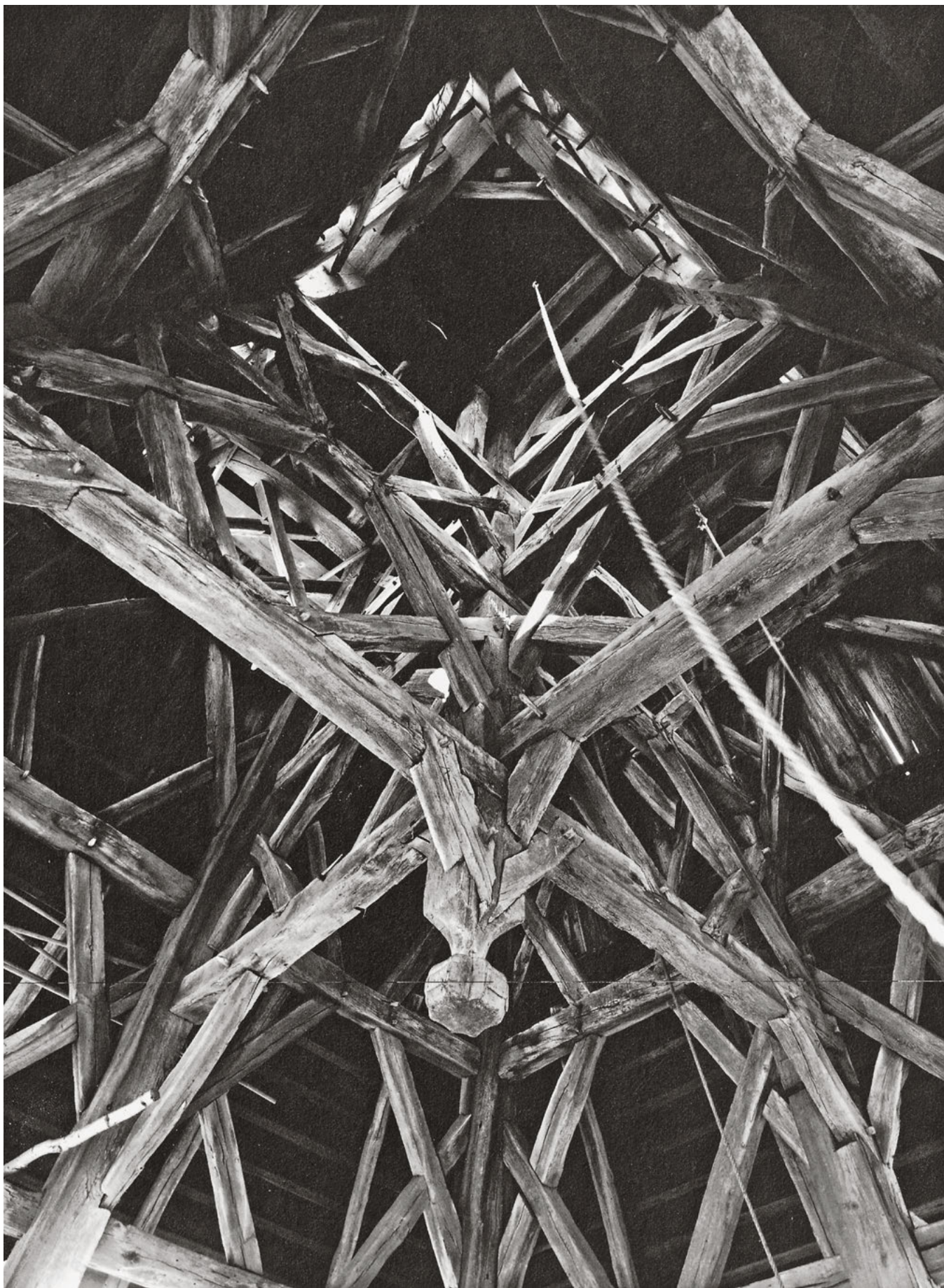
113 The truss-post construction of the bell-tower in Malé Ozorovce, Slovakia, demonstrates which types of construction were dared even in the countryside.
