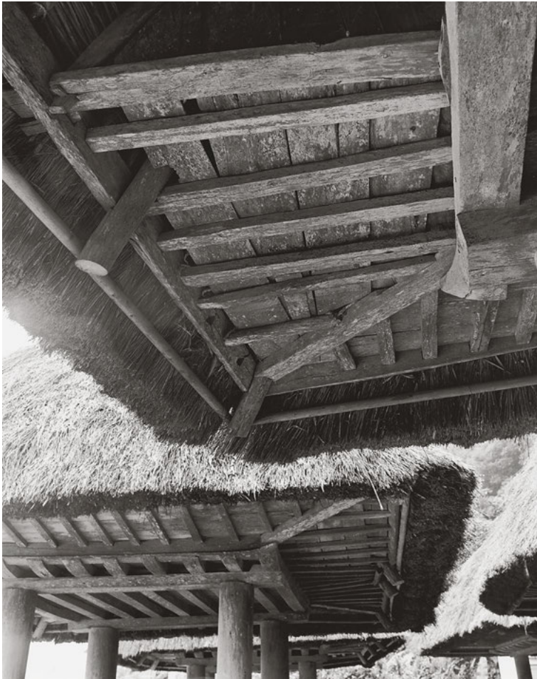
417 The eaves of the Kikunoyo Brewery in Meiji mura illustrate the principle. Underneath, the visible rafters ( kesho taruki ) at an angle corresponding to the ideal of beauty; above, the hidden notaruki carry the roof covering.
