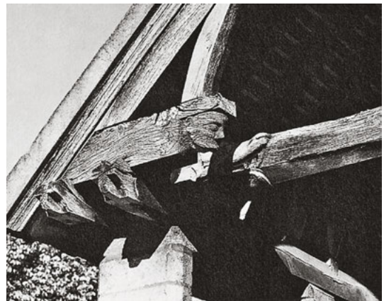
550 Behind the expressively shaped interrupted tie beam, the carved dragon's head symbolizes, inimitably, the task of the tie beam, namely to restrain the feet of roof slopes which are trying to spread apart. – St Nicholas' Church in Beaune, Burgundy, France
