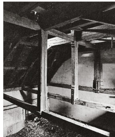
9 Two-part truss posts carry the tie beams in Schloß Thürintal, NE Austria.
