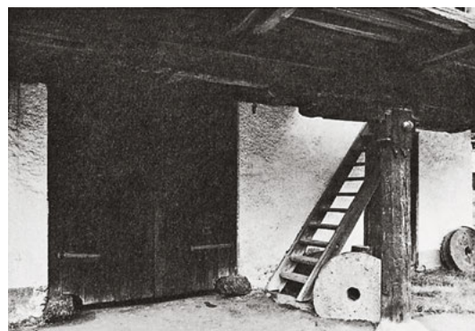
521 This giant bolster under a beam conveys especially clearly, via its function, the value of aesthetic impressions as opposed to economic considerations. – Kirchberg, Tyrol, Austria
