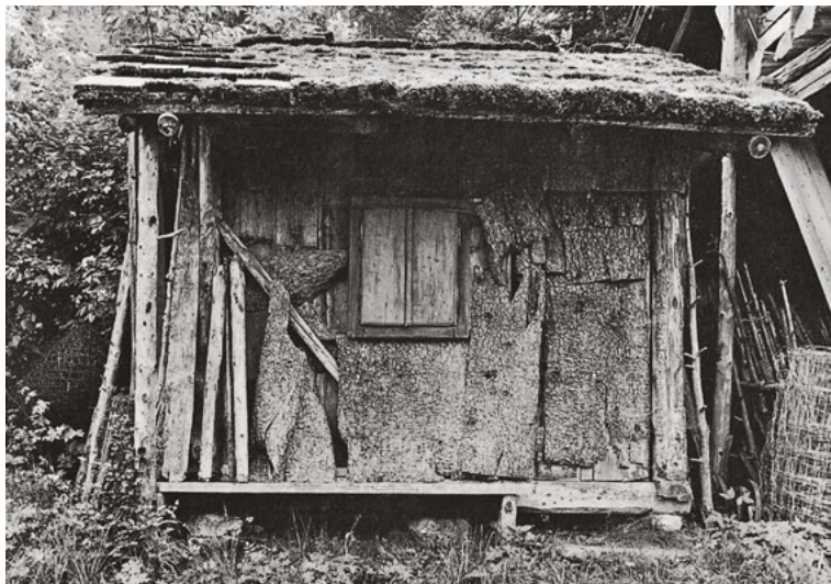
72 Spruce bark protects this small shed in Grundlsee, Steiermark, Austria, against rain.
