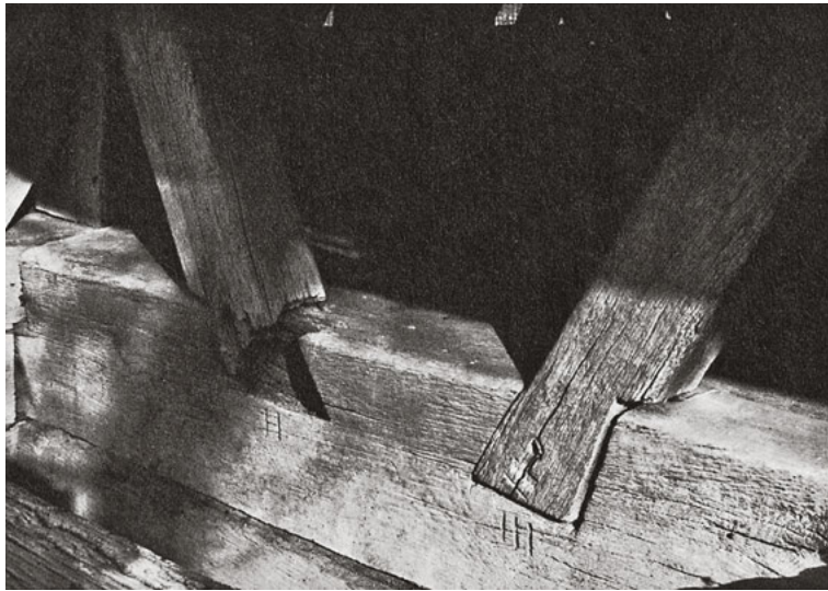
190 The down braces on the bell-tower in Stará Halič, Slovakia, are fixed to the sill beam with single-dovetail lap joints.
