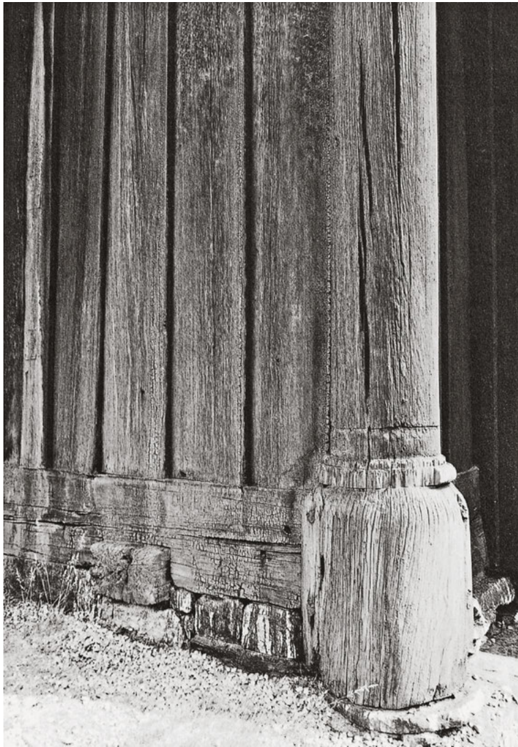
468 The planks of the stave wall to the church in Torpo, Buskerud, Norway, are joined exactly like grooved shingles.
