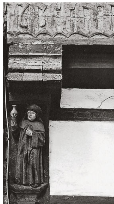
65 Richly carved and painted brackets and sill beams characterize the appearance of those timber-framed buildings in Brunswick, Lower Saxony, Germany, which have survived intact.
