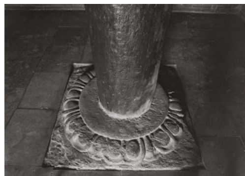
603 Stone column footing from the Kaiyuan si Zhonglou built in the Tang period. - Zhengding, Hebei
