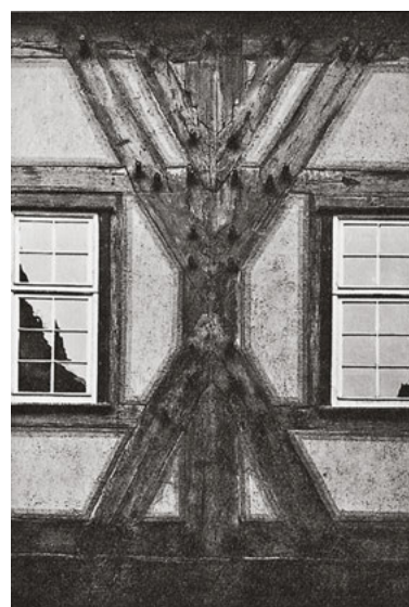
522 In extreme cases the visual appeal strived for was no longer the shape of the lap itself but rather the figures created by the laps. – Town hall in Esslingen, Baden-Württemberg, Germany
