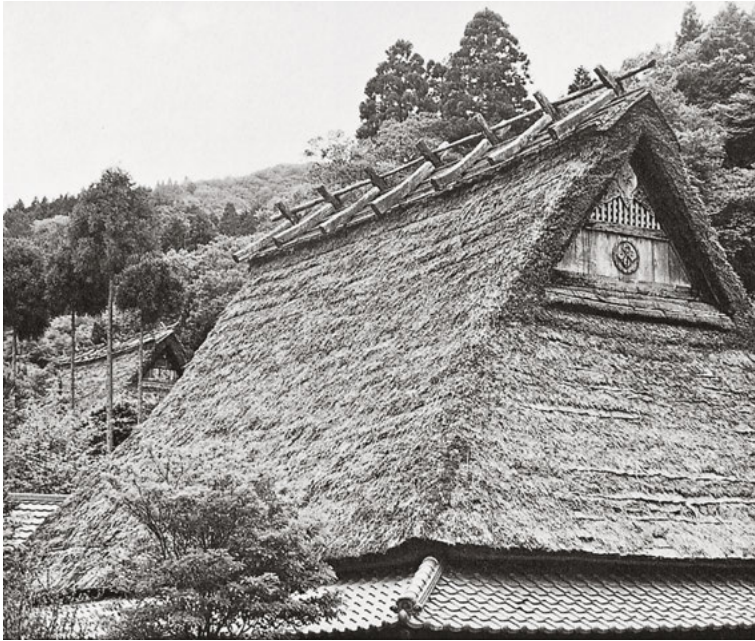
464 Owing to its comparatively short life, the amount of work required and its cost, thatched roofs are also becoming a rarity in Japan. – Hanase, Kyoto, Japan
