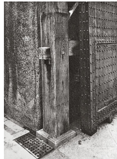
462 Renewed column base on the Osakajo sakuramon, Osaka, Japan.
