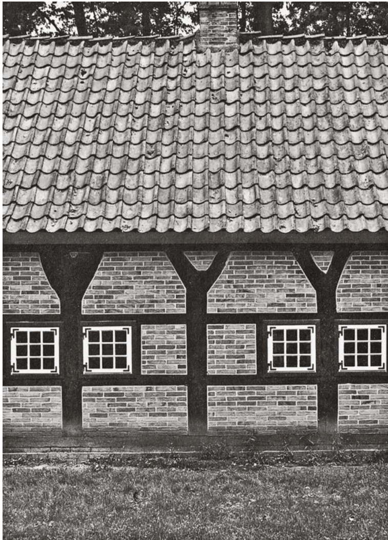
103 The amount of work required to build in the forked columns in the former Foeth House in Menslage, Lower Saxony, Germany, may well have been less than for conventional up braces. Apart from this, these columns create an unmistakable appearance. – Cloppenburg Open-air Museum, Lower Saxony
