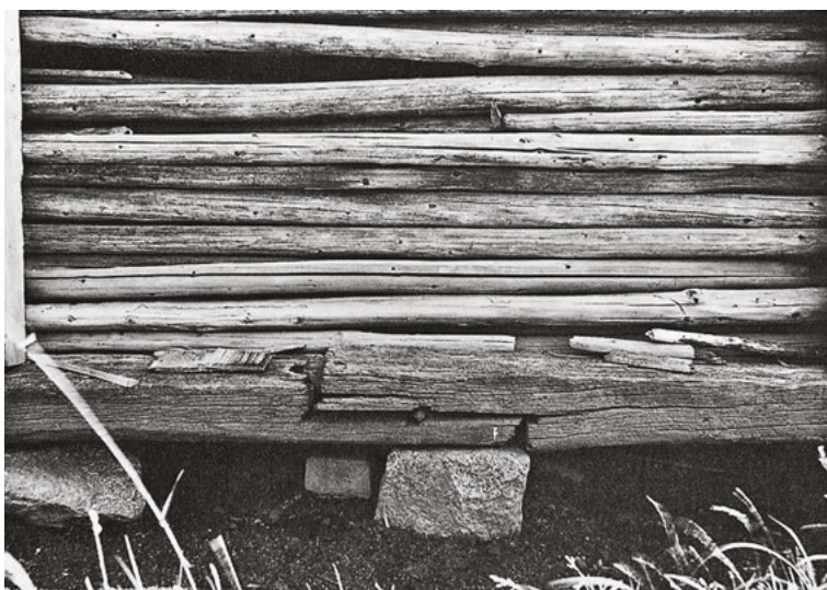
502 The bridled abutment prevents lateral buckling. – Iwate Futsukamachi, Iwate, Japan
