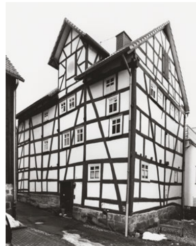
327 Diagonal cross bracing over several storeys characterise this house in Gemünden an der Wohra in the state of Hesse, Germany.
