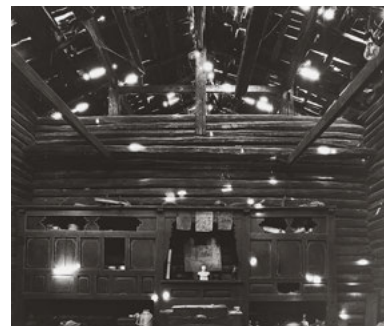
580 The purlins in the roof of this "Grand-mother's room" in Zepo, are borne in part by columns that stand on the ground and in part by columns interlocked with several logs of the wall construction via reversed forked tenon joints.
