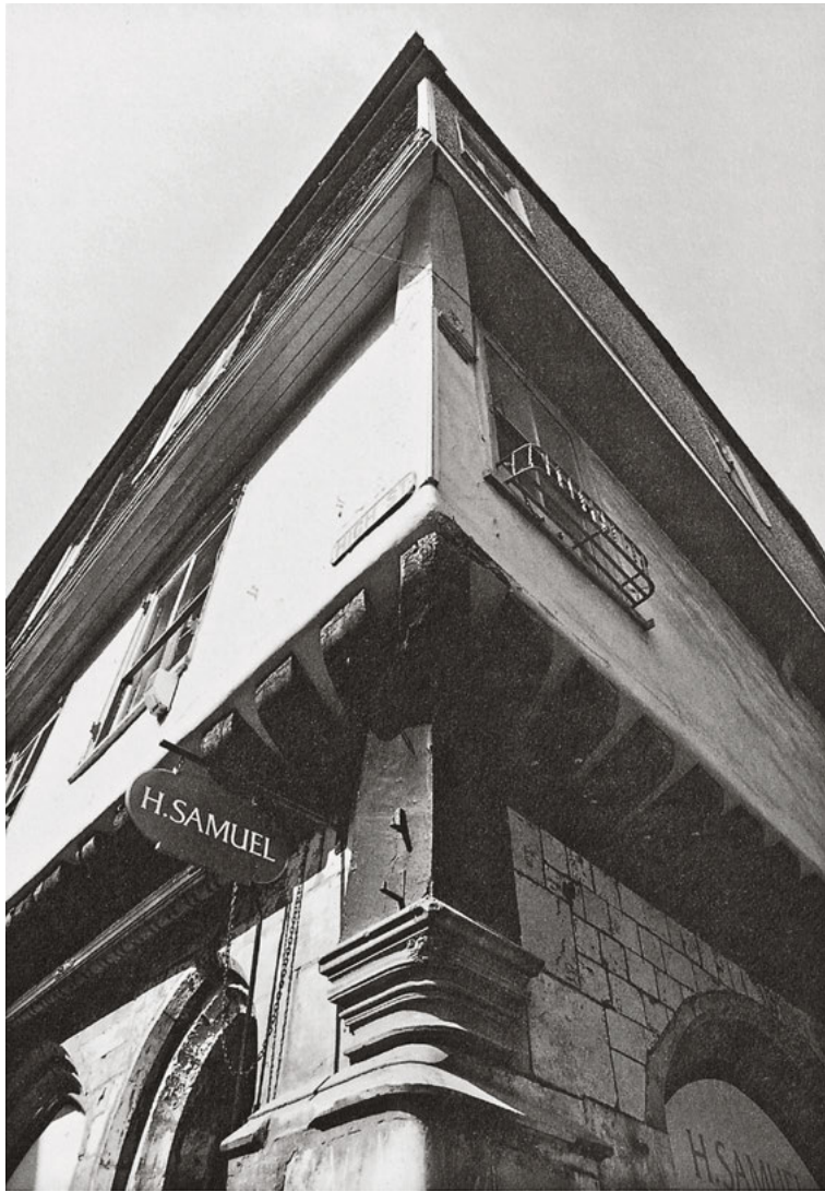
368 The inclusion of tail beams at beam level was necessary in order to be able to cantilever the sill beams in one plane beyond the storey below. – Canterbury, Kent, England
