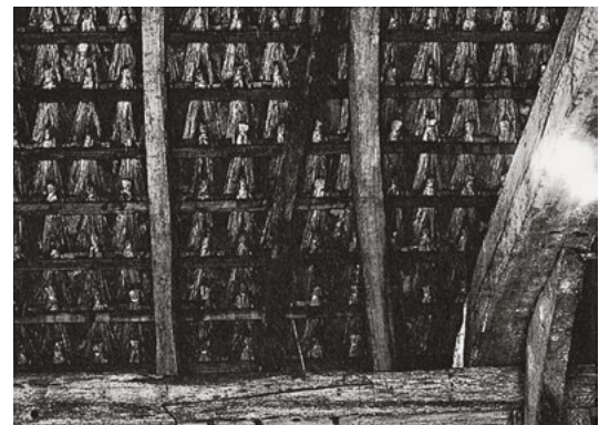
509 Splicing joint in the head beam of the barn in Grönloh, Lower Saxony, Germany, in the Cloppenburg Open-air Museum.
