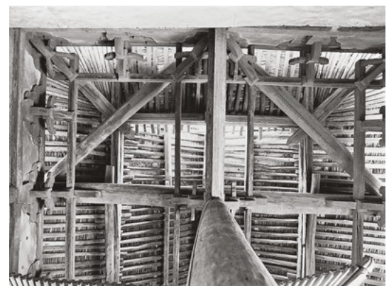
620 View of the underside of the roof construction of the Xia si Shanmen in the Lower Guangsheng si complex.
