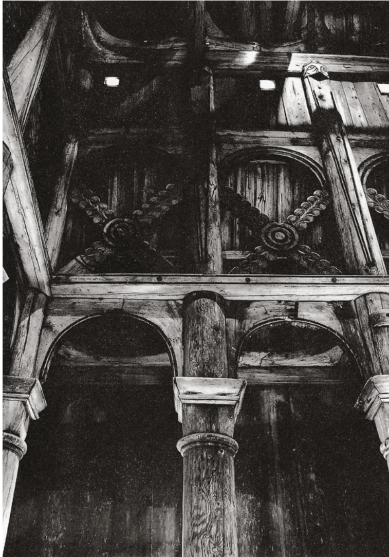
20 As they rise, the tapering of the staves or columns in Torpo, Hallingdal, Norway, is emphasized most effectively by the carved shape of a head at the top.
