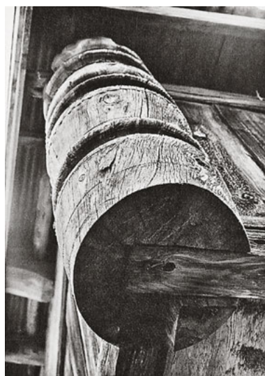
456 The corner column of the jettied svalgang of this stabbur in Øverbø, Telemark, Norway, constitutes optimum protection for the L-joint of the sill beams.
