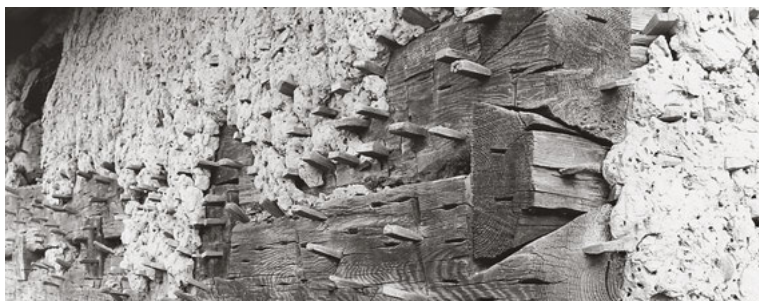
245 Timber wedges as a plaster base for a kitting (store hut) in Dąbrowka Łubiańska, Poland.
