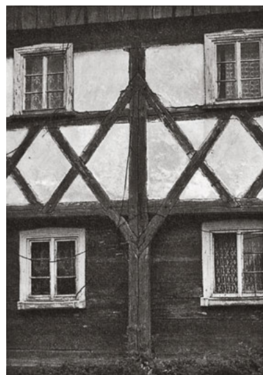
329 Lattice girders enabled a generous spacing of the columns in Umgebinde construction. – Heřmanice, Czech Republic
