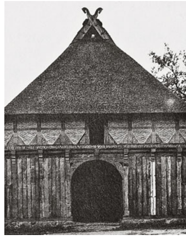
558 The rosette, in this case carved in the triangle formed by posts and down braces, was a very discreet form of constructional cover-up. – Brümmer farm from the Lüneburg Heath, Lower Saxony, Germany, in the Hösseringen Open-air Museum
