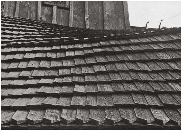
37 Left: The cleft shingles laid at a relatively flat pitch on the roof of the church in Inovce, Slovakia, will probably last considerably longer than the sawn vertical planks.
