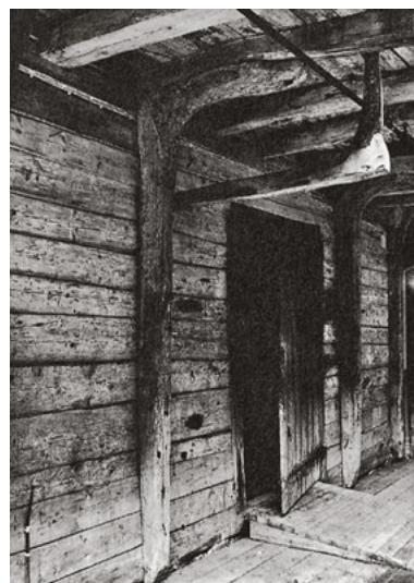
59 Root and branch beginnings like on these columns in Bryggen in Bergen, Hordaland, Norway, contribute considerably to their durability and perhaps also to their aesthetic appeal.
