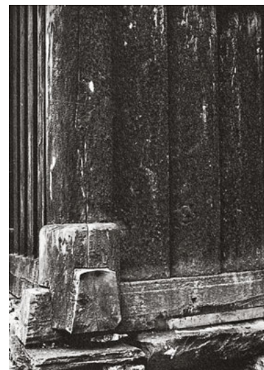
279 The trapezoidal cross-section of the beams underneath the support had the effect of providing a stabilizing, wide bearing. The taper towards the top allowed the supports to slip down as the timber shrank. – Corner of svalgang , stave church in Hopperstad, Sogn, Norway.
