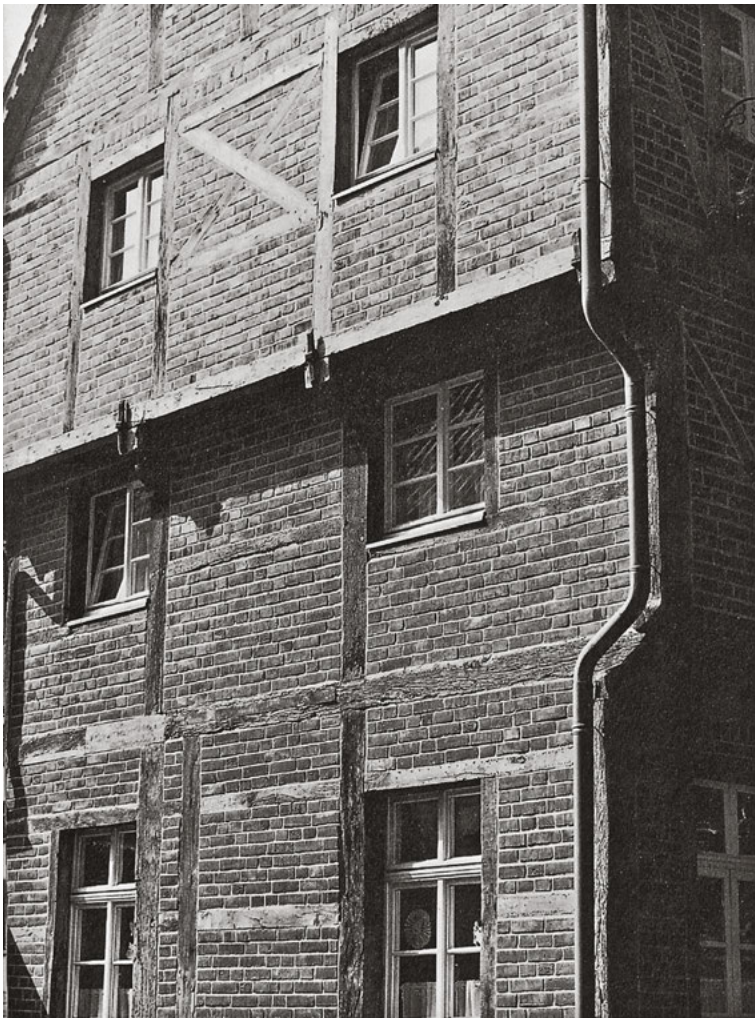
367 Before the introduction of trimmer beams the construction could be jettied using the projecting tie beams or the projecting header beams if they were supported on joists. – Goekmanns Spieker in Nottuln, North Rhine-Westphalia, Germany
