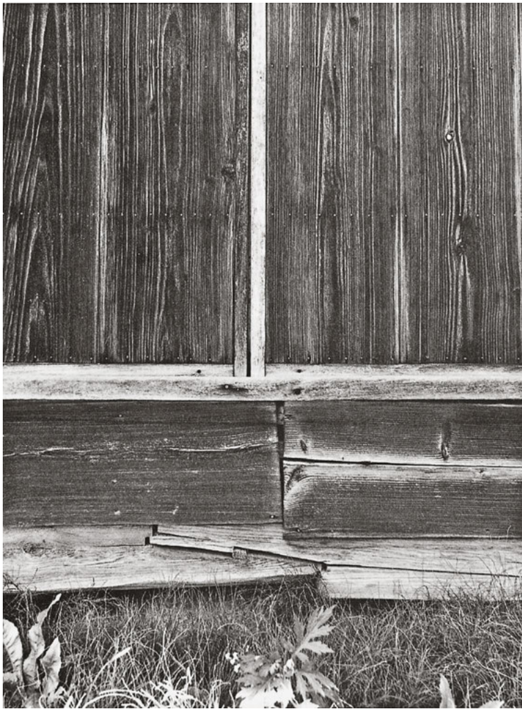
501 A kanawa-tsugi in a sill beam. – Iwate Futsukamachi, Iwate, Japan
