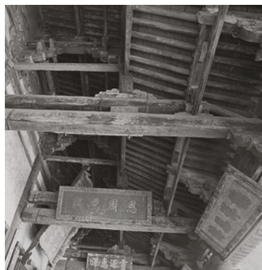
598 Looking upwards from below, one can identify which parts of the construction of the main façade carry which set of eaves.
