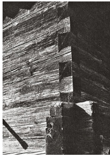
265 Many different forms of Klingschrot can be found. This specimen in St Corona, NE Austria, exhibits very accurate jointing.
