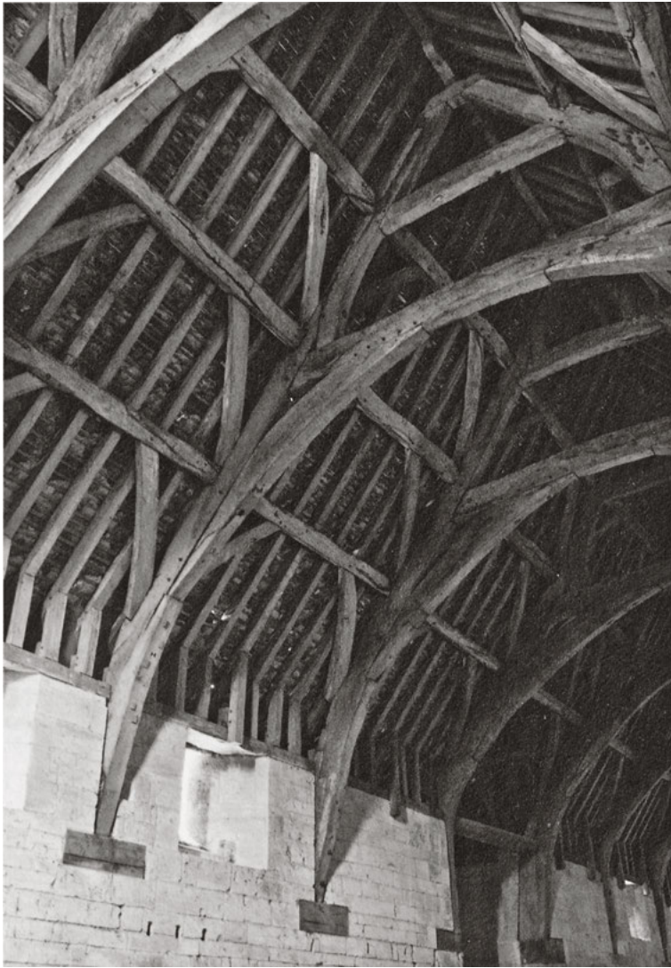
106 The cruck construction over the tithe barn on Barton Farm at Bradford on Avon, Wiltshire, England, in which nearly every truss is built differently. One variation: the roof slope timber runs through to the connecting piece below the ridge.
