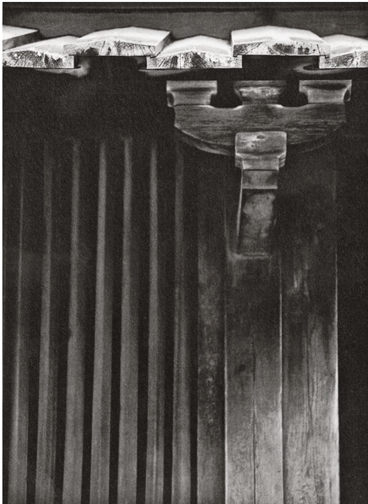
472 The roof covering to the Nyakuochi jinja, Hyogo, Japan, formally embodies the essence of the bamboo roof concept in timber.
