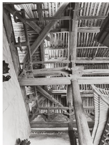
646 In the Xia si Shanmen in the Lower Guangsheng si, the diagonal braces at the corners exhibit an arrangement characteristic of the Yuan period.
