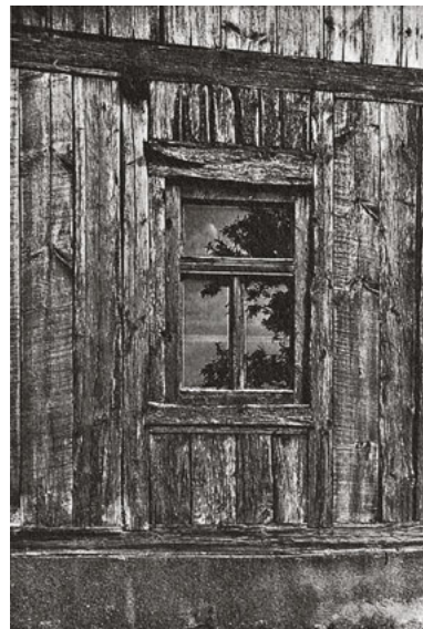
152 Column-and-beam construction with vertical plank filling in Goricko, Slovenia.
