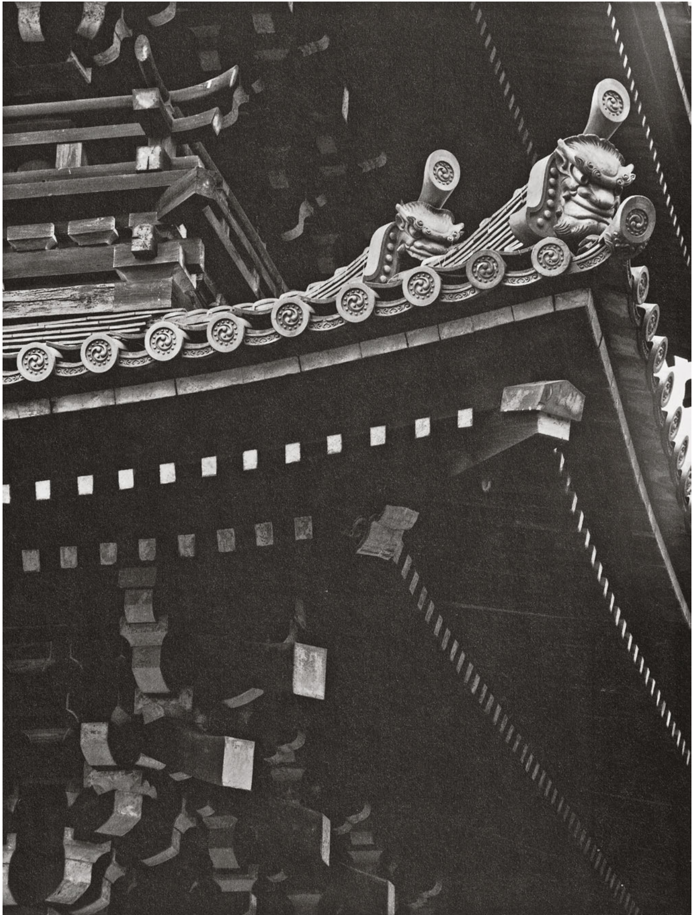
420 The ornamental roofing tiles placed on the very ends of the hips reinforced the impression of the raised eaves corners. – Shinyodo in Kyoto, Japan
