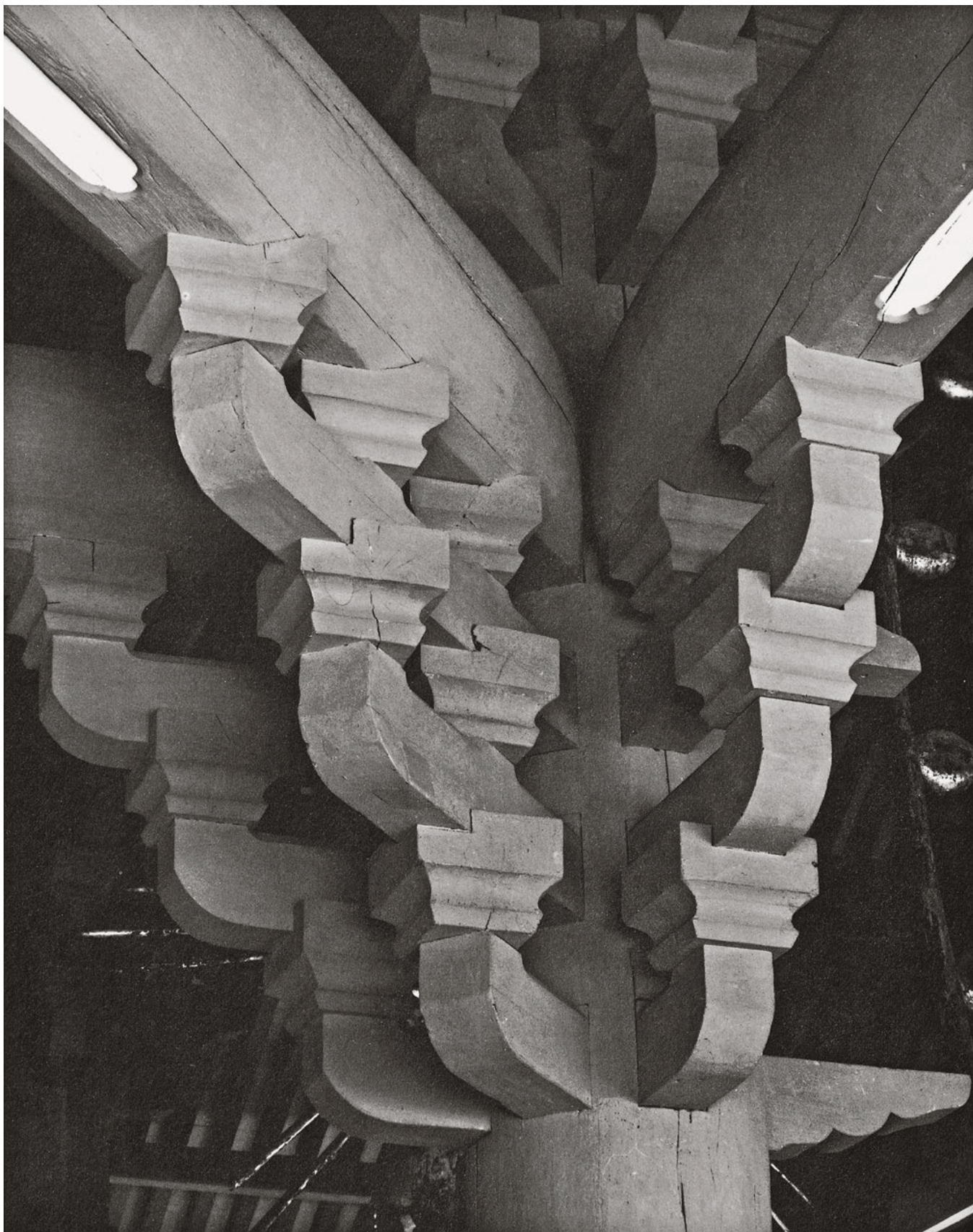
342 Besides being an admirable engineering solution, the way in which the, relative to the column, unbelievably large beams are attached to each of the four columns of the Jodo-ji jododo is really quite impressive.
