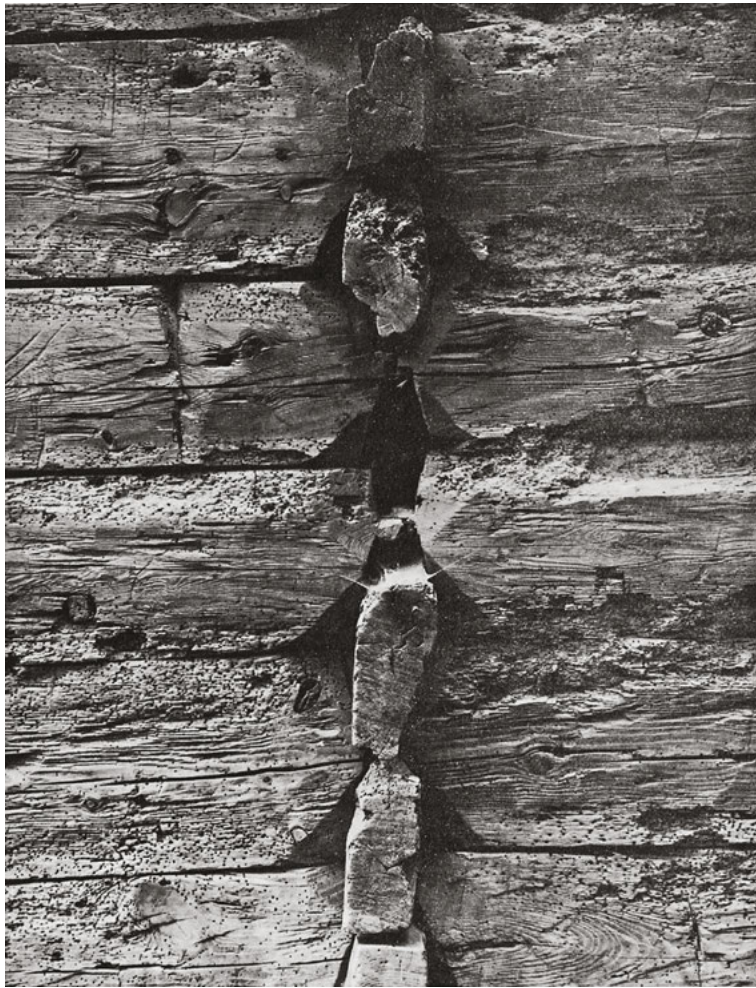
293 An accurately fitted kinning was decisive for sealing the joint. – Bergen, Hordaland, Norway.
