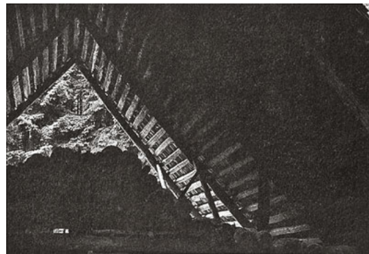
288 A very odd Ansdach roof is hidden, protected from wind and weather, under the pitched roof of a lumberjack's hut near Mixnitz, Steiermark, Austria.
