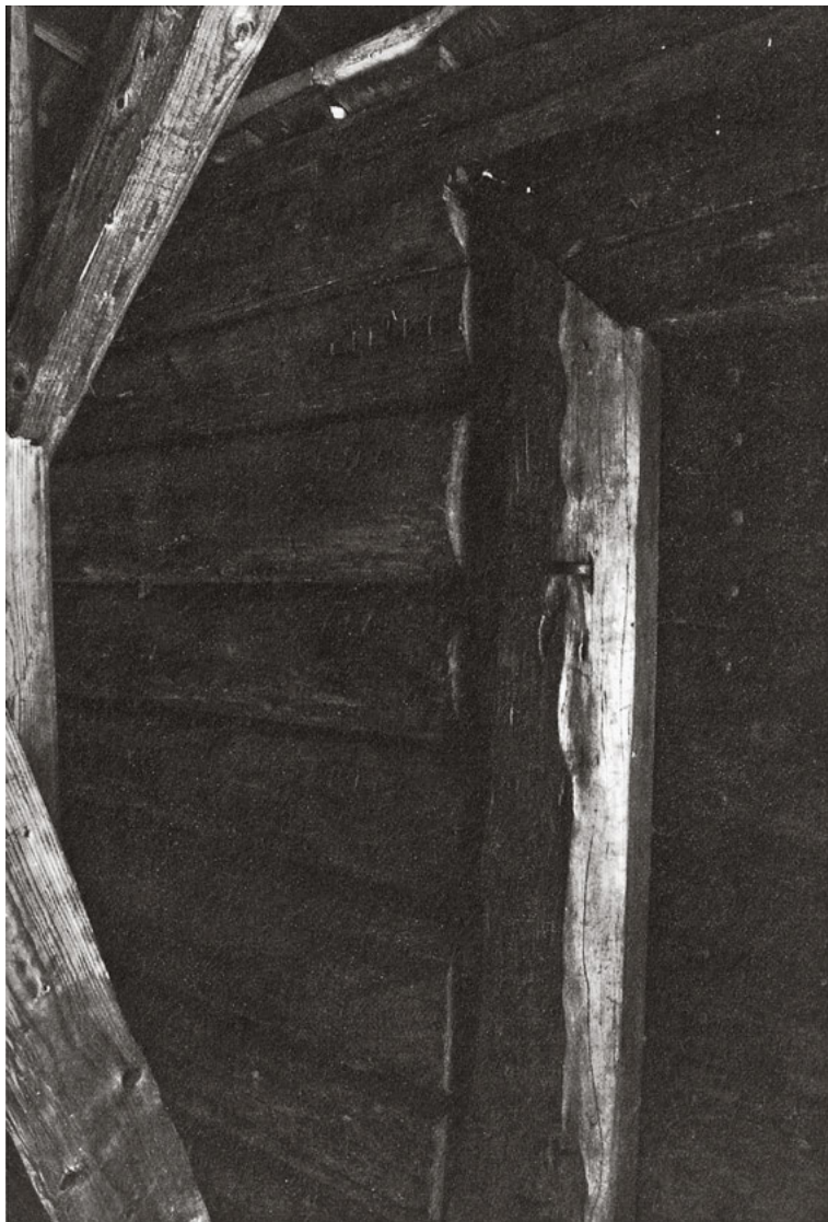
162 The logs of the Kosmas and Damian Church in Lukov-Venecia, Slovakia, are numbered successively, starting at the bottom.
