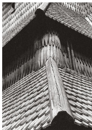
23 The ridge covering on the stave church in Heddal, Telemark, Norway, will not fulfil its function for very long.
