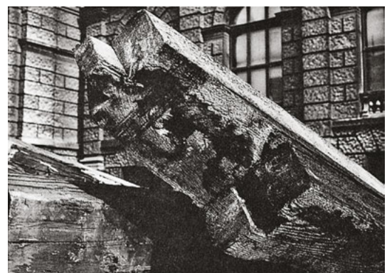
504 A beam from the old roof truss of the Natural History Museum in Vienna, Austria.
