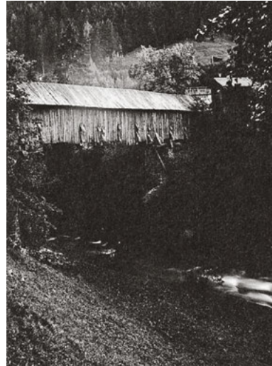
46 On this wooden bridge in Strengen, Tyrol, Austria, the whole of the side facing the prevailing wind is covered with planks.
