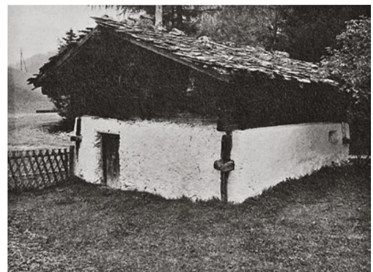
250 A stone wall secured with wooden anchors in Vinaders, Tyrol, Austria.
