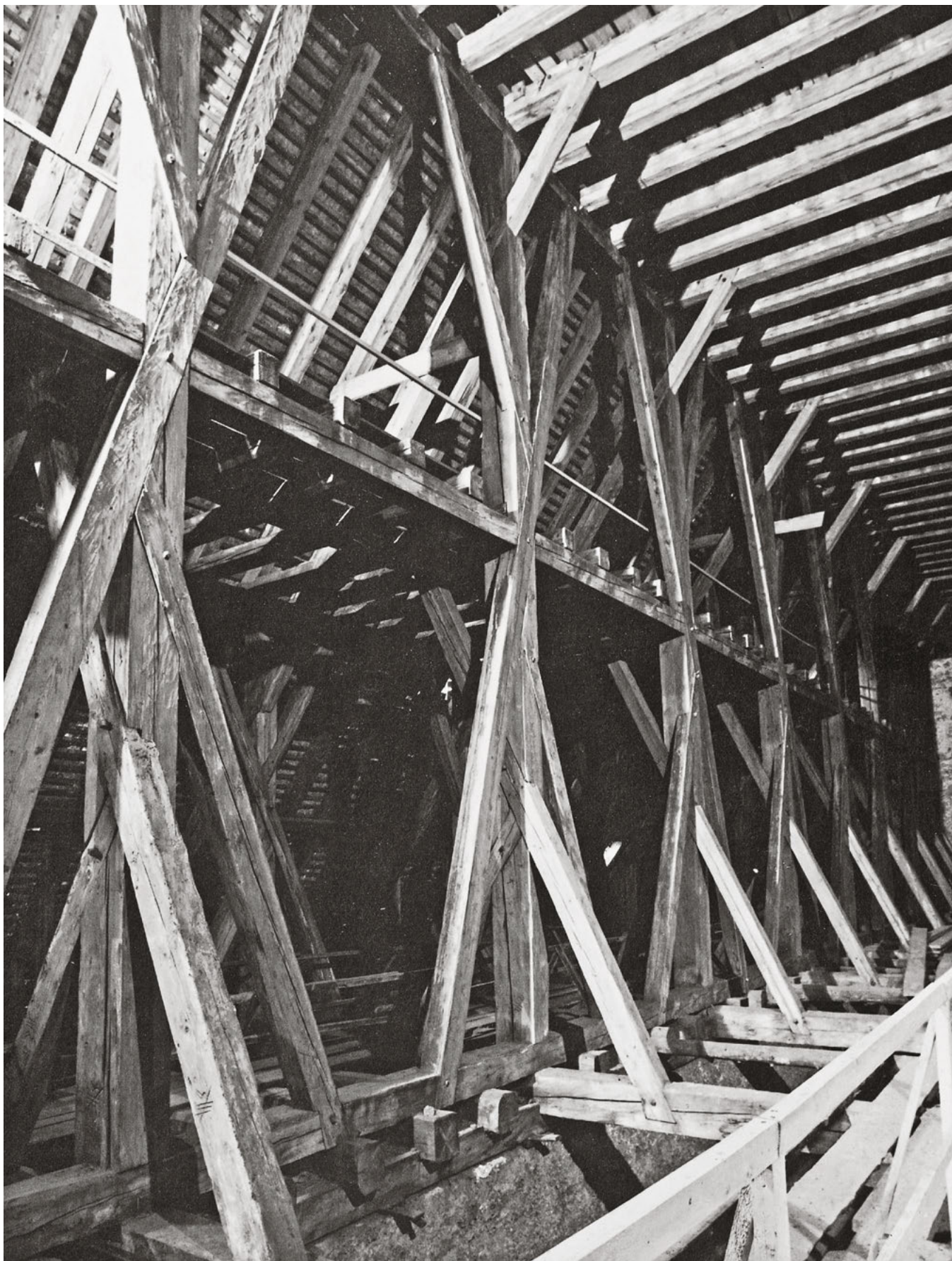
405 Just the queen-post assemblies of the Gothic Collegiate Church in Neuberg, Steiermark, Austria, consume a vast quantity of timber.
