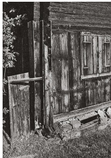
35 The projecting ends of logs were often clad for protection. – Farmhouse in Gaschurn, Vorarlberg, Austria.
