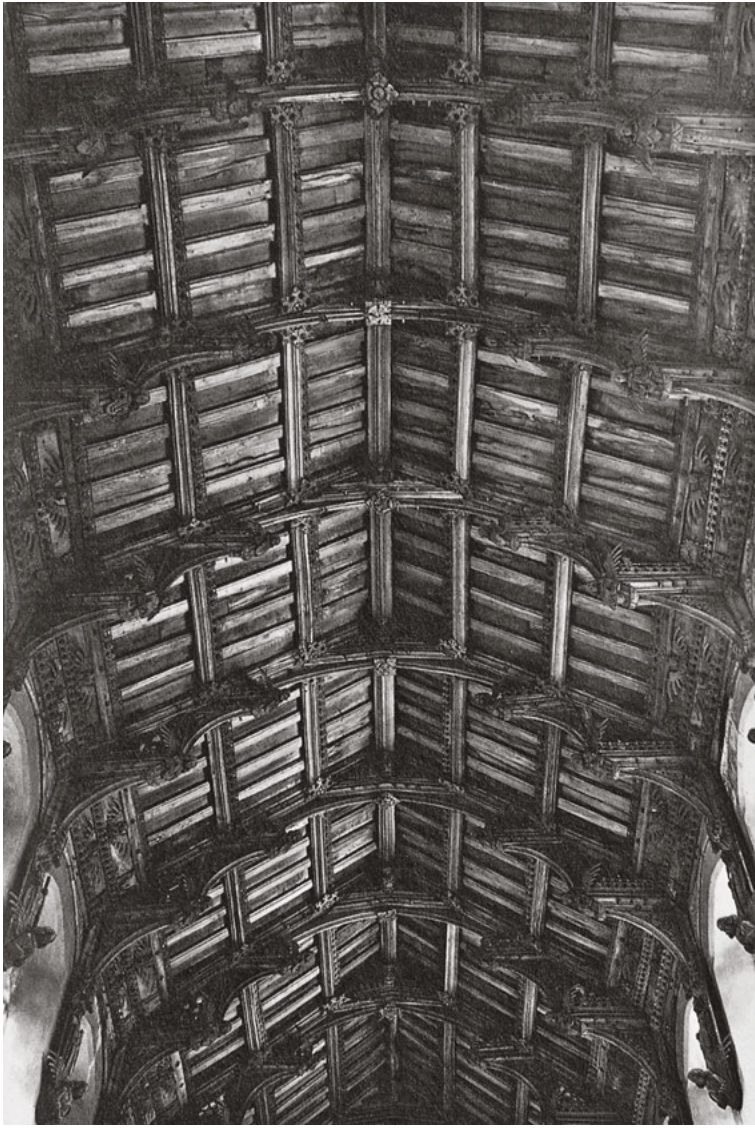
109 The hammer beam roof to the church in Woolpit, Suffolk, England.
