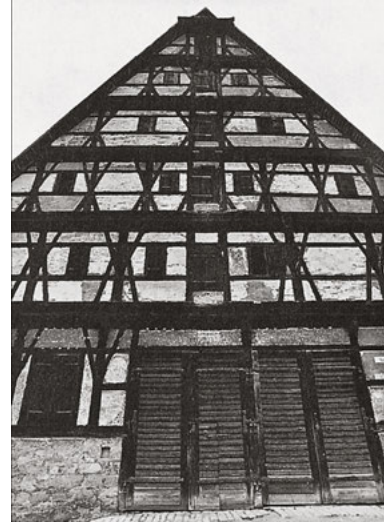
395 Moving down from the ridge, the number of supports must be increased from floor to floor in order to be able to carry the loads. – Kornhaus am Bauhof in Dinkelsbühl, Bavaria, Germany
