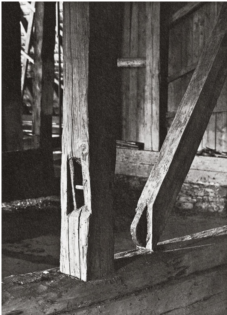
195 The tenon parallel with the grain in the upper step joint especially designed for truss posts (according to: ibid. , Fig. 87) is very much at risk. The second version would be just as effective and much less problematic with respect to twisting of the wood.
