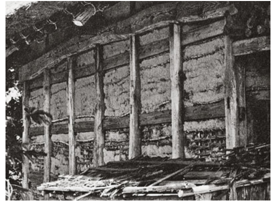
229 Wattle-and-daub infill panels on a minka in Iwate Futsukamachi, Iwate, Japan.
