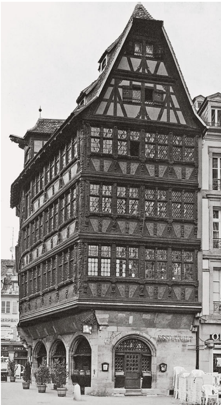
387 Sprocketed eaves lent many buildings a characteristic “kink” in the shape of the roof. – Kammerzell House, Strasbourg, Alsace, France
