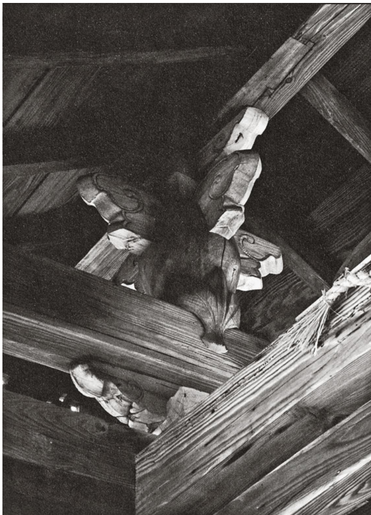
179 The ridge purlin above the gateway of the shokei-yashiki residence on Miyajima, Hiroshima, Japan, is joined adjacent the support.
