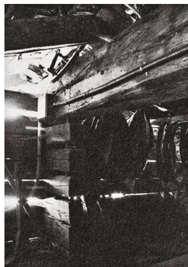
310 The one and only function of the short, wall-like stack of stub logs is to prevent the members of the gable end from buckling. – Feld, eastern Tyrol, Austria
