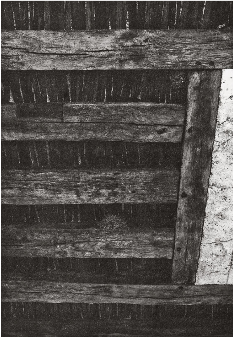
220 The gaps between the beams over a passageway through a house in Coulommiers, Île de France, are filled in with loose, unworked wooden sticks laid next to each other; these then carry a filling material.
