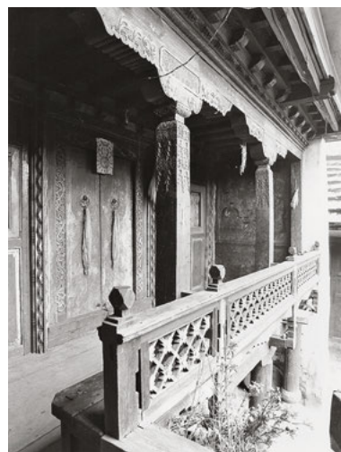
634 The columns of the veranda in this farmhouse in Lijiazui are richly decorated in front of the entrance to the house's altar. The columns bear a large block as well as a short and a longer bolster.
