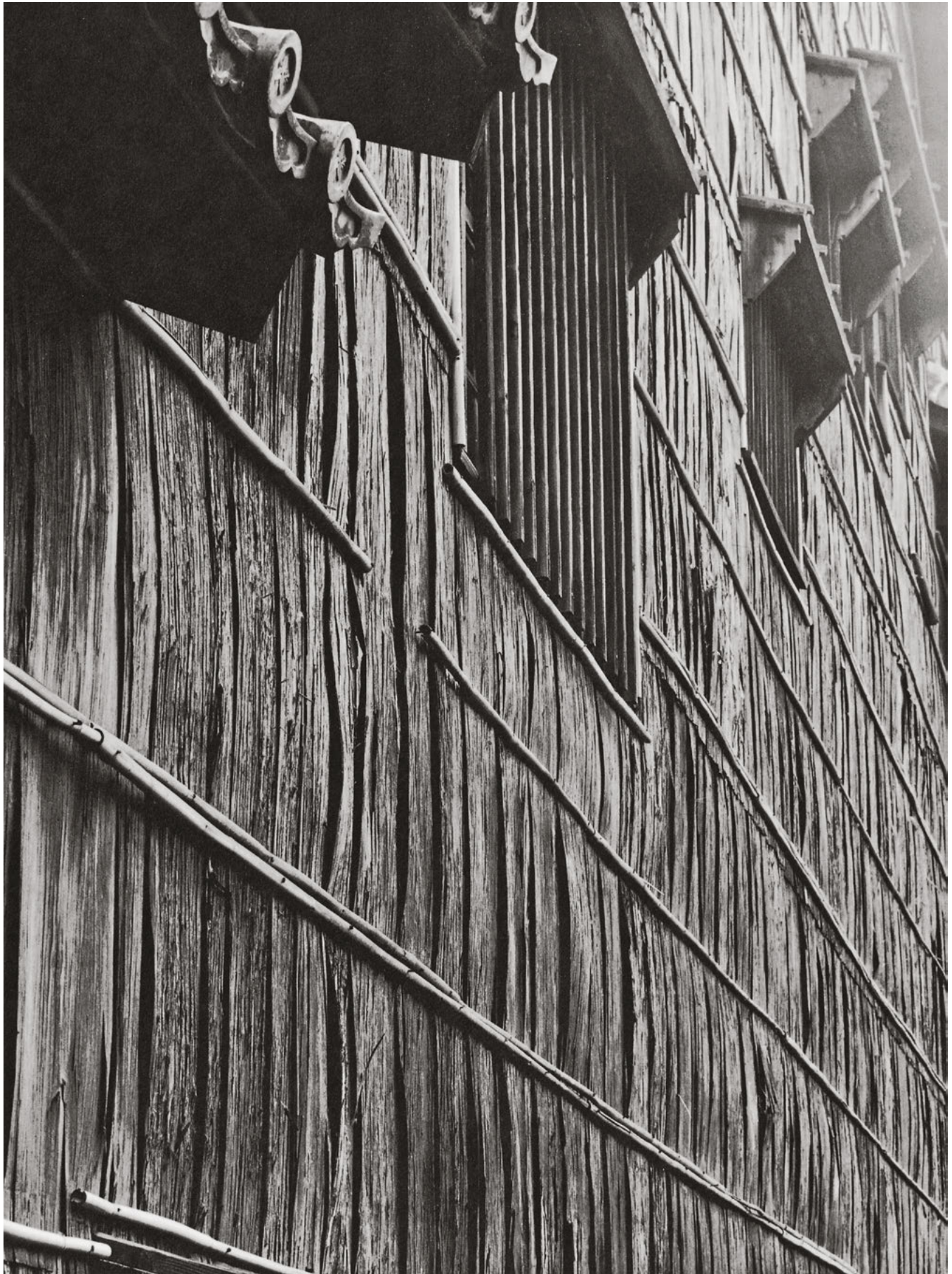
70 Cypress bark cladding on the wall of the Tomatsu House from Nagoya, Aichi, Japan, in the Meiji mura.
