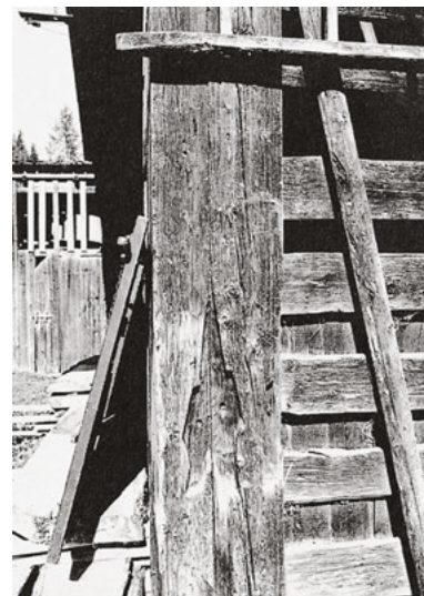
5 The corner column of this barn in Zaunhof, Tyrol, Austria, is made from two older columns. This can be recognized from the lap-joint housings and nail holes of former bracing members.
