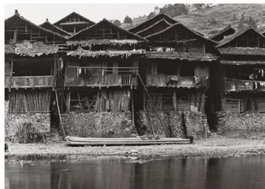
583 The many open and permeable sections of external wall show how important ventilation was. - Pingliu, Guangxi
