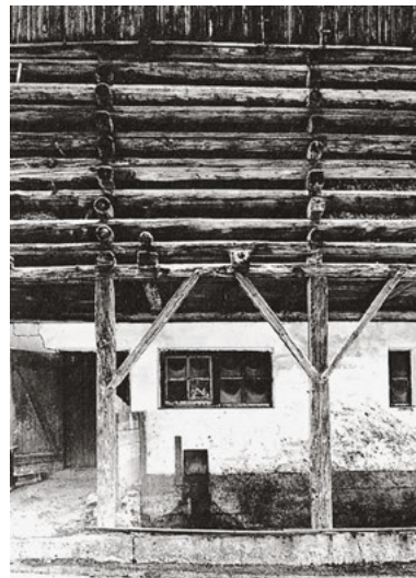
2 In technical terms the loading capacity parallel to the grain is greatest. However, in a structure, as compressive forces increase so does the susceptibility to buckling. – Cowshed on a farm in Zaunhof, Tyrol, Austria.
