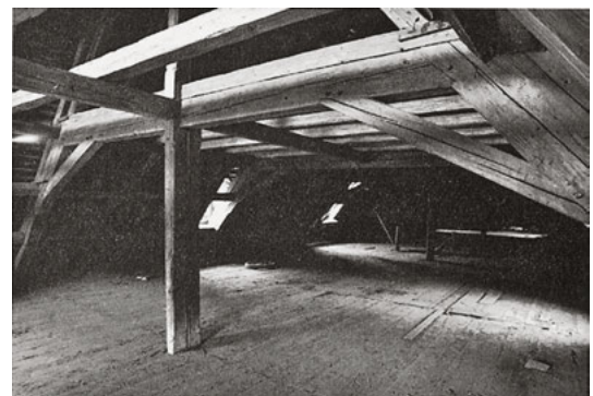
398 In warehouses it seemed obvious to include a row of king struts passing through every floor for additional support. – Primmersdorf, NE Austria
