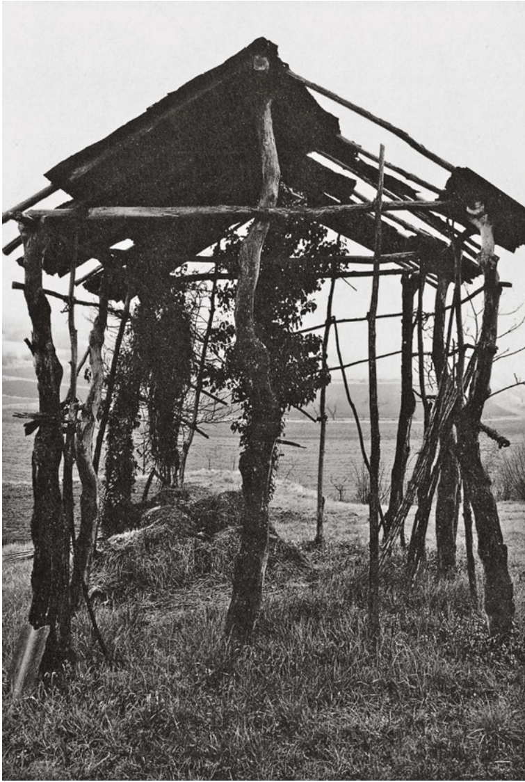
86 A very primitive construction made from pieces of wood simply gathered from the forest which clearly illustrates the principle of column-and-beam construction. – Near Ferenci, Slovenia
