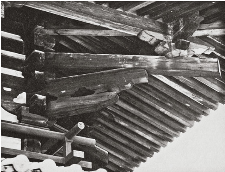
376 The cantilever brackets of the Horyu-ji gojunoto, Nara, Japan, were obviously overloaded as the bearing for a lever arm, not least due to their distinctive and unique “cloud-pattern” shaping.
