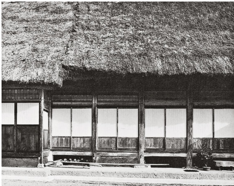
474 Air circulation below the building was at least as important as that within. – Ainokura, Toyama, Japan
