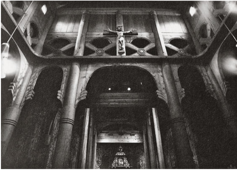
97 During the refurbishment of the stave church in Heddal, Telemark, Norway, no further attention was paid to selecting naturally bowed timbers.
