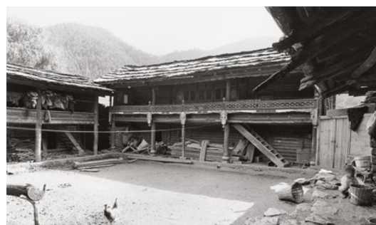
606 View from a "Grandmother's room" of an interior courtyard formed by four buildings in Dacun, Yunnan.
