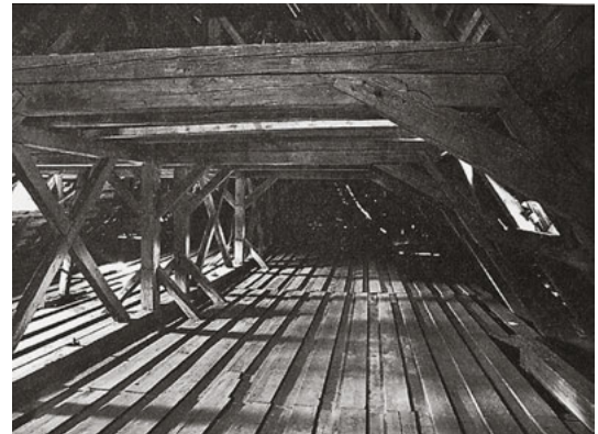
397 In churches in many places, truss posts were still included in the roof construction, not least because of the often heavy ceilings attached underneath. – Liberk, Czech Republic
