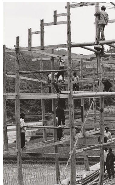
581 The unfinished skeletal timber framework shows clearly how precisely the rough-cut pine trunks have been worked with an adze in order to connect as many columns as possible with a horizontal beam. - Pingpu, Guangxi
