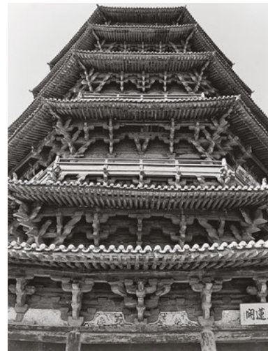
644 From even a cursory glance at the eaves of the Yingxian muta, it is clear that it has a large number of different dougong .
