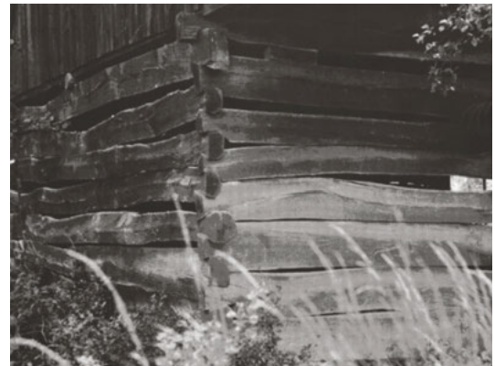
75 As column-and-beam construction was unknown in this region, even such totally unsuitable timbers as these were pressed into service for log construction, like for this cowshed in Stará Halič, Slovakia.
