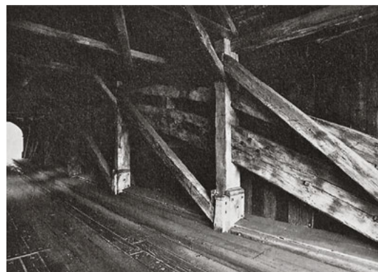
126 Johannes Grubenmann used indented beams to strengthen the girder members of the strutted frame abutting every truss post on the Rümlang bridge near Oberglatt, Zürich, Switzerland.
