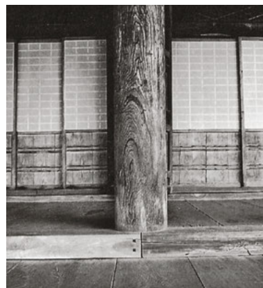
66 The column and floorboards of the Zuisen-ji in Inami machi, Toyama, Japan, illustrate the impressive grain of keyaki wood.
