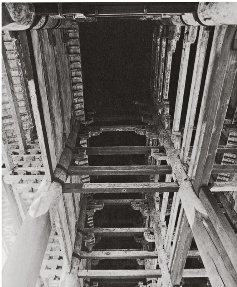
61 In 1199 as Todai-ji nandaimon, Nara, Japan, was rebuilt after its destruction by a typhoon, there was still sufficient timber available for selecting the almost 20-m-high columns.
