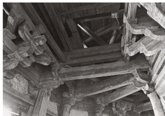
629 In the open storeys one can see additional columns placed to the left and right of the walkways. Occasional openings in the ceiling reveal a view of the structure of the intermediate inaccessible storeys.
