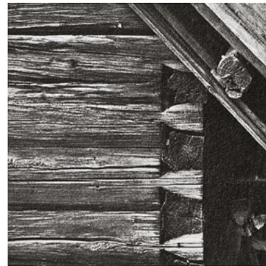
300 The pieces of end grain have been sprung off and so reveal the hidden cogs. – Molzegg, NE Austria
