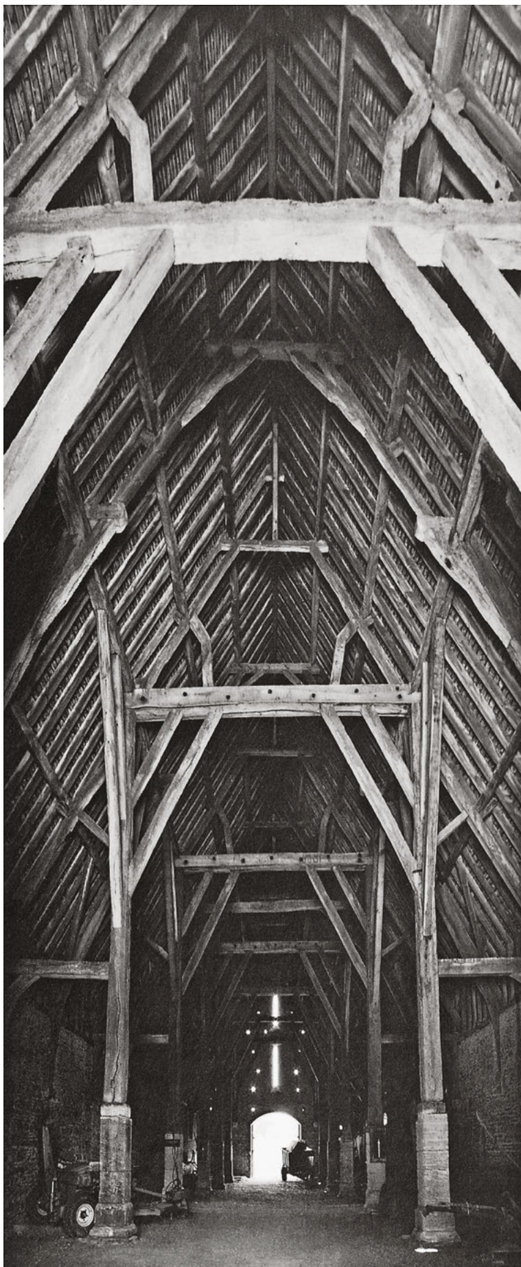
403 The enormous length of the spars (14 m) in the tithe barn at Great Coxwell, Oxfordshire, England, necessitated a well-thought-out support system. Secondary spars back up the principal spars. Besides the header beam of the reversed assembly there are a number of other purlin-like members which assist in bracing the spars longitudinally. Cruck frames support the header beams of the reversed assembly between the principal frames, with secondary spars (bearing on short hammer beams) again being used above the header.
