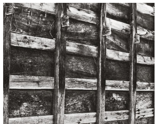
156 The panels between the column-and-beam skeleton of this barn in Shirakawa mura, Gifu, Japan, are filled with boards.
