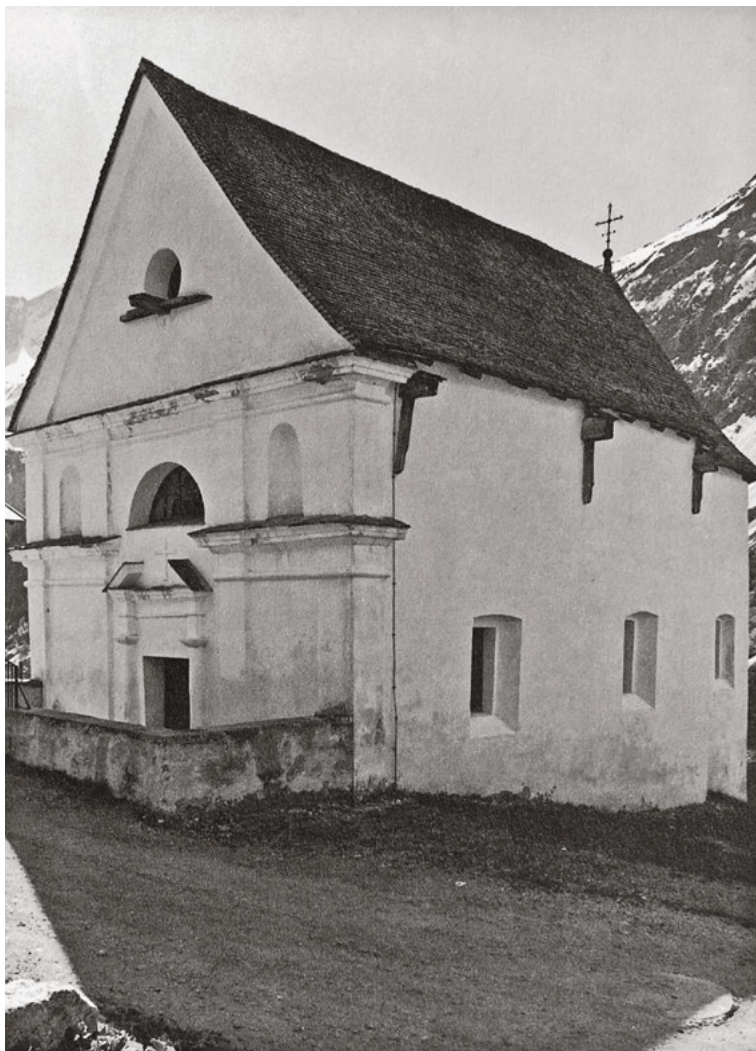
250 A stone wall secured with wooden anchors in Vinaders, Tyrol, Austria.
