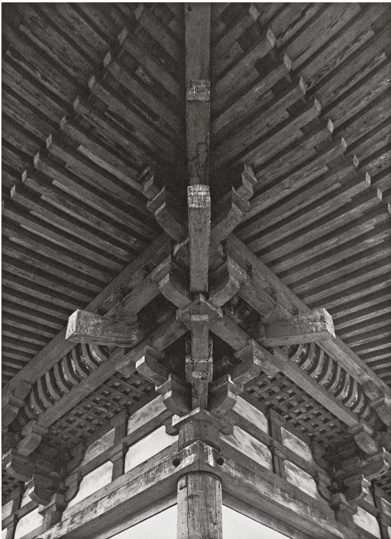
429 In the To-ji kodo, Kyoto, Japan, the still very basic bracketing is arranged exclusively above the columns.
