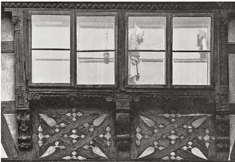
557 The plastered surfaces were only for show; they conceal flat panel infills. – Strasbourg, Alsace, France
