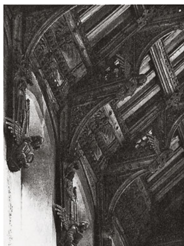
513 Detail of the hammer beam roof over the Church in Woolpit, Suffolk, England.
