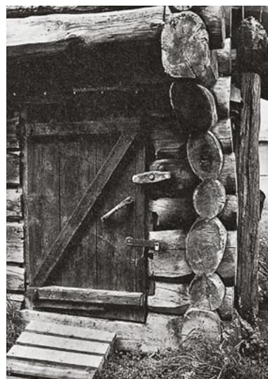
316 The owner of this farmstead near Vågåmo, Oppland, Norway, certainly believed it was worth the savings to provide the door as shown here instead of installing a proper framed opening!
