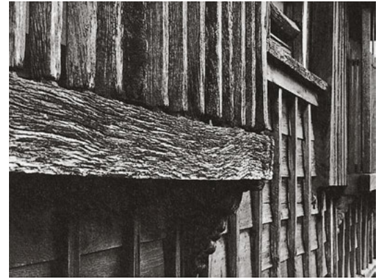
37 Left: The cleft shingles laid at a relatively flat pitch on the roof of the church in Inovce, Slovakia, will probably last considerably longer than the sawn vertical planks.
