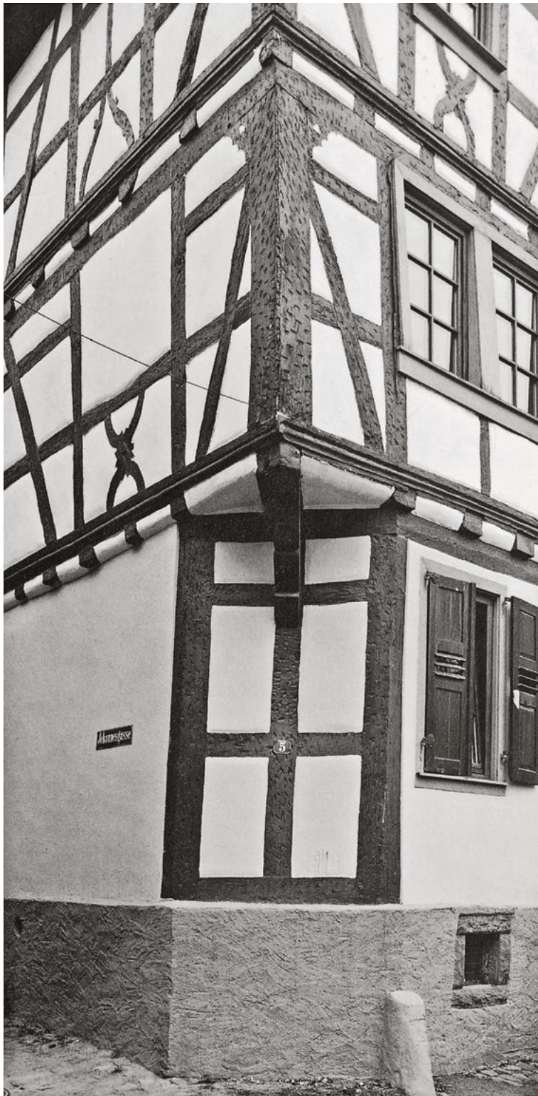
477 One corner which, apart from the ends of the beams, exhibits no exposed end grain. – Heppenheim, Bavaria, Germany
