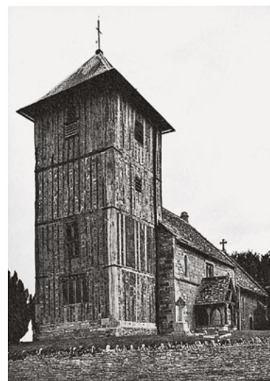
518 The panels between the columns are no wider than the columns themselves! – Upleadon, Gloucestershire, England
