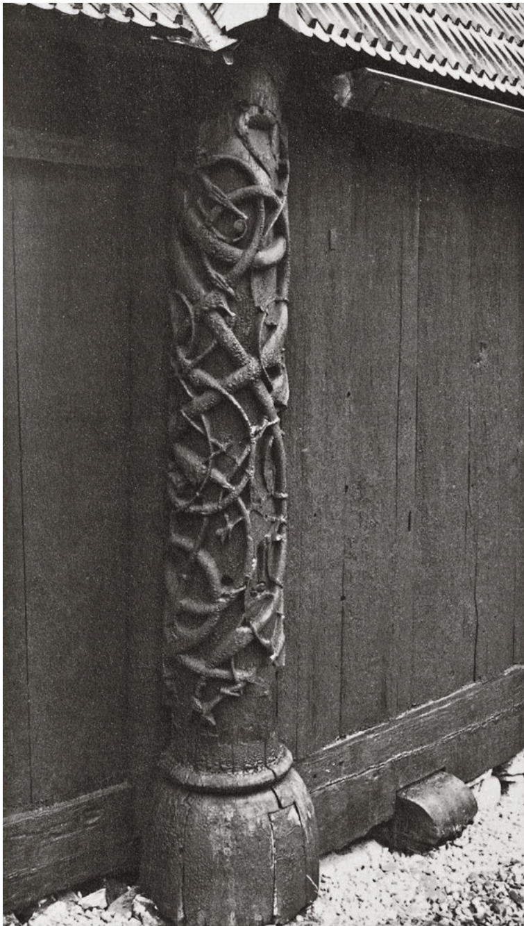
154 The stave wall of the church in Urnes, Sogn, Norway, is restrained by means of a wedging plank.
