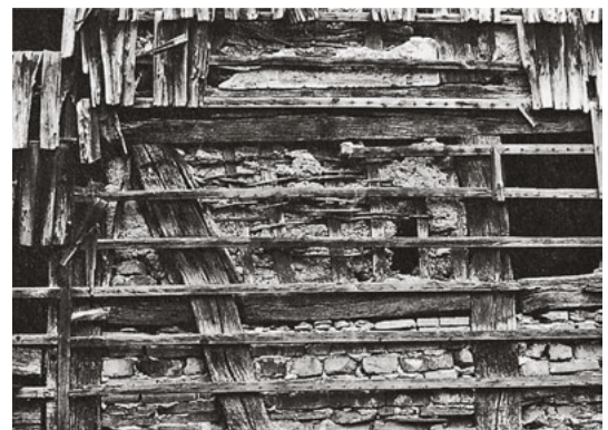
155 In the timber-frame construction of the towns, the wattle-and-daub filling was gradually replaced by stone and brick. This example from Michelstadt, Hessen, Germany, suggests that shingles were at one time cheaper than plaster.
