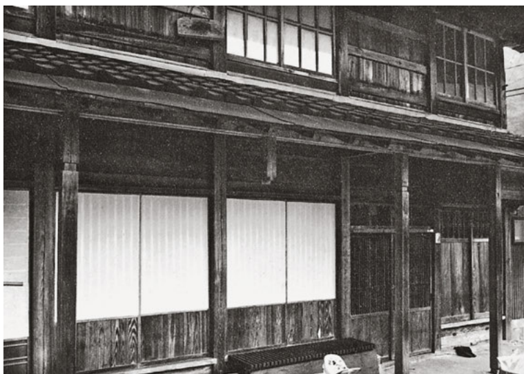
415 The dovetail clearly shows that the (now missing) rail was suspended. – Suganuma, Toyama, Japan
