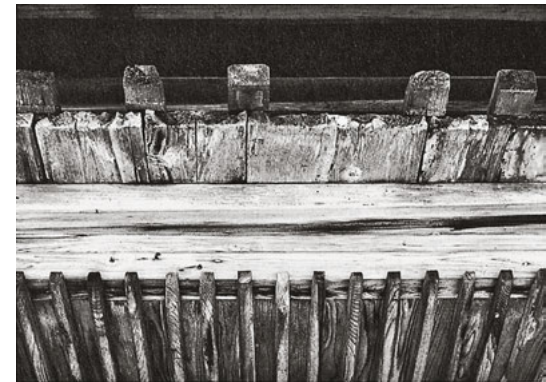
472 The roof covering to the Nyakuochi jinja, Hyogo, Japan, formally embodies the essence of the bamboo roof concept in timber.
