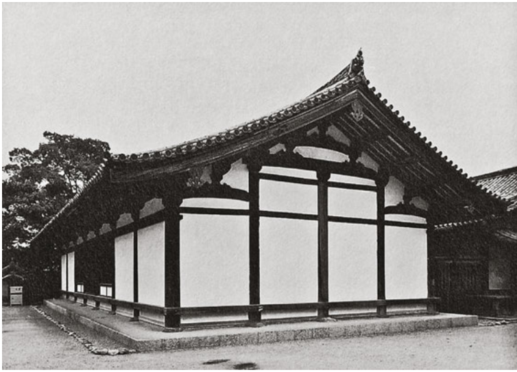
416 The very early construction of the Horyu-ji dempodo allows the division of the frame into moya and hisashi to be easily recognized.
