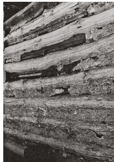
54 The variously filled gaps between the logs were subsequently coated with daub. – Log building in Šumiak, Slovakia.
