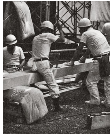
132 Carpenters fabricating a sill for a building in the Ise-jingu complex, Mie, Japan.
