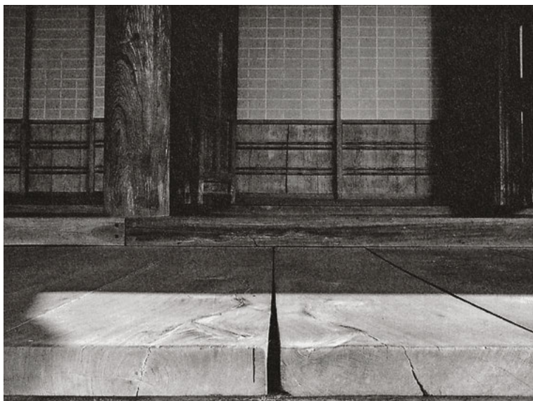
25 Even in planks, the nature of the cracks reveals how wood dries. – Entrance area of the Zuisen-ji hondo in Inami machi, Toyama, Japan.
