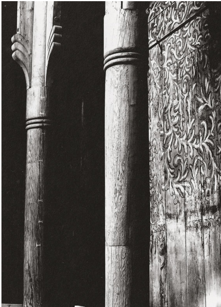
18 The new columns of the stave church in Heddal, Telemark, Norway, erected during its reconstruction in 1952, can be recognized by the up to 20-mm-wide crevices, next to which the fine cracks of the old columns remain almost invisible.
