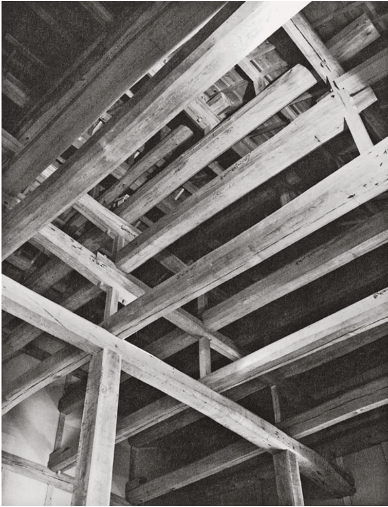
395 Moving down from the ridge, the number of supports must be increased from floor to floor in order to be able to carry the loads. – Kornhaus am Bauhof in Dinkelsbühl, Bavaria, Germany
