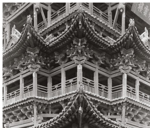
613 Eaves detail of the Dongyue miao Feiyun lou in Wanrong, Shanxi.
