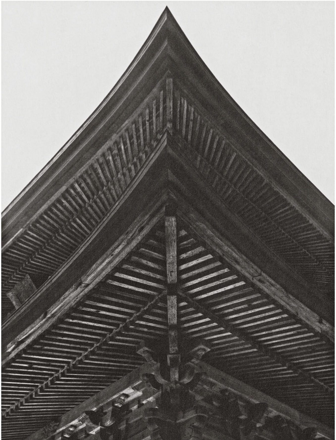
445 The rafters laid parallel cover the mokoshi area, the radial ones the moya . – Engaku-ji in Kamakura, Kanagawa, Japan
