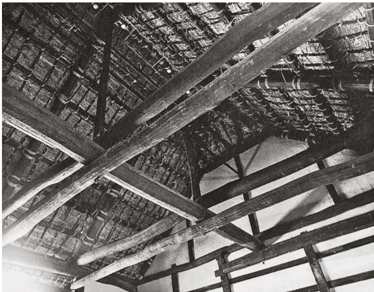
390 The shinzuka-gumi roof is normally thatched but is also encountered with tiles or shingles. The tie beams are doubled to cope with the very wide span of this minka in Kitakata, Fukushima, Japan.
