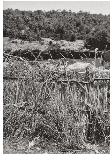
217 This temporary sheep fold near Xanthi, Macedonia, Greece, was fenced off using loose brushwood and reeds simply placed in a row.
