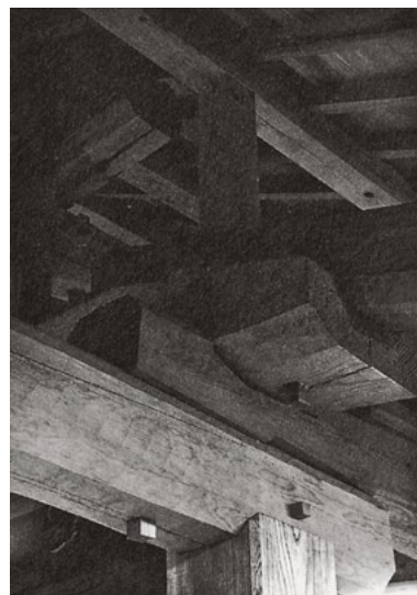
133 Traditional timber construction is easily discernible on the newly built Kyuhonjin kinenkan in Hirata, Shimane, Japan.
