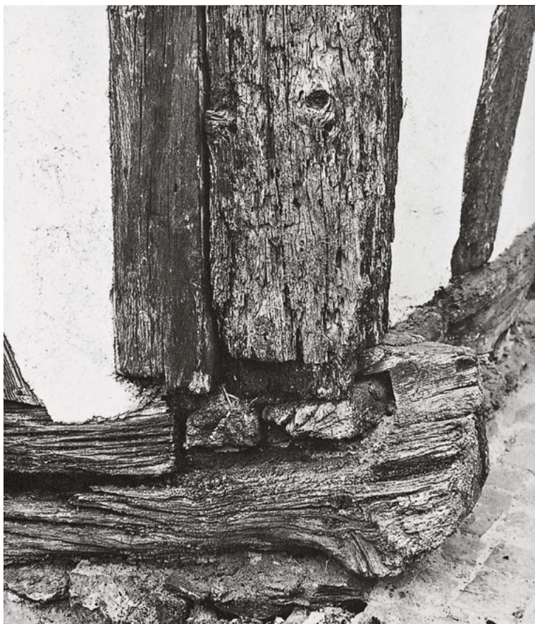
455 Far less effective was the tenon in the column's end grain which only engaged with one sill beam. – Niederneunforn, Thurgau, Switzerland
