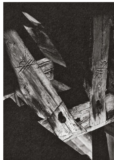
117 A carpenter’s mark as an aid to assembly in the roof truss of the monastery church in Neuberg an der Mürz, Steiermark, Austria.
