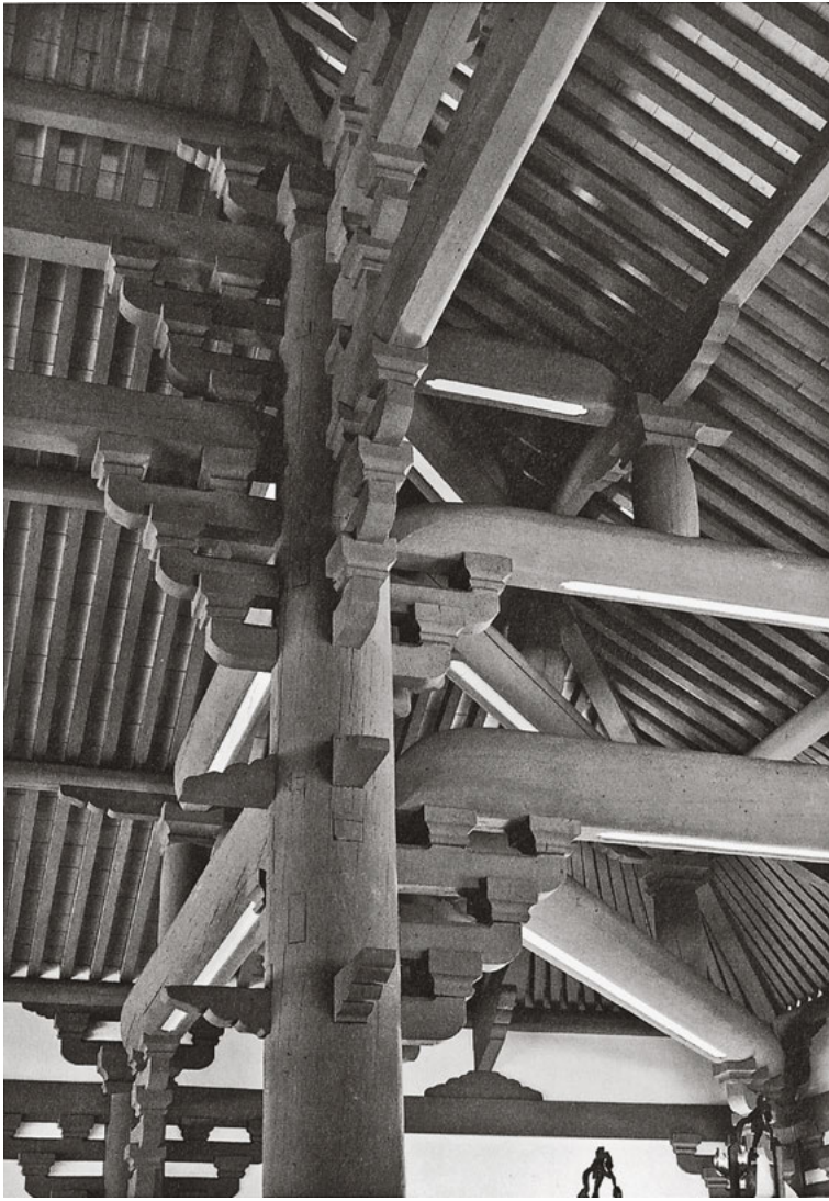
437 The exposed roof construction of the Jodo-ji jododo, Hyogo, Japan.
