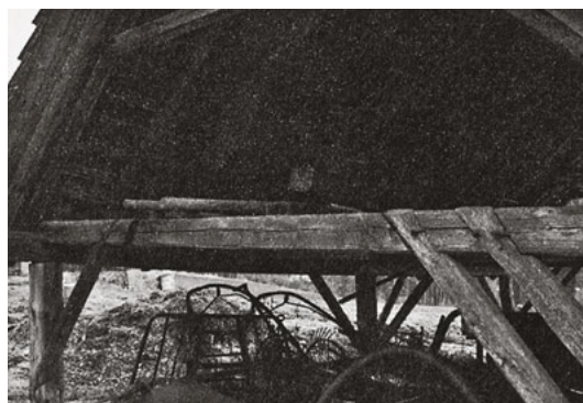
243 In the transition to nailing of the lap in its housing, the first change was the replacement of the jointing wedge by the jointing nail. – Sagrad, Carinthia, Austria
