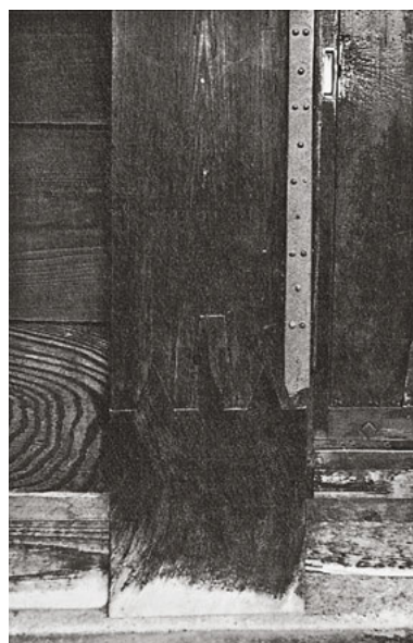
567 Transferring the functional parts of a joint to the inside was in no way abandoned with the coming of the exclusively decorative features on the surface. – Sumiya, Kyoto
