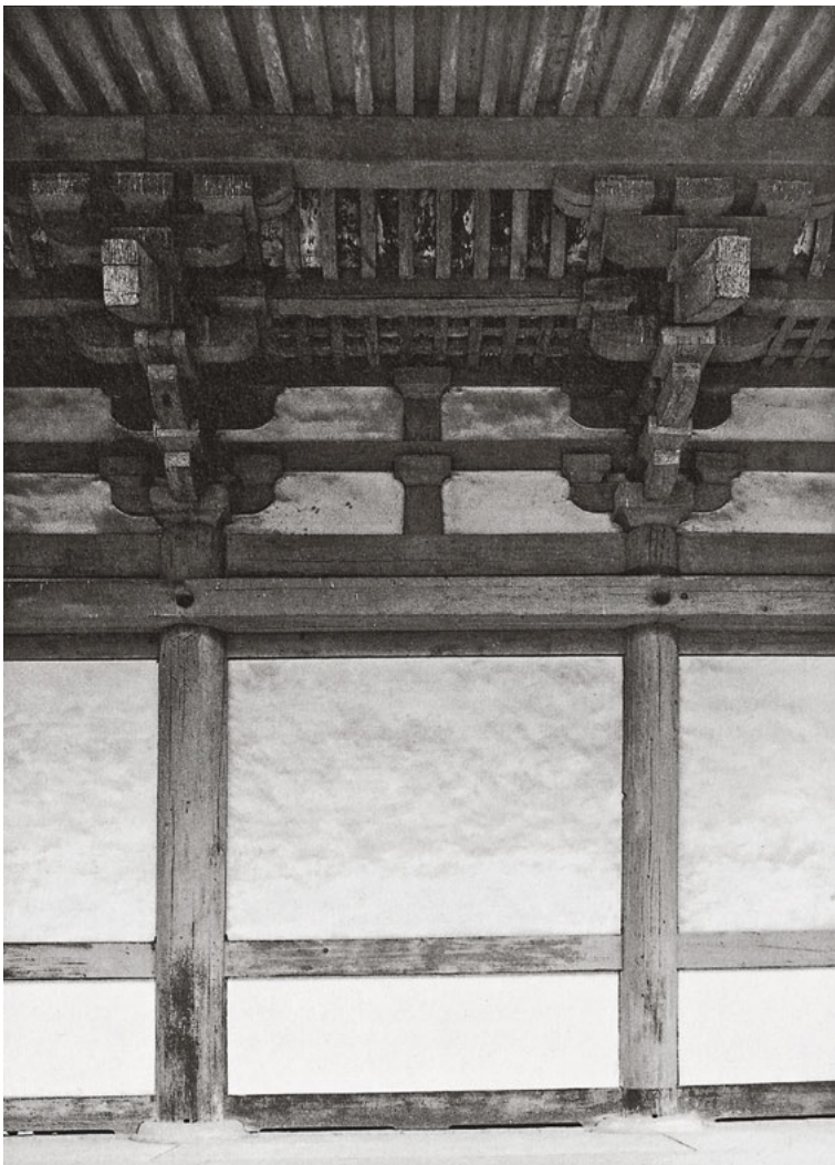
33 The bases of the columns of the To-ji kodo, Kyoto, Japan, all have ventilation slots.
