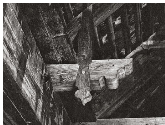
119 When a dovetail is cut so accurately as here in this suspended interrupted tie-beam on the Kubel bridge, Appenzell, Switzerland, its form also fulfils sober expectations.
