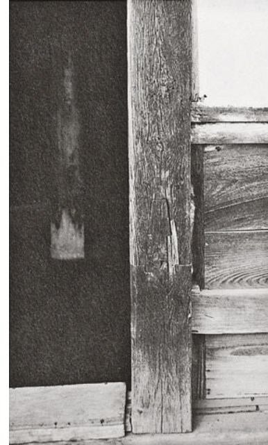
461 The most diverse well-known splicing joints were employed. – Sasaki House from Nagano in the Nihon minka en
