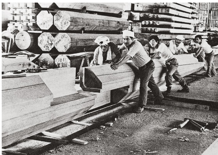
498 Assembling two pieces of the central column of the re-erected Yakushi-ji Pagoda, Nara, Japan. (photo: Teraoka, Fusao; in: Nishioka et al., Soshisya, 1981)
