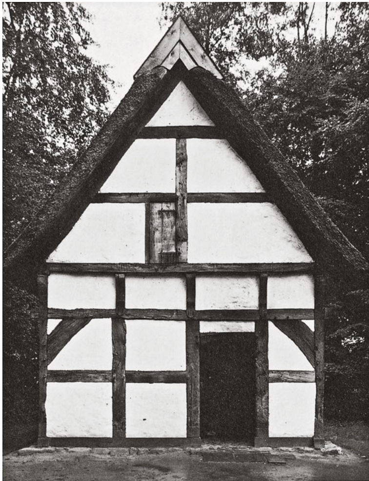
350 The kneebraces reveal the location of the anchor beam essential to the construction; furthermore, we can see that a raised-header assembly has been employed. – Bakery from Astrup, Lower Saxony, Germany, in Cloppenburg Open-air Museum.
