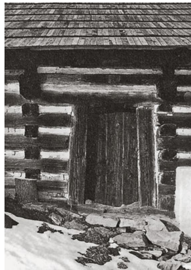
315 Belt and braces! Despite the adjoining intermediate walls, the builder still included door jambs! – Sâdek, Czech Republic
