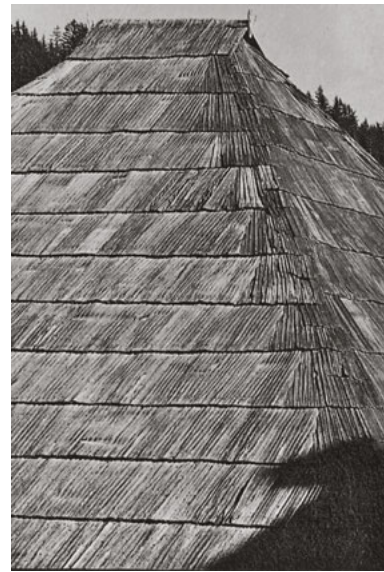
110 With cleft shingles there is absolutely no waste because they are not even given a groove. When laid properly, every branch inclusion, every bow can be followed in the surface of the roof. – Greschitz, Carinthia, Austria
