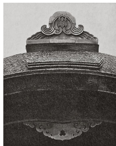
123 The bargeboards converging in the centre of the gable meet almost perfectly. – Rinshun kaku, Wakayama, in the Sankei-en, Yokohama, Japan.
