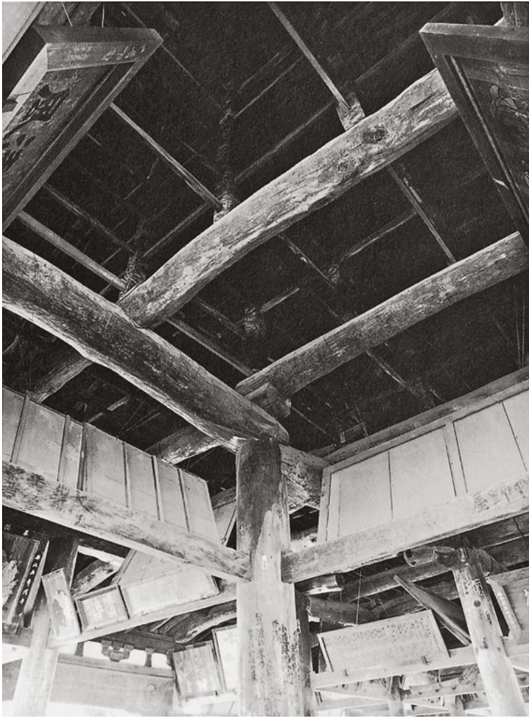
392 A wagoya-gumi (Japanese roof) over the Senyo kaku in Miyajima, Hiroshima, Japan.
