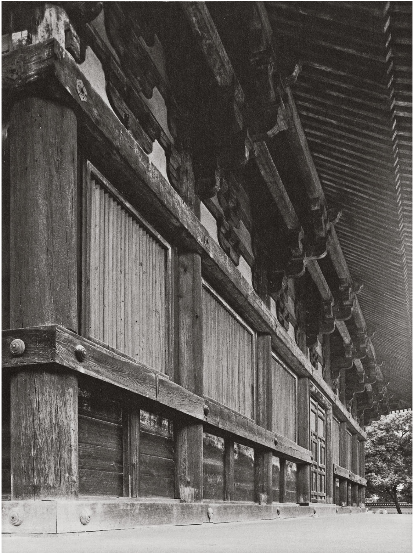
36 On the To-ji kondo, Kyoto, Japan, the sill, rail and header are all covered in such a way that no end grain remains exposed to the weather.
