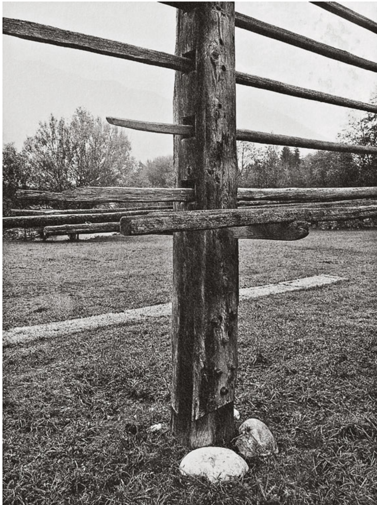
459 If the recesses cut for the column tenons had been formed with a slope from centre to edge, then the water really could have drained off!
