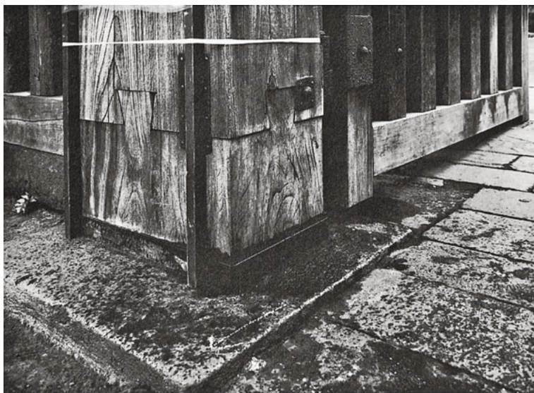
570 Shiho-ari joint on the gateway to the Honmon-ji in Tokyo, Japan.
