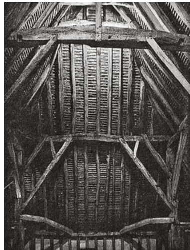
519 The lower up brace was so long that it itself was braced top and bottom. – Barley barn in Cressing Temple, Essex, England
