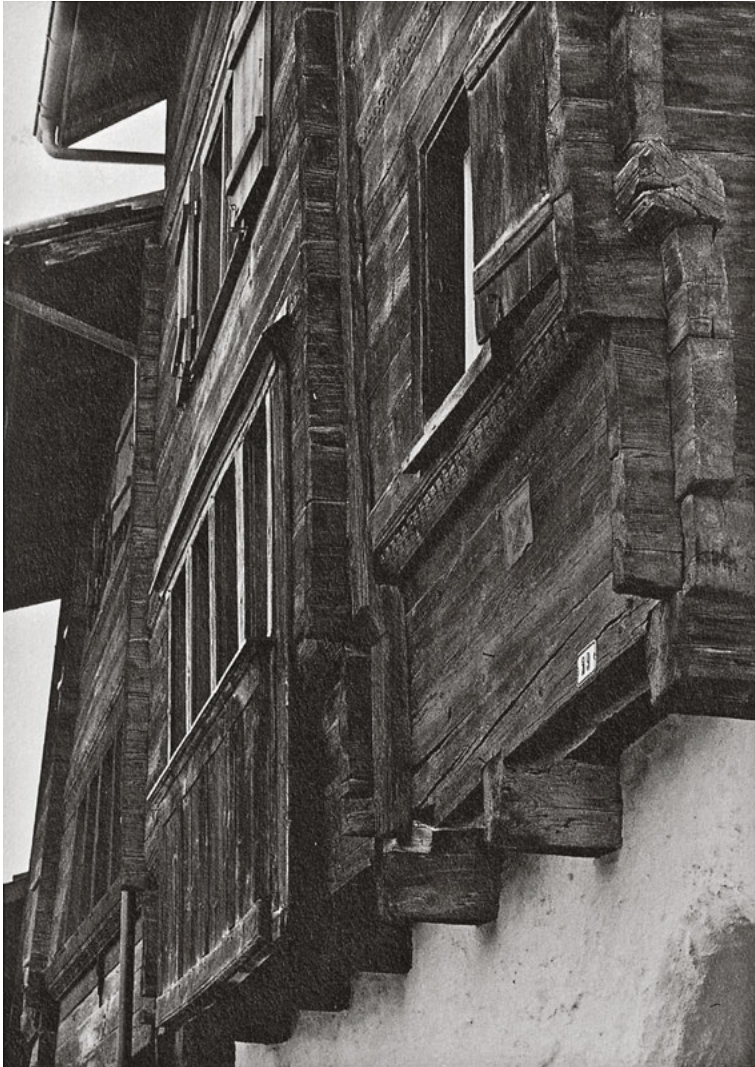
322 To highlight the wall divisions by means of the carved spandrel beneath the windows, the spandrel cantilevers by the width of the member. – Werdenberg, St Gallen, Switzerland
