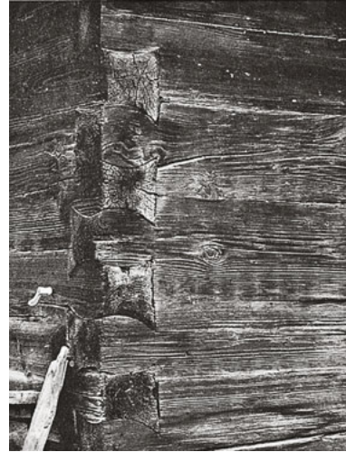
264 The production of curved joint interfaces required a tool which allowed more accurate working than was possible with the hatchet and more effective than the chisel. – Westendorf, Tyrol, Austria
