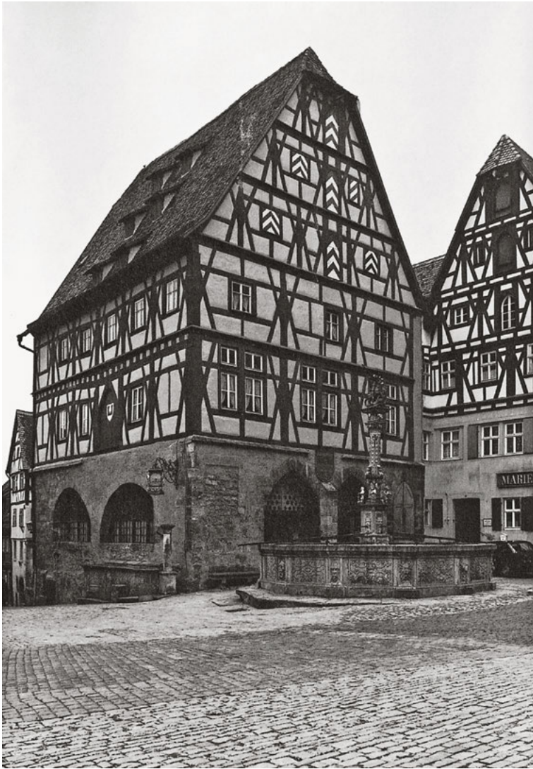
385 We can see from the gable end that the roof space was utilized right up to the ridge. – Rothenburg, Bavaria, Germany
