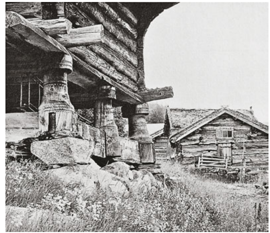
475 Raising European buildings on stilts or staddles may also have been carried out to help with ventilation. The main reason, however, was to protect the stored goods from animals. – Gudbrandsgard, Buskerud, Norway
