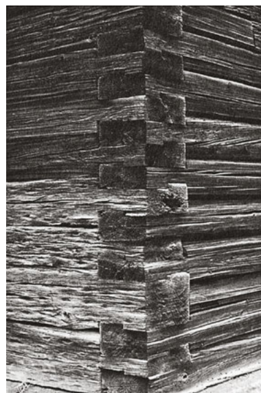
295 Shaped, notched and tabled pectination was used to join the logs of the church in Loučná Hora, Czech Republic.
