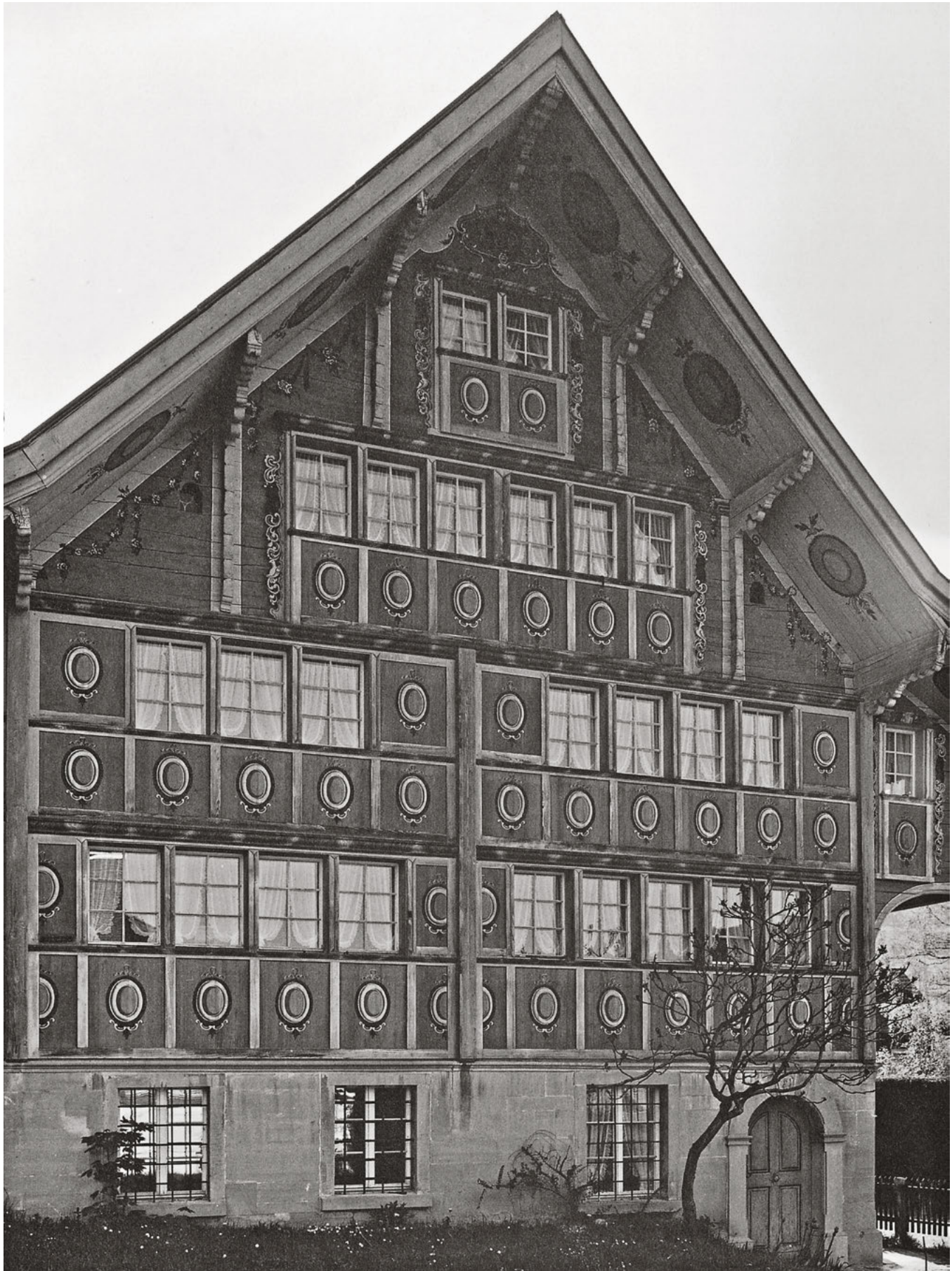
381 If the rafters deflected excessively – due to a long span from eaves to ridge or heavy roof loads –, then intermediate purlins were inserted. – Grub, Appenzell, Switzerland
