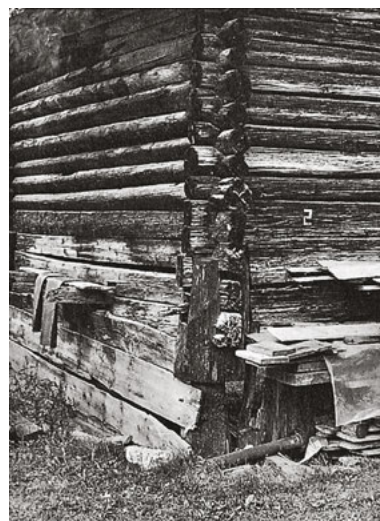
277 The form of stilt used on this storehouse from Längenfeld, Tyrol, Austria, makes it resistant to bending.
