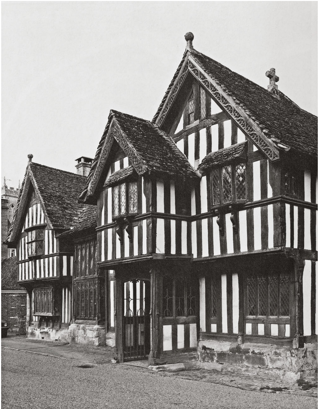
353 The jowl of the column head suggests a rigid joint between the incoming members and hence the reliable stability of the structure. – Potterne, Wiltshire, England
