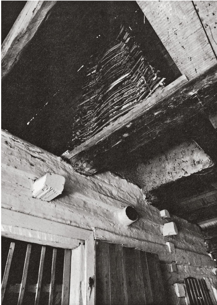
229 Wattle-and-daub infill panels on a minka in Iwate Futsukamachi, Iwate, Japan.
