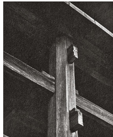
527 Above the column of the kakezukuri construction the viewer is only aware of the line of the seam of the joint between two beams. – Ishiyama-dera hondo, Shiga, Japan
