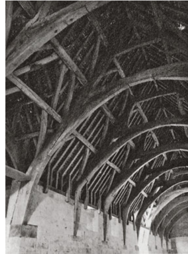
107 Another variation: at the fixing point of the lower collar beam the two roof slope timbers are pieced together in such a way that only a very detailed inspection reveals the join.
