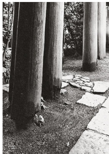
29 Wood suffers most damage at the air-ground transition, as shown by these torii in the Zeniarai benten in Kamakura, Kanagawa, Japan.
