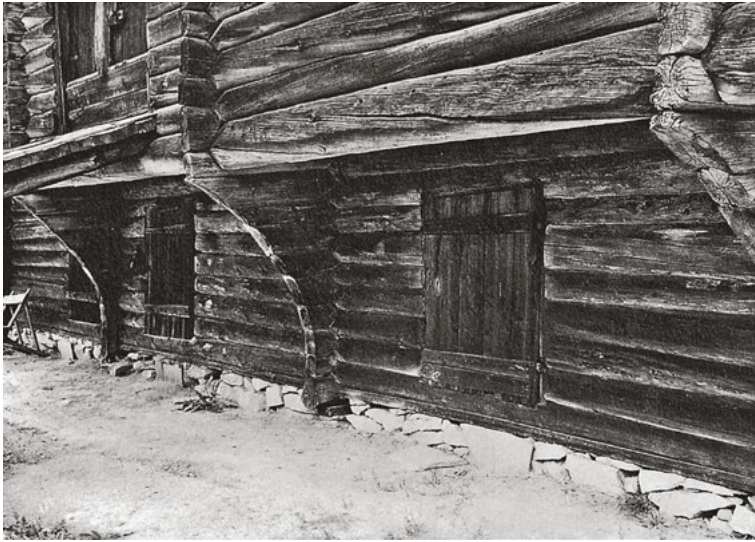
321 Brackets are easily incorporated in log construction. – Bygdøy Open-air Museum, Oslo, Norway
