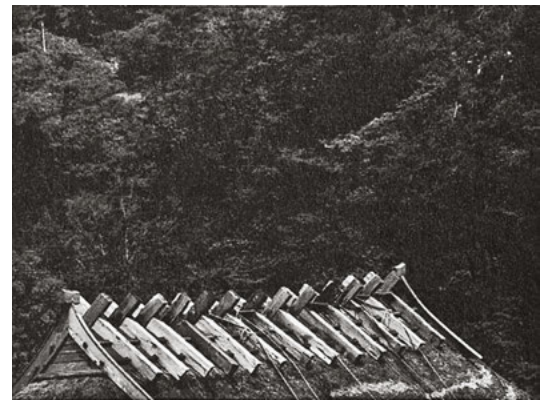
189 The crossovers formed by these simple lapped joints both secure and decorate the ridge covering of this minka in Tamugimata, Yamagata, Japan.
