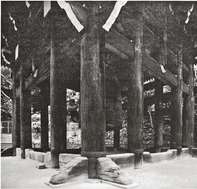
281 Column-and-beam construction under the Chion-in bell-tower, Kyoto, Japan.
