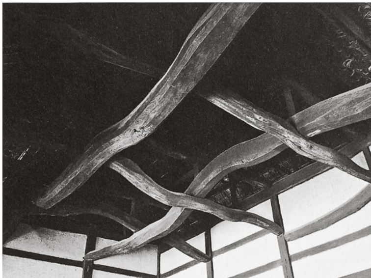
13 Beams in Sakuta House, Chiba, Japan, in the Nihon minka en.
