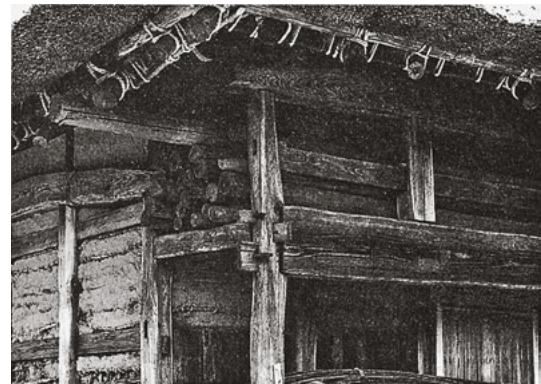
253 On prestige buildings joints such as this one on a minka in Iwate Futsukamachi, Iwate, Japan, would only be allowed in non-exposed positions.
