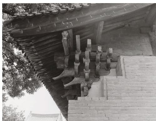
604 Only the dougong in the Tian Wang dian of the Zhenguo si in Pingyao, Shanxi, project out of the walled masonry enclosing the loadbearing columns. The temple was built during the Period of Five Dynasties.
