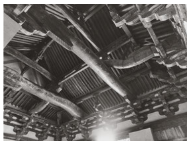
652 The small Youxian si temple in Gaoping uses beams with irregular dimensions and forms that must have presented the carpenters with a challenge. Noteworthy is the unconventional extension of the intermediate dougong in the central axis, which display a remarkable economy of means.
