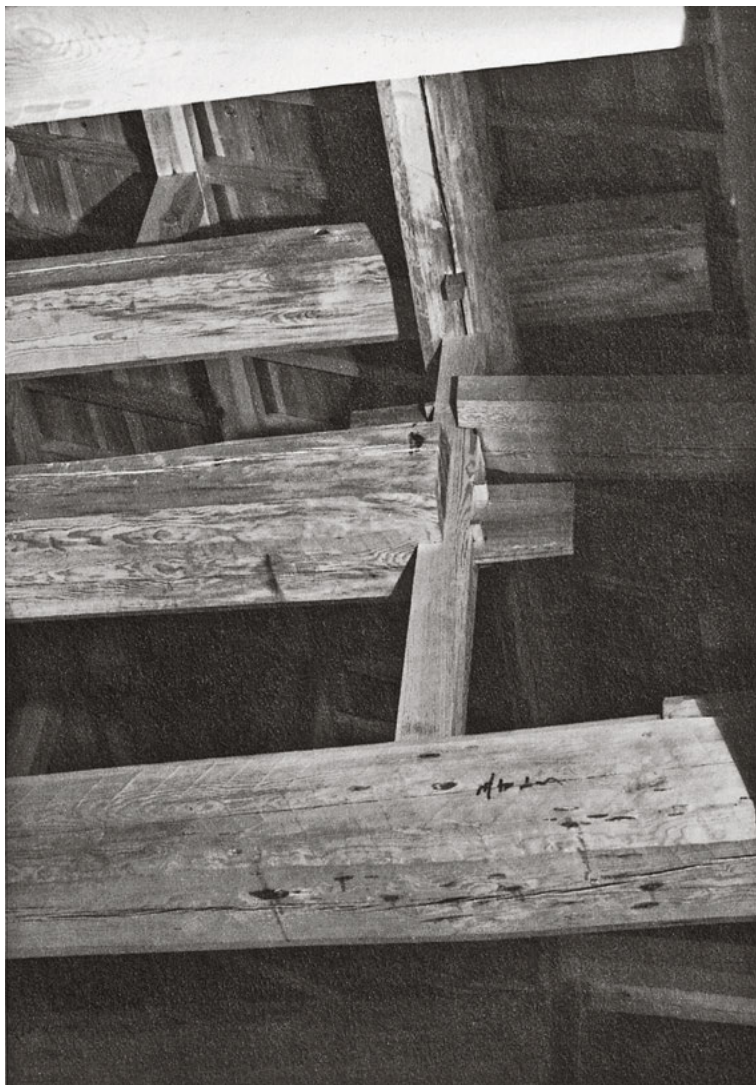
211 In the Todai-ji nandaimon, Nara, Japan, the solution in 1199 was to treat each member equally, all parts being weakened in the same way. (according to: Zairai koho no kenkyu , 1993, Fig. 4-40-7)
