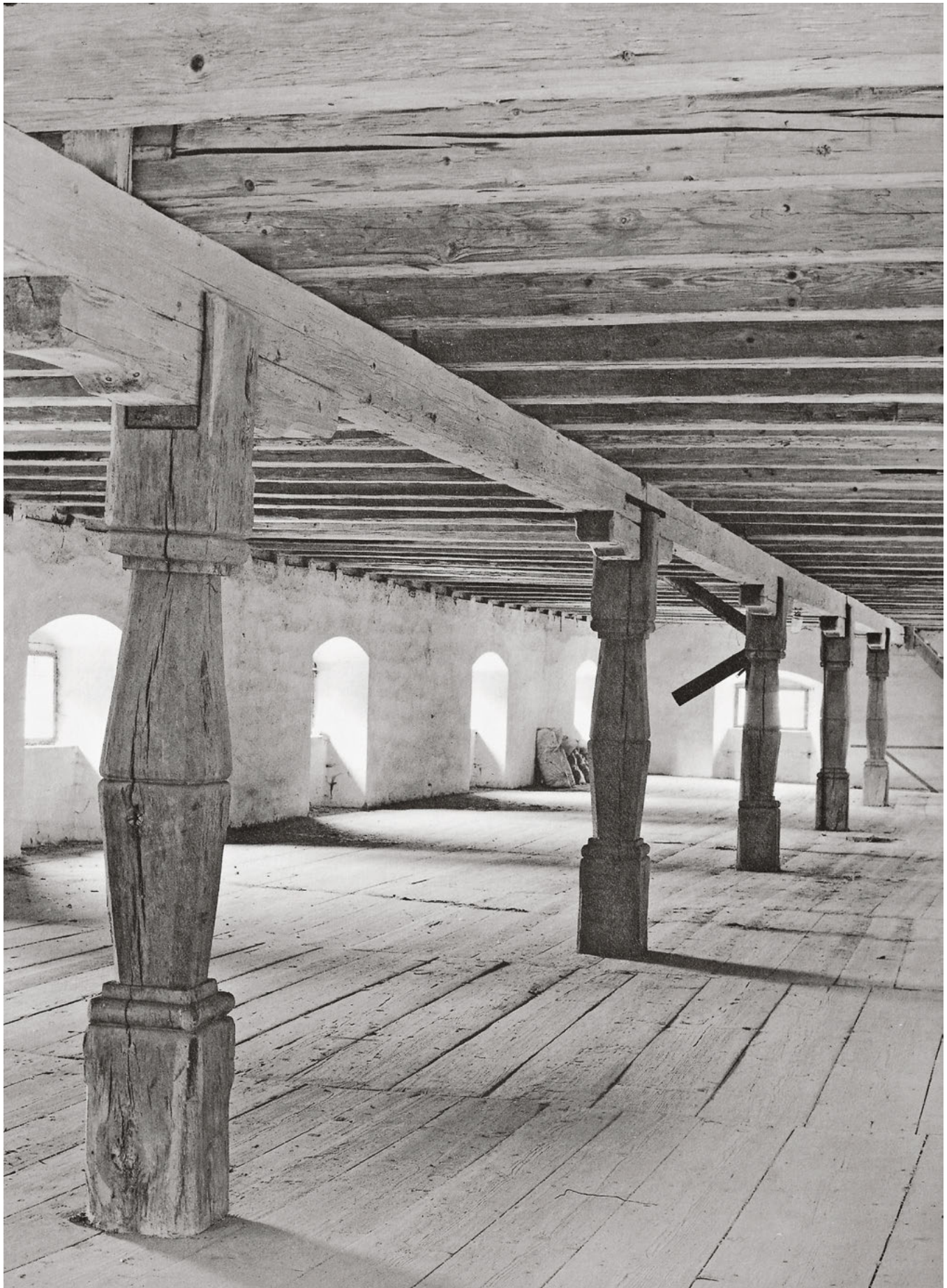
7 Granary beam supported on columns. – Primmersdorf, NE Austria.
