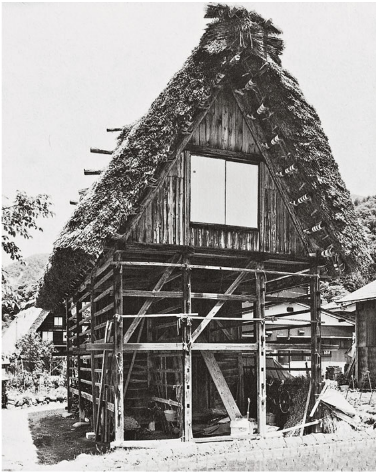
388 This roof has been specially designed for thatching. – Barn in Shirakawa mura, Gifu, Japan
