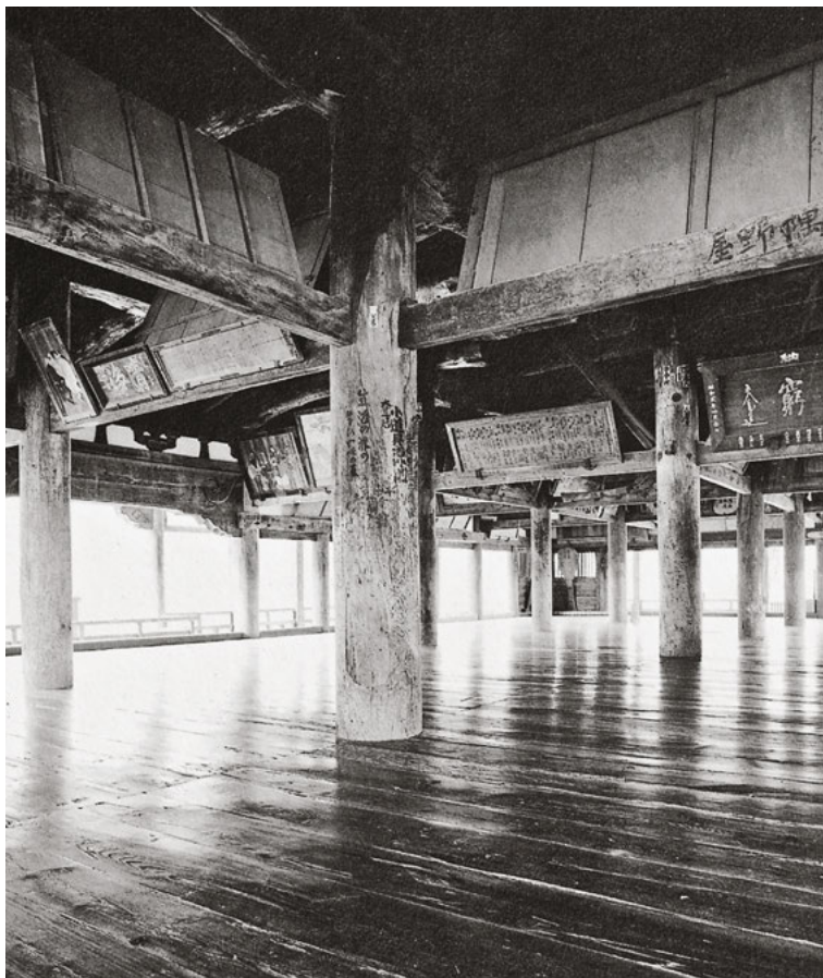
8 The roof in the Senyo-kaku in Miyajima, Hiroshima, Japan, is supported by columns arranged on a grid.
