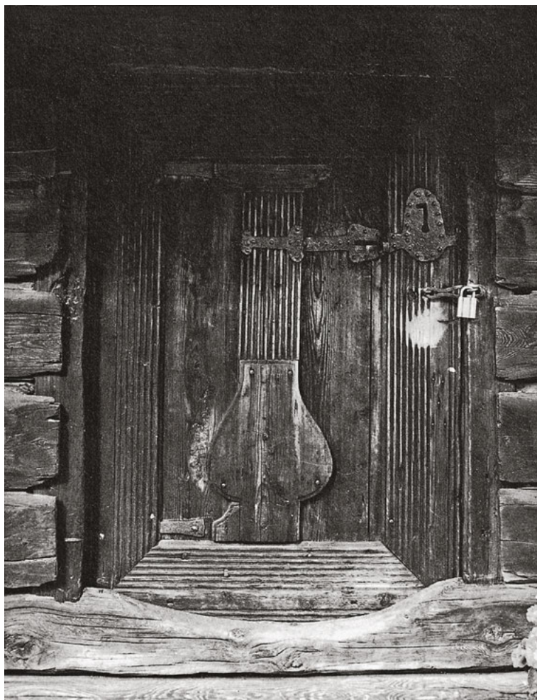
316 The owner of this farmstead near Vågåmo, Oppland, Norway, certainly believed it was worth the savings to provide the door as shown here instead of installing a proper framed opening!
