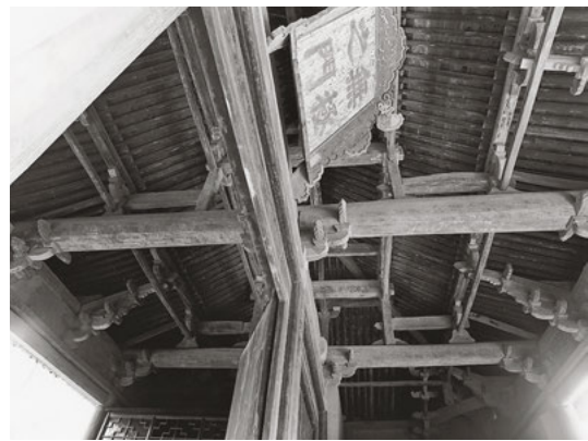
654 Many details of the roof construction of the Longhuan gateway building to the Yongle gong exhibit an increasing tendency towards more slender cross-sections.
