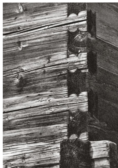
120 Corner of a log building in double Klingschrot. – Hasleiten, NE Austria.
