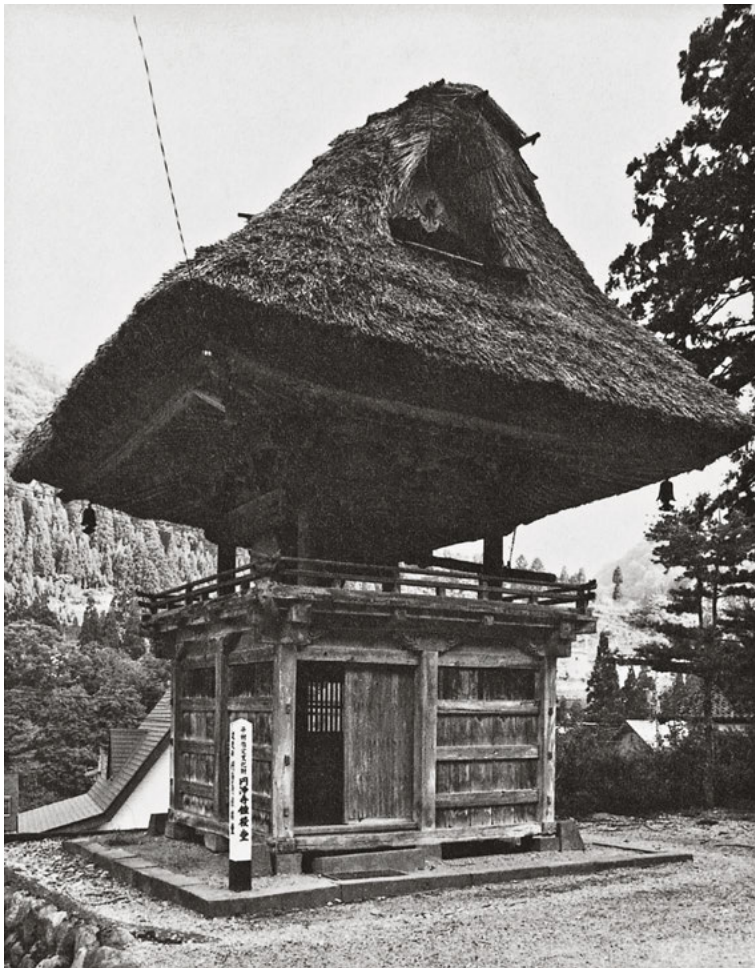
419 The pitch of the roof on the outside is different to that on the inside. – Enjo-ji shoro tou in Kaminashi, Toyama, Japan
