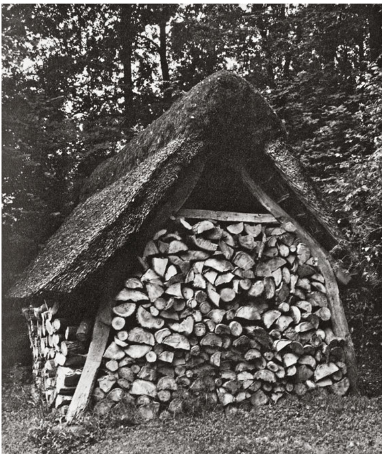
105 Covered firewood store in Cloppenburg Open-air Museum utilizing the cruck or A-frame type of construction.
