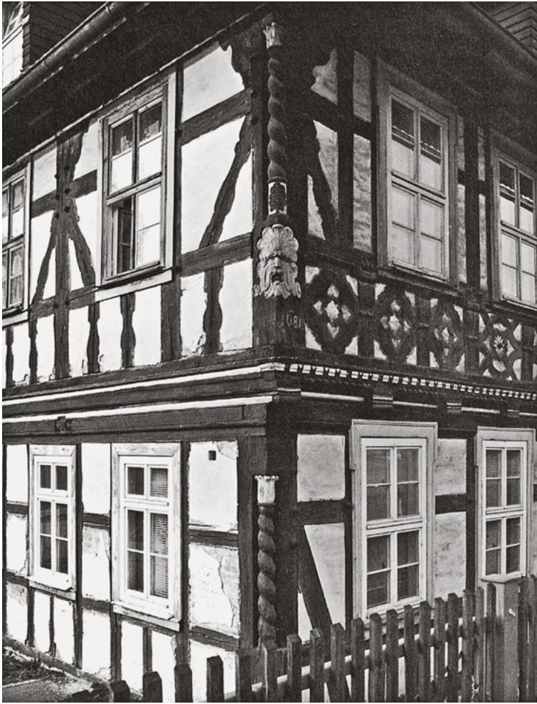
374 The jettying of the upper storey hardly casts a shadow here. – Schleusingen, Thuringia, Germany
