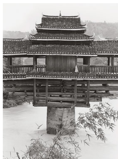
632 Bridge pier of a cantilevered bridge in Zhengyang, Guangxi.
