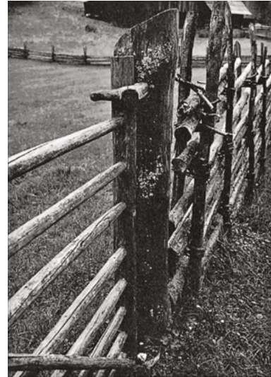
87 The fixing of a gate to a wooden fence. – Stübing Open-air Museum, Austria
