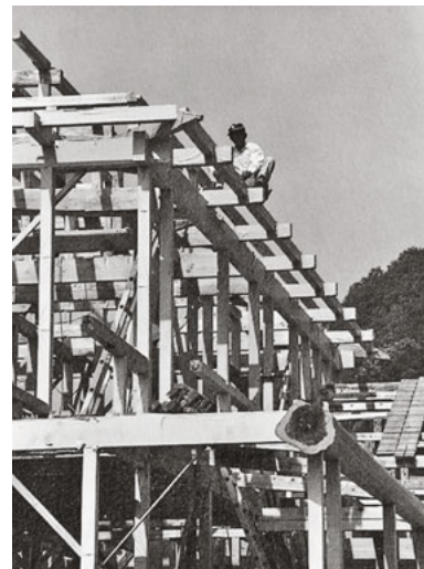
99 The construction of a new building in Kibitsu, Okayama, Japan, making use of traditional construction. The timbers remain wrapped in protective paper for as long as possible.
