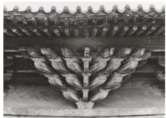
645 An intermediate dougong of the Shanhua si in Datong, Shanxi.
