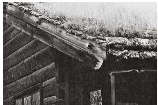
71 Birch bark forming the insulation layer beneath the sods of grass on the roof. – Maihaugen Open-air Museum in Lillehammer, Oppland, Norway.
