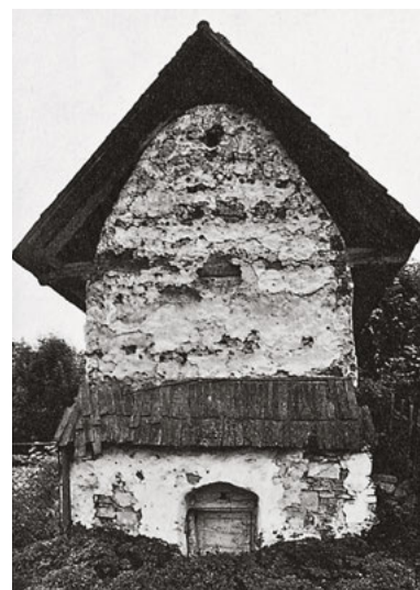
274 The fire-resistant daub shell of this storehouse from Petrov, Slovakia, is a visible expression of the value of the building’s contents or rather the fear of losing them.
