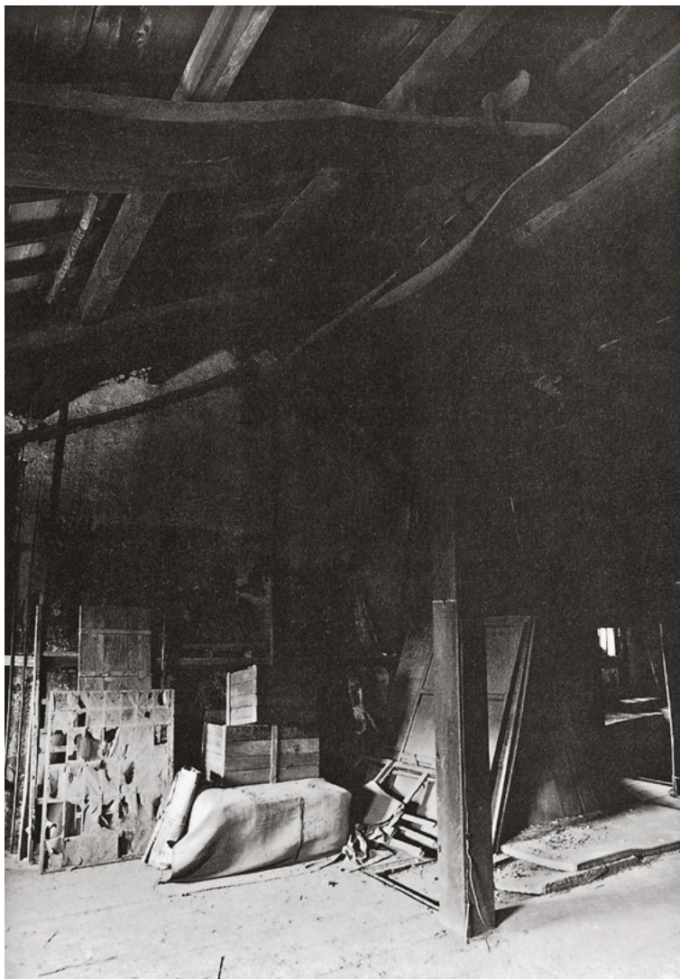
398 In warehouses it seemed obvious to include a row of king struts passing through every floor for additional support. – Primmersdorf, NE Austria
