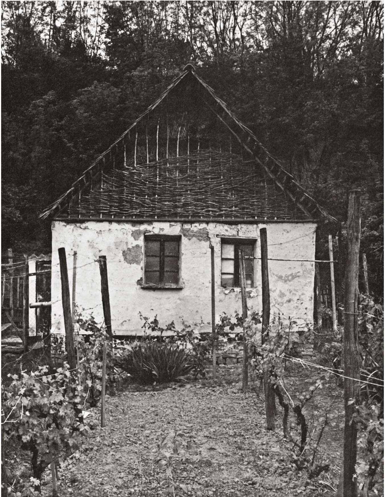
225 The wattle gable is the last surviving reminder of the wattle house. – Dunaszekcső, Hungary
