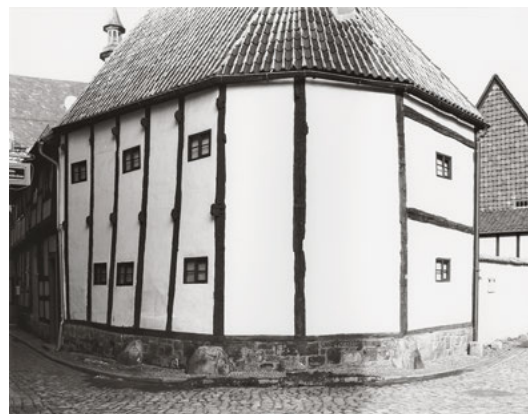
355 Nails or wedges are required to prevent through-tenons from coming apart. – Quedlinburg/Saxony-Anhalt, Germany
