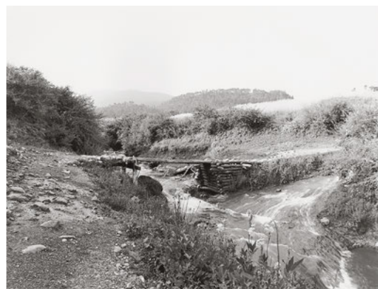
631 Layered logs form a primitive but resilient form for a bridge pier. Lijiazui, Sichuan
