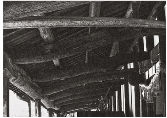
417 The eaves of the Kikunoyo Brewery in Meiji mura illustrate the principle. Underneath, the visible rafters ( kesho taruki ) at an angle corresponding to the ideal of beauty; above, the hidden notaruki carry the roof covering.
