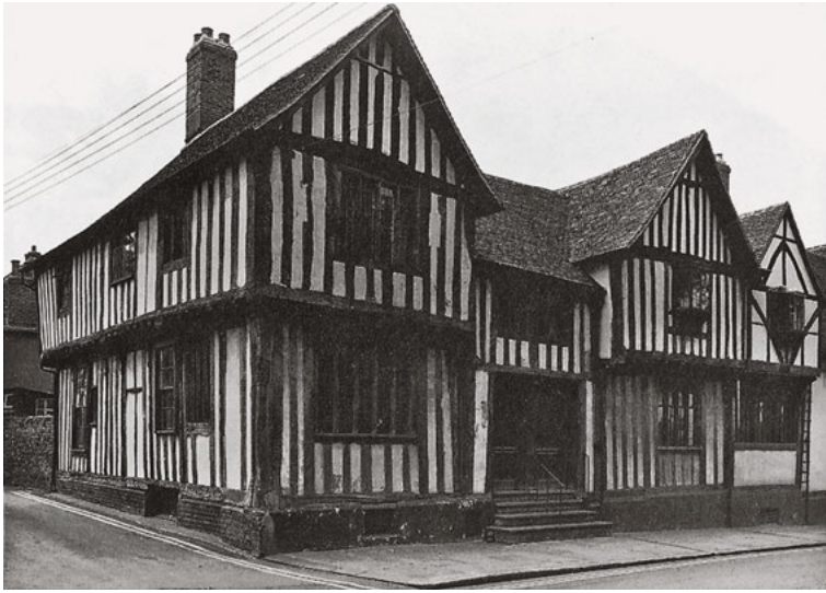
386 The spar triangle forms a rigid construction. – Sudbury, Suffolk, England
