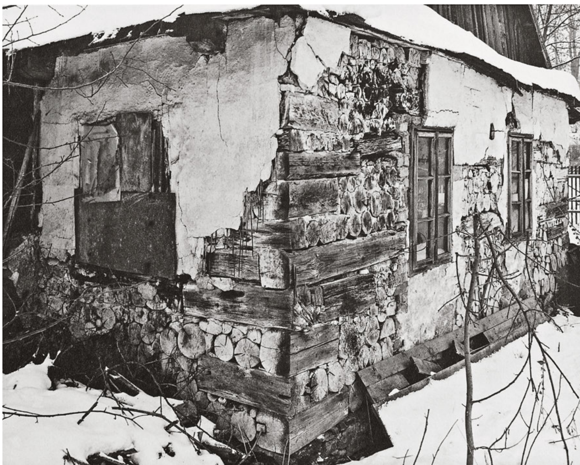
493 The short Holzschelte (billets of wood) used to build the walls led to such houses being called Scheitholzhäuser . – Vitanov, Slovakia
