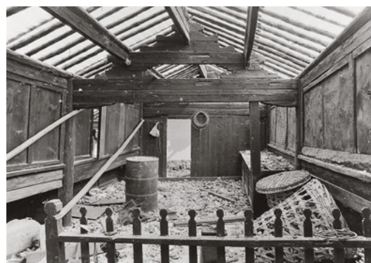
601 The roof construction of this old house in Baisha San Yuan Cun, Yunnan, here without roof covering, shows the care that has gone into shaping the ends of the beams that give the roof its form.
