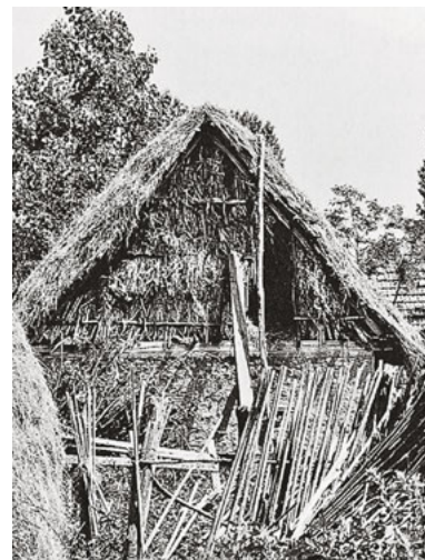
489 This house near Cicirlău, Maramureș, Romania, is still wholly in wattlework. The walls are covered with daub.
