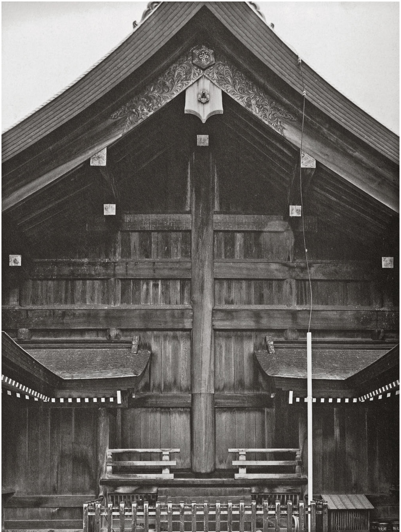
383 Larger columns meant less of them but still had to divide up the area below the roof according to the needs of the layout. – Izumo taisha, Shimane, Japan
