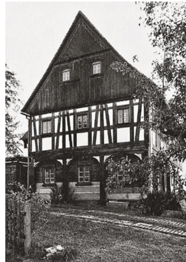
488 Relieving columns (which exploit the considerably greater compressive strength of the material parallel with the grain) were placed in front of the ground-floor log construction in order to carry the load of the roof or even an upper storey. – Jonsdorf, Saxony, Germany
