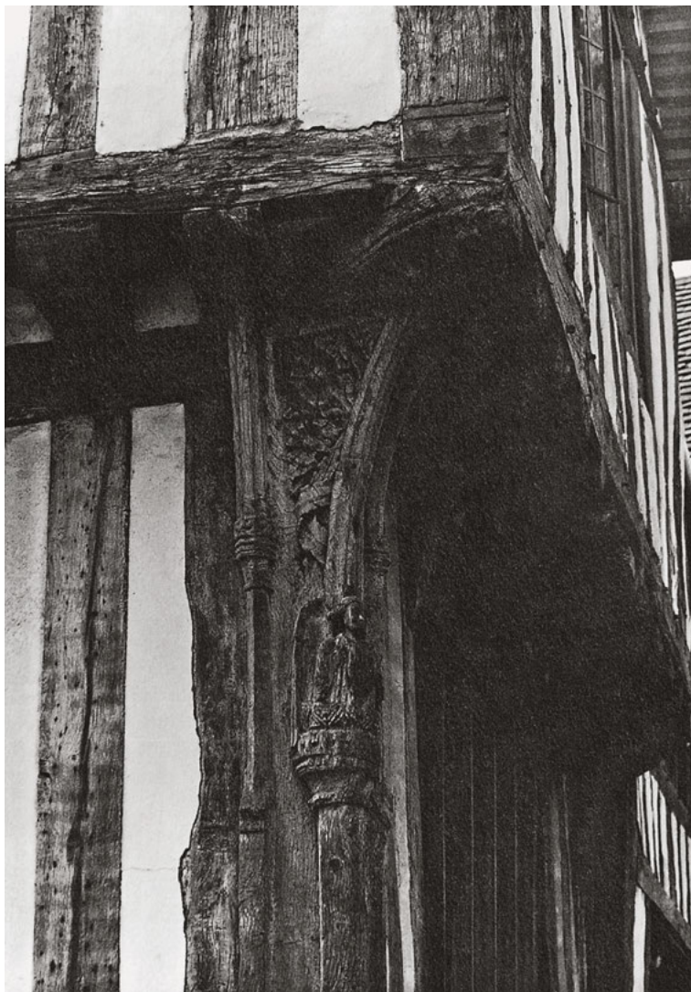
372 This naturally grown corner column was emphasized through carving and the observer was made aware of its function just like Phleps wished to see in the German examples. (Phleps, 1967, p. 137 ff.) – The Chantry, Sudbury, Suffolk, England
