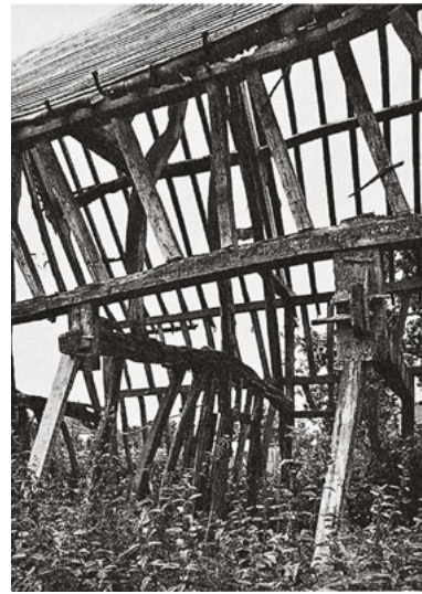
249 Anchor beams defined the room divisions and also served to carry the roof construction. – Bouttoncourt, Normandy, France
