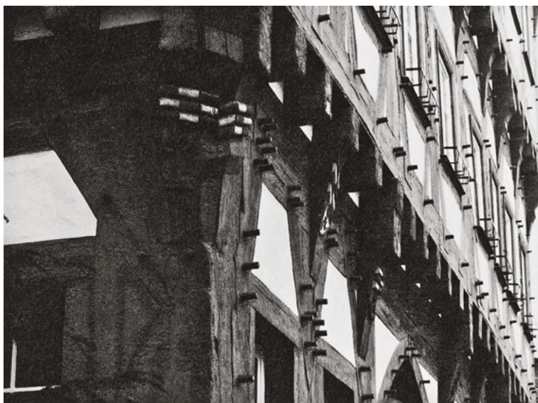
241 Wooden nails secure the lap joints on the town hall in Markgröningen, Baden-Württemberg, Germany.
