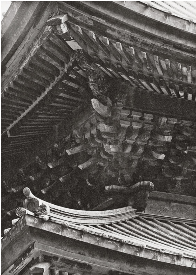
444 Eaves corner – Kencho-ji butsuden in Kamakura, Kanagawa, Japan
