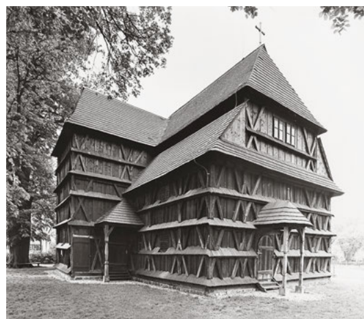
41 Miniature roofs protect the sill and all horizontal rails of the church in Hronsek, Slovakia.
