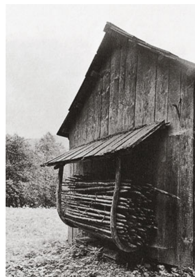
12 These bowed timbers enable a design clear of the ground in the virtually always damp Salzkammergut region. – Gössl, Steiermark, Austria.
