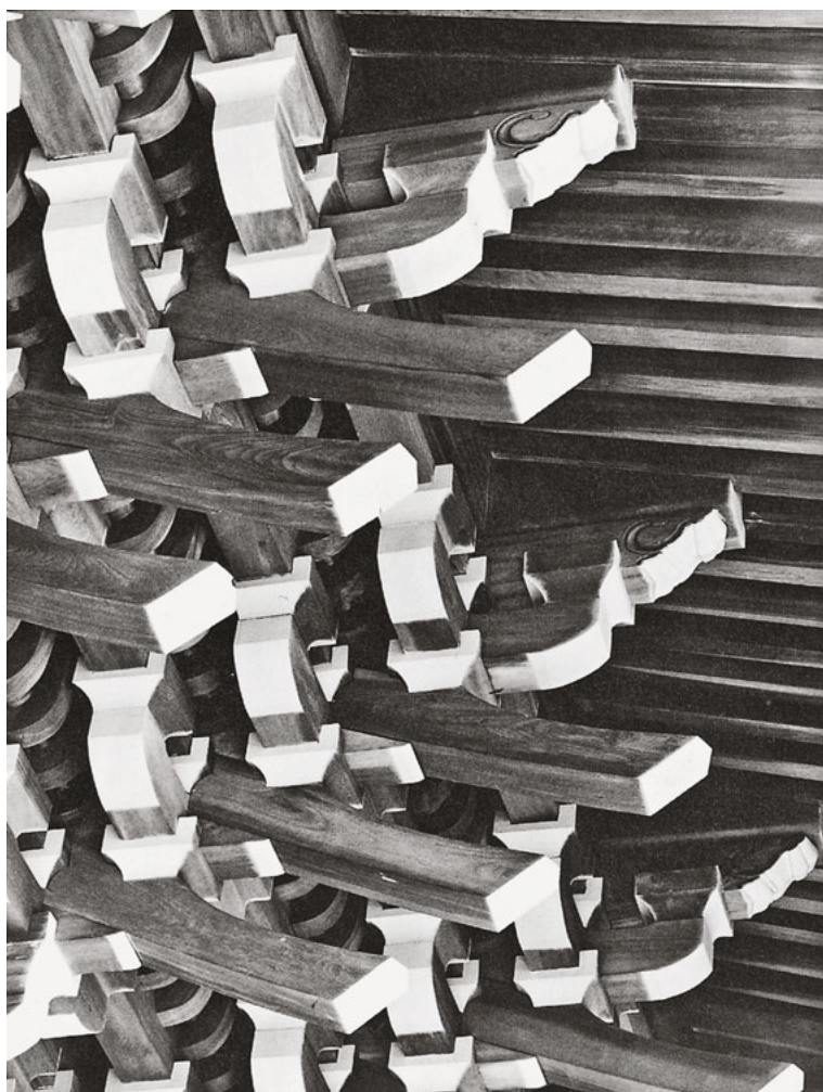
441 The bracket complexes so typical of the zenshuyo . – Zuisen-ji taishido, Toyama, Japan
