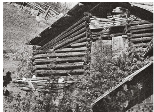
53 "Airy" timberwork on a barn in Köfels, Tyrol, Austria.
