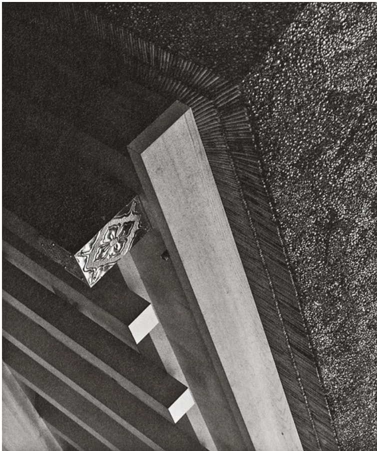
526 Two staggered layers of straw form the eaves termination. Piece by piece each straw is placed in a sleeve closed at the front and then sewn together into mats each approx. 20 cm wide.
