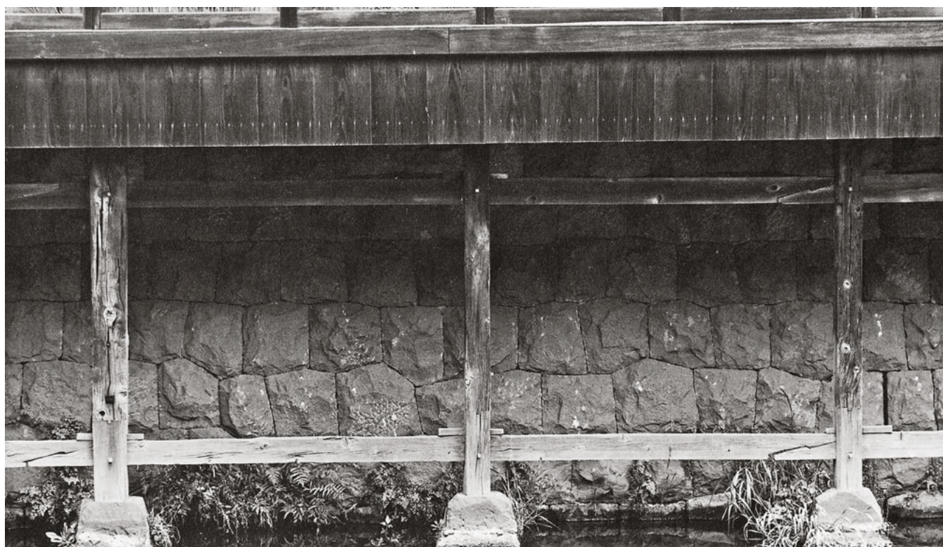
500 Every support of the Rinshun kaku in the Sankeien, Kanagawa, Japan, has a new base. The horizontal members which brace the construction are in each case spliced at the point where they intersect the support.
