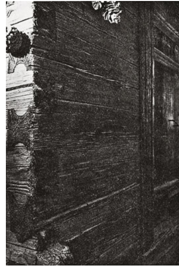
544 Why the Kugelschrot ( Kugel = sphere) should be so named is really not at all clear; parallel with the grain it is a half-cylinder, on the end grain a semicircle. – Grafenbach, Carinthia, Austria
