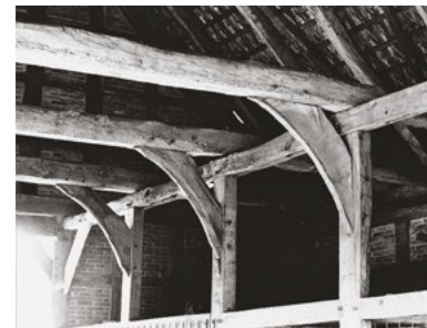
352 In normal assembly the beams are laid on top of the header which bears on the columns. – Barn from Grönloh, Lower Saxony, Germany, in Cloppenburg Open-air Museum.
