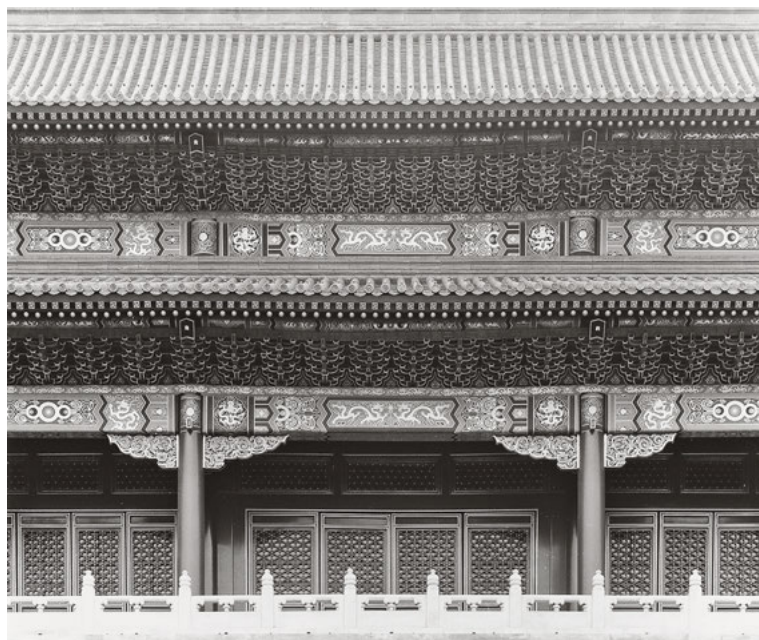
647 A section of the façade of the Gate of Great Harmony (Taihe men) in the Forbidden City illustrates the primary decorative function of the later dougong . The eight intermediate dougong are almost impossible to differentiate from those over the columns.
