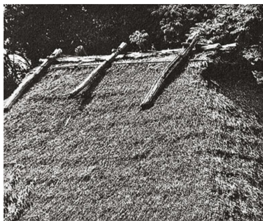
247 Ridge "finials" fasten the ridge covering of a cowshed from Tsuruga, Fukui, Japan. – In the Toyonaka minka shuraku
