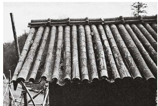
469 Unsurpassed in its lightness, ingeniously simple in its water drainage concept, the bamboo roof nevertheless is burdened by too many disadvantages for it to be a winner in our modern world. – Yokohama, Kanagawa, Japan (photo: Kawashima, Chuji)
