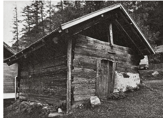
313 Just the direction of the ridge-supporting column betrays the fact that this construction is borrowed. – Unterried-Lehn, Tyrol, Austria.
