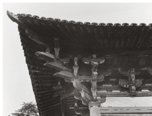
641 The dougong above the corner columns are much larger than the others due to the increased weight and larger roof overhang at the corners. Foguang si Dongda dian
