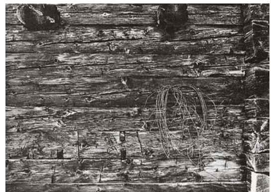
467 Angled jointing nails hold the pieced logs in the assembly. – Stall, Carinthia, Austria
