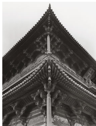
614 Both eaves of the Dule si Guanyin ge show how the rafters fan out at the corner. To make that possible they are cut to a wedge shape at their inner ends.
