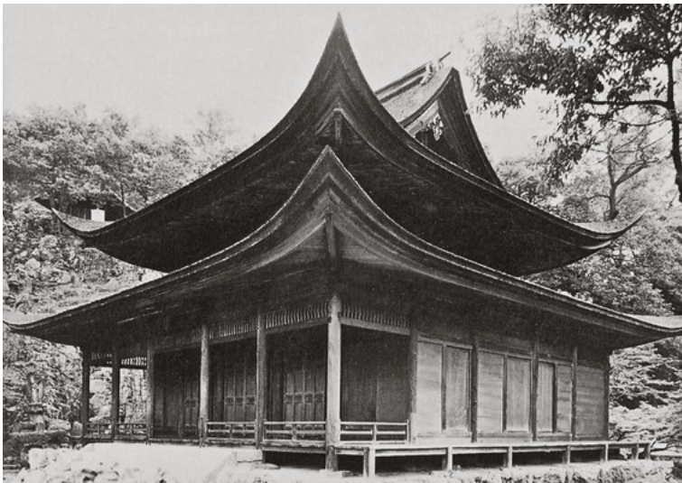
74 The Eiho-ji kannondo, Gifu, Japan, is one of the very few temples with planking to the eaves.
