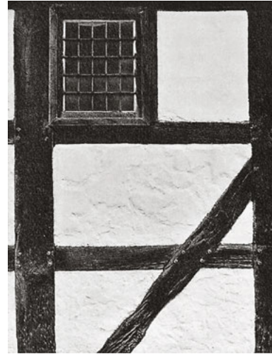
537 The wooden nail enables us to see immediately whether overlapping members are connected by way of a lap joint or a mortise and tenon. – Cloppenburg Open-air Museum
