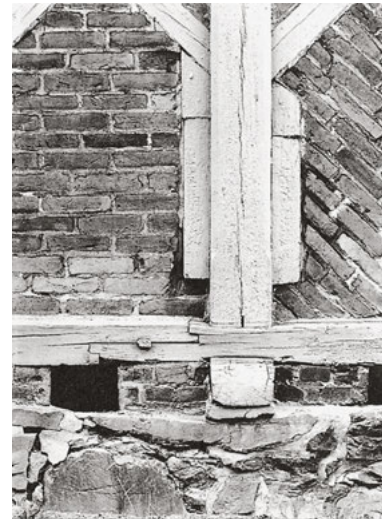
3 As a rule, horizontal timbers subjected to compressive loads cannot buckle; instead they are crushed. Therefore, the growth rings of rift-sawn wood are placed opposing the compression whenever possible. – Sill of a timber-framed building in Oslo, Norway.
