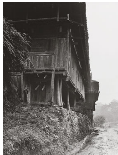
584 The overhanging columns of the cantilevered upper storey lend the construction its name: diaojiaolou . – Pingqiu, Guangxi
