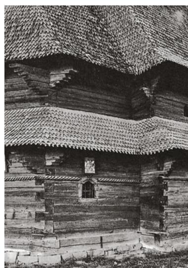
42 The wall of the church in Bogdan Vodă, Maramureș, Romania, is so high that a monopitch roof has been incorporated halfway up to protect against driving rain.
