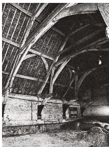
515 This form of construction can be studied at close quarters in this cowshed in Tarrant Crawford, Dorset, England.
