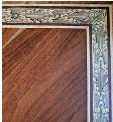
V-blocks break up long borders, and provide an opportunity to adjust patterned borders to join at the corners.
