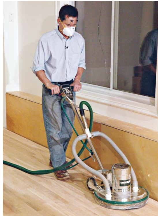
Use a buffer to blend in the scratches from the edger and the big machine.
