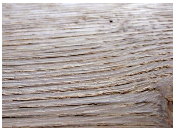
Grain raise: The wood surface is ridged and rough.
