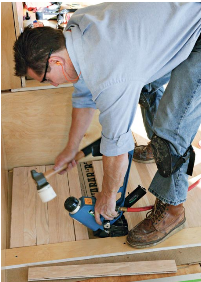
Wearing hearing, eye, and knee protection is an essential safety measure when installing hardwood flooring.
