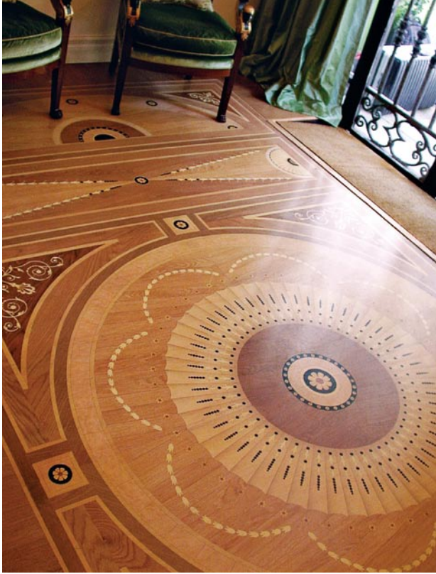
Faux painting allows limitless designs on wood floors. It can be freehanded or stenciled and is protected by the finish coat.
