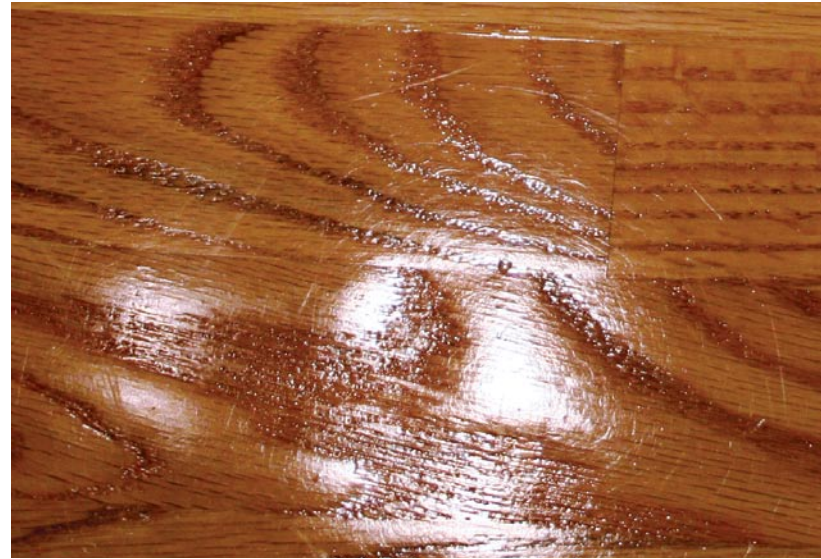
Screen sanding marks are spider web scratches in the finish.
