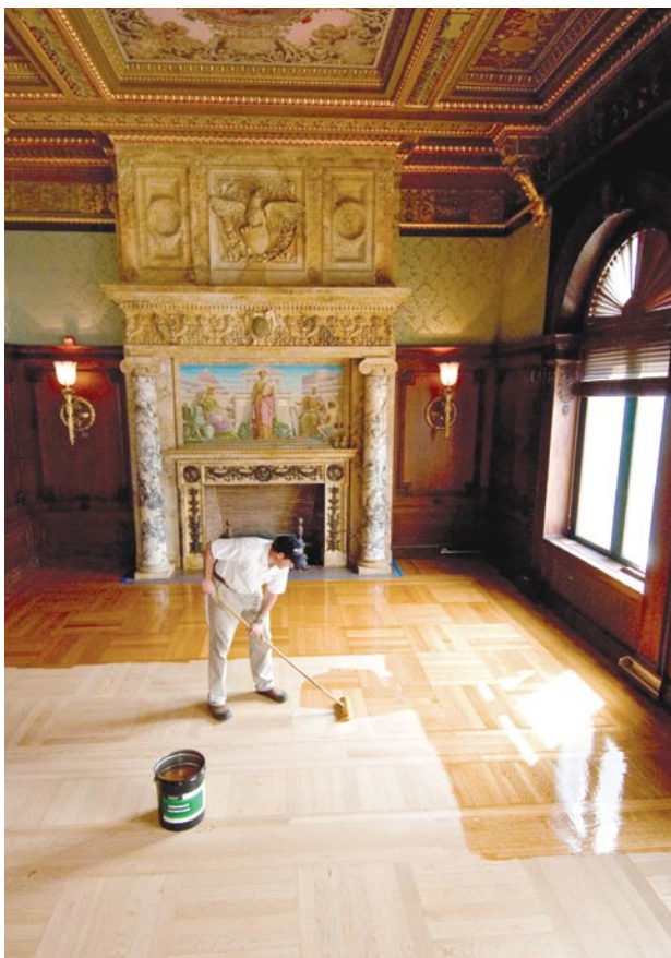
First-coating a newly sanded floor with sealer promotes better adhesion, reduces the chances of tannin staining, and, because sealers dry quickly, allows two coats in one day.
