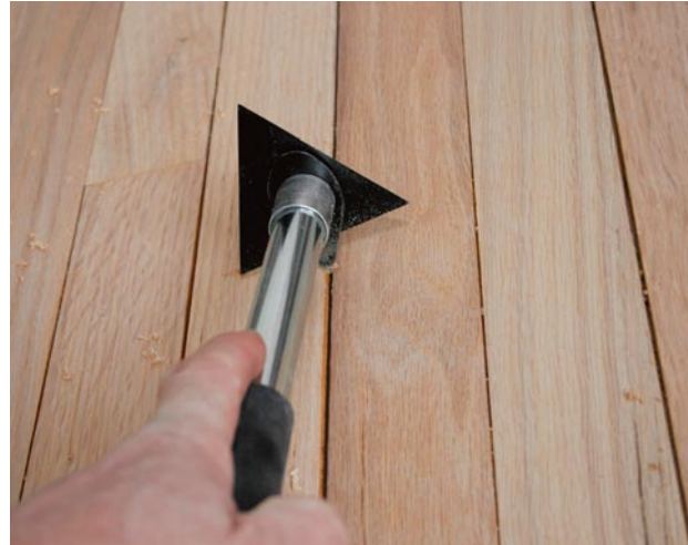
When stripping prefinished flooring, getting the old coating out of the bevels requires the attention of a scraper.
