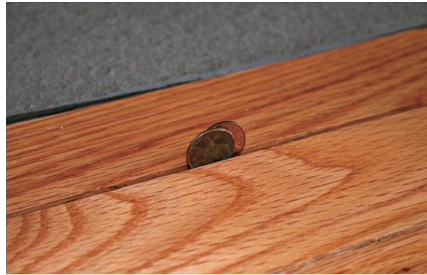
Gaps between the boards in wood floors may be normal.
