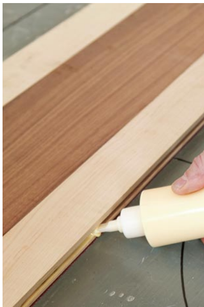
After you've installed the first few rows of flooring, remove the starter blocks. Apply wood glue into the groove of the first row.
