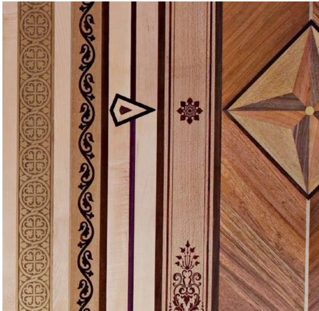
V-blocks break up long borders, and provide an opportunity to adjust patterned borders to join at the corners.
