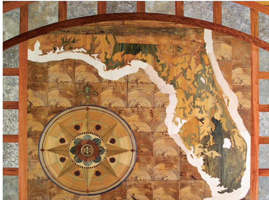
End-grain flooring is made from sections sliced from the end of thick beams. Typically glued down, end-grain flooring is extremely durable and was a favorite for old factory floors.
