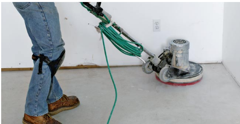
ABOVE LEFT A hood test must be performed over clean, bare concrete. Sand a small area for each test site.
