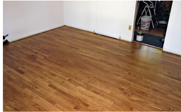
The same floor after application of two-part bleach and a medium-tone oil stain.
