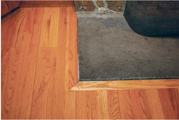
Installation near a room's focal point emphasizes the floor's workmanship, be it poor (left) or good (right).
