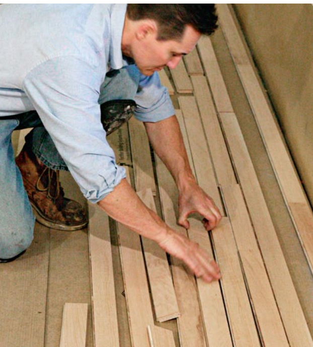
Narrower flooring—less than 3 in. wide—can be spread out in the room where it’s to be installed to acclimate.
