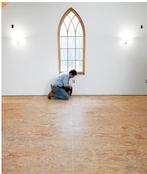
In wide rooms, starting the layout in the center and working toward both sides reduces problems with expansion. The starting point is a chalkline centered in the room, which automatically adjusts for out-of-parallel walls.
