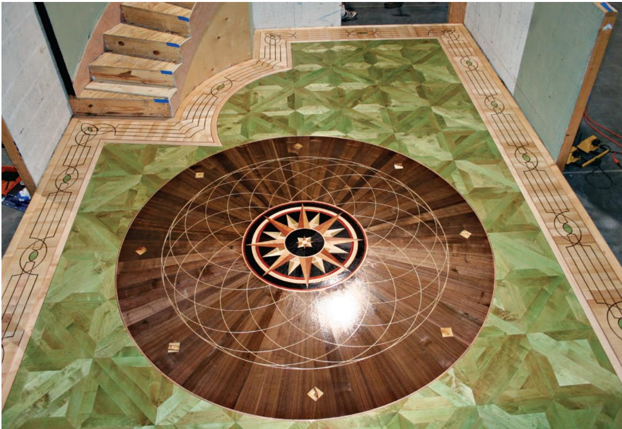
Dyes use smaller particles suspended in water or alcohol to lay down earth tones and create wilder effects.
