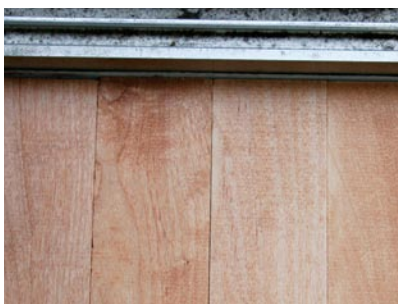
Picture framing occurs when the perimeter of the room finishes differently than its center.
