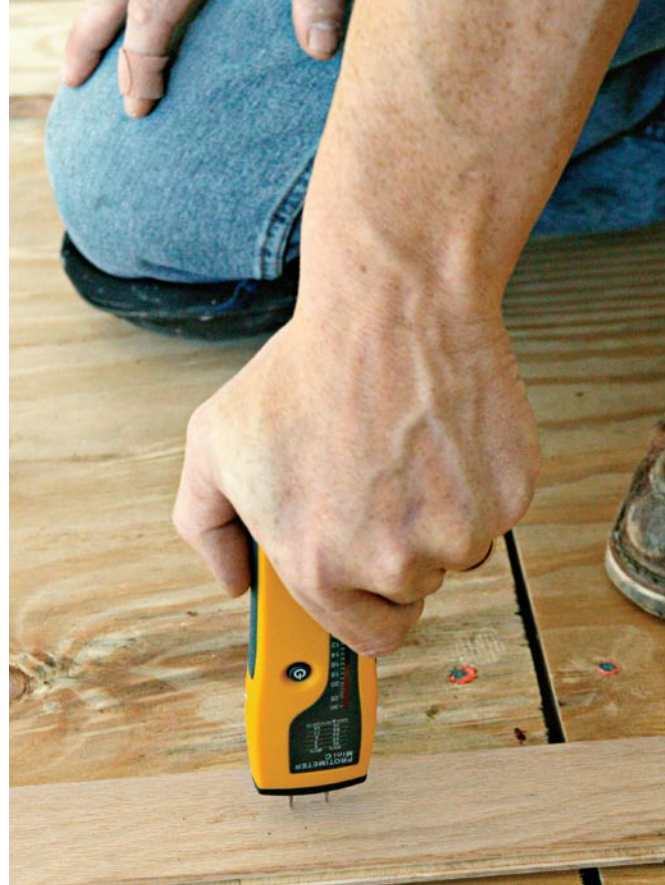
The only sure way to tell if the flooring is at the correct moisture content for the job is to measure it with a moisture meter.
