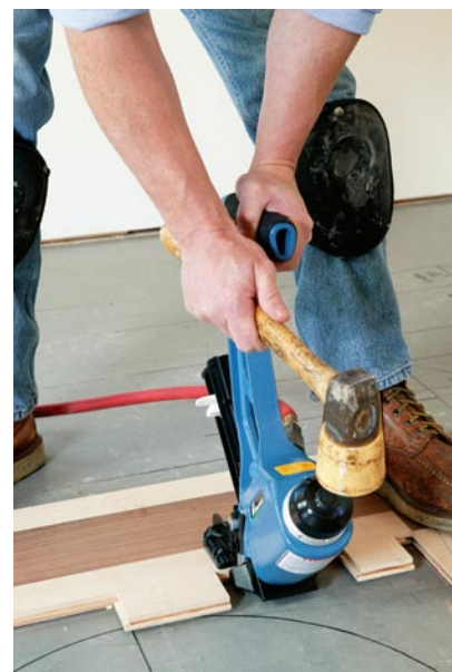
Blind-nail through the spline, using scraps of flooring to keep the spline aligned. Now the flooring installation can proceed in both directions.
