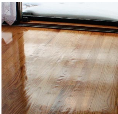
The first job of floor sanding is to flatten the surface. Here, a poor sanding job has created depressions that look terrible in raking light.
