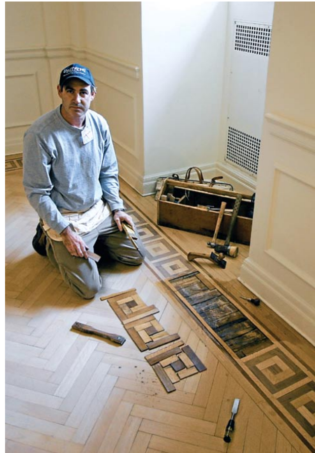
Pieces of a damaged border are removed carefully and replaced with wood of a similar age and grain pattern.
