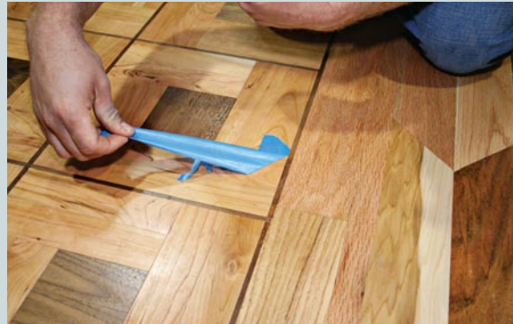
A little paint saved the floor from having a new accent strip surgically installed.
