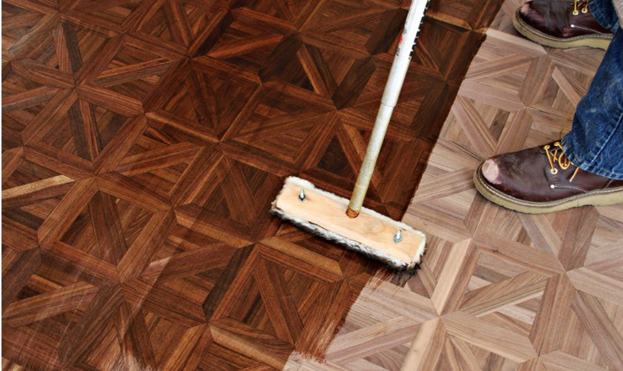
Pigment stains have relatively large particles suspended in an oil base and commonly create earth tones.
