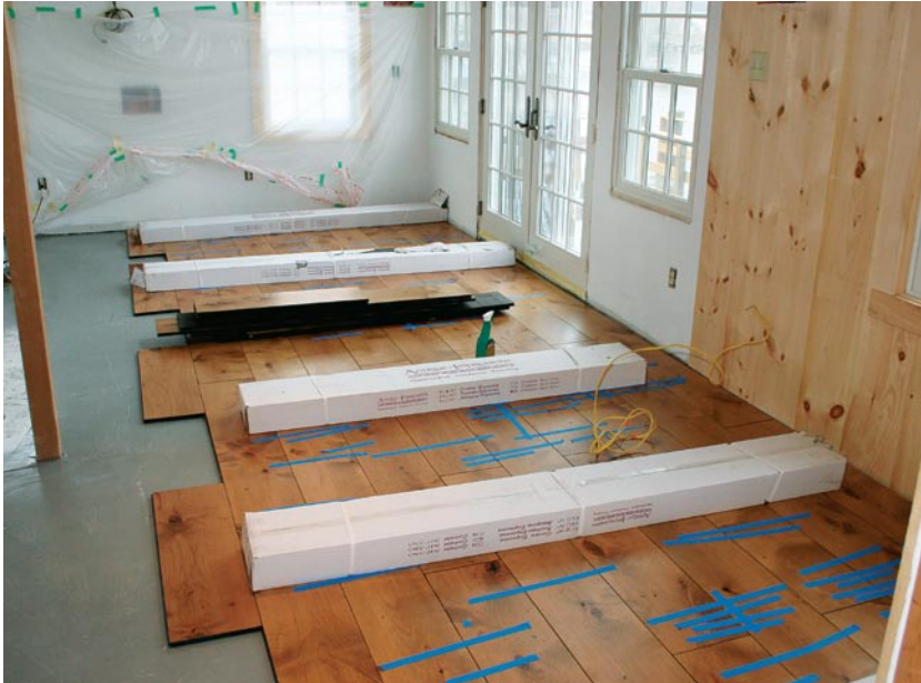
The author keeps wet-lay installations tight until the glue sets with 3M Scotch-Blue 2080 tape. Boxes of flooring add weight.
