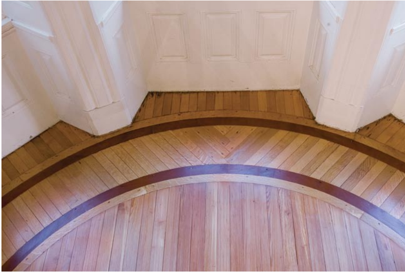
LEFT Aprons provide an area to make adjustments so the floor can flow smoothly to the wall.
