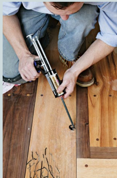
Fill knotholes with 5-minute epoxy. Both 3M's black 420 epoxy and their clear epoxy work well. Clear epoxy allows the color of the knot itself to show through.
