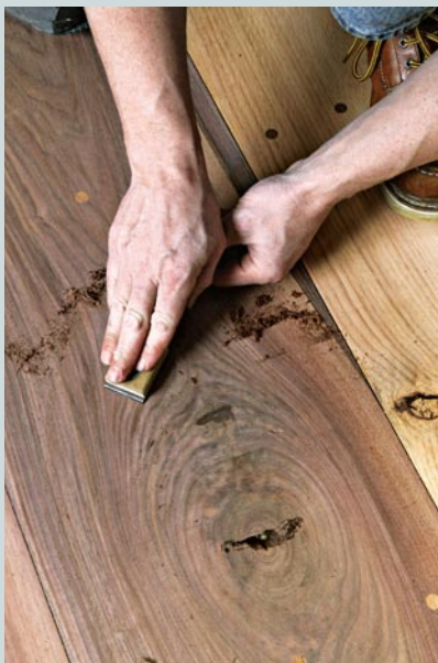
Scrape around knots, leaving the harder, longer wearing end grain gently proud of the surrounding floor.
