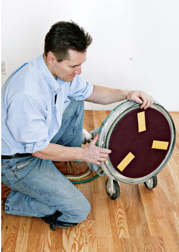
ABOVE LEFT Use a 3M Scotch-Brite pad with abrasive strips to sand between coats. Use 180-grit abrasive strip for oil-based polyurethane and many water-based sealers, and 240-grit abrasive strips for waterborne finishes.
