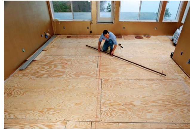
Trammels turn any length stick into a compass.
