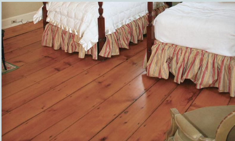
Colonial-era wide-plank floors were installed directly over the joists, with no subfloor. Cut nails provided effective holding power in some cases for centuries.
