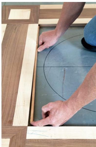
Insert a spline, or slip tongue, into the glue in the groove and tap it into place.
