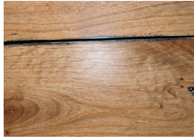
Bleed-back occurs when stain seeps up from the grain or from the spaces between boards.
