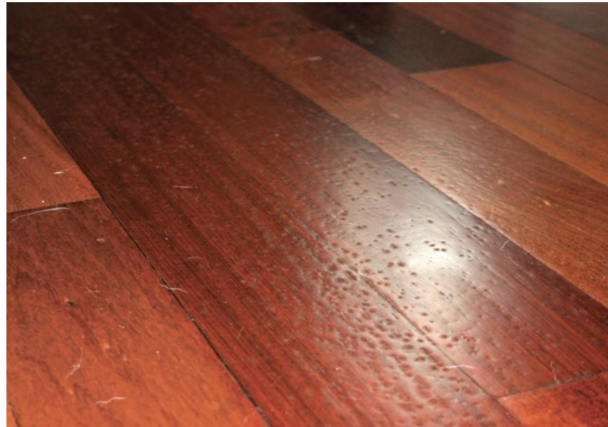
Orange peel: The finish surface has the texture of an orange peel.
