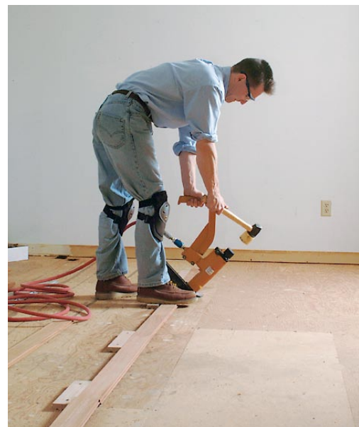
Screw temporary blocks to the subfloor along the chalkline. The blocks keep the first row straight as it's nailed down.
