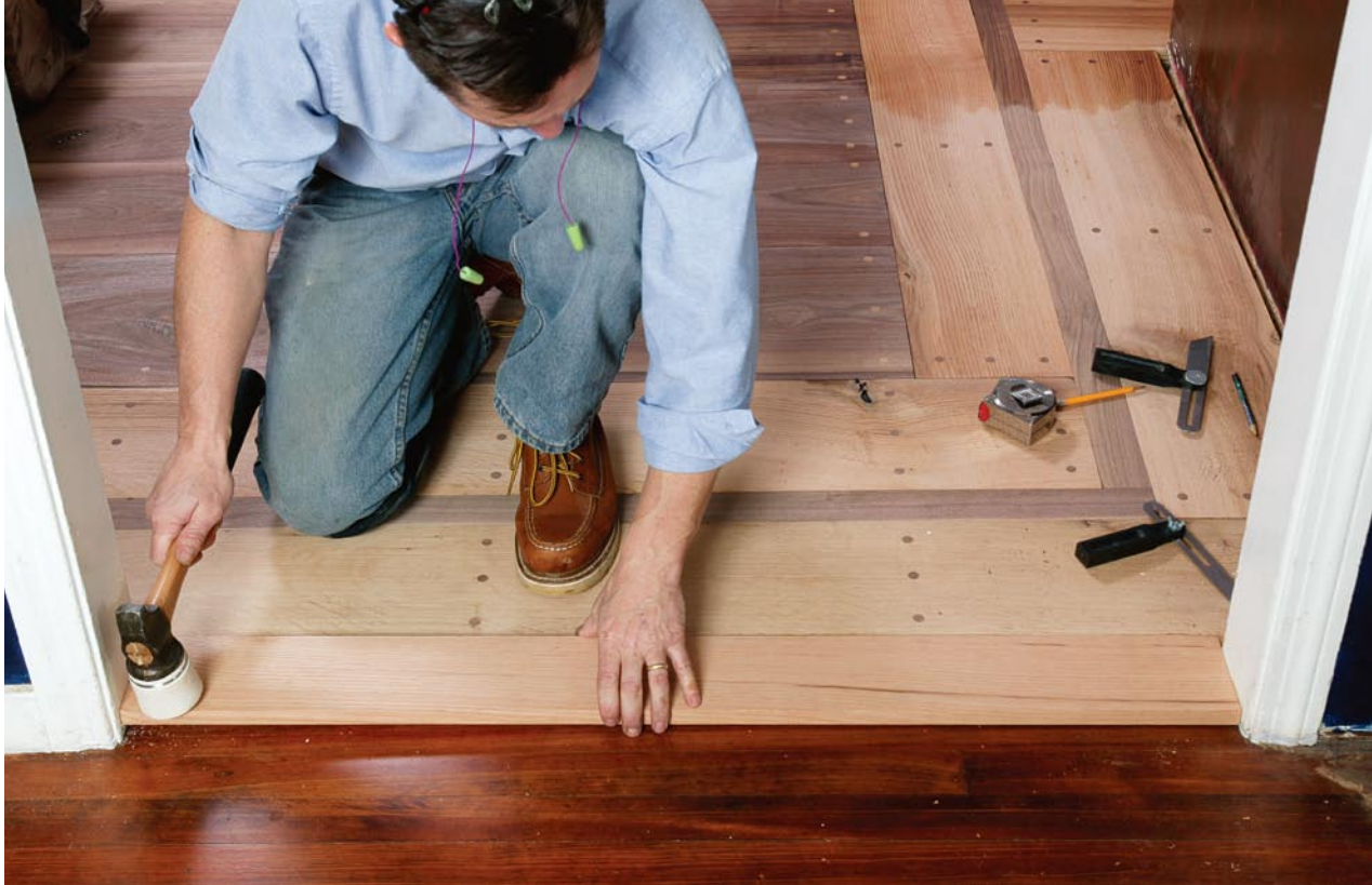
A reducer is used to transition between two flooring materials with different heights, typically at a doorway.
