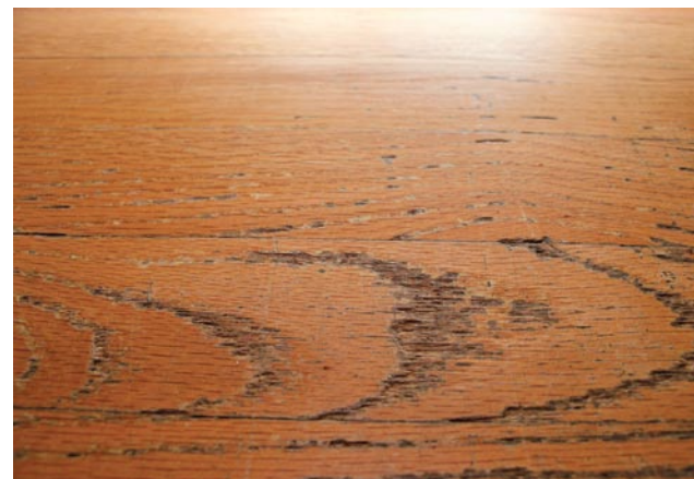
Shellout is wear in the softer spring or early wood.
