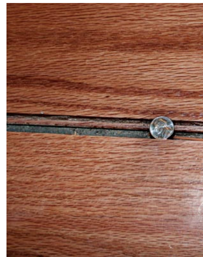
If wood flooring is too wet when installed—often because it picked up excess moisture from construction sources such as drying concrete, plaster, or paint—gaps will open up as it dries.
