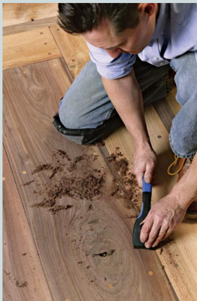
Scrape with the grain of the wood.
