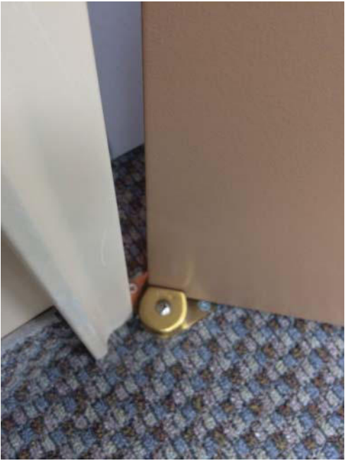
FIGURE 1.83 Floor-Mounted Bottom Offset Pivot (Source: Courtesy of Scott J. Tobias)
