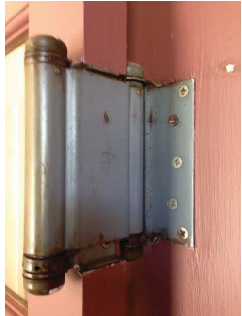
FIGURE 1.25 Double-Acting Spring Hinge (Source: Courtesy of Scott J. Tobias)
