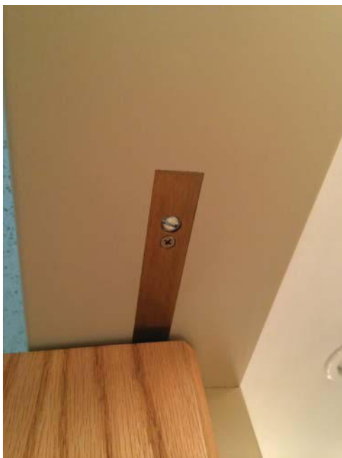
FIGURE 1.86 Center Bottom Pivot Arm
