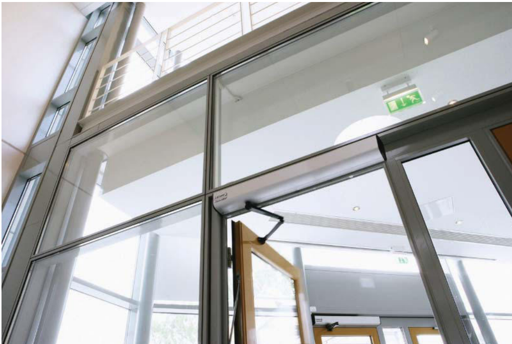
FIGURE 5.17 Surface-Mounted Powered Door Operator (Source: ASSA ABLOY Entrance Systems)
