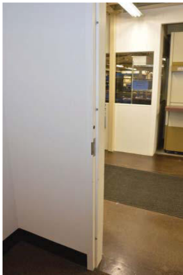
FIGURE 9.45 Single Metal Door Frame Silencer Installed (Source: Courtesy of Scott J. Tobias)
