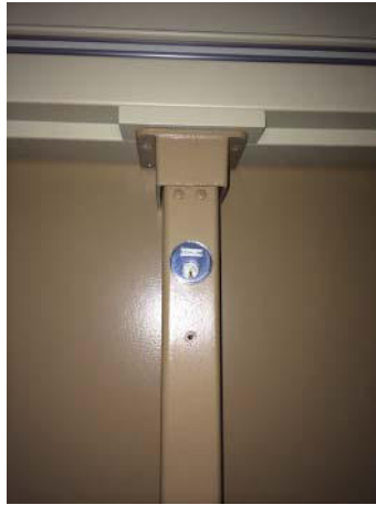
FIGURE 2.93 Lockable Removable Mullion (Source: Courtesy of Scott J. Tobias)
