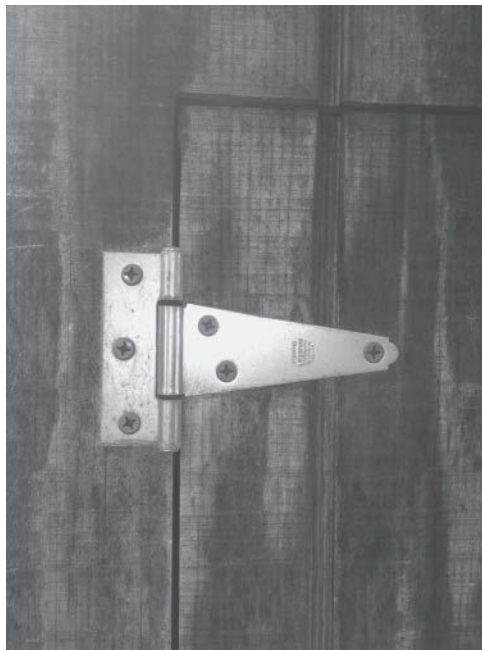
FIGURE 1.29 Tee Hinge (Source: Scott J. Tobias)
