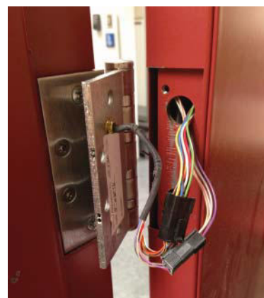
FIGURE 1.38 Molex® Connector Wired to Door (Source: Copyright © ASSA ABLOY, Inc. All rights reserved.)
