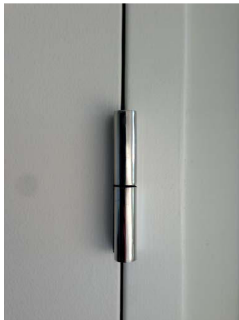
FIGURE 1.9 Two-Knuckle Hinge (Source: Courtesy of Scott J. Tobias)
