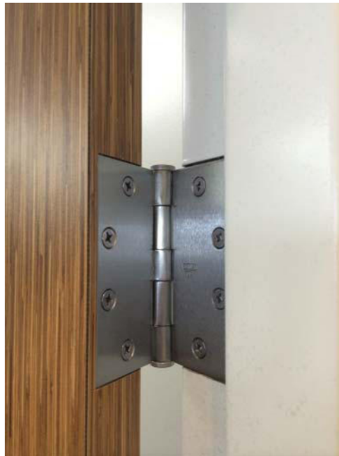
FIGURE 1.3 Nonbearing Full Mortise Butt Hinge
