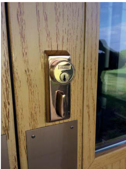
FIGURE 2.69 Exit Device Auxiliary Control (Source: Courtesy of Scott J. Tobias)
