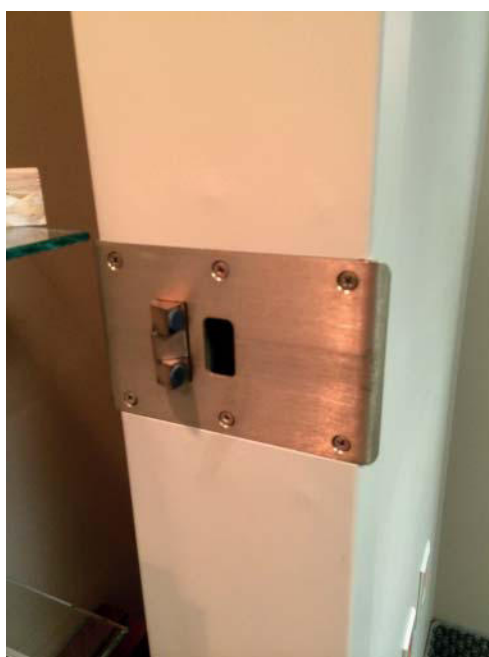
FIGURE 1.94 Double Lipped Strike with Built-In Emergency Stop
