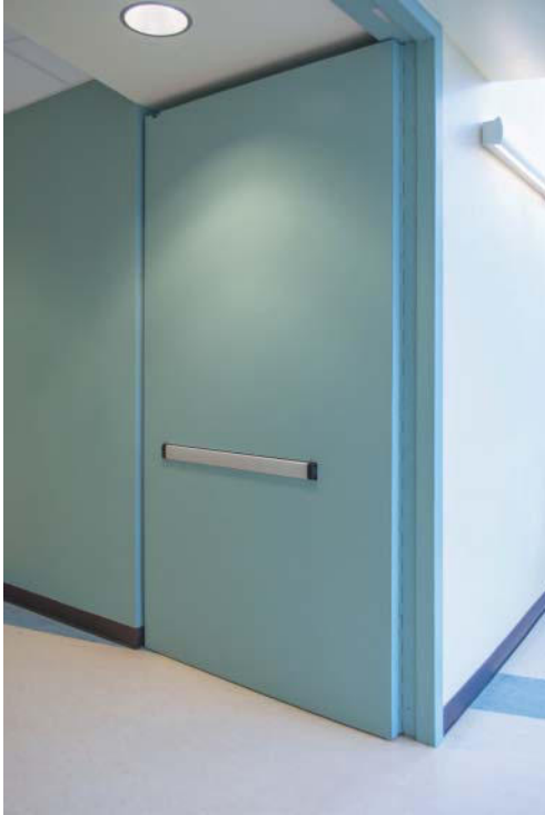
FIGURE 2.52 Integrated Exit Device
