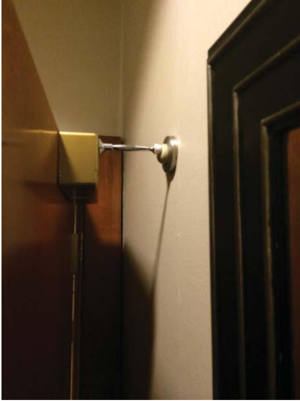
FIGURE 7.6 Electromagnetic Hold-Open Armature Extension (Source: Courtesy of Scott J. Tobias)
