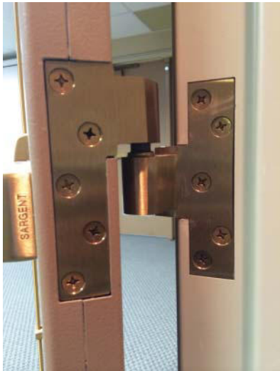
FIGURE 1.84 Intermediate Offset Pivot (Source: Courtesy of Scott J. Tobias)
