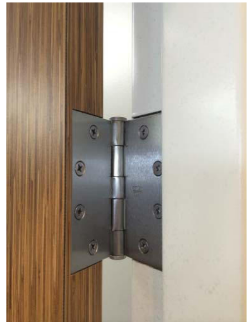
FIGURE 1.46 Full Mortise Hinge
