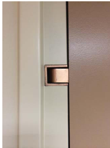
FIGURE 1.96b Closed Pocket Pivot (Source: Courtesy of Scott J. Tobias)
