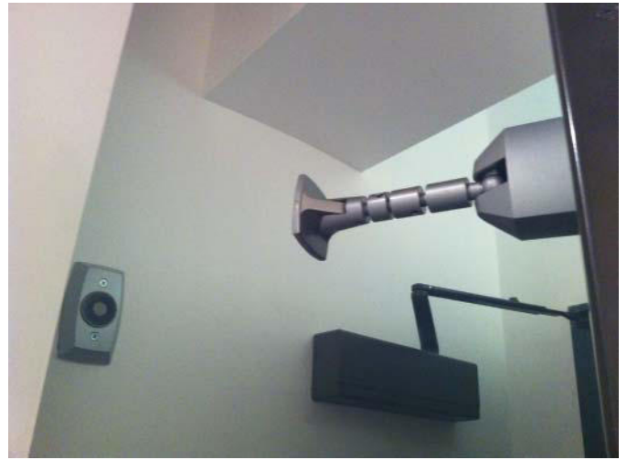
FIGURE 7.7 Electromagnetic Hold-Open Swivel Armature Extension (Source: Courtesy of Scott J. Tobias)
