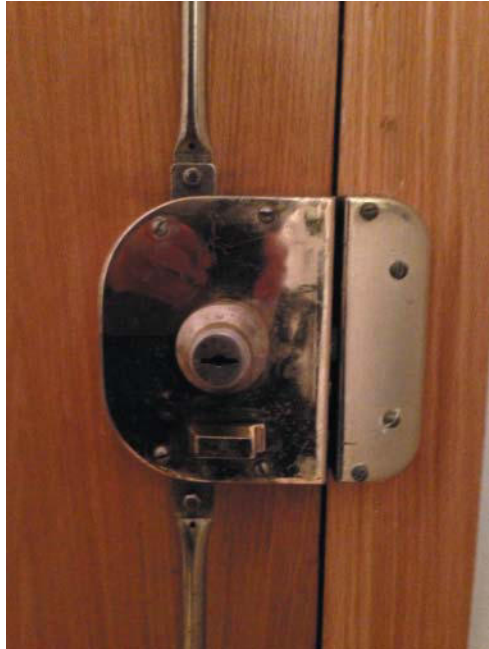
FIGURE 2.178 Rim Lock (Source: Courtesy of Scott J. Tobias)
