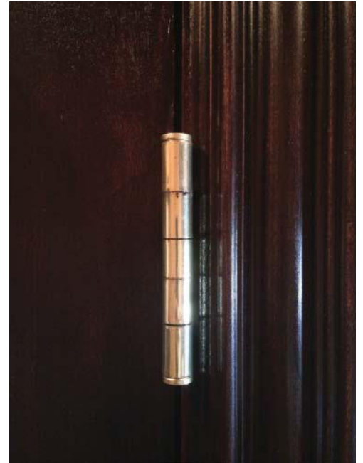
FIGURE 1.7 Five-Knuckle Hinge Barrel
