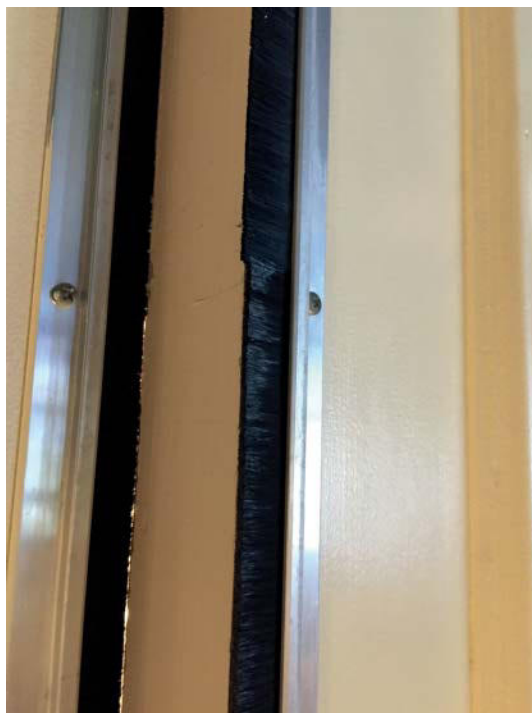
FIGURE 8.28 Meeting Stile Brush Weatherstripping (Source: (Courtesy of Scott J. Tobias)
