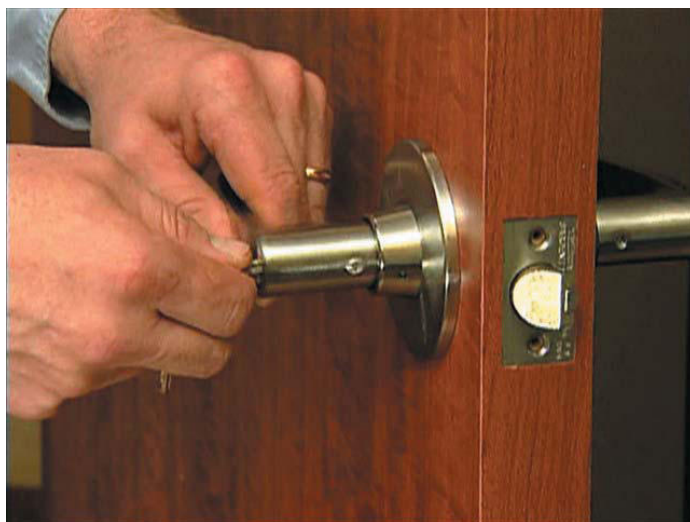
FIGURE 2.179 Bored Lockset Being Installed on Door (Source: Courtesy of SARGENT® Manufacturing Company)
