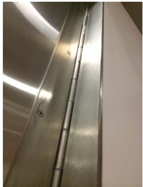
FIGURE 1.61 Pin and Barrel Continuous Hinge (Source: Courtesy of Scott J. Tobias)
