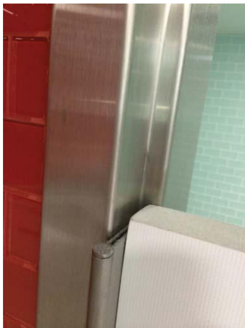
FIGURE 1.62 Pin and Barrel Continuous Hinge
