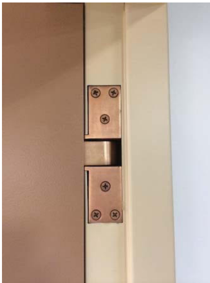
FIGURE 1.96a Open Pocket Pivot (Source: Courtesy of Scott J. Tobias)
