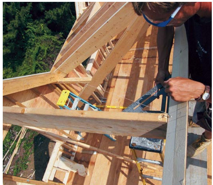
Corner of the valley. Angles that are taken on each side of the string determine the corner cuts that are needed for the ends of the valley rafter.
