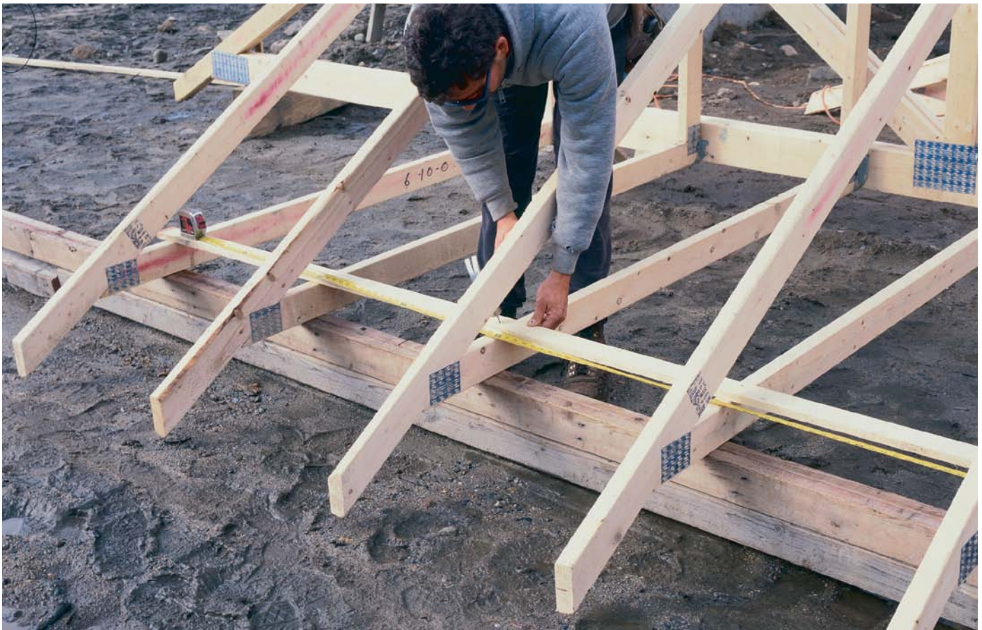
A furring-strip spacer keeps the tails in place. Before the system can be squared, the tails of the face jack trusses are spaced according to the layout and held in position with a piece of 1x3.
