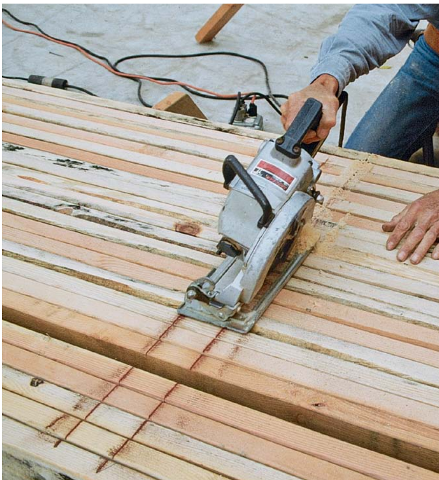
One method for gang-cutting bird's mouths is to cut the heels with a worm-drive saw (above) and the seats with a worm-drive saw fitted with a swing table, an accessory base that adjusts from -5^{\circ} to 68^{\circ} (right).
