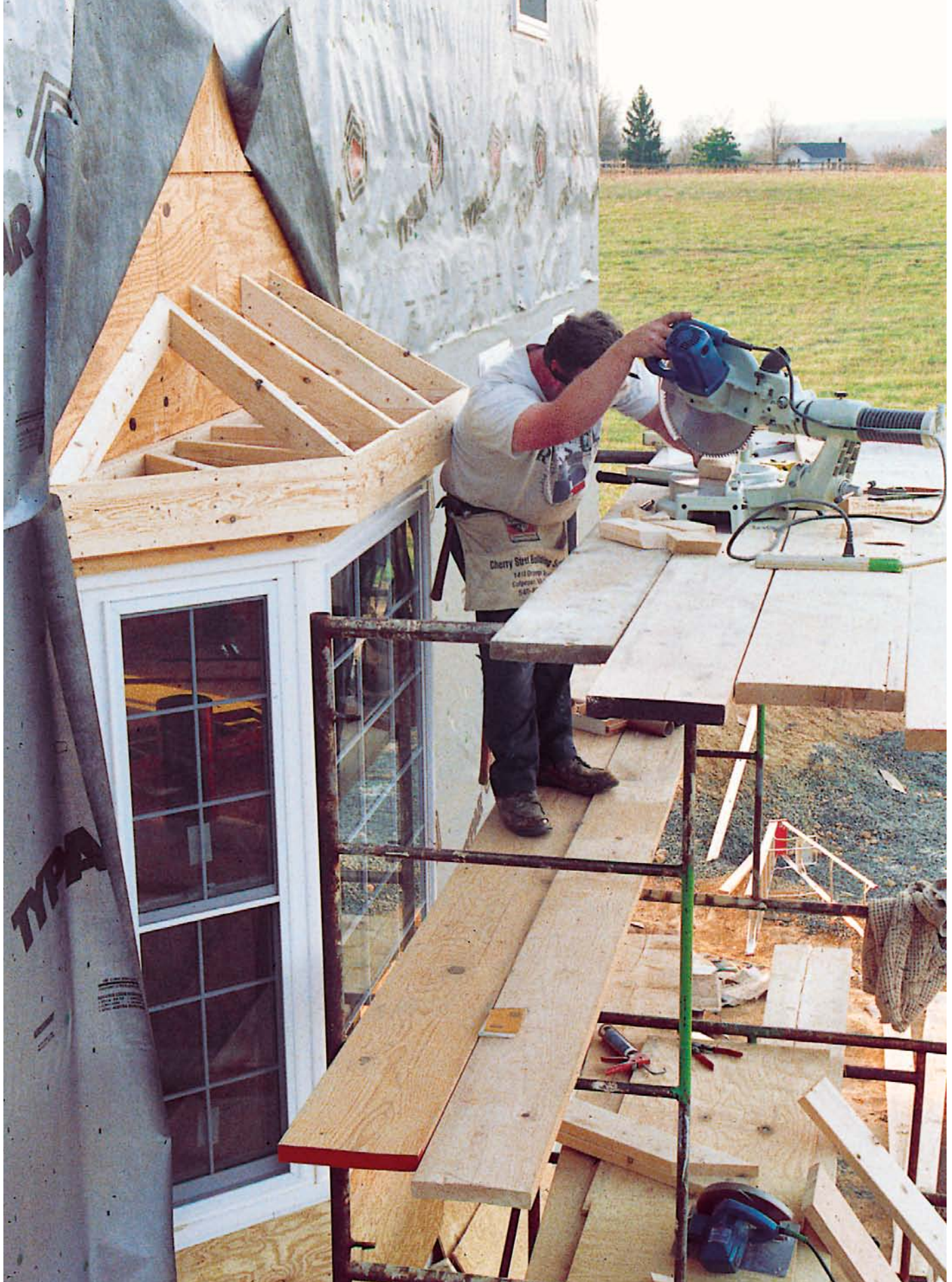
A sturdy scaffold makes for efficient bay-roof construction. The walk-board height allows work to be done at waist level. The boards behind serve as a workbench, saving a lot of climbing up and down.
