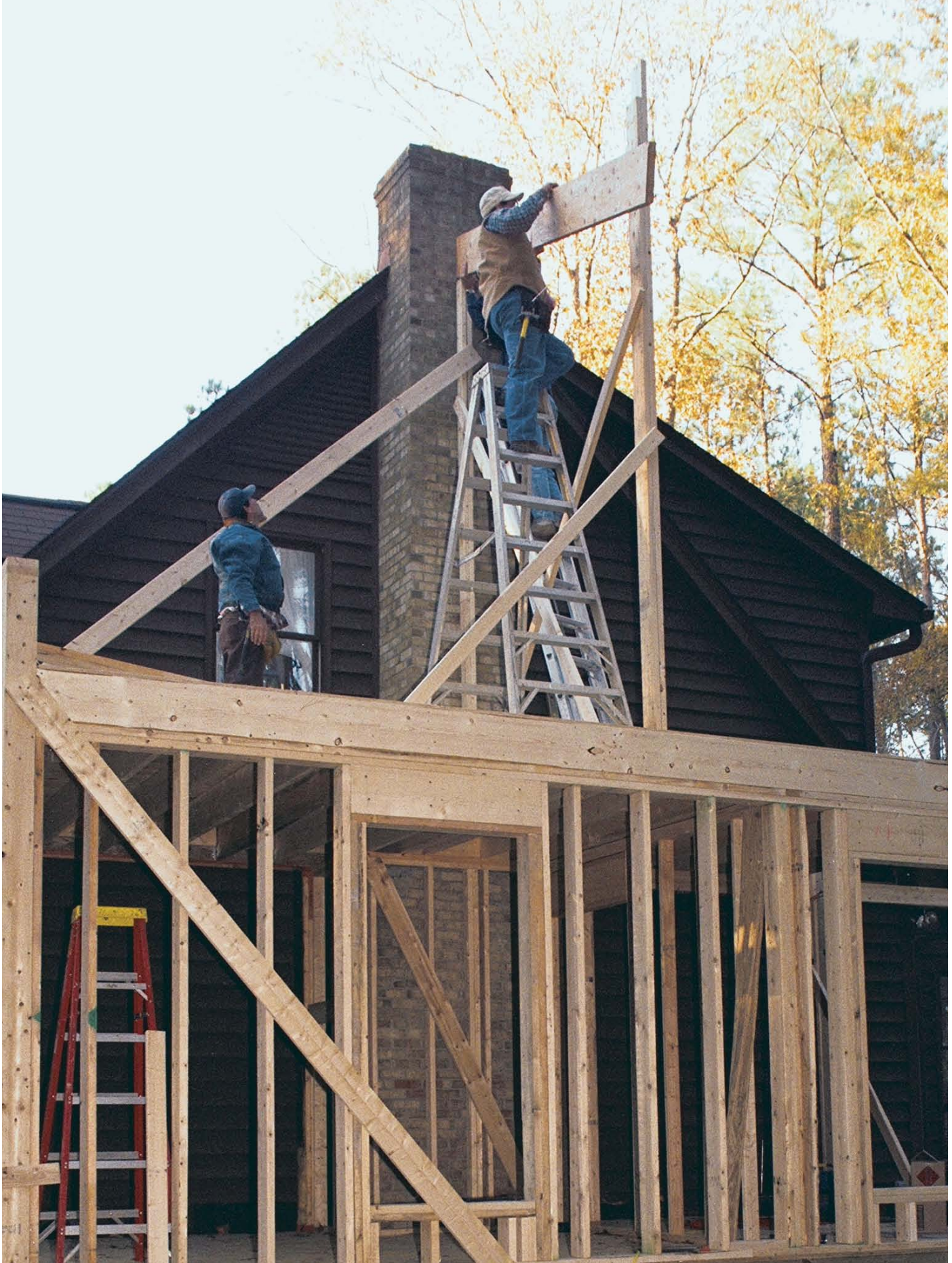
Setting the ridge. Temporary posts are set up to hold the ridge at the right height. The posts are braced 2x4s with a 2x4 scrap nailed to the top that rises 10 in. above the top of the post. The ridge is set on top of the post and nailed to the scrap of wood.
