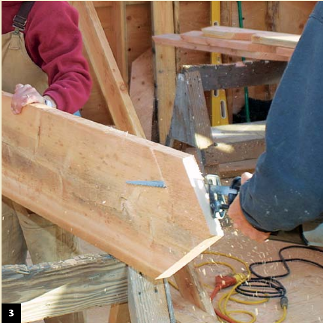
2. Saw set at 90° rides on first heel cut for a 72° angle
