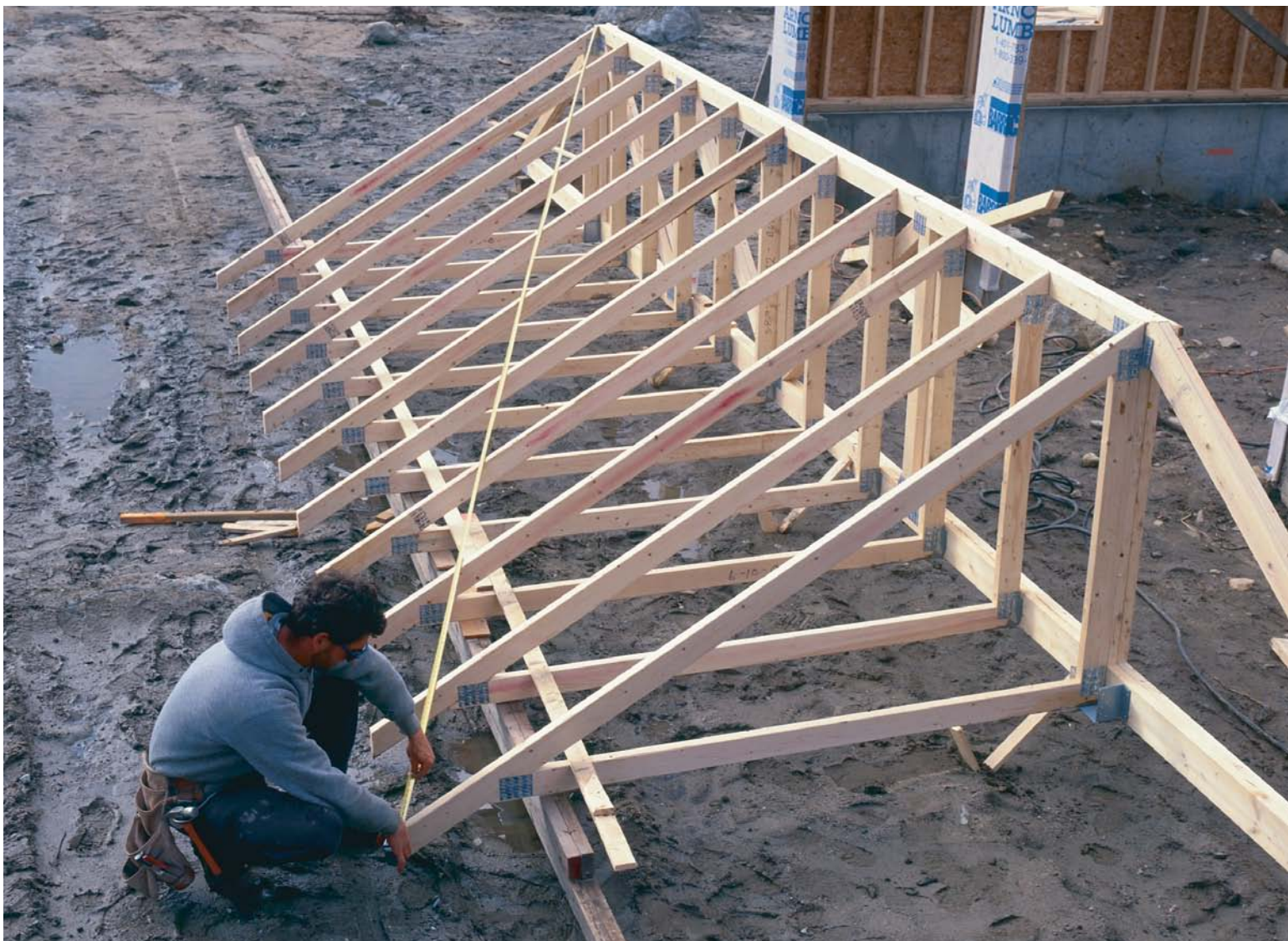
Diagonal measurements square the system. Measurements are taken between the two outermost jack trusses, and the tails of the trusses are moved in unison until the measurements are equal.
