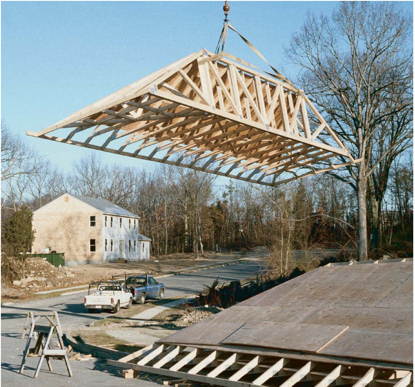
The hip goes up in one piece. Like a giant box kite on a string, an entire hip section is lifted to its home atop a two-story house.
