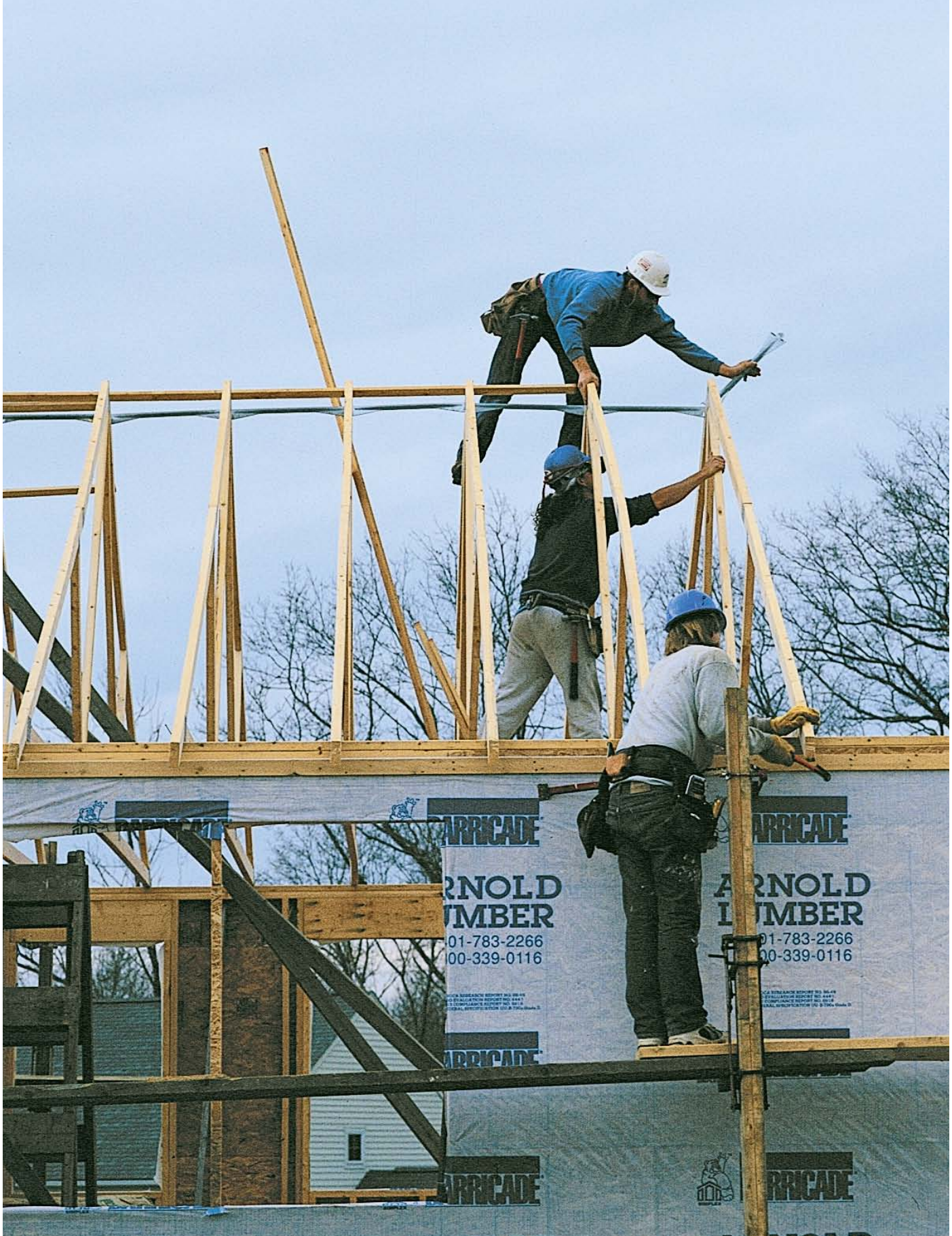
Spacers lock the peaks in position. One crew member holds the trusses in place while another attaches truss spacers (made by Truslock, Inc.) along the peaks of the trusses. Strapping replaces the spacers so that only a couple of 16-ft. lengths of spacers are needed. The crew member at the rear of the house taps the truss into position on the wall plate and nails it home.
