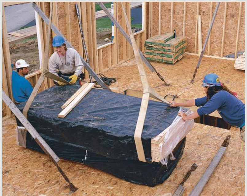
Prepackaged loads of sheathing are easier to handle. The lumber company bundles the sheathing in stacks of 15 to 20 sheets for easy strapping and lifting.
