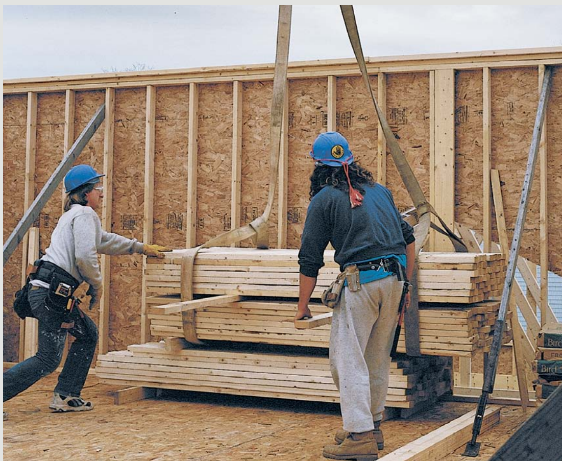
Interior wall framing on the rise. Lumber is stacked ahead of time for an easy crane hoist; crew members land the framing lumber inside the house where it will be out of the way until it's needed.
