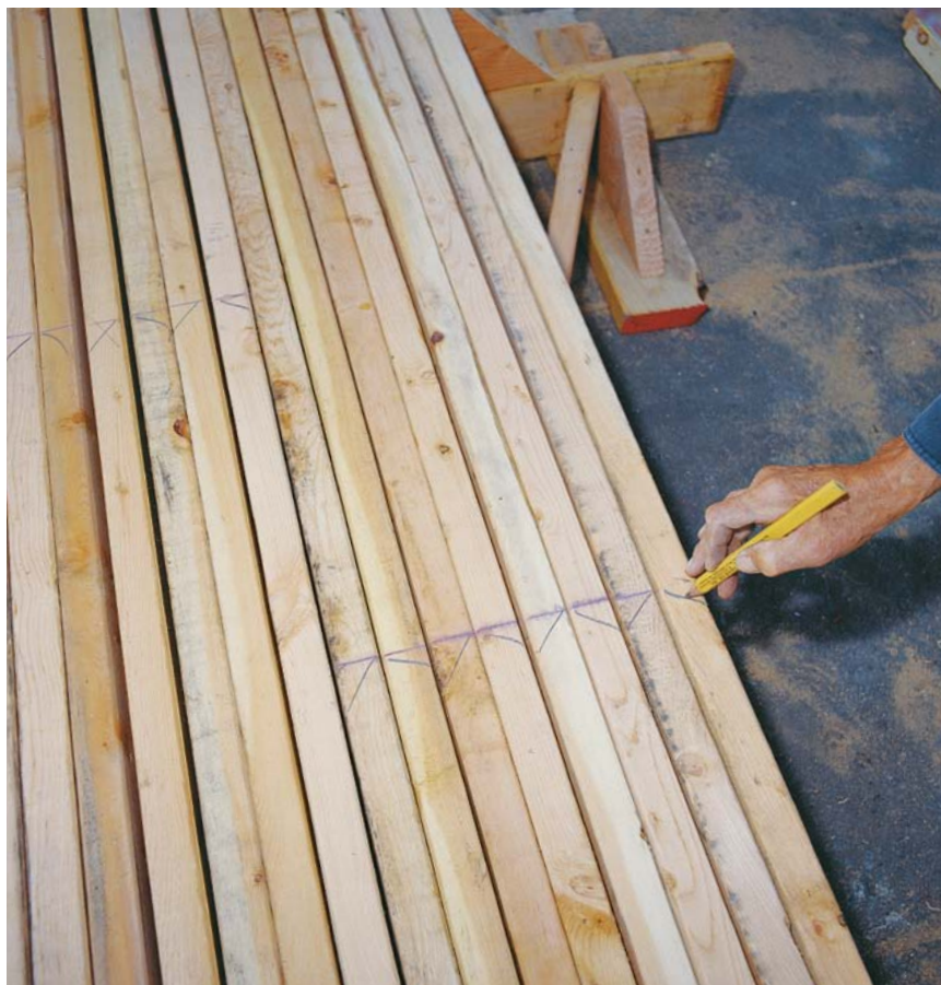
Jack rafters are laid out four pairs at a time. Jacks oppose each other in pairs along both sides of the hip rafter. Each successive pair is shorter by a specified length than the pair above it. Diagonal marks remind the author to make his 45° cuts in opposite directions.
