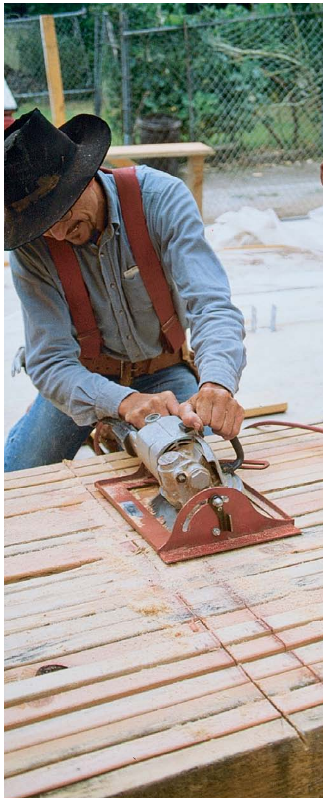
One method for gang-cutting bird's mouths is to cut the heels with a worm-drive saw (above) and the seats with a worm-drive saw fitted with a swing table, an accessory base that adjusts from -5^{\circ} to 68^{\circ} (right).
