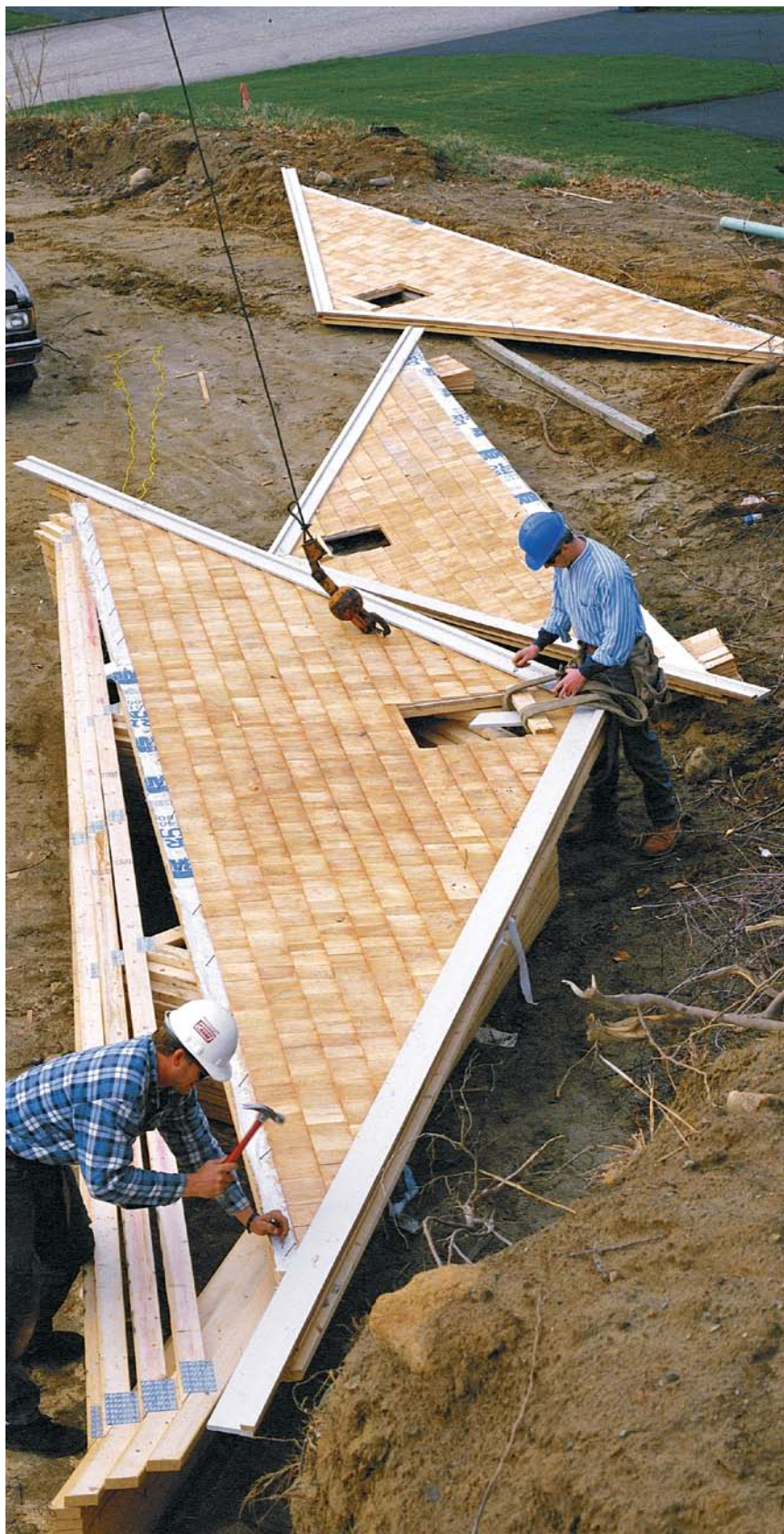
Nails for attaching the gable truss are started on the ground. To facilitate setting the gable truss, nails are started along the bottom chord. When the truss is in position, a crew member on a ladder will drive the nails into the top plate of the gable-end wall.
