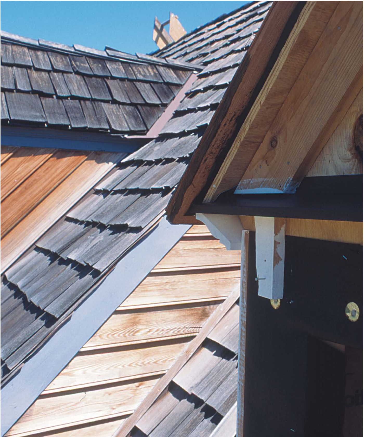
Water-table flashing protects window and trim. The crown that forms the bottom of the pediment will go below the flashed water table and miter with an eave crown (seen poking out past the corner).
