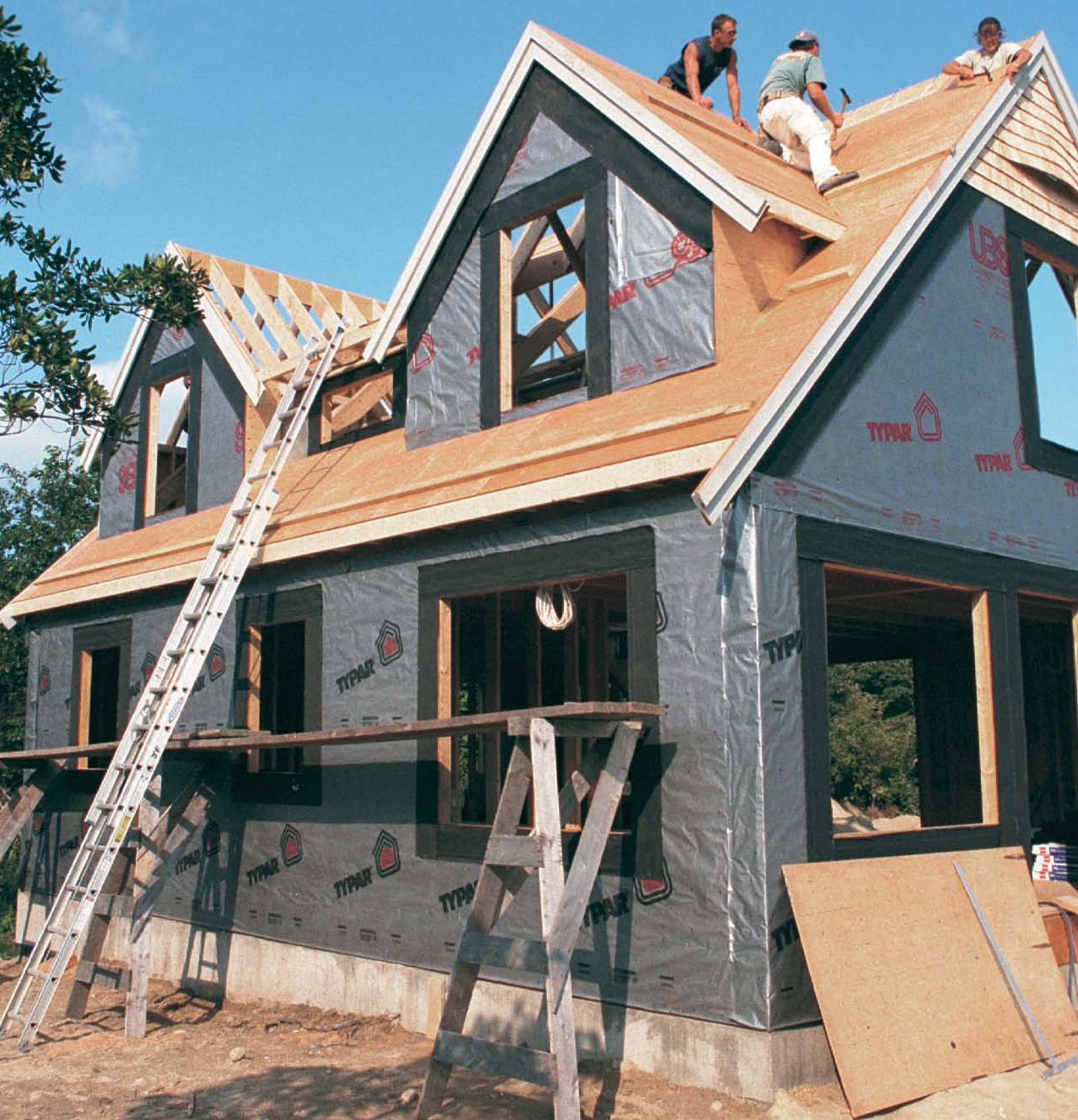
Skinning the dormer. When the framing is complete, the sheathing is applied, bringing out the final dramatic shape of the Nantucket dormer.
