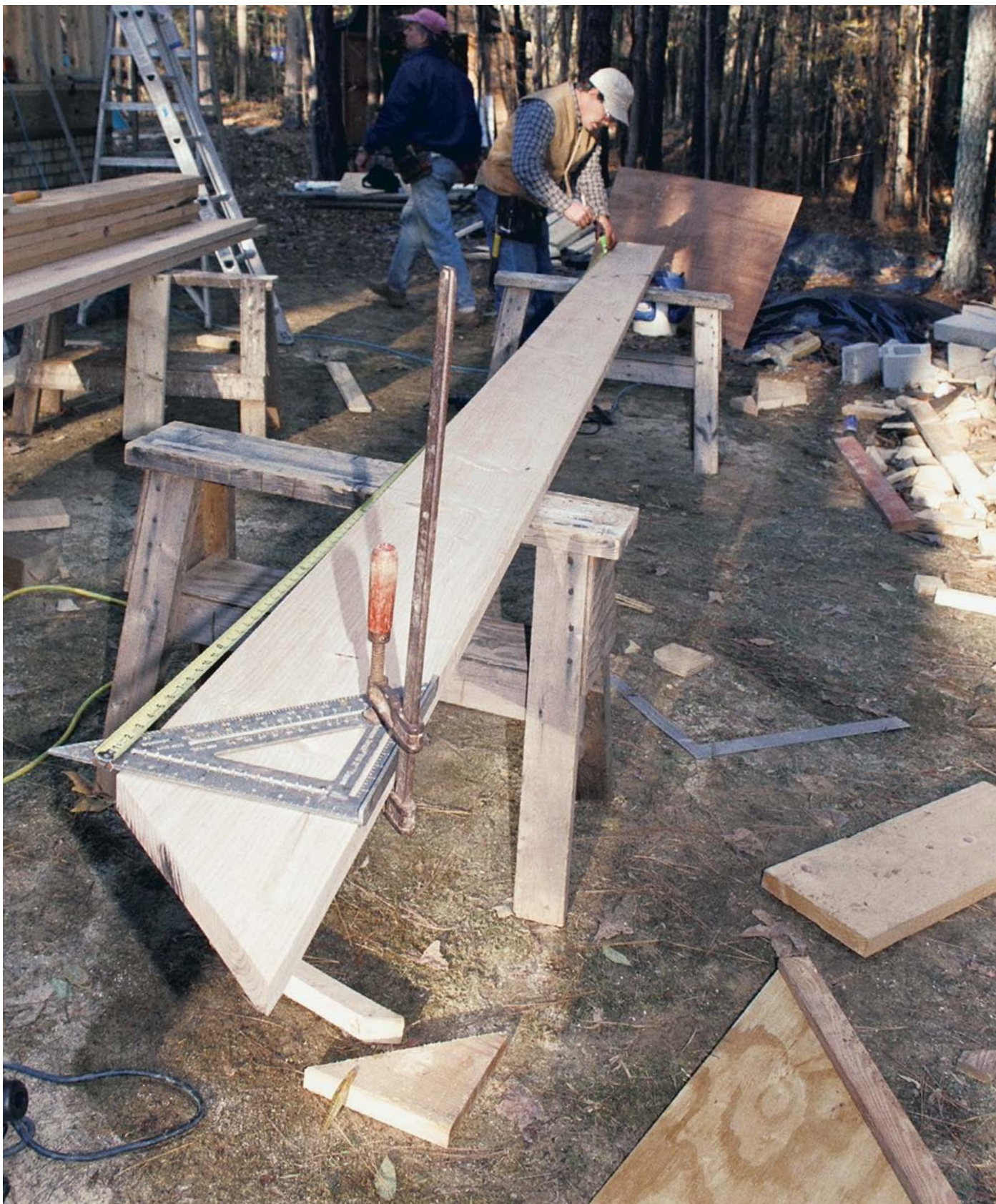
A clamped square serves as an extra pair of hands. It's easy to measure along the bottom of the rafter if you clamp a square to the bottom of the plumb cut and run your tape from there.
