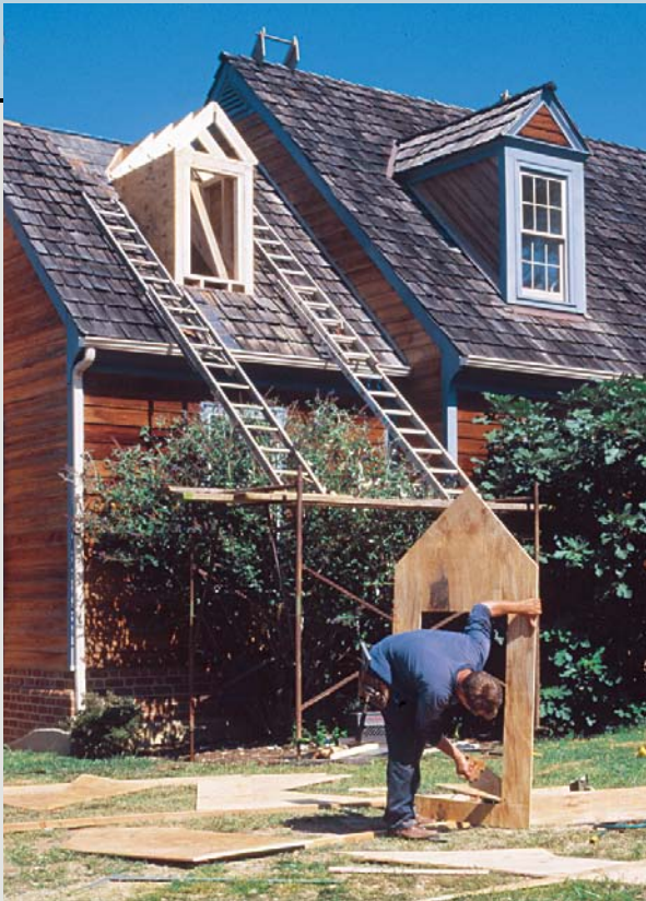
In the doghouse. Narrow dormers are prone to racking. To stiffen this one, the author sheathed the front wall with a single sheet of plywood.
