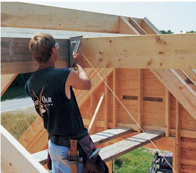
Finding the plumb cut. A rafter square held in the corner against the string determines the angle of the valley plumb cuts.
