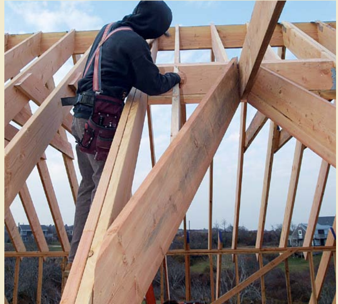
Just as if it grew here. When the valley is in place, the 72° heel cut lies flat against the doubled common rafters. The rafter bottoms are kept flush, and the dormer roof sheathing hides the height difference in the rafters.
