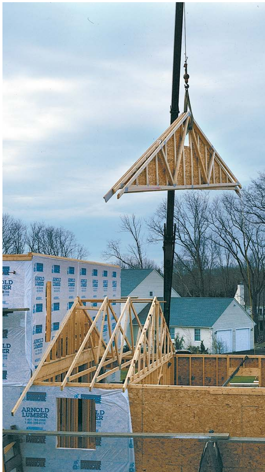
The first gable truss is sent up with two regular trusses. By sending the first three trusses up together, the crane will be able to hold the gable truss steady while the other trusses are set and while braces are attached to the gable truss.
