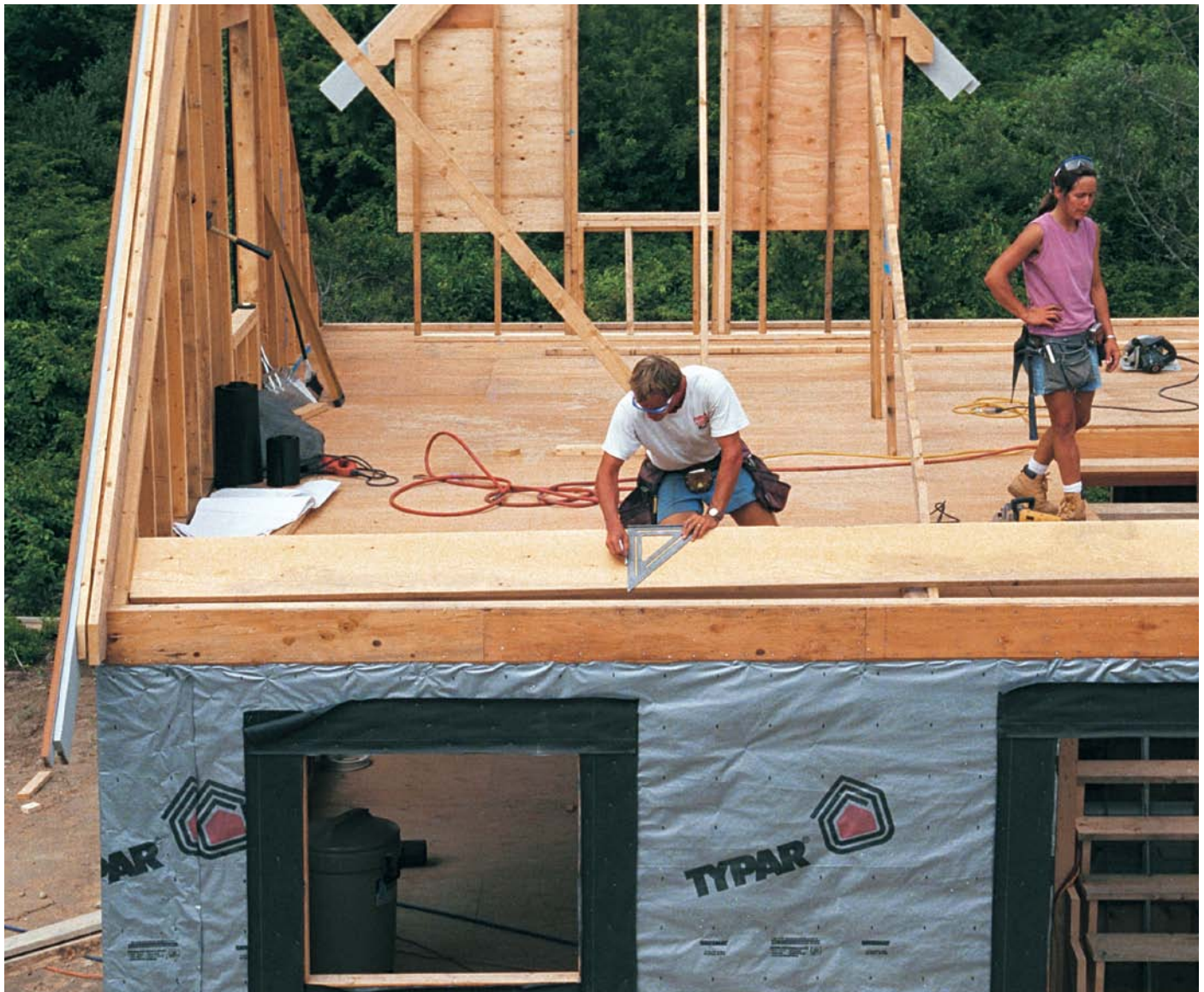
Laying out the ridge. To get the rafter layout to match precisely, the layout on the plates is transferred directly to the ridge stock.
