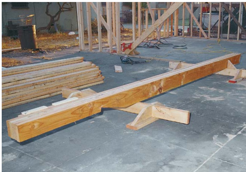
All four hip rafters are laid out and cut at the same time. Short site-built sawhorses hold the rafter stock for layout and cutting. With all of the boards stacked together, only one set of measurements needs to be taken. Templates (see the photos on p. 53) do the rest.
