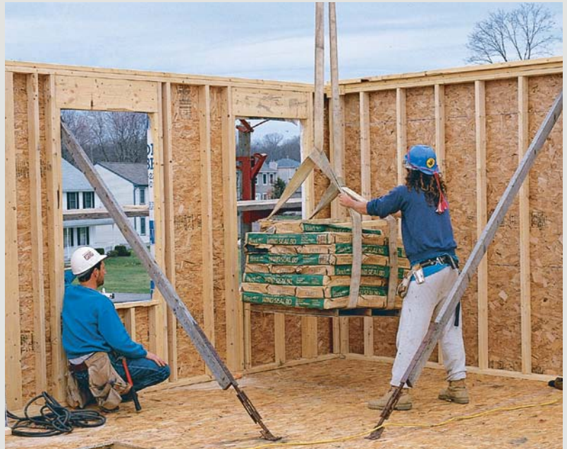
Roof shingles are dropped near a window. The crew member on the left signals the crane operator while the other crew member guides the pallet of shingles to its temporary home.
