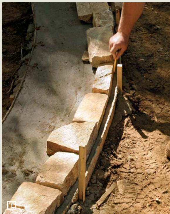
The first course sets the curve of the wall.
