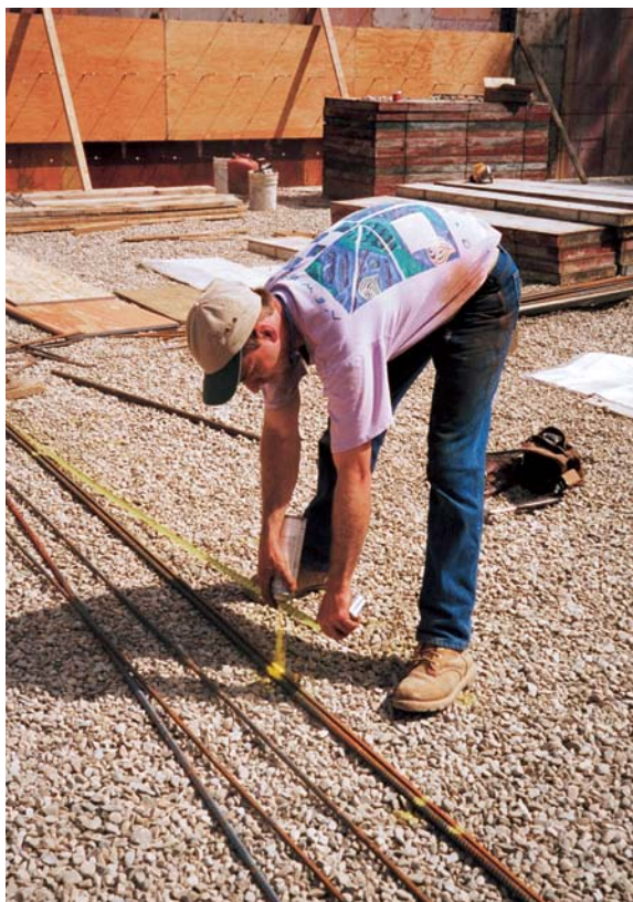
SPRAY PAINT MARKS THE SPOT. A spray can that's made to shoot upside down marks the position of bends or cuts on a piece of rebar. The mark is waterproof, easy to read, and nearly indelible.
