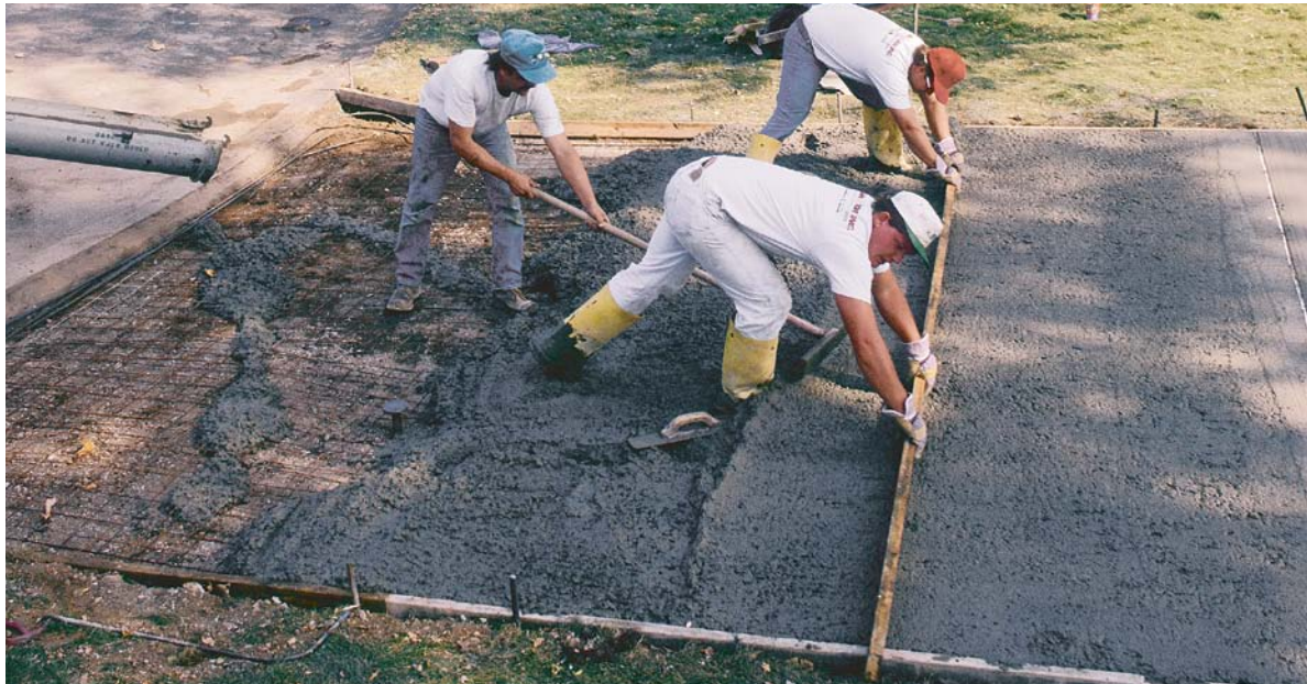
SCREEDING CUTS CONCRETE TO THE RIGHT HEIGHT. A long, straight 2×4 or aluminum box beam is pulled across the surface of the concrete while it is moved in a side-to-side motion. Screeding brings the level of the concrete down to the top of the forms and consolidates it at the same time.
