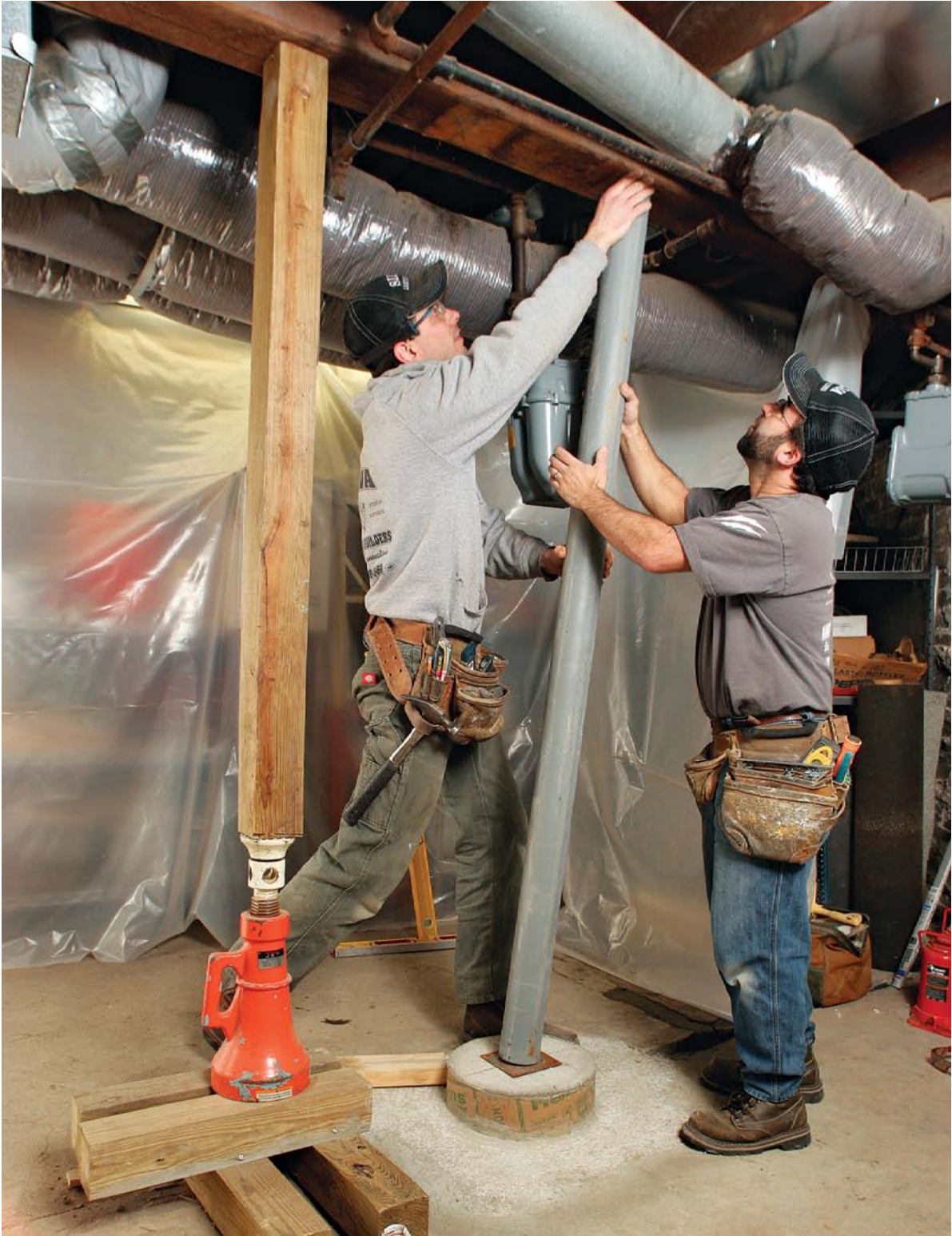
A PROPER FOOTING AND POST add floor support that will never fail again.
