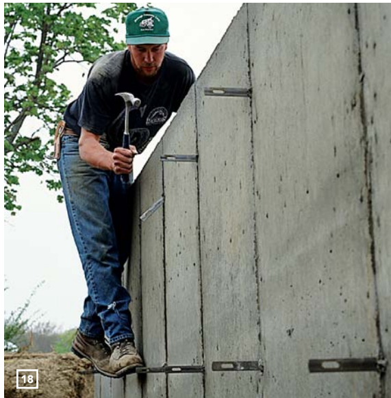
18 THE ENDS OF THE FOUNDATION RODS are then broken off with a hammer.
