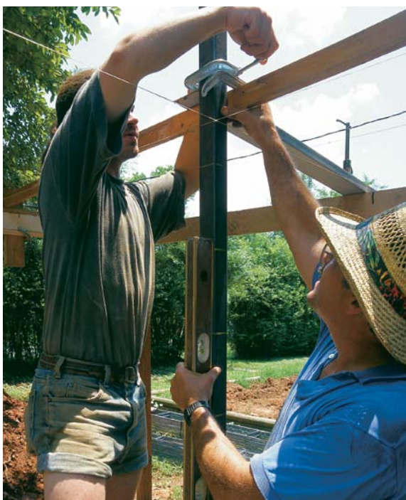
MEASURE FROM THE TOP DOWN. Steel story poles at the outside corners of the block foundation are nailed to the footings, held in place with 1×4 braces, and mark the corners of the foundation and the courses of block. String lines between the house and the poles mark the foundation height.
