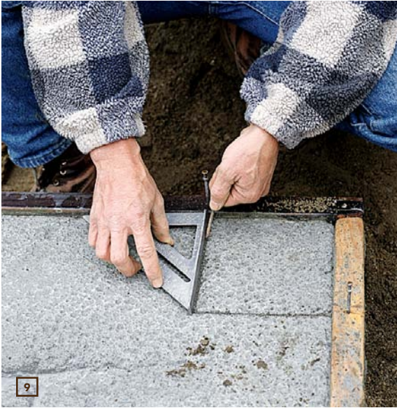
9 FOUNDATION CORNERS ARE MARKED ON TOP. While the concrete is still green, the corner of the foundation is marked on the footing.
