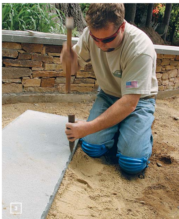
Chisel the outside edge.
