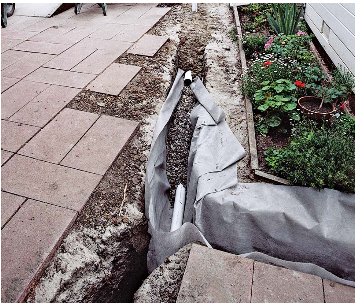
TWO PIPES. To drain a structure, remove subsurface water moving through the soil as well as runoff. The perforated pipe at the bottom of the trench (holes oriented downward) carries off the former. The top pipe carries away surface runoff from downspouts and drains. The pipe stub projecting above the tamped earth will attach to an area drain.
