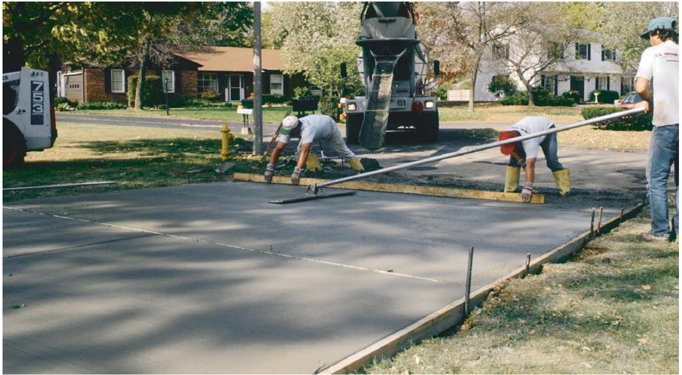
A BULL FLOAT SMOOTHS THE CONCRETE AND FILLS VOIDS. As the crew member in the foreground pulls the wide blade of the bull float over the concrete, surface tension is created, bringing water to the surface and filling in imperfections from screeding.
