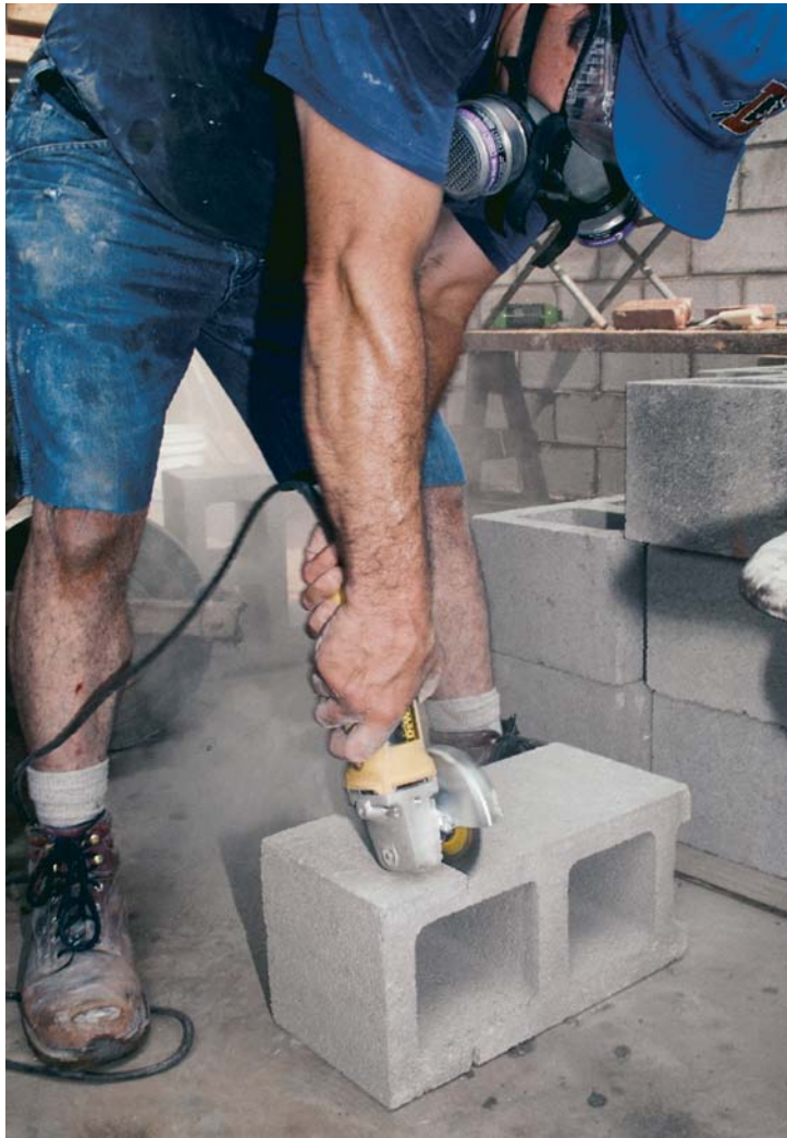
A GRINDER MAKES A CLEAN CUT. To avoid ragged edges in cut blocks, use a grinder equipped with a diamond blade, and give the block a tap with the hammer to get a clean split. This procedure is messy, however, so a respirator and eye protection are important.
