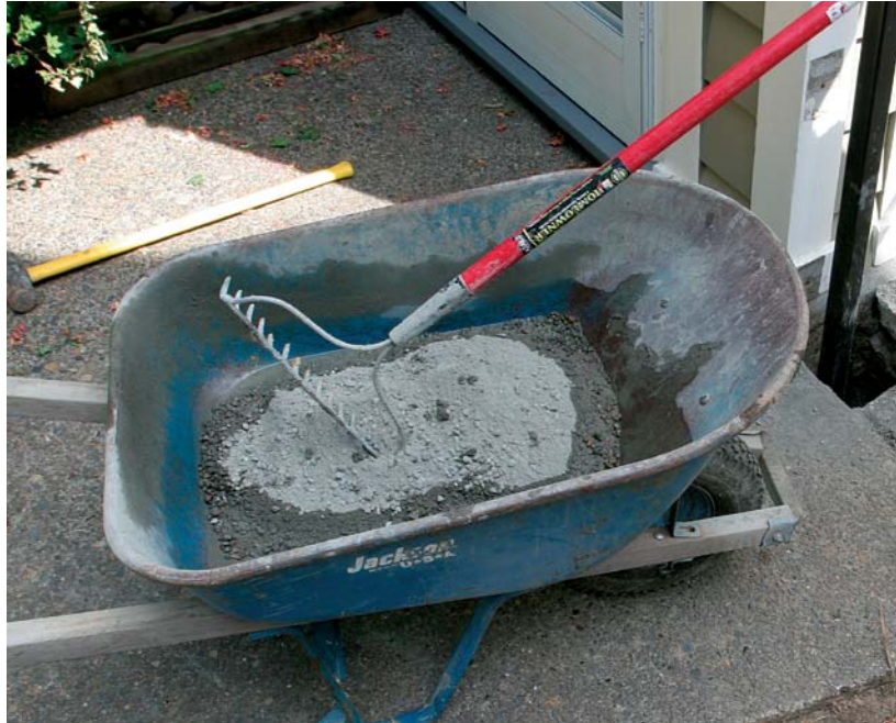
a common garden rake is the ideal tool for mixing small batches of concrete.
