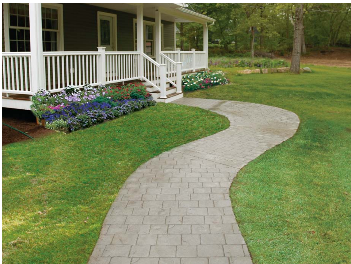
FORMING, POURING, AND STAMPING a concrete walkway creates an inviting path to any front door.
