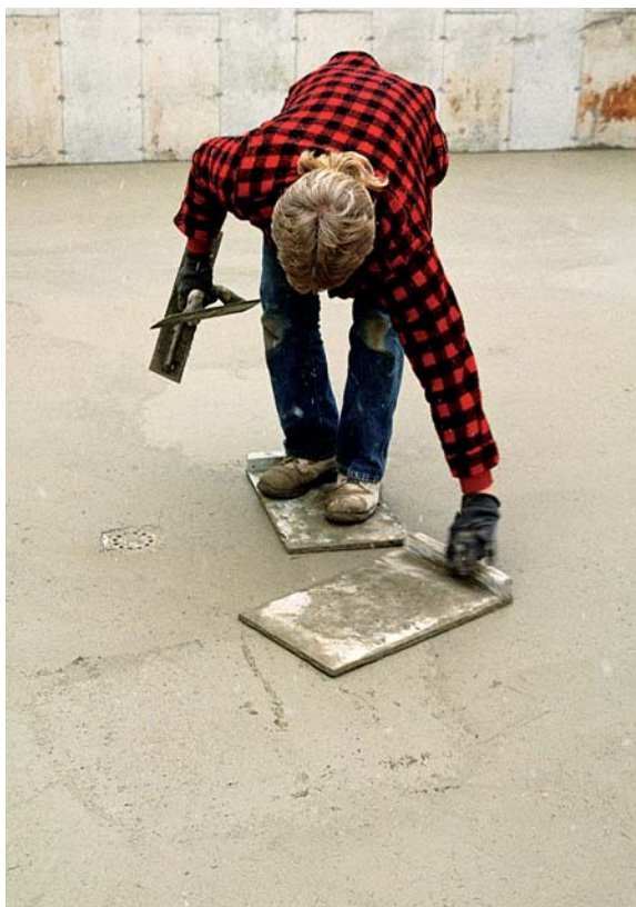
CEMENT SHOES. Knee boards—pieces of plywood with strips of wood on one edge—allow you to move around on fresh concrete without sinking in because the boards distribute weight over a large surface area. Concrete finishing is done from knee boards while the concrete is in a plastic state, meaning it's neither liquid nor solid.
