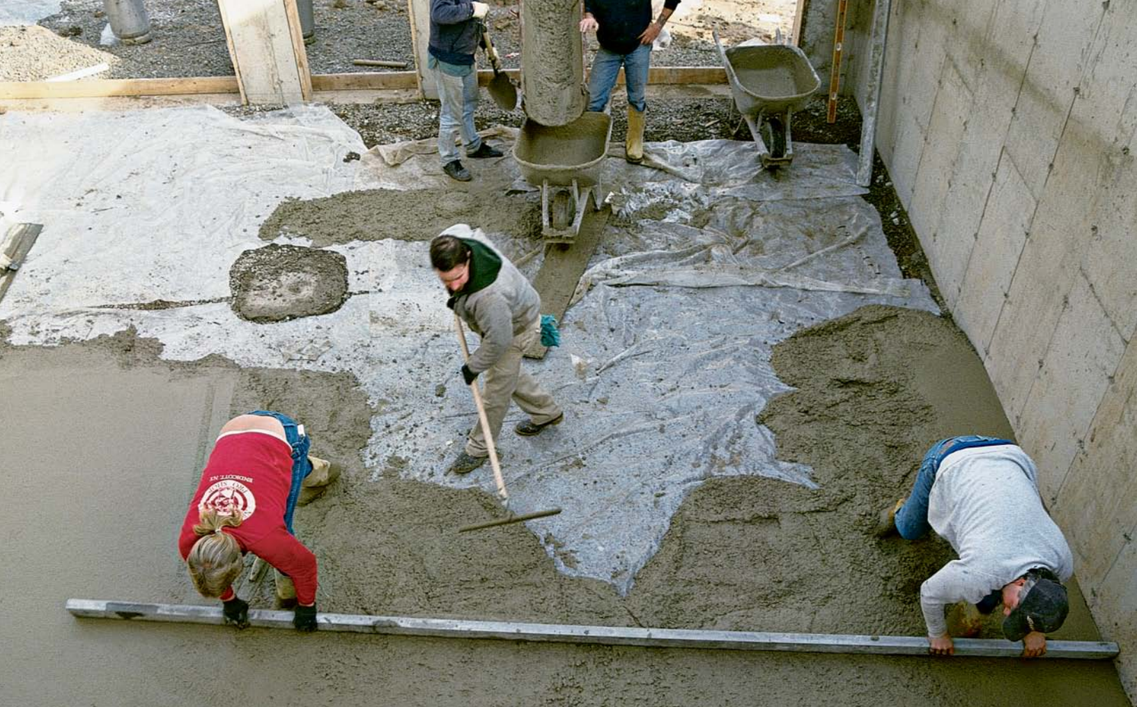
USING A SCREED RAIL. Two workers use a magnesium straightedge, or screed rail, to level freshly placed concrete. The ends of the rail glide over previously leveled concrete strips, called wet screeds. A third worker rakes the concrete behind the screed rail to adjust for high and low spots.
