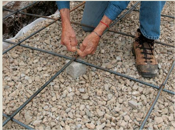
A REBAR GRID WORKS BETTER than steel mesh to prevent cracks. Held together with tie wire, a rebar grid set on 2-in.-tall concrete spacers stays put during the pour and the screeding. Wire mesh often ends up at the bottom of the slab, where it can't provide structural support.
