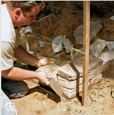
Corners anchor the wall.
