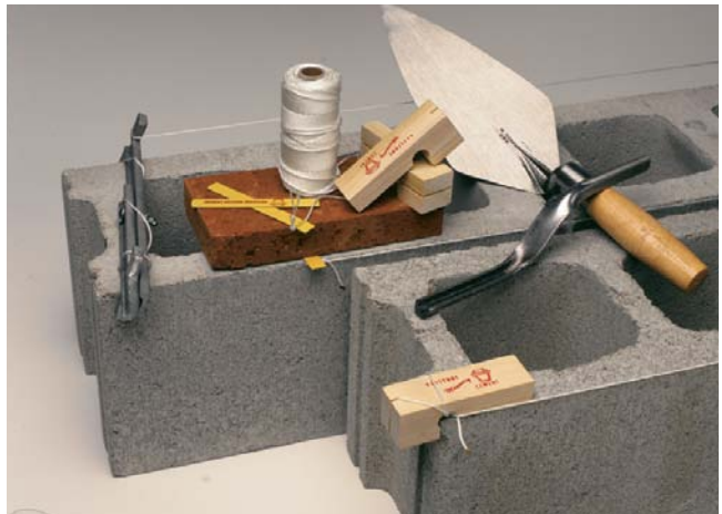
THE BASIC TOOLS FOR WORKING WITH CONCRETE BLOCK. To get started laying up block requires a trowel, a pointing tool, line blocks, and string (mason twine). Also helpful are line stretchers (left) and twigs, shown next to the string.
