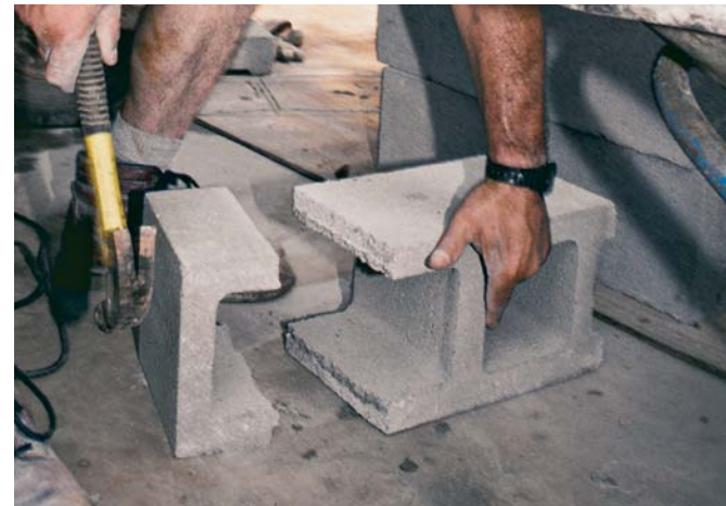
A GRINDER MAKES A CLEAN CUT. To avoid ragged edges in cut blocks, use a grinder equipped with a diamond blade, and give the block a tap with the hammer to get a clean split. This procedure is messy, however, so a respirator and eye protection are important.
