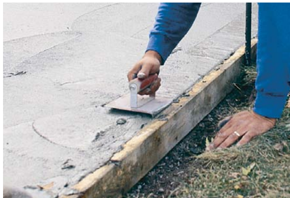
WORKING THE EDGES. A crew member with a flanged edging tool works along the perimeter of the slab to consolidate material and to rough-cut the rounded edge.
