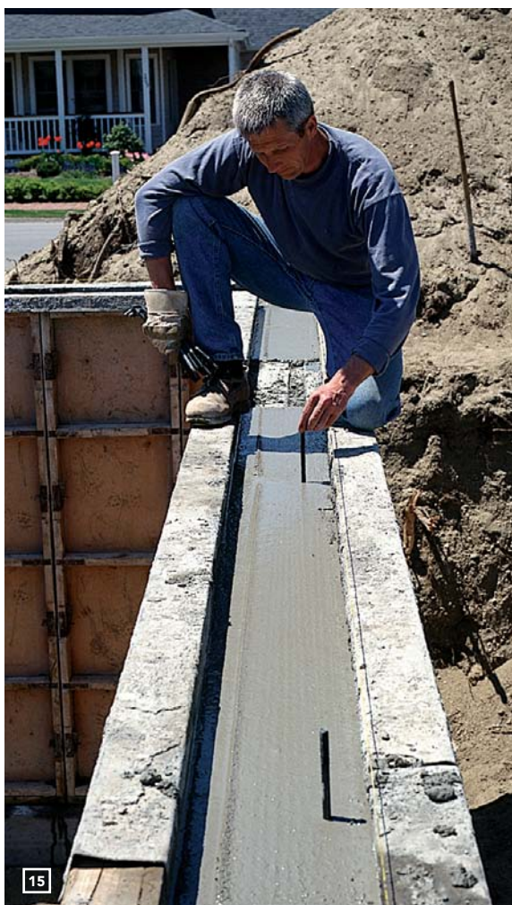
15 ANCHOR BOLTS ARE INSERTED while the concrete is still soft.
