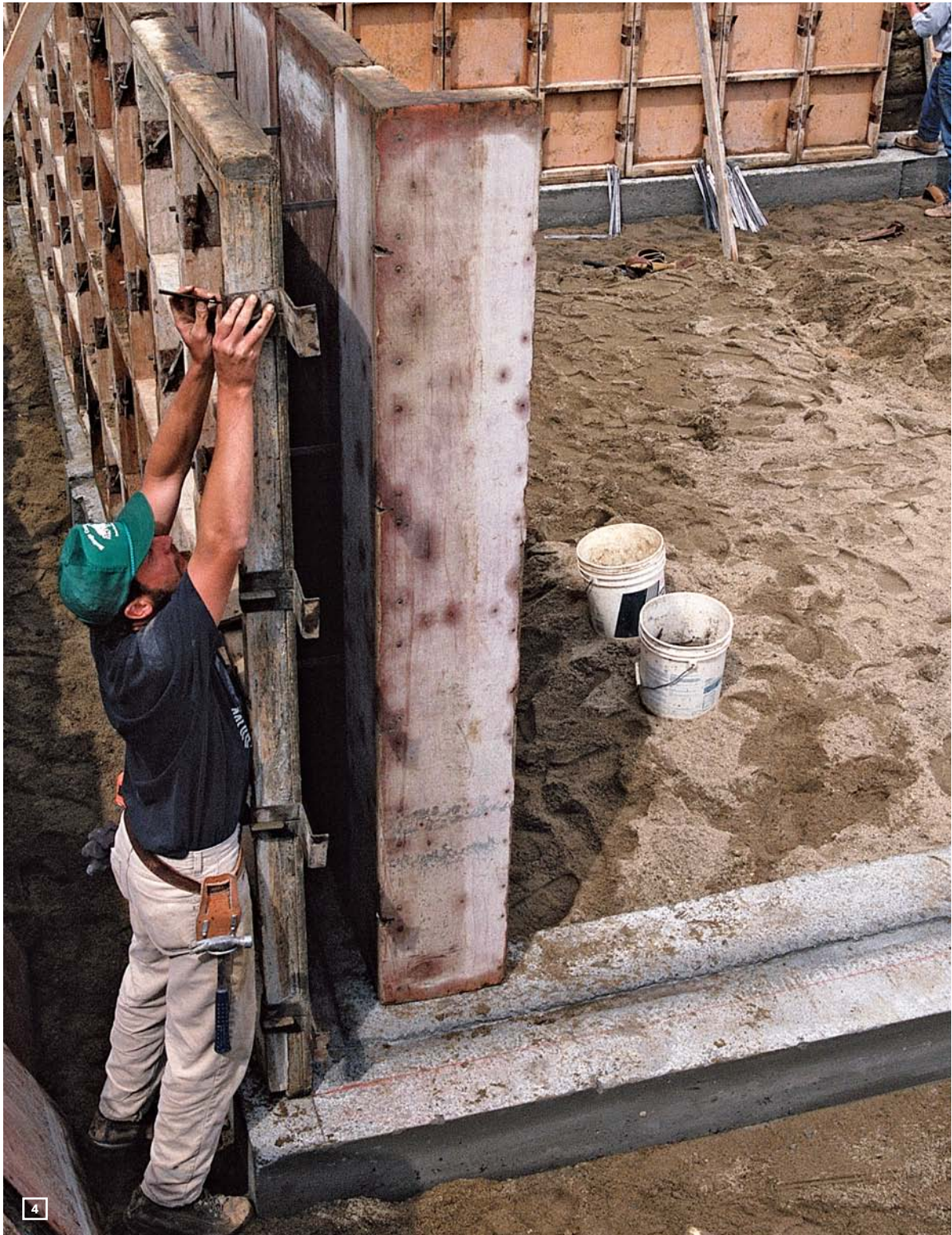
4 FORMING STARTS IN A CORNER that uses a right-angle form for the inside and special brackets for the outside.
