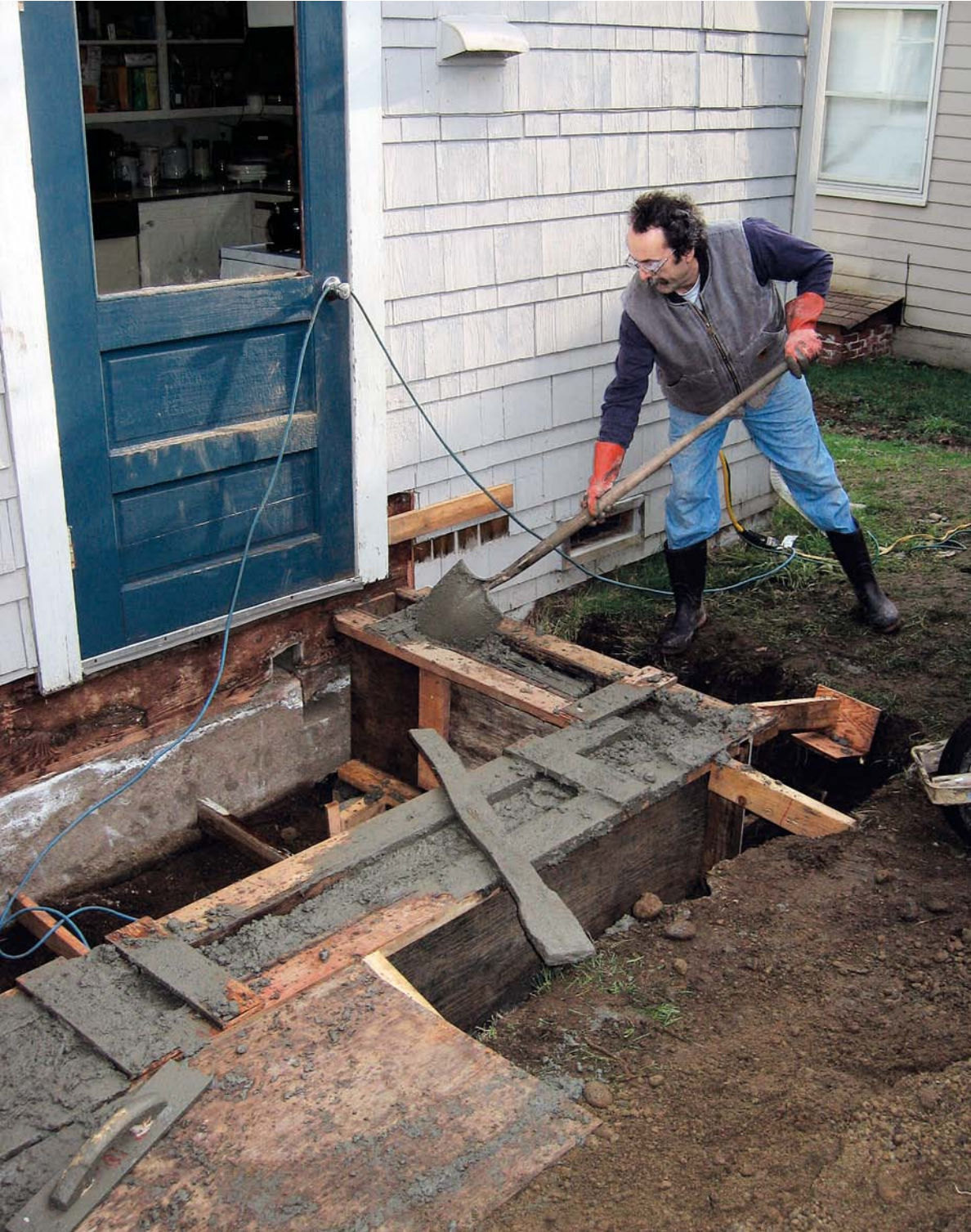
FOR SMALL JOBS, you can save time and money by pouring the footings and foundation at the same time—but there are some pitfalls to be aware of.
