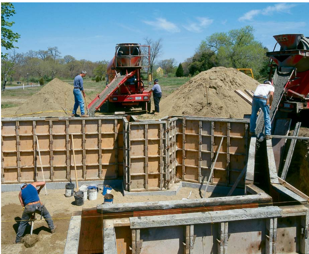
THIS FORM SYSTEM, preferred by the authors, includes form panels that can be reused many times, depending on how they are handled.
