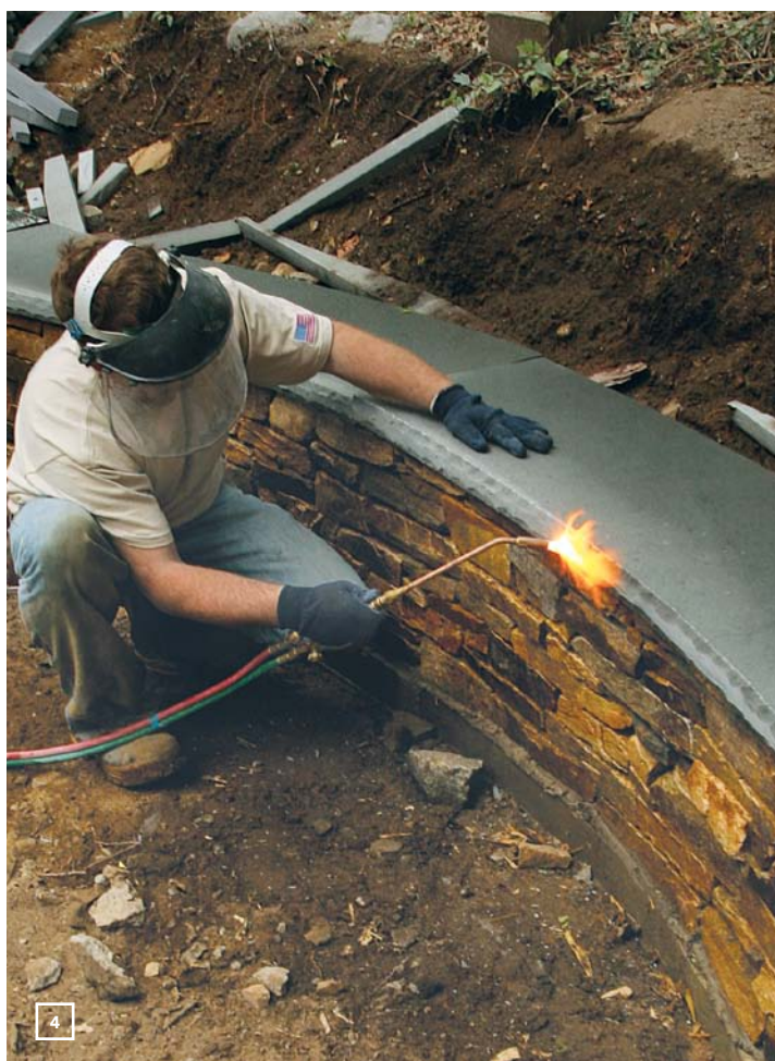
Torch the chiseled edge.
