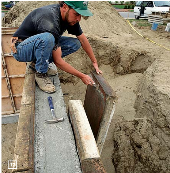
17 AS EACH FORM IS REMOVED, excess concrete along the top is scraped off.
