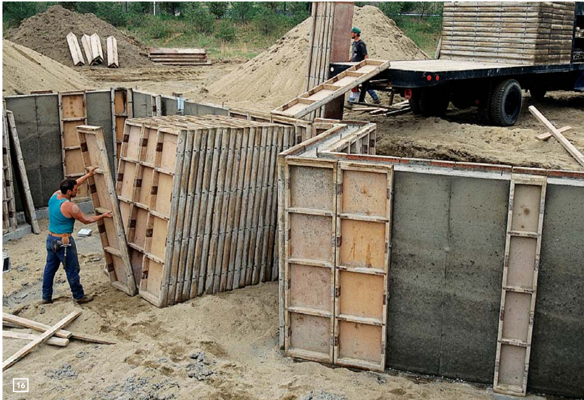
16 FORMS ARE STRIPPED and carried to the truck. After the concrete has cured overnight, the crew strips off the forms and takes them to the truck to be stacked.
