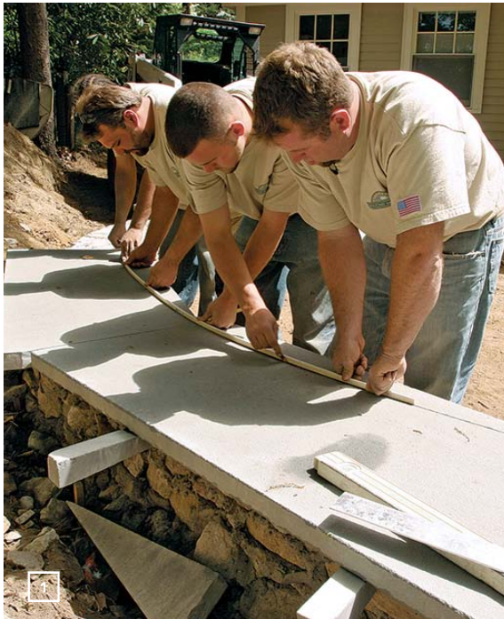
Determine the overhang.
