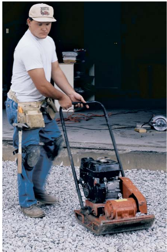
RECYCLED CONCRETE FORMS THE SUBBASE. Coarsely crushed concrete is compacted to provide a drainage layer and a capillary break to prevent moisture from wicking up.
