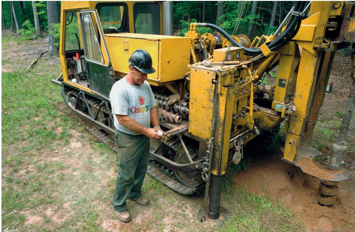
FINDING OUT WHAT'S DOWN THERE. Taking samples from a series of drillings enables engineers to determine subsurface soil characteristics.
