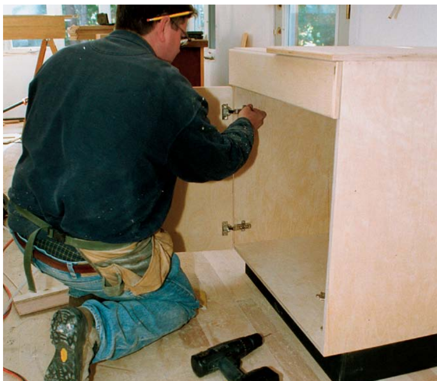
If holes have been drilled correctly , hinges installed on cabinet doors should snap easily into place on the base plates. These hinges allow the author to fine-tune the fit of the door.
