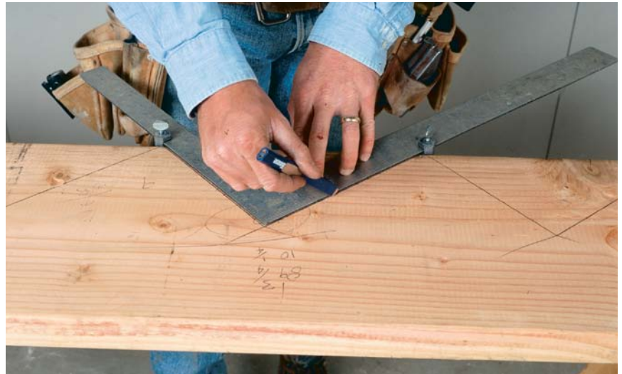
Stair gauges streamline layout. Small clips called stair gauges are attached to the framing square at rise and run measurements to keep the orientation of the framing square the same for each step layout.
