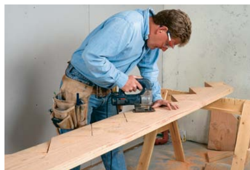
Finishing the cut. A jigsaw is used to complete the cuts in each corner, cutting the wood that the circular saw can't get. A handsaw will also work instead of a jigsaw.
