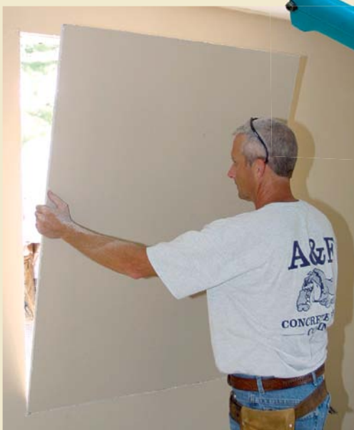
The wallboard comes out, making way for the new window.
