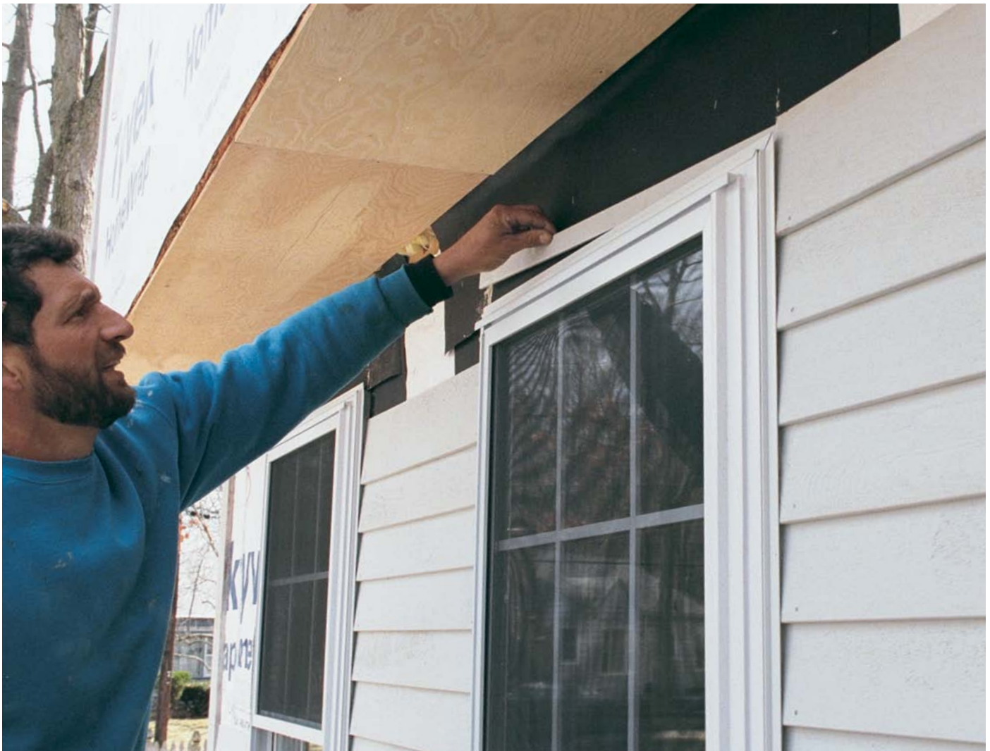
The top of a clapboard fills the space above the windows. This keeps the next course from bowing inward as it's nailed. With vinyl windows such as these, the authors leave a \frac{1}{16} -in. to \frac{1}{8} -in. expansion gap between the windows and the clapboards and caulk it.
