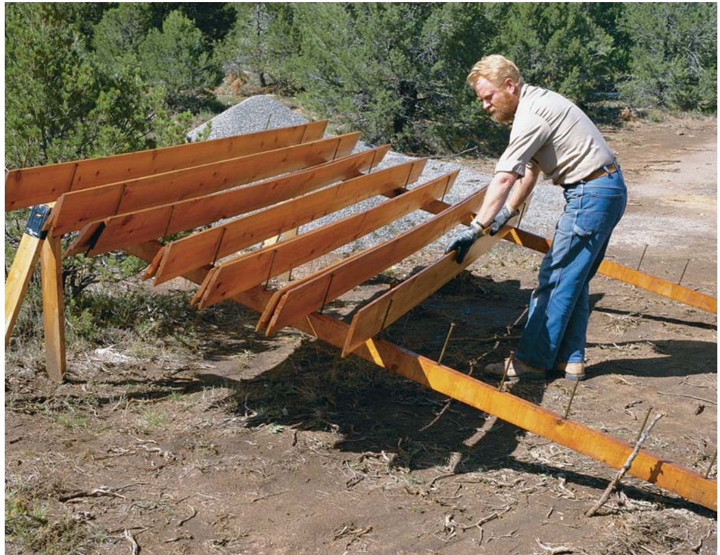
Drying rack. A pair of tilted 2x4s with 80d nails supports the siding as it dries.
