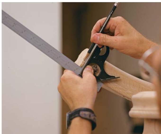
Using a combination square to transfer the railing angle to the fitting. The author aligns the square's blade with the string (top) and marks the tangent on the fitting. Maintaining the blade angle (bottom), he flips the head over and draws the correct angle.
