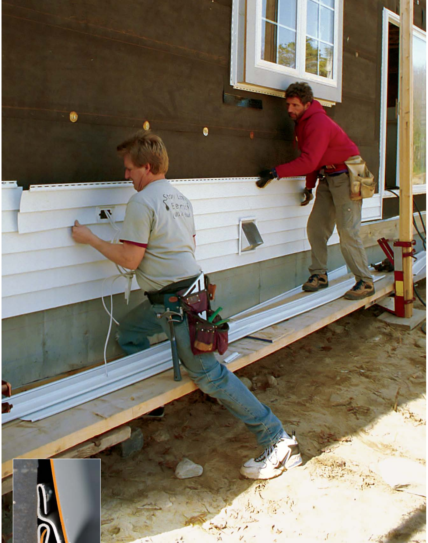
Pushing up locks panels together. The bottom edge, or butt, of one panel clicks into the locking channel at the top of the preceding course, and the siding goes up.
