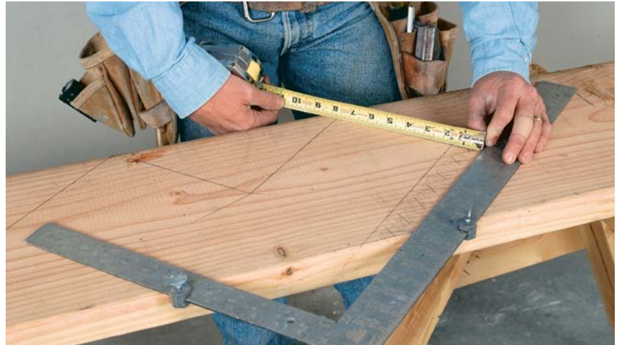
Subtract the thickness of a tread. For the bottom rise to be the correct height, the thickness of one tread must be subtracted from the bottom of the stringer. Moving the square to the other side of the stringer makes it easier to complete the lines.
