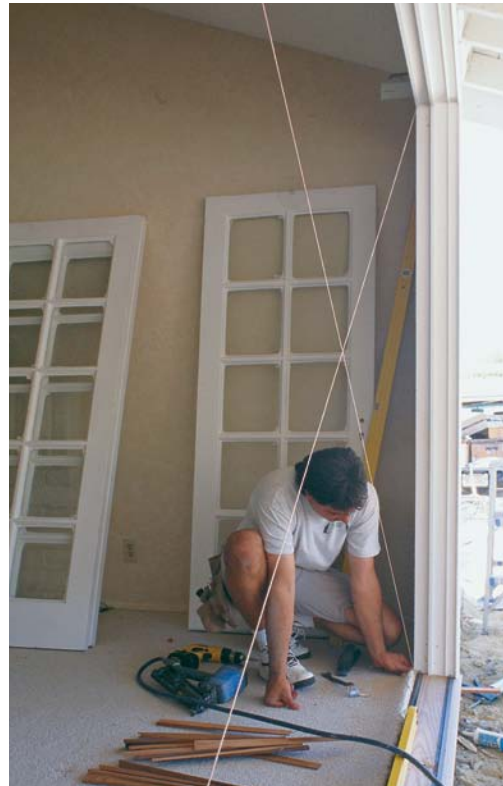
Checking for cross-legged jambs. Strings stretched from corner to corner will touch in the middle if the jambs are in precisely the same plane, which ensures the door slides smoothly.
