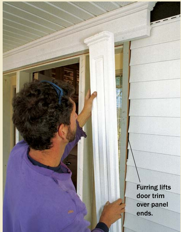
Door trim replaces J-channel. At a front door, a furring strip lifts the door trim enough to let siding panels tuck in behind.
