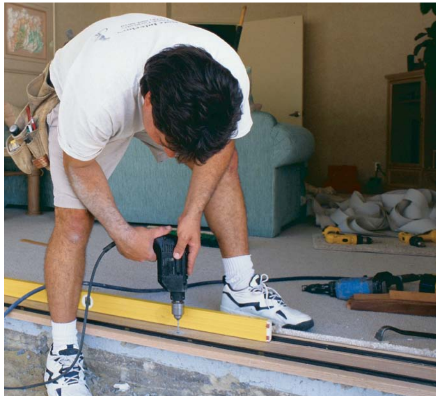
Drill anchor holes during the dry fit. After the frame has been tested in the opening, anchor holes are drilled through holes in the sill with a masonry bit.
