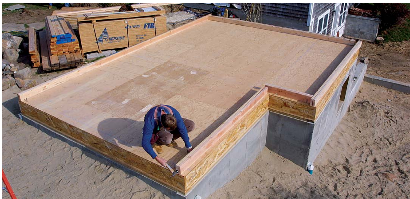
Plates on deck. When wall positions are laid out, cut all the top and bottom plates (the long horizontal members) for the exterior walls, and place them on their layout lines.
