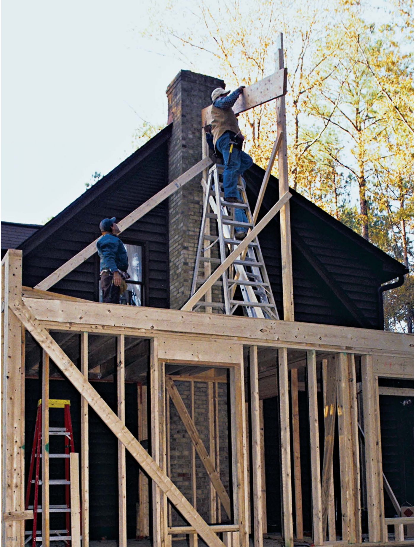
Setting the ridge. Temporary posts are set up to hold the ridge at the right height. The posts are braced 2x4s with a 2x4 scrap nailed to the top that rises 10 in. above the top of the post. The ridge is set on top of the post and nailed to the scrap of wood.
