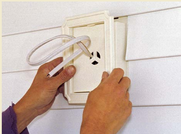
Utility boxes create receiving channels. A snap-on molding holds panel ends around a light box near the front door.
