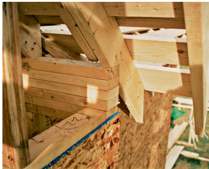
Additional top plates provide bearing for the kickout's 2x6 rafters while picking them up enough to line up the fascia boards.
