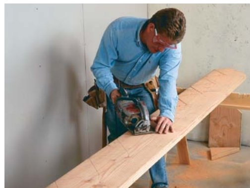
First cuts are made with a circular saw. Overcutting the lines will weaken the stringer, so the initial cuts with a circular saw should never extend beyond the layout lines.
