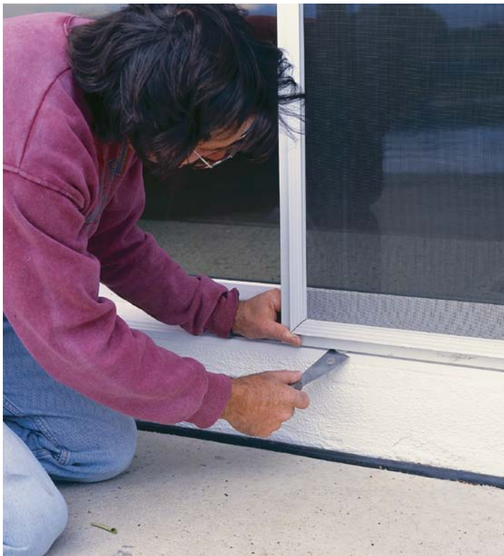
A putty knife puts screen wheels on track. If the screen panel rides on spring-loaded wheels, a stiff putty knife can be used to depress the wheel and guide it onto its track.
