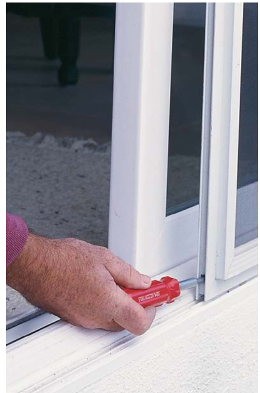
Screws adjust the screen wheels. Screws in the edges of the screen adjust the height of the spring-loaded wheel as well as the tension on the springs to keep the screen from binding.
