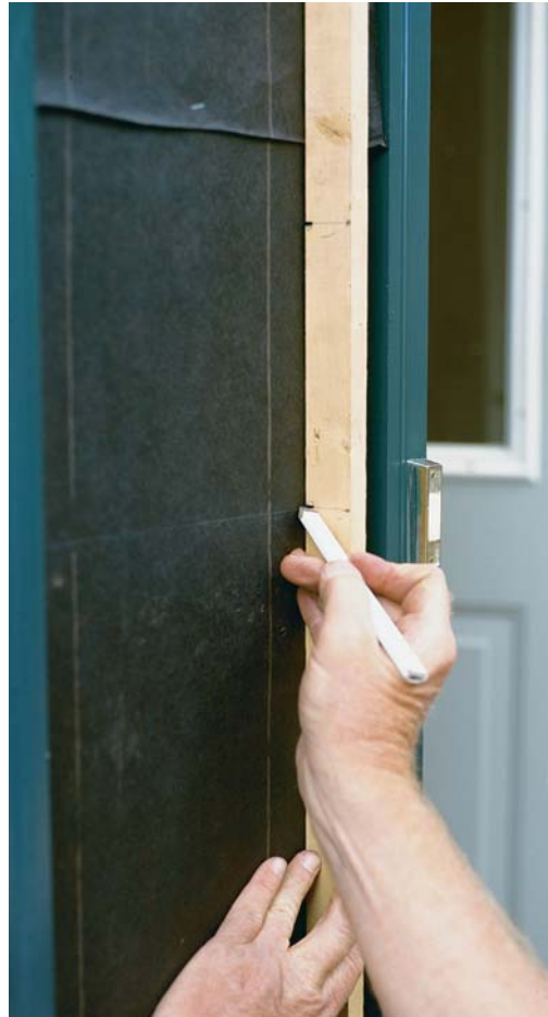
Layout pole. The author uses a water level to locate the bottom courses of siding on all the walls. Then he marks the subsequent courses with the help of a 12-ft. stick with saw kerfs that correspond to the tops of the siding boards.
