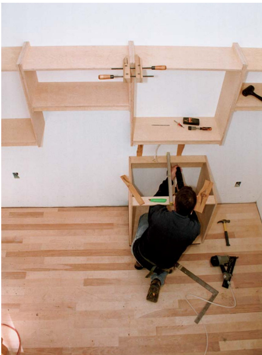
To make leveling them easier, the author installs the bases separately from the cabinets. With the bases secured, he then sets the cabinet boxes in place and screws them to the wall.
