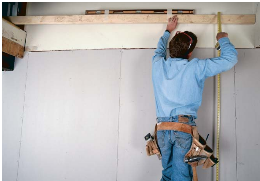
Measuring the overall rise. A 2x4 extends a 4-ft. level over to where the staircase will land. Measuring the rise at this point minimizes the chance of error from a basement floor that might not be level.
