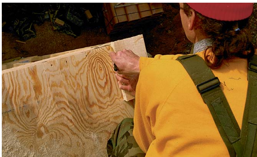
2x6 template. A 2x6 block is used to mark an exterior wall's width on the plywood deck. The author sights down to the floor below to make up for possible irregularities in the alignment of the floor joists.
