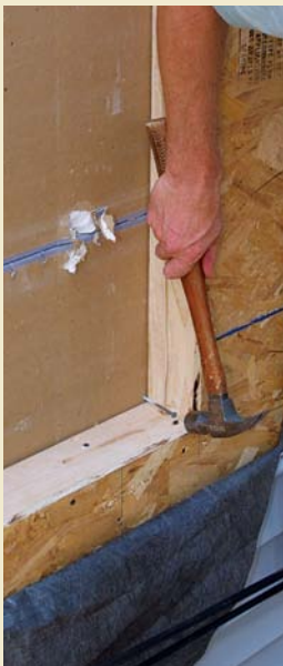
Nails driven into the corners from the outside transfer the opening to the inside.
