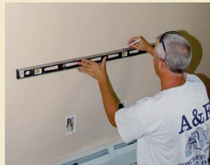
Inside, the corners are connected and the opening is drawn.
