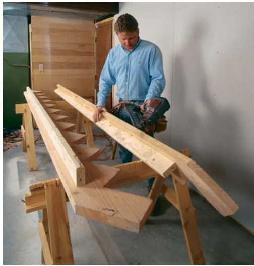
Strongbacks stiffen the stringers. Strongbacks, or 2x4 stiffeners, are nailed to the sides of the stringers to keep them from flexing.
