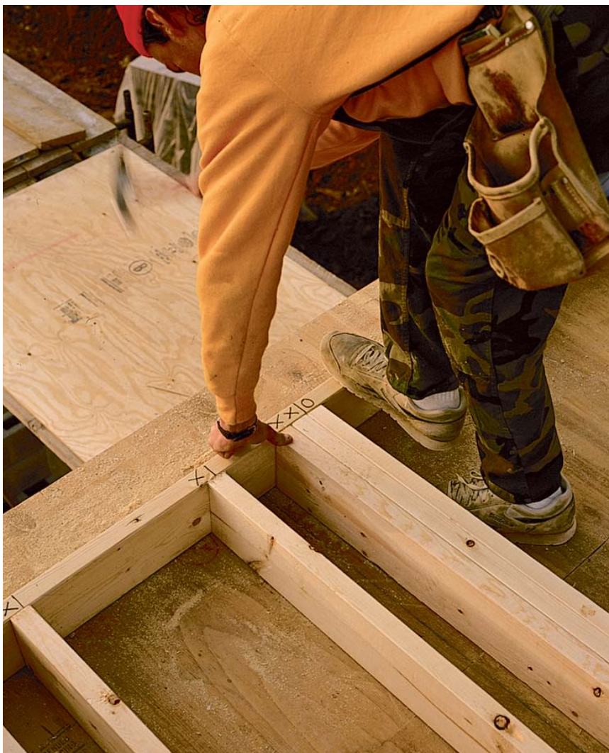
Through-nailing. As in other methods of framing, the author prescribes through-nailing the bottom of the studs, the jacks, and the cripples. As he works his way down the plate, he aligns each component to its mark and nails it.
