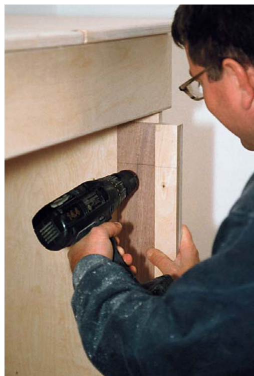
A jig locates screw holes for hinge plates inside the lower cabinets.
