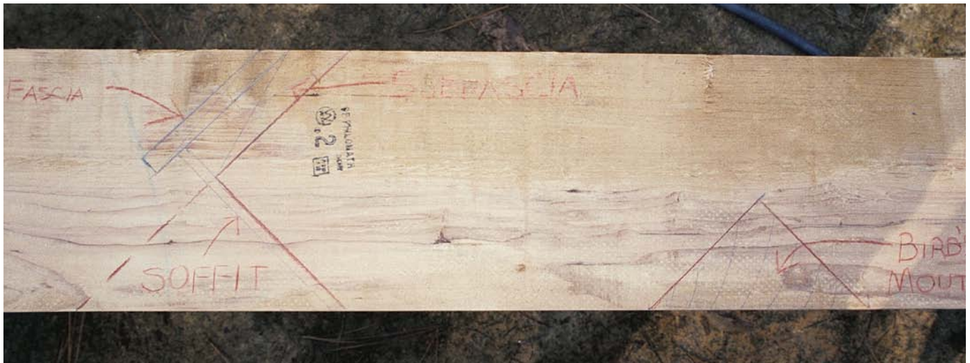
Visualizing the bird's mouth and rafter tail. Red lines on this marked-up rafter show where cuts will be made for the bird's mouth, at right, and rafter tail, at left. To determine the correct cut for the tail, the author marked out the subfascia, soffit, and fascia board.
