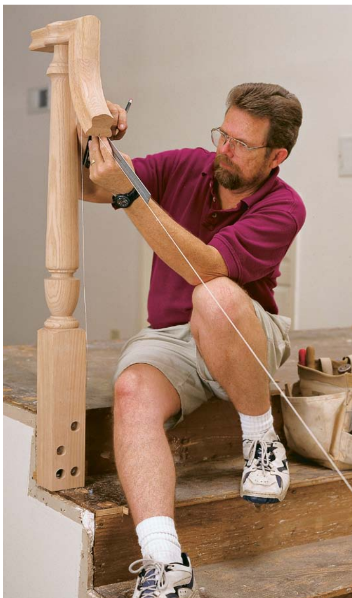
Taut string establishes the angle and height of the railing. The author fastens a stringline with tape between two fittings to check the position of the railing and to determine the proper angle at which to cut the fittings
