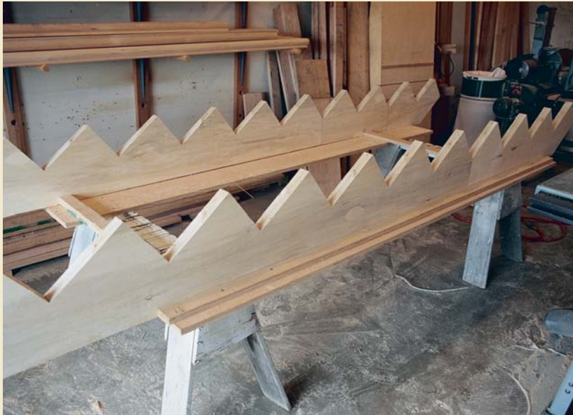
Assembly jig holds the stringers parallel and square. A simple jig made from strips of plywood holds the stringers at the proper width while the author is attaching treads and risers.
