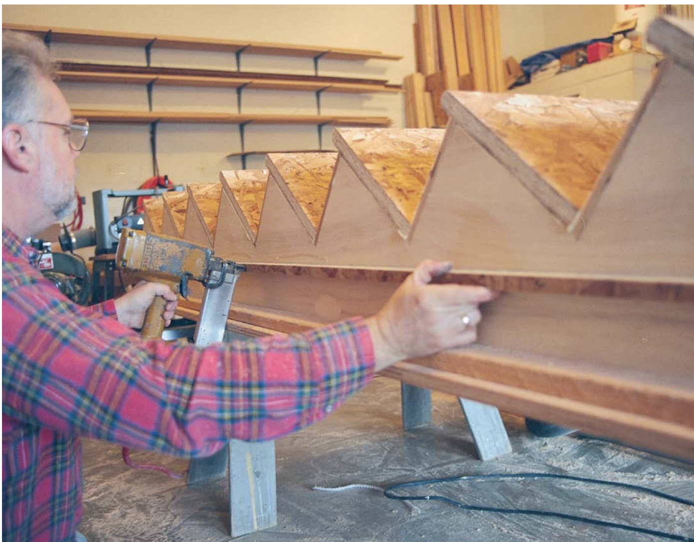
A spacer strip allows room for drywall. A 1-in. strip stapled to the stringer will keep the stringer away from the wall studs so that drywall can be slipped in behind the stringer after the stairs are installed.
