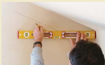
Draw a level line from the corner.
