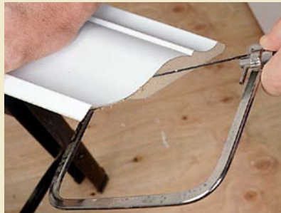
Back-cut the cope , to ensure a tight joint.
