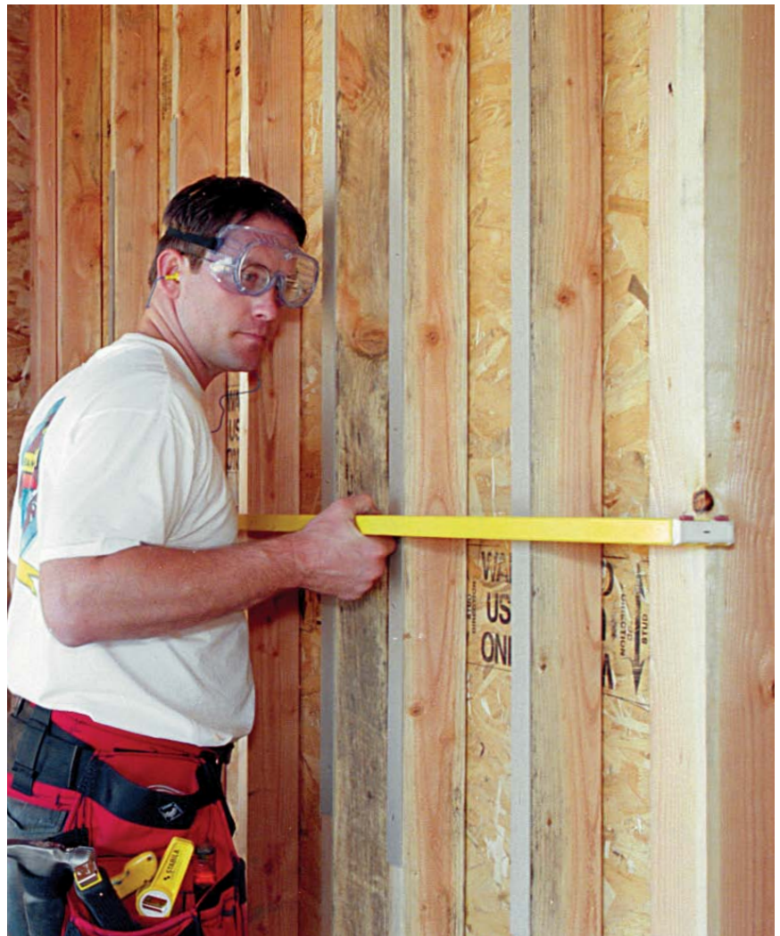
Checking the plane of the wall. After the offending studs have been planed and shimmed for vertical straightness, the author then checks across the studs to see how they line up horizontally.
