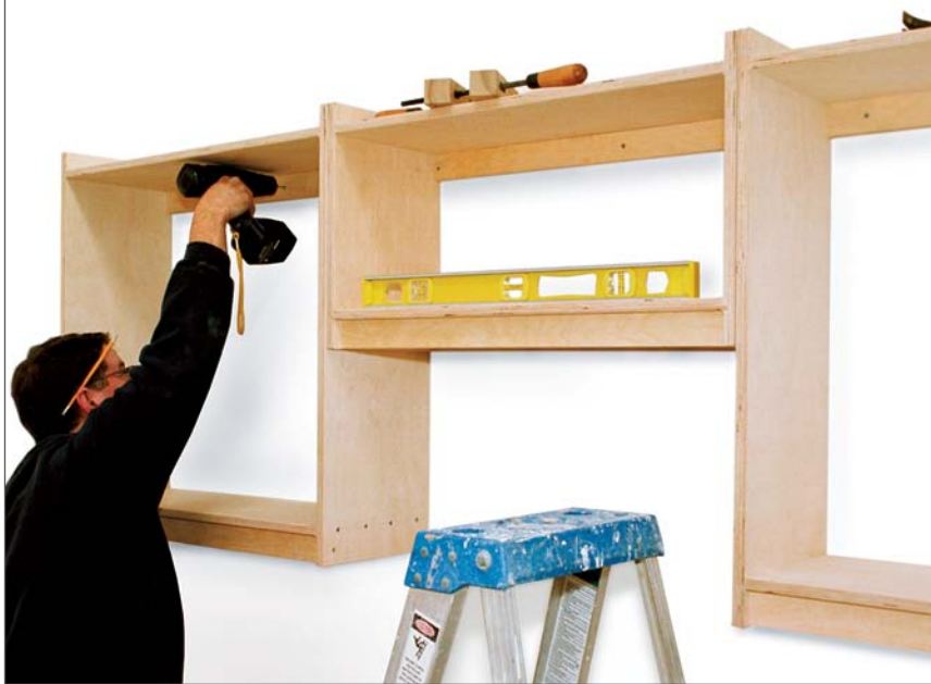
After marking stud locations, the author hangs upper cabinets. Without backs and doors, these boxes are light enough for one person to hold in place as they are screwed to wall framing.
