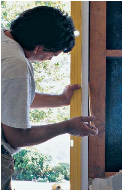
Shims bring the jamb out to the level. After the sill is leveled and the jambs are plumbed top to bottom, shims are inserted behind the jamb until the jamb touches the level.
