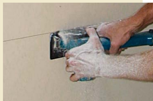
A trim saw with a carbide blade cuts the wallboard with minimal mess.
