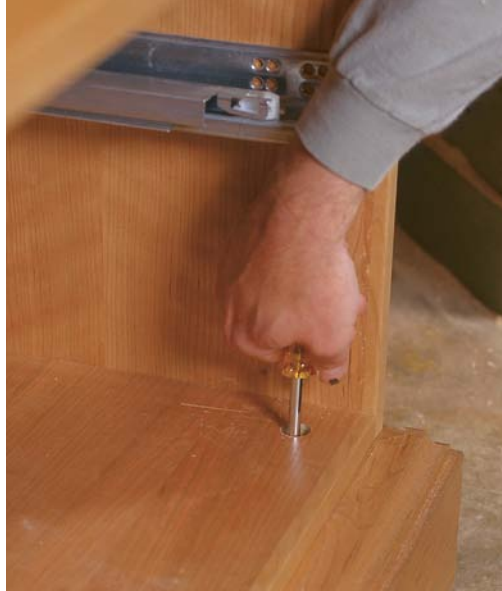
Hidden levelers ease installation. After assembling the entertainment center in the house, the author adjusts the levelers through holes that will be concealed by drawers.
