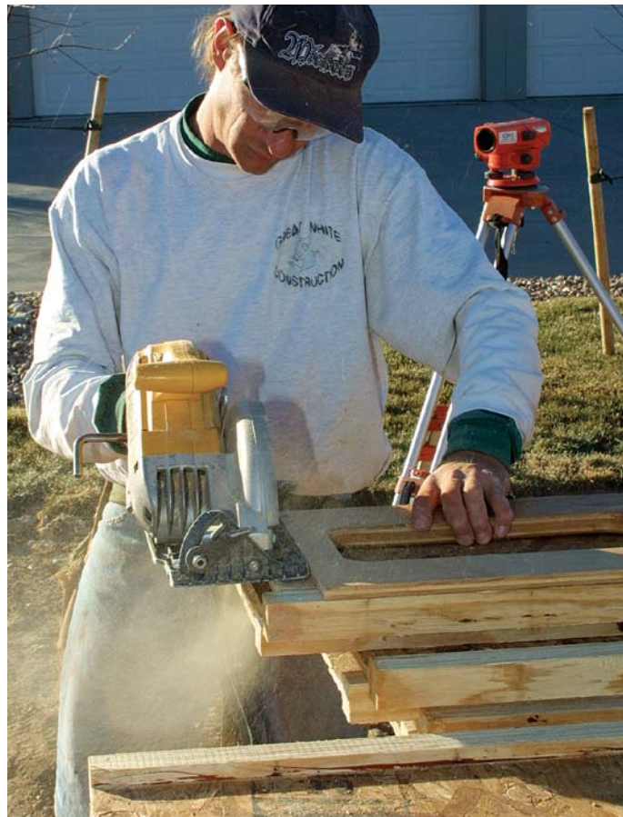
Square one end of each joist while sorting and stacking. Because I-joists are cut to approximate length at the lumberyard, it is easier just to square one end as you are sorting them.
