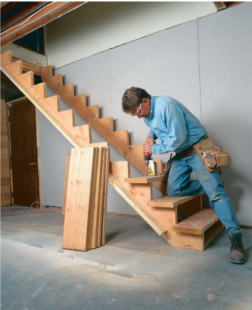
Treads are attached with screws. Screwing the treads to the stringers is the best way to keep the staircase from squeaking. Predrilling the holes prevents the screws from snapping while they're being driven.
