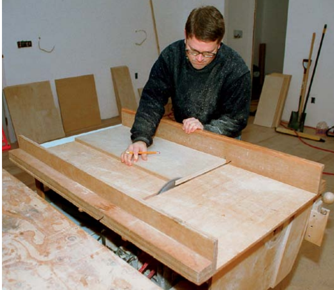
A tablesaw cutoff box ensures that cabinet parts will be square. When working with Baltic birch, don't assume that factory edges are square.
