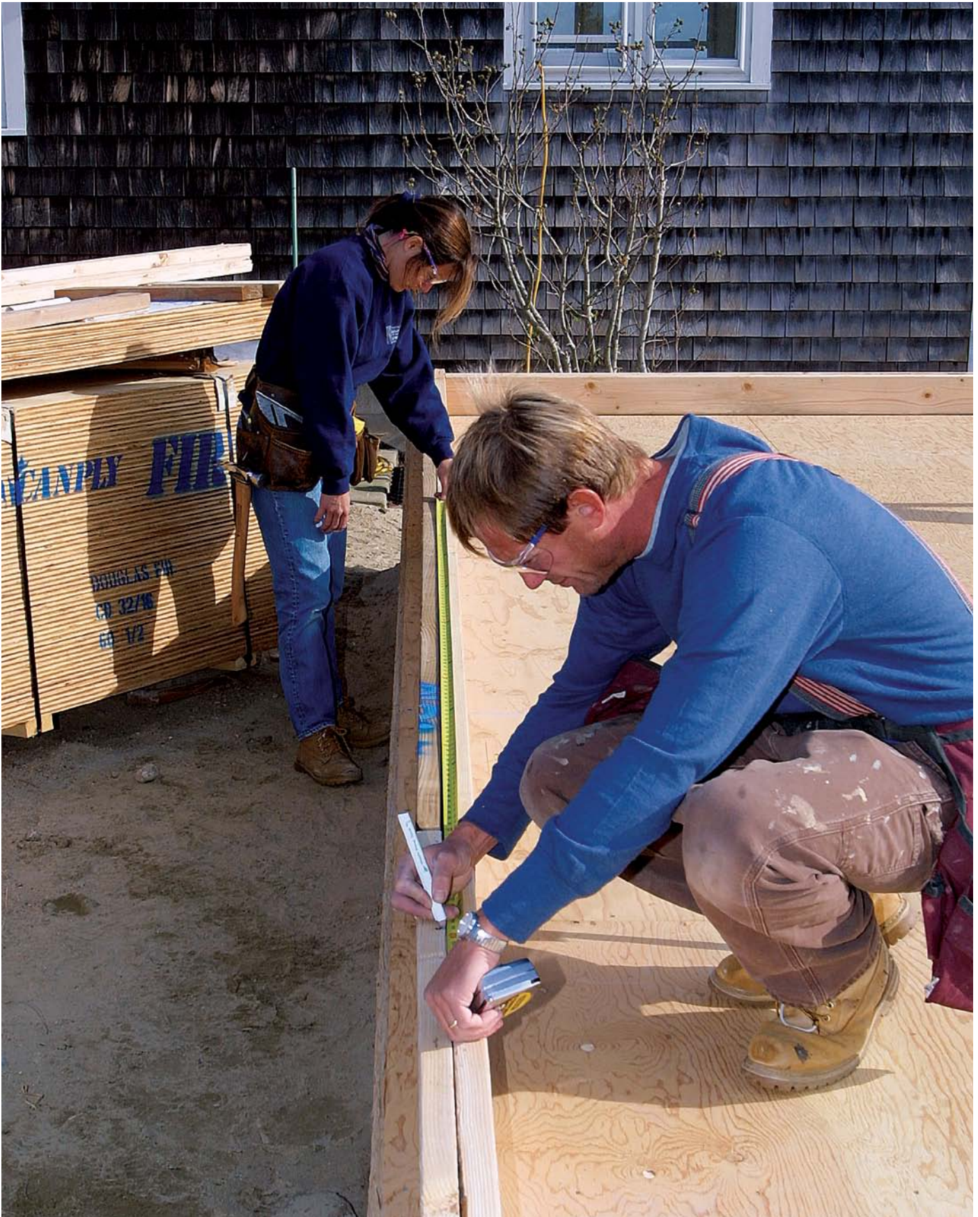
Everything from rafters to kitchen cabinets fits better when you get the walls square and the studs in the right places.
