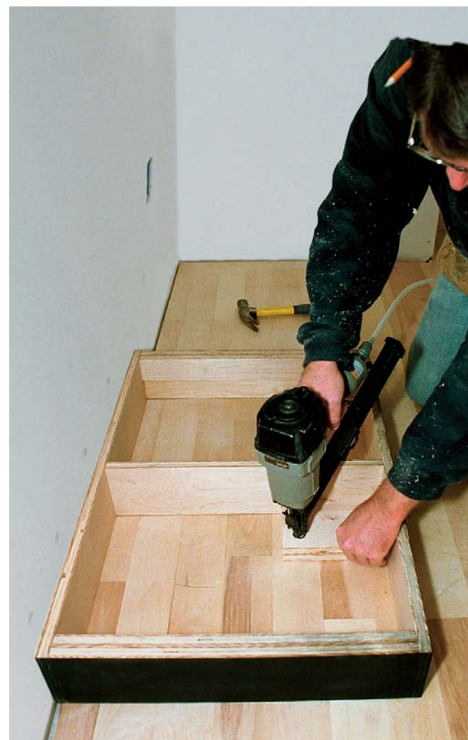
To make leveling them easier, the author installs the bases separately from the cabinets. With the bases secured, he then sets the cabinet boxes in place and screws them to the wall.
