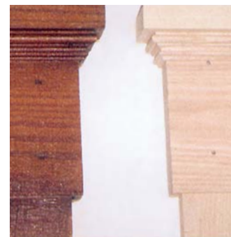
A tablesaw and a shaper were used to make ash molding (right) that matches the original chestnut trim (left).
