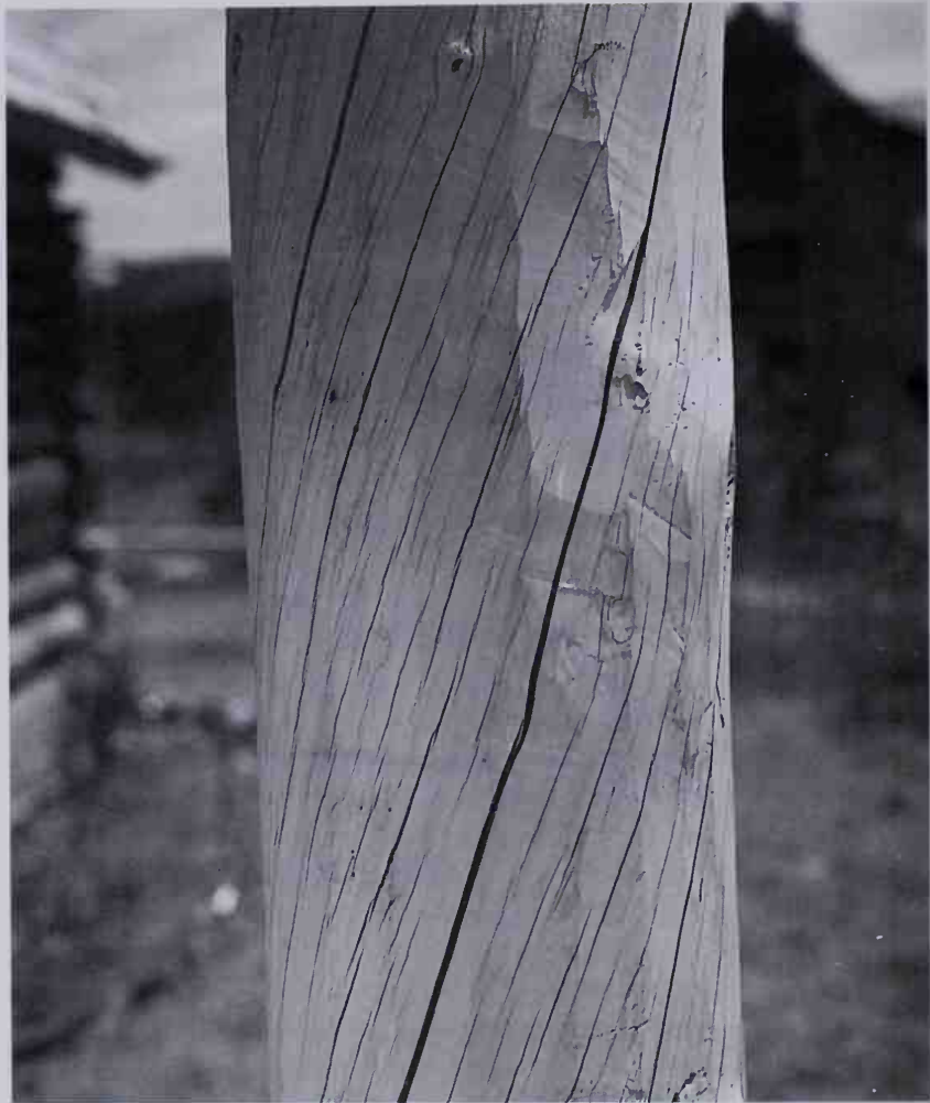
The radial checks in this fir post indicate that the tree grew in a spiral motion as it followed the daily movement of the sun.
