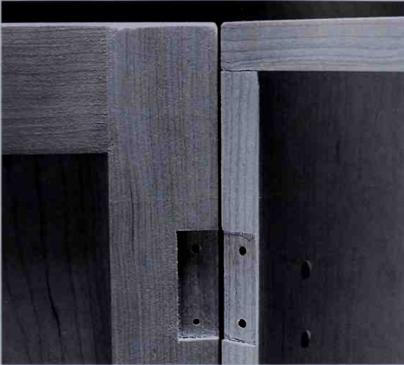
The completed hinge mortises in the cabinet door and carcase.
