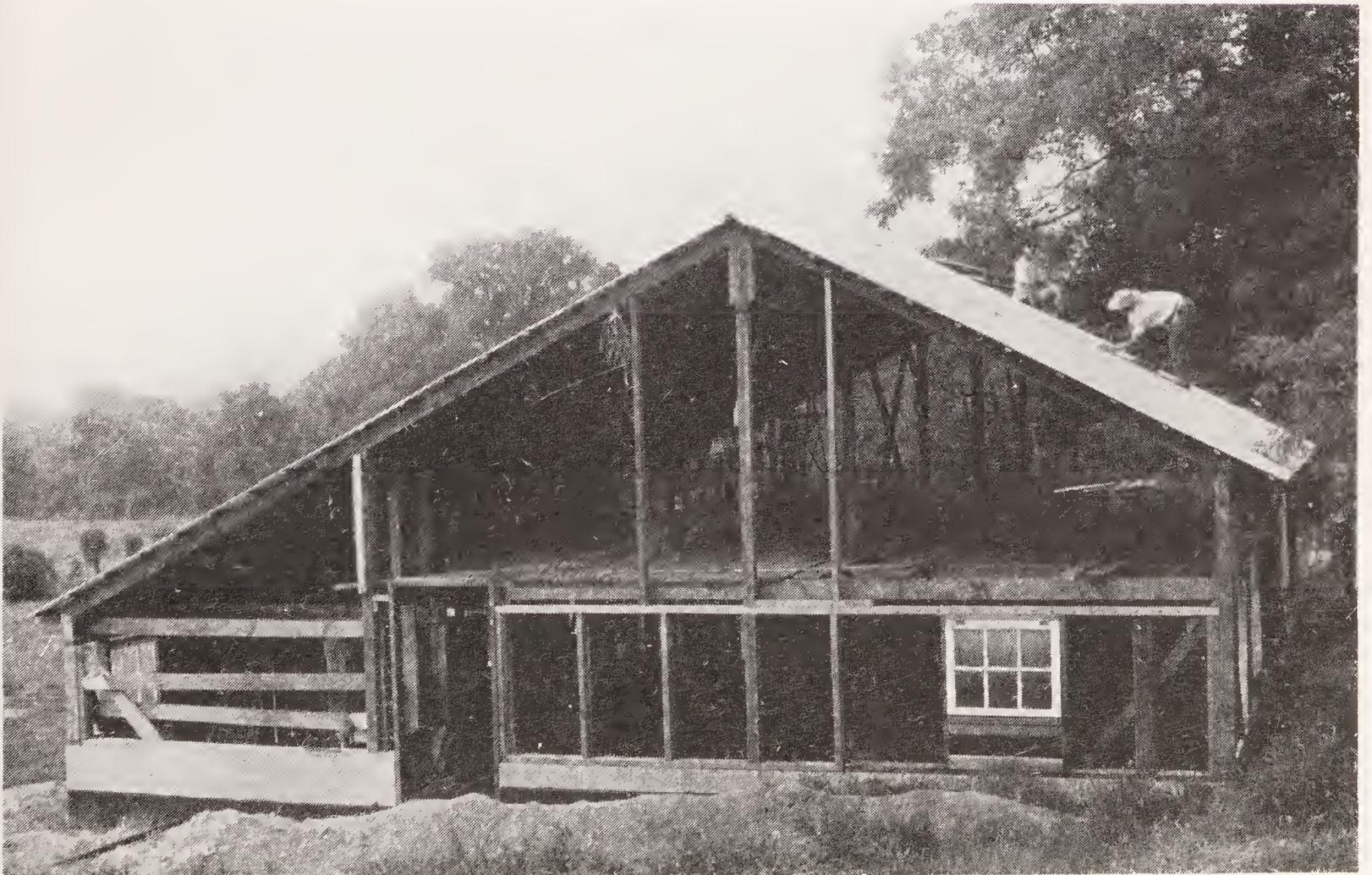
and the footing was sometimes precarious, but gradually the rafters fanned out—22 on the south side, then 22 on the north—each nailed to the ridgepole and the loft studs.
