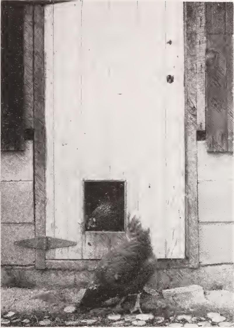
This outside door to the hen pen, with its "customized" opening permitting the birds to hop out into their yard, is just an old brooder house door turned upside down; the present "hatch" door was the former window. We added a hinged board that hooks to the inside of the door and makes it possible to close the opening in bad weather.
