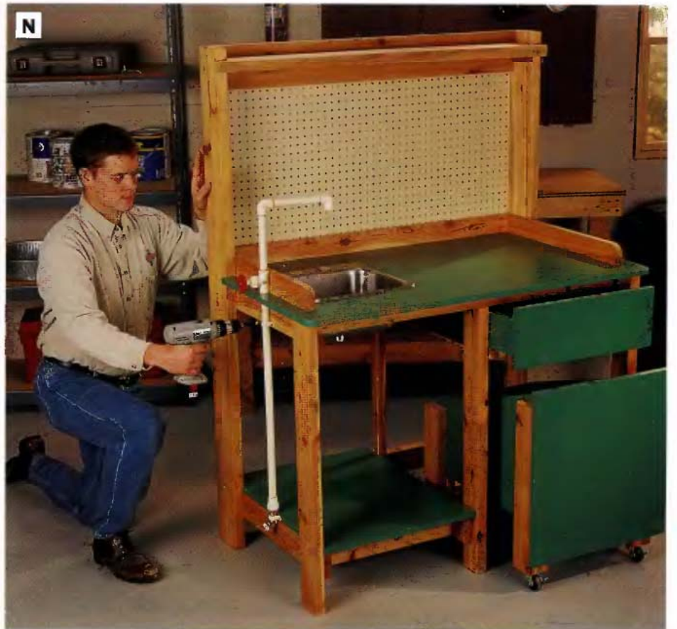
PHOTO N: Use strap clamps to attach the plumbing assembly to the bench.
