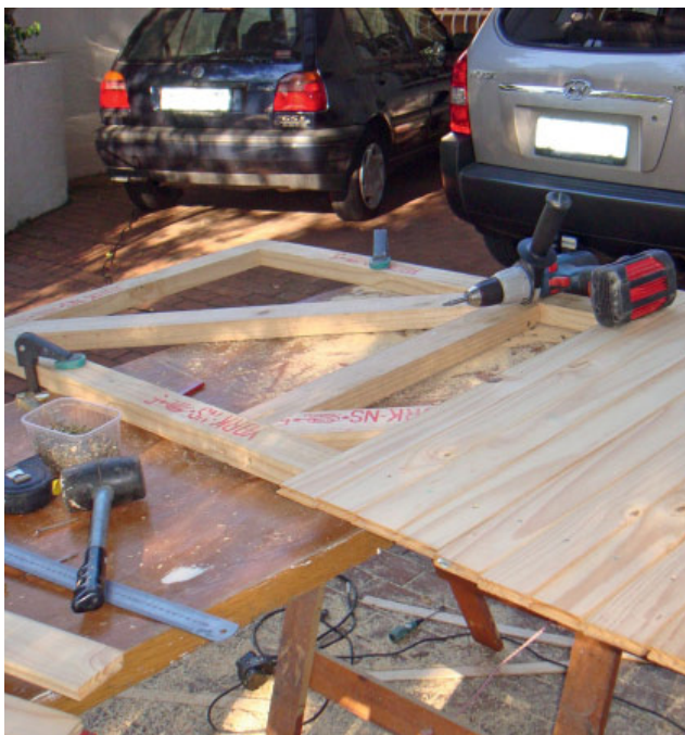
The photograph above shows the tongue-and-groove timber being fixed to the door structure shown on page 147. Note the overlap on both sides, which is then trimmed off using a jigsaw.
