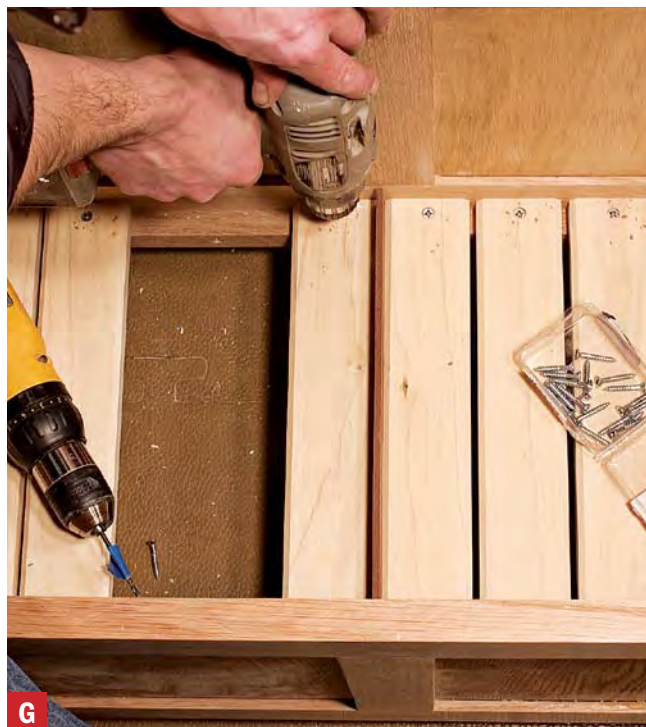
G Plank by plank. As you install the planked bottom, start from the outside ends and work inward.
