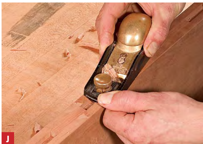
J Shave away the evidence. To remove remaining blade marks and glue stains, plane the strip flush with the rail. Don't get carried away; stop planing as soon as your blade starts shaving the rail.
