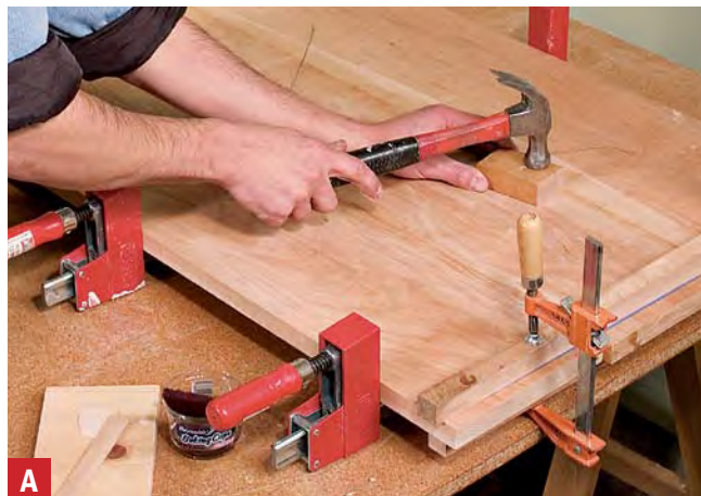
Hammered into alignment. You can expect boards in a glued-up panel to shift somewhat as they're clamped tight. With a hammer and scrap block, a few taps can pull the edges flush (before the glue sets).
