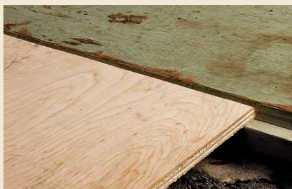
A sheet of ¾" plywood makes an adequate ramp for the small difference in height between the shop floor and the driveway.
