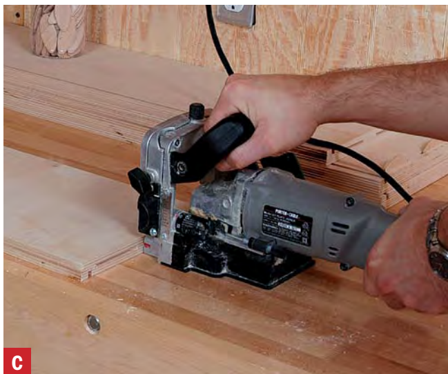
C Cut slots in the ends. Lay the top and bottom flat on the bench, align the biscuit joiner with the edge of the piece, and plunge to make the cut.
