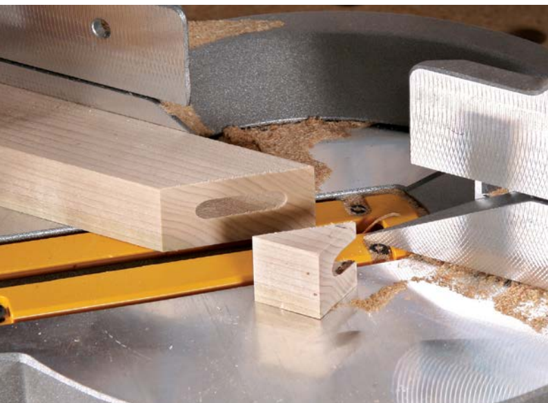
Miters after mortises. After using a Domino to cut the mortises on his frame members, Hansuld cuts the miters with a chopsaw.
