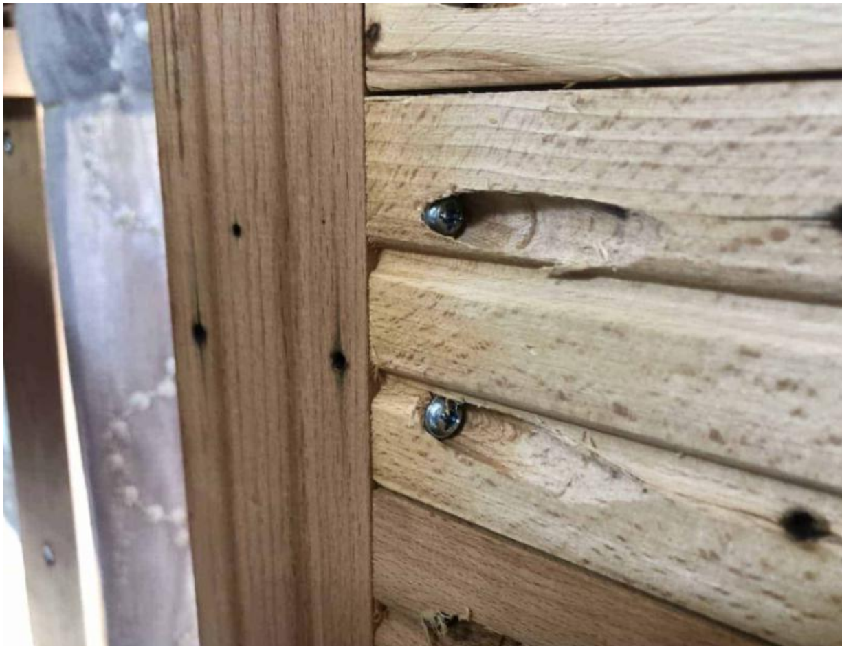
Edge Joint Example of Pocket Joints
