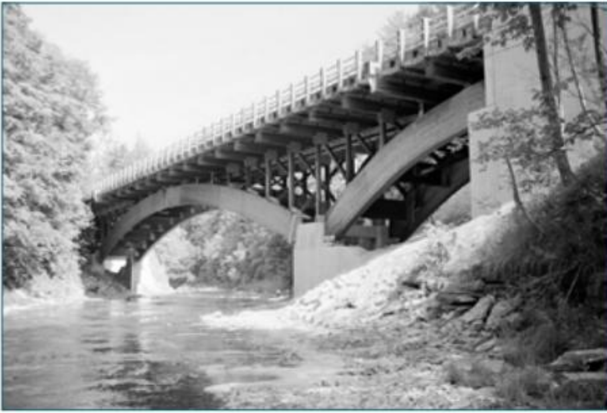
Figure 17–10. The Alton Sylor Memorial Bridge is a glulam deck arch bridge crossing Joncy Gorge in Angelica, New York. The center three-hinged arch spans 52 m (171 ft) and is the longest clear span in the United States. (Photo courtesy of Laminated Concepts, Inc., Big Flats, New York.)
