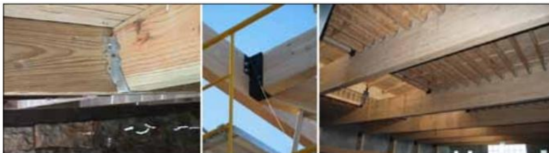
Figure 8-28. Typical joist hanger connectors.
