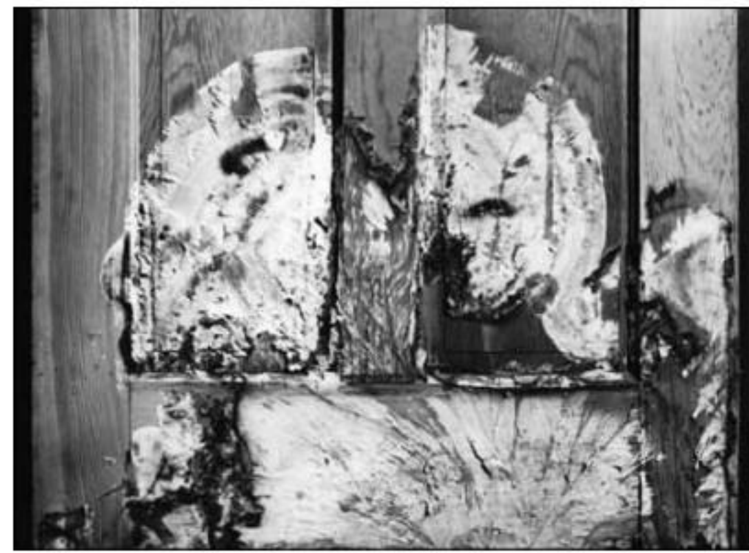
Figure 14-4. Mycelial fans on a wood door.
