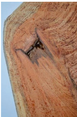
Fig. 5.93 Walaba ( Eperua ssp.) branch node with decayed knot
