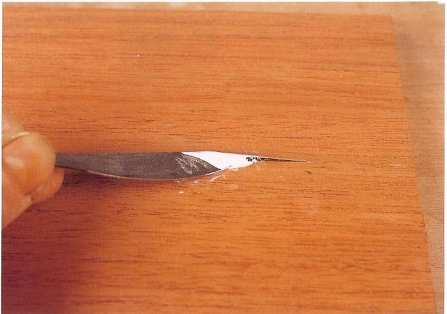
Fig 4.35 Splitting a blister along the grain and inserting fresh glue with an artists' palette knife.
