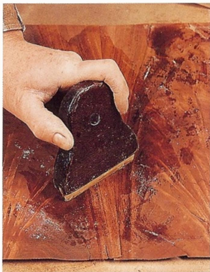
Fig 4.22 The second veneer is laid so that its internal edge overlaps that of the first veneer and the line drawn making the joint.
