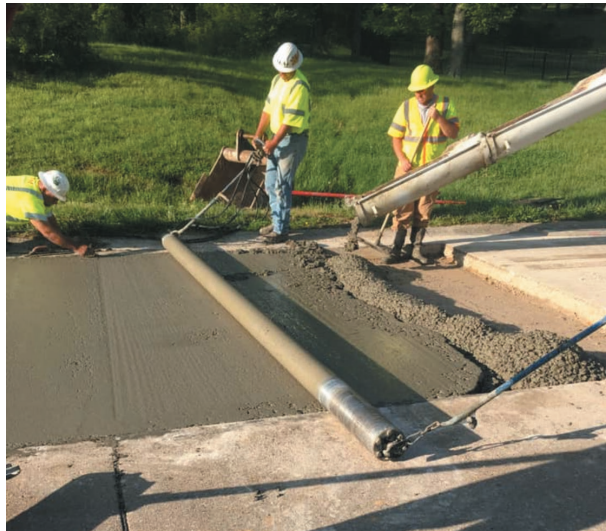
Fig. 31.3 Concrete workers wearing correct PPE: hi-vis jackets, footwear and hard hats
