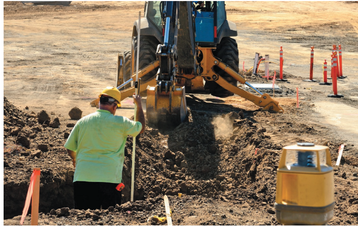
Fig. 31.25 Laser level monitoring depth of trench
