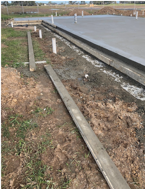
Fig. 30.19 Falsework and brackets removed and first formboard carefully stripped
