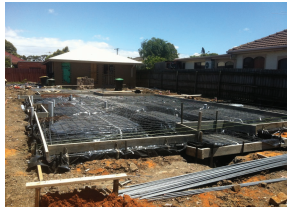
Fig. 12.25 Reinforcement materials used for slab on the ground
