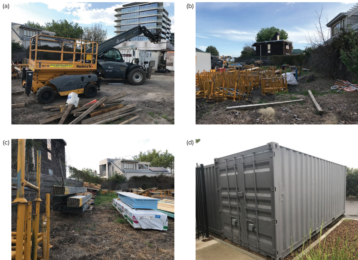
Fig. 12.28 Laydown yard showing: (a) EWP and telehandler forklift; (b) scaffold storage cages and baskets; (c) packs of materials; (d) lock-up shipping container
