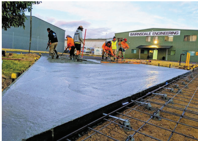
Fig. 31.37 Dowelled construction joint placed every 18 metres
