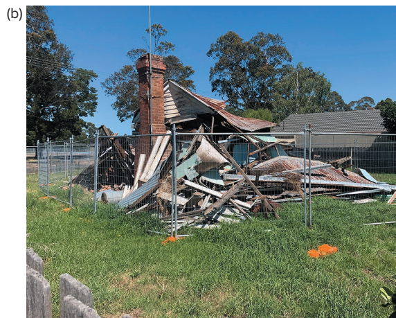
Fig. 34.15 An old house that through neglect has collapsed in on itself. Specialist demolition contractors and hazardous product removalists will need to be engaged to clean up the mess, as there could be any number of hazards present
