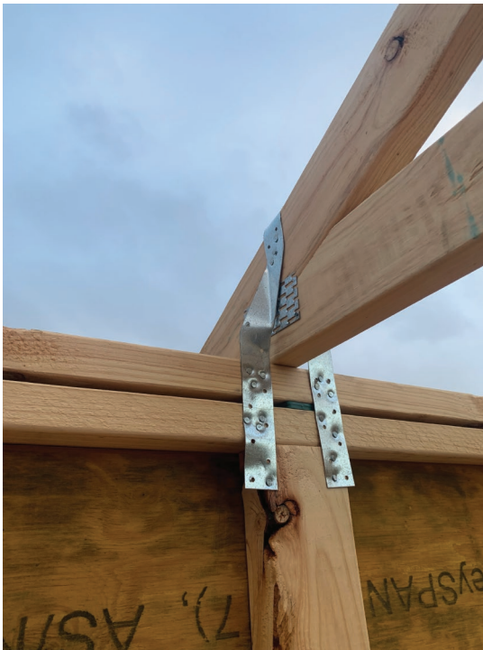
Fig. 23.18 A cyclone strap truss anchor nailed in place
