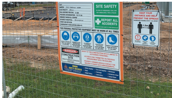
Fig. 30.1 Site entrance signage covering emergency, PPE and COVID-19 information
