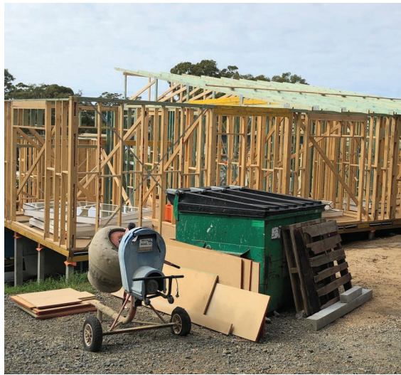
Fig. 6.10 Building waste and site rubbish should be separated
