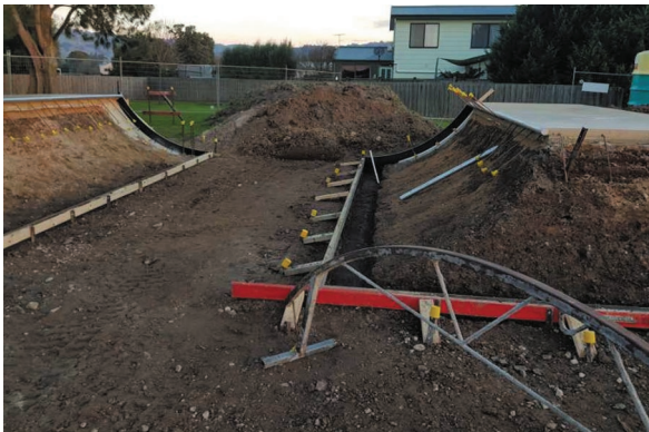
Fig. 31.5 Using curved concrete screeds to achieve the desired shape of the concrete
