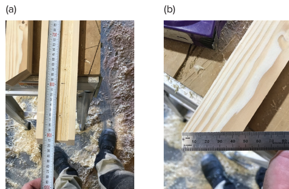
Fig. 33.58 (a) The length of capping; (b) angle cut of the baluster
