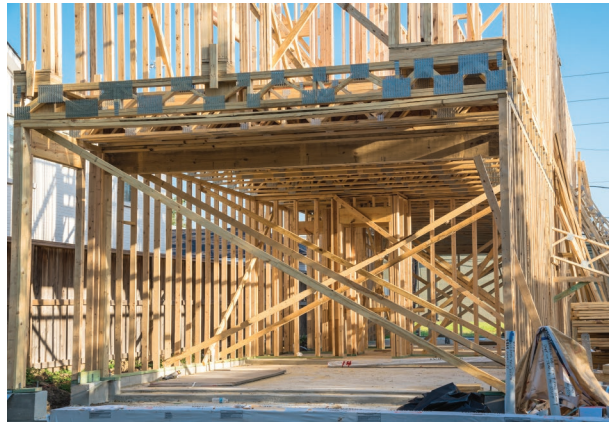
Fig. 18.44 Engineered timber upper floor joist
