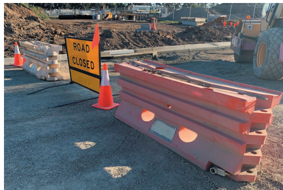
Fig. 15.31 Plastic water-filled barriers, signage and flags
