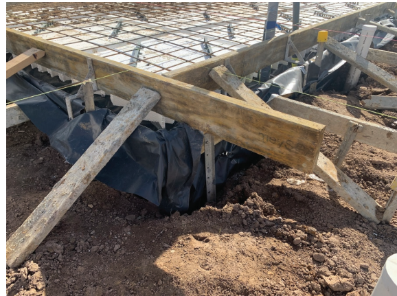
Fig. 30.14 Extra pegs and ledgers installed to help support bracketed formwork
