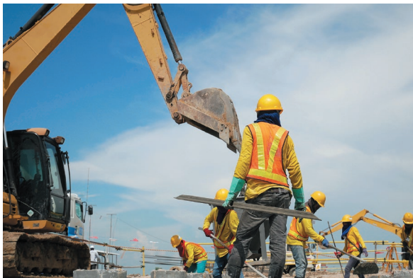
Fig. 1.15 Worker in front of an excavator wearing high-visibility clothing
