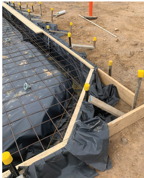
Fig. 30.15 Wider timber fitted to the inside of the formwork to create a blockout for an entrance door, plus narrower timber fitted to create a waterproof rebate for the metal external cladding to sit in
