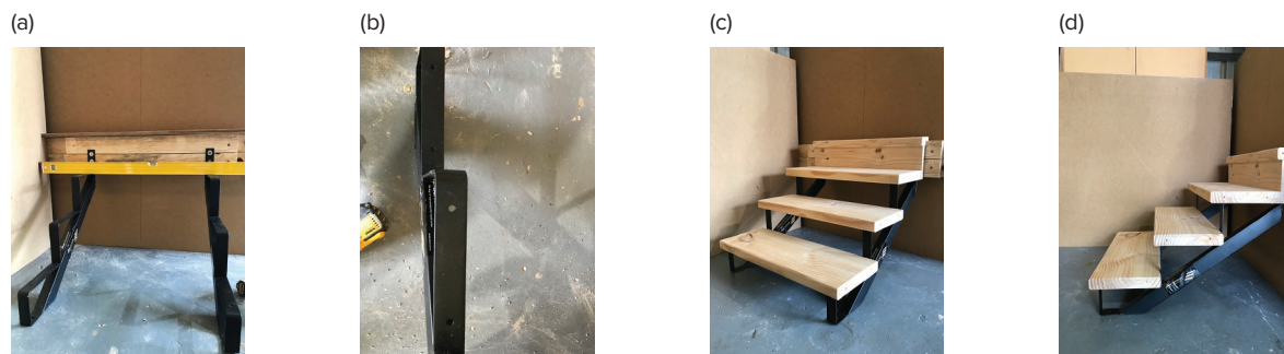
Fig. 33.16 Prefabricated powder-coated stringers: (a) levelling stringers; (b) stringer fixing points; (c) installed treads and top riser and nosing; (d) side view of installed staircase
