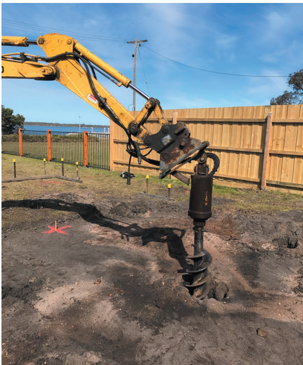
Fig. 15.23 Marking paint and timber pegs used to mark the position of the pier holes
