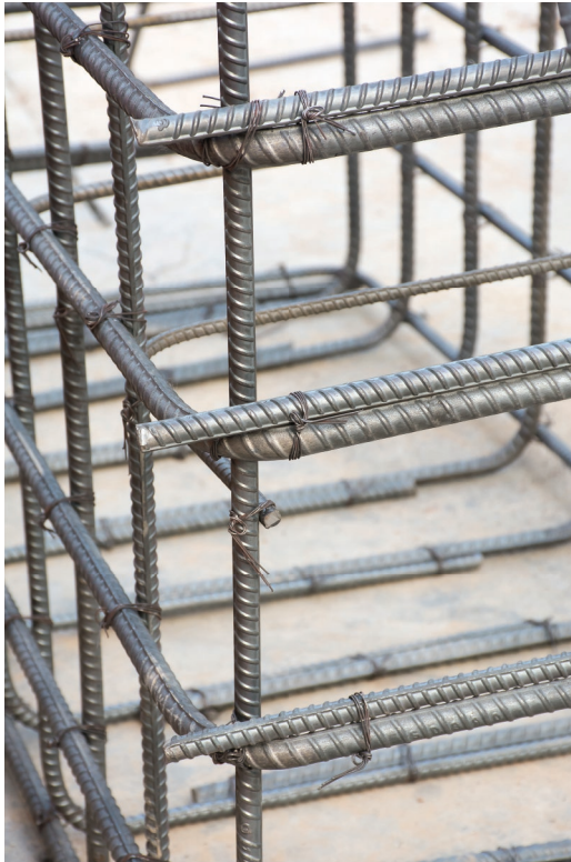
Fig. 31.10 Reinforcing cage out of deformed bar
