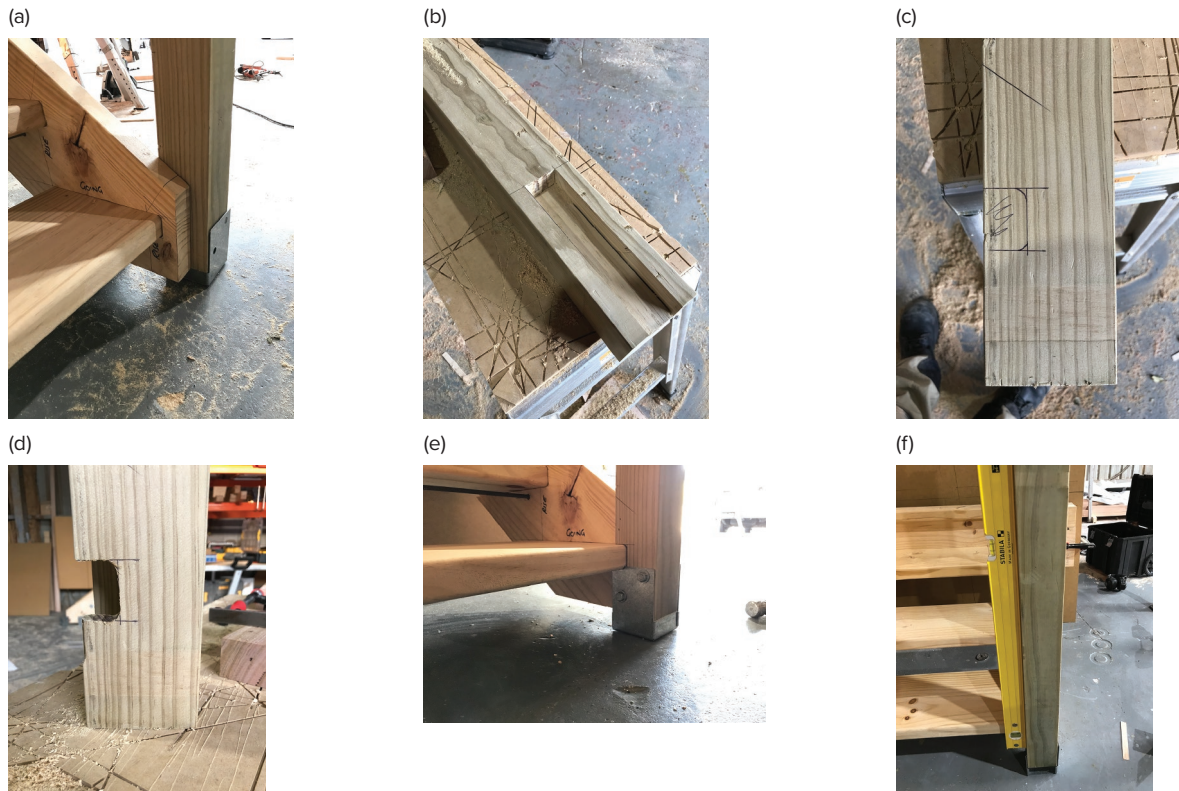
Fig. 33.49 (a) Setting up and marking position of post; (b) housing post to suit stringer; (c) marking tread nosing into post; (d) nosing routed into post; (e) post anchor installed and post attached to stringer; (f) plumbing post
