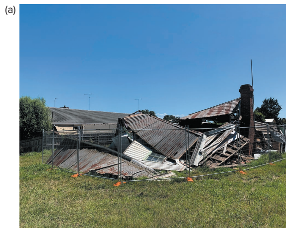
Fig. 34.15 An old house that through neglect has collapsed in on itself. Specialist demolition contractors and hazardous product removalists will need to be engaged to clean up the mess, as there could be any number of hazards present
