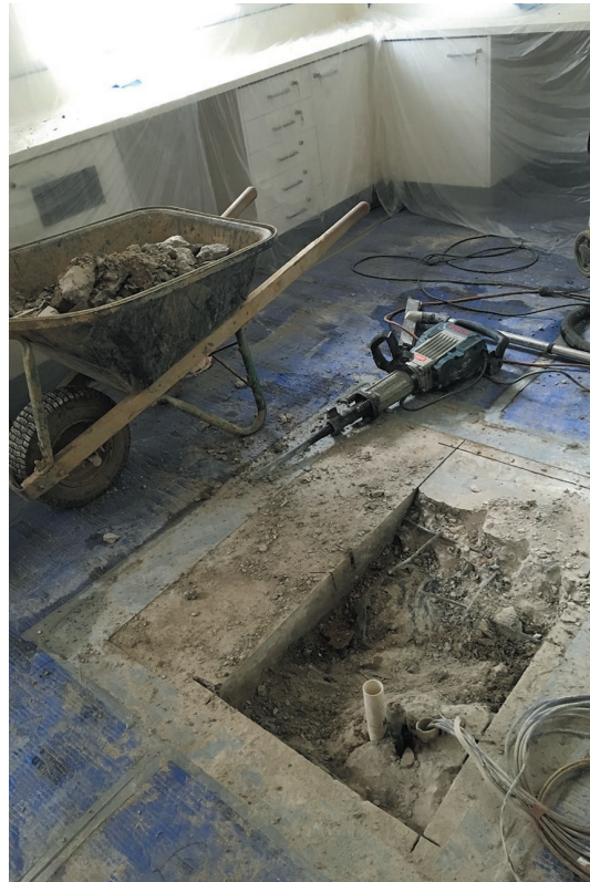
Fig. 34.13 Kitchen renovation with partial concrete slab demolition. Note: the electric jackhammer, wet and dry vacuum system and all existing cabinetry are protected
