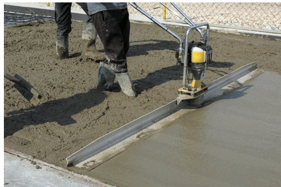
Fig. 31.30 Vibrating screed
