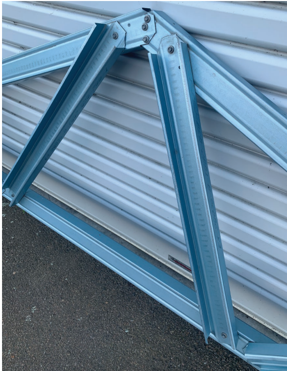
Fig. 23.37 Steel truss webbing joint detail
