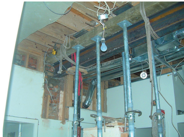
Fig. 34.22 Temporary propping of floor joists in upper floor—note services
