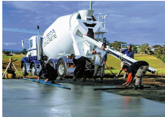
Fig. 31.29 Screeding concrete
