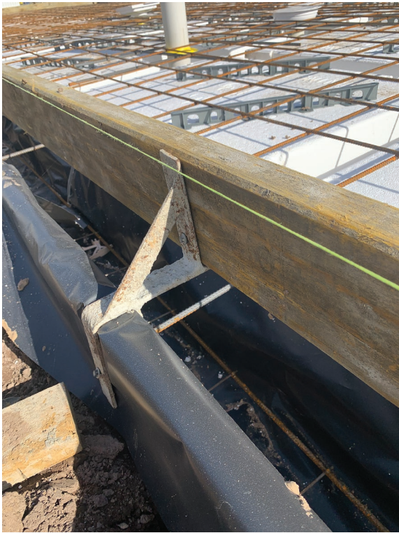
Fig. 30.13 Slab rebate formed using formwork brackets
