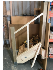
Fig. 33.67 Temporarily positioned baluster to set up a handrail
