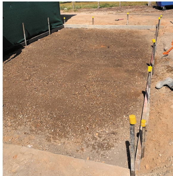
Fig. 31.28 Road base ready for final compaction before pouring
