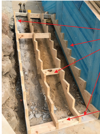
Fig. 33.83 Installation of bottom flight
