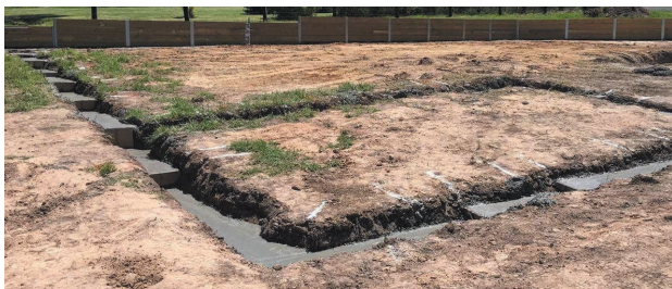
Figure 15.27 Stepped perimeter strip footing
