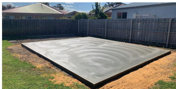
Fig. 30.10 A completed garage slab (note the blackout that has occurred for the roller door position)
