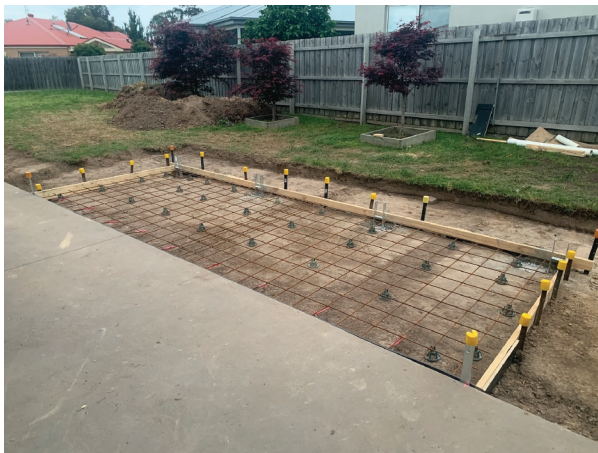
Fig. 30.4 Simple ' under to over ' formwork construction
