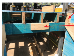
Fig. 33.77 Setting up cleat for middle stringers (carriage stringers)
