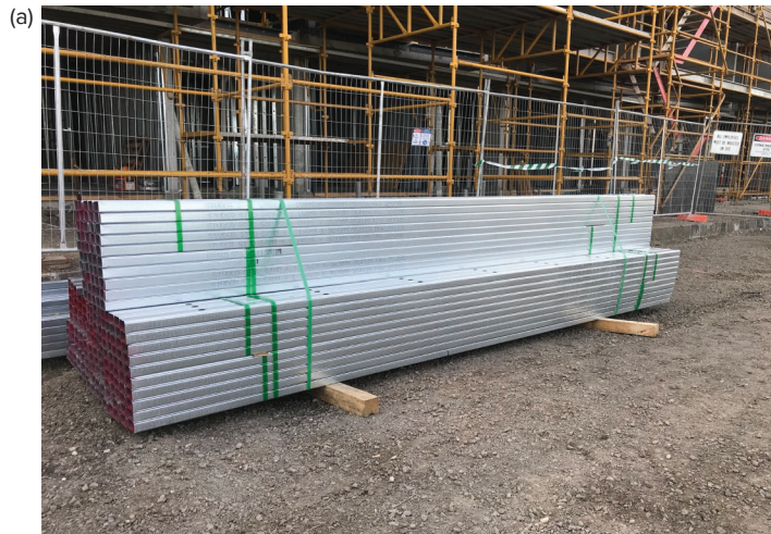
Fig. 12.9 (a) Banded metal studs; (b) banded materials ready to be delivered to site
