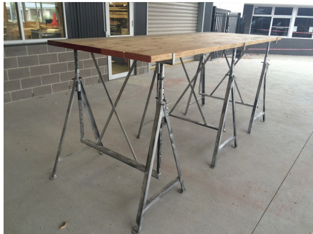
Fig. 26.11 Place planks on trestle
