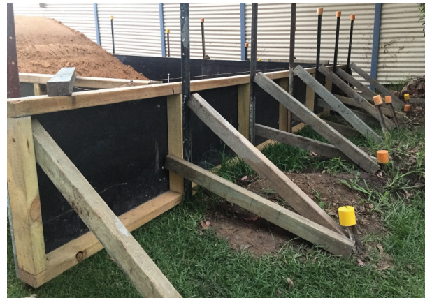
Fig. 30.18 Soldier wall formwork pegged and braced from the top and bottom
