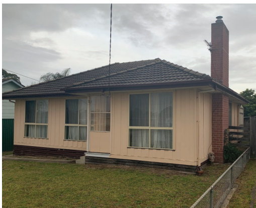
Fig. 1.18 Post-war fibro home with external asbestos cement sheeting
