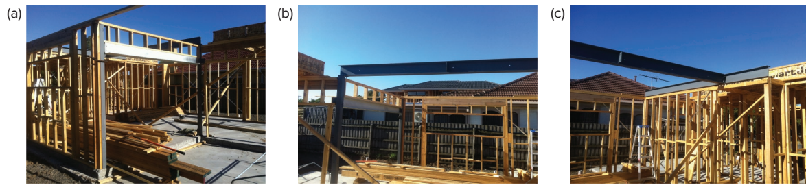
Fig. 12.26 (a) Structural steels used for large door opening; (b and c) structural steel to support second storey of dwelling
