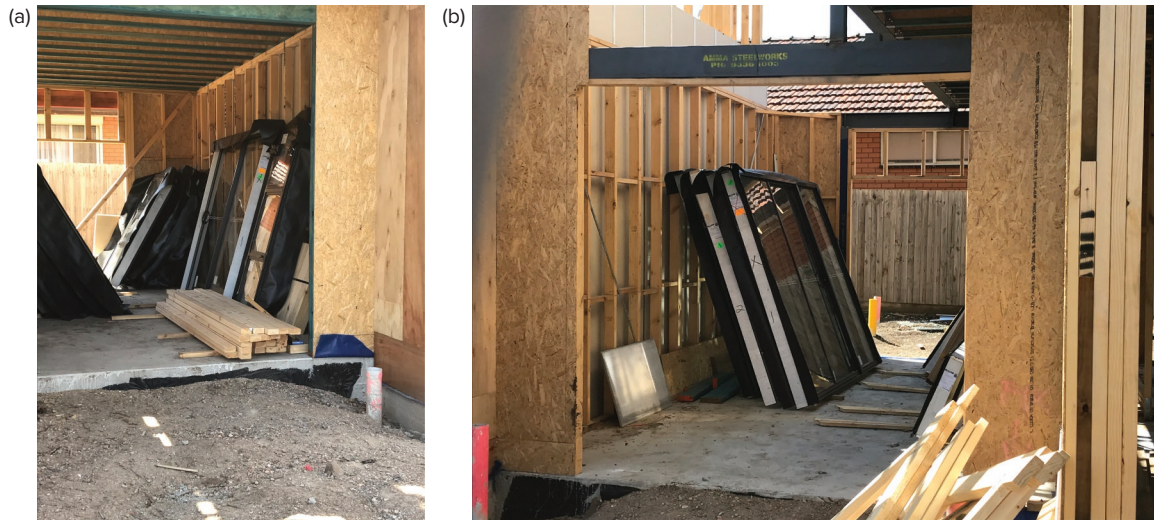
Fig. 12.18 (a) and (b) Windows stored on-site
