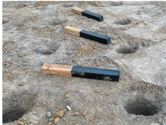
Fig. 15.30 Pier holes bored to the correct depth for the coated timber stumps
