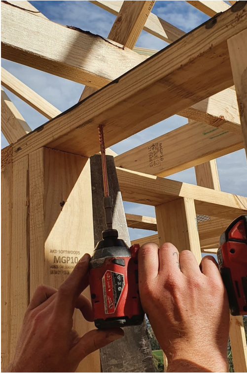
Fig. 23.13 Driving the screw through the top plate
