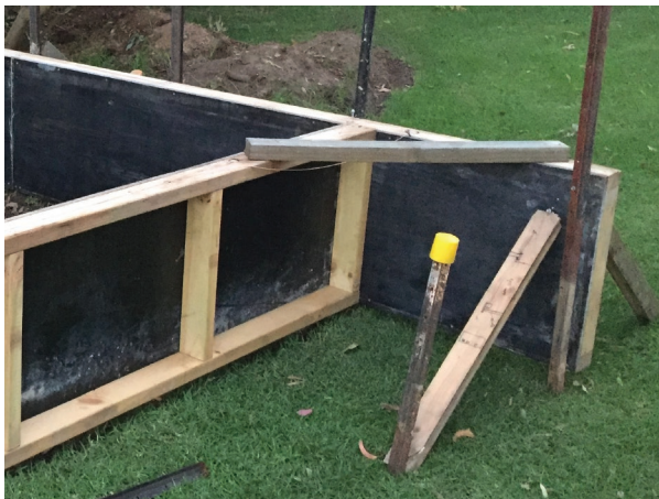
Fig. 30.17 Extender soldier wall formwork with the corner pegged and braced for stability
