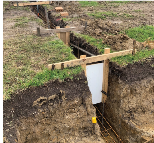
Fig. 30.8 Excavation of footings on a steep block (note the shutters in place to form up for the stepped footings)
