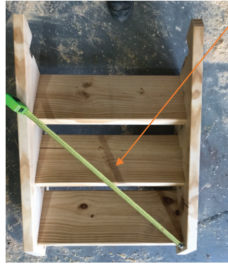
Fig. 33.40 Squaring staircase unit
