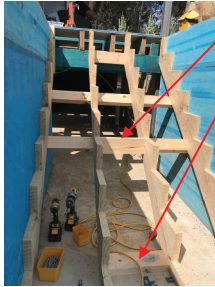
Fig. 33.79 Bracing and solid blocking stringers
