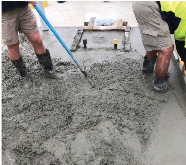
Fig. 30.2 Gum boots are essential PPE when pouring large areas of concrete
