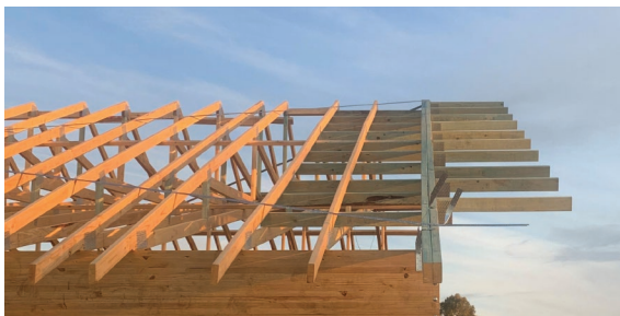
Fig. 23.21 Verge sprockets forming the verge overhang on the gable end
