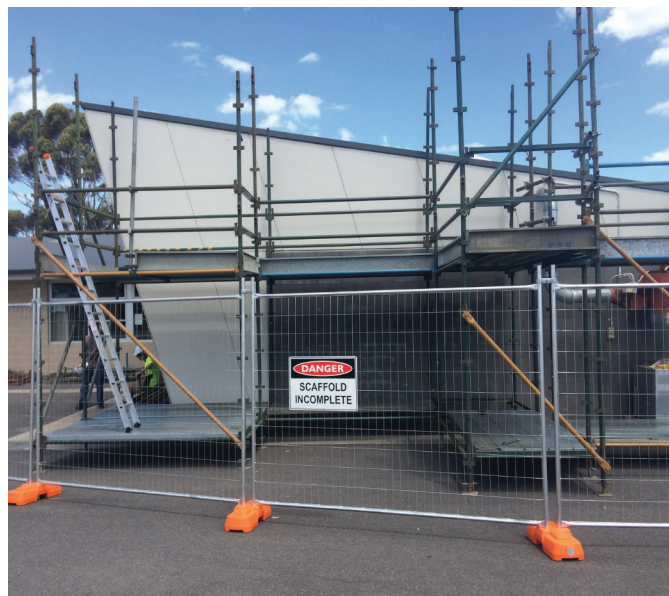
Fig. 26.6 Temporary fencing around building site
