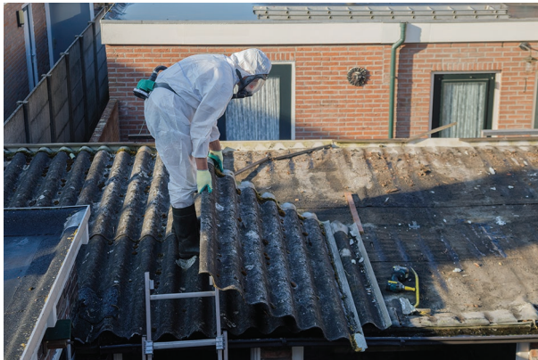
Fig. 34.3 Specialised tools allow whole sheets of asbestos sheeting to be removed without breakage
