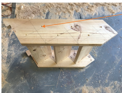
Fig. 33.39 Assembly of stringers and treads
