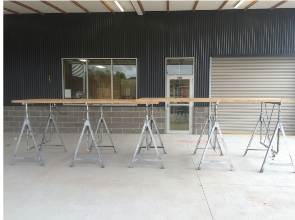
Fig. 26.12 The finished scaffold
