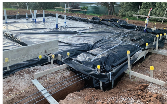
Fig. 30.9 String lines set up for formwork construction
