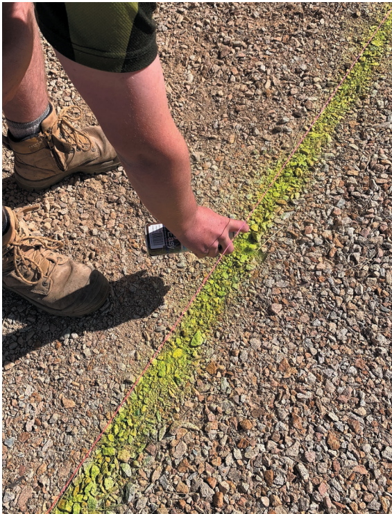
Fig. 15.21 Marking paint used to mark out the perimeter of the excavation
