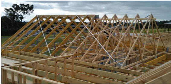
Fig. 23.34 Speed brace fitted in a diagonal pattern before the roof battens are fitted
