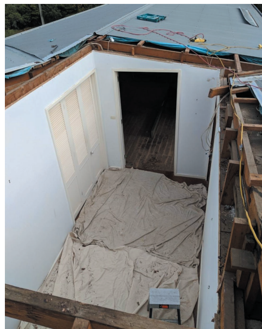
Fig. 34.21 Partial roof and ceiling frame demolition; tarpaulins will need to be fitted to ensure there is no damage from the outside elements
