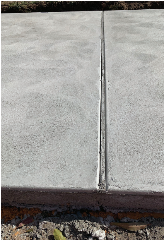
Fig. 31.39 Finished foam expansion joint
