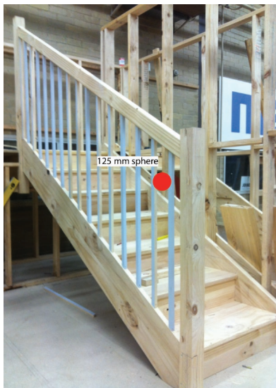
Fig. 33.4 Apprentice practice staircase and rake balustrade
