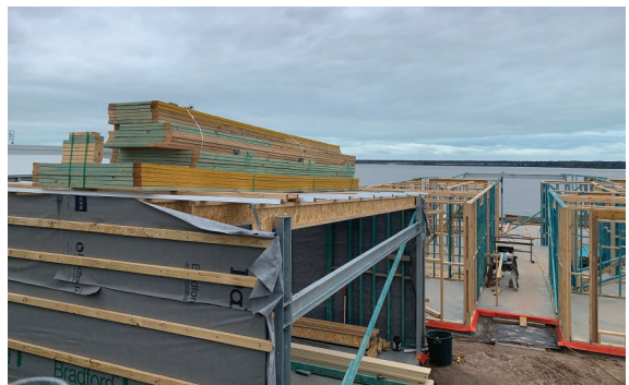
Fig. 23.29 Trusses placed on the frame for easier handling during installation
