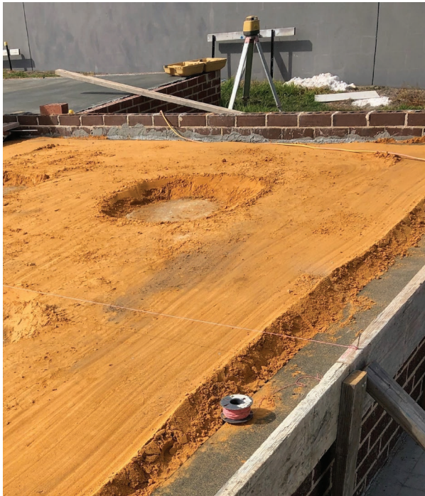
Fig. 30.3 Laser level set up for formwork construction and foundation preparation
