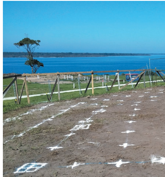
Fig. 15.22 Marking paint and lime used to mark out the auger boring positions on this sloping site
