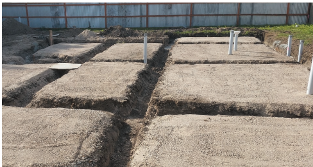
Fig. 15.25 Typical excavation for a slab on ground
