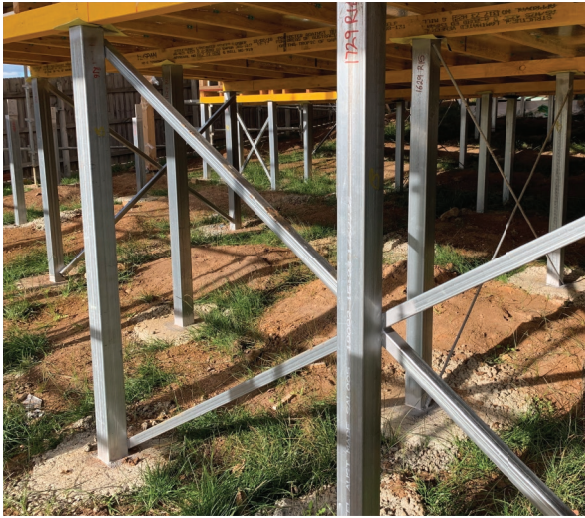
Fig. 31.1 Steel stumps supporting a house—set on concrete pads and backfilled to ground level with more concrete
