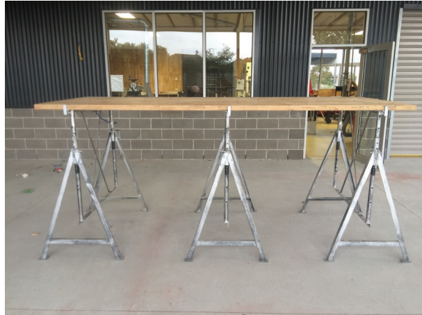
Fig. 26.3 Trestles and planks scaffolding
