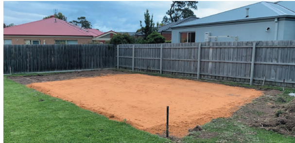
Fig. 31.6 (a–c) Preparation and concreting a slab for a free-standing steel garage shed: (a) sand blinding placed and compacted; (b) simple corner-lapped formwork, vapour barrier and reinforcement installed (note the section of formwork lying flat to allow easy access when barrowing the concrete in, plus the plastic bag of bar chairs ready to be installed when the pour begins, to lift the reinforcement to the correct height; (c) the completed concrete slab after the formwork has been carefully removed to avoid any damage to the edges
