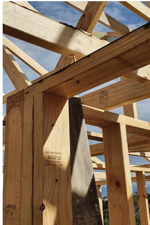
Fig. 23.16 The screw fixed into its final position
