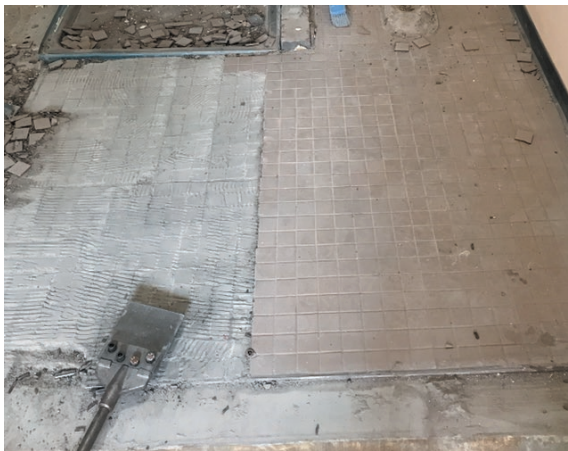
Fig. 34.14 Removal of ceramic floor tiles using a hand-held tile scraper
