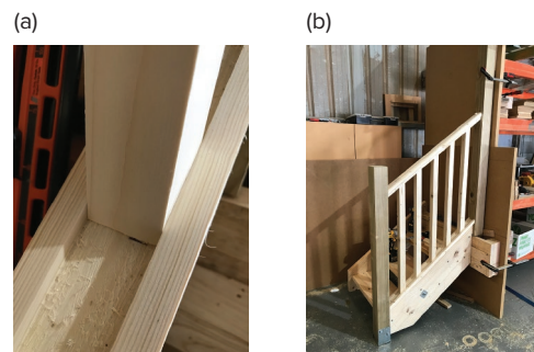
Fig. 33.68 Capping mark-out
