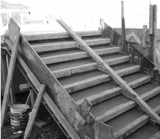
Fig. 32.3 Formed and poured concrete stairs
