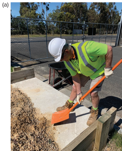
Fig. 1.17 (a–d) Shovelling loose materials such as sand or dirt: (a) keep the legs apart with one foot in front and close to the end of the shovel; (b) put weight on front foot, place both hands on the shovel with each hand resting against a leg, and bend legs and push forward using body weight to push the shovel; (c) step back onto back foot with loaded shovel and keep the load close to your body; (d) step and turn feet and body in the direction of where the material needs to be placed. Keeping the load close to your body, roll your forearms, wrists and hands to dislodge material
