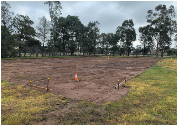
Fig. 15.7 Building area with the topsoil removed, ready for set-out
