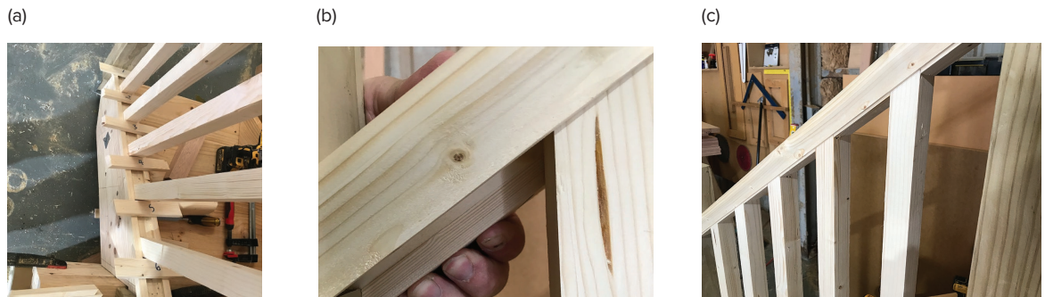
Fig. 33.70 (a) Oversized fillet timbers numbered; (b) scribing fillet; (c) installed fillet timbers
