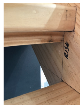
Fig. 33.42 (a) Gap reduced by attachment of a cleat; (b) cleat is in line with the rise
