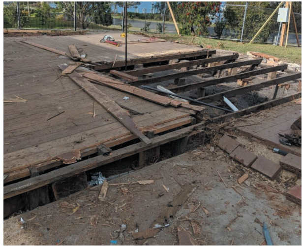
Fig. 34.16 Typical flooring and subfloor of an older house under demolition
