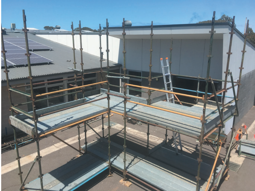
Fig. 26.22 Completed scaffold with toeboards, handrails and midrails
