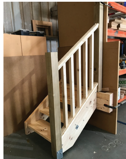
Fig. 33.71 Completed external staircase and rake balustrade
