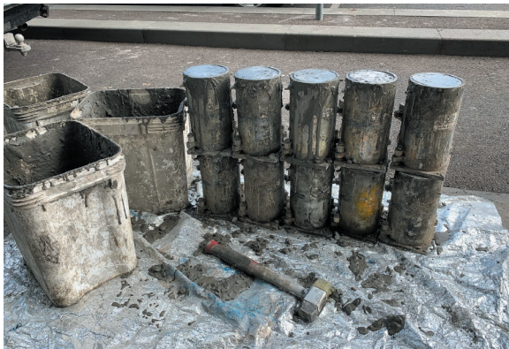
Fig. 31.43 Concrete testing cylinders filled and ready for transport
