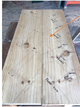
Fig. 33.33 Checking that the left and right stringers line up
