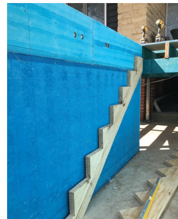
Fig. 33.76 Setting up cut/saw-tooth stringers
