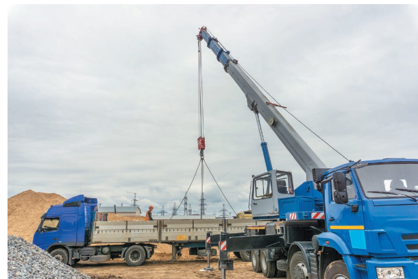
Fig. 1.14 Materials being raised by a crane
