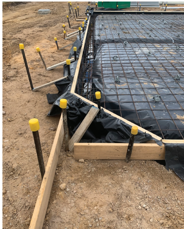
Fig. 30.12 Extra pegs to support the overhanging formwork
