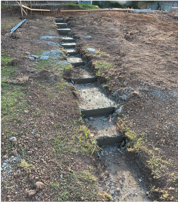
Fig. 31.27 The poured stepped footing ready for work to proceed
