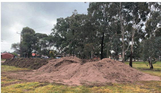
Fig. 15.8 Re-usable topsoil ready for removal from the site
