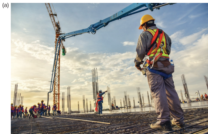
Fig. 1.16 (a) and (b) (a) Concreters working with a concrete boom; (b) pumping concrete
