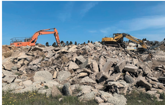
Fig. 31.40 Excess and clean demolished concrete piled for recycling
