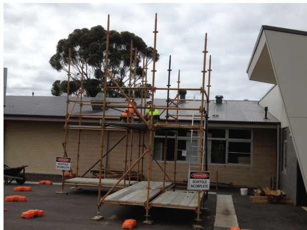
Fig. 26.1 Quickstage or modular scaffold
