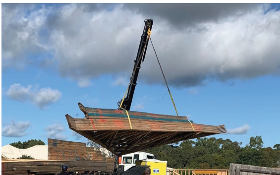
Fig. 23.28 Truss delivery using slings for correct lifting of the packed trusses
