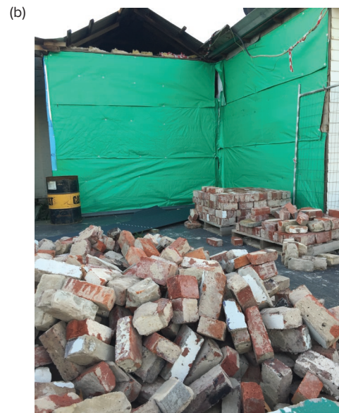
Fig. 34.28 (a) Reclaimed materials stacked and banded ready for removal from the demolition site; (b) demolished brickwork being cleaned and stacked on pallets ready for removal from the demolition site for re-use
