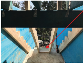
Fig. 33.78 Securing stringers into place
