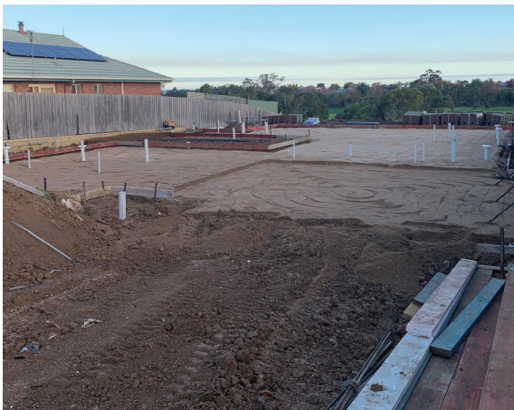
Fig. 30.5 Plumbing services cast in with the formwork construction for a waffle raft slab underway
