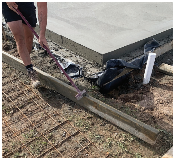
Fig. 30.20 A steel scraper ideal for cleaning formwork as it is stripped
