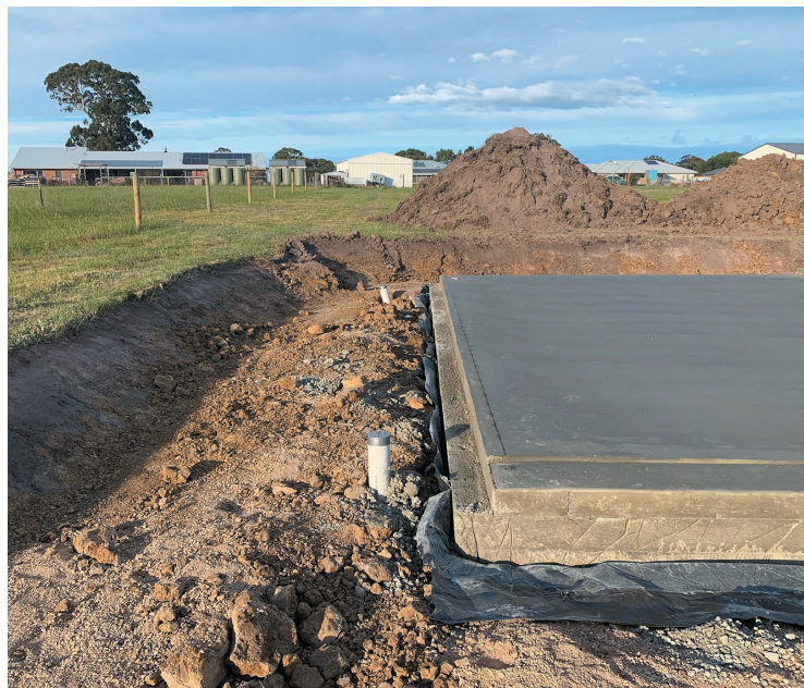
Fig. 15.1 A typical domestic site cut
