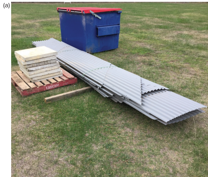
Fig. 34.28 (a) Reclaimed materials stacked and banded ready for removal from the demolition site; (b) demolished brickwork being cleaned and stacked on pallets ready for removal from the demolition site for re-use
