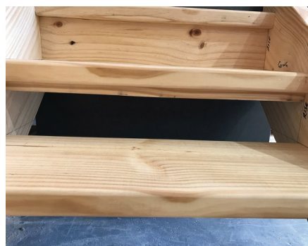
Fig. 33.42 (a) Gap reduced by attachment of a cleat; (b) cleat is in line with the rise
