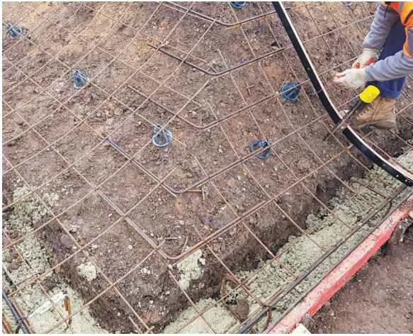
Fig. 31.4 Using templates to maintain the shape of the concrete
