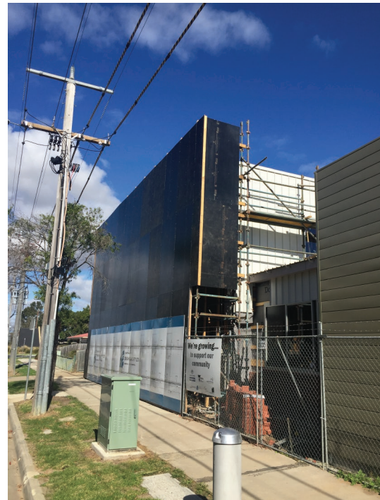
Fig. 34.6 Sheet hoardings fixed onto the scaffolding for the building facade demolition process and rebuild
