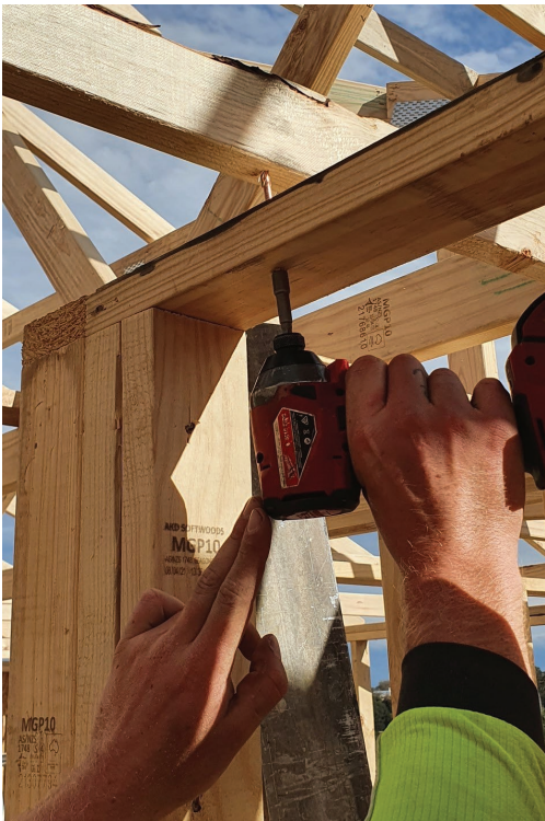
Fig. 23.15 Screw fully embedded into the truss with pilot hole cut
