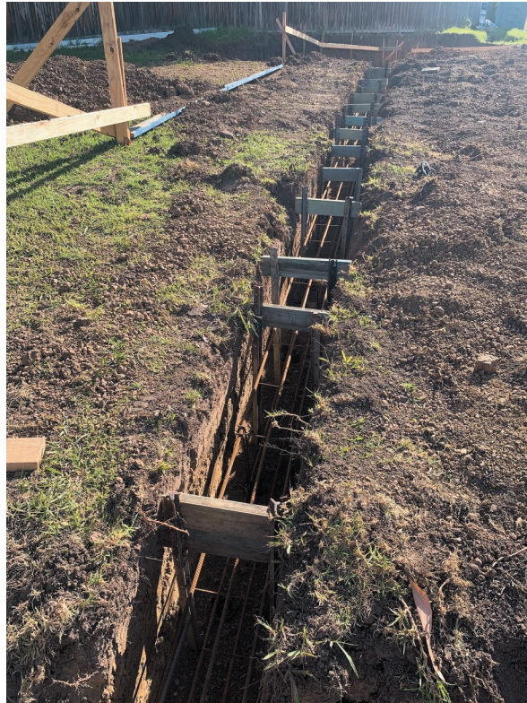
Fig. 31.26 A stepped footing excavation with mesh installed and timber block outs fixed at brick course height to create the steps
