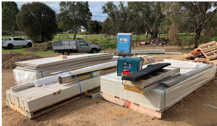
Fig. 6.9 Logical placement of building materials
