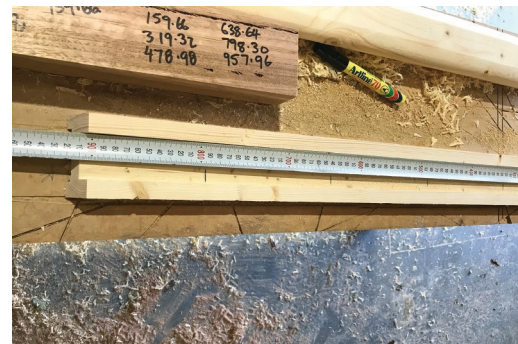
Fig. 33.62 Marking out the capping
