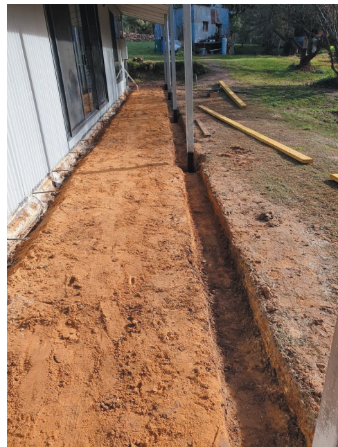
Figure 15.26 Hand-tool excavated verandah strip footing
