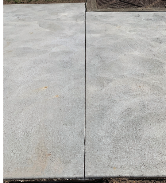
Fig. 31.36 Sawn control joint
