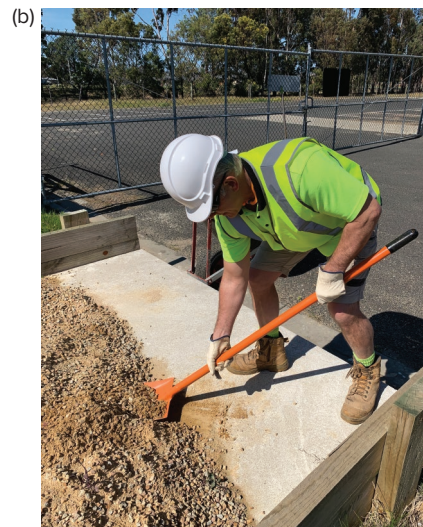
Fig. 1.17 (a–d) Shovelling loose materials such as sand or dirt: (a) keep the legs apart with one foot in front and close to the end of the shovel; (b) put weight on front foot, place both hands on the shovel with each hand resting against a leg, and bend legs and push forward using body weight to push the shovel; (c) step back onto back foot with loaded shovel and keep the load close to your body; (d) step and turn feet and body in the direction of where the material needs to be placed. Keeping the load close to your body, roll your forearms, wrists and hands to dislodge material
