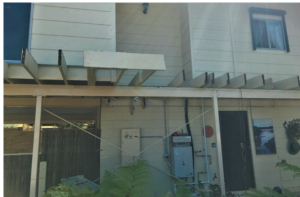
Fig. 34.23 Cantilevered timber balcony in the process of being demolished. The deep joists will be cut back to the building then correct propping will be installed for complete removal and replacement.
