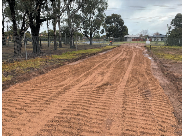
Fig. 15.18 All-weather access point
