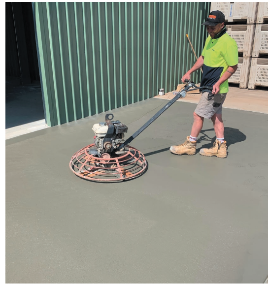
Fig. 31.33 Powered helicopter trowel
