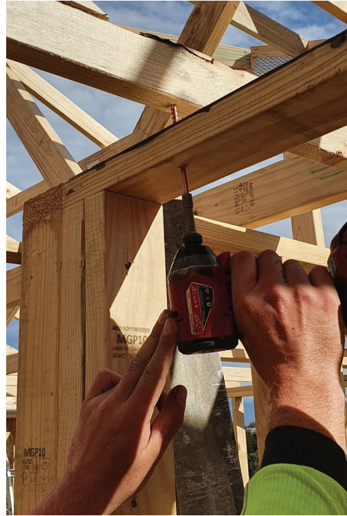
Fig. 23.14 Attaching the truss and cutting the pilot hole
