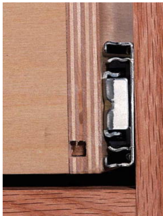
Check the slide's specification sheet for the required side clearance, and you'll be rewarded with smoothly operating drawers.
