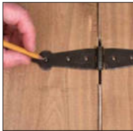
Surface-Mounted Hinges
