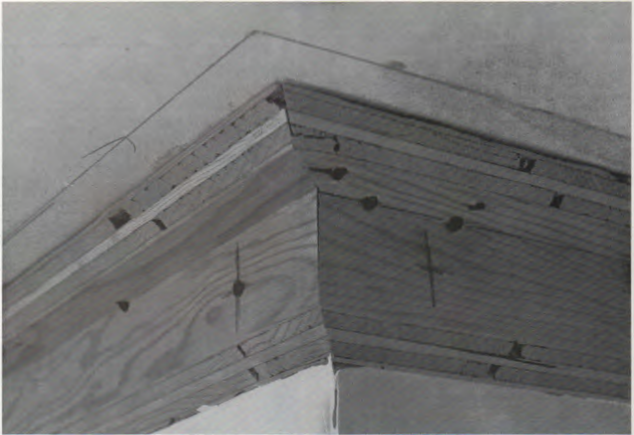
The finish carpenter is often called on site after the drywall is hung, too late to install proper backing for really wide crown molding. One solution is to nail or screw plywood backing outside the drywall.
