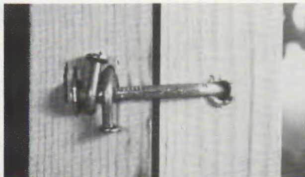
Clinched nails keep the trimmer from twisting off the king stud. First, drive a 16d nail into the trimmer, then bend it over. A pair of clinched 8d nails locks the larger nail in place.
