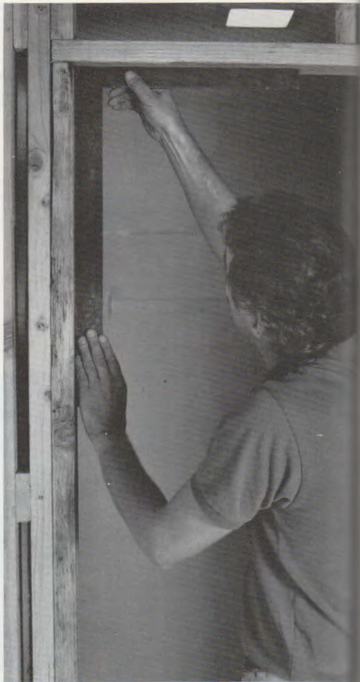
With a framing square, Savage checks a door opening for square. Checking both trimmers for plumb and the header for level is another way to test for square.
