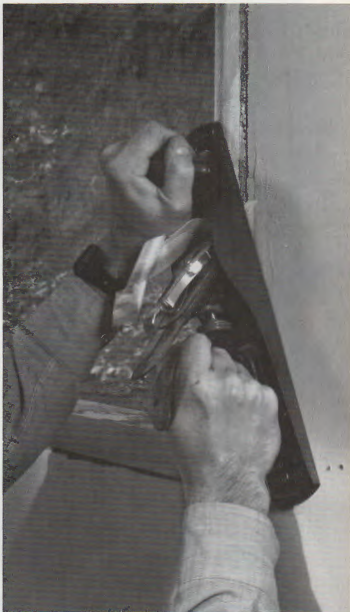
Jambs that stand proud of the drywall surface should be planed flush. Be careful not to plane too deeply, or you risk tearing the drywall's surface paper.
