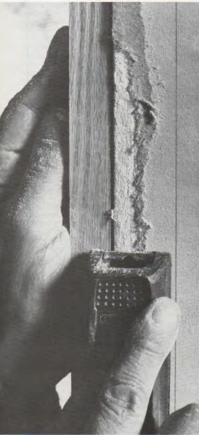
Drywall that projects above the jamb can be made flush with a Surform plane. A penciled line on the drywall shows the outward limit of the taper.
