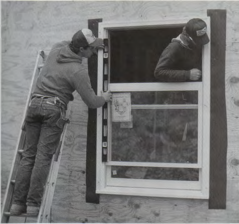
Once the rough opening has been prepared, the window is set from the outside of the house. The window is temporarily tacked through its nailing flange or through the exterior casing. It's then plumbed and leveled with wedges before being permanently nailed.
