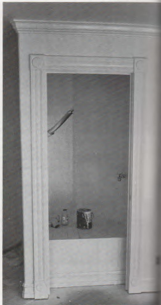
This door has been cased with commercially made plinth and corner blocks and molded casing. The plinth and block are wider than the casing, resulting in an equal reveal on both edges of the casing. The plinth has been held above the rough floor to allow for carpeting.
