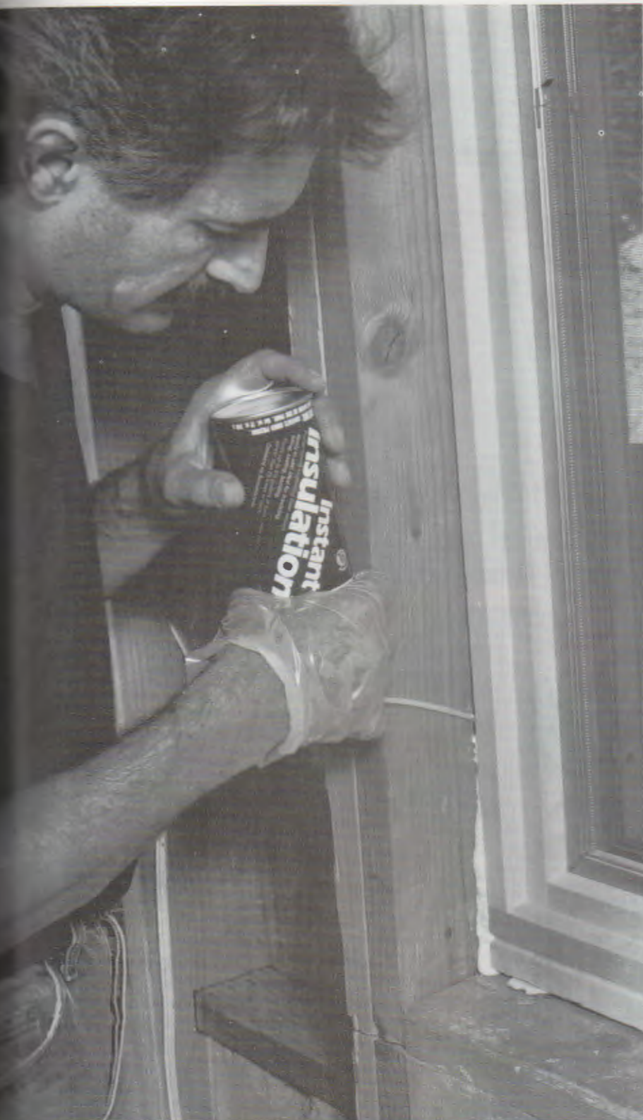
Expanding foam insulation seals gaps between the window jamb and the trimmer, header and rough sill. Don't inject too much, however, or it may cause the jambs to bow.
