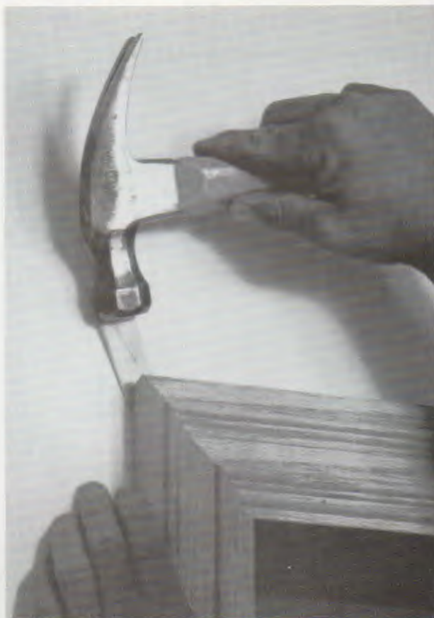
Slightly misaligned casings can be pared flush (top). As a desperate last resort, a wedge driven behind the casing flushes up both parts, above. The wedge is sawn flush, and the gap at the casing's back is caulked over.
