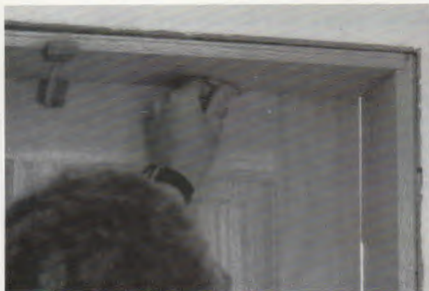
A shopmade sheet-metal clamp holds the door against the jamb for scribing. The drawing below shows how the clamp is made.
