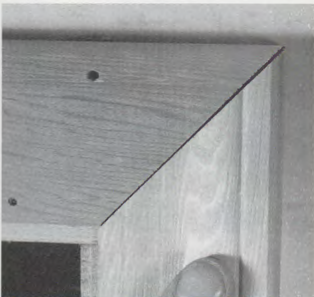
A perfect miter fits tightly with no gaps at the heel or toe, as shown in the door casing in the top photo. The miter in the photo above needs to be back-cut in order to fit properly.
