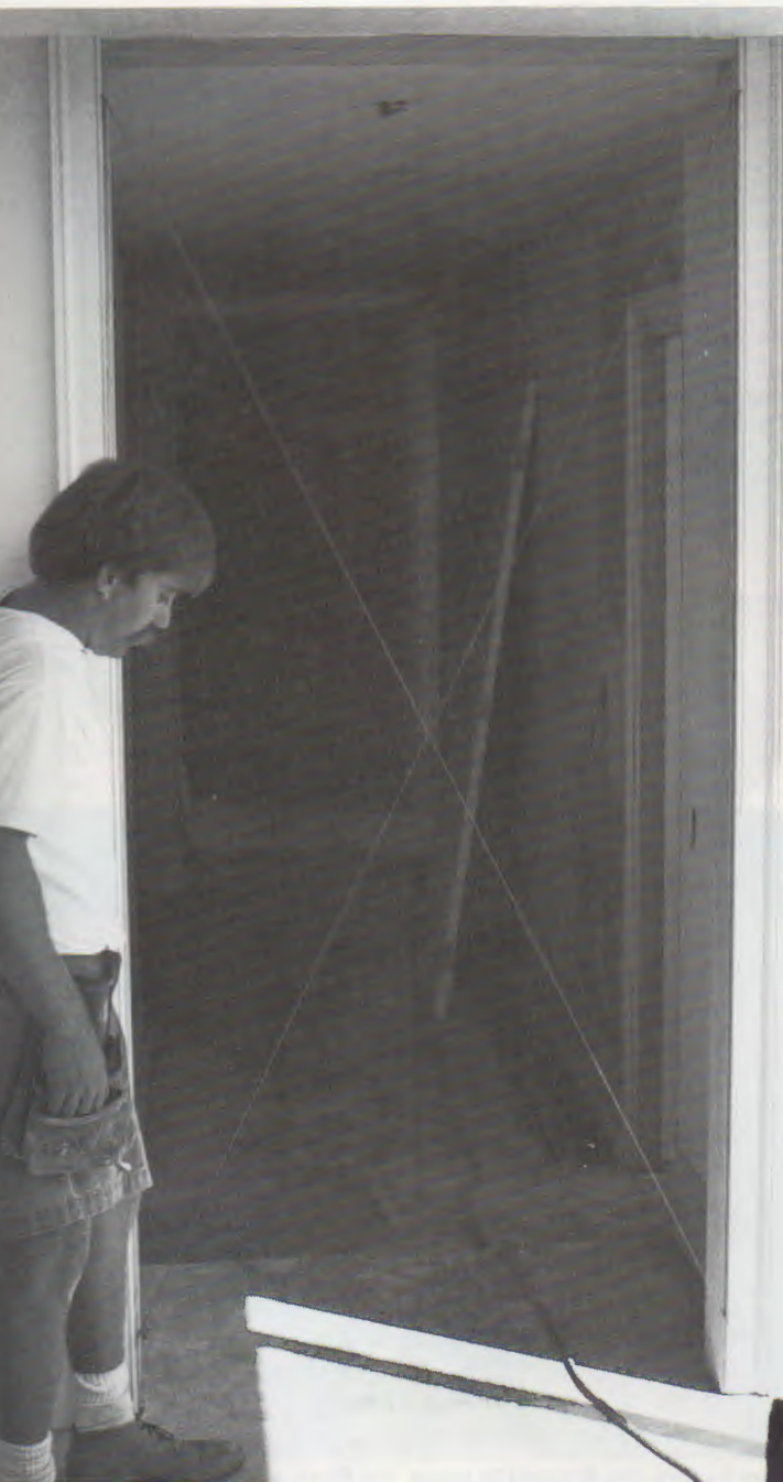
It's best to correct a twisted opening at the framing stage rather than cobbling a fix after the fact, as is being done here. If strings stretched across the opening just touch, the opening is true.
