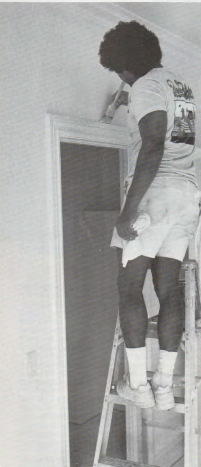
Begin cutting in casing along the edges adjacent to the walls. Then paint the flat surfaces, starting at the top and working down toward the baseboard.
