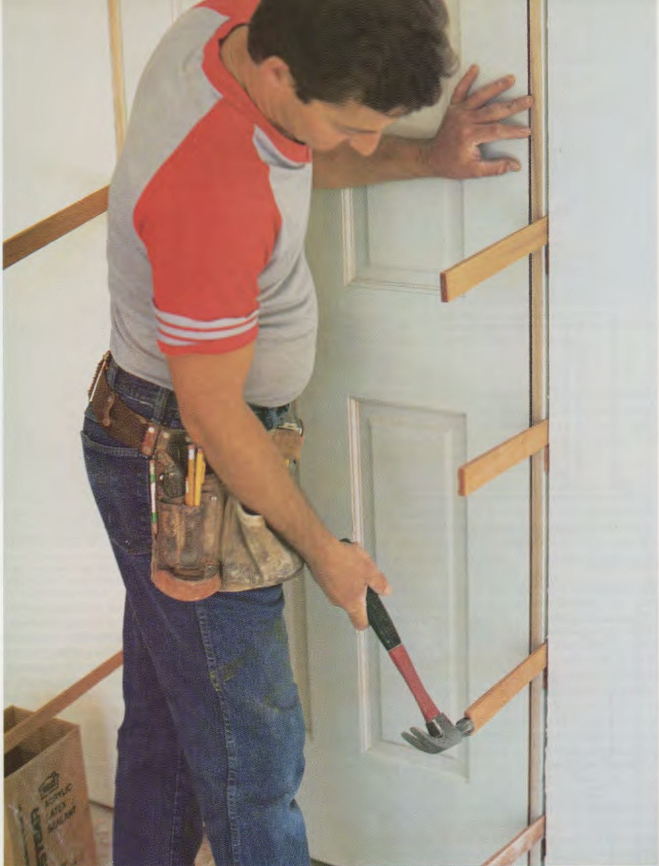
Hanging and trimming a door, the most complex and demanding job the finish carpenter must do, starts with setting and shimming the jamb.
