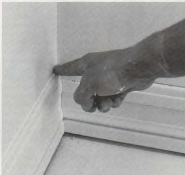
A standard caulking gun (top), preferably one without a notched feed plunger, is fine for caulking gaps in baseboard and casings. Cut the tube's tip at an angle and apply a fine bead, then smooth it with a moistened finger, as shown above.
