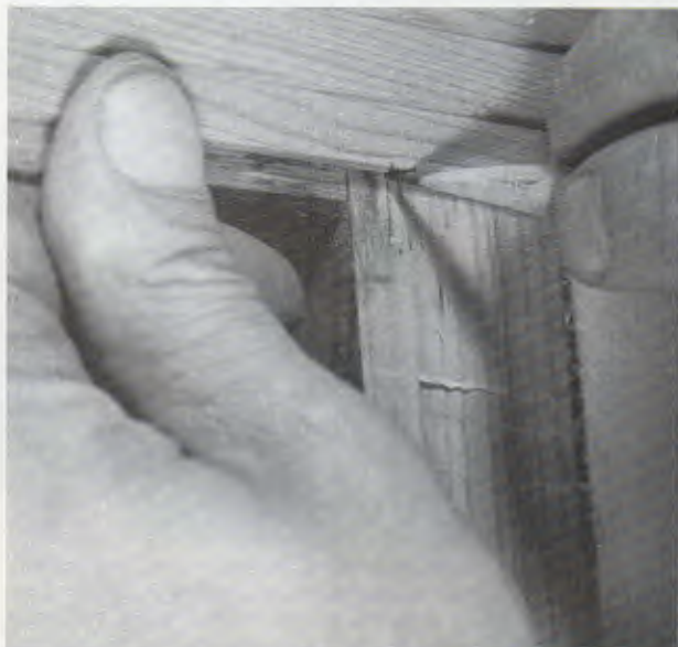
The length of a picture-frame window's head casing can be scribed directly from the reveal marks.
