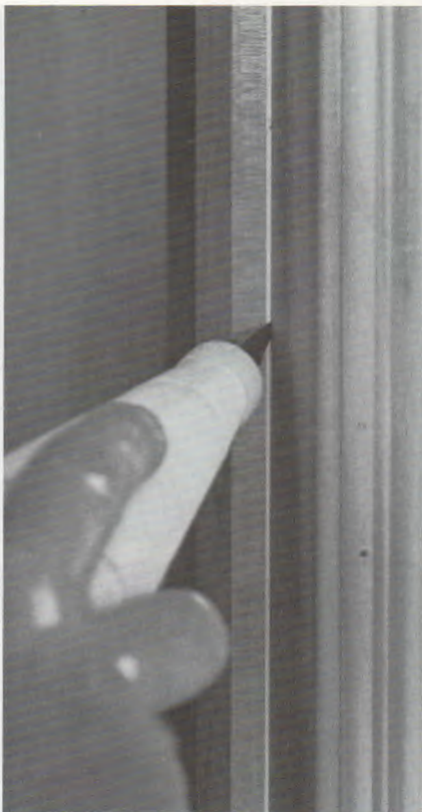
To apply a fine bead of caulk between joined parts, an icing bag is ideal. Icing bags are sold by bakery-supply outlets (and by some paint stores) and can be bought with tips of various sizes.
