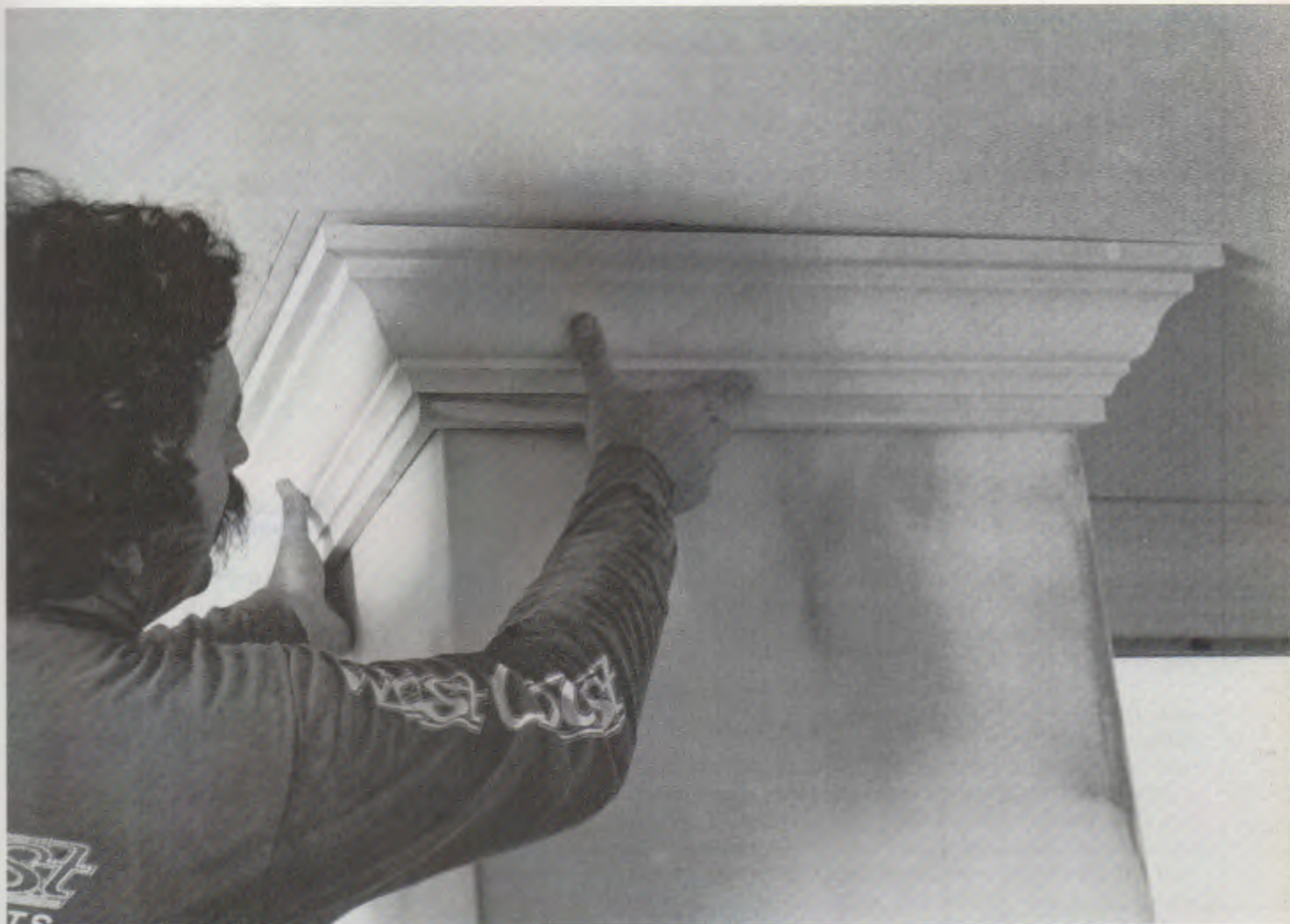
Crown molding turns outside corners with a miter joint. If possible, try to avoid finishing off a room with two outside miters. A cope or butt at one end will be more forgiving.
