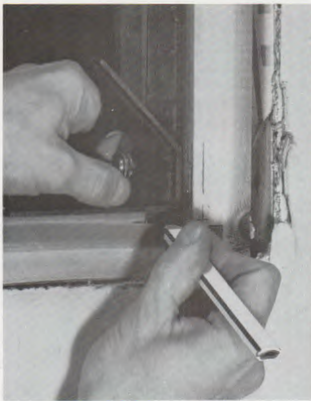
Two tools for marking casing reveals are the reveal gauge, top, and the combination square, above. The reveal gauge is a square scrap block with rabbets milled in all four edges, each corresponding to a common reveal dimension. The combination square can be set to the reveal and used as a marking gauge.
