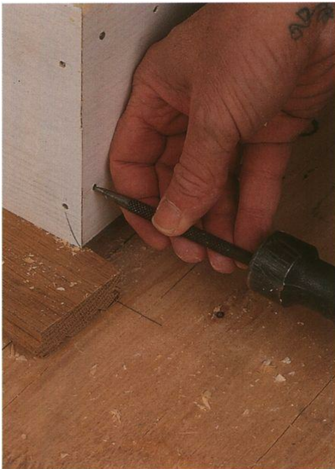
Nail from both sides of the outside corner and set the nails.
