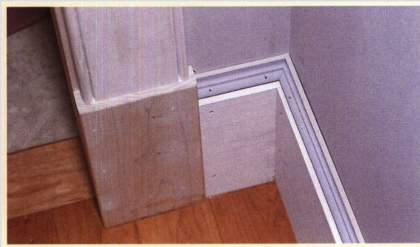
B. Inside corner at door casing.
