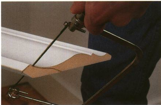
After cutting a reverse bevel, cut the profile with a coping saw.
