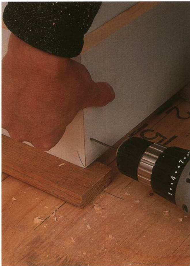
Predrill before nailing at the outside corners to avoid splitting the ends.
