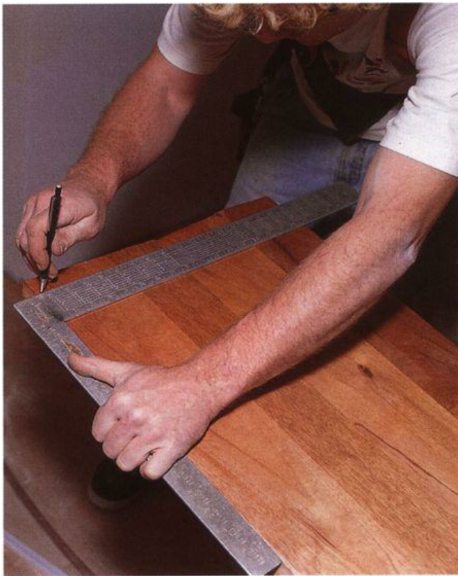
Carpenter Larz Allen squares up the end of a solid-wood countertop with a framing square.
