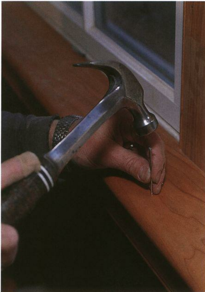
Nail through the stool to secure the top edge of the apron.
