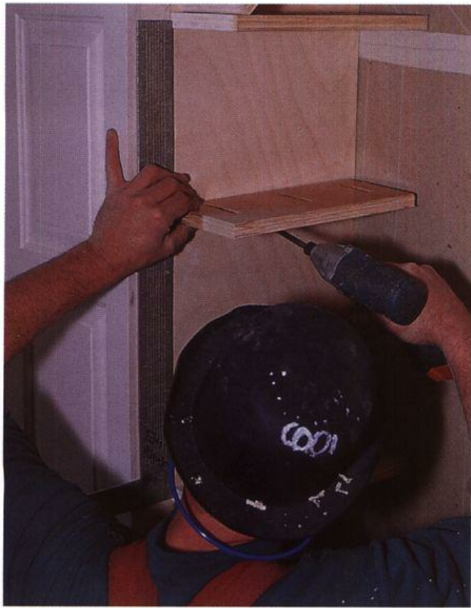
Plywood fins can be quickly installed on a cabinet (here, on the base of a case-style window bench). Use a framing square to align the fins, which have been predrilled for pocket screws.
