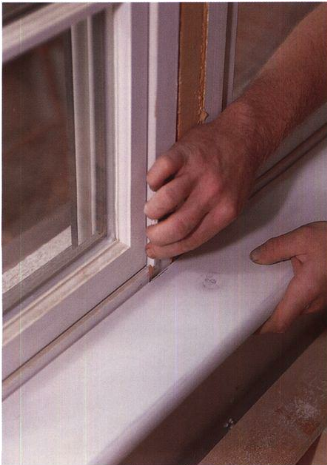
The stool may need to be scribed to fit tightly against a large window unit.
