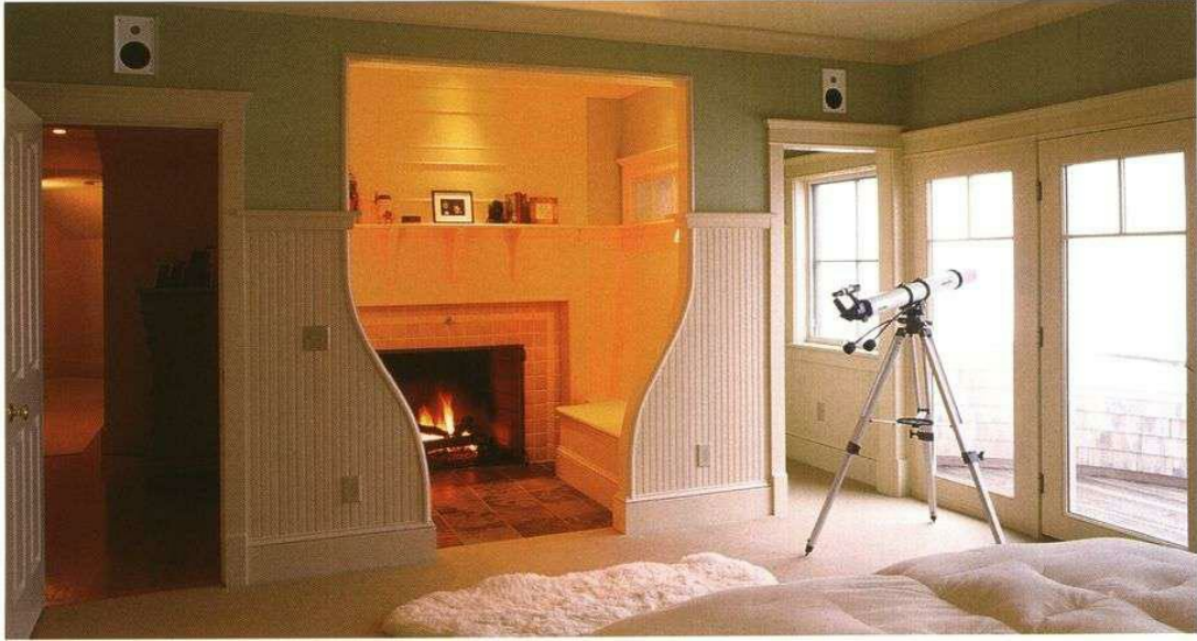
Tall wainscoting, applied to just one wall, requires minimal work but provides a distinctive interior touch.
