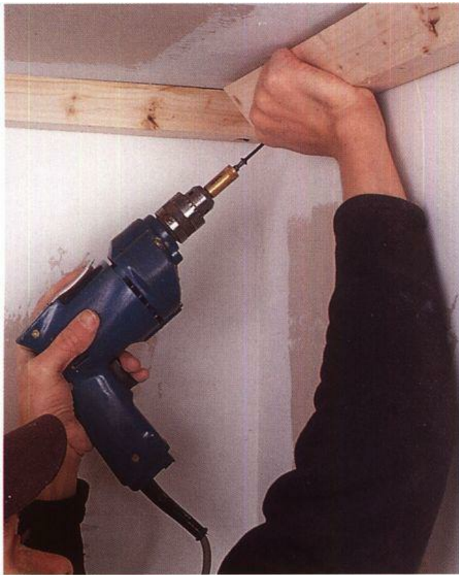
Backer can be screwed to the top wall plates; it doesn't have to be pretty, just secure.
