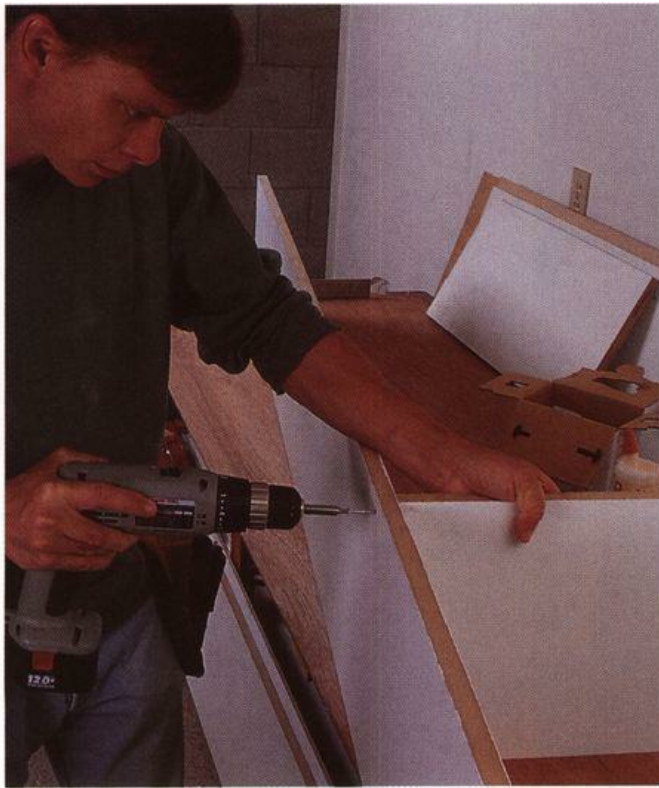
If the side of the shelf unit will not be seen, it can be secured with screws, which hold better in the panel end grain.
