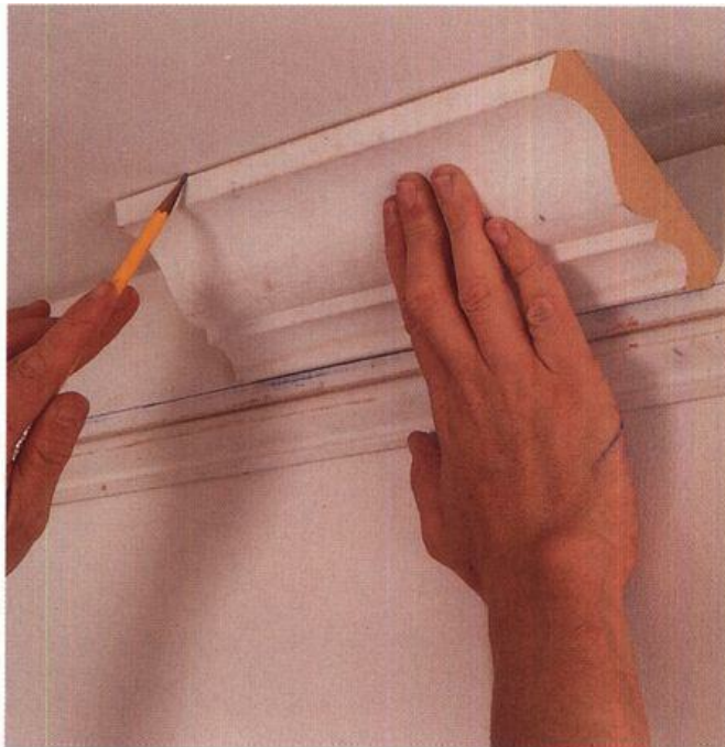
Check the fit of the top ceiling board with scrap crown molding.
