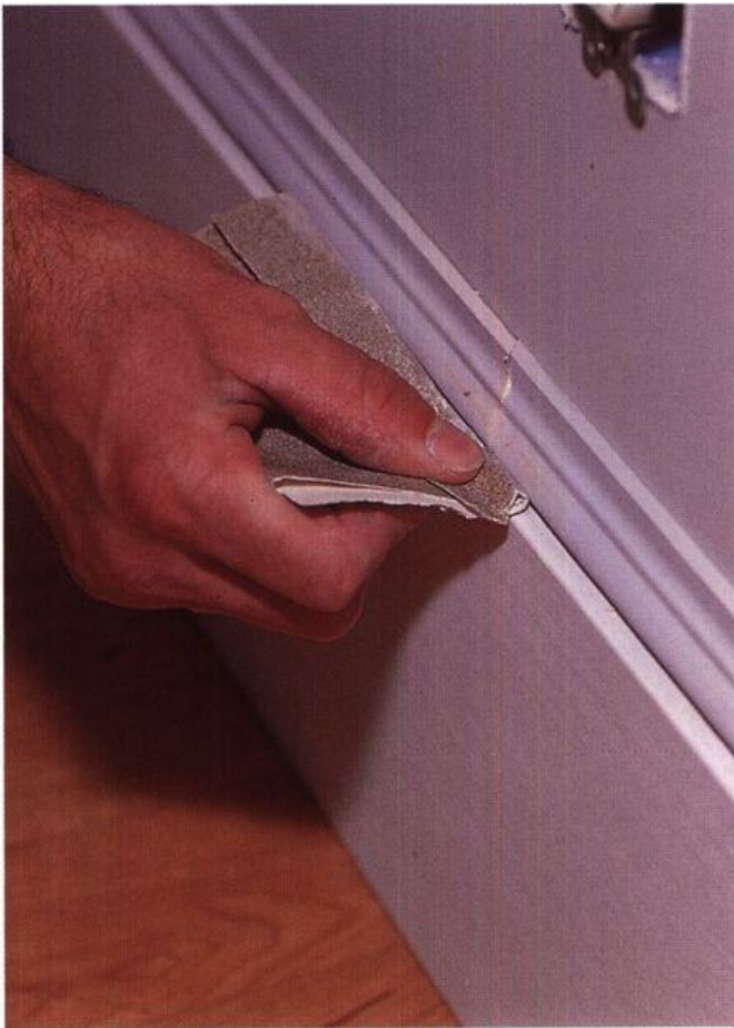
After nailing through the scarf joint, smooth the joint with sandpaper.
