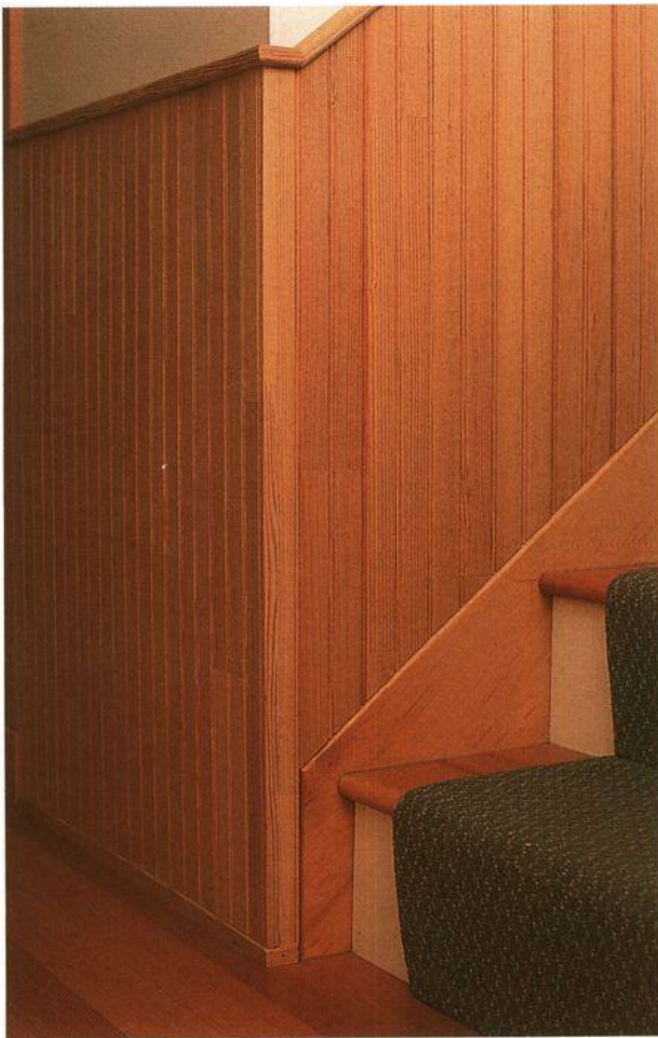
Bead-board wainscoting is the simplest to install and just as elegant as raised-panel wainscoting.
