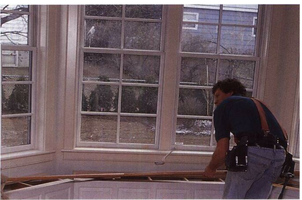
Case cabinet construction methods can be adapted to build a window.
