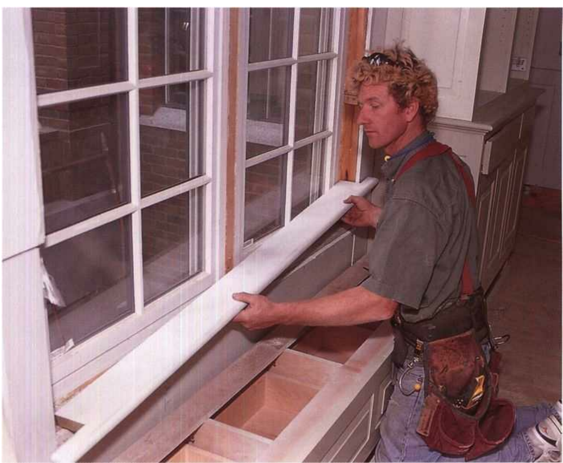
Then test-fit the stool.
