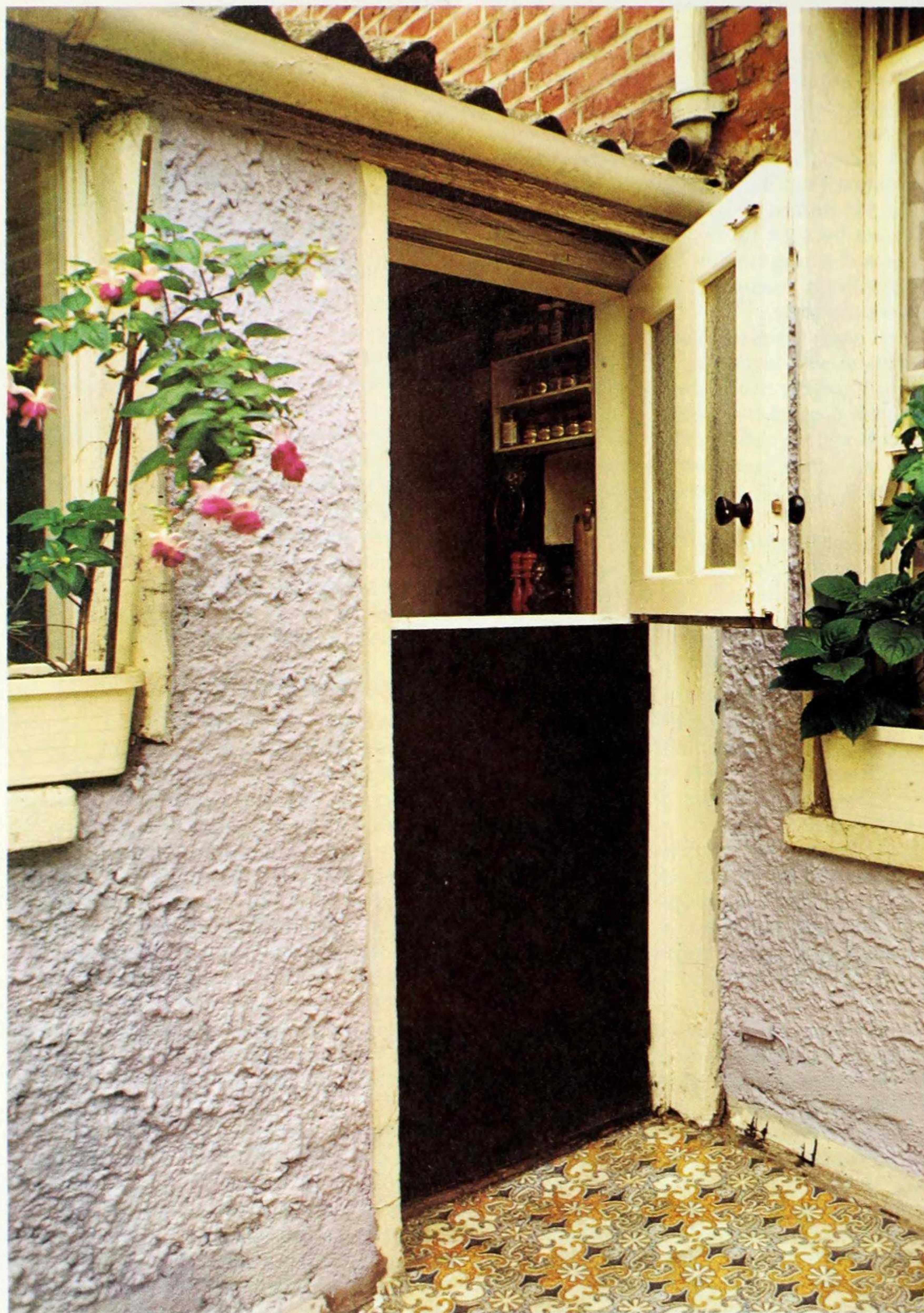
Left. A Dutch door from the kitchen to the garden prevents children tramping in and out on a wet day and yet provides extra ventilation.
