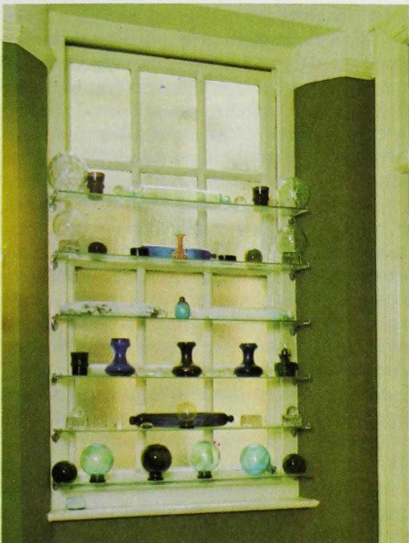
Fig. 9 (center left). Glass shelves are ideal for ornaments. Fig. 10 (below). They can be mounted invisibly on clear plastic buttons.
