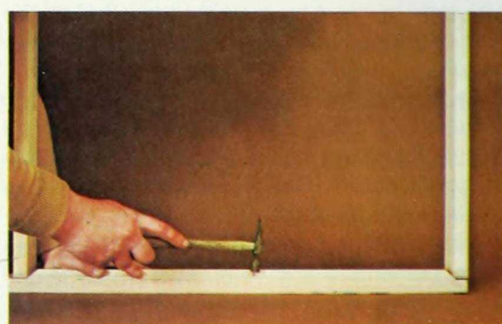
Fig. 6. Initially, tack the first length of cove molding in the middle only. This allows for adjustment when fitting the other pieces.
