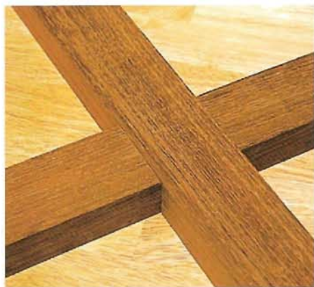
Above The completed cross-halved joint.
