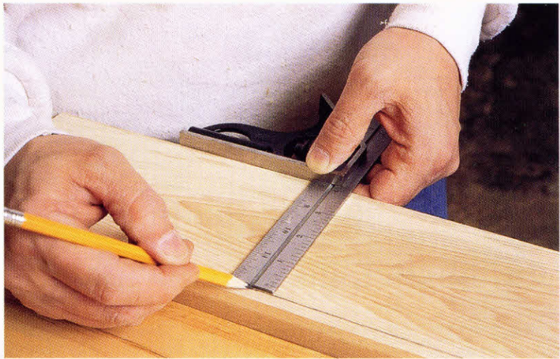
2-4. ♦ Here, a combination square is used to mark a board for a rip cut with a handsaw.
