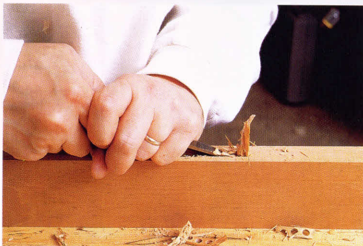
6-22. ♦ Using a narrow chisel to clean out the mortise waste. I am careful not to cut into the ends of the mortise as I do this.
