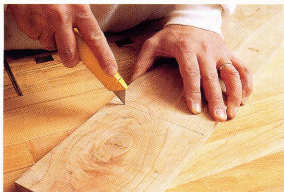
2-13. ♦ Deepen the line with a utility knife.
