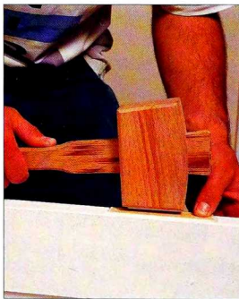
2 Add adhesive and tap the wood — sliver down into the recess.
