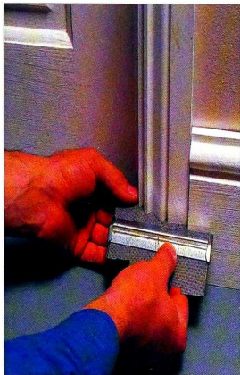
Above Use a profile gauge to transfer the shape of small obstacles to panels.
