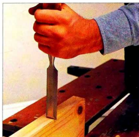
10 Chop out the waste with a chisel working along the scribed line.
