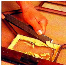
13 While the plaster is still malleable, trim away the excess with a chisel.
