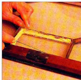
11 Press the glass gently into position on the wet plaster.
