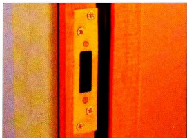
Above A striking plate set in an internal frame.
