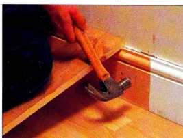
4 Hammer nails into the new section of board while holding a plank against the wood.
