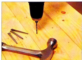
Above Drill pilot holes for floorboard nails to avoid splitting the wood.
