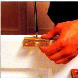
11 Insert the hinge into the recess and screw up tightly.
