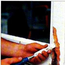
1 Chisel out all the rotten wood, making sure only sound wood is left.
