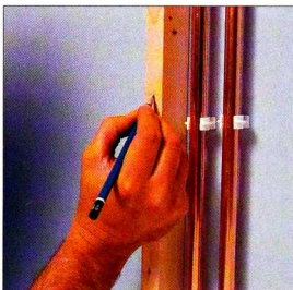
2 With a pencil, mark the positions for the side batten fixings.
