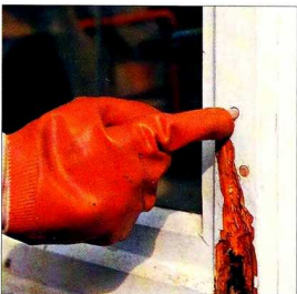
4 Push preservative sticks into the drilled holes and below the surface.
