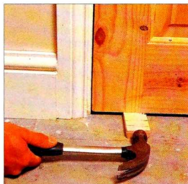
4 Offer the door into the frame. Use a wedge to square up if need be.
