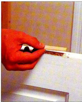
1 To fill an old hinge recess, cut a — sliver of wood slightly over size.
