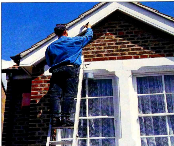
Above Paint bargeboards early on in your work schedule. By starting from the top and working down you ensure that any dislodged dirt or paint droplets only fall on unpainted surfaces.
