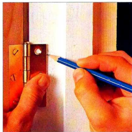
12 Mark the other part of the hinge on the door frame with a pencil.
