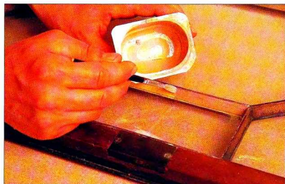
14 When the plaster is dry, stain it with a water-based stain mixed to match the colour of the original putty.
