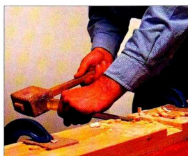
Above Use a chisel to cut a slot to fit over a joist if the board is too thick.
