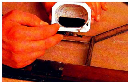
15 Apply a darker stain on top of the coloured plaster to try to mimic the patina of the original putty. This should blend the repaired glazed panel to match the others.
