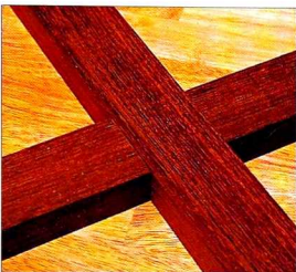
Above The completed cross-halved joint.
