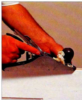
3 When the adhesive has set, plane — the surface flush and smooth.
