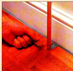
Above Drill a hole and cut out a strip to fit a panel around a pipe.
