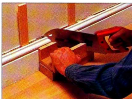
2 Cut away the damaged section with a mitre box and a saw.
