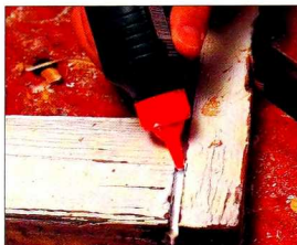
Above A loose window joint can be re-glued with fresh adhesive. Clamp it up while the adhesive dries.
