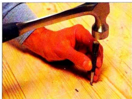
Above Hammer down protruding nails to prevent them damaging the floor covering.
