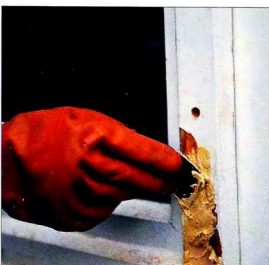
5 Fill the damaged area with exterior wood filler. Leave to dry before sanding.
