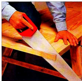
6 Saw off the bulk of the waste using your knee as a support on the end of the door.
