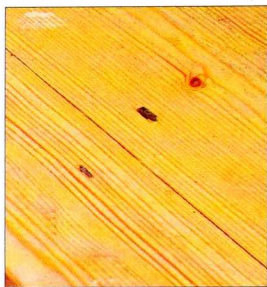
Above Punch any protruding floorboard nails below the surface of the wood to prevent them from damaging the new floorcovering.
