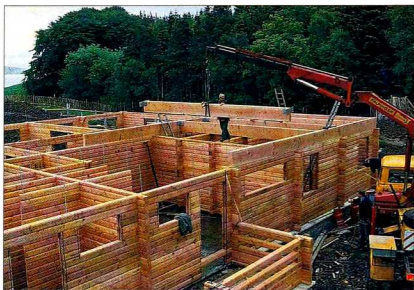
Above Houses being constructed from timber (lumber).
