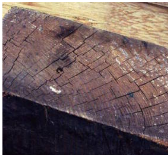
Splits typically radiate outward from the pith. Separations between the growth rings are called cup shakes . Although often hard to see, they're clearly evident on the end of this board.
