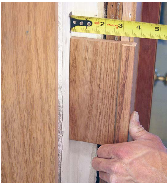
DOUBLE PLINTH BLOCK. At a corner, make a plinth block with two pieces fastened together. Rout the edges of only one side of each piece. (This doubled plinth is seen in the top left photo on p. 142).
