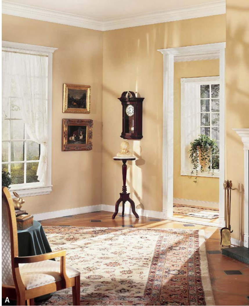
A The crown molding, fireplace mantel, and tops of the door and window in this room all share the same flared trim profile.
