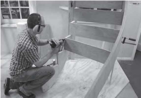
Figure 8.113 The risers (all except numbers 1 and 8) are installed ahead of the treads, and the circular staircase begins to take shape.
