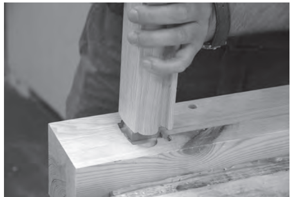
Figure 11.23 When the housing is complete, the handrail is offered back into its mortise.
