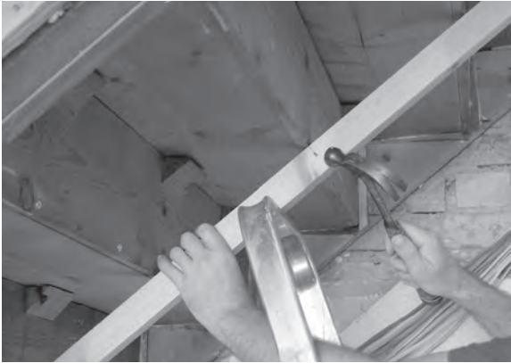
Figure 12.20 A narrow carriage is nailed temporarily to the steps, prior to marking.
