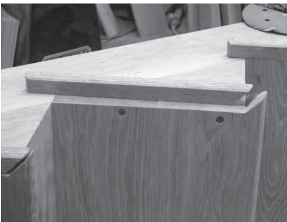
Figure 10.52 The treads are fixed to the open strings with glue and countersunk screws, before the nosing/scotia mitred returns are attached.
