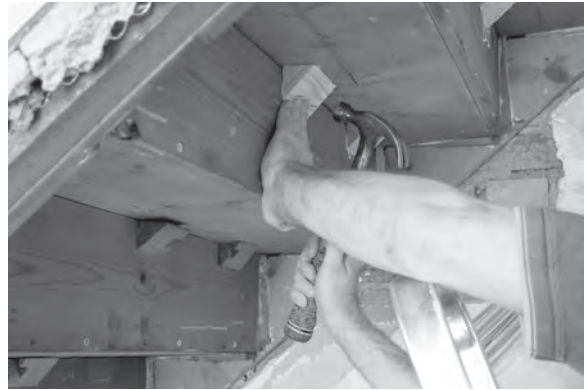
Figure 12.18 New glue blocks are held in place with pins while the glue dries.
