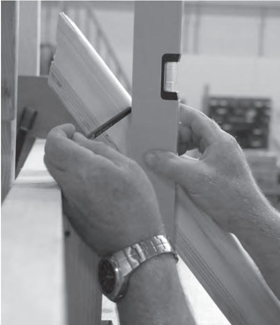
Figure 11.93 (above) and Figure 11.94 (below) Plumbing up from the line marked on the upper tread to form the handrail shoulder line can be done with a spirit level or steel roofing square.
