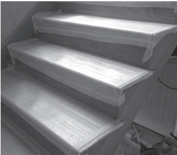
Figure 10.56 The stairs are protected during installation with sheet foam covering the treads. (Photo courtesy of Frank Turtle)
