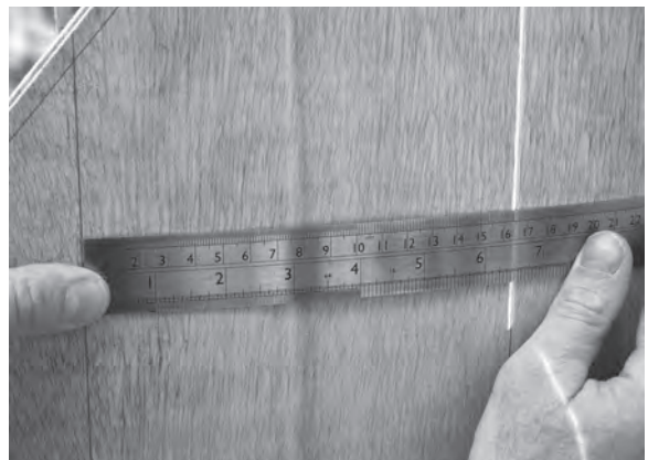
Figure 8.54 As the riser lines are marked on the string, the accuracy of the goings should be checked regularly.
