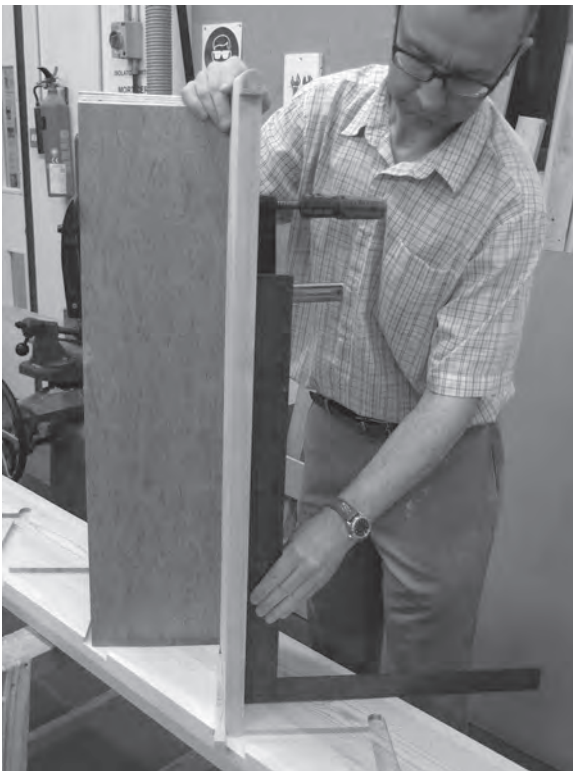
Figure 5.51 The opposite ends of the steps are held together with F-clamps; before continuing, use a steel roofing square to check that the steps are perpendicular to the string.
