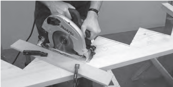
Figure 5.16 (above) and Figure 5.17 (below) The first cut when mitring the outer string is parallel with the riser lines.
