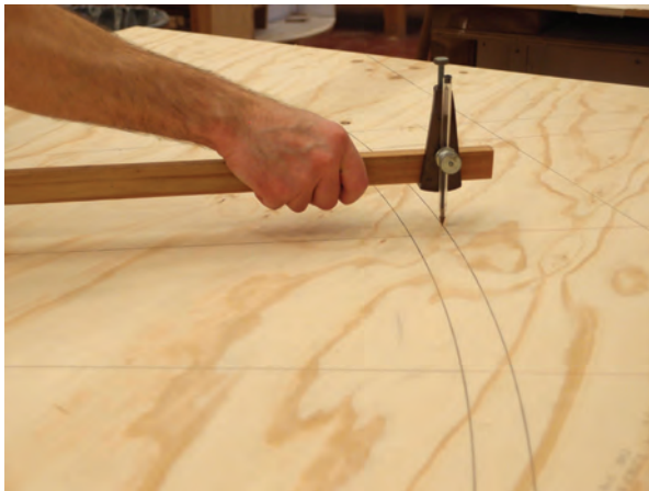
Above: Trammel heads clamped to a timber batten: perfect for setting out circular stair strings on a sheet of plywood. See page 119.
