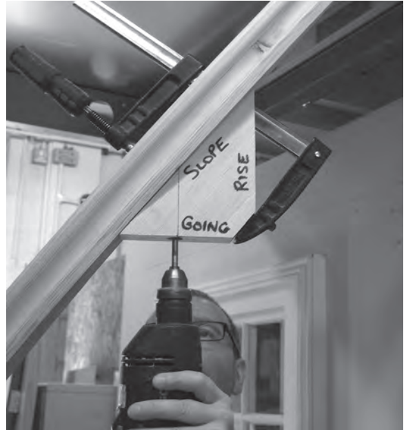
Figure 11.108 A pitch block clamped to the handrail is a useful aid which ensures that holes are drilled plumb and to the correct depth.
