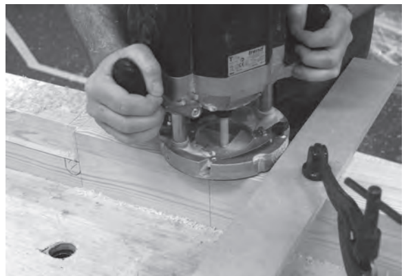
Figure 5.26 Use a straight edge when routing across the grain of the newel posts.
