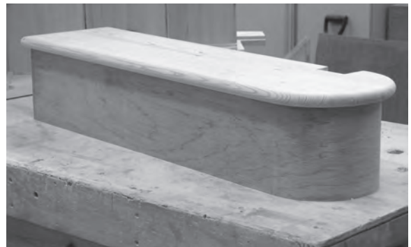
Figure 5.70 A D-step is an attractive starting step for a staircase (compare with curtain step, Figure 8.126).
