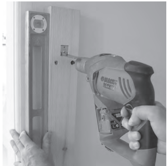
Figure 12.56 Plumb and screw the half newel to the wall using suitable fixings.
