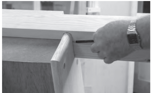
Figure 11.91 Mark a line on the upper tread where it meets with the top newel post.
