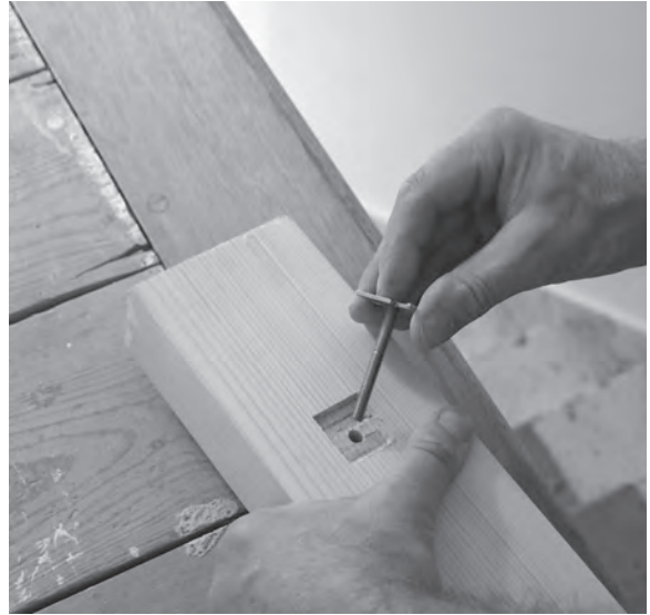
Figure 12.51 (above) and Figure 12.52 (below) The threaded portion of the Richard Burbidge handrail bracket is passed through the half newel and secured from behind with a nut and washer.
