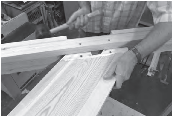
Figure 6.85 Timber bruising is avoided by using a rubber mallet to tap the newel post home.
