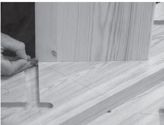
Figure 4.50 The rear of the tread is marked to finish flush with the face of the following riser.
