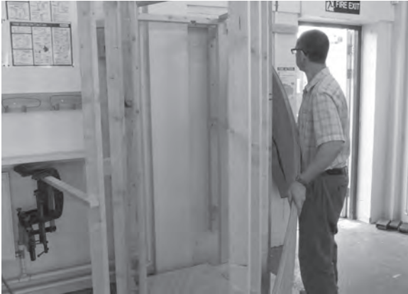
Figure 8.42 The wall string is carefully removed from the form.
