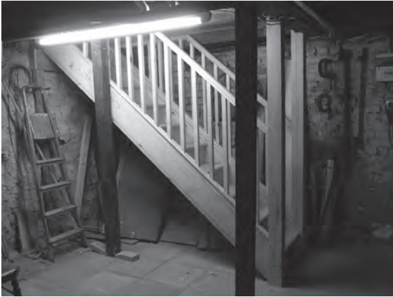
Figure 4.98 The installation is complete, making access to this cellar safe and comfortable.
