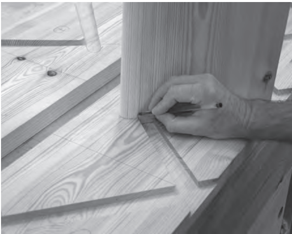
Figure 4.49 With a tread pushed fully into a housing, the riser position can be marked on the underside.
