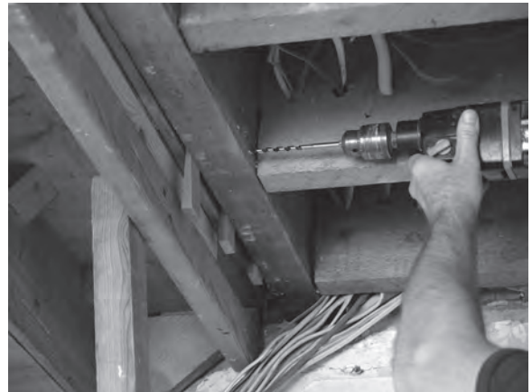
Figure 12.15 The space between the top riser and trimmer joist is packed prior to screwing, and clearance holes are drilled through the trimmer joist.
