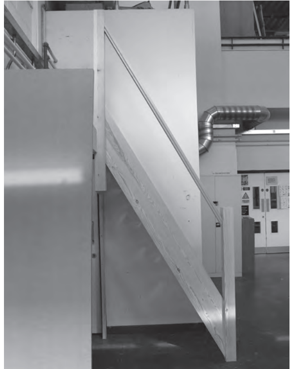
Figure 9.72 The very steep angle of pitch is evident from this side profile.
