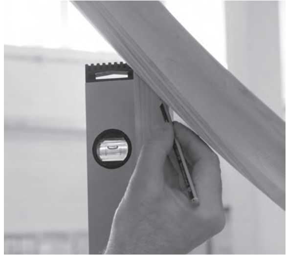
Figure 11.105 The plumb baluster is marked against the underside of the handrail and then adjusted to suit the depth of the groove.
