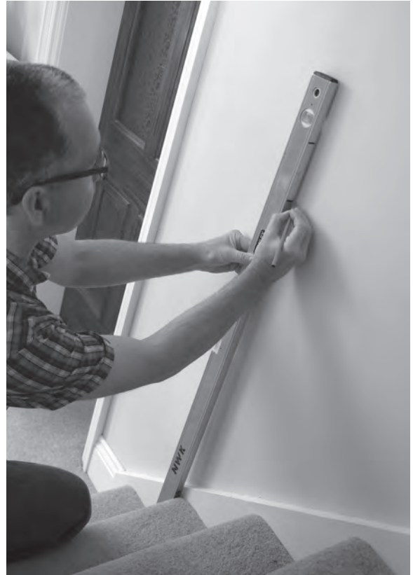
Figure 12.70 The brackets' fixing height is marked from the spirit level to the wall at the top and bottom of the stairs.
