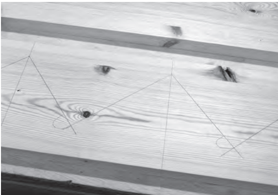
Figure 4.18 Defects should be concealed beneath the steps wherever possible.
