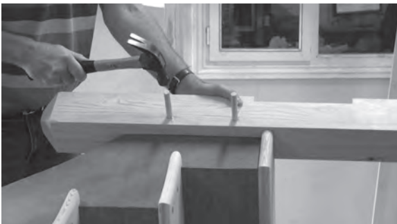
Figure 8.133 Pull the newel post up tightly by draw-bore dowelling through offset holes.
