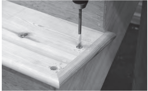
Figure 11.39 The treads are drilled to receive 18mm dowel.
