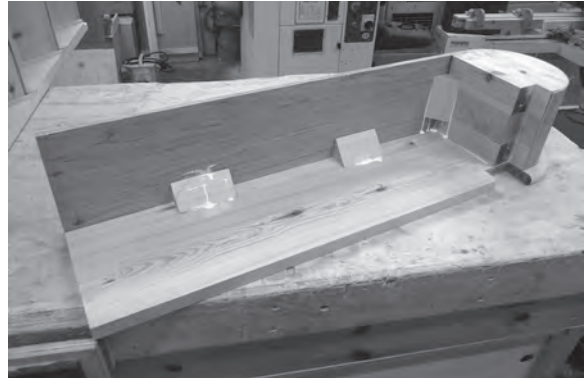
Figure 10.29 The D-step viewed from the underside. Glue blocks provide additional support where tread and riser meet.
