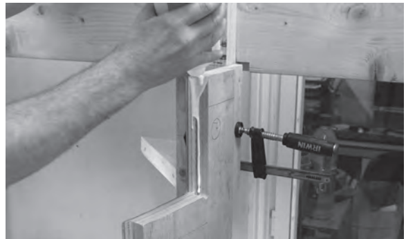
Figure 8.111 Apply PVA adhesive to the mitred ends of the open string. Start at the top of the string and work downwards.
