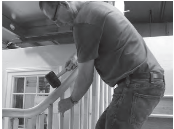
Figure 11.121 The installation and lowering of the handrail onto the tops of the balusters is a two-person job.
