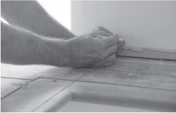
Figure 12.49 (previous page) and Figure 12.50 The new balustrade must run parallel to the landing nosing, so a string line is used to accurately mark the location of the half newel on the facing wall.
