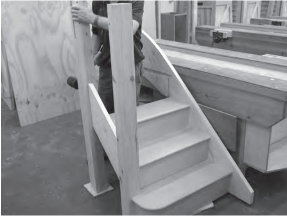
Figure 6.74 (above) and Figure 6.75 (below) The return flight is levelled and the intermediate newel post tested for fit.
