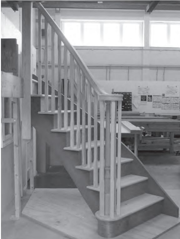
Figure 11.126 The completed circular staircase and balustrade.
