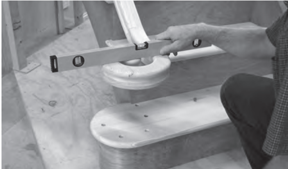
Figure 11.96 Prepare for marking the top newel's mortise by repositioning the handrail and checking that the volute is level across its width (as seen here) and length.
