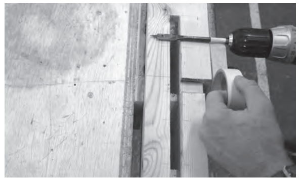
Figure 4.62 Masking tape wrapped around the bit ensures correct depth of hole.
