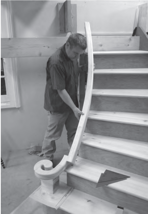
Figure 11.80 With the volute raised on timber blocks directly above the template, Steve positions the handrail next to it.
