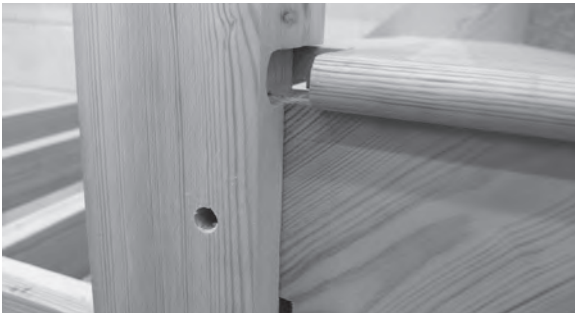
Figure 5.75 The upper flight's cut string meeting with the intermediate newel post.
