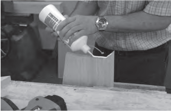
Figure 8.93 Apply a generous amount of PVA glue to the tread's mitred end.
