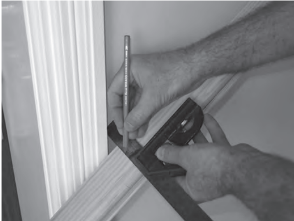
Figure 12.82 The handrail is marked to length at the top and bottom of the staircase.
