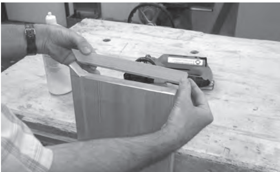
Figure 5.41 Apply a generous amount of glue to a tread's mitred end, line up the corresponding nosing return, and bring the two components together.
