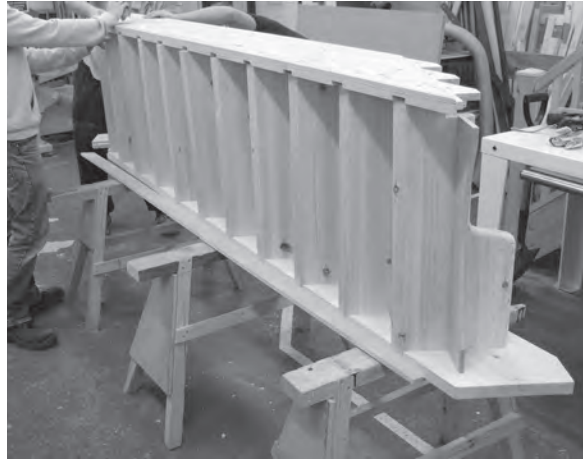
Figure 9.57 Lift the outer string into place, carefully locating the treads and risers into their housings.
