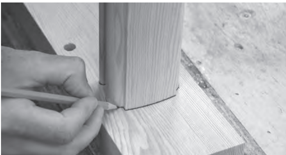
Figure 11.19 (above) and Figure 11.20 (below) Offer the horizontal handrail into the newel post's mortise and draw tightly around its profile with a sharp pencil, before removing and setting aside.
