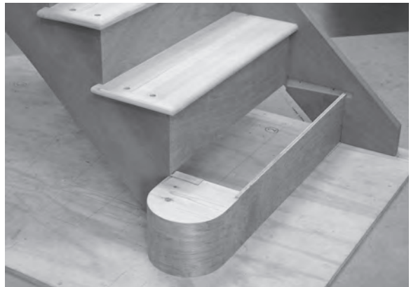
Figure 8.129 We are now ready to install tread number 1.
