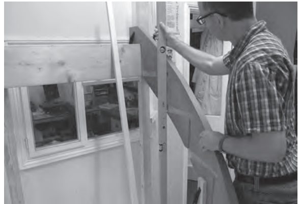
Figure 8.109 Check for plumb with a spirit level.
