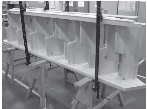
Figure 9.58 Apply pressure to the strings of the assembled staircase. Avoid clamp indentation by positioning narrow timber strips which also allow access to the strings' screw holes.
