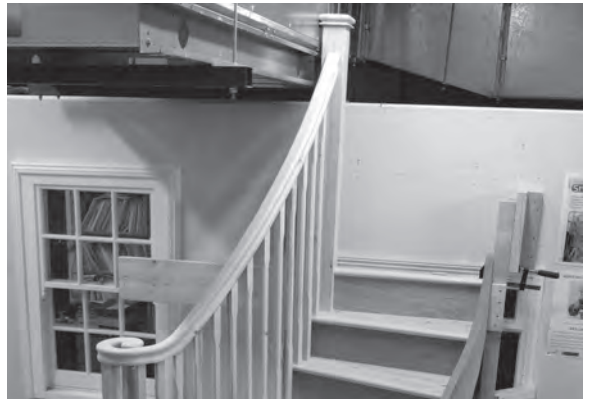
Figure 11.125 A cap on top of the top newel provides a finishing touch.
