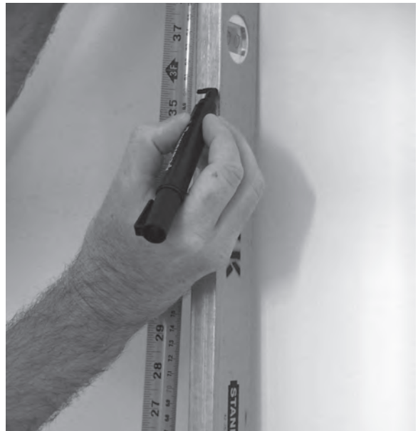
Figure 12.68 From the pitch line mark, the desired handrail height is also marked onto the edge of the spirit level.
