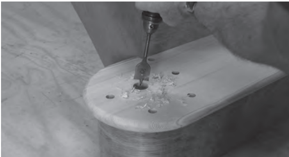
Figure 11.100 The hole for the volute newel's spigot is drilled through the curtail tread into the solid block below at the location marked using the volute template.
