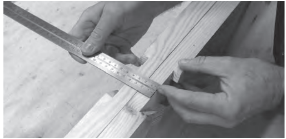
Figure 4.57 Ensure that the treads and risers are cut to the correct length by measuring the combined thickness of the strings, where there is a housing, and deducting this measurement from the overall width of the staircase.
