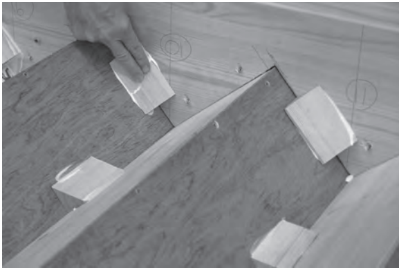
Figure 7.24 Apply glue blocks beneath the steps and where the treads and risers meet the outer string.
