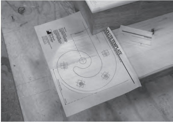
Figure 11.73 The template can be used after staircase assembly by trimming its corner so that it fits around the second riser and string while still aligned with the balustrade centre line.
