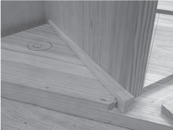
Figure 4.73 Glue blocks should be not less than 75 mm long with a sectional size of at least 38 mm × 38 mm.
