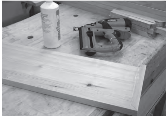
Figure 5.43 Set aside to dry while continuing with the rest of the treads and nosing returns.
