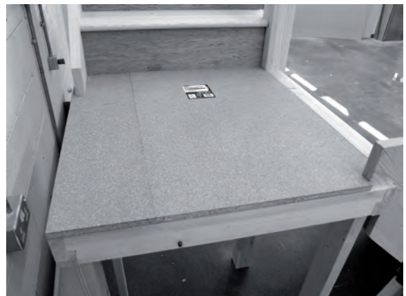
Figure 5.78 With space limited, the quarter landing is often decked before the lower flight is offered up.
