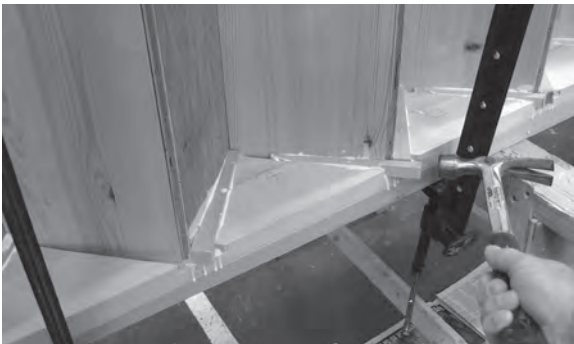
Figure 5.63 Glue and wedge all treads and risers to the wall string.
