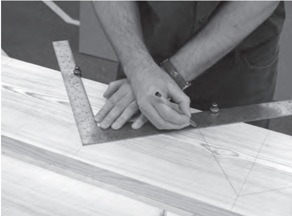
Figure 4.24 Steps on strings being marked with stair gauges fixed to a steel roofing square.
