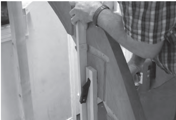
Figure 8.108 Check the height with the storey rod and prop the mid-part of the string.
