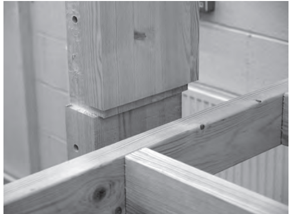
Figure 7.26 (above) and Figure 7.27 (below) The half landing's trimmer joist is screwed to the notched intermediate newel post.
