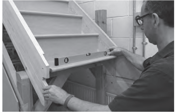
Figure 6.92 Check the flight for level.
