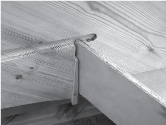
Figure 6.79 (above) and Figure 6.80 (below) Riser number 5 being lifted into its housings and held in place with a wedge. For clarity, the kite winder has been omitted.
