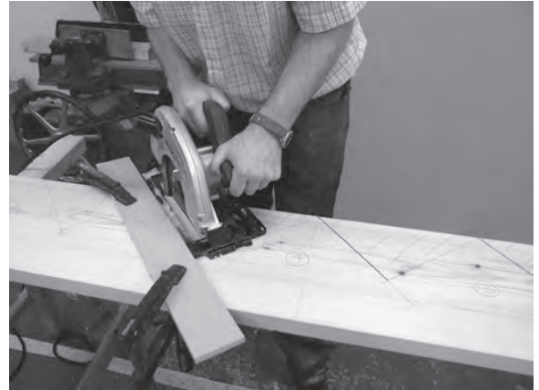
Figure 5.13 Cutting the steps of the outer string using a hand-held circular saw guided by a straight edge.
