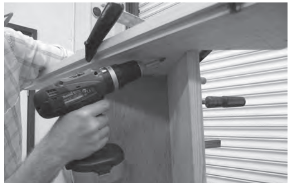
Figure 7.19 The outer string is pocket-screwed into the underside of the treads.
