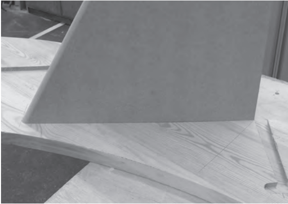
Figure 6.58 The wide side of the skew winder is seen here sitting nicely within its housing in the wall string.
