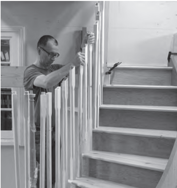
Figure 11.119 The trimmed and numbered balusters are glued into their respective dowel holes in the treads.
