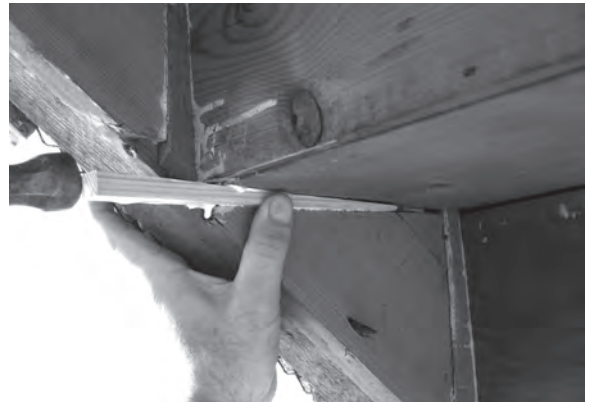
Figure 12.7 (above) and Figure 12.8 (below) Replace all loose and missing wedges if the flight's underside is accessible.
