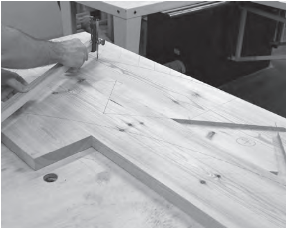
Figure 6.25 (above), Figure 6.26 (below), and Figure 6.27 (bottom) Use your preferred method for marking the string easings.
