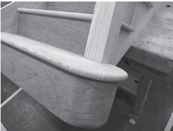
Figure 5.72 The outside of the lower flight, showing D-step, newel post, and cut string.
