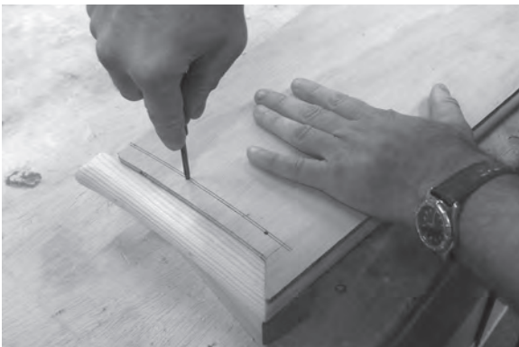
Figure 8.99 Use the template to mark the screw positions which should coincide with future balusters.
