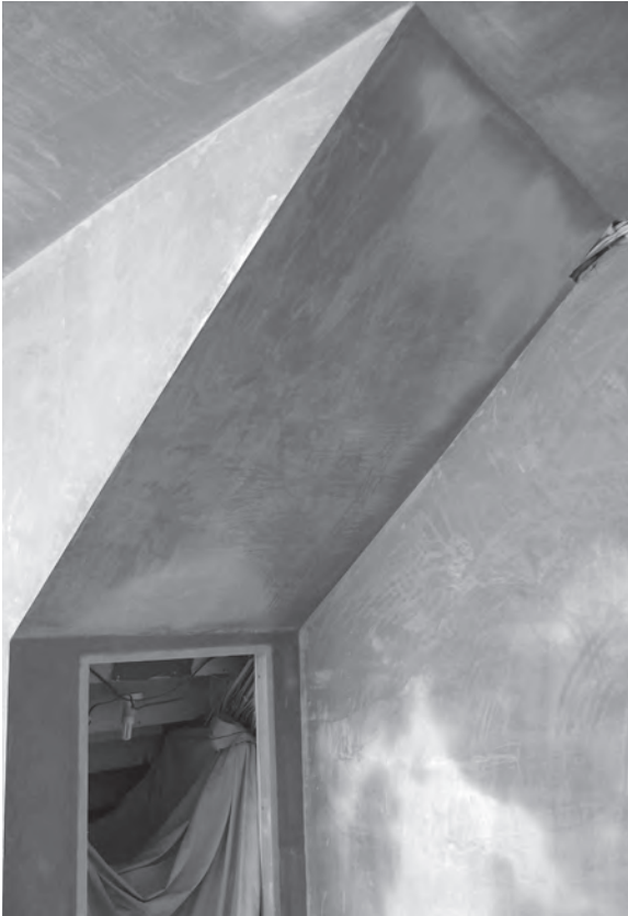
Figure 12.29 The room is plaster-skimmed, and the short section of electric cables still exposed (top right-hand corner) will soon be covered by cornice.
