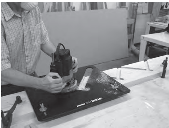
Figure 5.12 Working from left to right, rout the wall string housings to a depth of 12 mm.
