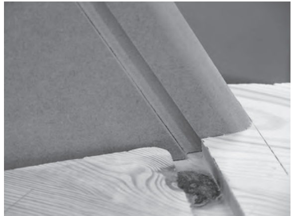
Figure 6.56 The skew winder now fits nicely within its housing, the tread's nosing is fully up, and the riser housings are perfectly aligned (compare with Figure 6.51).
