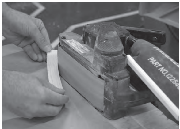
Figure 8.92 Use a belt sander to clean up the nosing returns' outside edges only.
