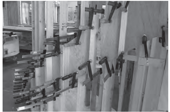
Figure 8.39 Clamping against wooden blocks between studs ensures that good contact is made between the layers, and that gaps are avoided.
