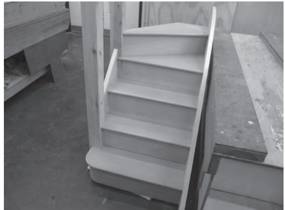
Figure 6.83 The square and kite winders (numbers 4 and 5), together with their risers, are fitted as part of the return flight.
