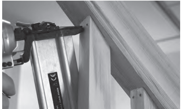
Figure 11.124 As well as gluing and dowelling, each baluster is nailed through its upper rear portion into the handrail.
