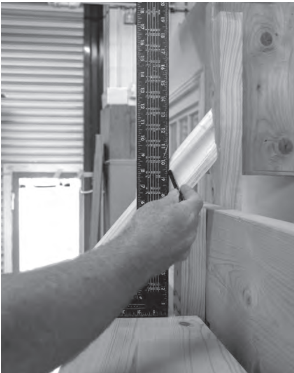
Figure 11.93 (above) and Figure 11.94 (below) Plumbing up from the line marked on the upper tread to form the handrail shoulder line can be done with a spirit level or steel roofing square.
