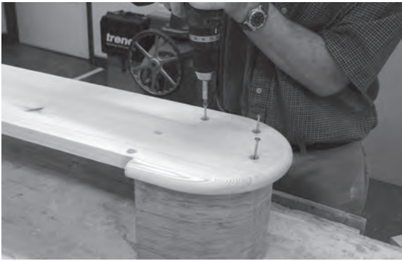
Figure 10.27 The curtail tread is screwed down into the laminated block through its pre-drilled holes.
