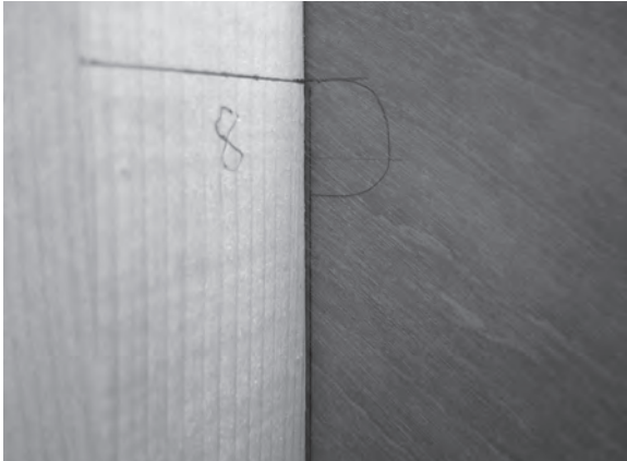
Figure 8.33 This close-up shows perfect alignment between the marked facing plywood and the stud at tread number 8.
