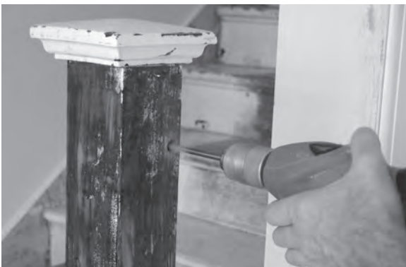
Figure 12.34 Prepare for draw-bore pinning by drilling a 12mm diameter hole into the newel post's side and through the mortise.
