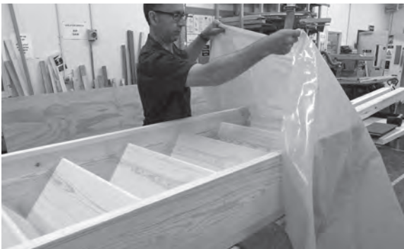
Figure 4.95 Cover the finished staircase with heavy-gauge polythene for protection during delivery and while on site.
