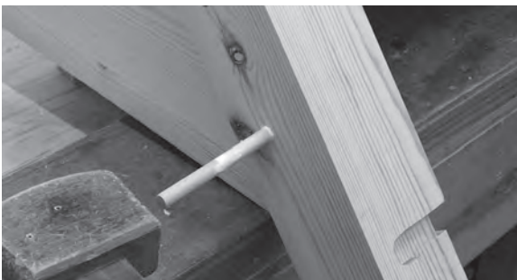
Figure 6.67 Drive wooden dowel, tapered at the end and glued, into pre-prepared holes drilled through the newel post and string tenon.
