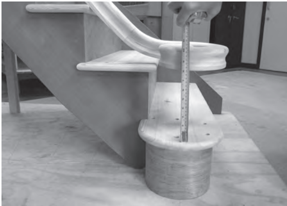
Figure 11.97 Carefully measure the height from the top of the curtail tread to the underside of the levelled volute.
