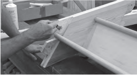
Figure 6.65 The return flight's outer string tenon is glued to receive the bottom newel post. Check that there is sufficient access on site before undertaking this task.
