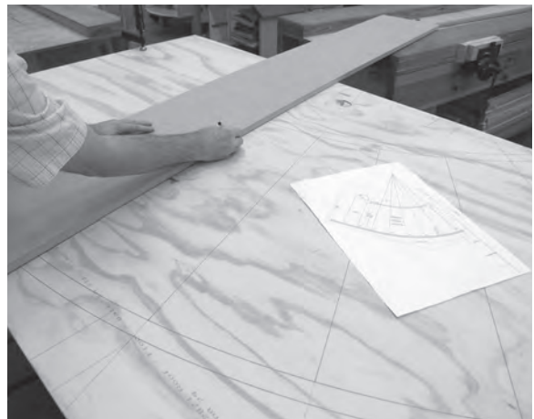
Figure 8.5 Having set out the tread positions, a straight edge, radiating from the geometric centre, is used to mark the riser lines.
