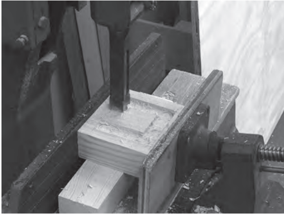
Figure 10.66 A mortiser is used to trench out the underside of the newel cap to suit the size of the newel post.
