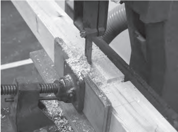
Figure 5.27 With the tread and riser housings routed, the newel posts are mortised for joining to the outer strings.
