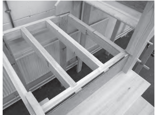
Figure 5.85 The quarter landing, with decking removed, showing timber shims between the trimmer joist and riser.
