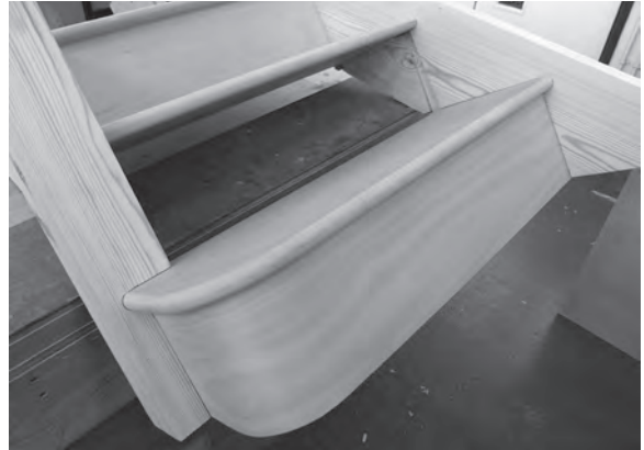
Figure 6.72 The bullnose step dry-fitted into its housings.
