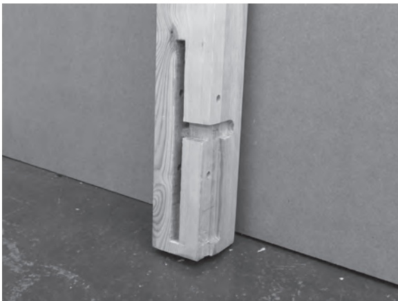
Figure 4.47 Sides 2 and 3 of the right-hand newel post.
