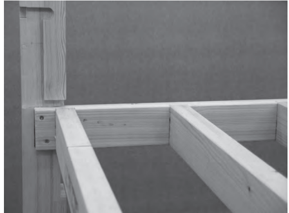
Figure 5.73 The outer corner of the quarter landing is supported by the intermediate newel post and, for speed, is often butted and screwed rather than 'let in', as seen here.
