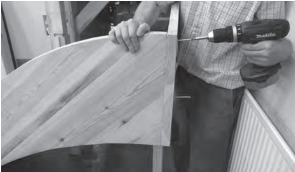
Figure 6.95 With the lower end of the main flight pulled clear of the wall, the strings are dry-fixed together, connecting the main and return flights.
