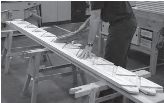
Figure 4.80 The first of the two strings is laid on top of the board. Ensure that the housings are free of dust.
