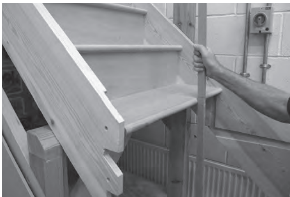
Figure 6.91 Use a storey rod to confirm that tread number seven is at the correct height.
