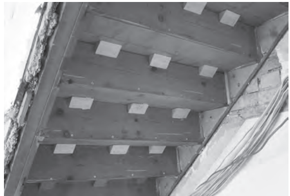
Figure 12.19 Few of the old glue blocks remain. Note the electric cables hanging beneath the flight.
