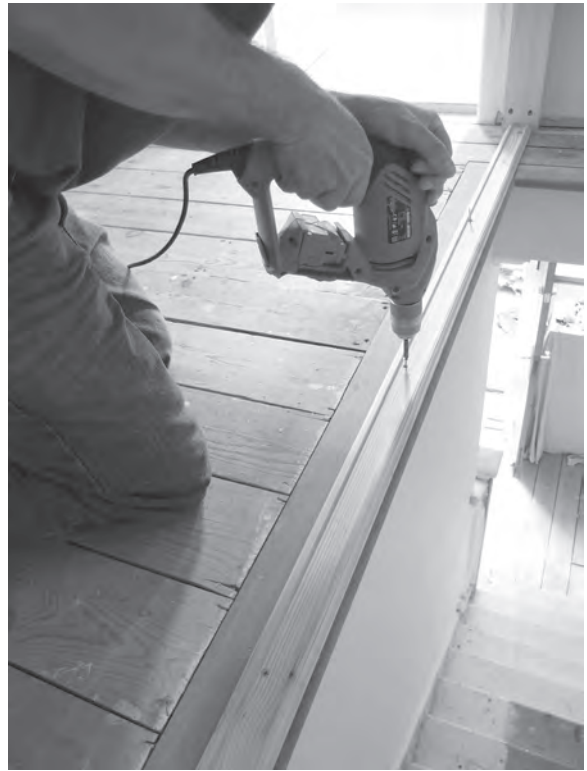
Figure 12.59 The baserail is fixed to the floor using 4.0 \times 32\text{ mm} wood screws ( 1\frac{1}{4} inch 8s) at centres not exceeding 230 mm.
