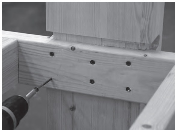
Figure 7.26 (above) and Figure 7.27 (below) The half landing's trimmer joist is screwed to the notched intermediate newel post.
