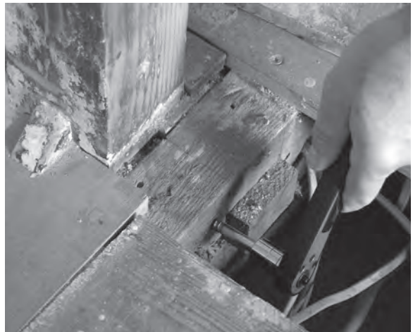
Figure 12.42 (above), Figure 12.43 (below), and Figure 12.44 (bottom of page) The loose newel post is secured to the adjacent trimming joist with two coach screws.
