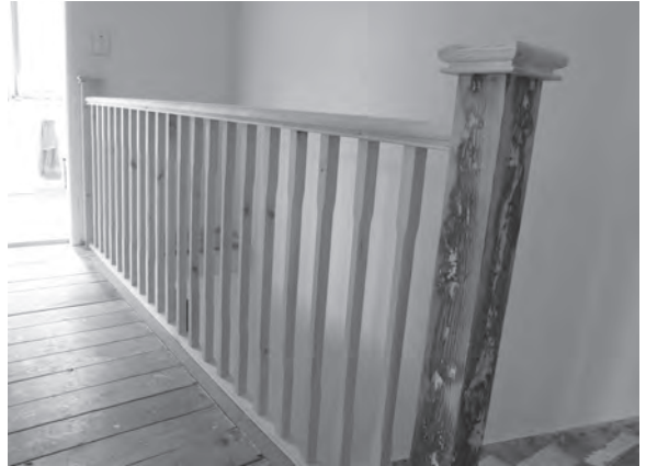
Figure 12.63 The newly installed balcony railing.
