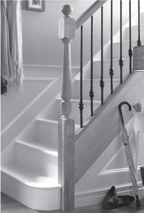
Figure 10.30 The quarter-round of a bullnose starting step provides an attractive feature at the foot of a staircase. (Photo courtesy of Richard Burbidge Ltd)
