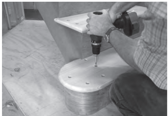
Figure 8.130 Glue and screw through the pre-drilled baluster dowel holes into the solid block below. The locations of these holes were marked using a volute template - see chapter 11.
