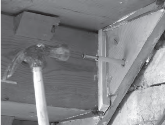
Figure 12.10 Tap the frame fixing until the sleeve is just within the string's countersunk hole.
