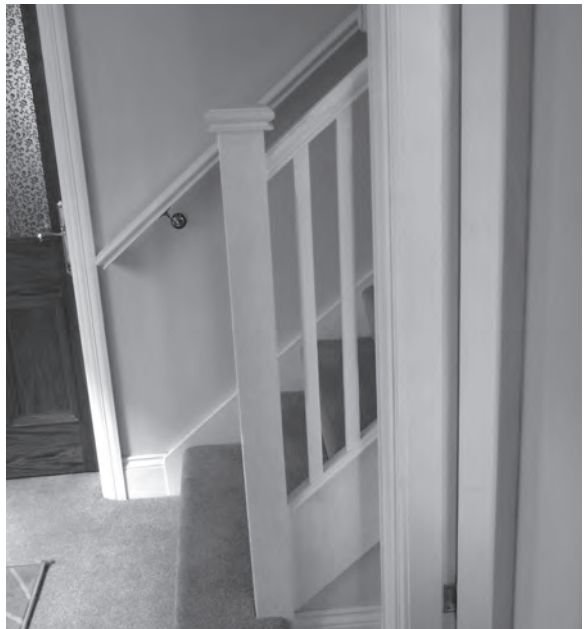
Figure 12.94 The two handrails, level and parallel.
