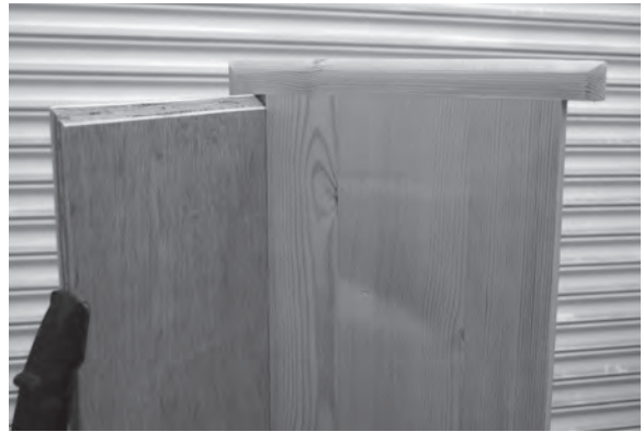
Figure 7.17 F-clamps hold the steps perpendicular to the wall string.
