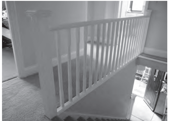
Figure 12.64 The balcony railing now painted and carpets laid.
