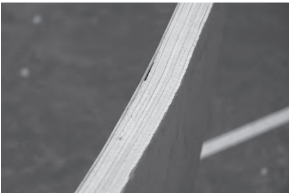
Figure 8.23 Once the wall string has been fully laminated, the slight bulge caused by the lengthening joint will be unnoticeable.
