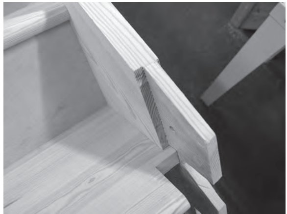
Figure 4.93 Tread number 1, showing the L-shaped cut that will allow it to sit within the housings of the newel post.
