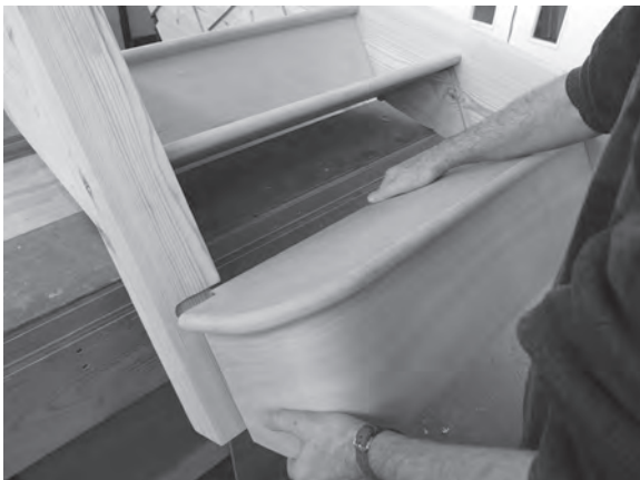
Figure 6.71 Locate the bullnose step firstly in the housing of the inner return string and then into that of the bottom newel post.
