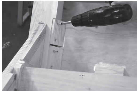
Figure 6.73 Glue and screw angled blocks to the bottom newel post provide support for riser number 2 and the bullnose step.
