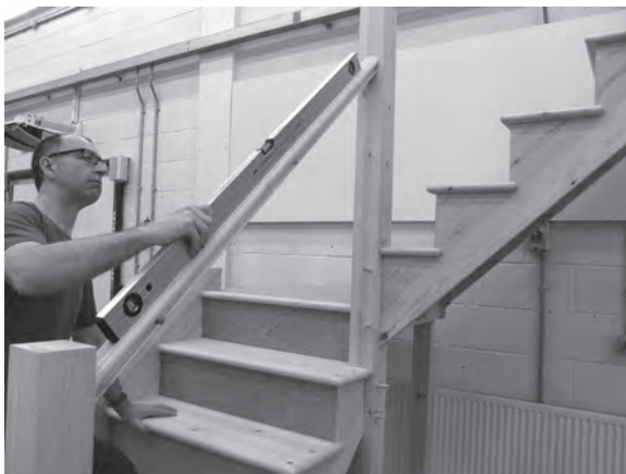
Figure 11.42 Use a long spirit level to check the straightness of the handrail.
