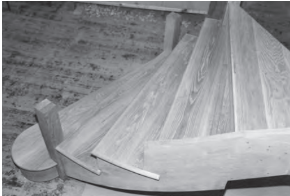
Figure 10.62 (above) and Figure 10.63 (below) The circular section of the newly built Ascot staircase – still in the workshop – with its open-to-closed right-hand string.
