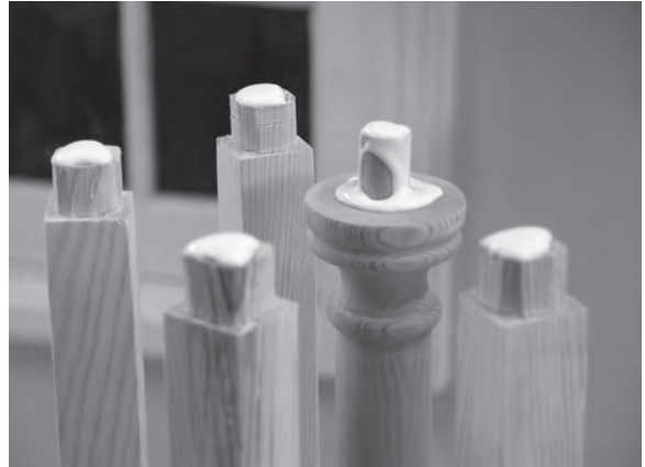
Figure 11.120 Glue is applied to the tops of the volute newel and all balusters ahead of handrail installation.
