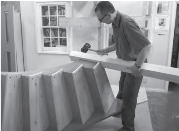
Figure 8.132 With the staircase on its side, the newel post can be fitted to the open string.
