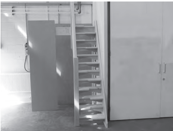
Figure 9.71 The erected staircase. Note the full top riser hiding the landing joist.
