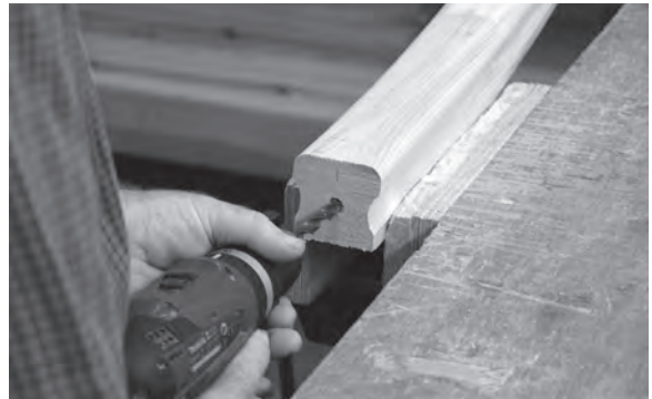
Figure 11.83 A 9 mm hole in the handrail will receive the engineering-thread-half of the double-threaded rail bolt. When drilling for the rail bolts, it is essential that the drill is held at 90° to the surface.
