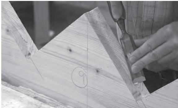
Figure 5.22 Finish the mitres with a sharp chisel.
