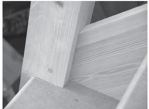
Figure 6.69 The outer string's shoulder has been pulled nicely up to the bottom newel post.
