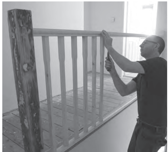
Figure 12.60 The new balusters are housed, glued, and skew-nailed top and bottom.
