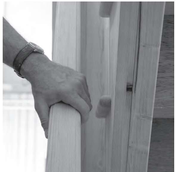
Figure 7.29 (above) Adequate finger room ensures comfortable use of the handrail.
