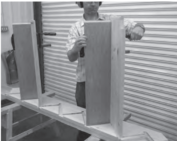
Figure 7.16 Two end steps are located within their wall-string housings and loose wedged.
