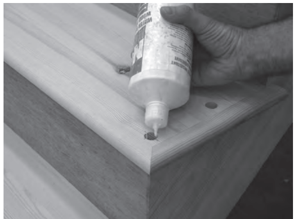
Figure 11.44 Glue is trickled in and around the tread's dowel hole ready to receive the baluster.
