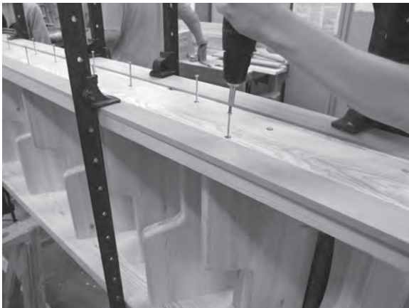
Figure 9.60 'Dovetail' the screws for a better hold of the treads' end grain.
