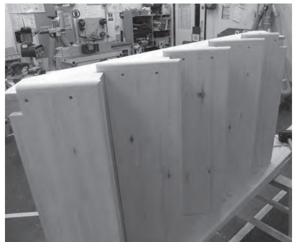
Figure 5.61 The treads are fixed. Note the notching (for newel posts) at the back of the closest tread on the left and at the front of the farthest tread on the right.
