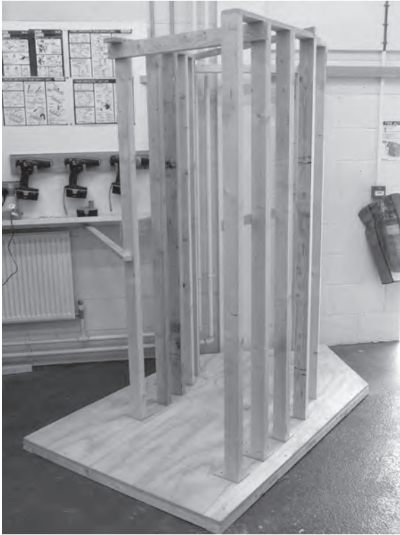
Figure 8.17 The studs must be perfectly plumb and stiffened with the use of bracing.
