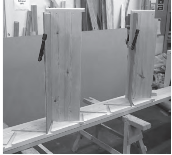
Figure 5.52 Only two steps are required at this stage; further treads and risers will be added once the outer string has been positioned.
