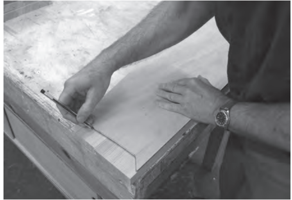
Figure 8.80 (above) and Figure 8.81 (below) Realign the template and use both parts in turn to mark the nosing returns.
