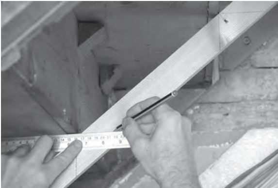
Figure 12.21 Using a steel rule, the tread and riser lines are extended onto the carriage.
