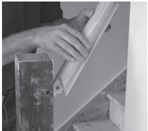
Figure 12.35 The handrail's tenon, with its offset draw-pin hole, is coated with PVA adhesive and inserted into the mortise.
