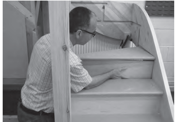
Figure 6.97 Riser number 4 is installed.
