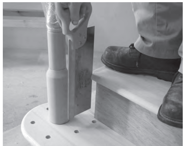
Figure 11.102 Tread number 2 is notched to allow the curtail step's final baluster to be screwed through the face of the second riser and into the cut string behind.
