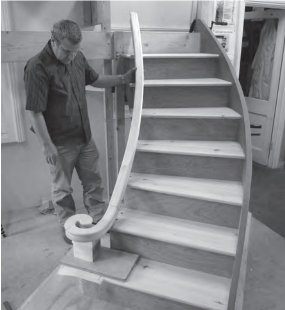
Figure 11.85 With the components dry-fixed together, Steve levels the volute and checks the handrail for correct alignment before gluing.
