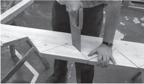
Figure 5.15 Avoid weakening the string by finishing the cuts with a hand saw.
