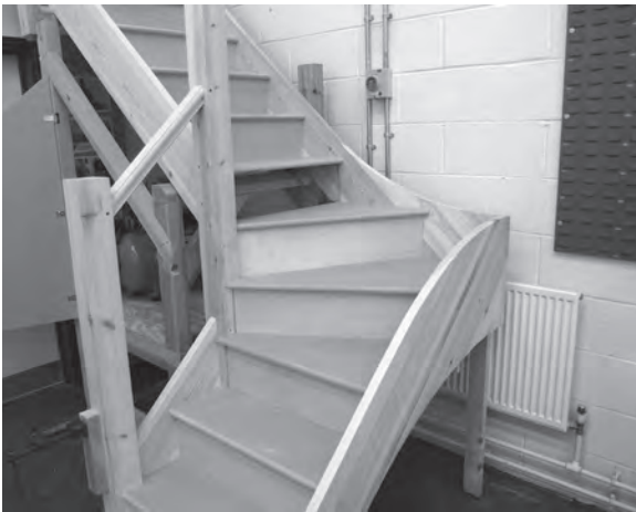
Figure 6.100 With the skew winder and riser number 6 now fixed our last remaining gap is for the first straight riser of the main flight, riser number 7.
