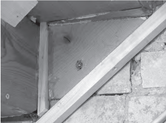
Figure 12.25 (above) and Figure 12.26 (below) Timber battens fixed to the strings level the underside of the flight and provide clearance for the electric cables.
