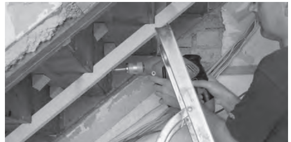
Figure 12.23 The carriage is screwed to the underside of the steps.
