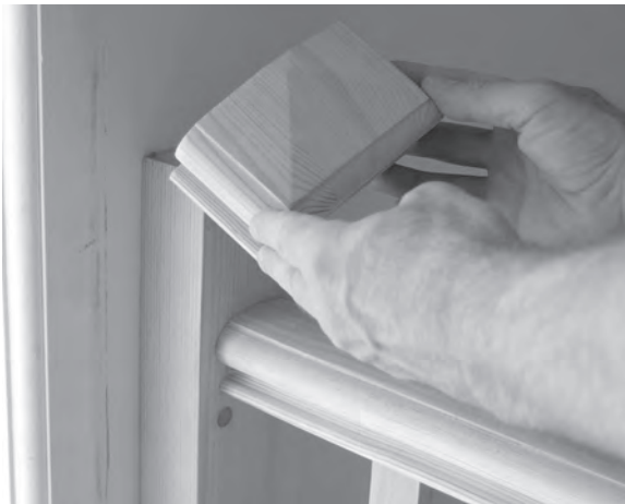
Figure 12.62 One and a half newel caps provide finishing touches to the new installation.
