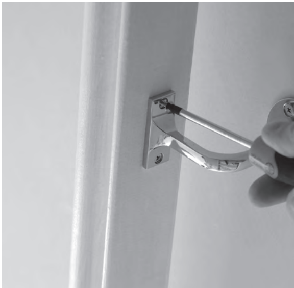
Figure 12.92 Screw up through the brackets into the underside of the handrail. Note: there is no ploughed groove on the underside of wall-mounted handrail.
