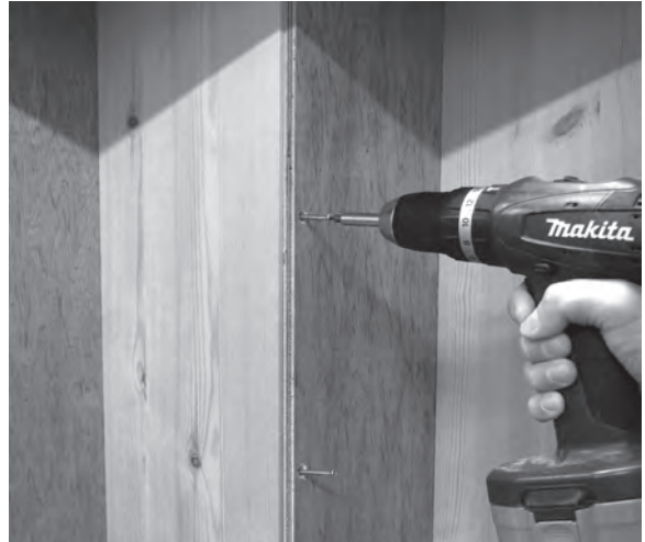
Figure 5.64 Screw risers to backs of treads.
