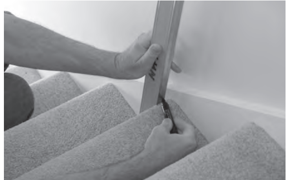
Figure 12.67 The pitch line is marked on the edge of a plumbed spirit level held against a tread nosing.
