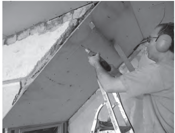
Figure 12.28 The flight's underside is lined with 12.5mm plasterboard secured with drywall screws.
