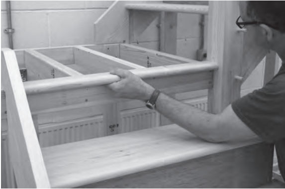
Figure 5.83 Insert the landing nosing within its housings.
