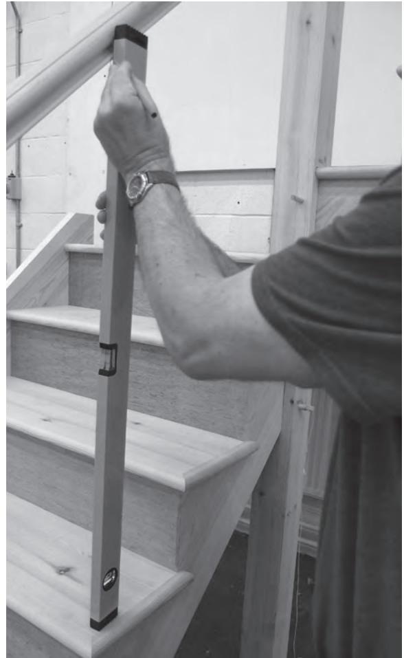
Figure 11.37 Plumbing up from the marked treads is necessary when dowelling balusters into the underside of the handrail.
