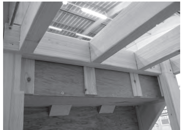
Figure 5.86 Beneath the landing, access is available to screw the top riser to the preceding tread.
