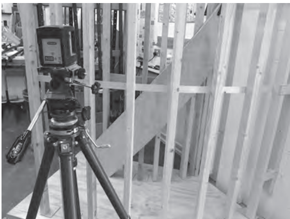
Figure 8.52 (above) and Figure 8.53 (top right) A laser level allows the accurate transfer of riser lines from the rod to the open string.
