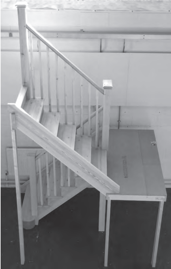
Figure 11.48 The completed dogleg staircase and balustrade.
