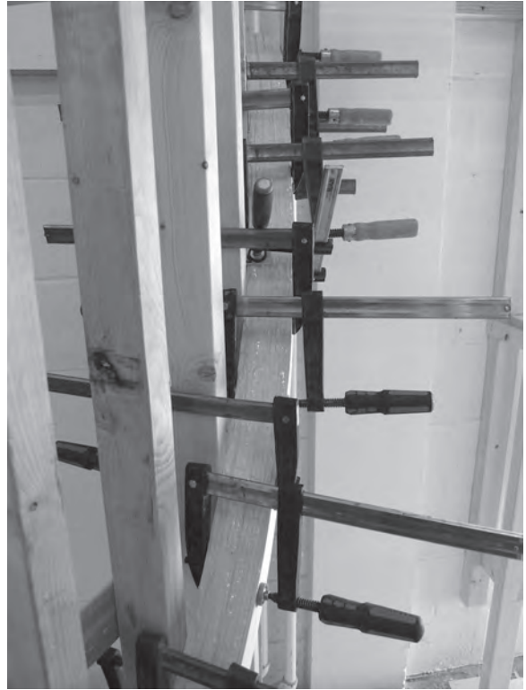
Figure 11.54 The circular handrail's upper surface must be kept square to the vertical studs of the bending form.
