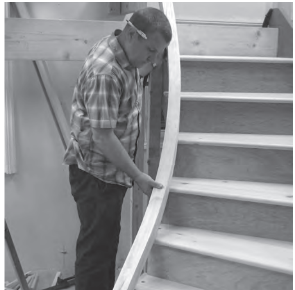
Figure 11.64 Regular checks are essential. Here Steve checks that the curve of the handrail matches that of the staircase.
