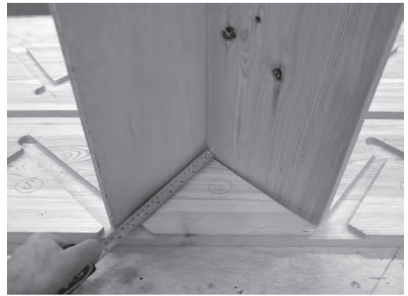
Figure 4.69 With a single step inserted into a string housing, the required length of wedges can be measured.
