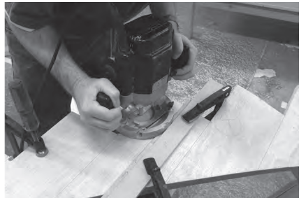
Figure 8.68 The first stage in mitring the string is to use a router to 'let in' the risers.
