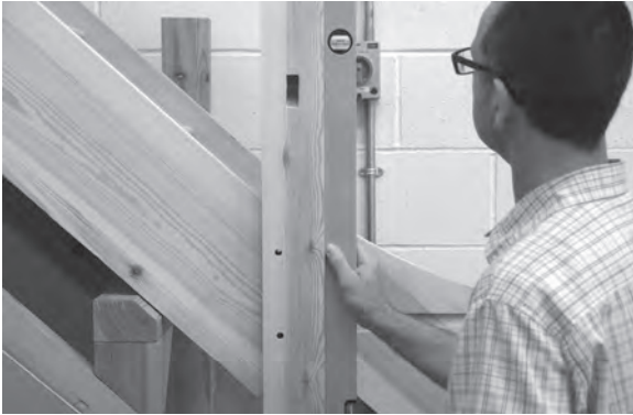
Figure 6.94 Check the intermediate newel post for plumb.
