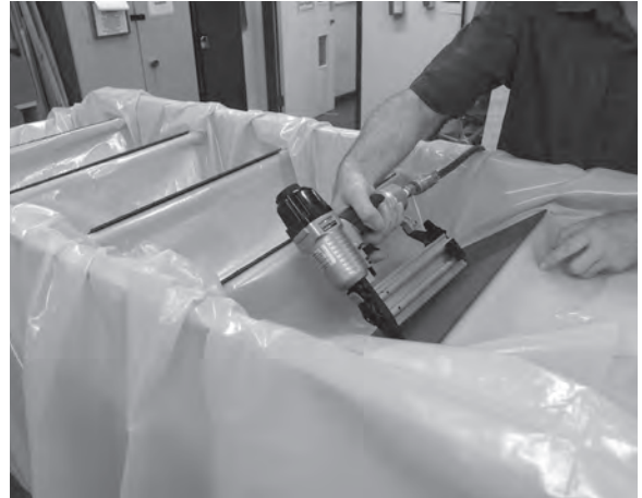
Figure 4.96 The polythene is held down, and the treads protected, by hardboard false treads pinned to the stair treads.
