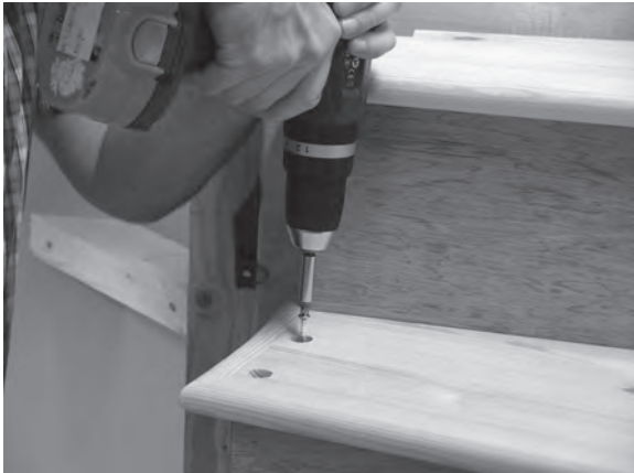
Figure 8.117 (above) and Figure 8.118 (below) At the open end, screw down through the tread's baluster dowel holes into the string below.
