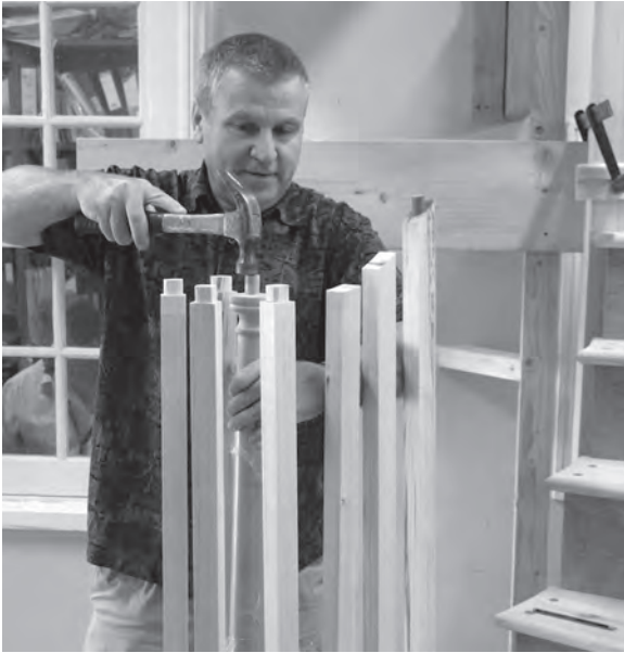
Figure 11.110 With the handrail lifted clear, the balusters that will follow the curve of the volute are inserted into the holes drilled in the curtail step.
