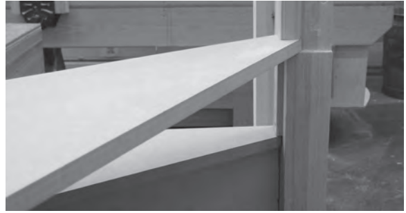
Figure 6.82 The narrow end of the kite winder meeting with the intermediate newel post.
