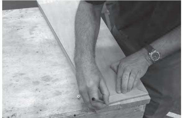
Figure 8.80 (above) and Figure 8.81 (below) Realign the template and use both parts in turn to mark the nosing returns.
