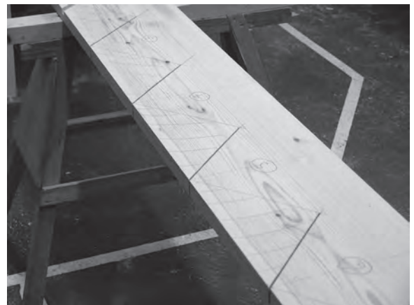
Figure 5.14 With the riser lines cut it's now time to start the tread lines.
