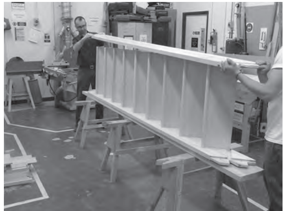
Figure 4.83 The opposite string is lifted into position.
