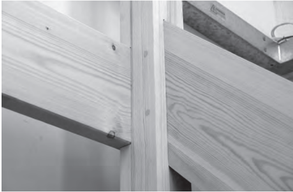
Figure 6.89 The top newel post is hooked securely over the landing joist.
