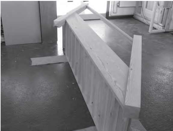
Figure 9.70 The staircase is ready for fixing.
