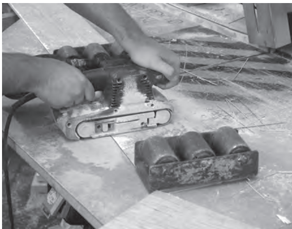
Figure 10.13 The plywood riser's inner surface is belt sanded, making it thin enough and flexible enough to bend around the semicircular block.
