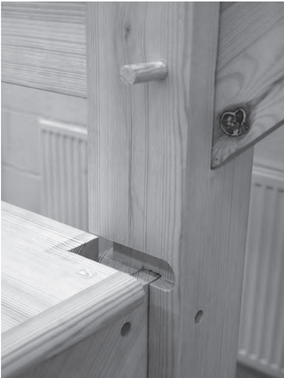
Figure 5.80 The lower flight's cut string meeting with the intermediate newel post.
