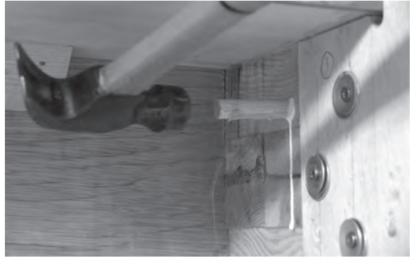
Figure 11.123 Secure the volute newel by gluing and dowelling through the curtail step's solid block into the newel post's spigot.
