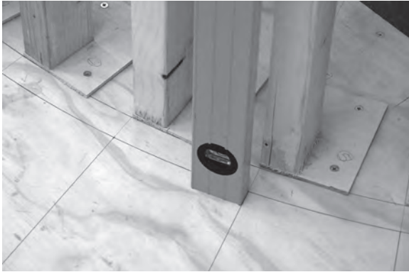
Figure 8.50 (above) and Figure 8.51 (below) Riser lines are transferred from the rod to the open string by plumbing up using a spirit level.
