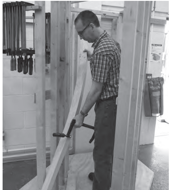
Figure 11.56 After 48 hours, the handrail can be removed from the clamps and bending form.
