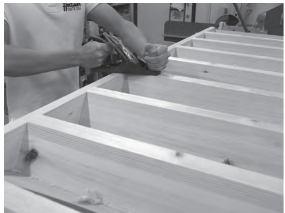
Figure 9.63 Plane and sand the angled backs of the treads flush with the underside of the strings.
