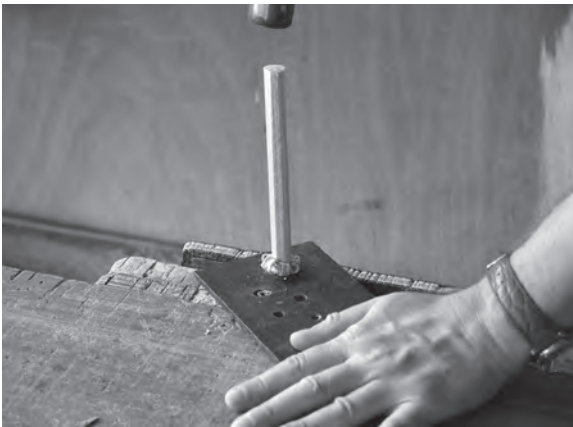
Figure 4.67 Plane the sharp corners off and hammer the short timber pieces through the hole in the metal plate.
