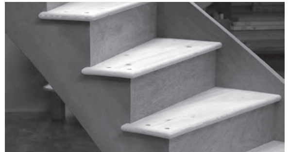
Figure 8.124 The open side of the staircase – also gap-free.
