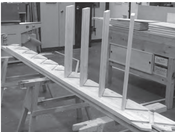
Figure 4.81 (above) and Figure 4.82 (top right) The treads and risers are inserted dry into their housings.
