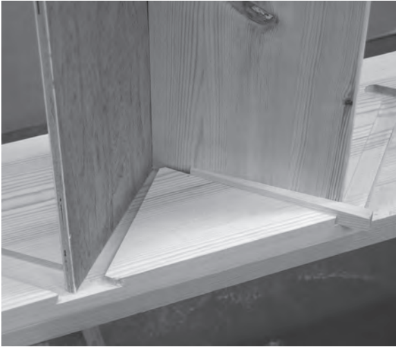
Figure 5.50 Loosely and temporarily wedge the steps to hold them in place.
