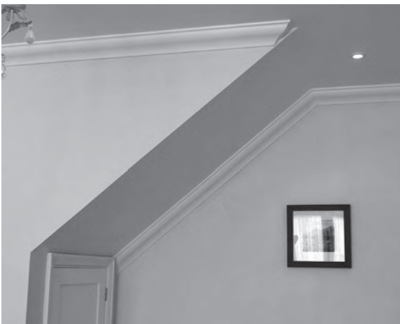
Figure 12.30 The newly decorated room beneath the now creak-free staircase.
