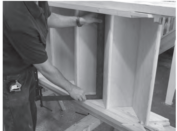
Figure 4.86 A steel roofing square can also be used to check that the treads and risers are square to the strings.
