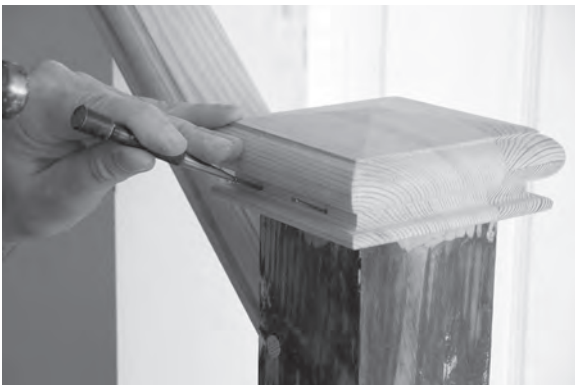
Figure 12.38 A new newel cap is glued and nailed to the top of the newel post.
