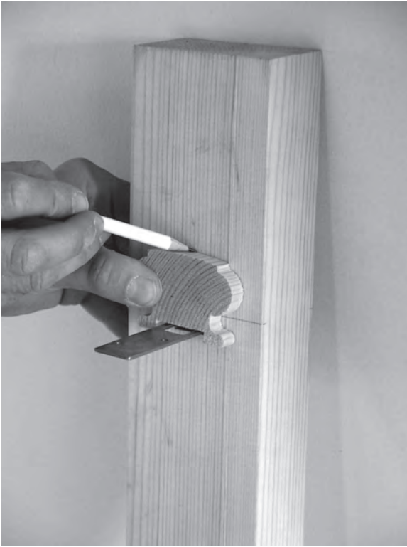
Figure 12.53 Rest an offcut of the new handrail on the bracket and mark its top on the half newel. The top-of-handrail height should also be marked on the upper newel post.
