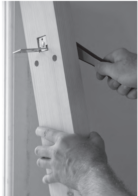
Figure 12.51 (above) and Figure 12.52 (below) The threaded portion of the Richard Burbidge handrail bracket is passed through the half newel and secured from behind with a nut and washer.
