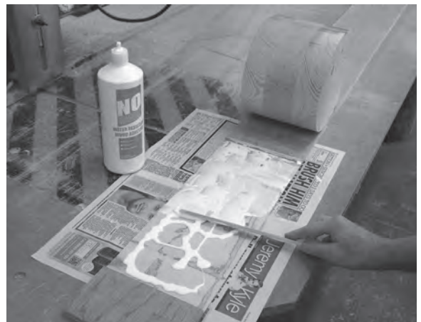
Figure 10.14 PVA adhesive is applied to the carefully positioned plywood riser and block.
