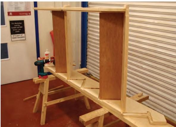
Left: These two steps are the first and last to be carried by the cut and mitred outer string (seen top). Laying face up on the trestles is the closed inner wall string to which the treads have been temporarily dry-wedged while being glued and screwed to the open string. See page 112.
