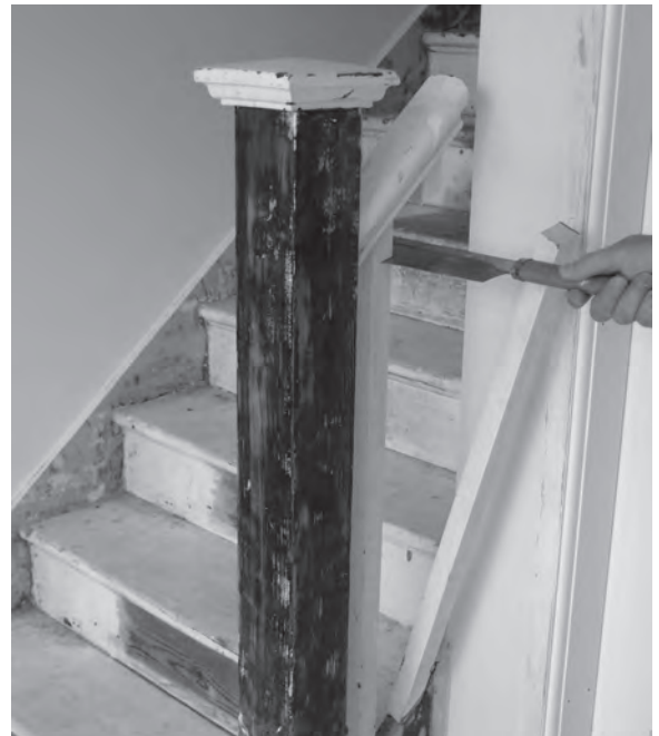
Figure 12.31 Broken or damaged balusters are removed by sawing through at an inclined angle and then pulling the two parts from their fixings.
