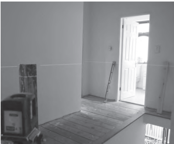
Figure 12.54 The handrail height marked on the upper newel post is transferred to the facing wall with a laser level.
