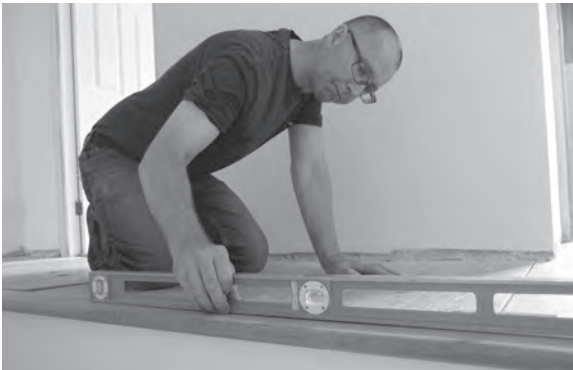
Figure 12.46 (above) and Figure 12.47 (below) The floor and upper newel post are checked for level and plumb.
