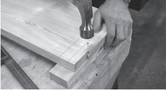
Figure 5.30 The marked treads and over-width nosing returns are nailed together.
