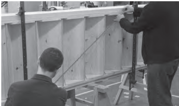
Figure 4.85 With the help of a second person, check the staircase for square by measuring a pair of diagonals.
