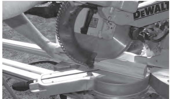
Figure 12.84 Use a chop saw to mitre the ends of the handrail. The offcut from one end will become the mitred return for the other.
