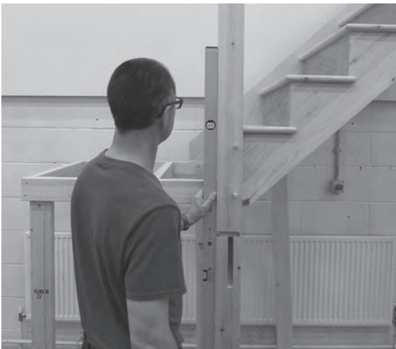
Figure 5.76 When fully up, the intermediate newel post should be checked for plumb.
