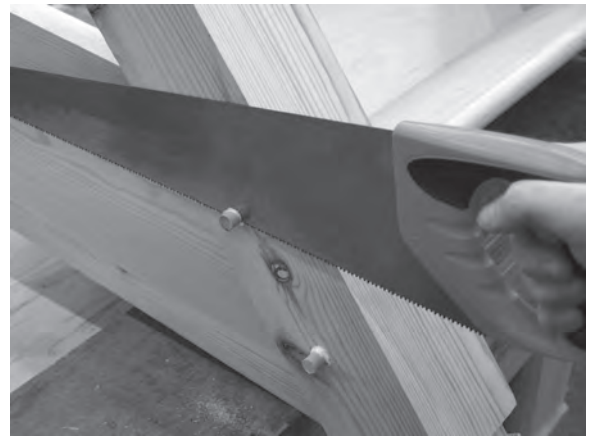
Figure 6.68 Cut the dowel flush with the newel post.
