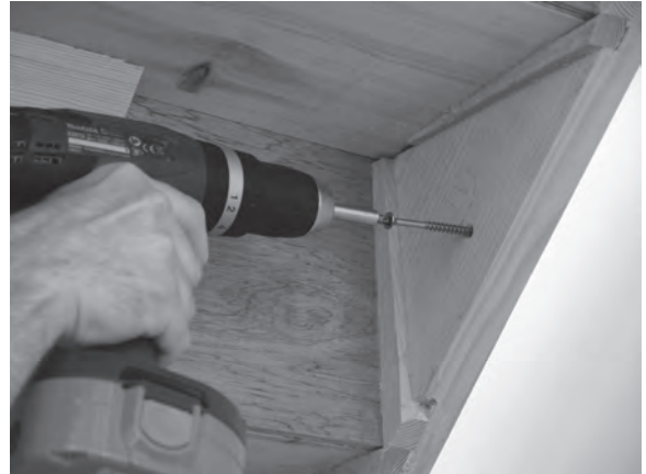
Figure 5.77 Fix the flight to the wall by screwing through the wall string.
