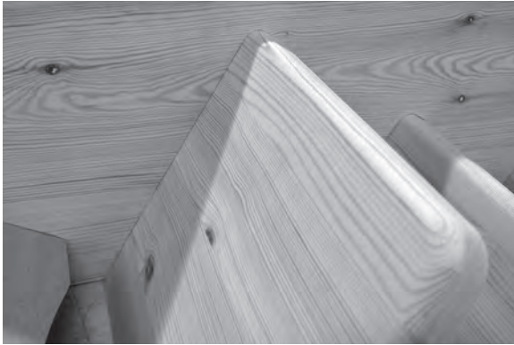
Figure 9.59 Before screwing, check that the tread nosings are fully up in their housings.
