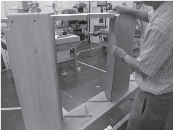
Figure 5.59 Locate the remaining risers in their wall-string housings and glue and nail to the cut string.
