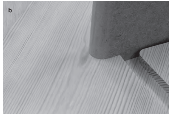
Figure 3.43a & b The tread nosing fits nicely, and the corner beneath the nosing is now square.
