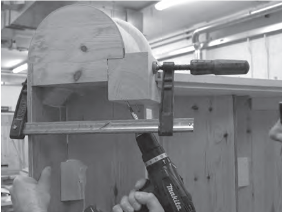
Figure 5.71 The D-step, viewed from the underside, meets with the bottom newel post which is glued and screwed to the step's solid block.
