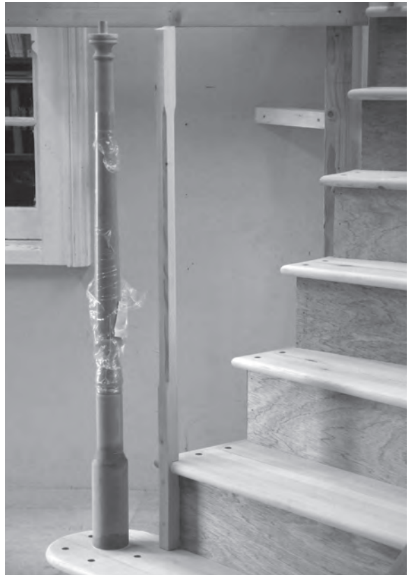
Figure 11.117 The first two components are glued in place while polythene protects the volute newel during installation.
