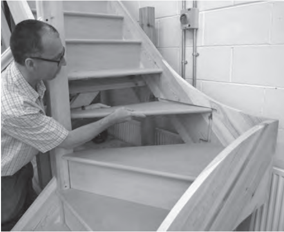
Figure 6.99 With the kite winder and riser number 5 fixed in place, skew winder (number 6) is inserted into its housings.
