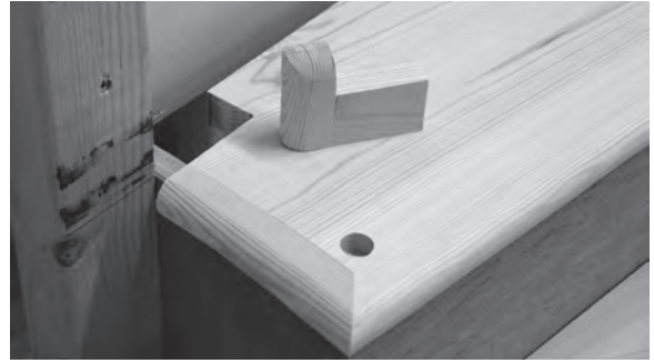
Figure 8.115 The notched rear of tread number 7, below which the open string's tenon is just visible.
