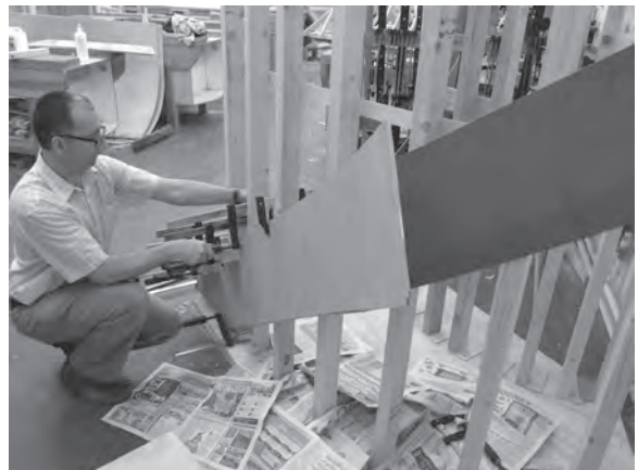
Figure 8.36 Lay down newspaper to catch the glue drips as the flexi ply is clamped in place.
