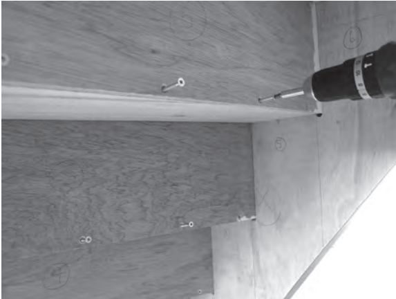
Figure 8.121 Fix each riser to its preceding tread.
