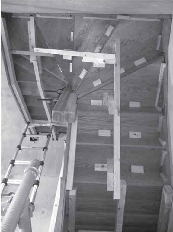
Figure 10.55 This view of the flight's underside shows a centre carriage supporting the steps. (Photo courtesy of Frank Turtle)
