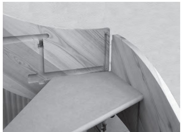
Figure 6.98 The wall and return strings are temporarily separated, providing access for locating kite winder number 5 and its return-string wedge.
