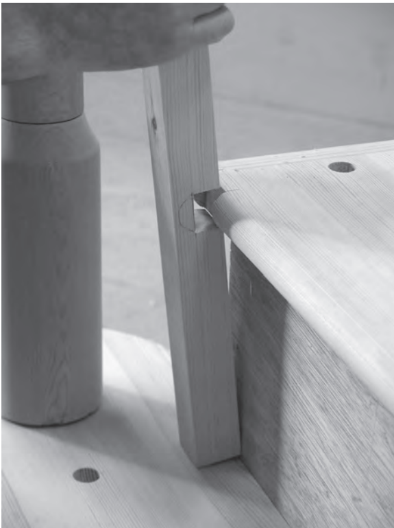
Figure 11.104 The housed baluster is tested for fit.
