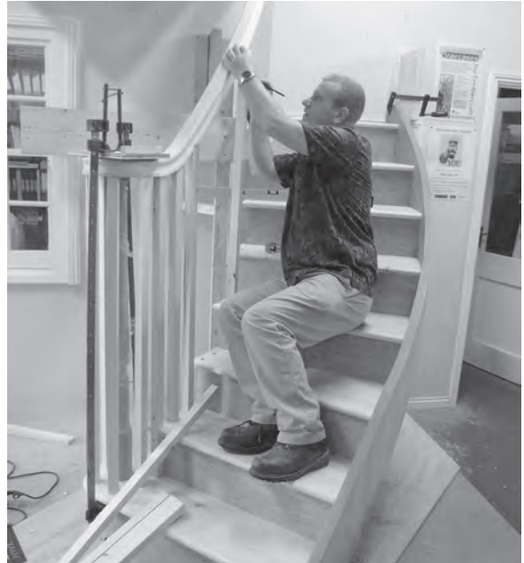
Figure 11.112 The handrail is repositioned, and each baluster is individually marked and cut.
