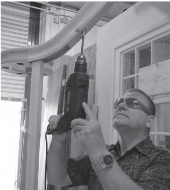
Figure 11.107 An 18mm diameter hole is drilled to a depth of around 38mm, allowing dowel penetration of at least 25mm.
