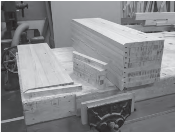
Figure 5.40 The treads and nosing returns are ready for fixing.
