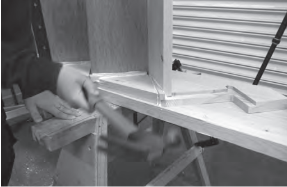
Figure 7.23 Glue and wedge the treads and risers to the wall string.
