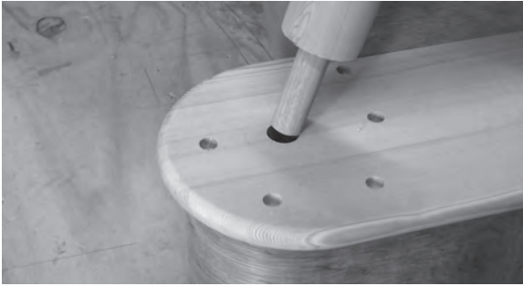
Figure 11.99 The volute newel's spigot should be a minimum of 100 mm long.
