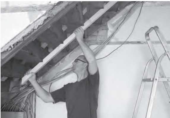
Figure 12.22 The notched carriage is offered into position in the centre of the flight.
