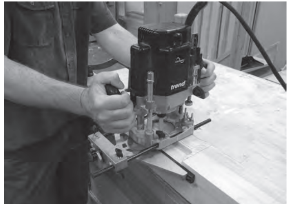
Figure 5.25 Use the router's fence attachment when cutting parallel to the newel posts' long edges.
