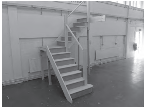
Figure 5.88 The finished staircase.
