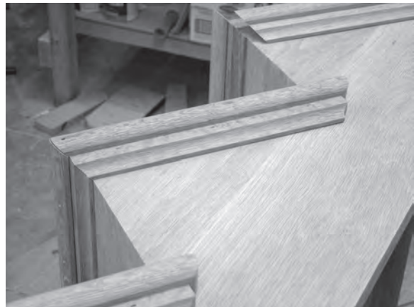
Figure 10.54 The combined nosing/scotia mitred return (a single item) intersects nicely with separate items, the tread and scotia moulding.
