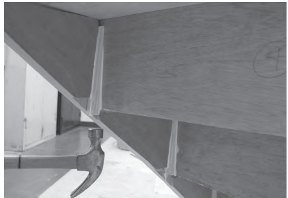
Figure 8.120 Glue and wedge the steps.
