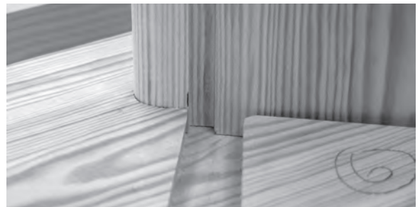
Figure 4.53 The housing is checked against the string for correct alignment.
