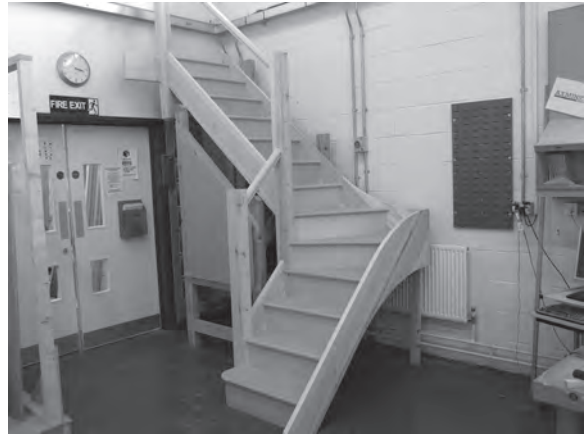
Figure 6.101 All three winding steps are now complete, and so with the exception of balusters and newel caps, the staircase is complete.
