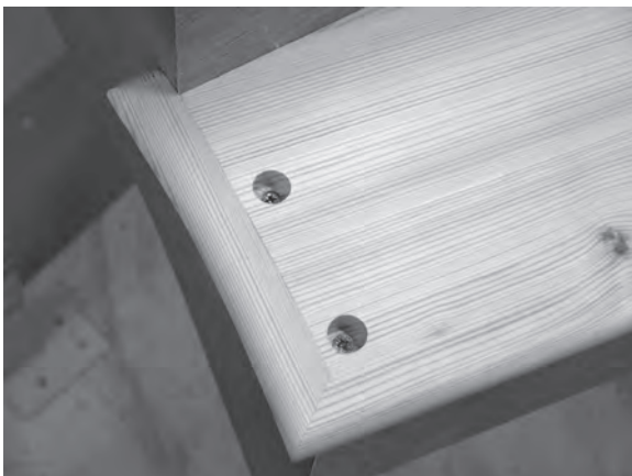
Figure 8.117 (above) and Figure 8.118 (below) At the open end, screw down through the tread's baluster dowel holes into the string below.
