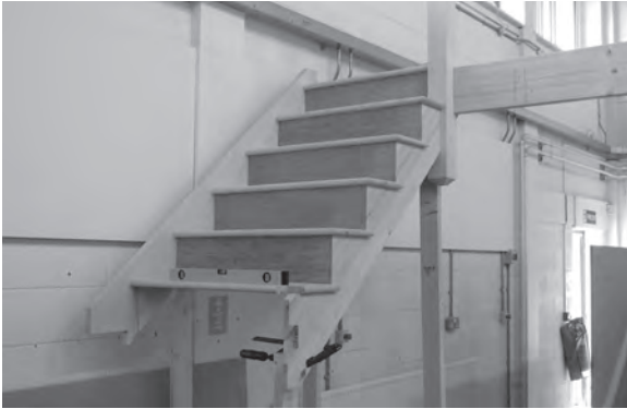
Figure 5.74 The upper flight supported, at the top, by the landing joist and, at its lower end, by temporary props.
