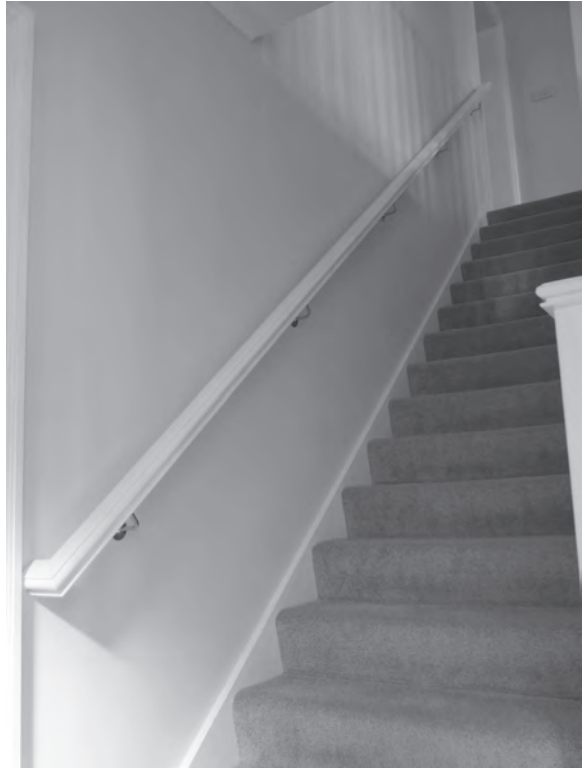
Figure 12.93 The newly installed wall-mounted handrail.
