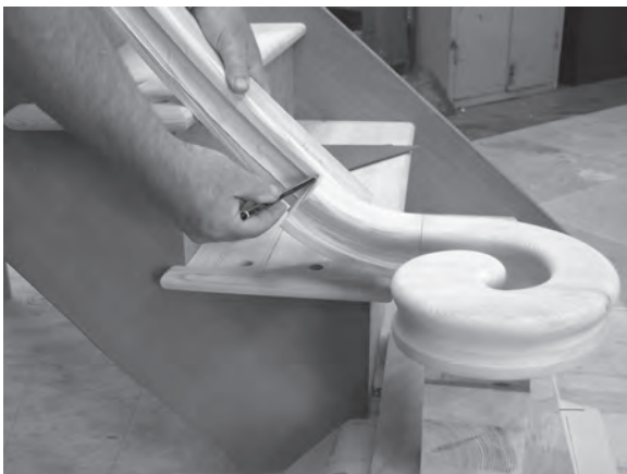
Figure 11.81 The handrail is marked for cutting by scribing a line against the trimmed end face of the upward easing.
