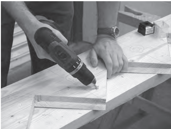
Figure 7.15 Pocket-screwing from beneath the treads means that all fixings are hidden.
