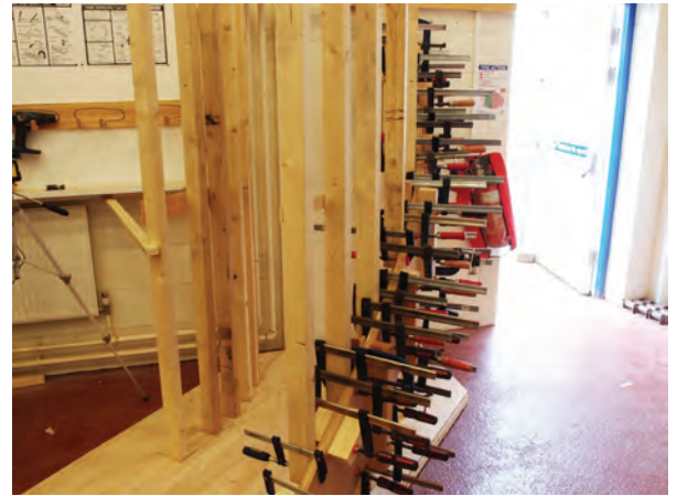
Laminating a circular stair string round a bending form requires the availability of a clamp or two. The glued-up string must stay in clamps for 48 hours in order to retain its shape. See page 129.
