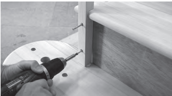
Figure 11.115 The notched baluster is glued and screwed through the face of the second riser into the cut string behind.
