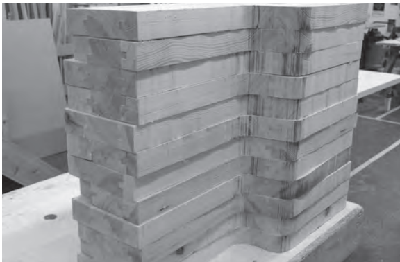
Figure 9.31 The six panels are now twelve alternating treads, ready to be planed to their finished thickness of 40 mm.
