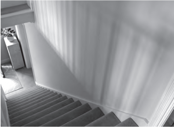
Figure 12.65 A new continuous handrail will be fixed to this wall.
