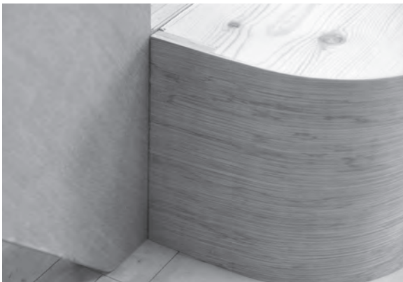
Figure 8.127 The rear of the curtail riser needs trimming carefully if it is to fit nicely against the open string.
