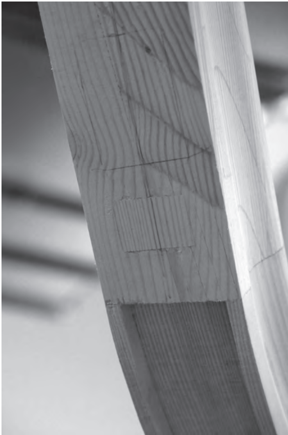
Figure 11.89 The rail bolt access hole is patched.
