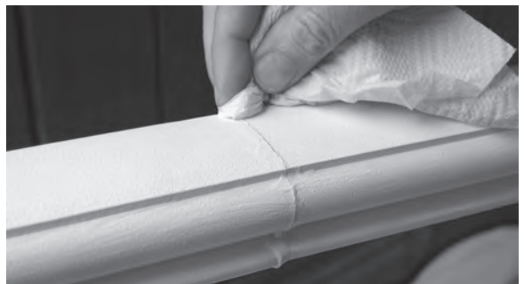
Figure 12.90 Wipe excess glue from the tightened joint.
