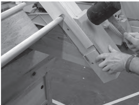
Figure 5.68 The bottom newel post, protected by a scrap piece of timber, is tapped into place.
