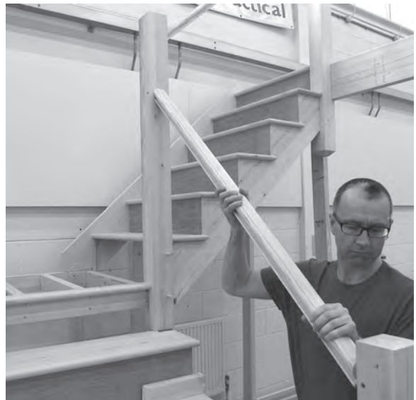
Figure 5.82 Install the handrails before pulling joints up tightly.
