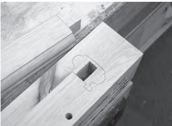
Figure 11.19 (above) and Figure 11.20 (below) Offer the horizontal handrail into the newel post's mortise and draw tightly around its profile with a sharp pencil, before removing and setting aside.
