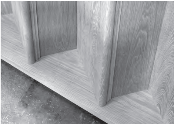
Figure 10.50 (above) and Figure 10.51 (below) Tread and riser housings routed into the wall strings include an allowance for the scotia mouldings.
