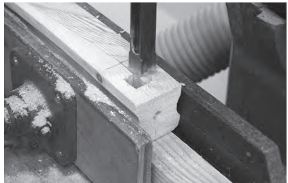
Figure 11.84 An access hole in the underside of the handrail can either be drilled or, as seen here, mortised.
