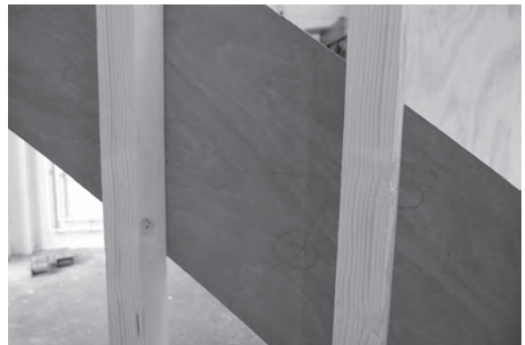
Figure 8.32 Accurately aligned riser and tread lines indicate that the facing plywood is correctly positioned.
