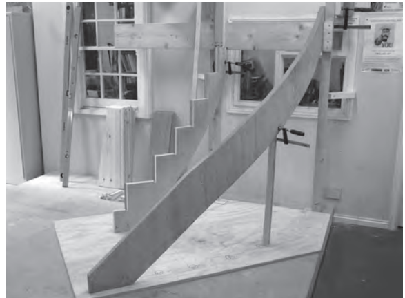
Figure 8.110 Both strings are correctly positioned and secured in place.
