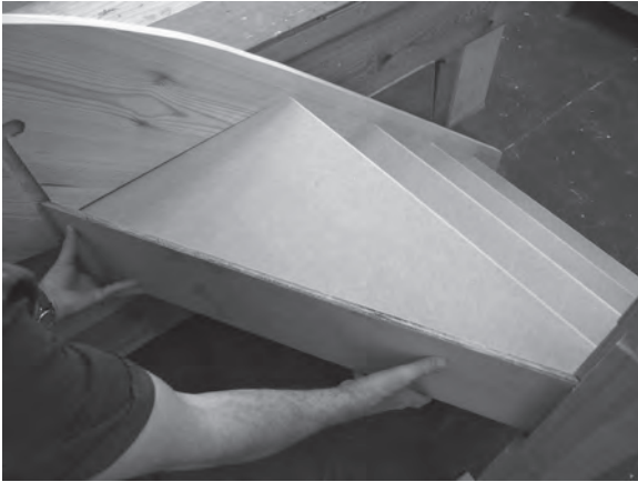
Figure 6.79 (above) and Figure 6.80 (below) Riser number 5 being lifted into its housings and held in place with a wedge. For clarity, the kite winder has been omitted.
