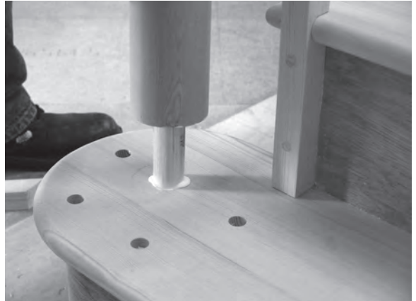
Figure 11.116 The baluster screw holes are pelleted and the volute newel's spigot glued and inserted into the curtail step.
