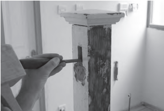
Figure 12.33 All remaining waste is removed with a wood chisel.
