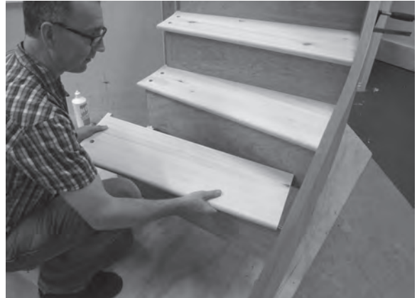
Figure 8.119 Avoid damaging the treads' nosings and the wall string by carefully 'angling' the treads into their housings.
