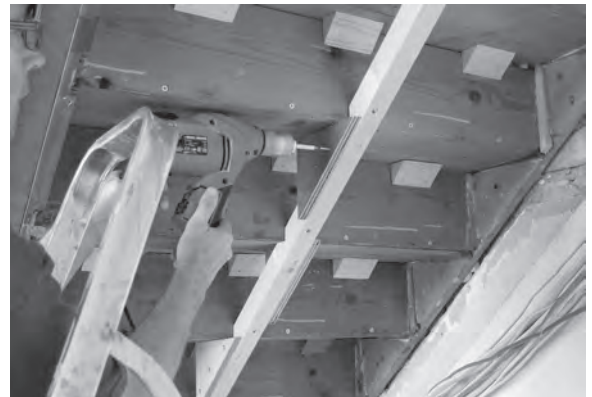
Figure 12.24 The tread centres are supported by triangular plywood cleats screwed to the carriage.
