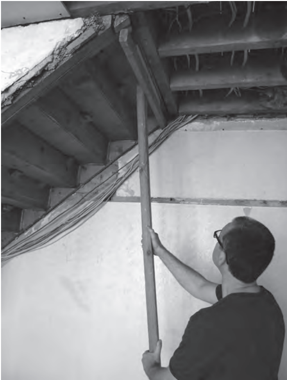
Figure 12.14 A prop is used to push up a sagging tread ready for fixing.
