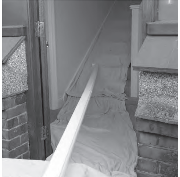
Figure 12.88 Make sure that access to the handrail's final location is possible before gluing and screwing the two halves together.
