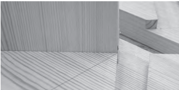
Figure 4.56 Check the fit of the first tread planed against the string before cutting and planing the remaining treads.
