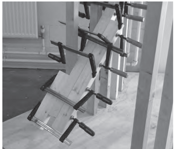
Figure 11.55 Straightness at the foot of the staircase is maintained by clamping straight timber to the laminated handrail.
