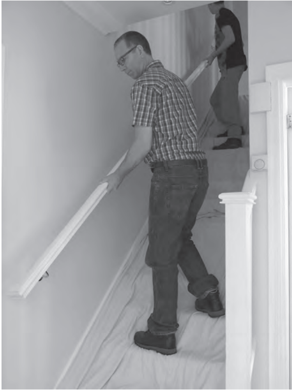
Figure 12.91 The handrail is lifted carefully into place.
