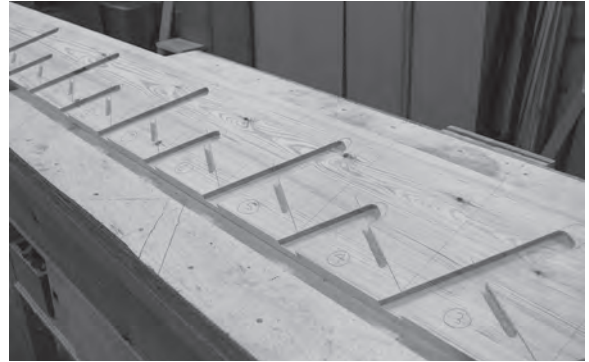
Figure 9.20 The routing of the wall string is complete.
