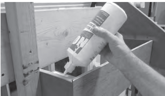
Figure 8.114 Glue the open string's horizontal surface and install the first of the treads, again working from the top down.
