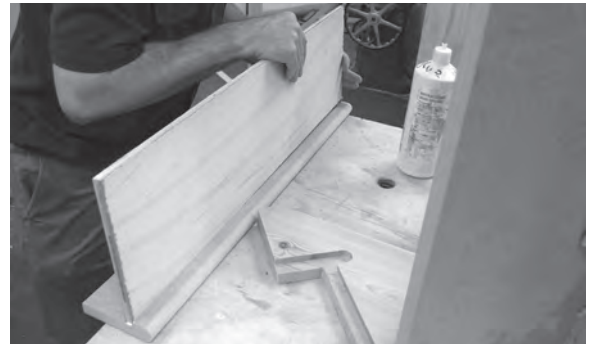
Figure 6.87 The top riser (number 13) is glued to the underside of the landing nosing.
