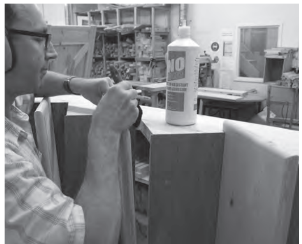
Figure 7.22 Apply glue generously before fixing the treads and risers.
