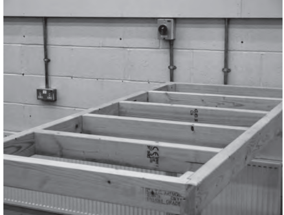
Figure 7.25 The half landing.
