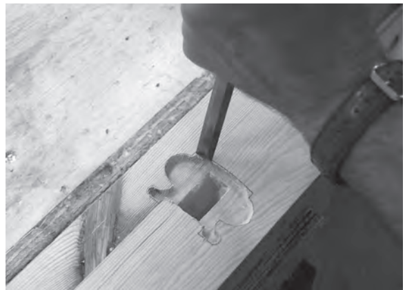
Figure 11.22 Remove all the remaining waste by using a sharp chisel to get into the corners that the router is unable to.
