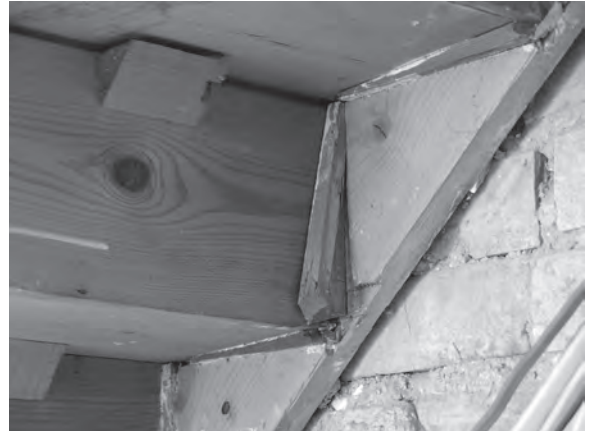
Figure 12.7 (above) and Figure 12.8 (below) Replace all loose and missing wedges if the flight's underside is accessible.
