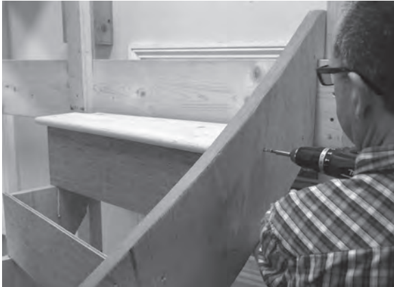
Figure 8.116 Screw through the pre-drilled holes in the wall string into the end grain of the tread.
