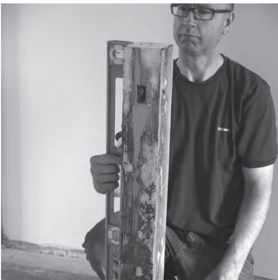
Figure 12.46 (above) and Figure 12.47 (below) The floor and upper newel post are checked for level and plumb.
