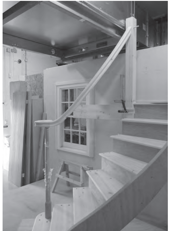
Figure 11.101 With the handrail dry-fixed between the two newel posts the marking and cutting of the balusters can begin.
