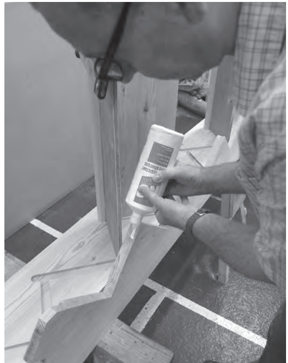
Figure 5.53 Before lifting the outer string into place, spread PVA adhesive onto the string's corresponding steps.
