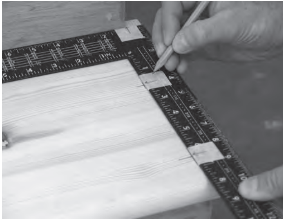
Figure 11.36 Baluster locations can be marked quickly and accurately using a steel roofing square aligned with the balustrade centre line.
