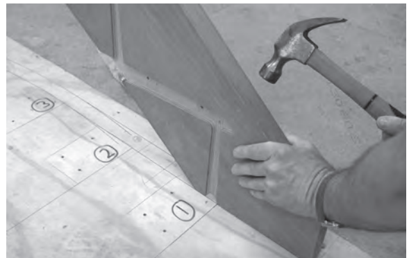
Figure 8.106 and Figure 8.107 Align the bottom end of the string with the rod and secure by skew nailing.
