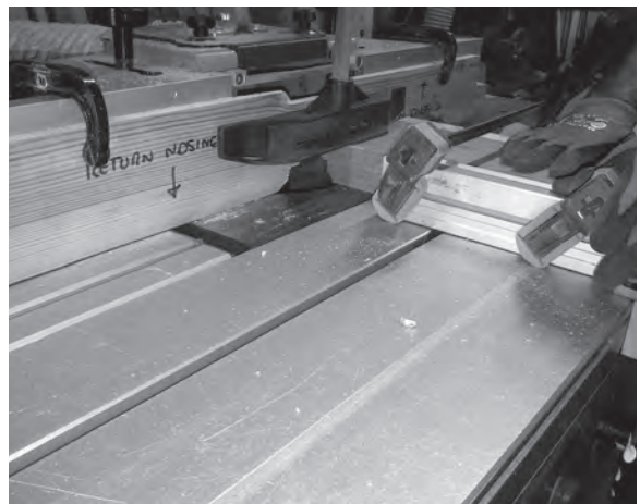
Figure 10.45 (above) and Figure 10.46 (opposite page, top left) The end grain of wide boards are spindle to produce combined nosing and scotia mouldings. (Both photos courtesy of Frank Turtle)
