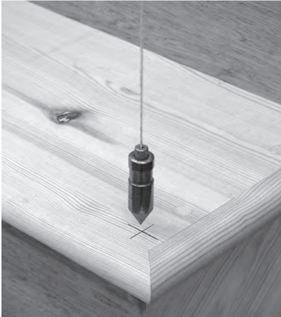
Figure 11.38 Use a plumb bob to check that baluster locations marked on the handrail correspond with those marked on the treads.
