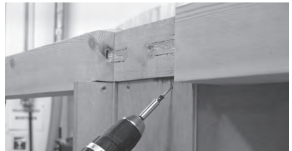
Figure 6.88 The assembled top step is placed into its housings and screwed, on one side, into the wall string and, on the other, into the top newel post. The riser is screwed to the back of tread number 12.
