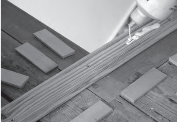
Figure 12.61 Timber fillets are glued and pinned into the grooves in the baserail and handrail between each baluster.
