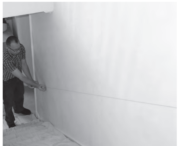
Figure 12.71 A chalk line, parallel with the pitch line, is snapped against the wall.
