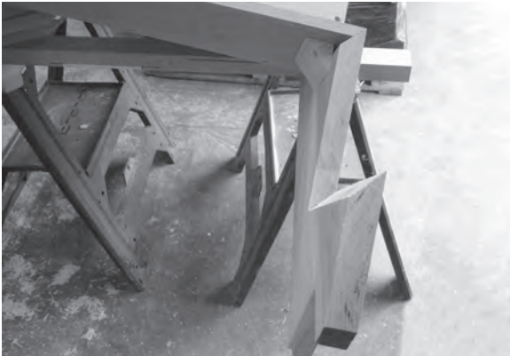
Figure 10.43 Using a chop saw to mitre the strings' riser lines highlights the difference in thickness between the string and the riser, which backs against an angled glue block.
