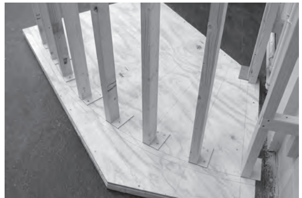
Figure 8.16 With the fixing of the studs, our work, which has so far been two-dimensional on a flat sheet of plywood, is now developing three-dimensionally.
