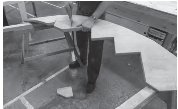
Figure 8.67 Remove the triangular waste pieces with a hand saw so that the string is not weakened.
