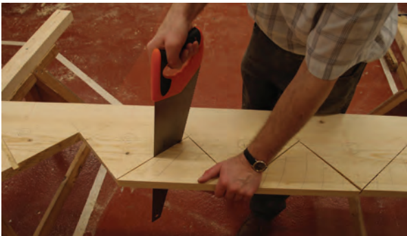
Much of the work in removing the triangular waste pieces from this open string is carried out with a hand-held circular saw. The cuts are stopped short of the intersecting riser and tread lines and finished with a hand saw so that the string is not unnecessarily weakened. See page 60.
