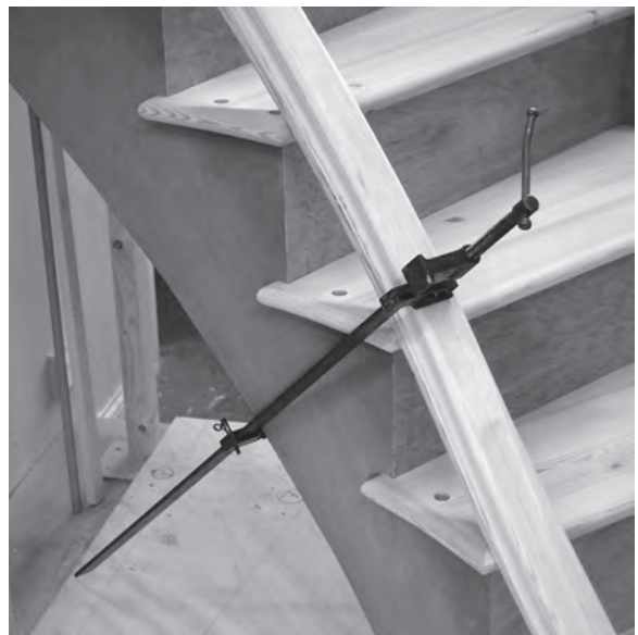
Figure 11.92 The handrail can be laid on the tread nosings and balustrade centre line, and secured with a sash clamp.
