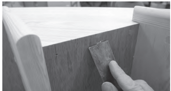
Figure 5.66 Nail holes visible on the riser faces should be filled before cleaning up.
