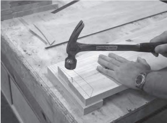
Figure 8.83 Nail through the waste part of the tread into the over-width nosing return below.
