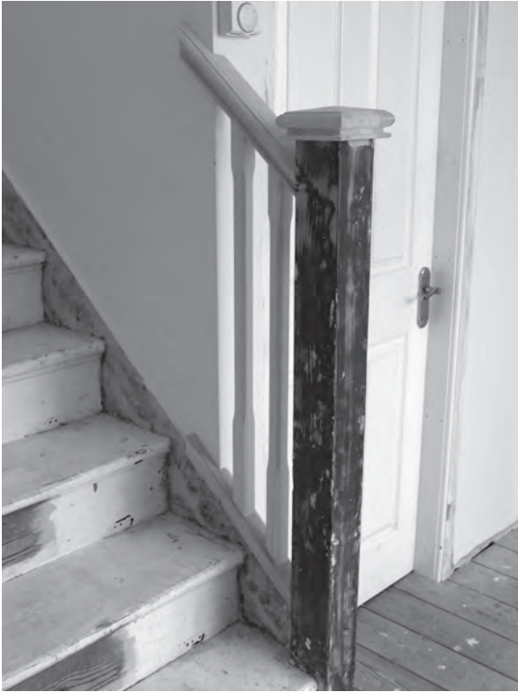
Figure 12.41 The short balustrade run at the foot of the stairs is complete.
