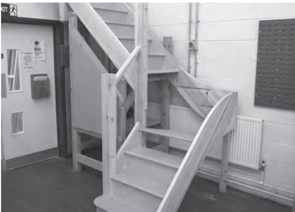
Figure 6.96 The main and return flights are now joined. Only the first of the three tapered treads – the square winder, which must be positioned ahead of the intermediate newel post – is in place at this stage.
