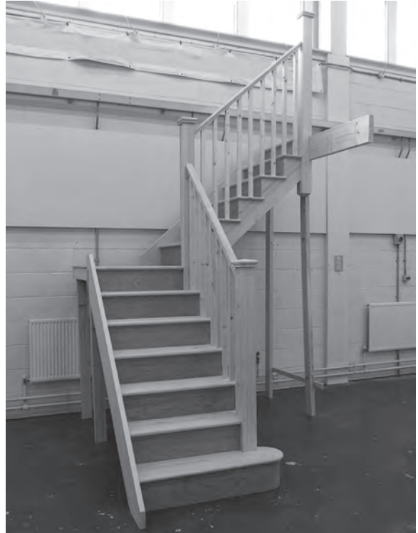
Figure 11.47 The completed quarter-turn staircase and balustrade.
