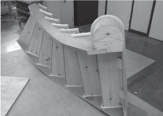
Figure 8.131 Laying on its side, the staircase's twisted appearance is clear to see and we now have access to glue and wedge riser number 1 and tread number 7.
