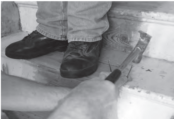
Figure 12.3 Under the weight of a helper, a settled tread can be held in place with nails 'dovetailed' into the riser.
