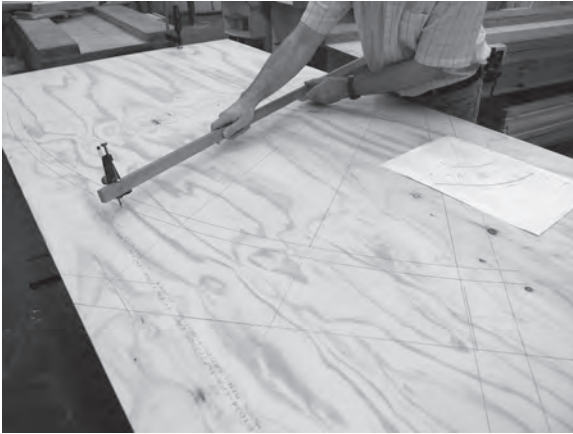
Figure 8.6 Trammel heads clamped to a timber batten are perfect for setting out the circular strings.
