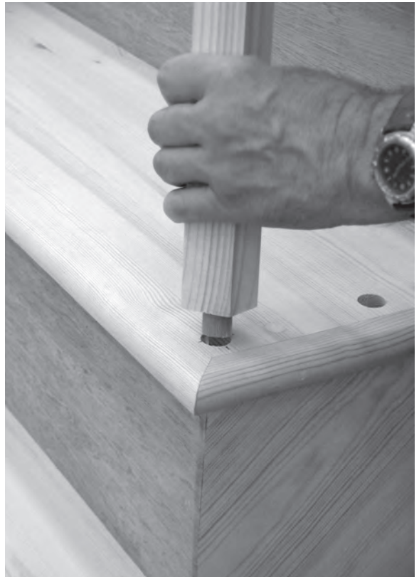
Figure 11.43 The first baluster is located, without glue, in the pre-drilled hole and plumbed; a line is then scribed against the underside of the handrail, to which the depth of the groove must be added.
