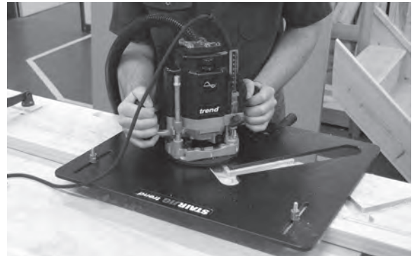
Figure 4.34 Stand facing the string's lower edge and rout each step, working from left to right.
