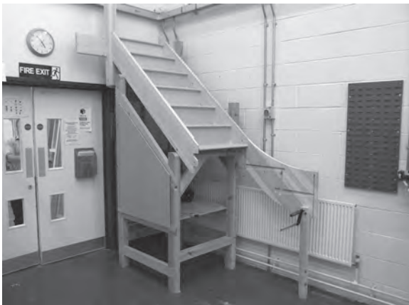
Figure 6.90 The main flight in position and temporarily supported at its lower end with props.
