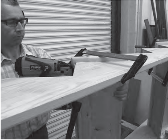
Figure 7.20 The mitred ends of the risers are glued and nailed to the outer string.
