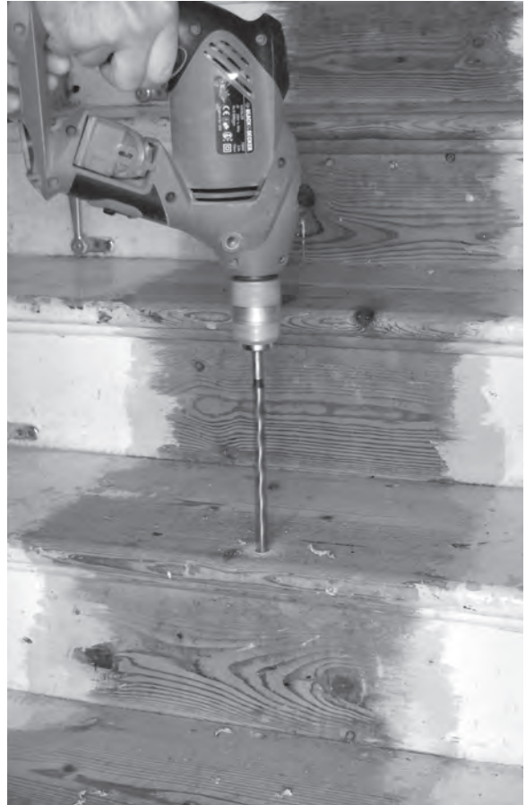
Figure 12.4 Prepare screw holes for pelleting with a 12mm auger bit.
