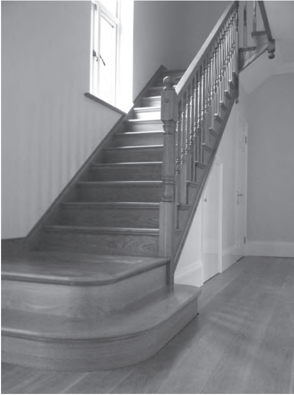
Figure 10.39 This beautiful open-string staircase – one of several flights spanning two stories – was manufactured in American white oak by Totally Bespoke Joinery Limited in Rochester, Kent. (Photo courtesy of Frank Turtle)
