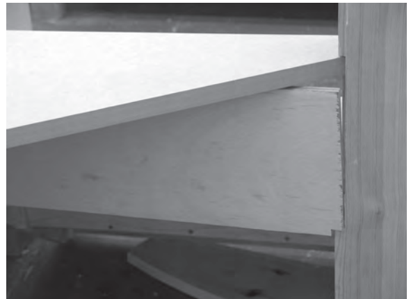
Figure 6.78 With the intermediate newel post replaced, riser number 4 is pushed forward and then upwards into its housing in the underside of the square winder. A small notch cut in the bottom corner of the riser permits access.
