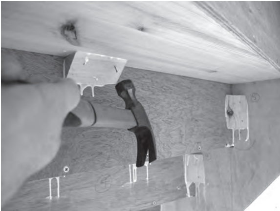
Figure 8.122 Support the steps with glue blocks which require pinning while the glue dries.
