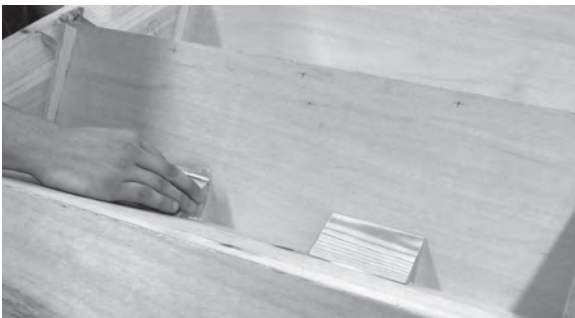
Figure 4.91 Apply glue blocks at equidistant spacings (150 mm minimum) with PVA adhesive using rubbed joints.
