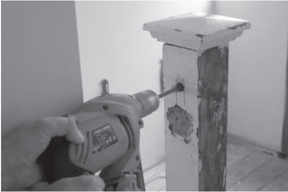
Figure 12.32 Start removing waste from the newel post's new mortise by drilling with an 18mm flat bit.
