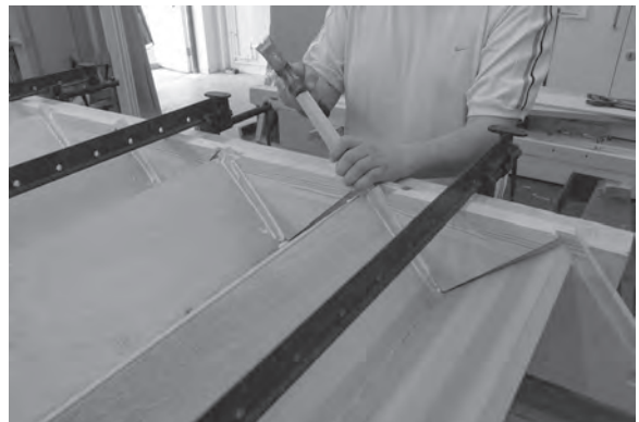
Figure 6.63 The clamped-up staircase is glued and wedged.
