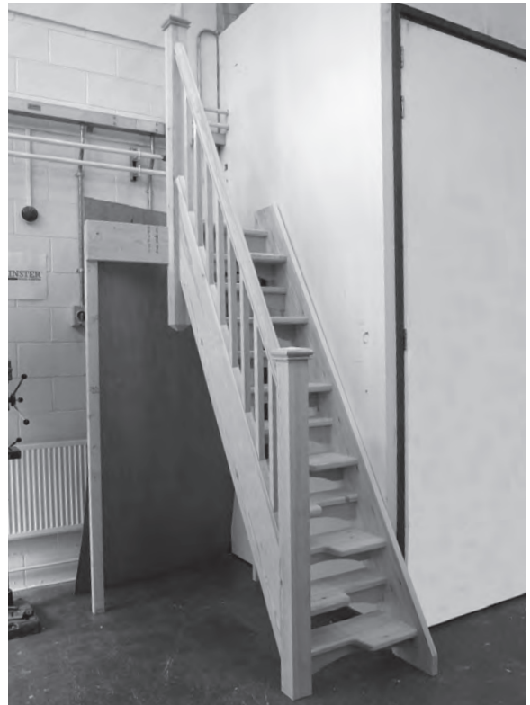
Figure 11.32 The completed alternating tread staircase with balustrade to its outside. (The fixing of wall-mounted handrail is demonstrated in chapter 12.)
