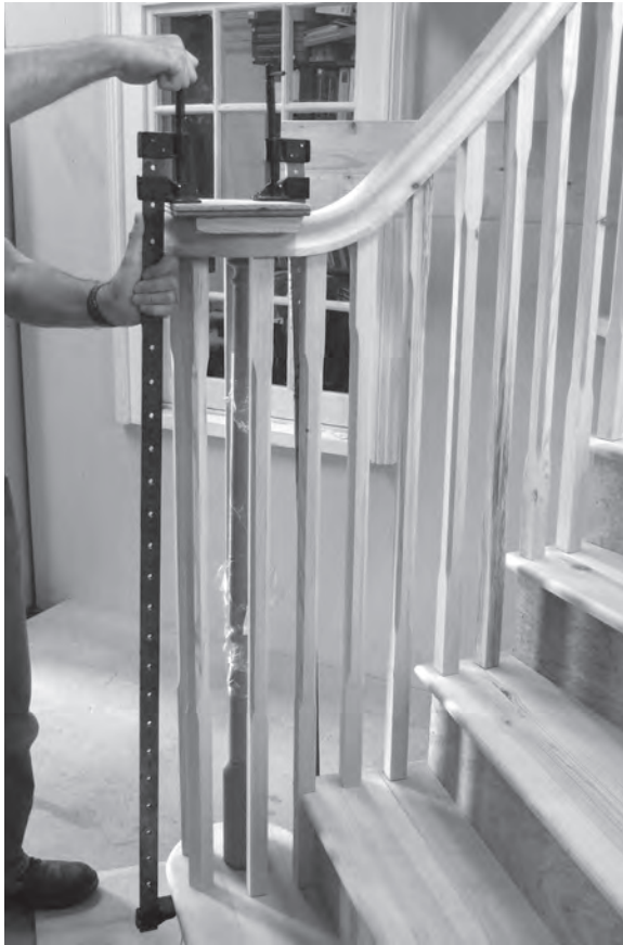
Figure 11.122 With a protective board on top of the volute, the volute newel and balusters forming the 'bird cage' can be pulled up by clamping gently against the curtail tread's nosing.
