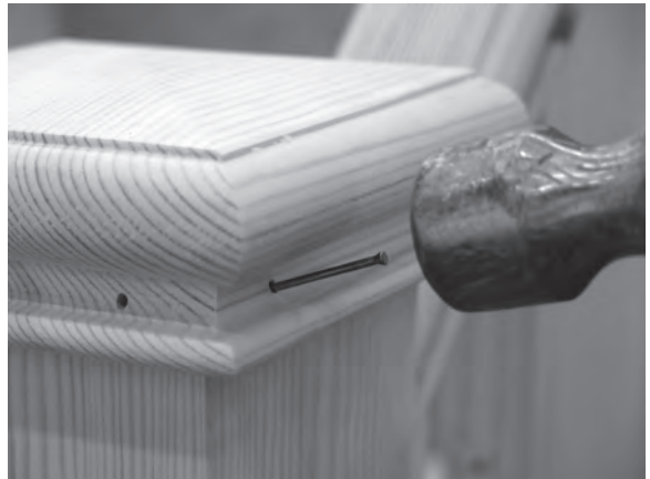
Figure 10.74 The newel cap is glued and nailed through pre-drilled holes in its sides into the newel post.
