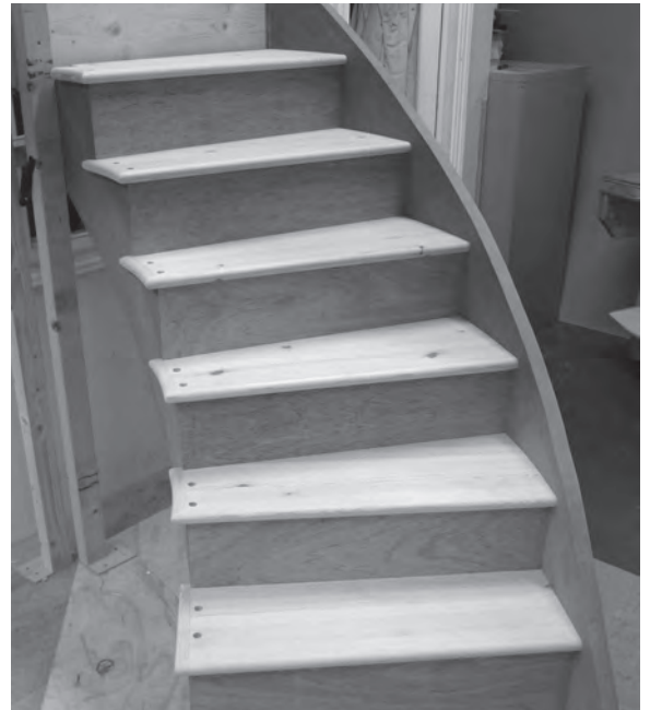
Figure 8.125 The staircase so far – looking good!
