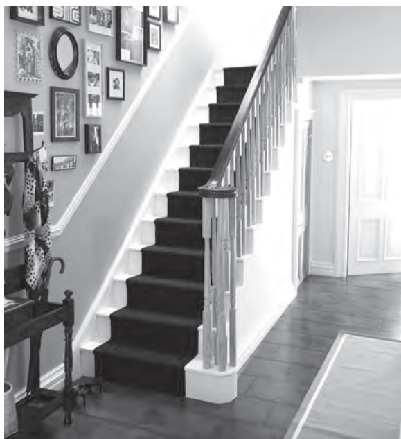
Figure 10.1 A curtail starting step corresponds to the handrail's volute, its projection forming the widest part of the flight. (Photo courtesy of Richard Burbidge Ltd)
