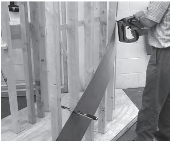
Figure 8.34 A gentle, sweeping curve must be maintained as the facing plywood is bent round the form. Pinning close to the facing plywood's edges will mean less damage later during its removal from the studs.
