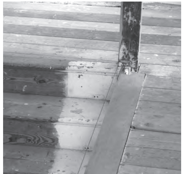
Figure 12.49 A string line is tied to the upper newel post and pulled parallel with the landing nosing.
