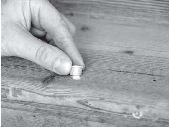
Figure 12.6 Use pellets to hide screws if the stairs are to remain uncarpeted.
