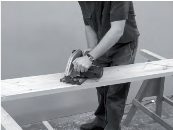
Figure 7.8 With practice, a hand-held circular saw can be used to accurately cut an open string without the need for a straight edge.
