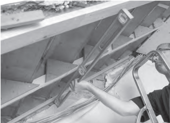
Figure 12.25 (above) and Figure 12.26 (below) Timber battens fixed to the strings level the underside of the flight and provide clearance for the electric cables.
