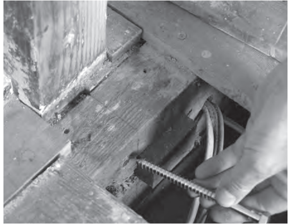
Figure 12.42 (above), Figure 12.43 (below), and Figure 12.44 (bottom of page) The loose newel post is secured to the adjacent trimming joist with two coach screws.
