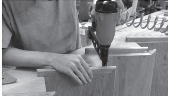
Figure 10.53 The nosing/scotia returns are glued and nailed in place.
