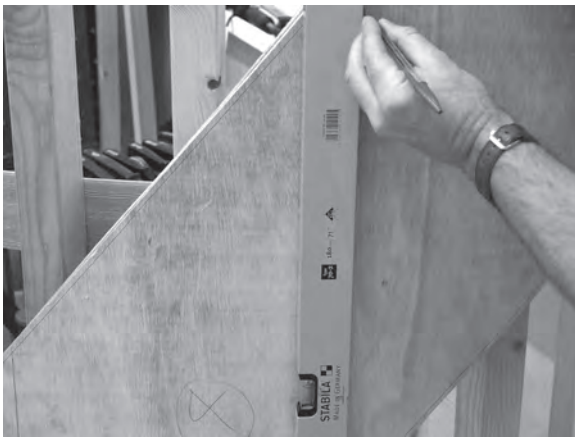
Figure 8.50 (above) and Figure 8.51 (below) Riser lines are transferred from the rod to the open string by plumbing up using a spirit level.
