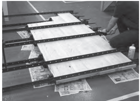
Figure 5.7 The strings (seen here), newel posts, and treads are glued up to achieve their finished dimensions.
