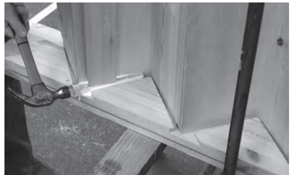
Figure 4.87 Glue and wedge the staircase.
