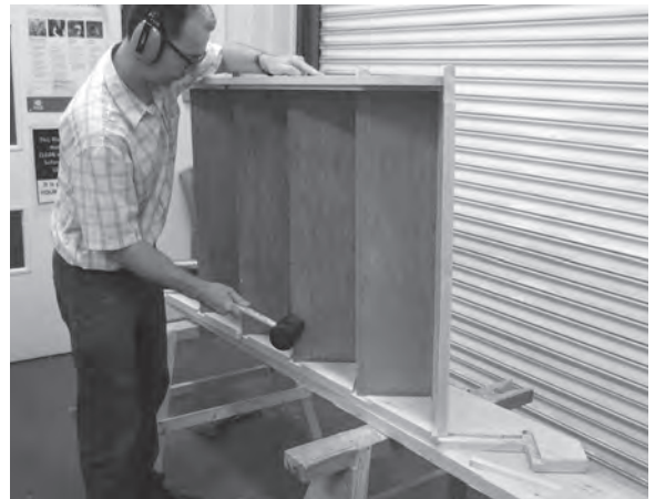
Figure 7.21 The remaining risers and treads are installed.
