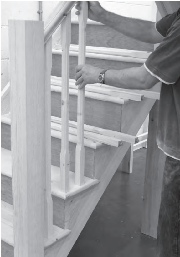
Figure 11.46 Lay the cut balusters in pairs on their respective treads ready for installation.
