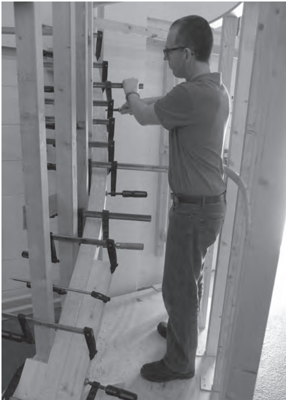
Figure 11.53 Following the pitch line of the circular staircase at its open side, the glued strips are clamped to the bending form.
