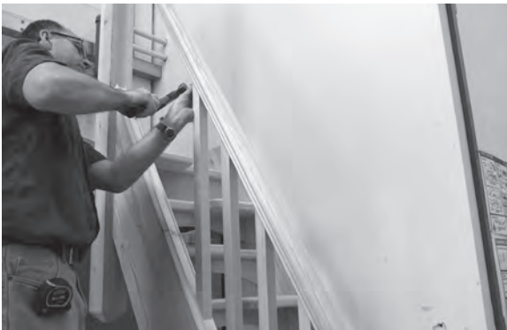
Figure 11.30 Glue and skew-nail each baluster at both ends before inserting the next pair of infill fillets which should also be glued and nailed.
