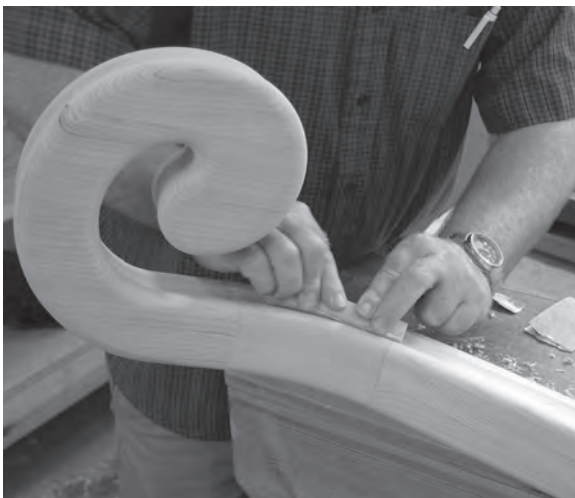
Figure 11.90 Steve gives the newly assembled handrail and volute a light clean up with 180-grit sandpaper.
