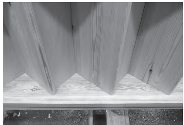
Figure 4.88 While gluing and wedging, ensure that the treads and risers are going up fully within their string housings.
