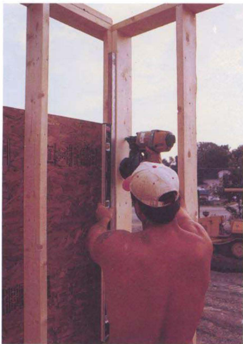
Use a level to plumb exterior corners before fastening corner studs and top plates.
