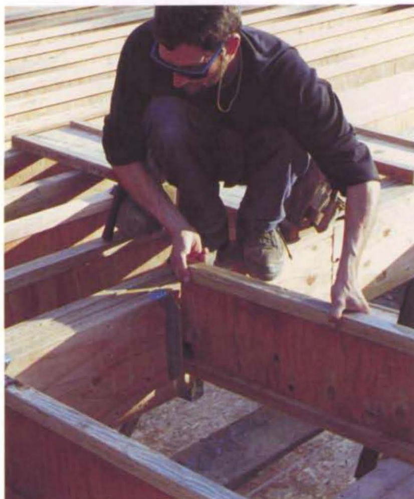
I-joists use special hangers with horizontal tabs that wrap over the flanges of adjoining I-joists or LVL beams. Squirting a little glue in the seat of the hanger minimizes the potential of a squeaky floor. (Photos by Roe A. Osborn, courtesy Fine Homebuilding magazine, © The Taunton Press, Inc.)
