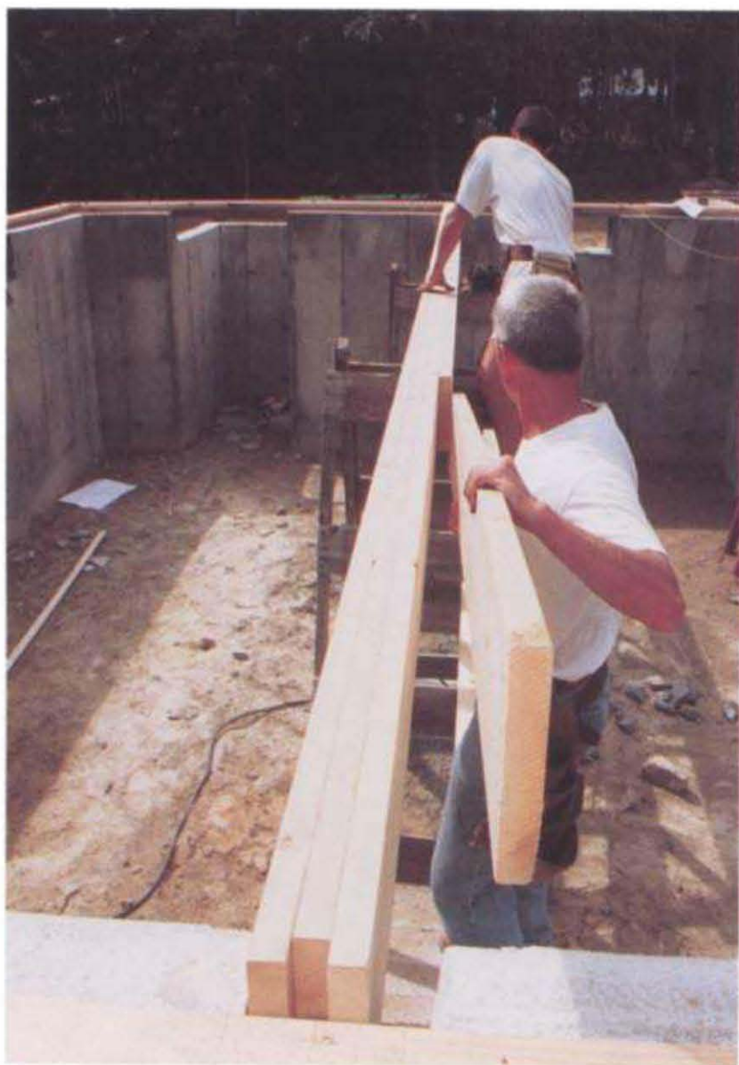
Add layers to the beam, one piece at a time. Check that the beam is straight before nailing off each layer, because it will be difficult to straighten the beam later. (Photo by Tom O'Brien, courtesy Fine Homebuilding magazine, © The Taunton Press, Inc.)
