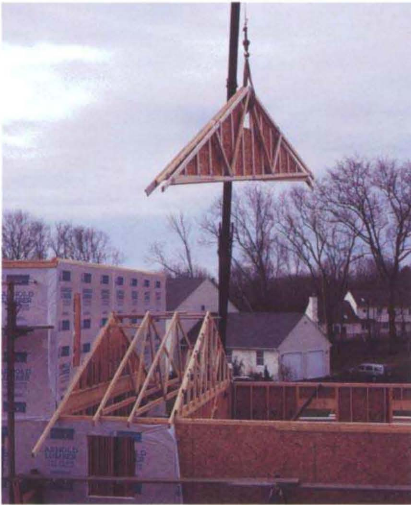
The first gable truss is sent up with two regular trusses. By sending the first three trusses up together, the crane will be able to hold the gable truss steady while the other trusses are set and the braces are attached to the gable truss. (Photo by Roe A. Osborn, courtesy Fine Homebuilding magazine, © The Taunton Press, Inc.)
