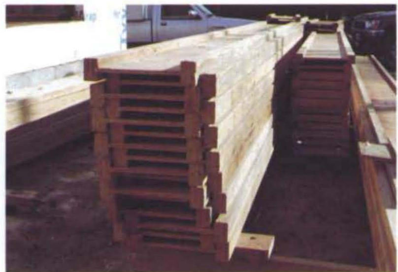
Whenever possible stack I-joists in the upright position or block them level every 10 ft., if stacked flat as above. (Photo by Roe A. Osborn, courtesy Fine Homebuilding magazine, © The Taunton Press, Inc.)
