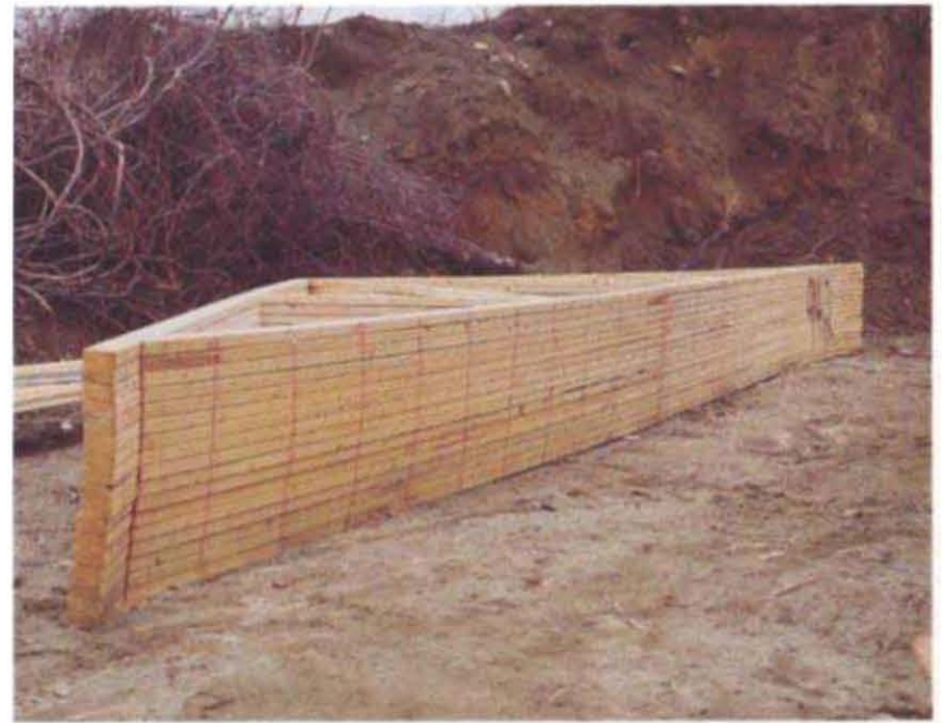
With the trusses stacked neatly on the ground, layout lines are drawn on all of them at once. The line closest to the tail will be used to position the truss on top of the wall plates. The other lines are for ceiling strapping. The top cords are laid out for roof sheathing. (Photo by Roe A. Osborn, courtesy Fine Homebuilding magazine, © The Taunton Press, Inc.)
