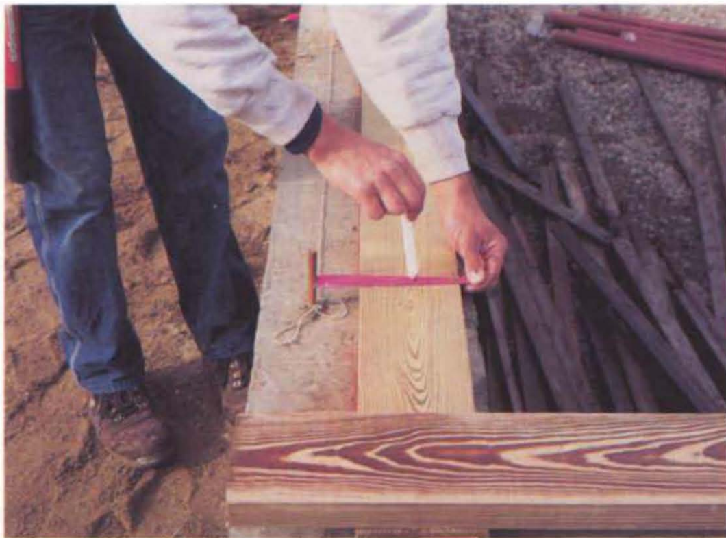
Mark the location of the foundation bolts on the mudsill for drilling. Line the mudsill plate stock on the opposite side of the chalkline and use an anchor bolt–marking tool to mark the bolt location. (Photo by Roe A. Osborn, courtesy Fine Homebuilding magazine, © The Taunton Press, Inc.)
