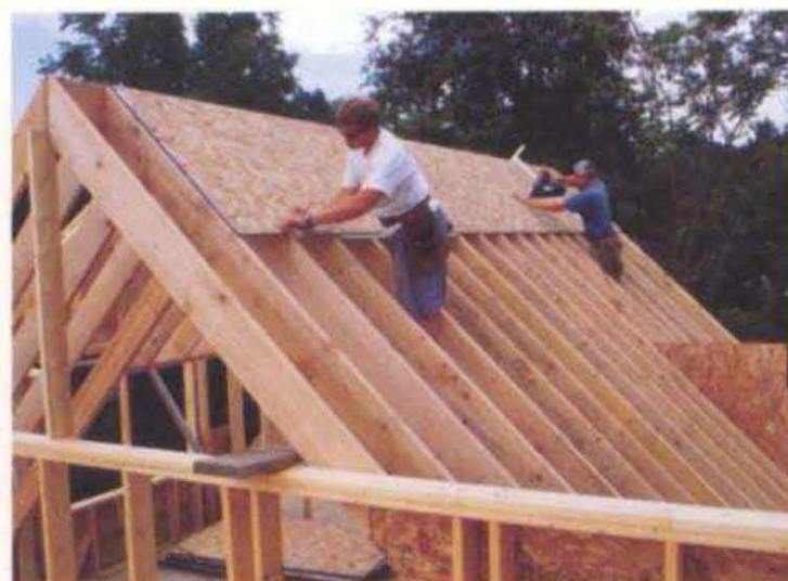
It's safer and easier to sheath a steep-pitched roof from the top down.
