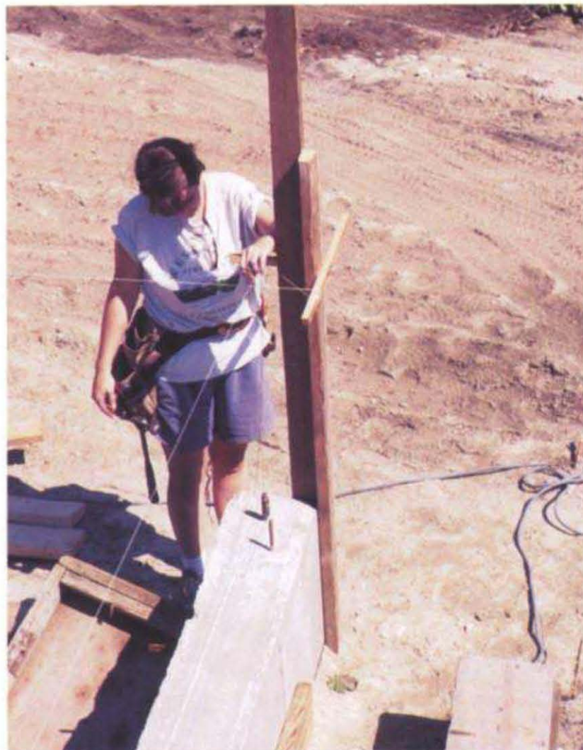
A site-built rig made from 2x stock and outriggers can be easily set up to support string lines over dropped portions of the foundation.
