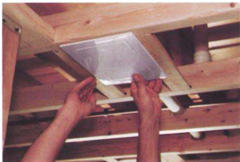
Access panels are framed to size as directed by the particular sub. (Photo by Tom O'Brien, courtesy Fine Homebuilding magazine, © The Taunton Press, Inc.)
