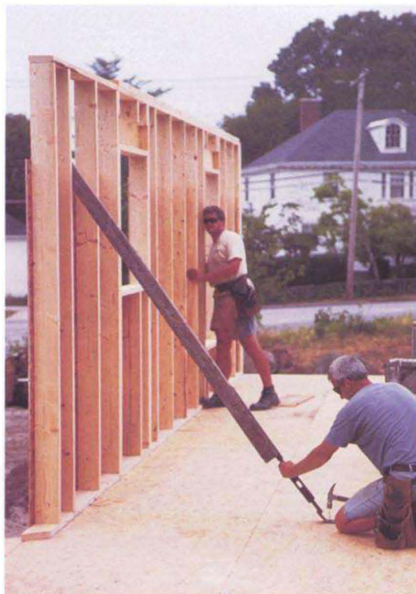
Nail adjustable wall braces or spring braces to the wall after it's tilted up. Have one worker eyeball the wall for plumb while another sets the brace.
