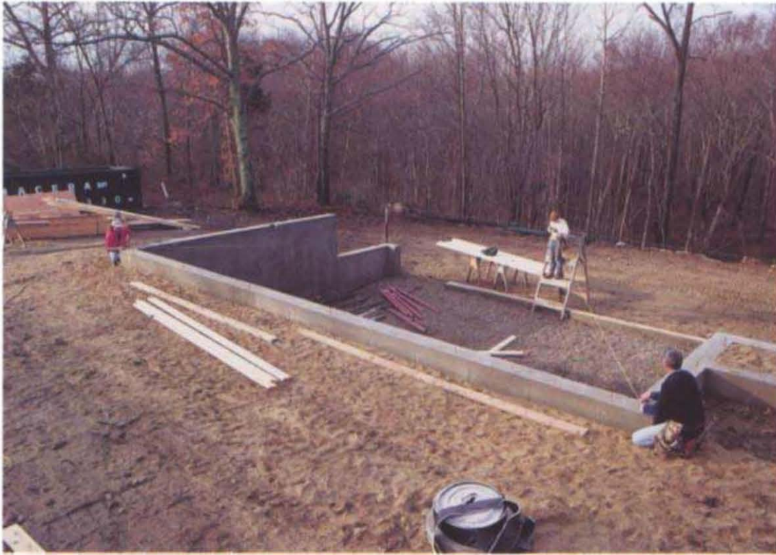
Square up the foundation by first finding the center of the opposite wall. Start the process by stretching two tape measures from the corners of the baseline you established and cross them at equal measurements over the chalkline (or, in this case, string) on the opposite foundation wall. (Photo by Roe A. Osborn, courtesy Fine Homebuilding magazine, © The Taunton Press, Inc.)
