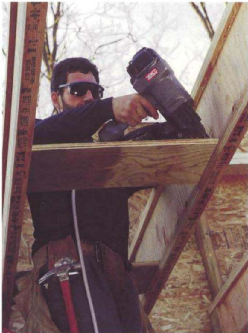
Pieces of sheathing nailed to the bottom edges of I-joist flanges provide blocking to nail the top plate of interior partitions that run parallel to the joists. (Photo by Roe A. Osborn, courtesy Fine Homebuilding magazine, © The Taunton Press, Inc.)
