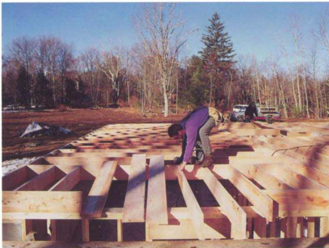
Nail through one layer of the in-floor header to support one end of the cantilevered joists. Later, nail on the additional layers of the header and install joist hangers to secure the connection permanently. (Photo by Roe A. Osborn, courtesy Fine Homebuilding magazine, © The Taunton Press, Inc.)
