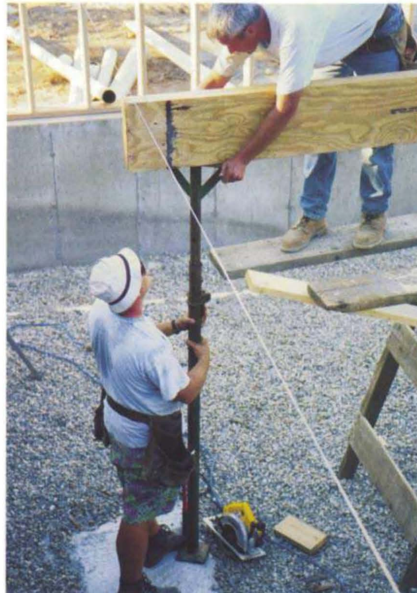
Heavy-duty screw jacks safely support heavy loads until they are ready for the permanent columns. The jacks also adjust loads very easily.
