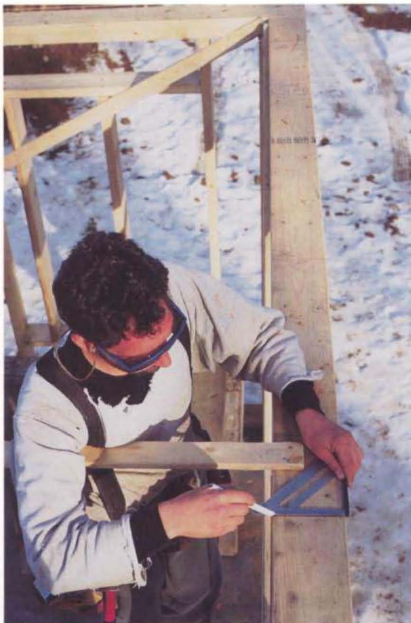
Draw a square line to indicate the side of each of the common joists marked out, and scribe an X on the side of the line where the joist will rest. (Photo by Roe A. Osborn, courtesy Fine Homebuilding magazine, © The Taunton Press, Inc.)
