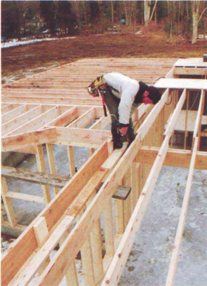
Install squash blocks to transfer concentrated loads through the floor joist system. The grain of the blocks is oriented vertically. The blocks can be installed when framing the floor deck or from beneath after the subfloor is installed. (Photo by Roe A. Osborn, courtesy Fine Homebuilding magazine, © The Taunton Press, Inc.)
