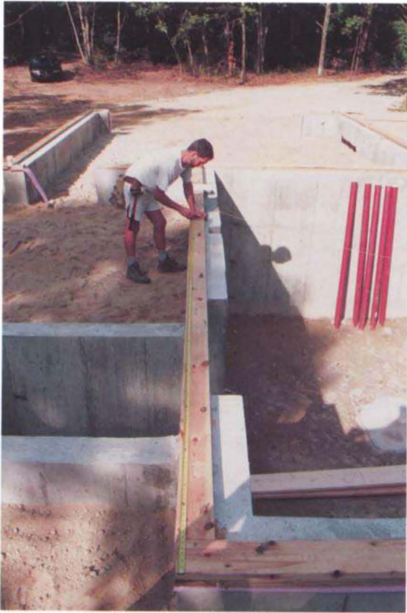
Measure and mark the precise location for the center beam within the beam pocket. Make the marks on the mudsill and line up the beam with the marks once it's installed. (Photo by Tom O'Brien, courtesy Fine Homebuilding magazine, © The Taunton Press, Inc.)
