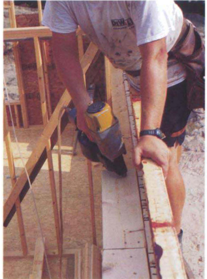
Before installing the subfloor, nail blocking on the inside edge of the wall plates that run parallel with the joists to carry drywall or ceiling furring below. The blocking can be 2x or 1x stock. Use leftover scraps or material too warped or knotty to frame with.
