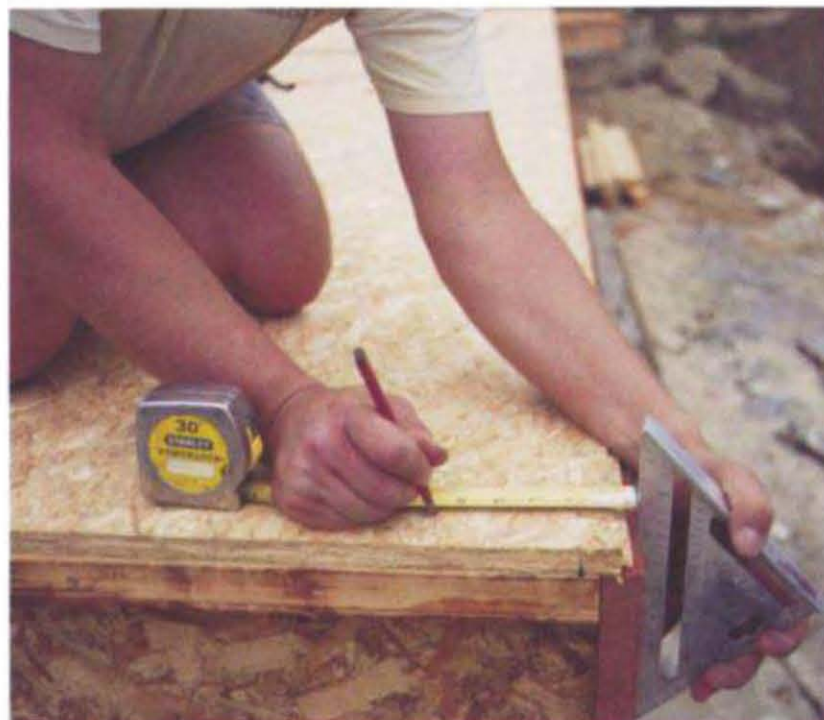
Mark the corners of the floor deck for the wall's bottom plate location, here a 2x6 wall. Measure from the edge of the rim joist, not the edge of the deck sheathing, in case the sheathing is trimmed inaccurately.
