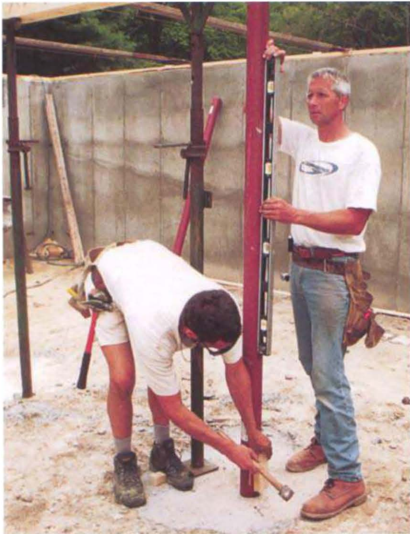
Nail the column cap plate to the bottom of the beam and tap the base until the column is plumb. (Photo by Tom O'Brien, courtesy Fine Homebuilding magazine, © The Taunton Press, Inc.)
