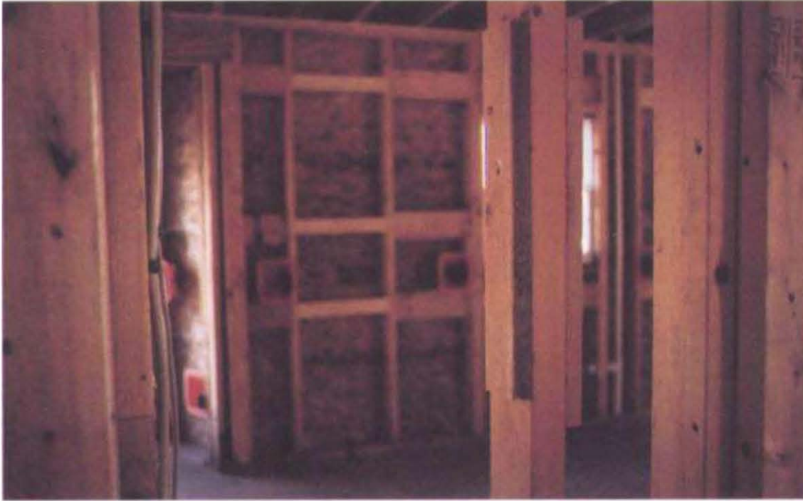
Closet blocking is installed during framing to ensure a solid backing when the shelves are installed.
