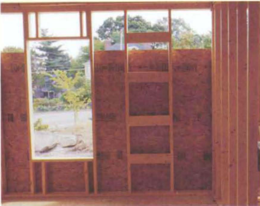
Ladder blocking nailed between adjacent common studs is easy to install during wall framing or after the walls are lifted. The blocks give fastening points for drywall at 16-in. or 24-in. intervals and space for insulation behind.
