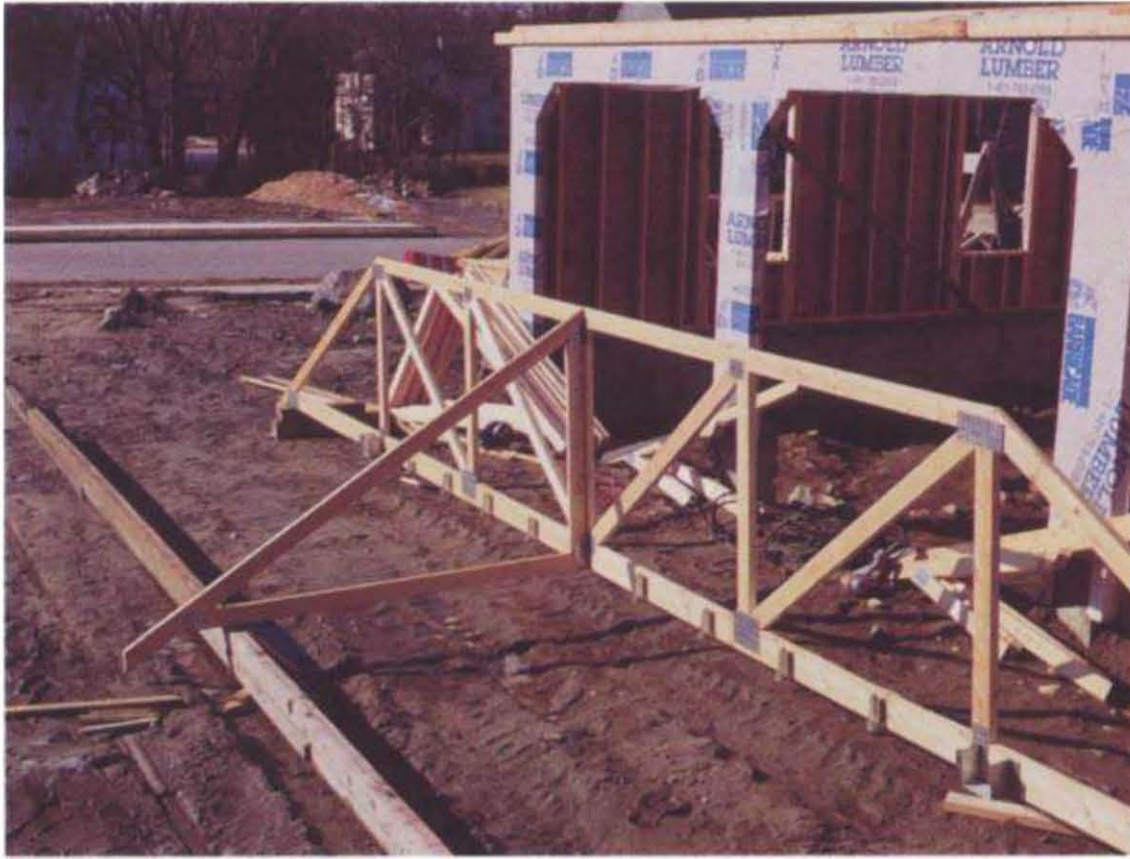
On a hip roof built with trusses, a jack truss holds the girder upright. The center face jack is tacked to the girder truss to keep it vertical while the rest of the face jacks are installed. (Photo by Roe A. Osborn, courtesy Fine Homebuilding magazine, © The Taunton Press, Inc.)
