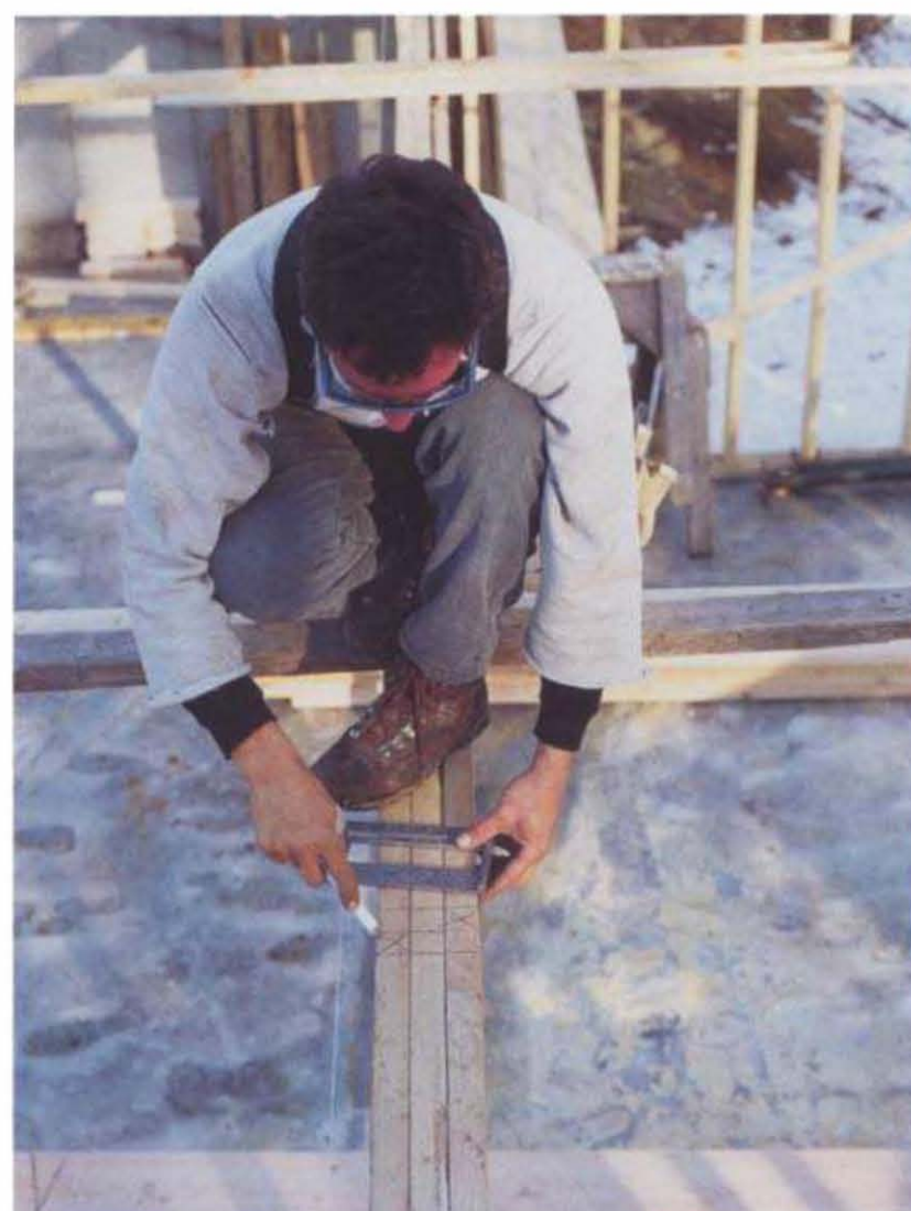
Clearly mark out the joists that will lap over the center beam with multiple lines. A single line will be obscured when joists are placed. Also indicate precisely where each joist will sit with Xs made toward the front or rear of a beam. F and R symbols can also be used to avoid confusion. (Photo by Roe A. Osborn, courtesy Fine Homebuilding magazine, © The Taunton Press, Inc.)
