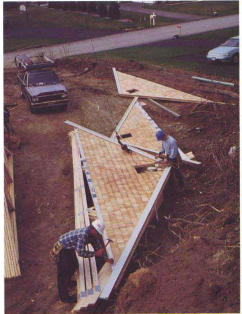
To facilitate setting the gable truss, nails are started along the bottom cord. When the truss is in position, a crew member on a ladder will drive the nails into the top plate of the gable end wall. (Photo by Roe A. Osborn, courtesy Fine Homebuilding magazine, © The Taunton Press, Inc.)
