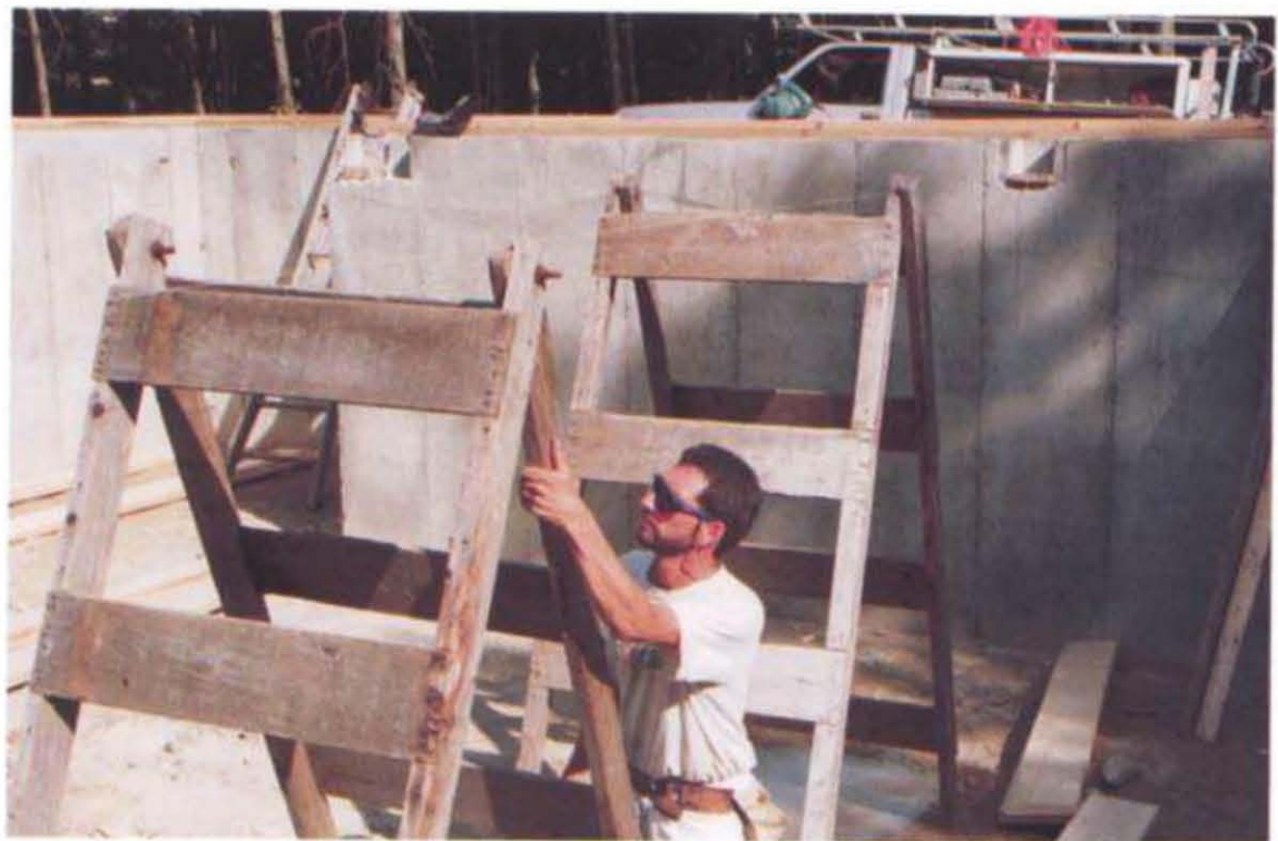
Set up staging to support the beam temporarily during assembly and installation. Gauge the height of the supports by running a string between the foundation beam pockets. (Photo by Tom O'Brien, courtesy Fine Homebuilding magazine, © The Taunton Press, Inc.)
