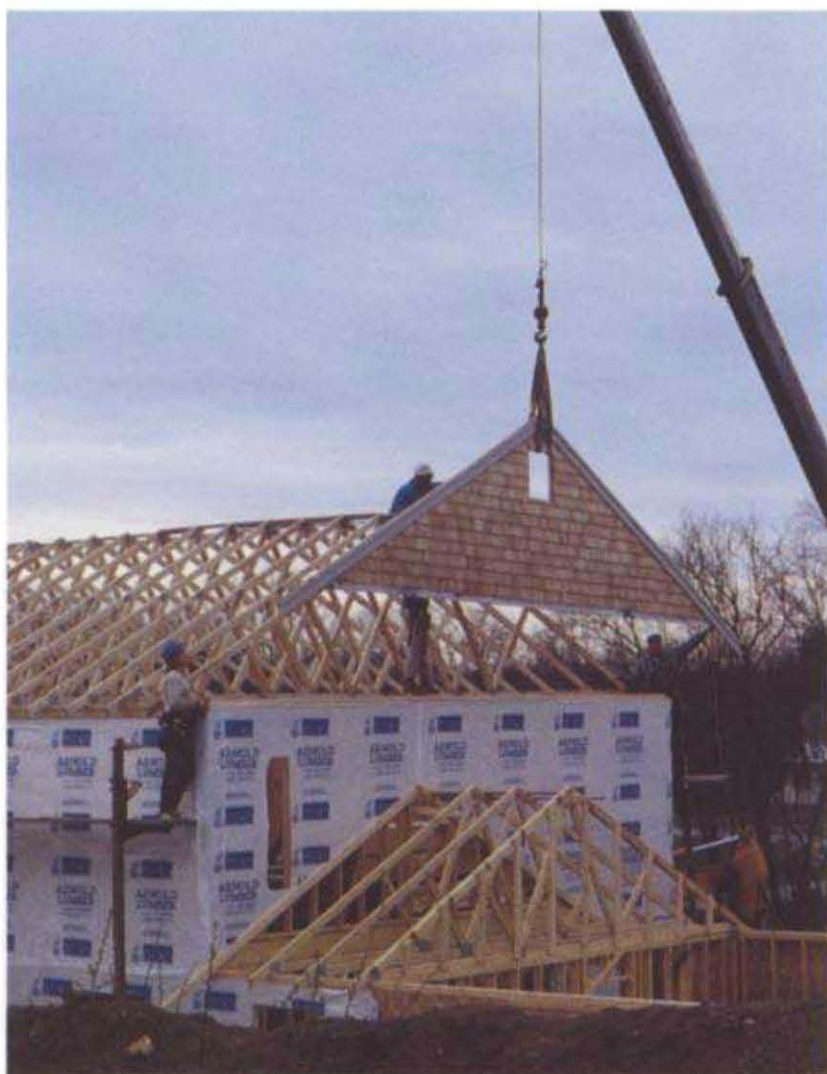
The gable end is lowered into place to complete the installation of the trusses on the main roof. (Photo by Roe A. Osborn, courtesy Fine Homebuilding magazine, © The Taunton Press, Inc.)
