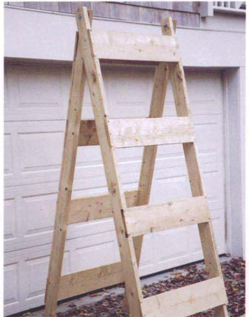
A-frames have a multitude of uses on a framing job and are easy to build.
