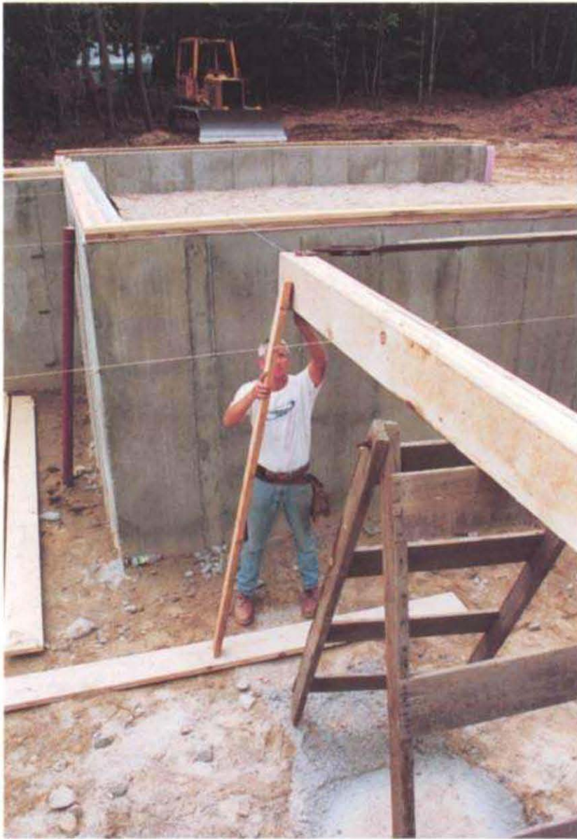
Sometimes beams are interrupted by a detail in the floor, like a stair opening or chimney hole. Let the beam run long into the opening space and trim the end later, after the opening size is established. (Photo by Tom O'Brien, courtesy Fine Homebuilding magazine, © The Taunton Press, Inc.)
