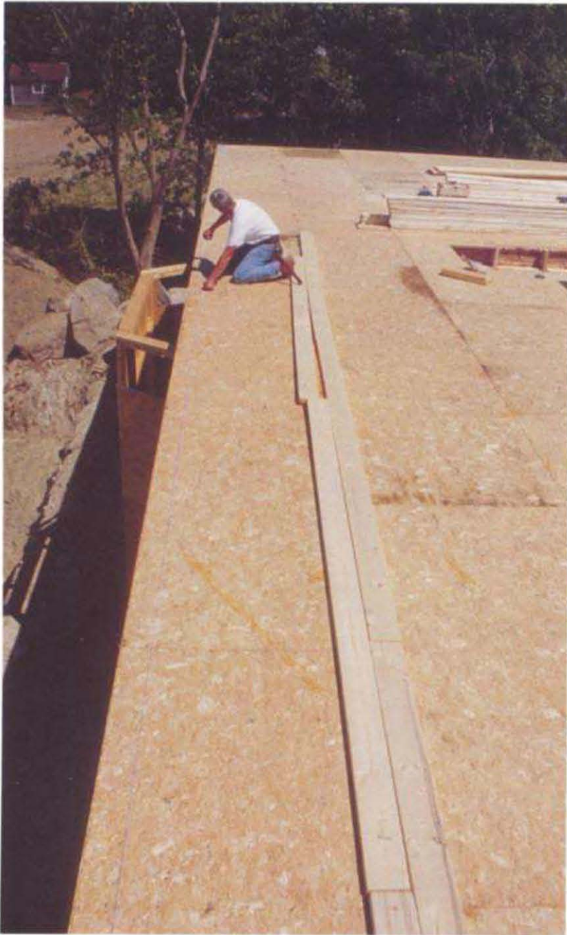
Lines snapped on the deck will be used to align the bottom plate of the wall once it has been lifted.
