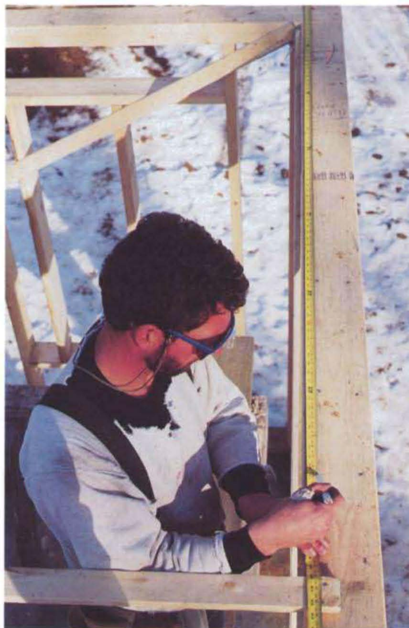
Stretch a tape measure from the corner of the mudsill or top plate where the joist layout begins. Make marks for the side of each common joist. (Photo by Roe A. Osborn, courtesy Fine Homebuilding magazine, © The Taunton Press, Inc.)
