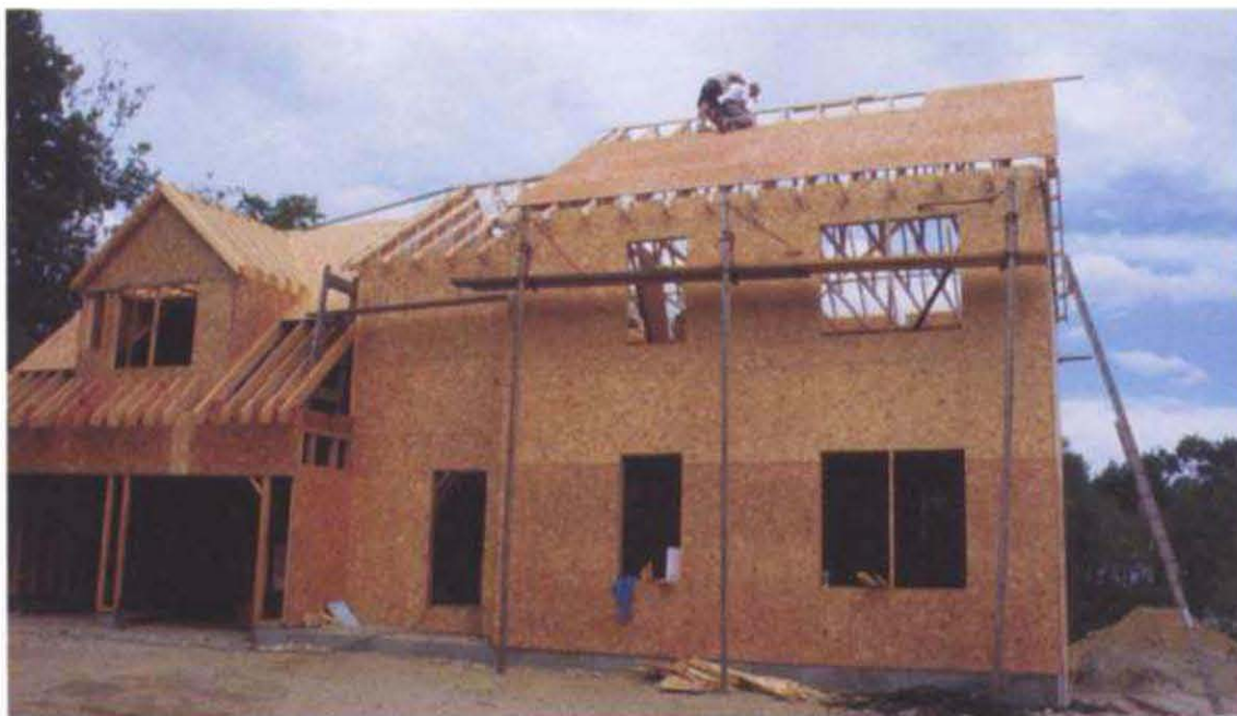
This house uses a combination of roof systems. It has a manufactured truss roof for the main house and a roof system made from cut-on-site rafters for the garage.
