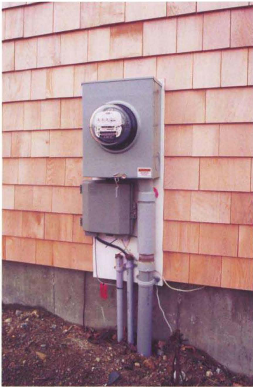
A backing for the electric meter makes for easy flashing and identifies the exact location in which the meter is to be installed.
