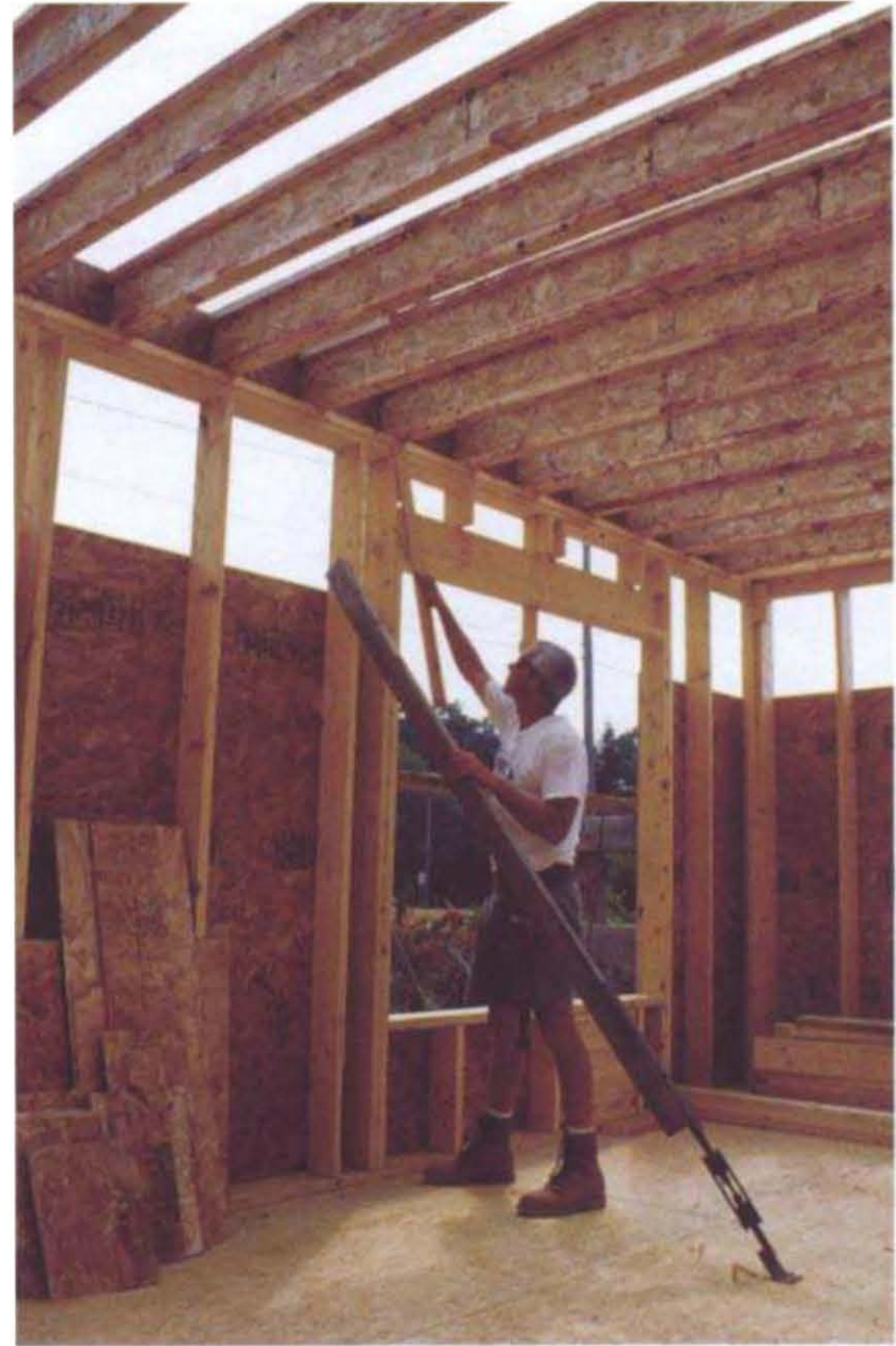
One person can do the job of two by using a turnbuckle to brace and straighten any framing member.
