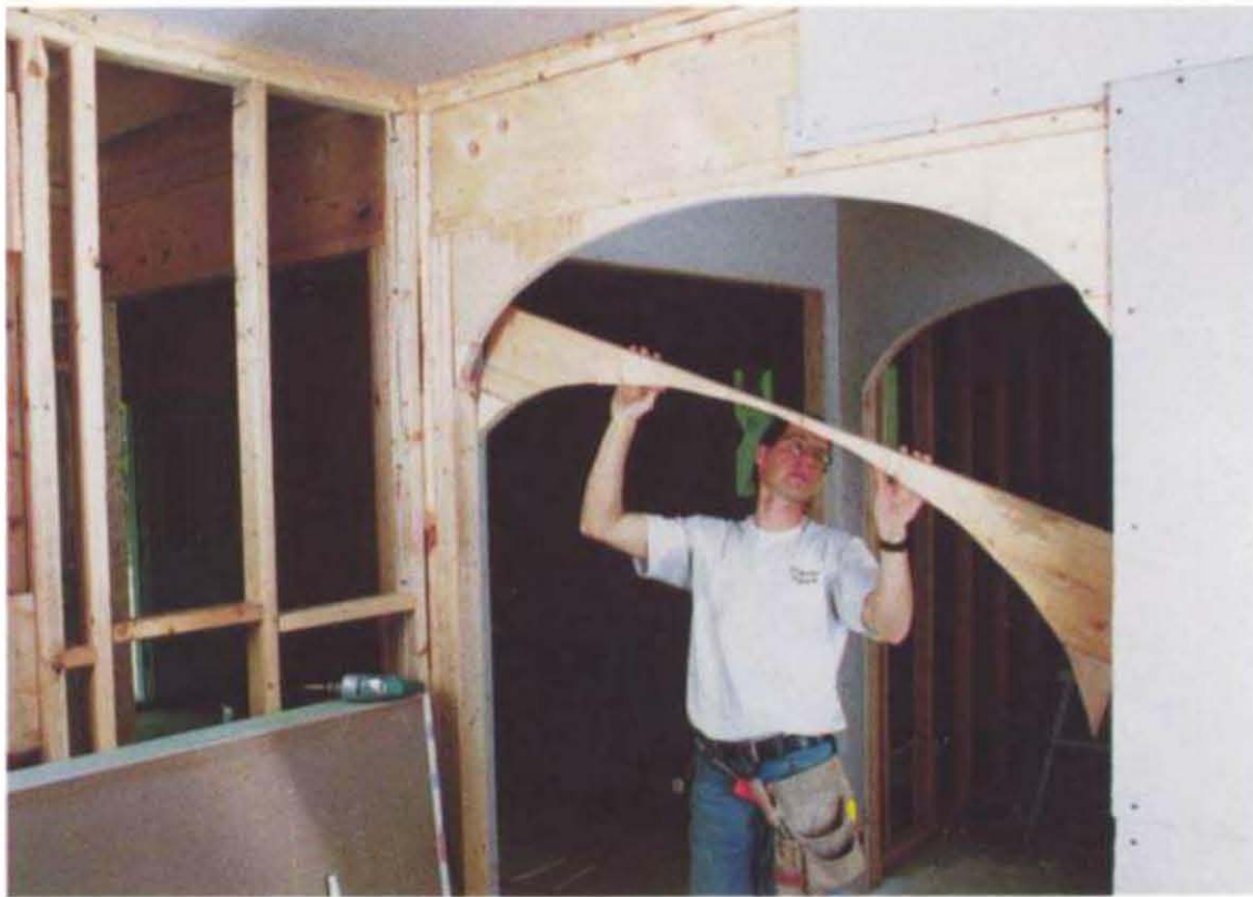
A radius detail is added to the door opening after it has been framed. (Photo by Tom O'Brien, courtesy Fine Homebuilding magazine, © The Taunton Press, Inc.)
