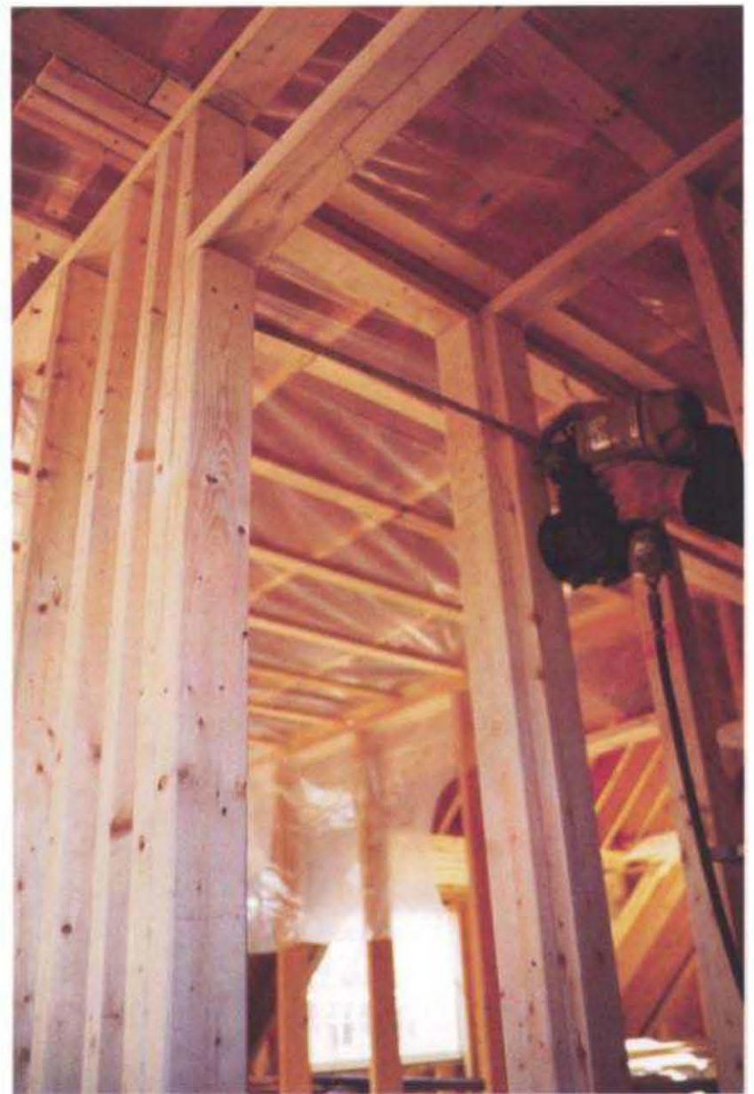
Skip short walls when snapping chalklines for the top-of-the-wall location. Frame the diminutive walls last and just measure from a nearby parallel wall.
