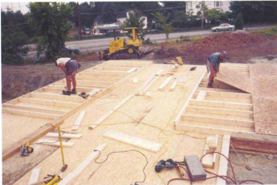
Exterior walls are framed on top of the recently finished floor deck and will be tilted upright after they are sheathed.
