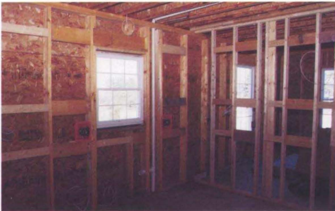
By blocking for all of the cabinets, the cabinet installer doesn't have to rely on attaching the cabinet to just studs, possibly giving the cabinet insufficient support. An upper kitchen cabinet loaded with dishes can be very heavy.
