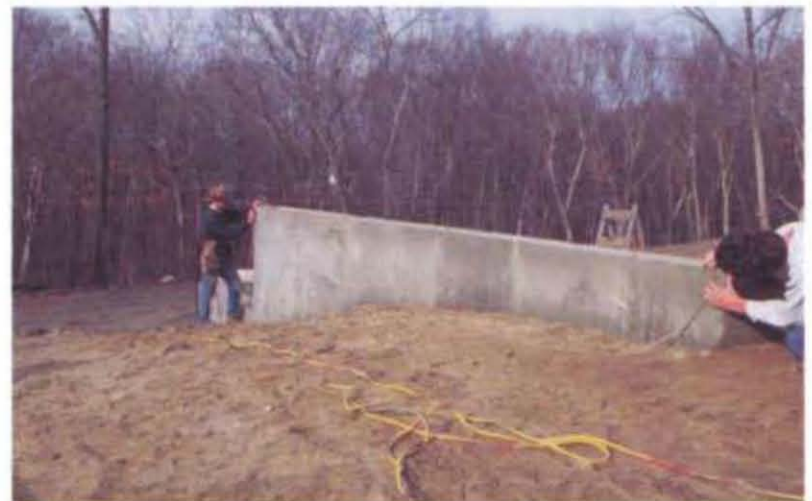
A water level is quick and easy to use. Raise and lower the hose until the meniscus matches the reference mark, then mark the advancing corner. (Photo by Roe A. Osborn, courtesy Fine Homebuilding magazine, © The Taunton Press, Inc.)
