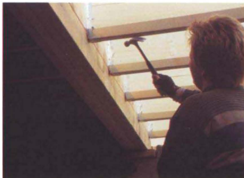
Metal joist hangers connect joists to beams and headers. Select hangers sized for the joists being installed.
