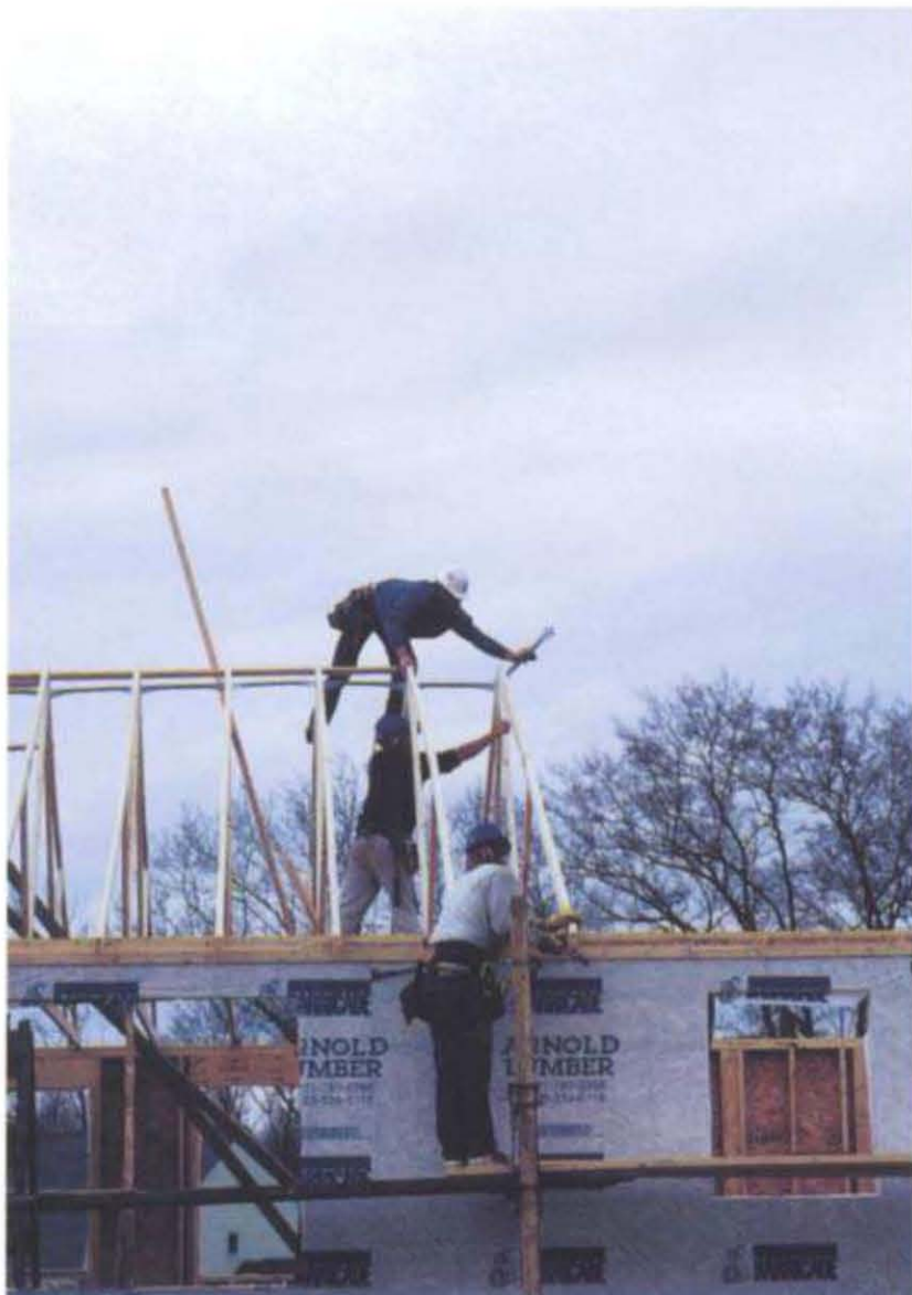
Truss spacers (made by Truslock, Inc.) are worth the investment if you will be doing most of your jobs with trusses. (Photo by Roe A. Osborn, courtesy Fine Homebuilding magazine, © The Taunton Press, Inc.)
