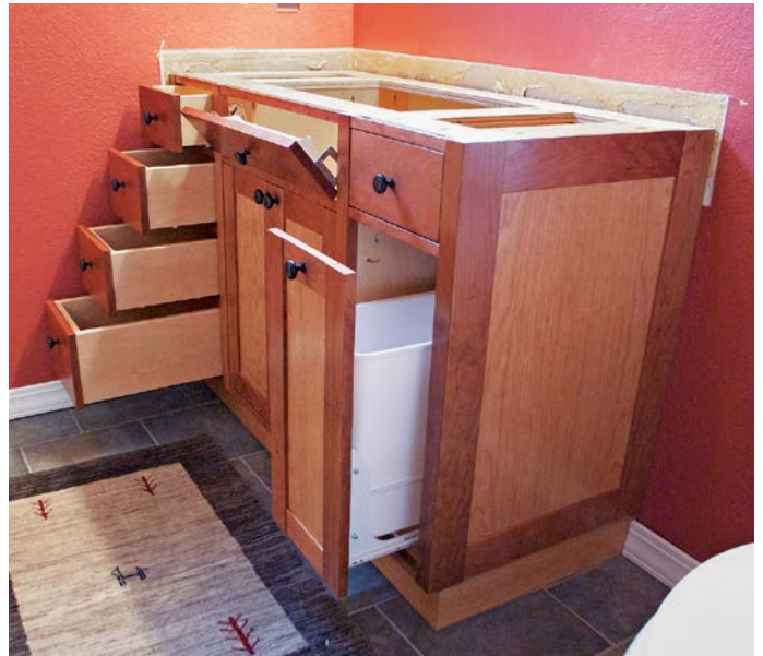
Finish up by installing the knob handles on the doors and drawer faces.
