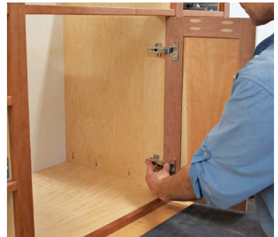
The hinges clip onto the bases, which makes installation a snap.
