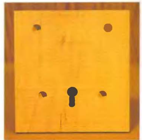
Face lamination with all holes bored out.
