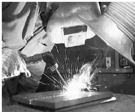
Fig. 1.6 Welding using shielded metal arc welding process
