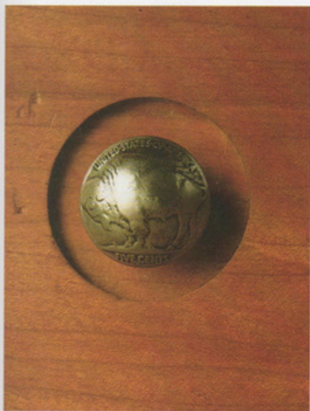
The drawer pulls were fashioned from buffalo nickels made by a flea-market craftsman for use as belt studs or buttons. Photo by Alec Waters.
