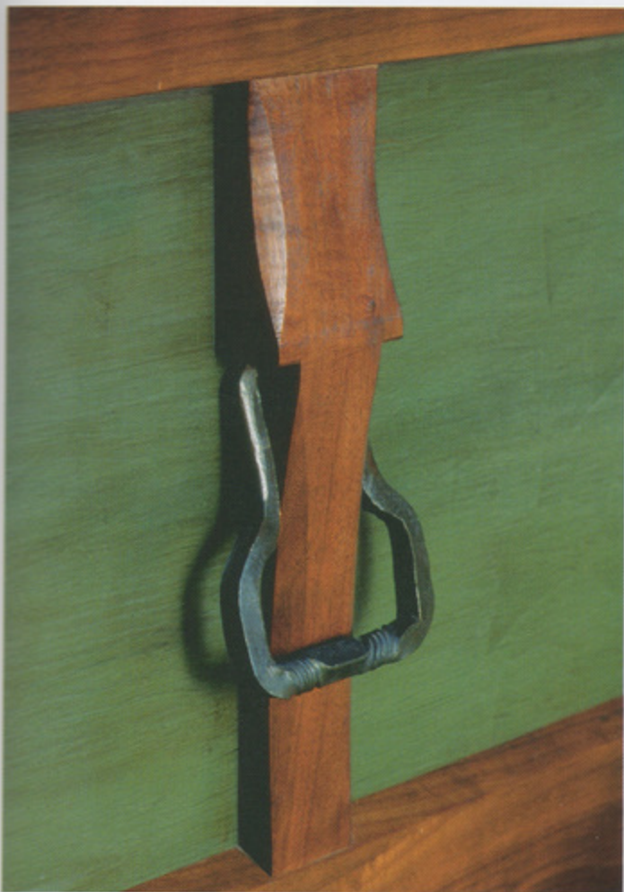
Forged iron handles are set into sculpted walnut blocks on the sides of the chest. Photo by Ray Fischer.
