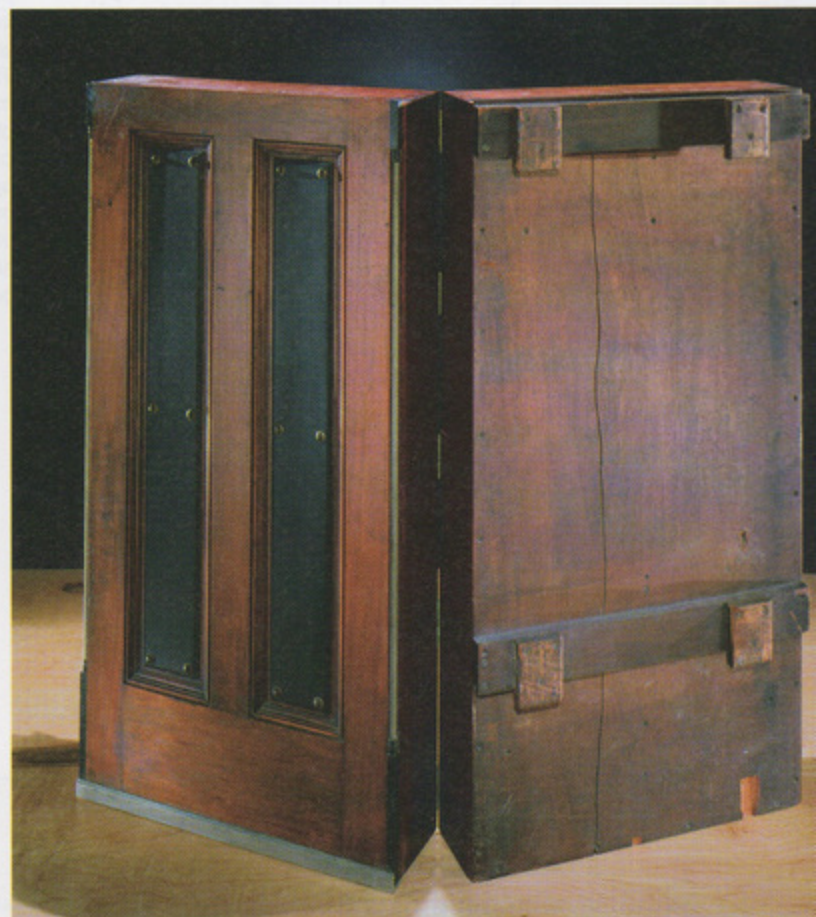
Above: A rear view of the Studley cabinet, shown open on p. 76. Two mounting rails are fitted to the back panel. Mating ledger strips would have been attached to the shop's wall studs. Photo courtesy of the Smithsonian Institution.
