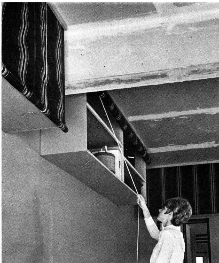
Canvas curtains roll up backwards; pulleys and most cords are hidden inside the cabinet under the 1 by 2 trim.
