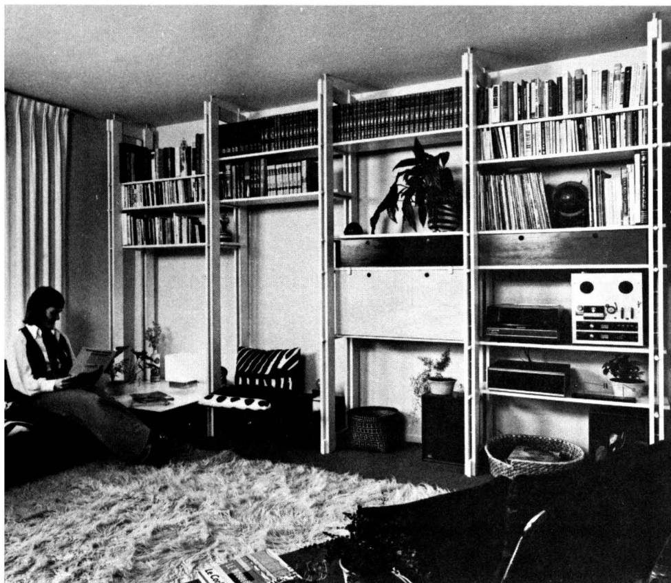
Small pegs fitted between vertical 1 by 4s support \frac{3}{4} " dowels; the dowels in turn support the 1 by 10 shelves.
