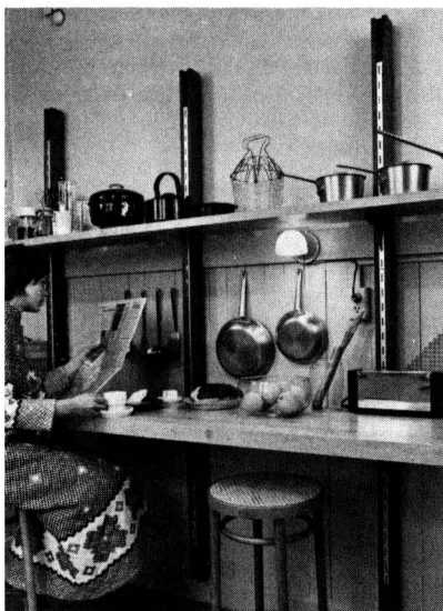
Kitchen counter and shelf are supported by heavy-duty tracks, fitted into 1" by 3/4" routed grooves in 3" by 3" redwood posts. Design: Edmund Ong, Architect.
