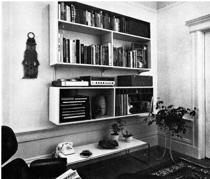
Subdivided boxes sit on brackets. Like the book wall shown at left, order of assembly is important. First screw standards to the wall and add brackets where you'll want shelves. Set the shelves on the brackets; then measure and cut the verticals to fit. Glue and nail them to the shelves. Design: Stuart Goforth, Architect.
