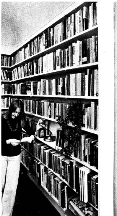
Wall of books is simply a system of shelving brackets and standards. Cut verticals to fit the already-mounted horizontal. Design: Fred W. Taylor.
