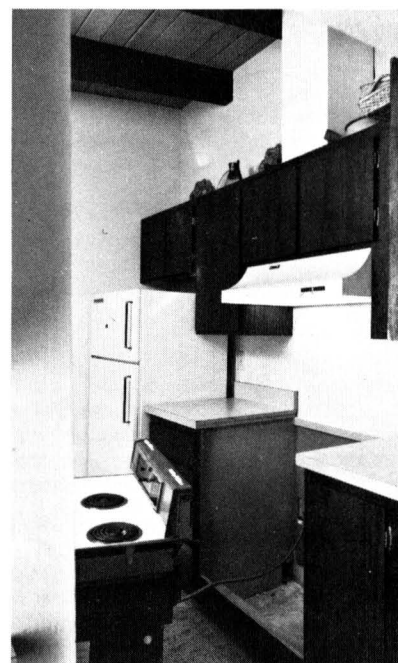
Stove unit easily fits into opening between modular cabinets. All cabinets are built using the same methods.
