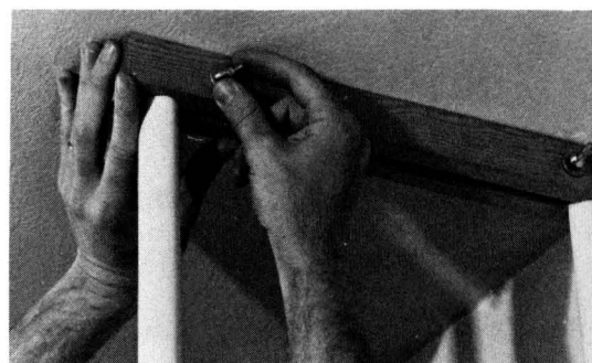
Push top supports against ceiling; then tighten wing nuts. This wedges shelving unit between ceiling and floor.
