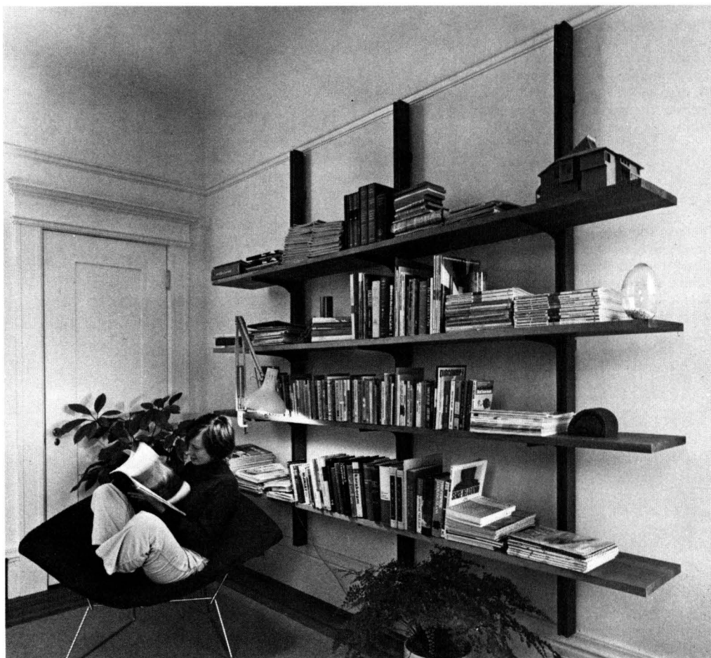
Grooves along lengths of 3" by 3" posts inset tracks for this system. Design: Edmund Ong, Architect.
