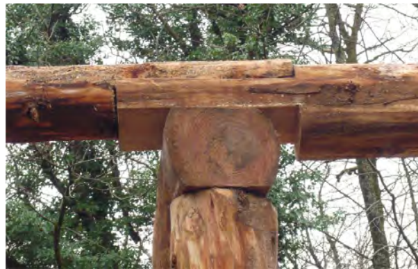
Fig. 7.20 The main joints are deceptively tricky to get to a perfect fit.
