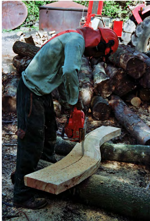
Fig. 7.36 Cutting the curved braces with a chainsaw.
