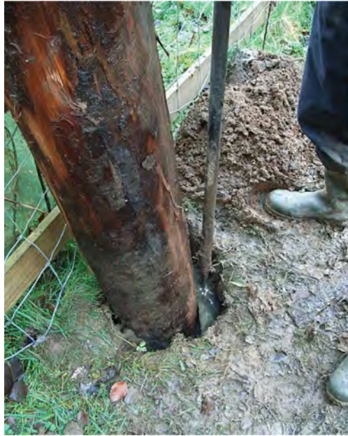
Fig. 7.8 Back filling the hole with tightly wedged rocks.
