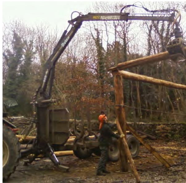
Fig. 7.19 Sam Hanafin using his timber grab to lift the joists into place.
