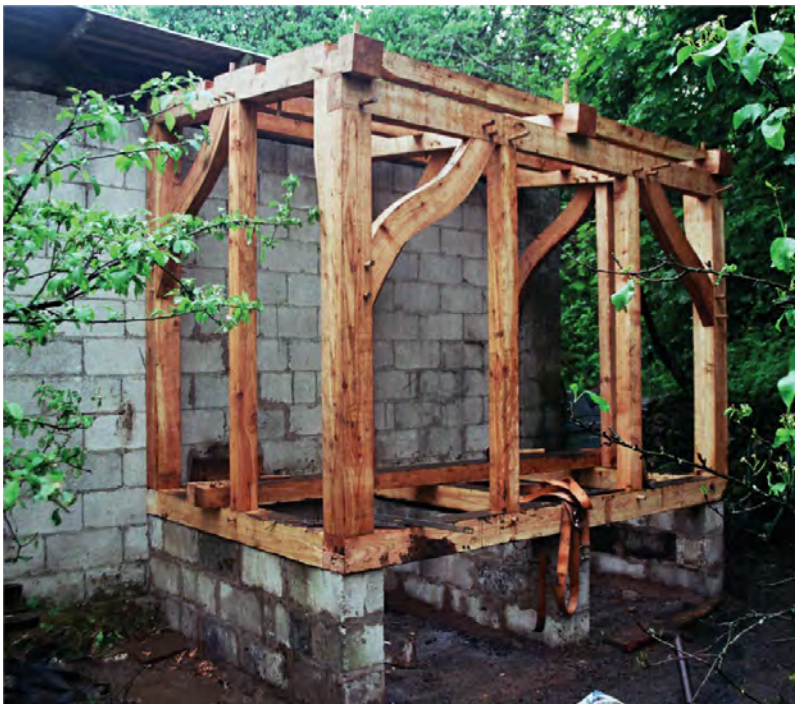
Fig. 7.38 The framework in place.
