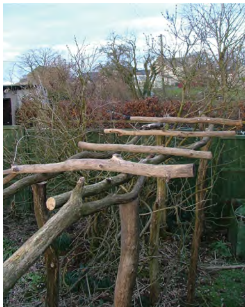
Fig. 6.16 The pergola with the cross struts fitted.
