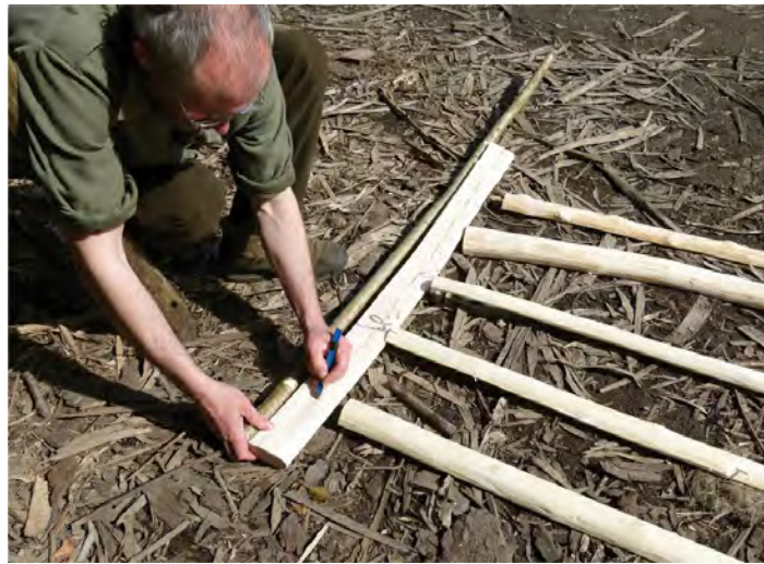
Fig. 8.6 Marking the positions of the end rails.
