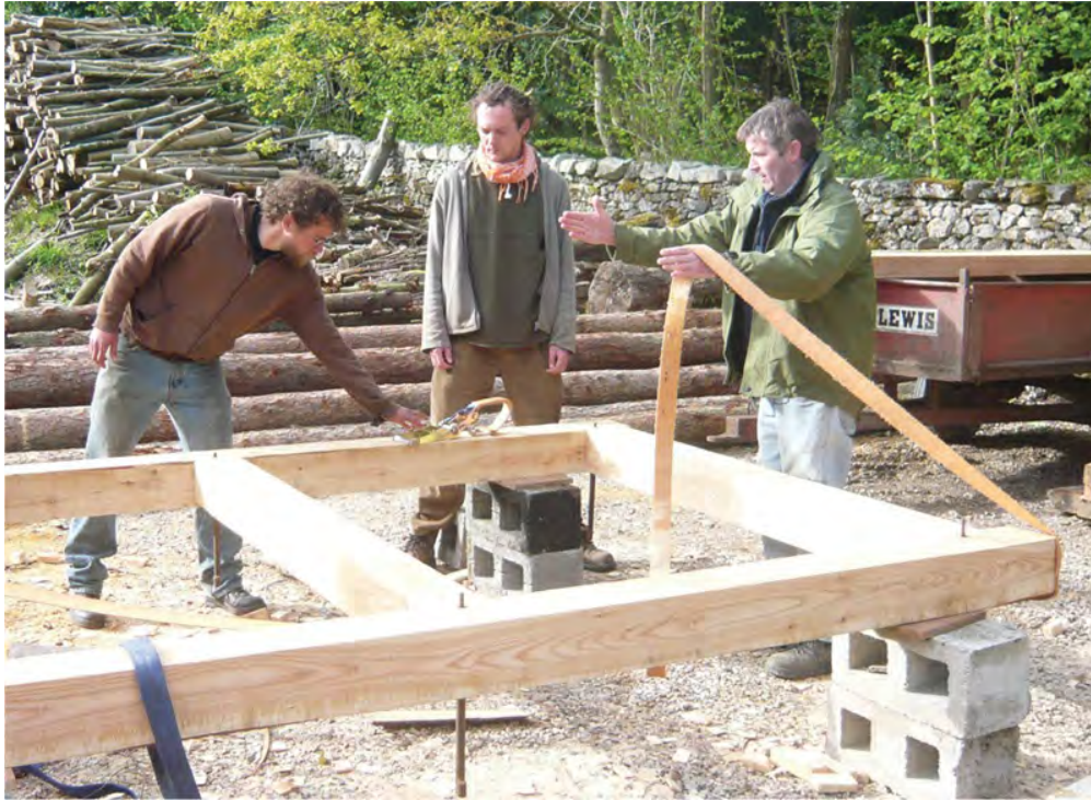
Fig. 7.31 Malcolm Lemmon teaches apprentices Sam Ansell and Rupert Hoskinson the finer arts of timber framing.
