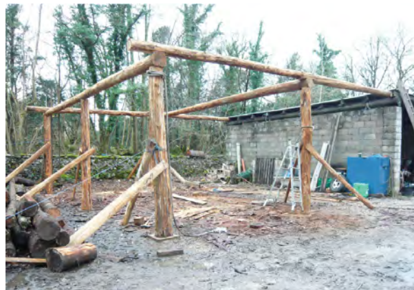
Fig. 7.21 The structure is held temporarily with struts.
