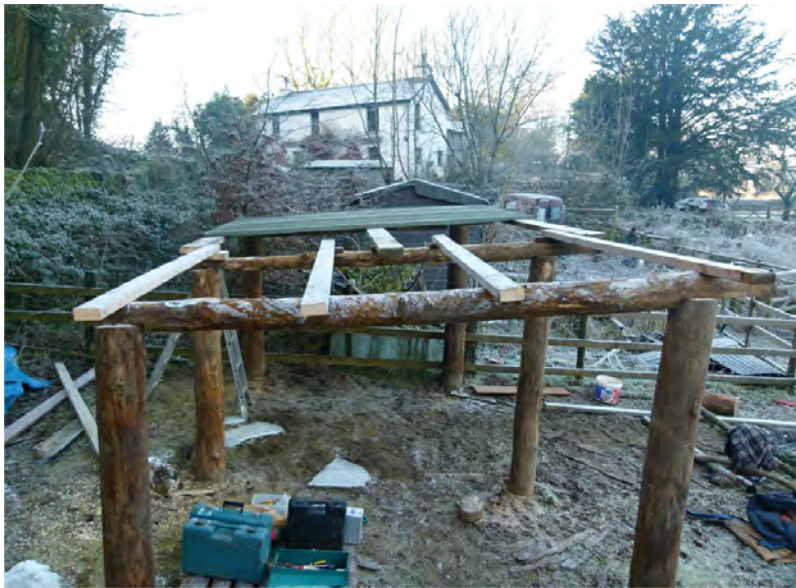
Fig. 7.13 The roof joists in place and the tin fixed to them.
