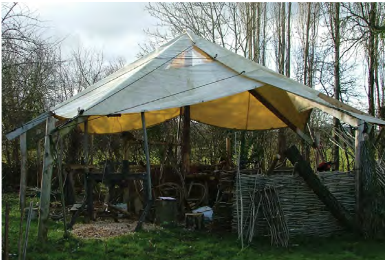
Fig. 7.2a Dave Jackson's shelter with a seven-sided design (Abbott, 2002). He has used sawn timbers for the roof but the main upright posts are of roundwood.
