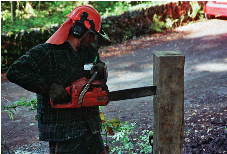
Fig. 8.12 A plunge cut with a chainsaw to make the mortice joint.
