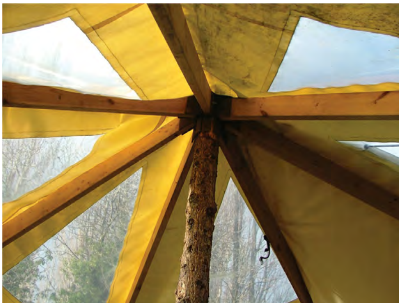
Fig. 7.2b It requires a crown piece to be made by a blacksmith, so that the seven roof timbers can be bolted securely into place. The tarp is square but has a slit to the centre so that the cut edges overlap.
