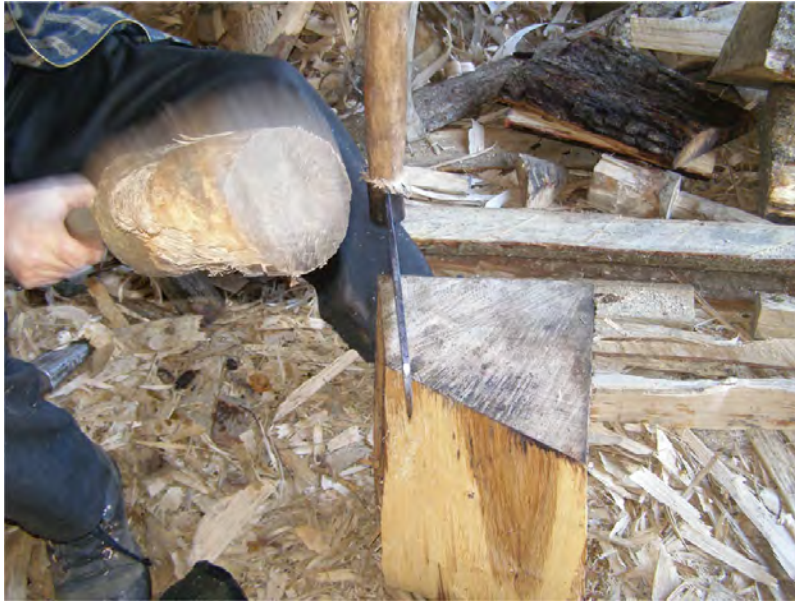
Fig. 7.42a Starting the cleft for an oak shake.
