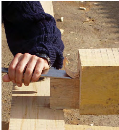
Fig. 7.33 Shaping the tenons with a chisel. (Photo: Wood Education Programme Trust)
