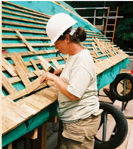
Fig. 7.45 Trimming the shakes before fitting.
