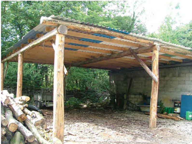
Fig. 7.16 Pole barn workshop.
