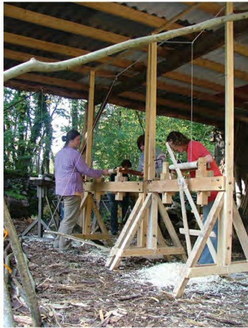
Fig. 7.23 The tin sheets fixed in place – workshops can begin.
