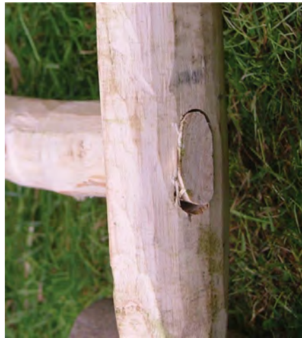
Fig. 8.7 Detail of the mortice and tenon joint.
