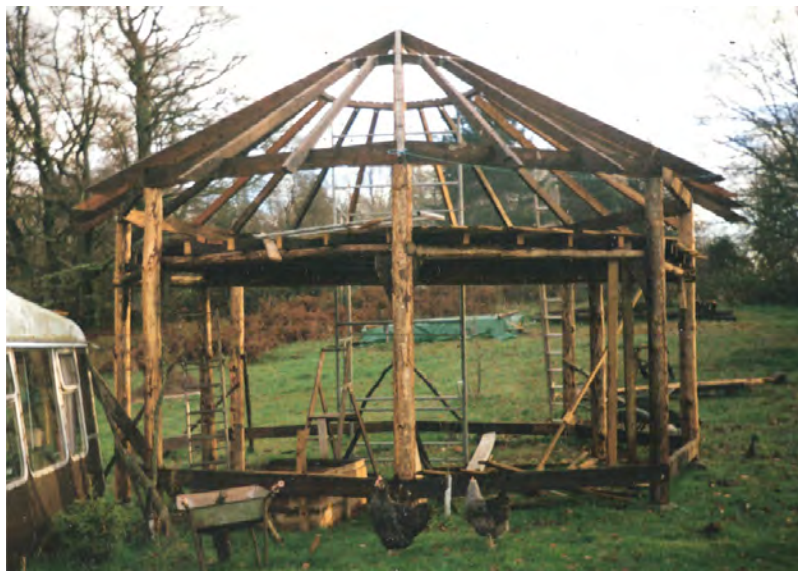
Fig. 7.24 The basic frame work of the octagonal bothy in place.
