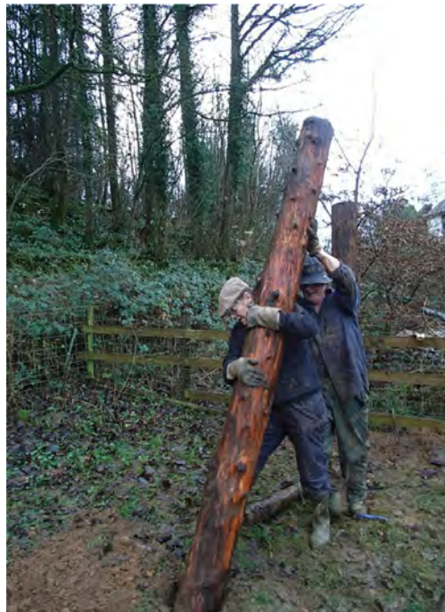
Fig. 7.7c Do make sure the hole is the right depth because once in the post is not coming out again.
