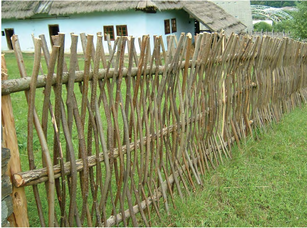
Fig. 8.18 This fence in Slovakia is made from small dimension coppice materials with three larger long horizontals per section; It was being used as sheep fencing.
