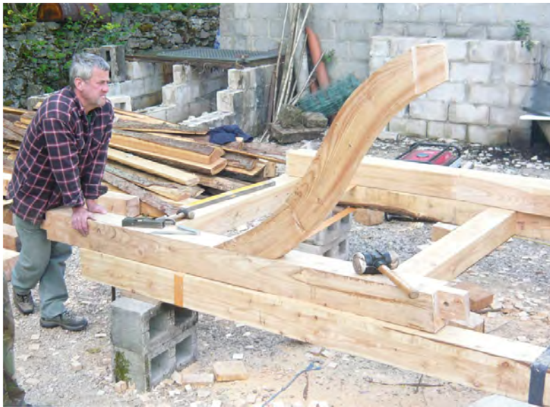
Fig. 7.37 Trying the curved brace for fit.
