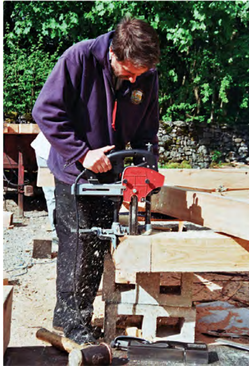
Fig. 7.32 Using an electric chain morticer.
