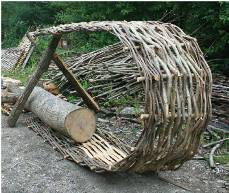
Fig. 6.23 Prop the archway so that it can be set in the right shape.
