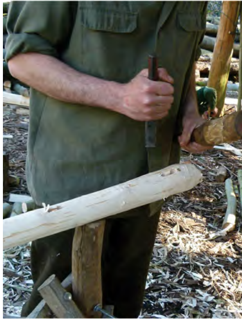
Fig. 8.8 Remove the waste wood from the mortice joints with a chisel and mallet.
