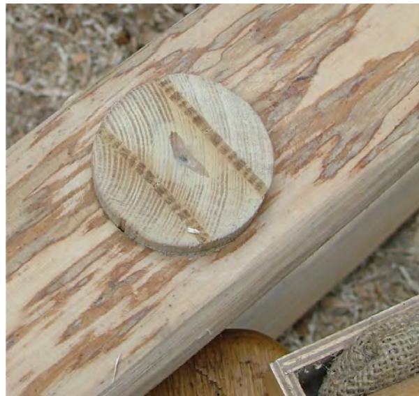
Fig. 6.26 The tenons with two oak wedges.
