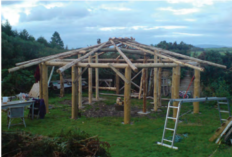
Fig. 7.27 A twelve pole construction with a reciprocal roof frame. (Photo: Phil Daube)
