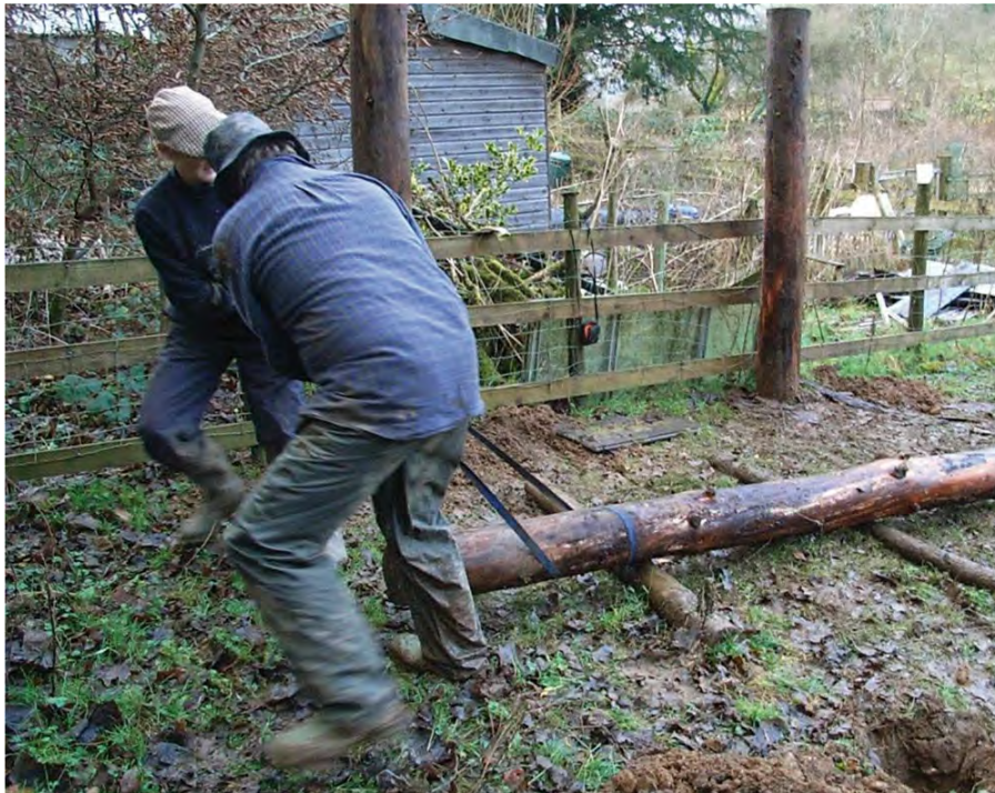
Fig. 7.7a The posts are pulled into position using time-honoured methods of rollers and ropes.
