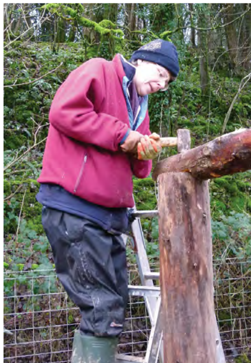
Fig. 7.11 Cut away the waste wood either with axe or chainsaw.
