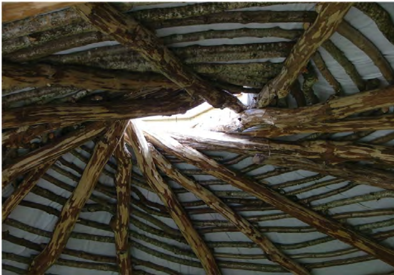
Fig. 7.29b Note the use of unpeeled hazel poles to support the membrane.
