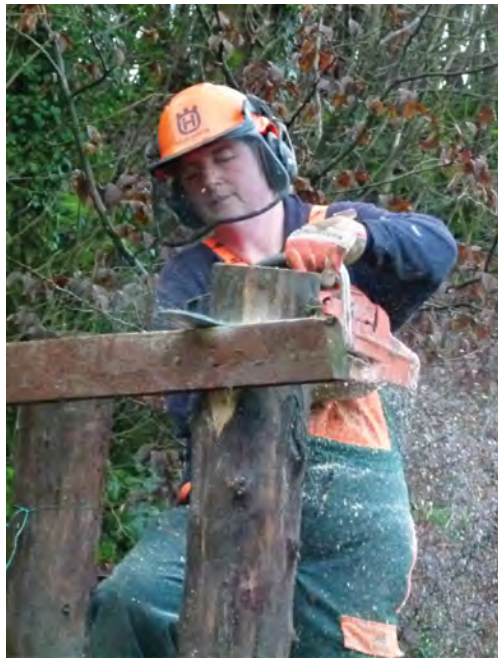
Fig. 7.9 Cutting the top of the post off at the correct angle.
