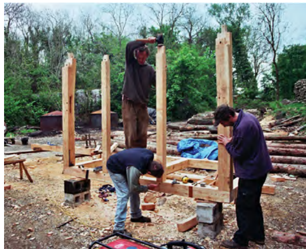
Fig. 7.35 Trying the frame wall posts.
