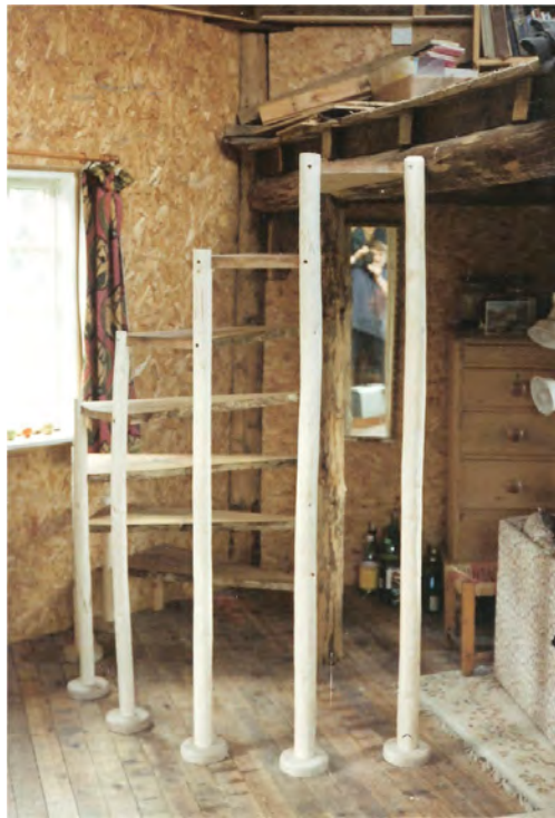
Fig. 7.25 The staircase was made of cleft ash and elm planks all sourced on site.
