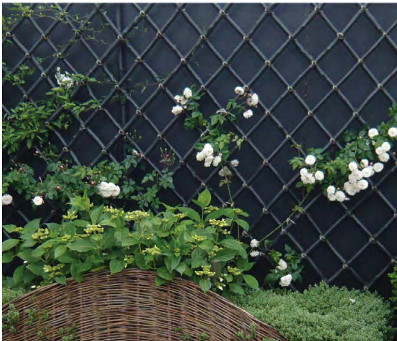
Fig. 6.1 Detail of hazel trellis, peeled and painted.
