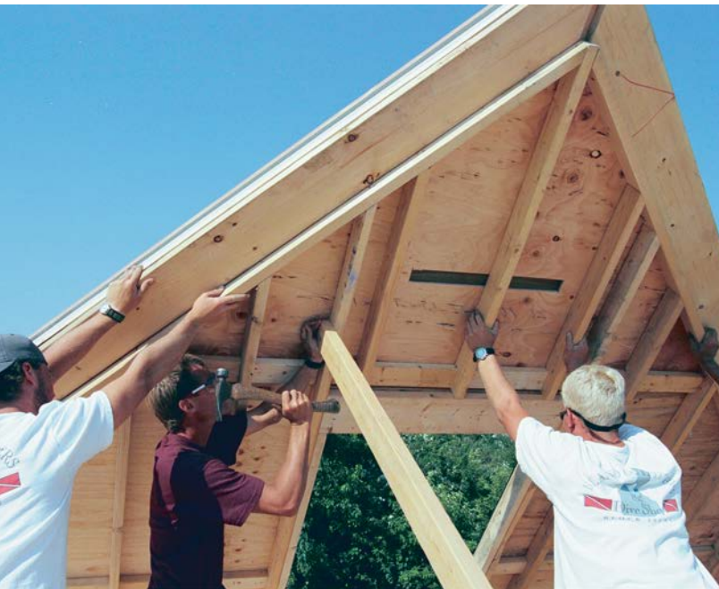
BRACES HELP WITH THE LIFT. With the wall held in place at about a 45-degree angle, 2× braces are nailed high up on the studs (above). The braces then help to control the final push (right) and finally are nailed to blocks attached to the floor framing.
