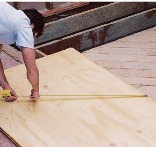
FIT THE BOTTOM PLATE. The plates are marked to be cut using a tape as a compass.
