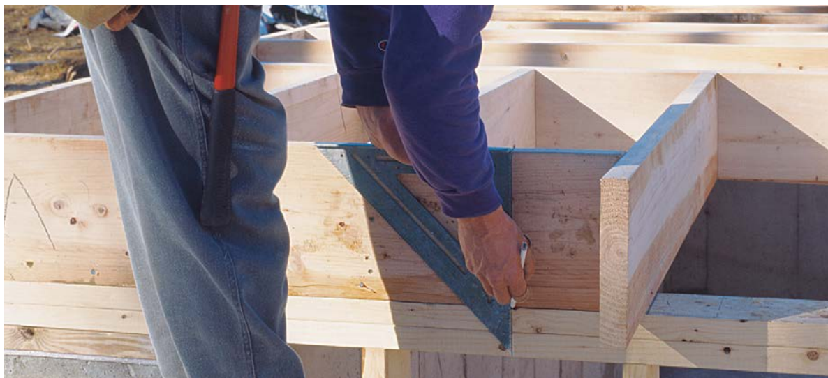
BAY STARTS HERE. After the bay joists are tacked in place, the outside edge of the bay is carried up from the face of the sill onto the rim joist.
