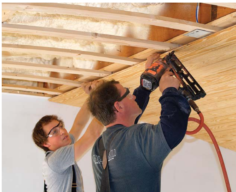
WOOD PANELING ADDS DETAIL. You can finish the ceiling with wood paneling or drywall.
