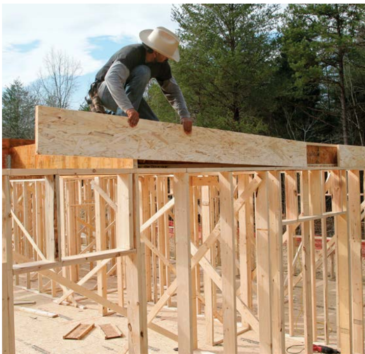
MOVE HEADERS INTO THE FLOOR FRAME. Window and door headers generally aren't needed in gable-end walls. Where headers are needed, the band joists (or engineered rim board) often can satisfy header requirements, as over these gable-wall windows.
