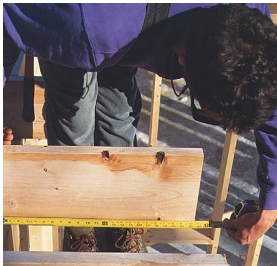
SETTING THE OVERHANG. With a 2-ft. cantilever, the longest joists overhang 22\frac{1}{2} in. The joists are then tacked in place.
