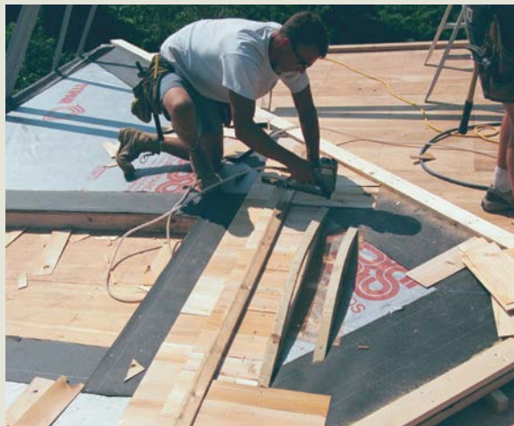
THE BOW IS FRAMED WITH 2×S. Beveled nailers are attached above and below the vent opening.
