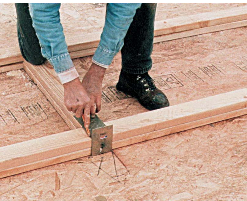
CHANNEL MARKER. This lightweight 3½-in.-wide tool enables carpenters to mark intersecting butt walls on all three sides of through walls with a pencil. A similar tool can be quickly site-built of plate scrap.
