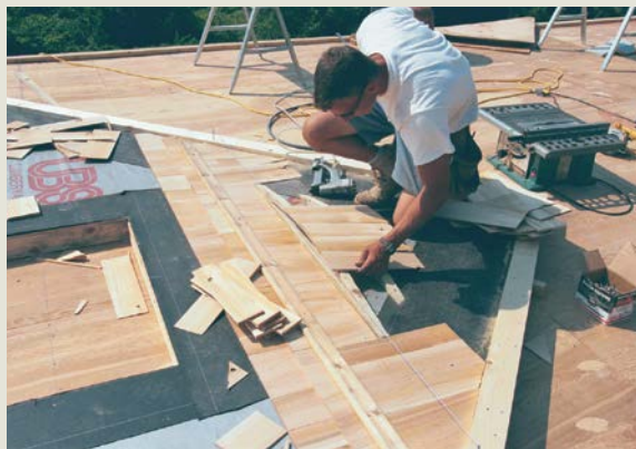
SHINGLES FOLLOW THE LINE OF THE BOW. Shingles are nailed to the nailers using a stretched string as a guide.
