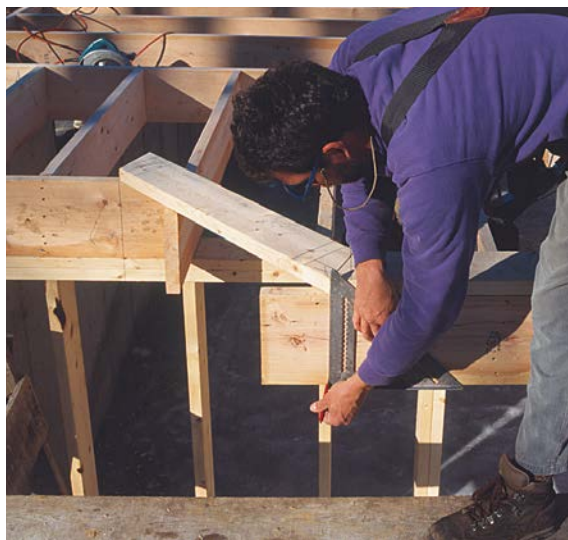
CUTLINES ARE SQUARED DOWN FROM THE PLATES. Lines are extended down from the corners of the plates for the rim-joist cuts, and the lengths of cantilevered side joists are marked 1½ in. from the outside edge of the plate.
