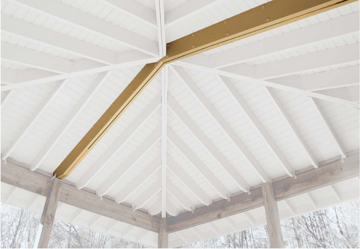
BOLTED BETWEEN RAFTERS , an angled steel flitch plate can eliminate the need for rafter ties in cathedral ceilings.
