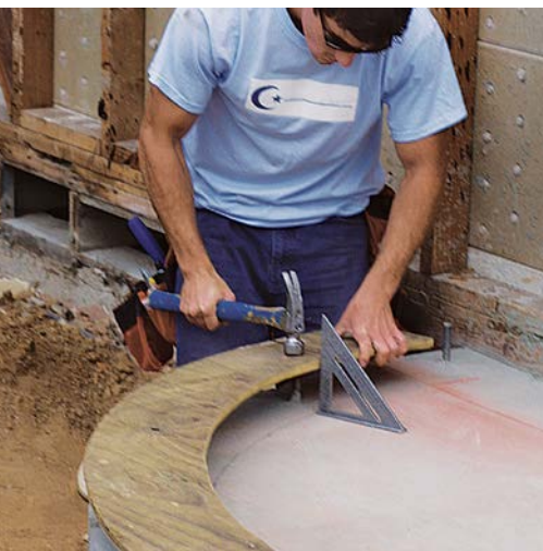
MARK FOR DRILLING. Using a square to ensure that the plate aligns with the layout line, the author taps the plate over the anchor bolts to mark the hole locations.
