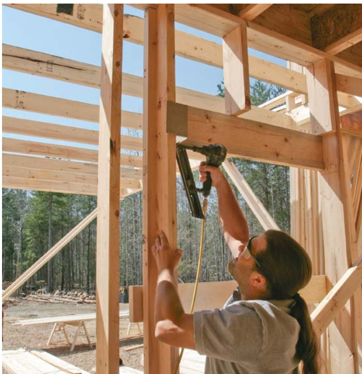
USE HEADER HANGERS. In areas where you need conventional headers, use steel header hangers to eliminate jack studs.
