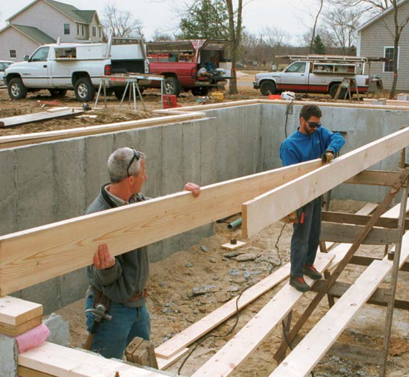
ALMOST A BEAM. The last board in the first layer completes the bridge between the foundation pockets. At this point, the first two layers are still only tacked together.
