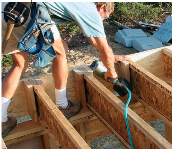
ATTACH SQUASH BLOCKS WHERE NEEDED
