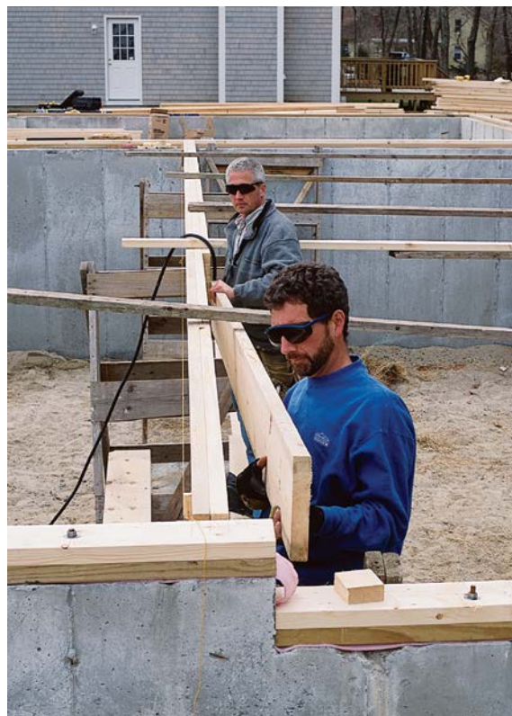
ONE PIECE AT A TIME. After the first two layers are braced straight and nailed off, each of the final layers is added one board at a time. After the entire layer is in place, the crew goes back and nails it off.
