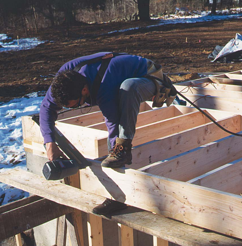
OUTER RIM JOIST IS LEFT LONG. Rim-joist stock is nailed to the cantilevered joists and left long until cutlines are transferred from the plates.
