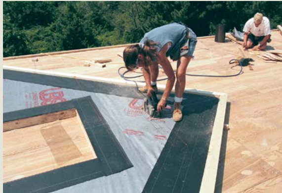
A HOLE FOR AIR BUT NOT WATER. A bow vent begins with a hole cut in the wall properly sized for the area to be vented.
