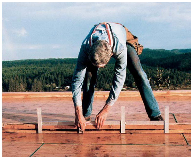
LAYOUT STICK. With tabs on 16-in. and 24-in. centers, a layout stick locates studs fast. The longer teeth come into play when plates are laid side by side and are marked on their faces rather than edges.
