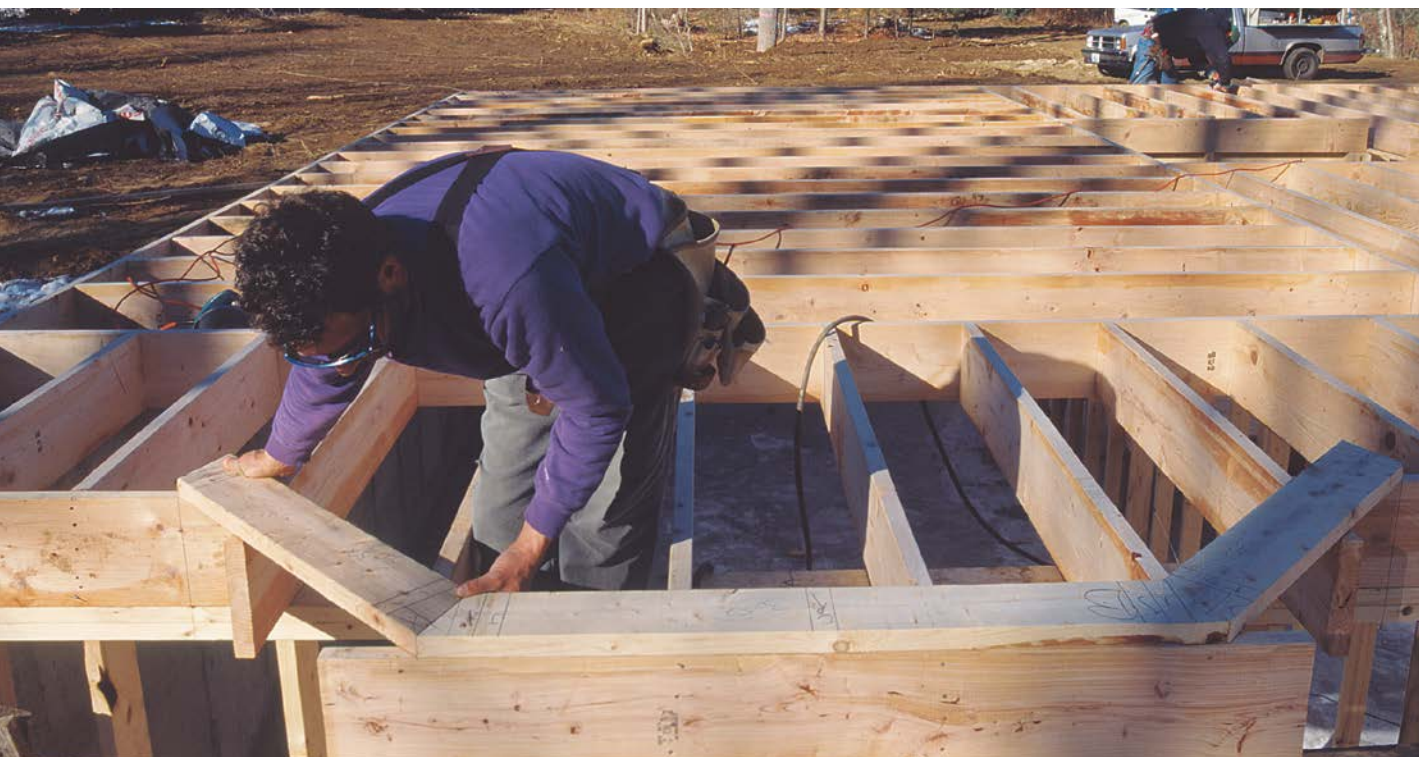
PRECUT WALL PLATES PROVIDE THE SHAPE OF THE BAY. The bay plates are laid on top of floor joists and rim joists that were run long and needed to be cut.
