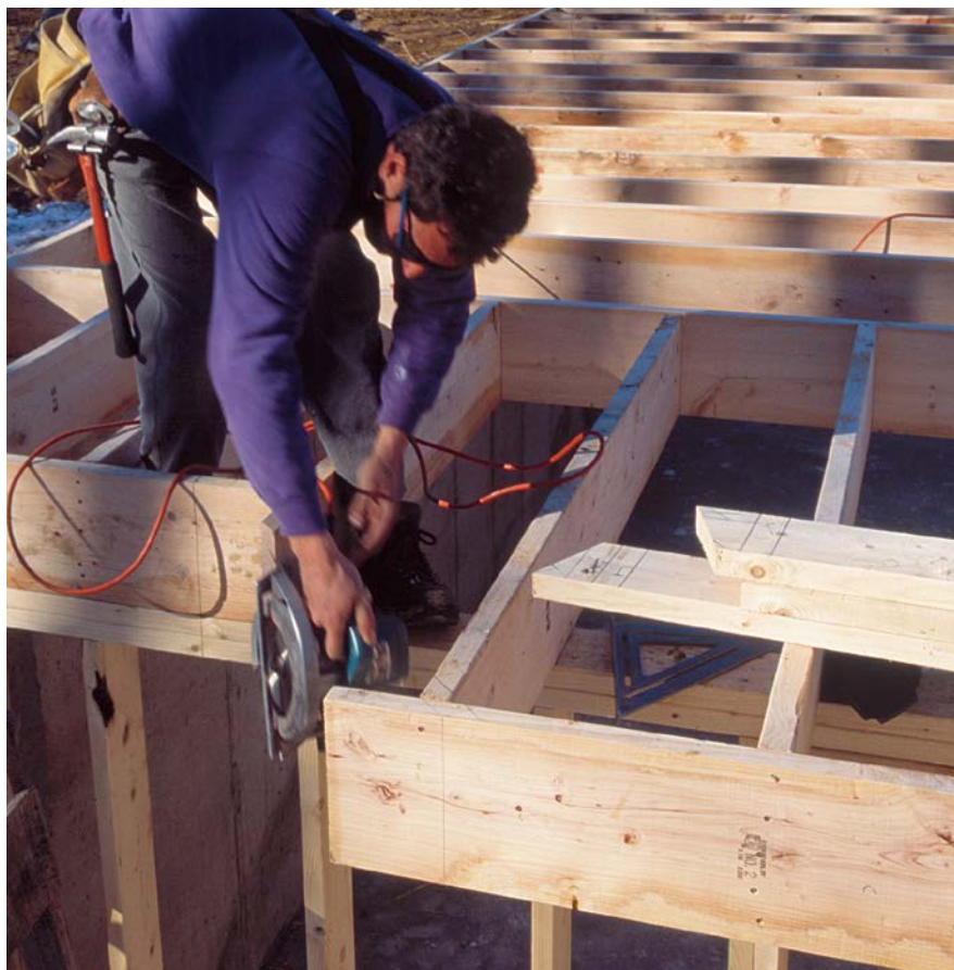
CUT DOWN WHERE THEY STAND. The cantilevered side joists and the outside rim joist are cut to length in place.
