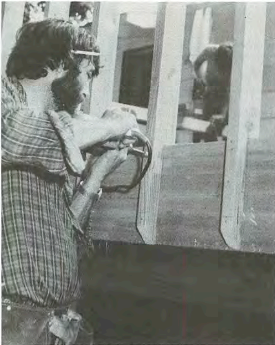
Fig. 1-3. Koppers Company's Wolmanized brand pressure-treated lumber being used to construct a deck.
