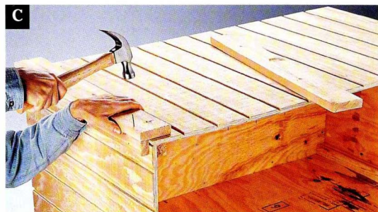
Attach the corner trim pieces flush with the edges of the corner battens to cover the plywood joints.
