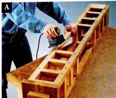
The tower for the windmill is basically two ladder frames joined by rails. Sand sharp edges smooth.
