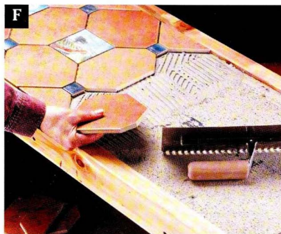
F Set the tile into the thin-set mortar, using a slight twisting motion.
