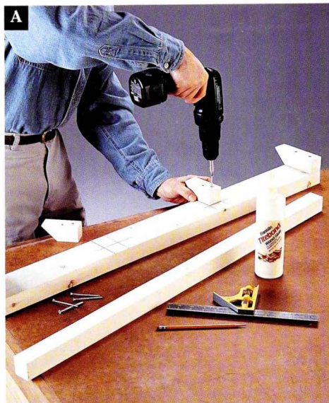
Use a combination square to mark the location of the center supports on the ledger, then attach with glue and screws.
