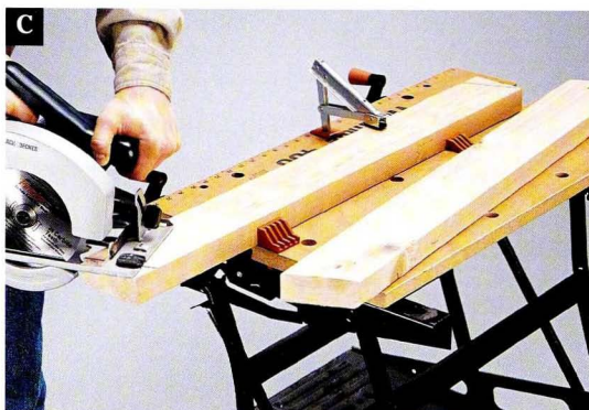
Miter-cut the middle supports and roof supports with a circular saw.
