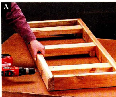
Use 1½" blocks to support the stretchers. Drill pilot holes and fasten the stretchers to the sides with 3" screws.
