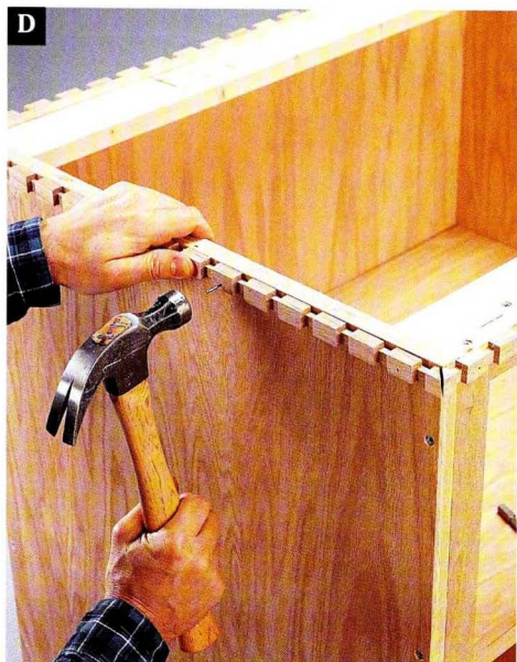
Fasten the dentil molding around the top edge of the cabinet with glue and brads.
