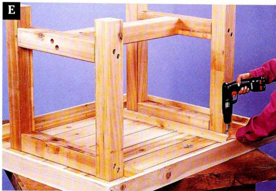
E Keep a firm grip on the tabletop slats when drilling deck screws through the cleats.
