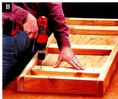
Position the frame over the plywood/cementboard core. Drill pilot holes and then drive 2" galvanized deck screws through the stretchers and into the plywood.
