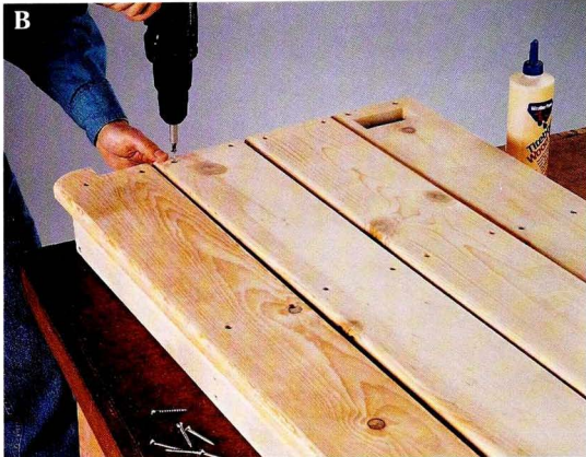
Attach the seat slats and nose slat to the top of the seat frame with glue and deck screws.
