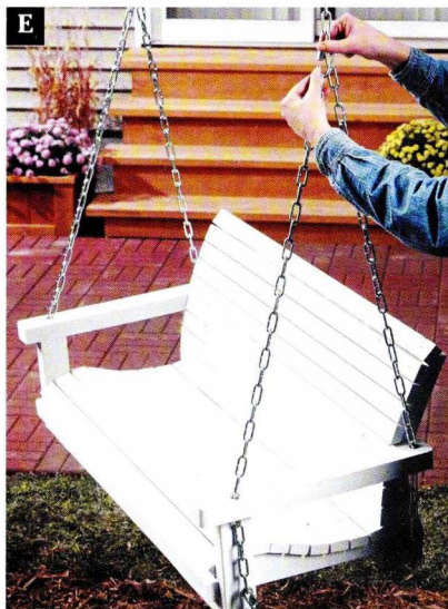
Suspend the swing and adjust the chain length and the position of the connectors until the swing balances.
