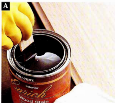
Prepare for the stain, then stir the stain thoroughly and apply a heavy coat with a brush or cloth. Stir the stain often as you work. Let the stain soak in for about 15 minutes (see manufacturer's directions).
