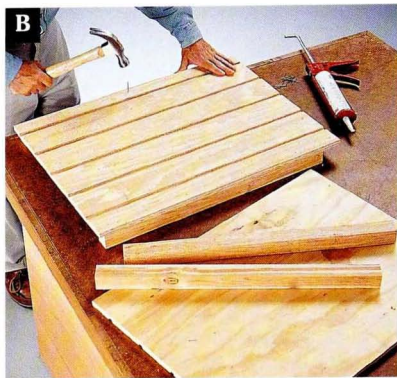
Position the corner braces beneath the small panels, and fasten them with adhesive and finish nails.
