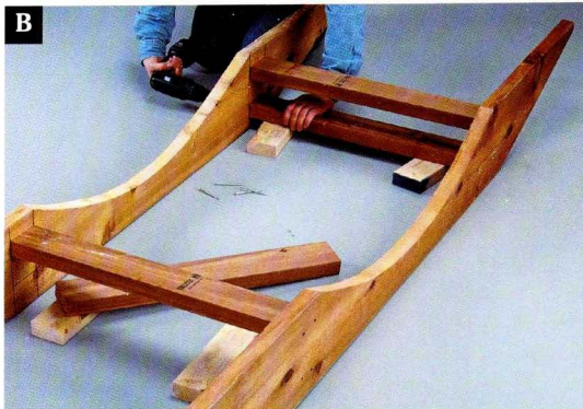
Attach pairs of stretchers between the stringers with 3" deck screws.
