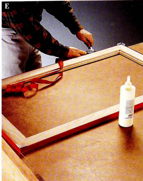
E Glue the miters of the top frame together, using a band clamp. Check for square by measuring diagonals.
