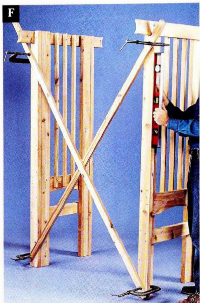
F Use long pieces of 1 × 4 to brace the side frames in an upright, level position while you attach the top beams.
