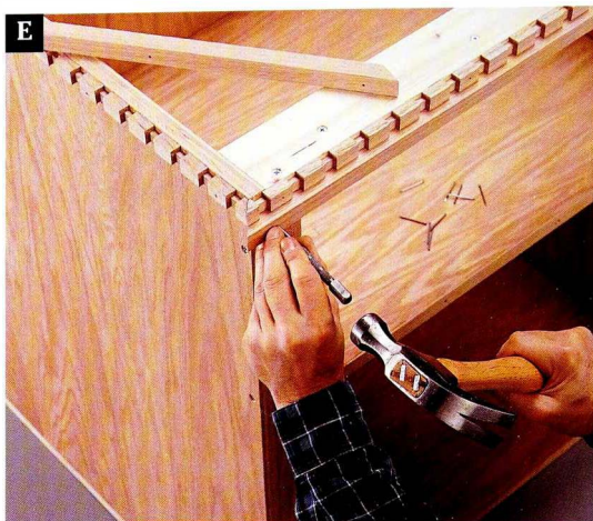
Attach the lower trim underneath the dentil molding, and set the nails with a nail set.
