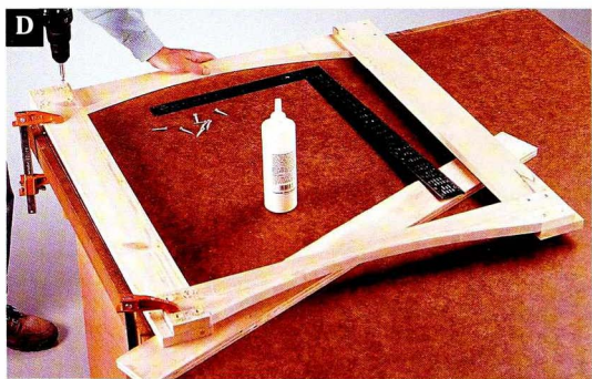
Assemble the arched front rails and the stiles into face frames.
