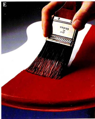
For a smooth surface free from lap marks, hold your paint brush at a 45° angle, and apply just enough pressure to flex the bristles slightly.
