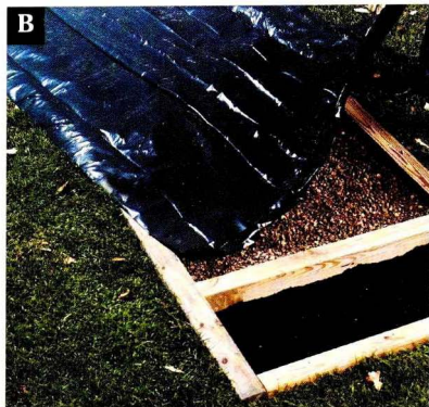
B Lay the first row of timbers, including the wall for the storage box. Fill the sandbox area with a 2" layer of gravel and cover with plastic sheathing.
