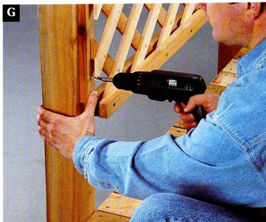
G Fasten 1 x 2 filler strips to the posts to close the gaps at the sides of the lattice panels.
