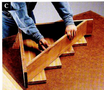
Lay the bin frame on the bottom boards and trace along the back inside edge to mark cutting lines.
