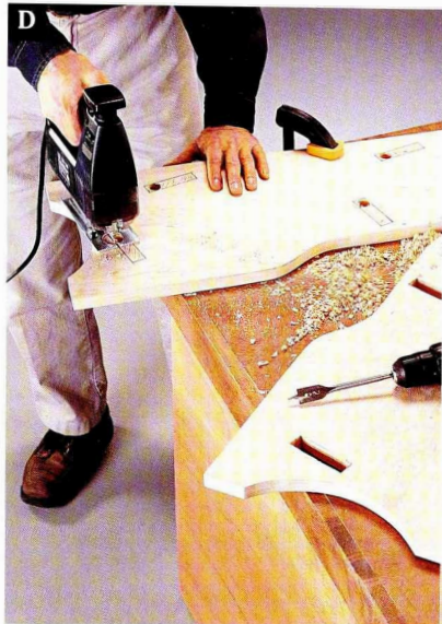
Drill pilot holes, using a backer board to prevent splintering, and cut the mortises with a jig saw.
