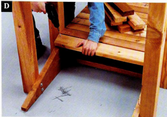
Attach the treads to the stringers with deck screws.
