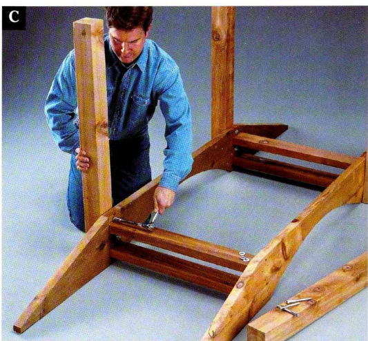
Cut the 4 x 4 posts to their finished height, then use lag screws to attach them to the outsides of the stringers.
