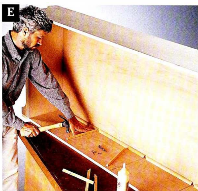
E Attach the shelf cleats with glue and brads.
