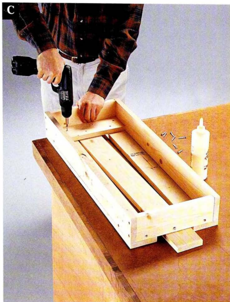
C Join the fixed-shelf slats to the stretchers with glue and \frac{1}{4} " screws driven through the undersides of the stretchers.
