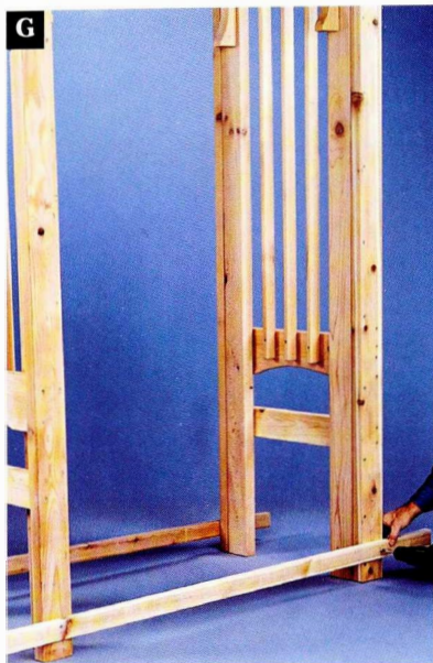
G Lock the legs in a square position after assembling the arbor by tacking strips of wood between the front legs and between the back legs.
