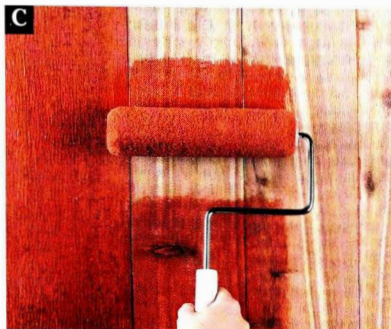
C Rough-sawn or textured woods can be stained with a \frac{3}{4} " nap roller. Cover one section at a time and roll back from dry to wet to prevent uneven color distribution.
