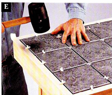
Tap the tiles lightly with a rubber mallet to set them firmly in the adhesive.
