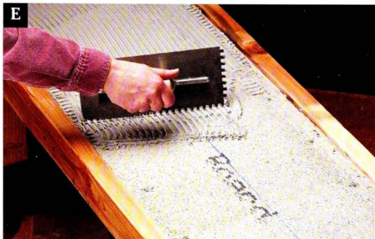
E Apply thin-set mortar over the cementboard, using a notched trowel.
