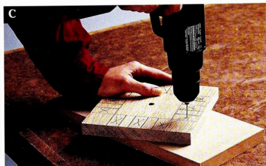
C Drill pilot holes through the plates for finish nails.
