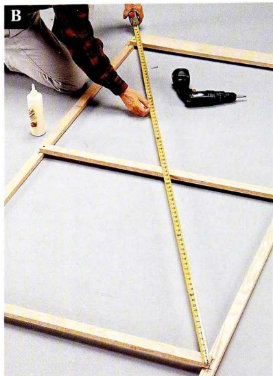
Measure the diagonals to check for square. If the measurements are equal, the frame is square.
