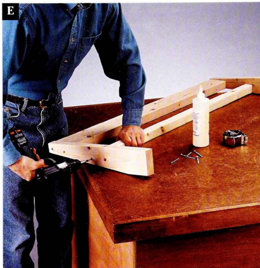
Glue the ends of the top and bottom rails, then drive deck screws through the posts to attach them to the rails.
