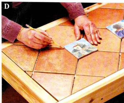
D Dry-fit the field tiles, using spacers. Set the accent tile in place and mark the field tile for cutting.
