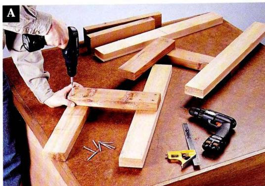
Seat rails are attached to the short posts and inside posts to make the bench frames.
