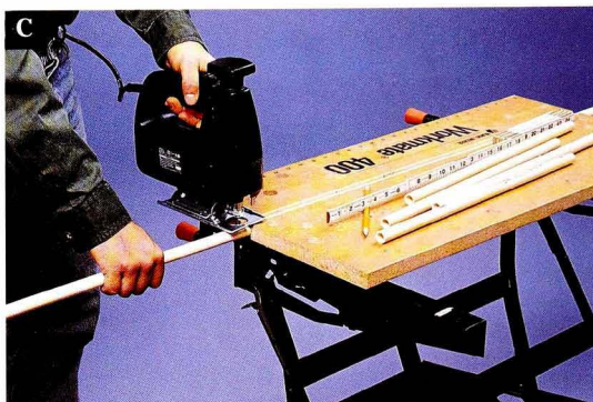
Use a jig saw to cut the CPVC tubing slats. For stability, arrange the tubing so the saw blade is very close to the work surface.
