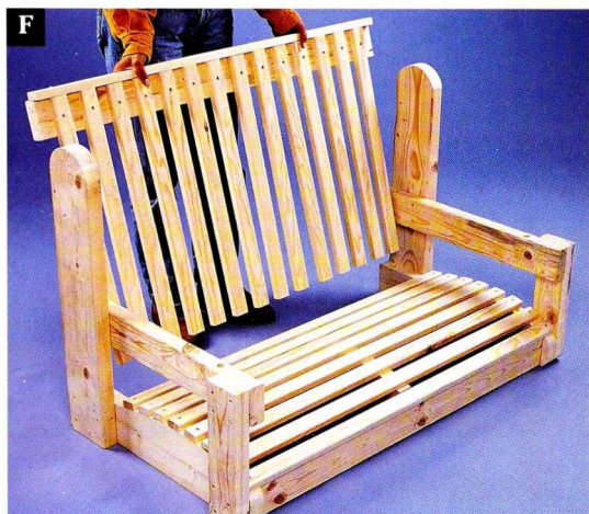
Slide the back assembly against the seat assembly and attach.
