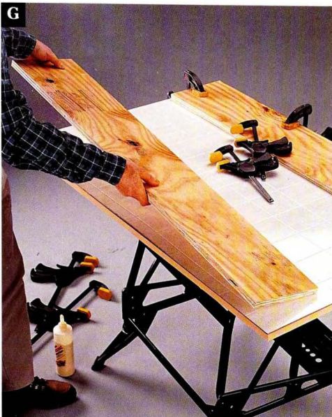
G Clamp scrap boards to the tileboard to distribute pressure and establish good contact.
