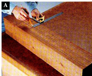
Lay out three \frac{1}{2} "-wide flutes on each column face using a combination square as a marking gauge.
