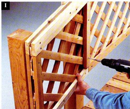
I Use deck screws to attach a trim strip over each joint between the end panels and center panels.
