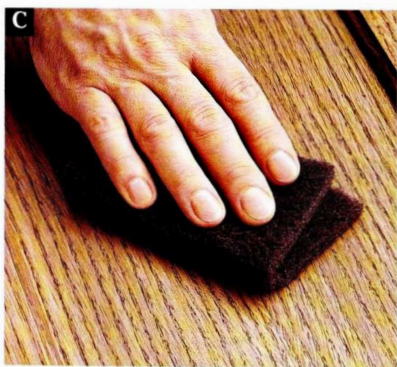
Apply light coats of stain until the desired color tone is achieved, buffing with an abrasive pad between coats. Buff the final coat of stain before top-coating.
