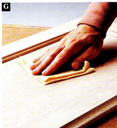
G Wipe the wood surface clean, using a cloth slightly dampened with mineral spirits.
