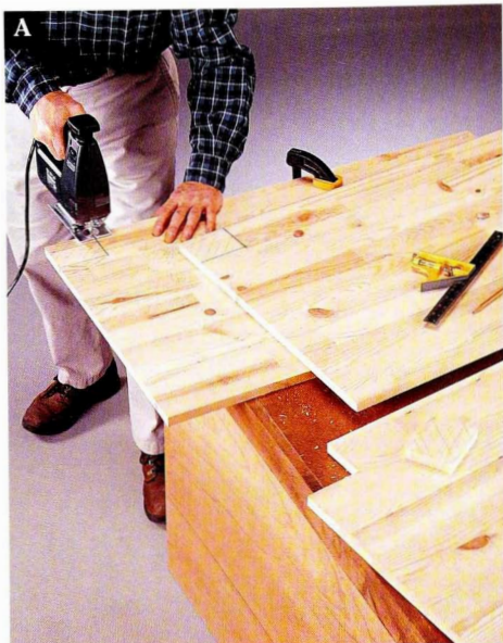
A Cut the toe board notches into the ends and divider using a jig saw.
