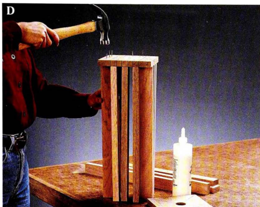
Attach the slats to the top plate with glue and 6d finish nails.
