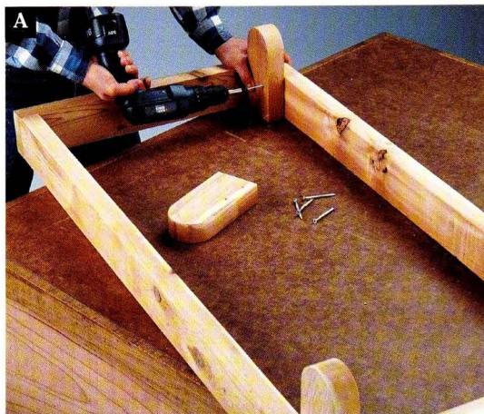
Fasten the 2 x 4 cedar feet to the inside frame corners with 3" galvanized deck screws.
