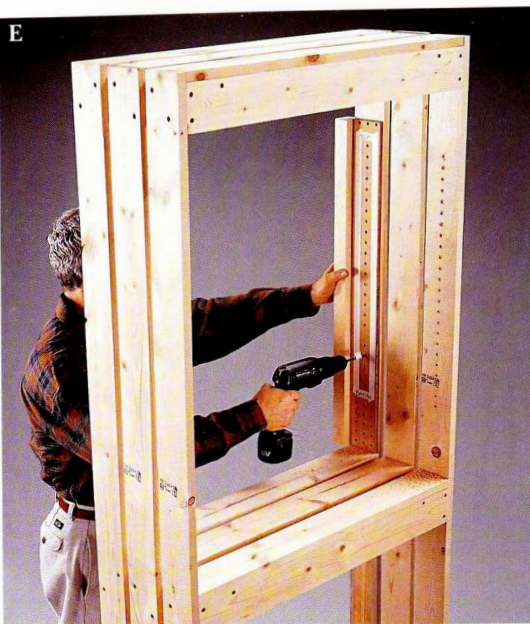
Use a pegboard template for uniform placement of peg holes.
