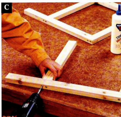
Once the final cap has been attached with deck screws and glue, the basic tray frame is complete.
