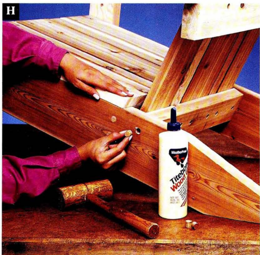
Glue cedar plugs into the counterbores to conceal the screw holes.
