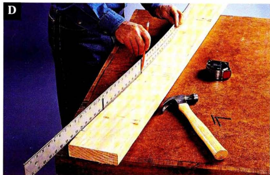
Use a flexible ruler pinned between casing nails to trace a smooth arch onto the aprons.
