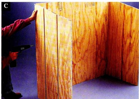
C Attach the end panels to the back panel, keeping the back panel flush with the back edges of the end panels.
