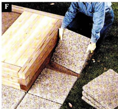
Place the pavers into the sand base. Use a rubber mallet to set them in place.
