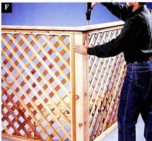
F Attach the long and short caps to the tops of the trellis frames. The long cap overlaps the long rail and the post.
