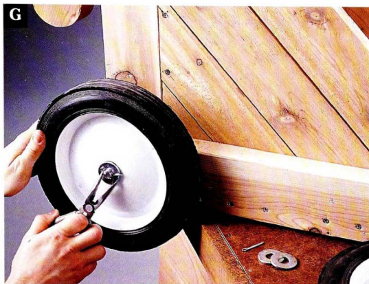
Secure the wheels by inserting a cotter pin into a hole at the end of each axle, then bending the ends of the pin down with pliers.
