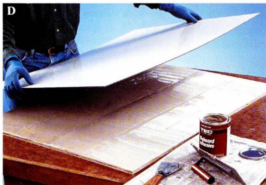
D Bond tileboard to the plywood tabletop with tileboard adhesive.
