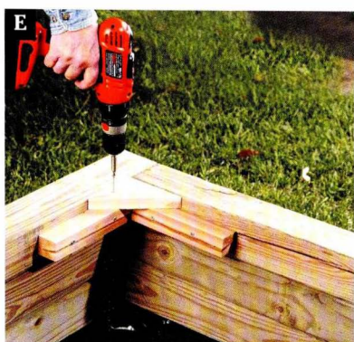
E Install 2 × 2 support cleats ¼" from the top of the sandbox. Attach the corner bench boards using galvanized screws.
