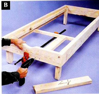
Assemble the frame pieces and legs, then add the support boards for the slats and backrest.
