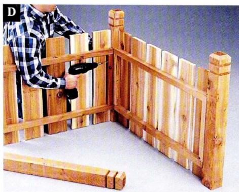
Stand the posts and panels upright, and fasten the panels to the posts by driving screws through the cleats.
