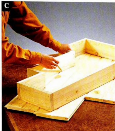
Trace the shape of the frame onto beaded siding and cut it to fit.
