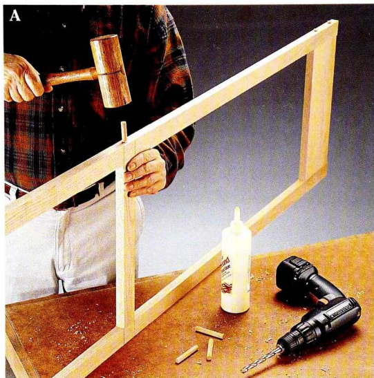
Use a wood mallet to pound \frac{3}{4} " glued oak dowels into the end frame.
