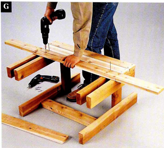
The longer face boards attached to the tall benches overhang the doubled posts so they cover the sides of the short bench frames when the tree surround is assembled.
