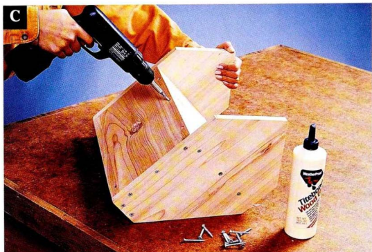
Attach the box bottom to the back with glue and screws driven through the back and sides.
