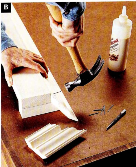
Attach the front crown and side crown to the bottom and supports with glue and 4d finish nails.
