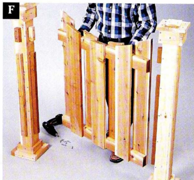
Set the completed fence panels between the cleats on the faces of the posts.
