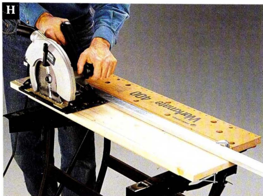
H Use a circular saw with a straightedge as a guide to rip-cut the door boards to size.
