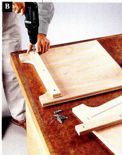
Center the end cleats over the kick spaces, leaving 3/4" at each end where the side cleats will fit.
