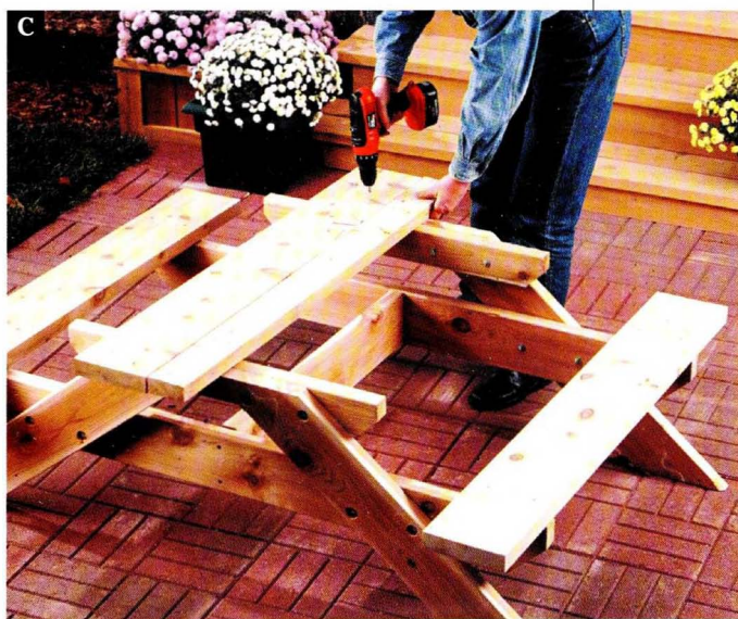
Install the table top boards by drilling pilot holes and inserting deck screws.
