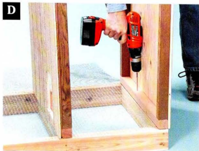
Attach the frames to the floor crosspieces.
