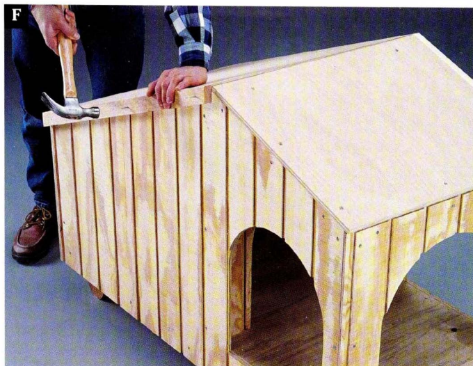
Cut each side roof trim piece to fit between the peak and the end of the roof panel, mitering the ends so they will be perpendicular when installed. Attach all the roof trim pieces with galvanized finish nails.
