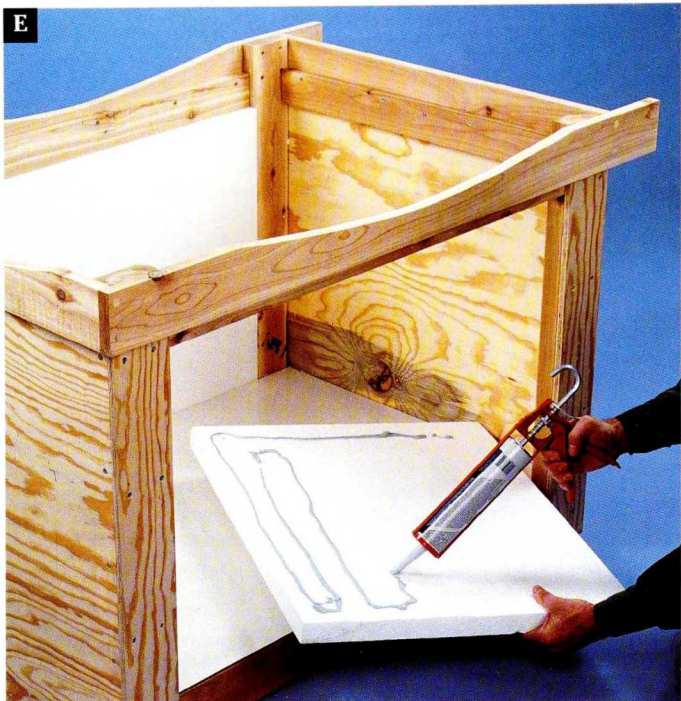
Use panel adhesive to install rigid foam insulation on the interior walls of the cooler compartment.
