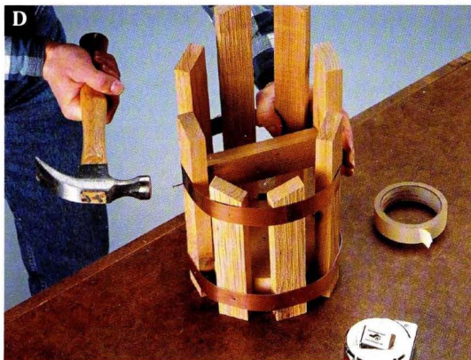
Brace the slats with a spacer as you tack on the copper straps.
