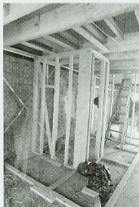
Interior walls are easy if floor and ceiling are flat and parallel.
