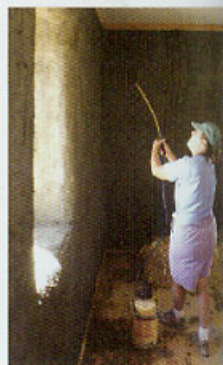
A water sprayer facilitates an even curing process.
