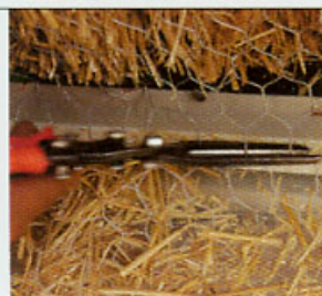
Trimming lath within the weep screed
