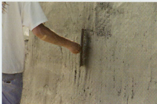
Scratched wet stucco provides a base for a brown coat.
