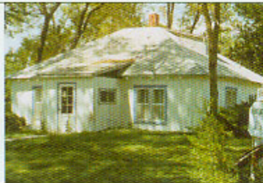
The Martin/Monhart House, Arthur, Nebraska, built c. 1925: Still in fine shape after over seventy-five years, this bale house features a useable attic space consisting of two small upstairs rooms.
