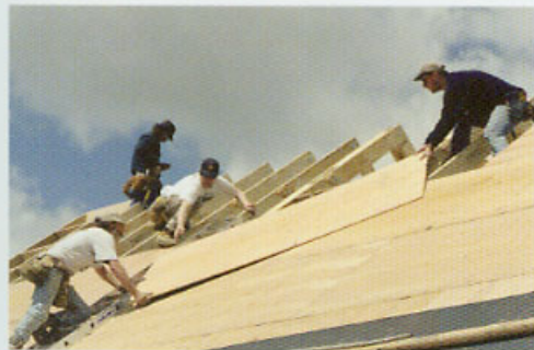
Sheathe trusses with plywood, but stagger the sheets to provide a strong roof surface.
