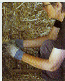
Use loose straw to fill the gaps.
