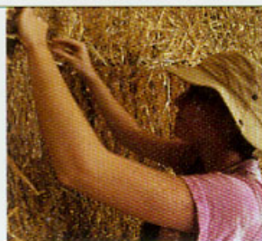
Cover flat portions of bale walls inside and out with standard chicken wire.
