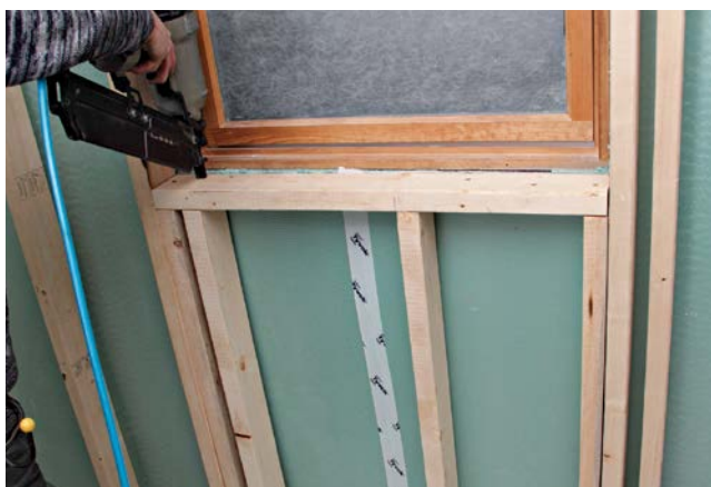
6a Install the horizontals . . .
