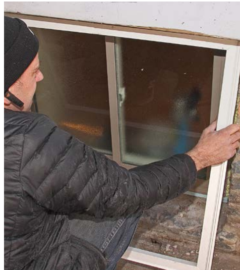
7 Slip the assembly in place and fasten.
