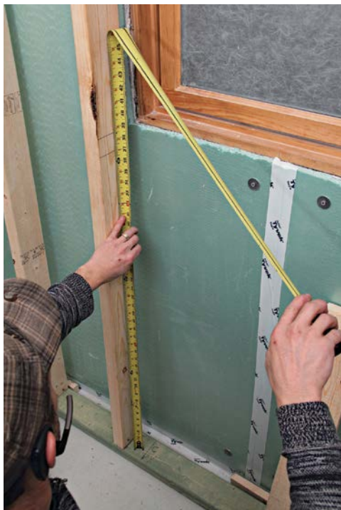
5 Measure for the bottom and top horizontals.
