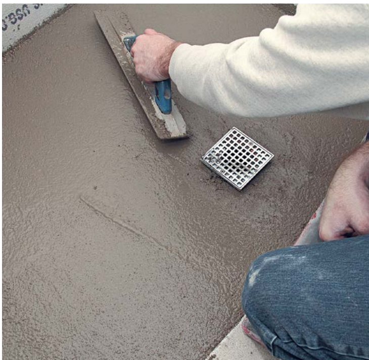
9 Smooth the concrete, checking again for slope. It should be below the drain cover by the thickness of the tiles plus \frac{1}{8} in. for mortar.
