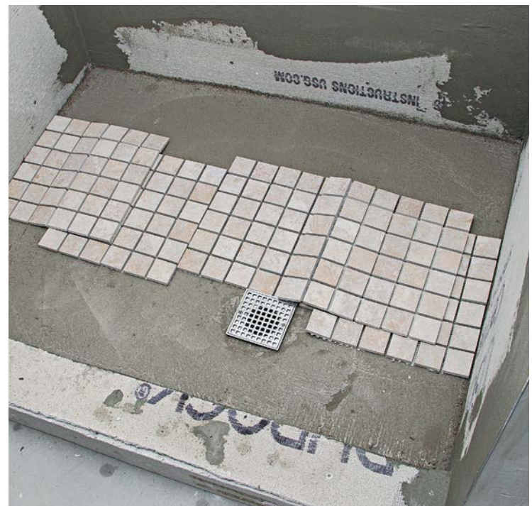
10 Allow the concrete to set, and lay out for the tiles.
