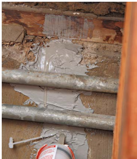
9 Repeat until liquid seeps out the top of the crack.
