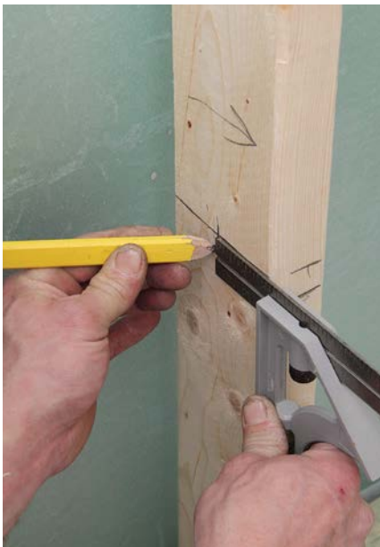
7 Mark the centers of the studs.
