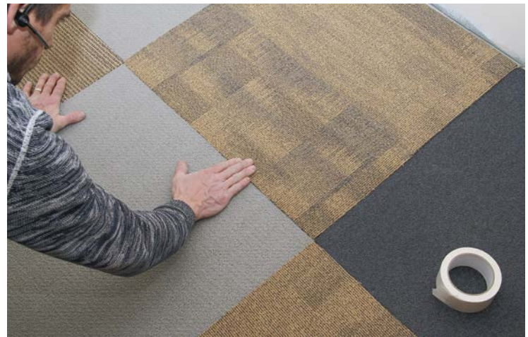
6 Once you are sure of the fit, press the tiles down to fasten securely to the floor.
