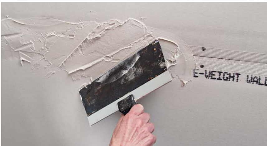
2 Fill a tapered joint with a good amount of compound.
