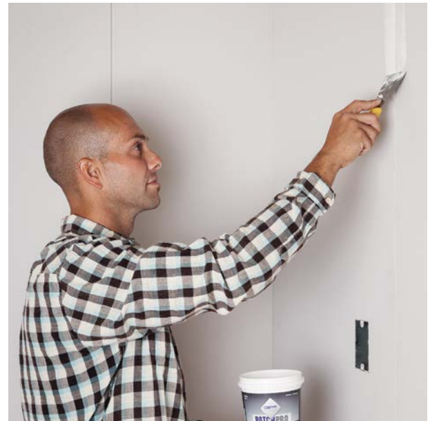
8 Apply a coat of patching compound and allow to dry; sand lightly and repeat with a second coat.
