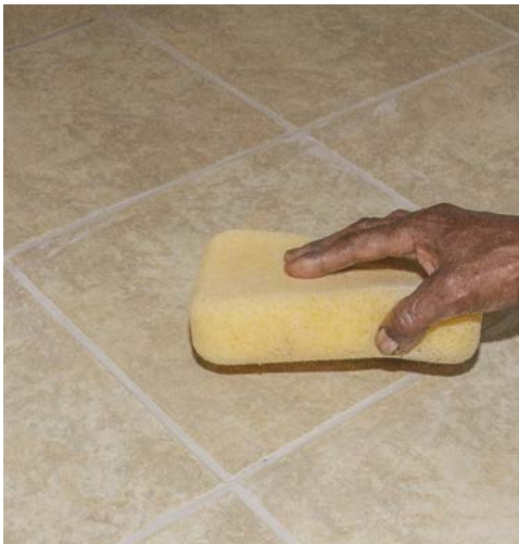
13a Gently wipe the tile surface clean of grout . . .
