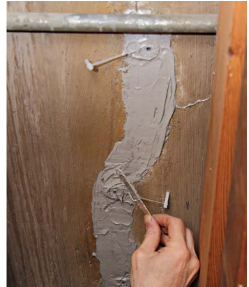
5 Apply epoxy all along the crack.
