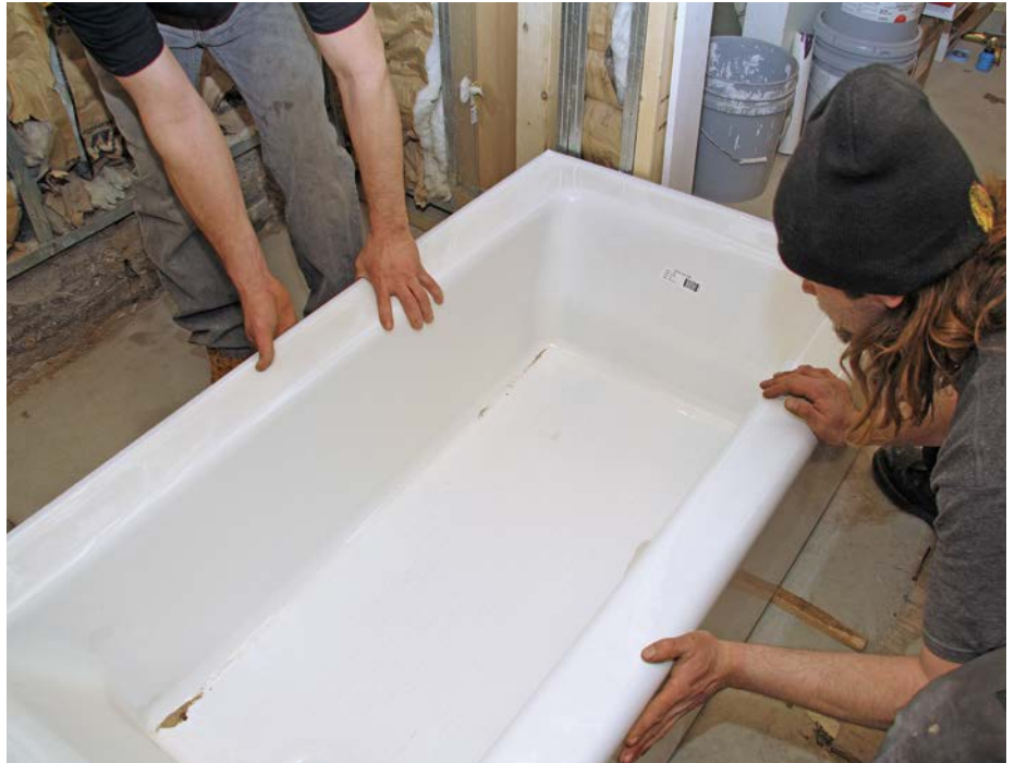
4b . . . and slide and/or tilt it into position.
