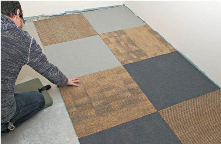
2 Arrange the tiles in a pattern if you like. Be sure seams fit snugly together.
