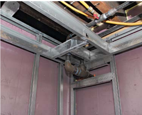
An opening is framed for an access panel to get at a shutoff valve.
