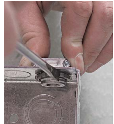
E Tighten the nut by pushing or tapping a screwdriver.
