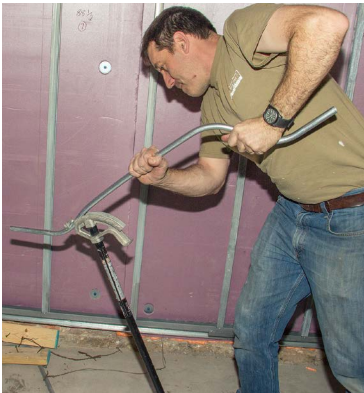
2 Multiple bends are sometimes easier to make with the bender positioned upside down.
