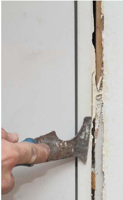
2 Scrape away any protrusions on the wall or jamb.
