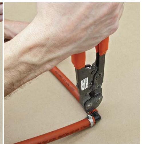
5 Place the clamp tool's end over the fitting wings and tighten all the way.
