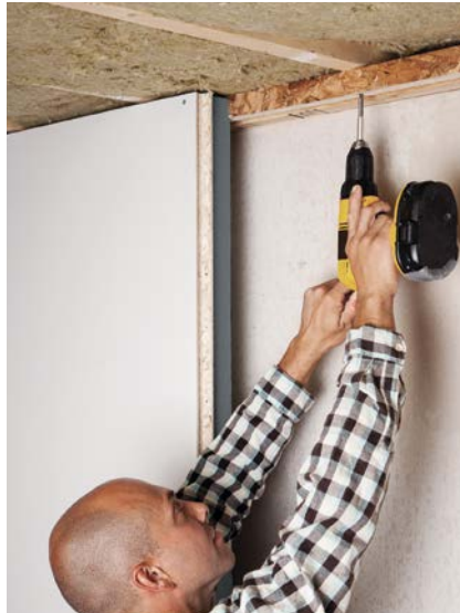
1 Attach the top track to hold the panels away from the wall.
