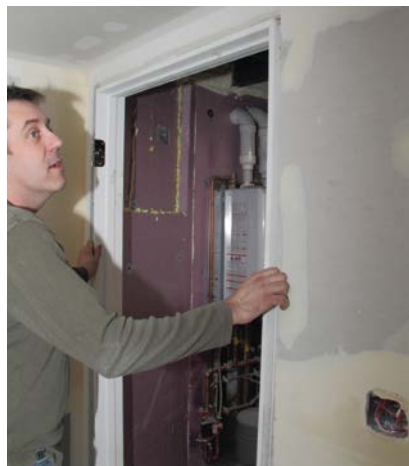
6 Carry and insert the jamb assembly into the framed opening.
