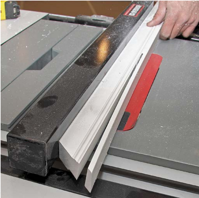
4 If the masonry sill is angled, rip-cut the bottom trim piece to follow the slope.
