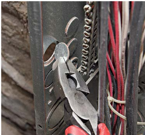
1 Shut off power at the main breaker. Remove a knockout slug at a convenient place.
