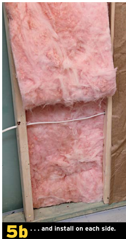
3 Press the insulation in place between studs, maintaining the fluff.
