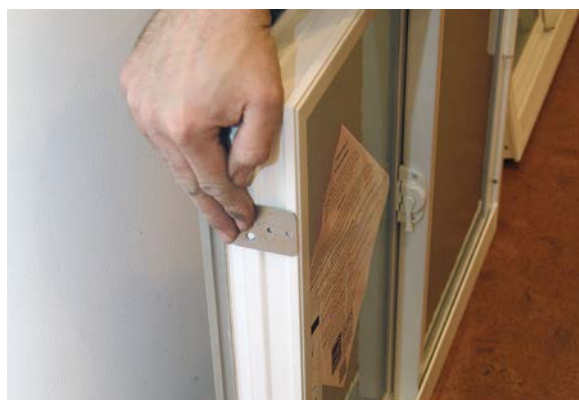
Some windows have special clips that provide extra rigidity. They should be inserted so that you will drive the mounting screws through them.
