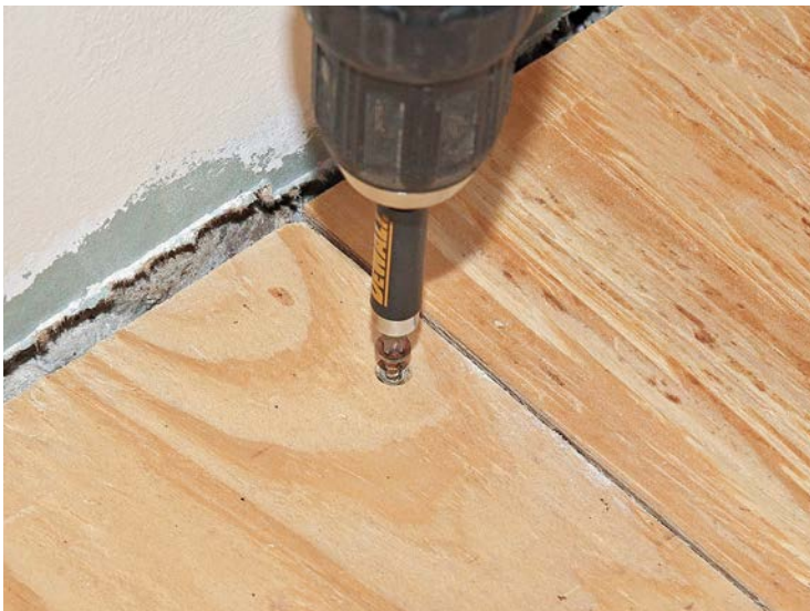
Drive occasional short screws to keep the sheets from separating.
