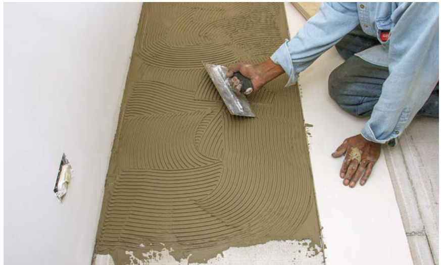
4 Use the notched side of the trowel to comb the thinset to a smooth surface.
