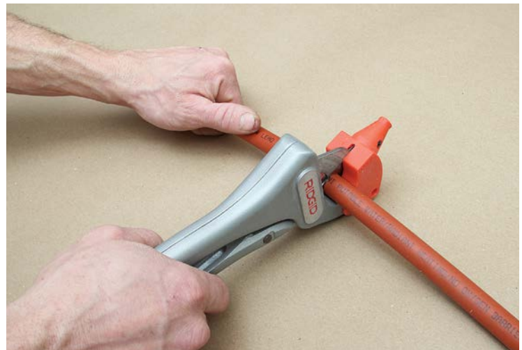
2 Make a clean, straight cut using a PEX or tubing cutter.
