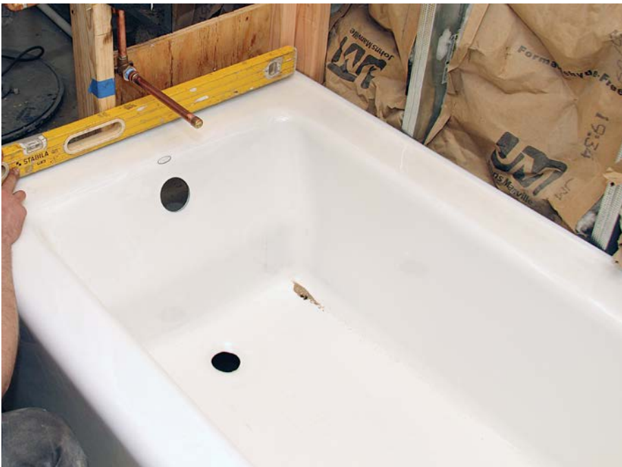
5 See that the tub is level in both directions.
