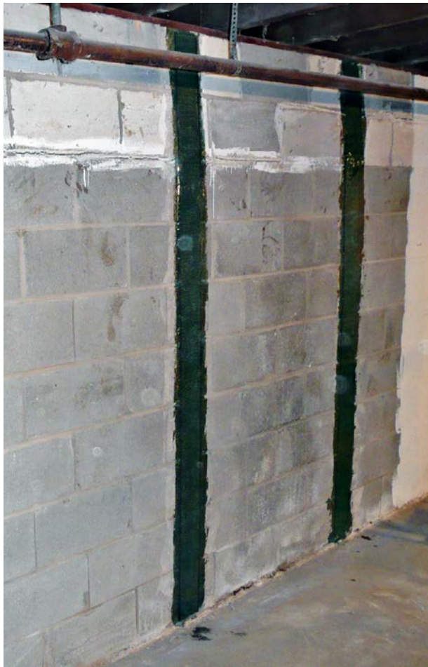
A carbon strap won't fix a bowed wall, but it will stop the wall from continuing to bow. The strap—and bowed wall—can be hidden behind drywall.
