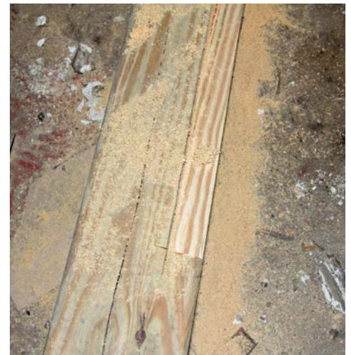
2 Often a beam needs to be notched in order to fit.
