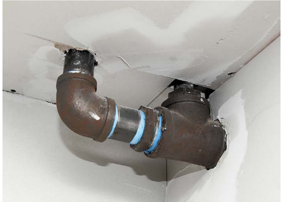
At tricky spots like this, you will need to improvise and perhaps use small pieces. Use construction adhesive where you cannot drive screws.
