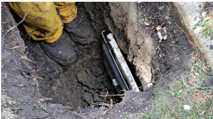
3 These plates are wide enough to stay still while the wall is pulled back into position.
