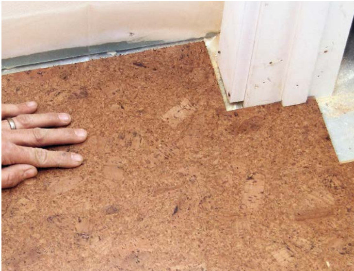
11 At a doorway, undercut the stop and casing molding, and cut the plank to fit neatly around the jamb.
