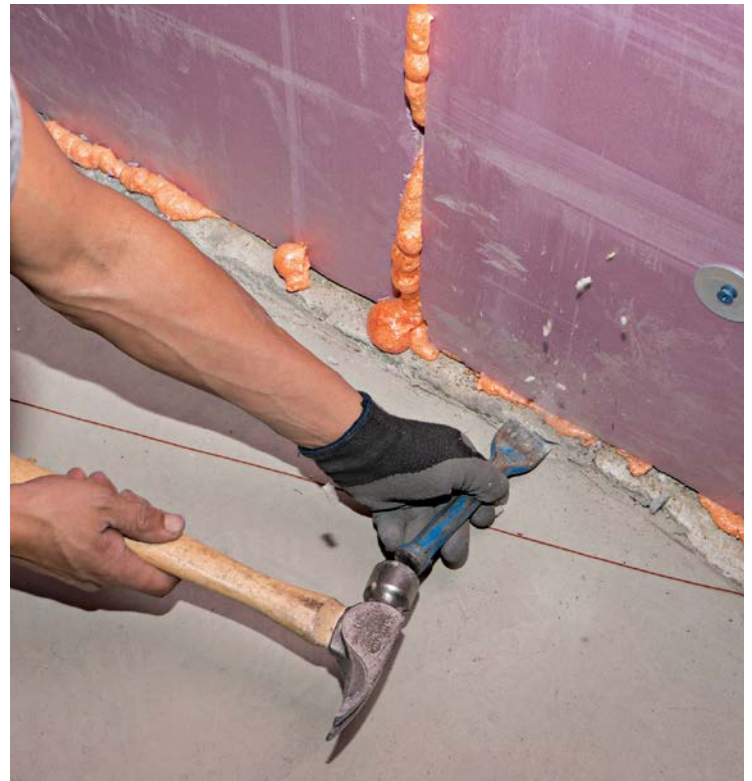
6 Chip away any obstructions that may get in the way of framing.
