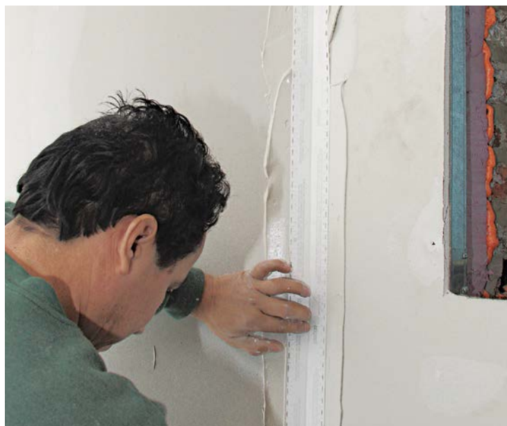
4 Gently press the tape and form a straight line.
