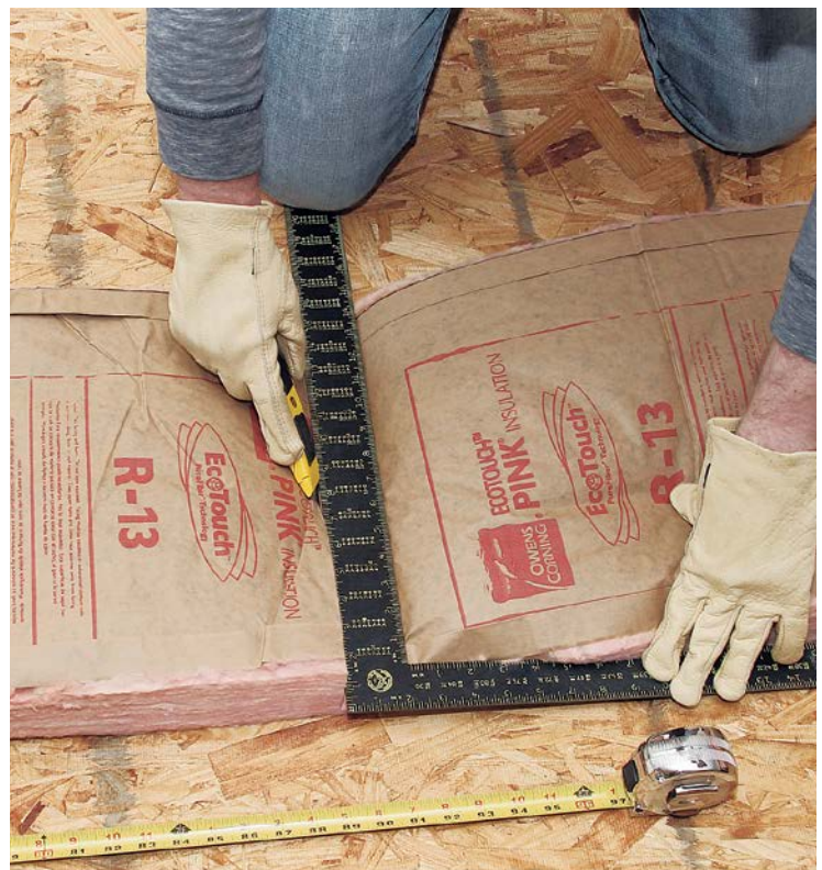
2 Compress the insulation and make a square cut.
