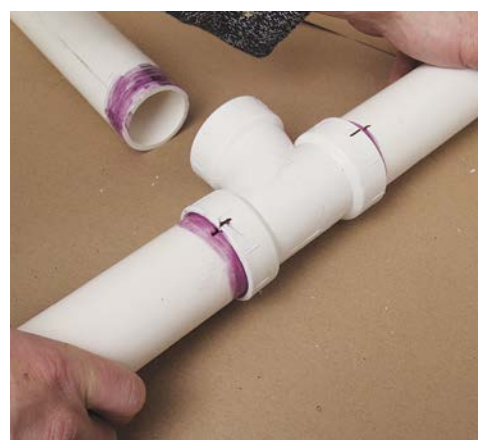
6 Push the pipe into the fitting, twist slightly, and hold still for a count of ten.
