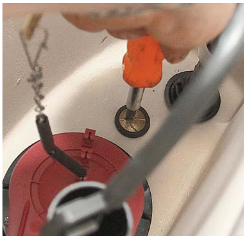
5b From inside the tank, hold the bolt still as you tighten the nut from below.
