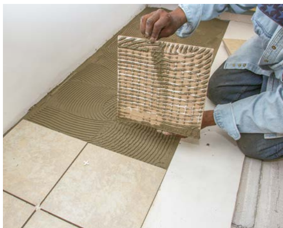
7 Periodically check the back sides to be sure tiles bed in the mortar.
