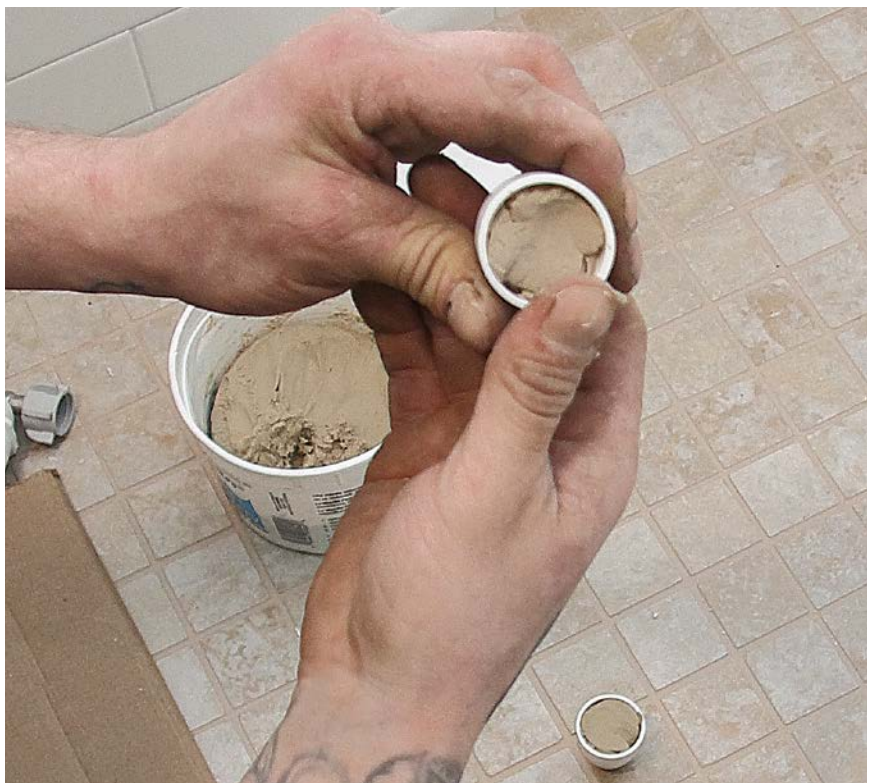
10 Fill the plastic caps with putty and snap them over the mounting bolts.
