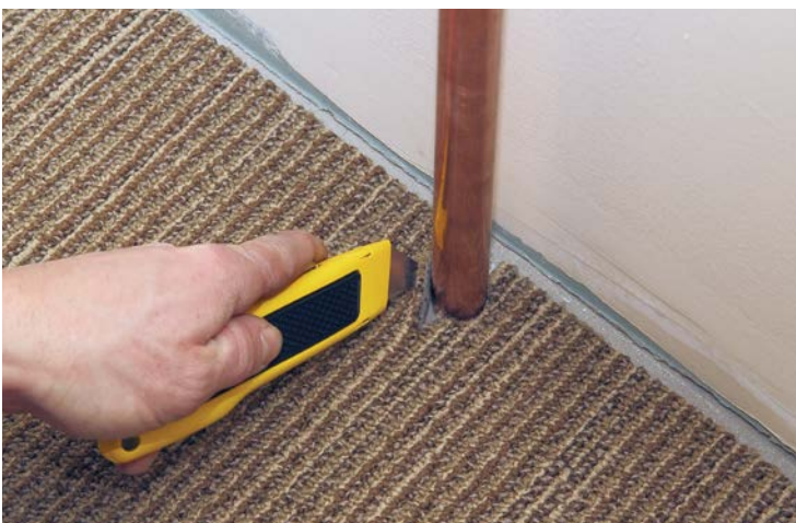
8 Position the tile and cut around the pipe with a utility knife.
