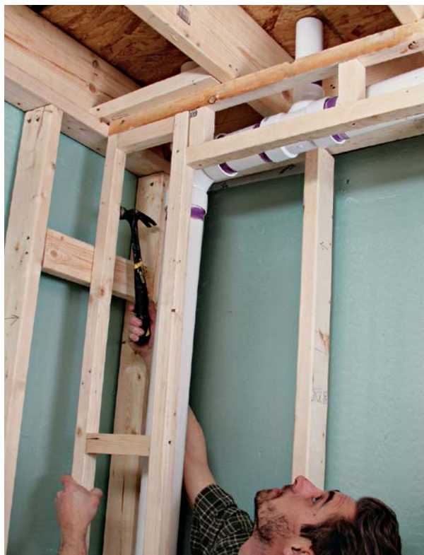
6 Tap in and attach one of the chase frames.
