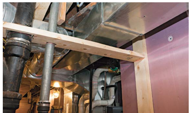
The laser line can be seen on the wall, the side stud, and pipes.
