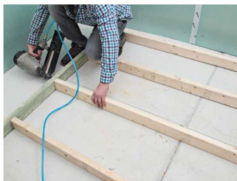
4 Fasten the studs to the plates, keeping them carefully aligned.
