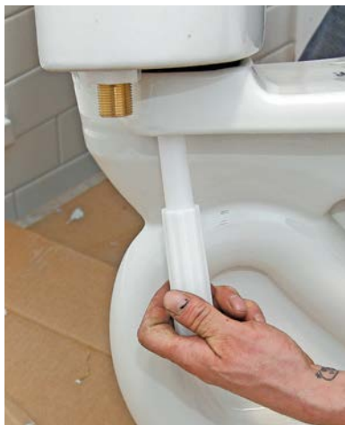
5a Mount the tank onto the bowl by tightening mounting nuts.
