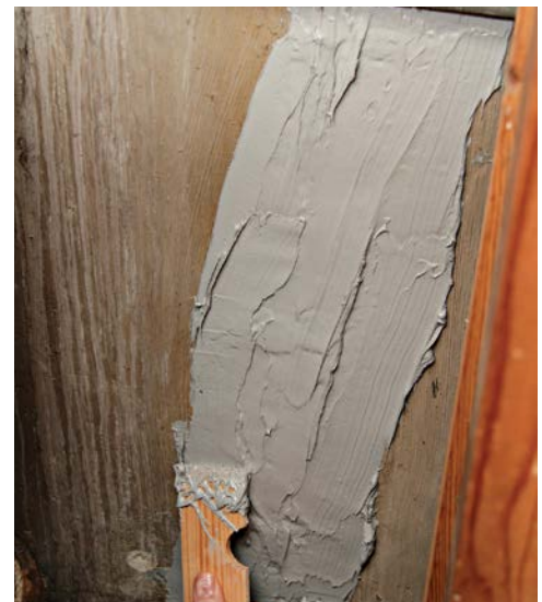
10 Snip off the port caps and smooth over the entire crack with additional paste.
