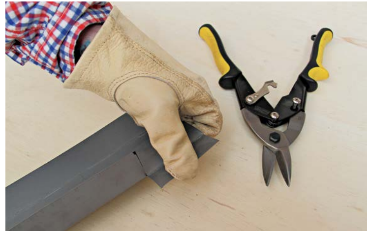
5b . . . for the other channel to fit over.
