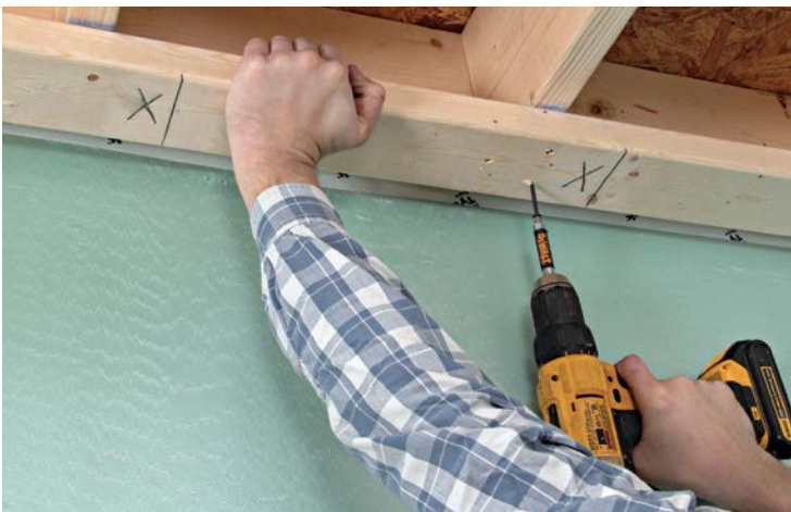
5 After attaching the bottom plate with powder-actuated nails or masonry screws, screw the top plate to the framing.
