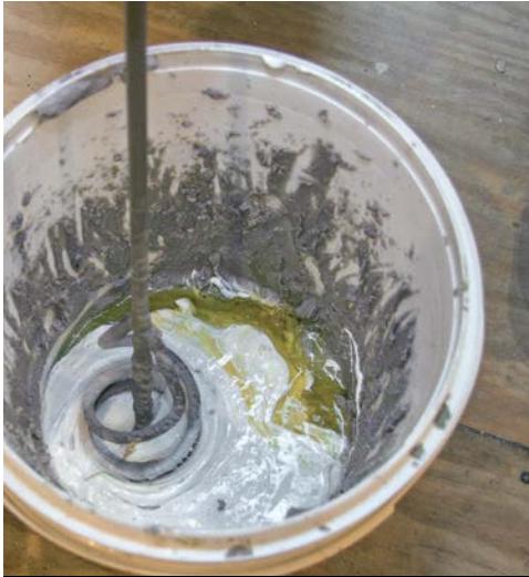
10 Mix a batch of epoxy grout according to the manufacturer's directions.
