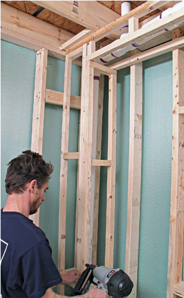
7 Attach the first chase frame, then build and attach another chase frame.
