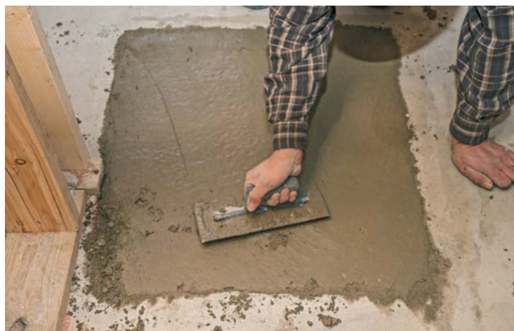
4 Smooth the patch with a magnesium float, then a steel trowel.
