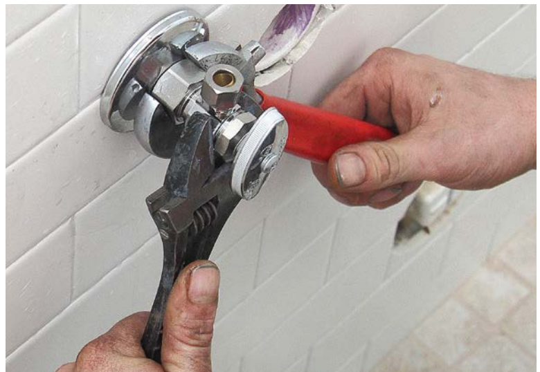
3 Hold the valve still and tighten the compression nut.
