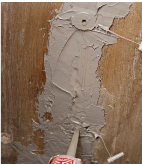
8 Once liquid starts to flow out the next-highest port, cap the bottom port and squirt into the next-highest one.
