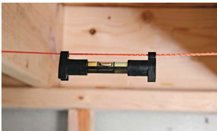
A line level lets you know when an individual mason's line is level.
