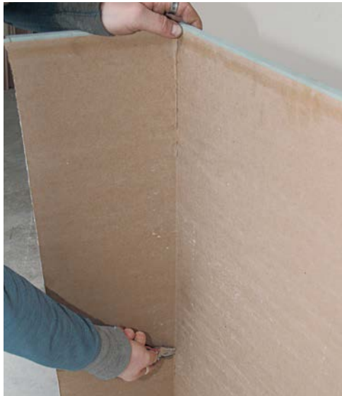
4 Slice through the paper on the back of the sheet to complete the cut.
