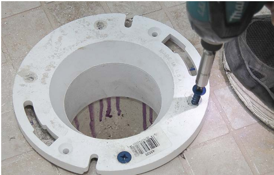
3 Drill pilot holes and drive masonry screws to anchor the flange to the floor.
