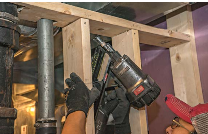
7 Attach studs with toenails or angle-driven screws.
