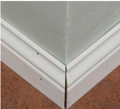
4 Test outside corner cuts with scrap pieces and adjust the saw if needed.
