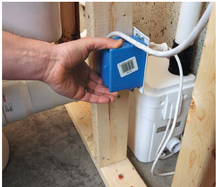
5 Install a new 15-amp circuit and hook it to a GFCI receptacle.
