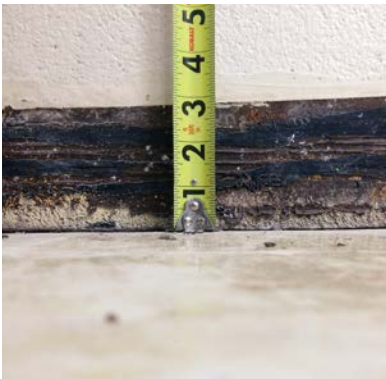
A floor that is 1 1/2 in. below the bottom of the wall (left) has sunk and needs to be raised and reinforced. After raising the foundation with a foundation pier and supporting it by pumping in concrete, as shown on p. 46, the floor is brought up to meet the wall and will not sink any farther (right).
