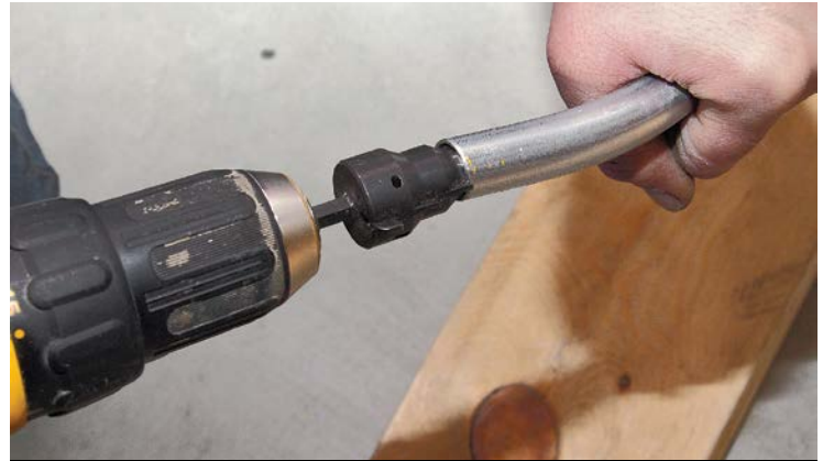
5 Be sure to remove all burrs with a reaming tool.
