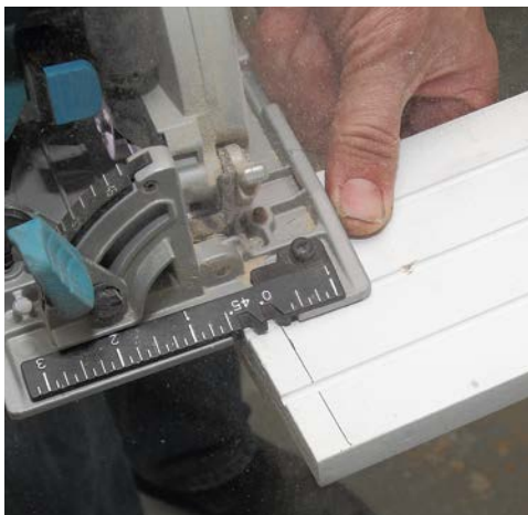
5 Cut side jambs as needed.
