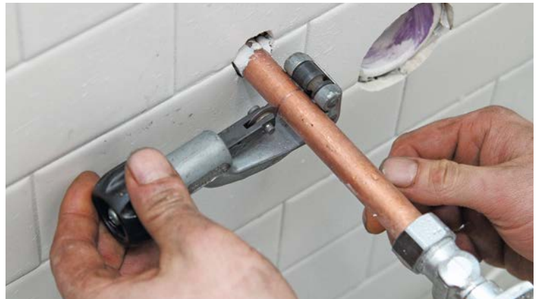
2 Cut the pipes with a tubing cutter.
