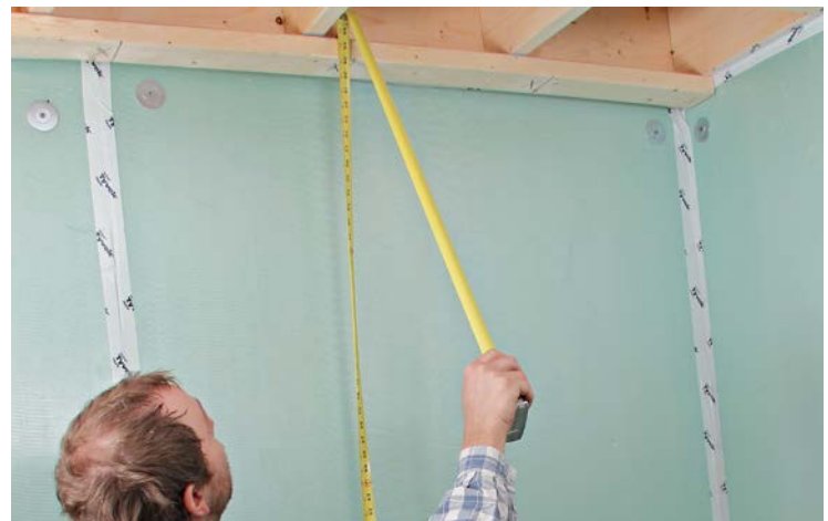
6 Measure for cutting each stud individually.
