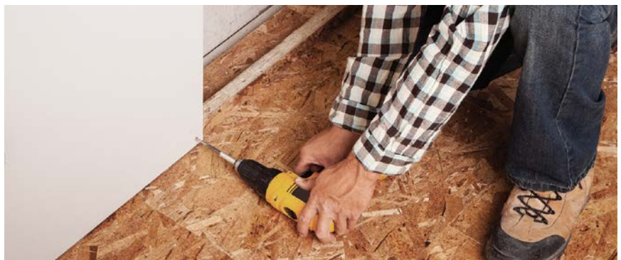
3 Attach the panel with screws driven into the top and bottom tracks.
