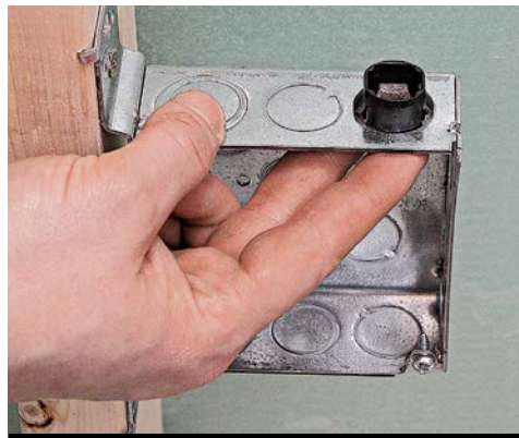
G Push or tap a plastic clamp up through a knockout hole.
