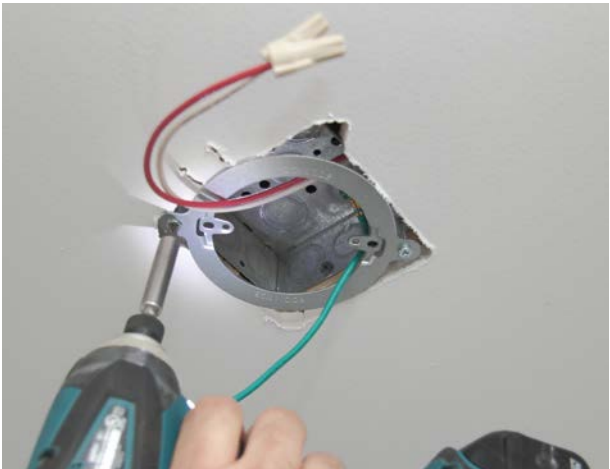
2 Attach the mounting strap.
