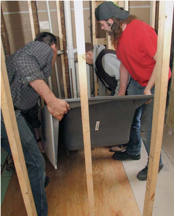
4a Wrestle the tub into the room . . .
