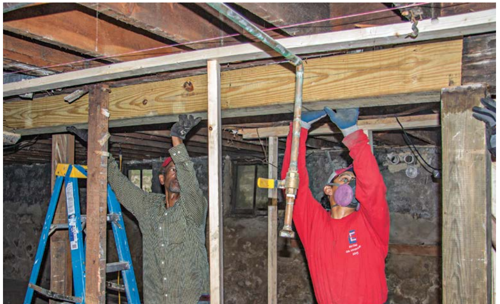
3 After setting in the beam, attach securely with angle-driven screws.
