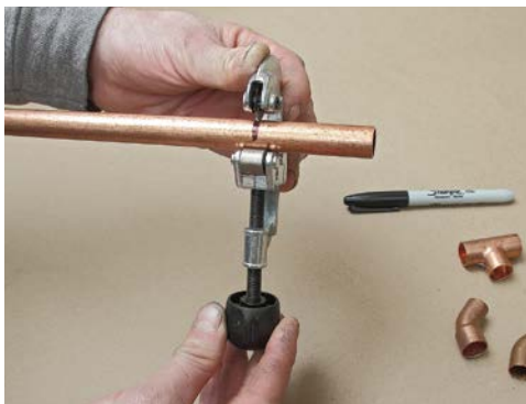
1 Tighten the cutting wheel on the cut line.
