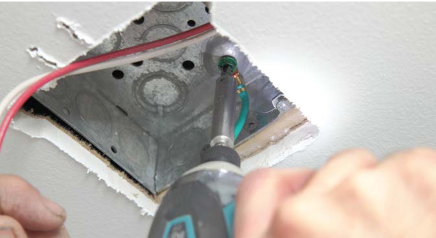
1 Connect the ground wire to a metal box or to the house's ground wire.
