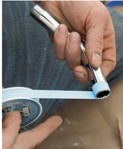
1 Wrap Teflon tape clockwise around both threaded ends of the shower arm.
