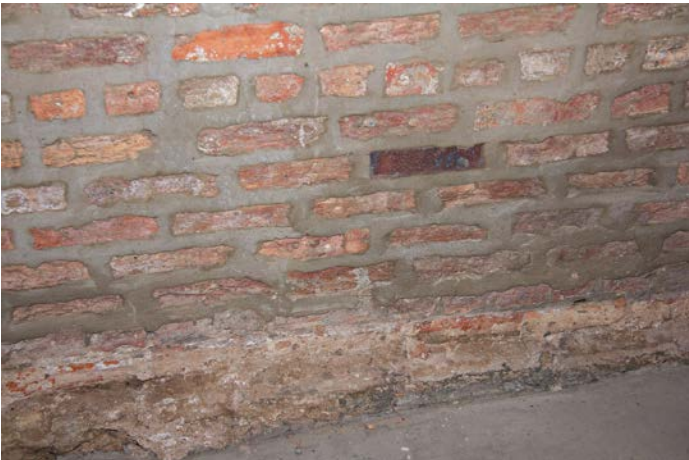
This common-brick wall has joints with extra mortar for added protection.
