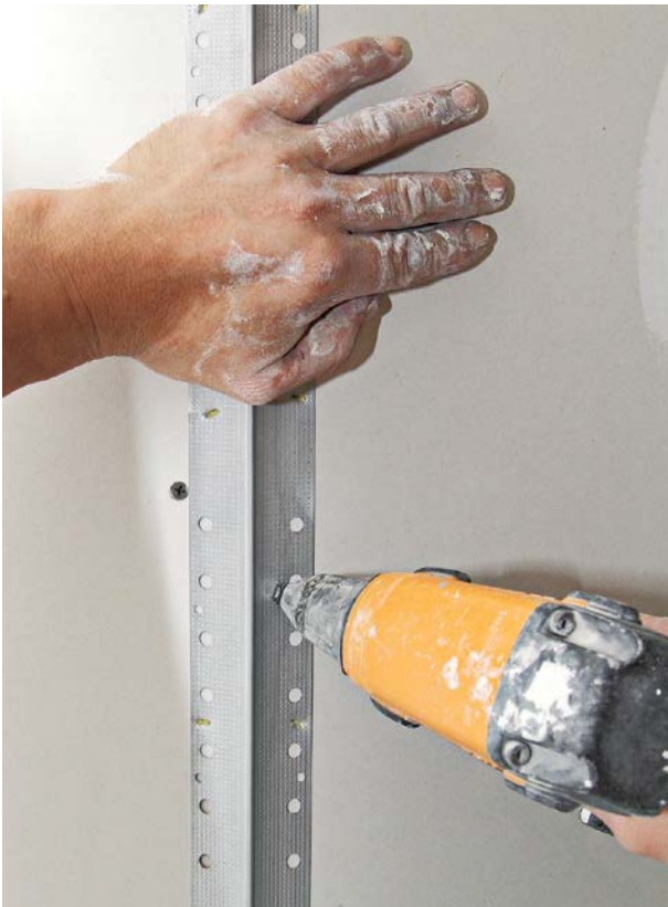
2 Press into place and drive fasteners on each side.
