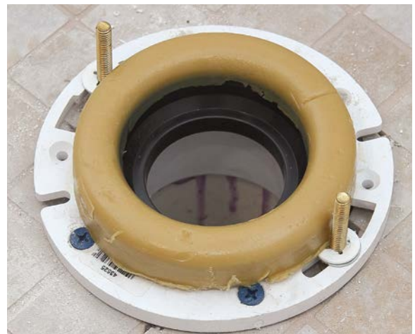
6 Position upward-pointing mounting bolts and a flanged wax ring onto the toilet flange.
