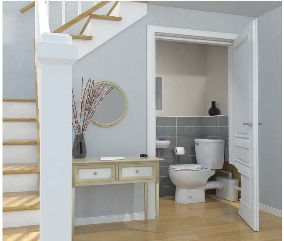
A powder room tucks under the basement stairway. Behind the toilet is an up-flush unit that pumps waste up to a drainpipe, so you don't have to cut into the floor.
