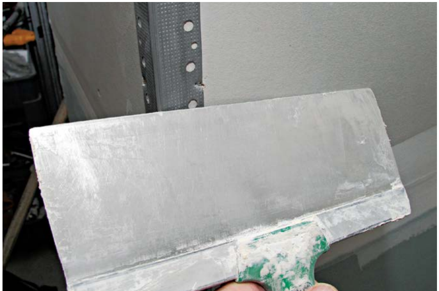
3 Test that nothing will stick out when you fill with joint compound.
