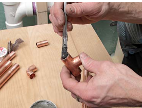
4 Burnish the outsides of the pipe ends and the insides of fittings.
