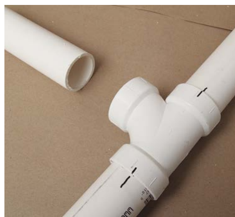
3 Assemble pipes and fittings in a dry run, and draw layout lines where needed.
