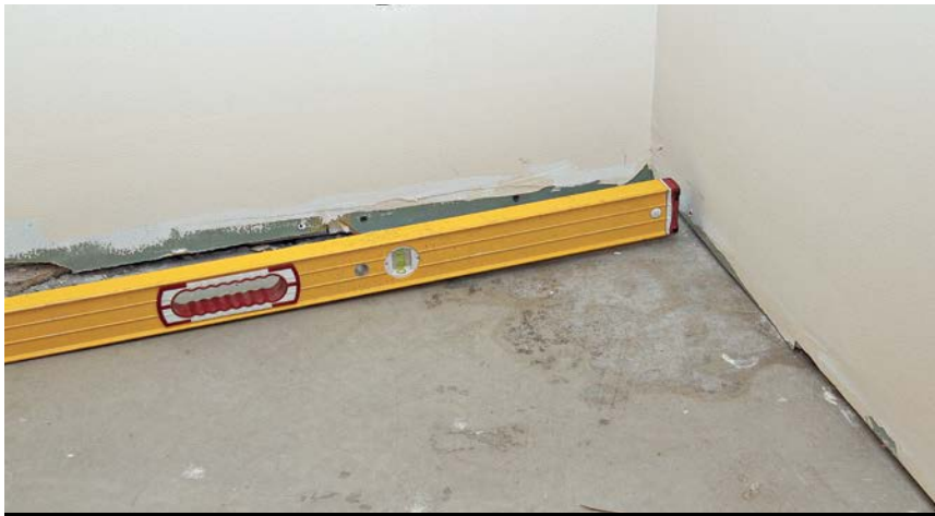
1 Use a long straightedge to check the floor for indentations.
