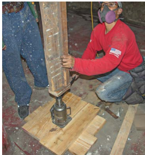
1 Temporarily support the joists before removing the damaged beam section.
