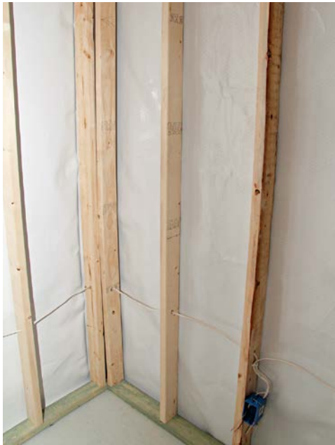
A thick plastic liner with a running drain below ensures against moisture buildup in the framing cavity.
