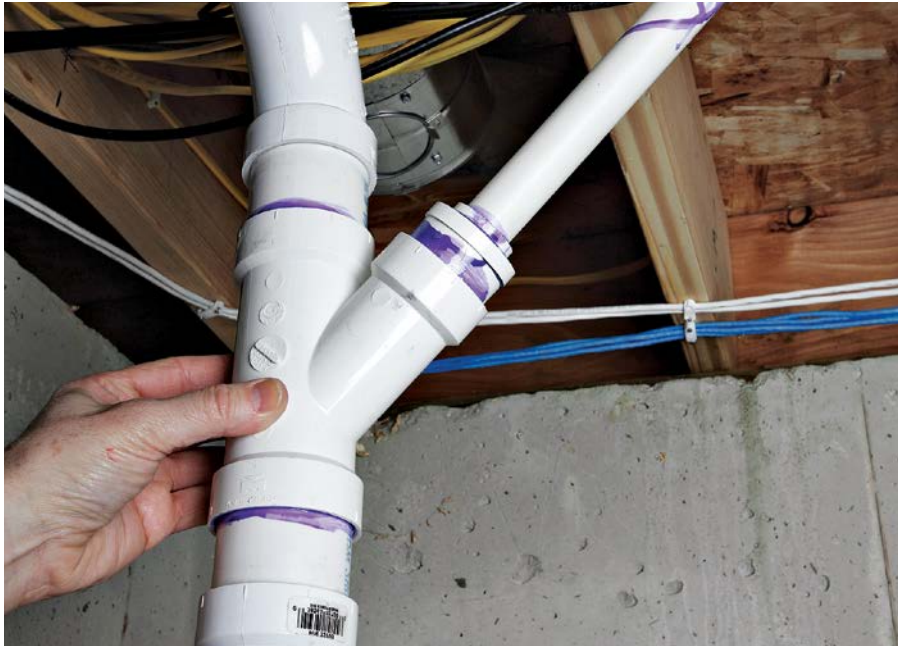
3 Install a Y fitting onto the house's stack, and run the discharge line into it.
