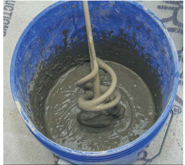
2 Mix a batch of reinforced thinset mortar.
