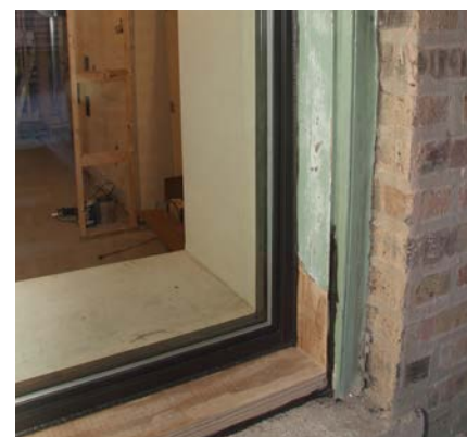
This old buck (and its outside trim) was in basically good shape, but the bottom pieces had some rot and so were replaced.
