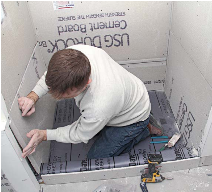
7a Attach backerboard pieces to the sides . . .
