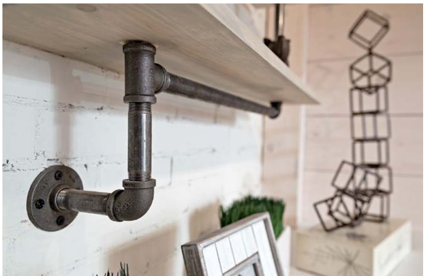
Even exposed black steel gas pipe can be appealing, especially if it is neatly installed and clean. Here, the excess pipe dope or Teflon® tape has been carefully removed.
