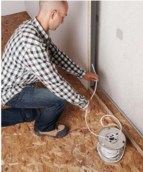
5a Feed electrical cable through channels in the panels . . .
