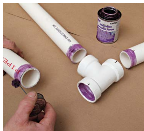
4 Apply PVC primer to the pipe ends and insides of fittings.
