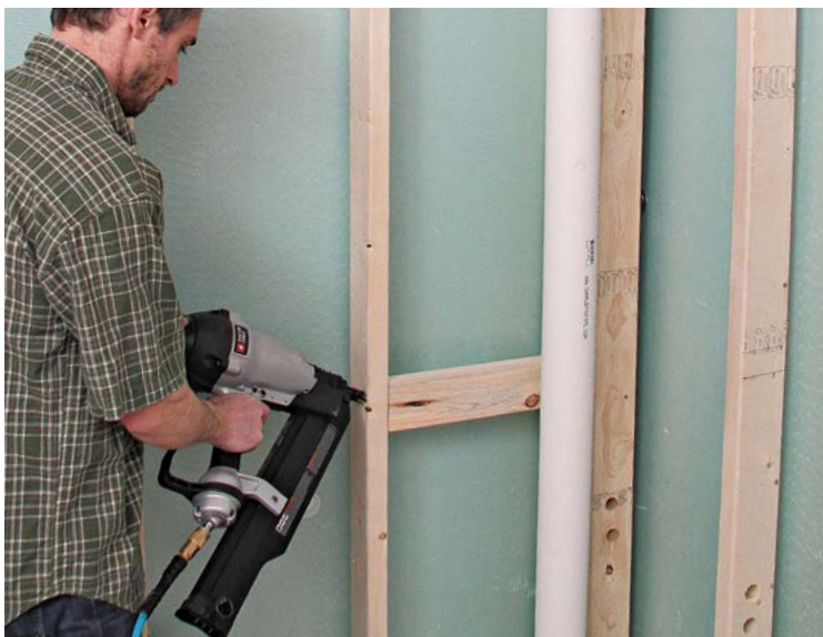
2a Attach blocking pieces where needed to support chase framing.
