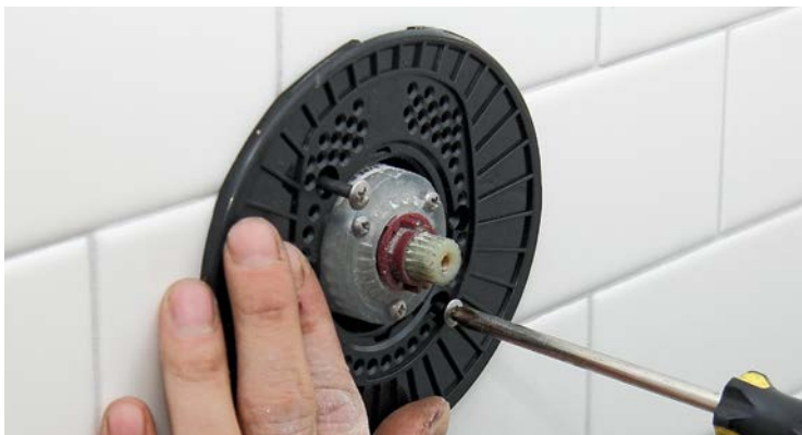
4a Mount the escutcheon. Here, a plastic plate is screwed on . . .
