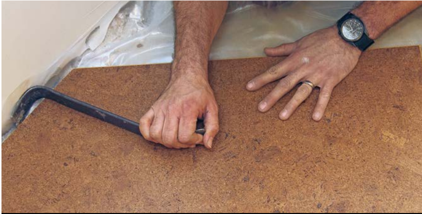
7 Use a flat pry bar to move a plank over and tighten the joint.
