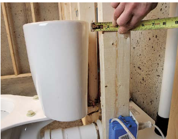
8 Connect the toilet to the unit, leaving space for the tank lid and drywall.
