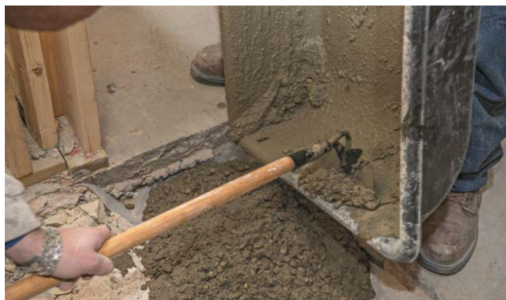
2 Mix and pour batches of high-strength concrete.
