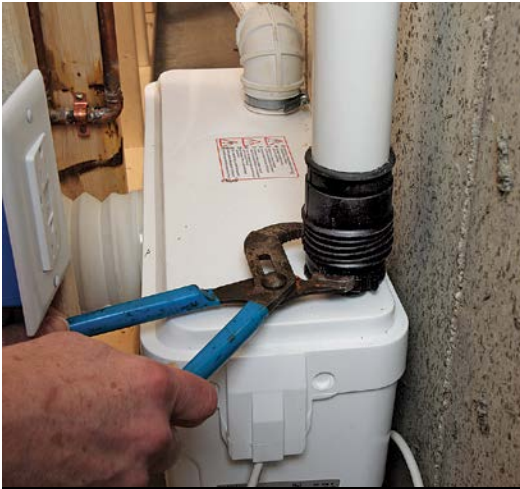
6a Connect a vent pipe to the up-flush unit . . .
