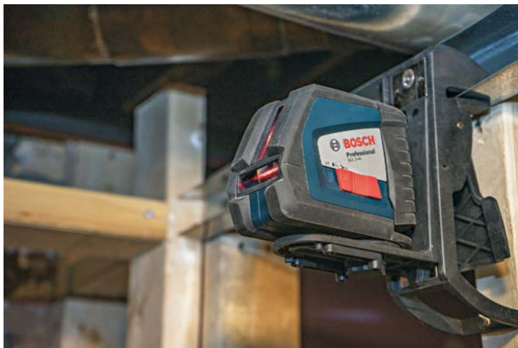
A laser level makes it easy to keep track of a ceiling's level over even a large area.
