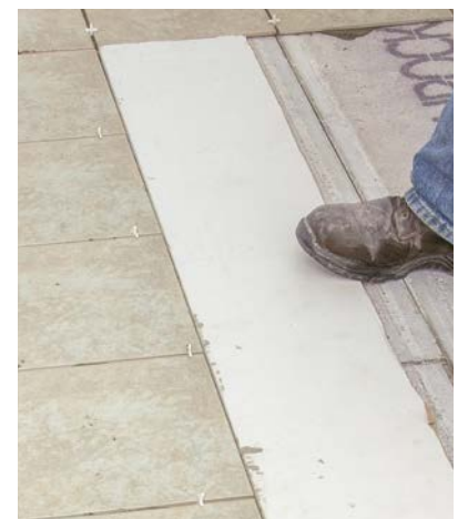
9 Every six or seven rows, align tiles with a straightedge.
