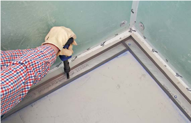
4 Anchor the bottom channels with powder-actuated nails.
