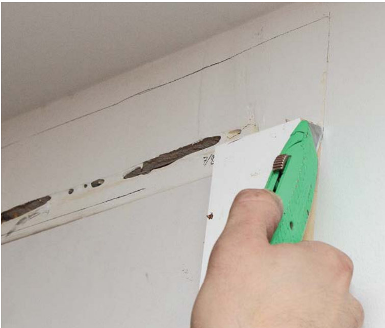
6a If the wall is angled, cut through the paper around where the casing will go . . .
