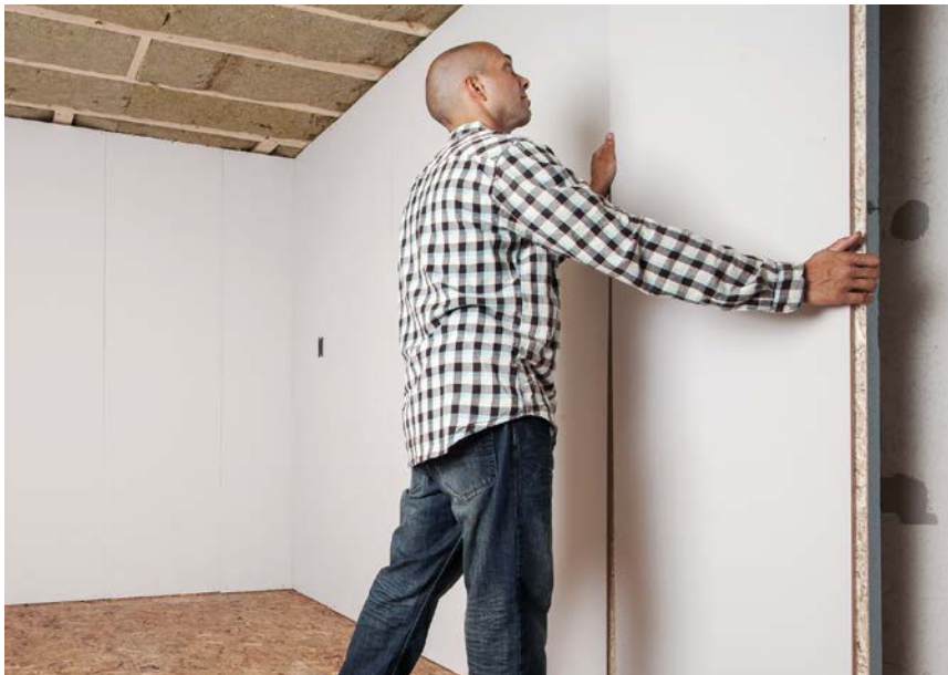
7 Continue installing panels, measuring and cutting them to height as you go.
