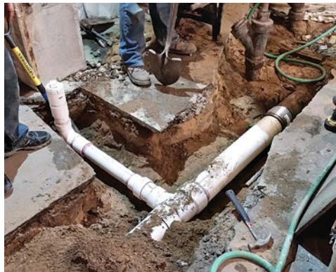
Cut channels in the concrete and connect new pipes to the existing drain line.
