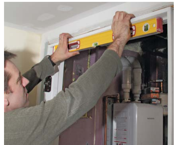
7 Check the head jamb for level.
