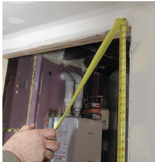
2 Measure for the height of the jambs.
