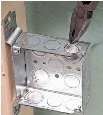
C1 Poke open a knockout slug . . .
