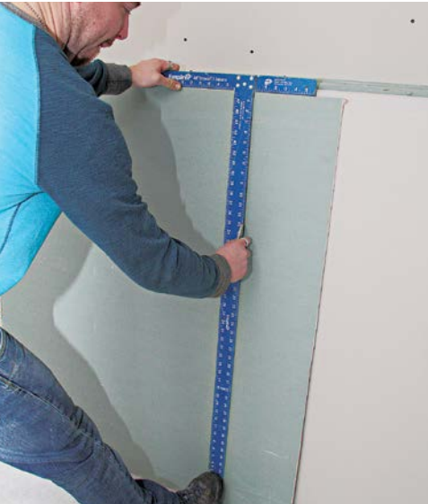
2 Hold the square firmly with a hand and foot, and cut through the paper.
