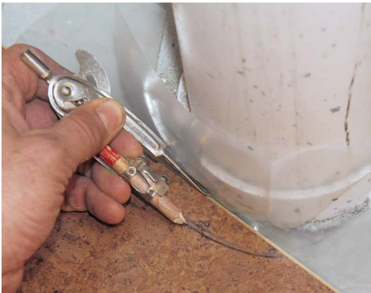
13 Keep the compass correctly adjusted as you mark for the cut.
