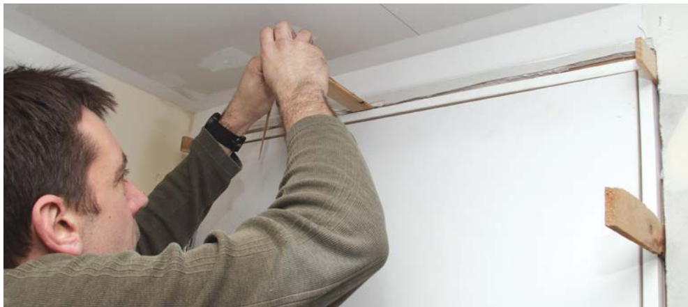
13 Check for an even \frac{1}{8} -in. gap all round, and install a pair of shims at the head jamb.
