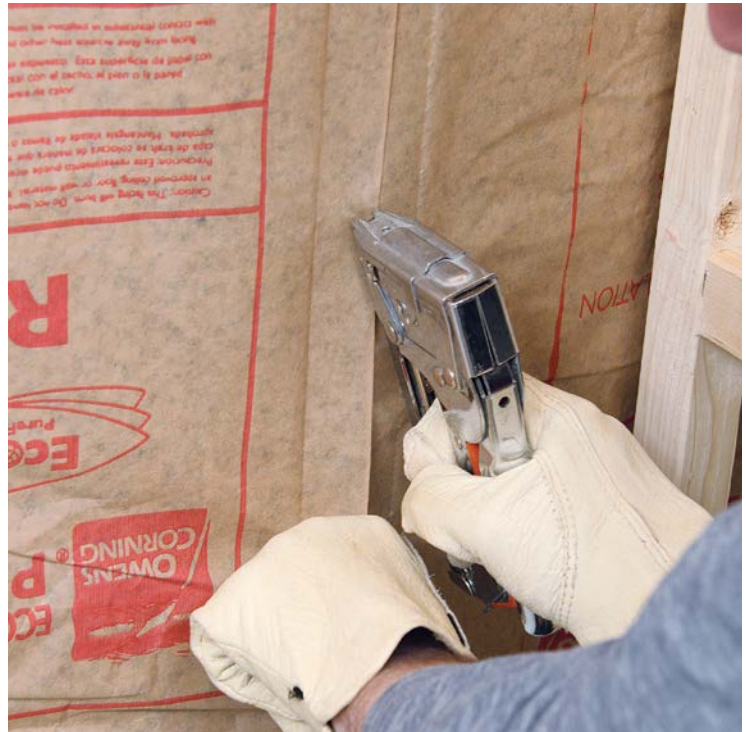
4 Pull the tabs taut as you drive staples into studs.
