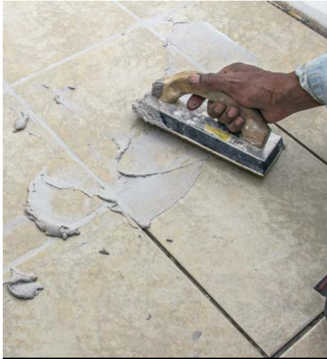
11 Hold the grout float flat and press grout into the joints.
