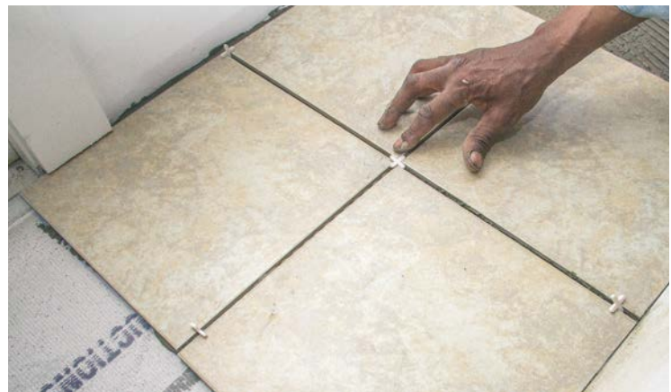
6 Slip in plastic spacers to maintain consistent and straight grout lines.
