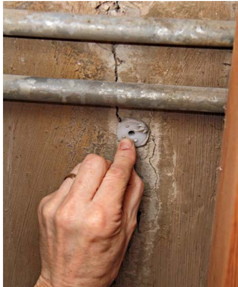
4 Apply a small amount of epoxy to an injector port's flange, and press into place.
