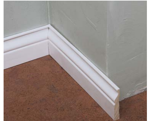
3 The cope-cut piece should fit snugly.
