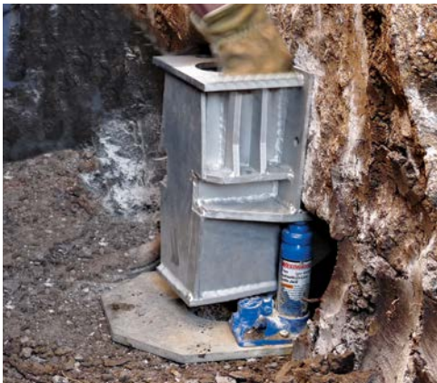
Raising a sunken foundation calls for digging a big hole and firing up heavy-duty equipment in order to add a bracket for support.
