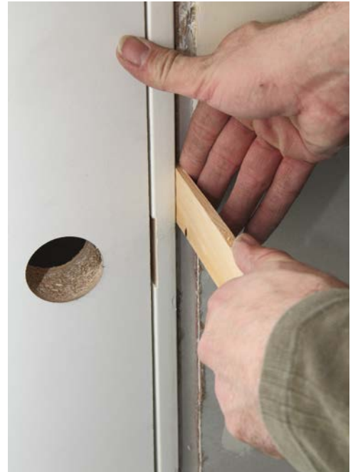
12 Also shim the latch-side jamb.
