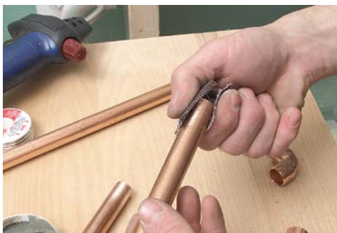
4 Burnish the outsides of the pipe ends and the insides of fittings.
