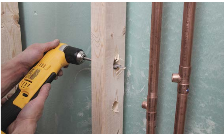
5 Bore holes with a right-angle drill.
