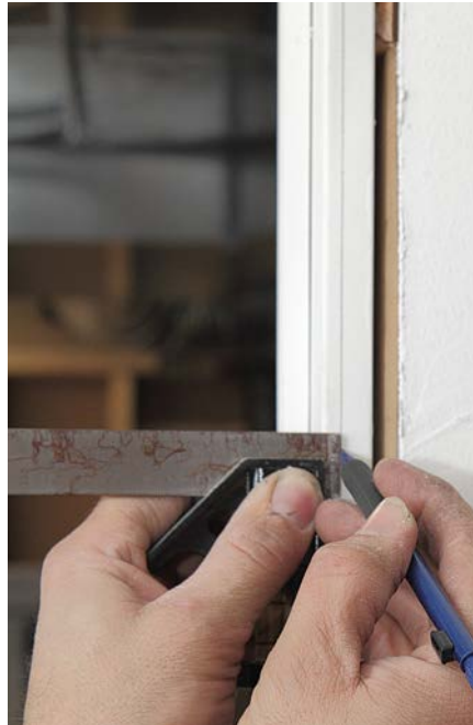
3 Mark the reveal on the jamb edges.
