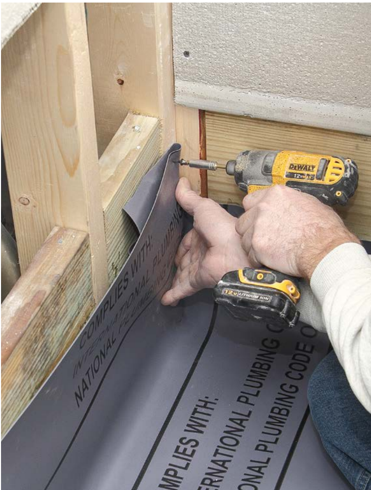
4 Make folds at the corners and drive screws several inches above the floor to attach.
