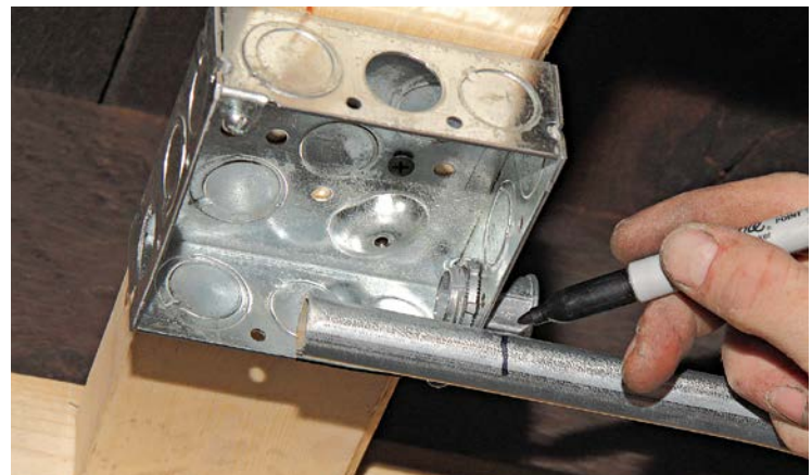
3 Mark for cutting conduit so it enters the box's clamp.
