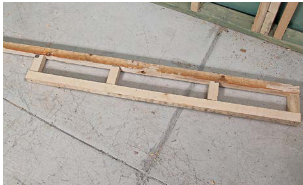
4 Build a soffit frame.
