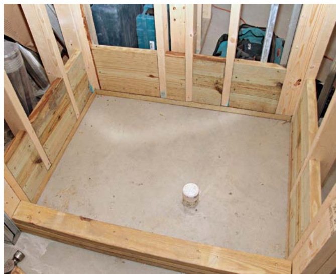
A well-framed shower stall includes blocking pieces at the bottom so the wall will stay firm even if kicked.
