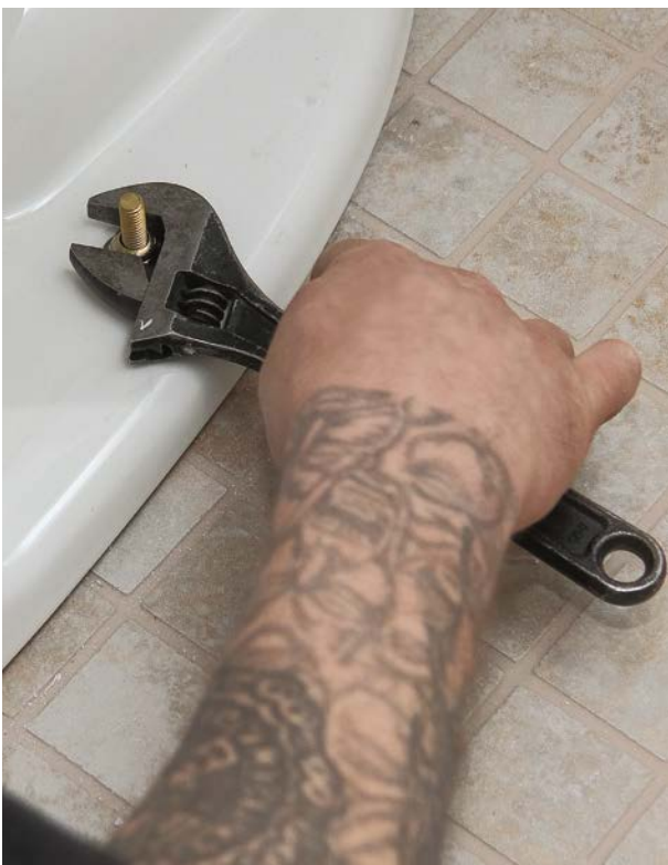
9 Tighten the mounting bolts and cut them to height if needed.
