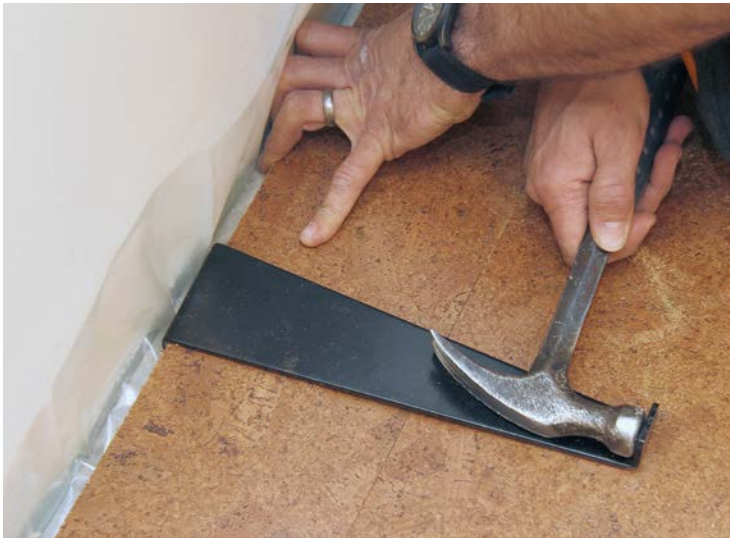
9 Use a pulling tool and hammer to achieve a tight joint.
