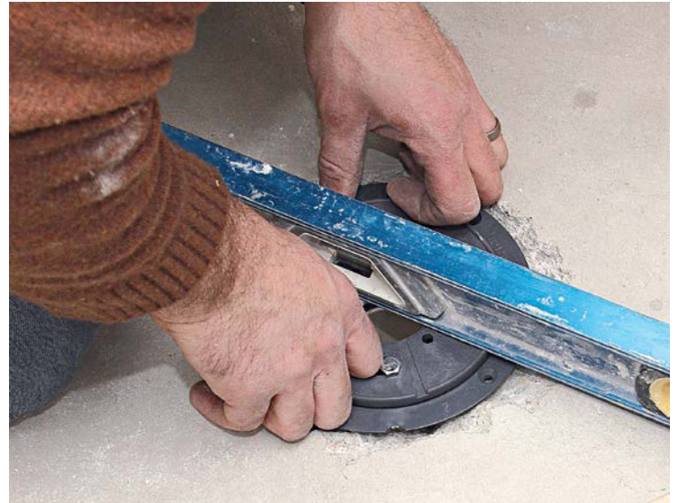
2b ... then apply cement, and attach the flange so it is level.
