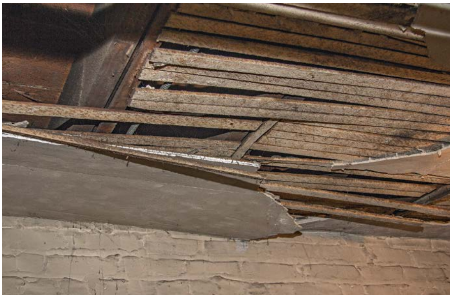
Old plaster often fails in a basement. Depending on the amount of damage, you may repair, replace, or cover over it.
