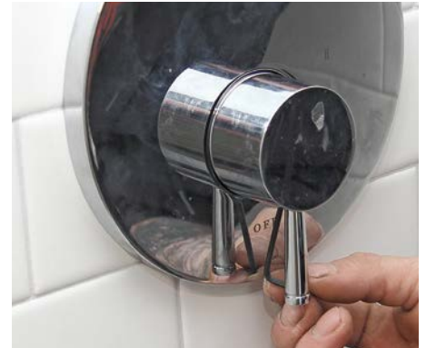
5b . . . then attach the handle.
