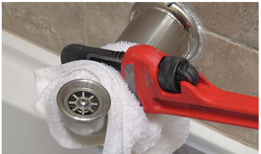
7 Protect the spout from scratches and tighten with a wrench.
