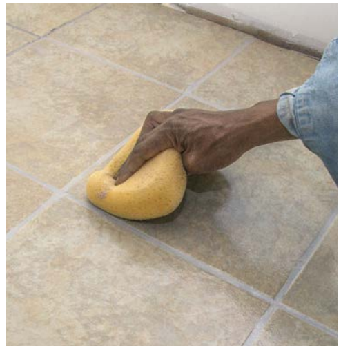
14 Use the sponge to form grout lines that are consistent in depth.
