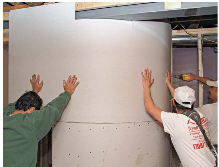
4 Work with helpers to bend and attach two layers of drywall.
