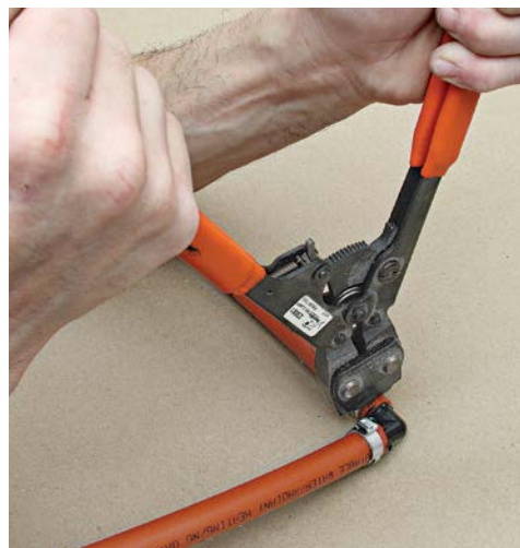
5 Place the clamp tool's end over the fitting wings and tighten all the way.
