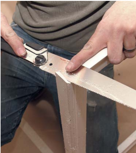
6 If one piece was rip-cut, use a handsaw to cut off the resulting protrusion.
