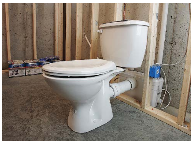
9 Screw the toilet to the floor and finish making connections.
