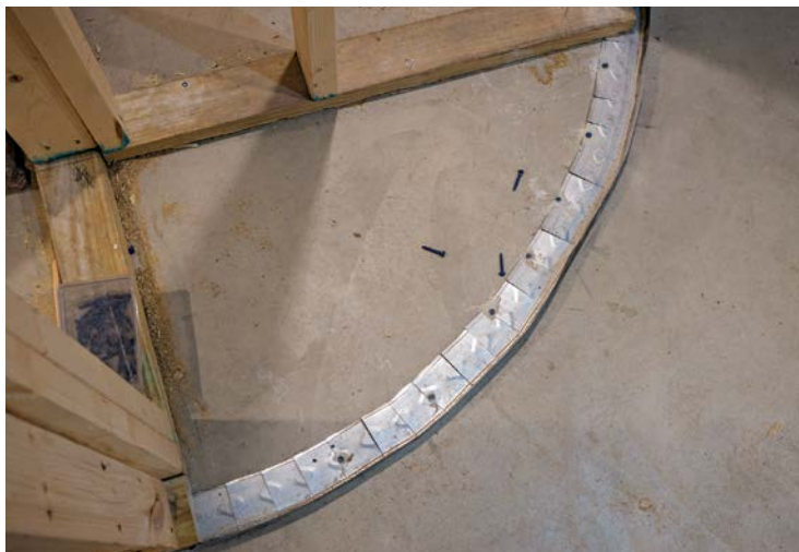
1 Cut off one flange and make a series of cuts to create bendable plates.
