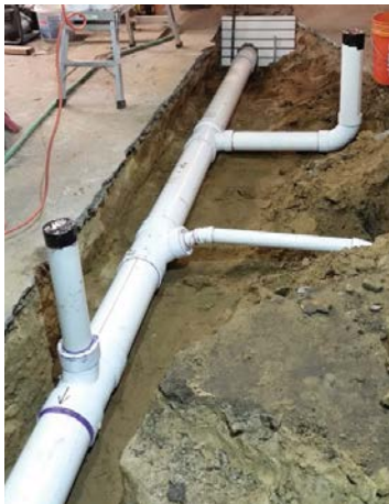
Install a main drainpipe as well as branch pipes, check that they are all sloped downward, and make sure they emerge at the right points in the floor.
