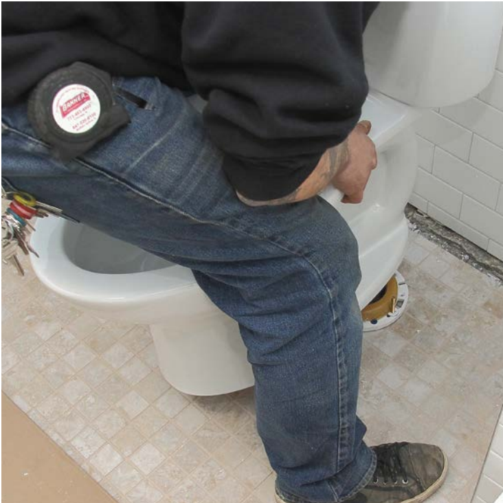
7 Lower the toilet so the mounting bolts thread through the holes in the bowl.
