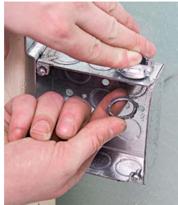
D Insert a metal cable clamp and slip on the nut.
