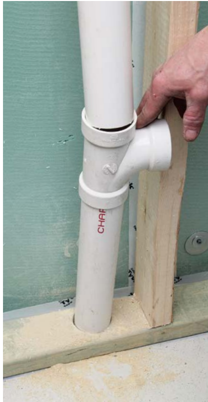
4a Move the pipes and slip in the fitting...
