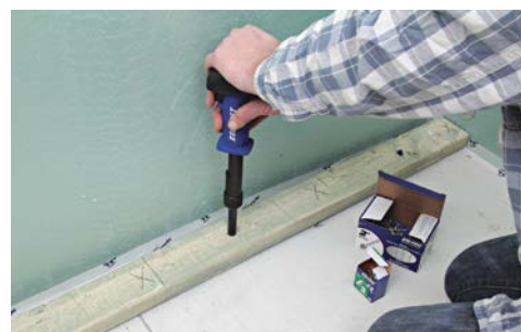
8 Shoot nails or drive screws every 16 in. or so with a powder-actuated nailer.
