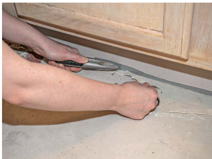
Remove any other obstacles. Here, vinyl cove base curves out to get in the way. The bottom portion is being cut away; new molding will cover the rest of the base cove.
