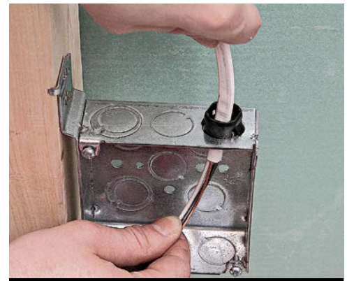
H Carefully poke cable into the box; be sure you don't push too far.
