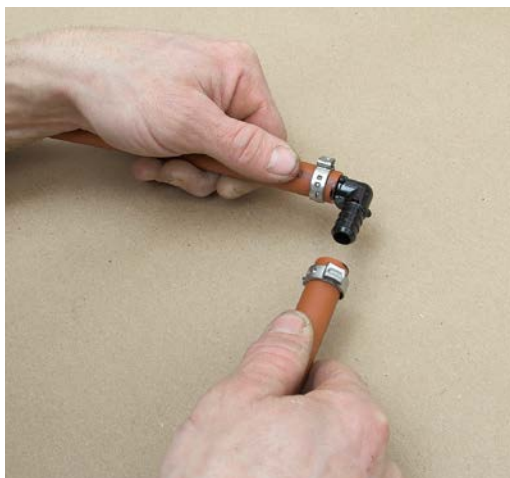
4 Insert the barbed fitting ends into the tubing, and see that the rings are positioned over them.
