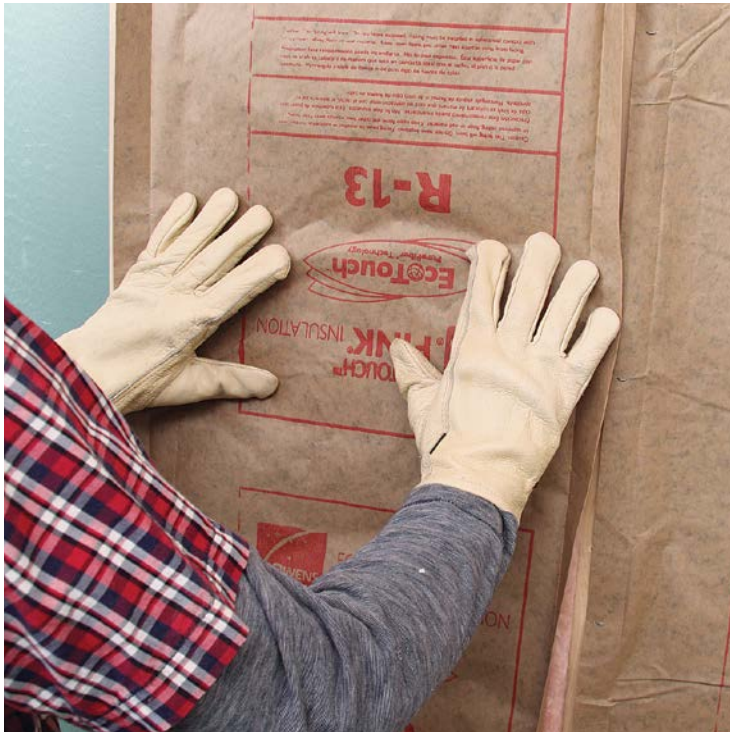
3 Press the insulation in place between studs, maintaining the fluff.
