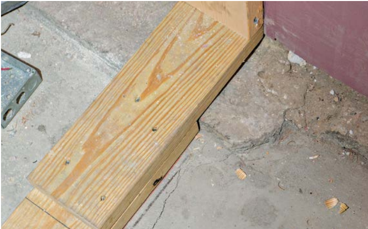
5 Basement framing often calls for improvisation. Here, a change in the concrete floor's elevation is accommodated by simply attaching a short board.
