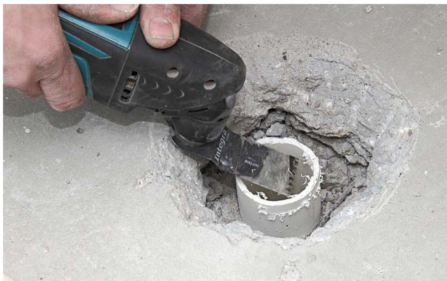
1 Chip away around the drainpipe and cut it flush with the floor.
