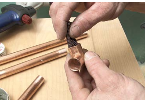
4 Burnish the outsides of the pipe ends and the insides of fittings.
