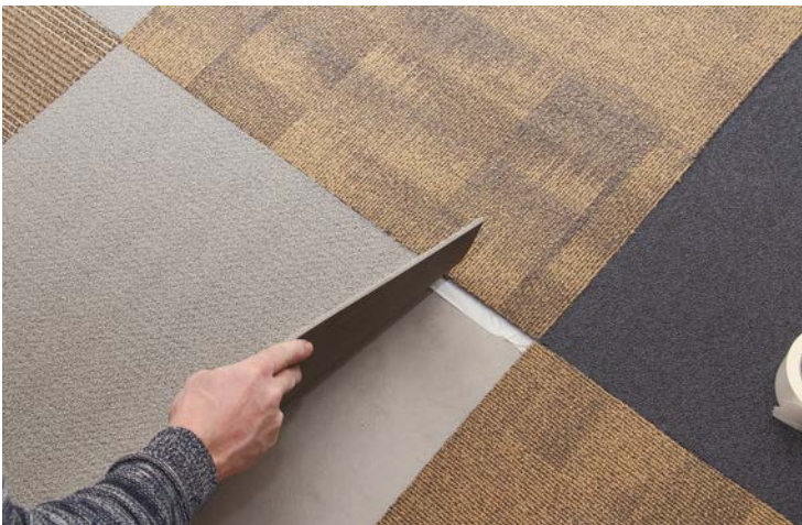
5 Gently set the next tile in place.
