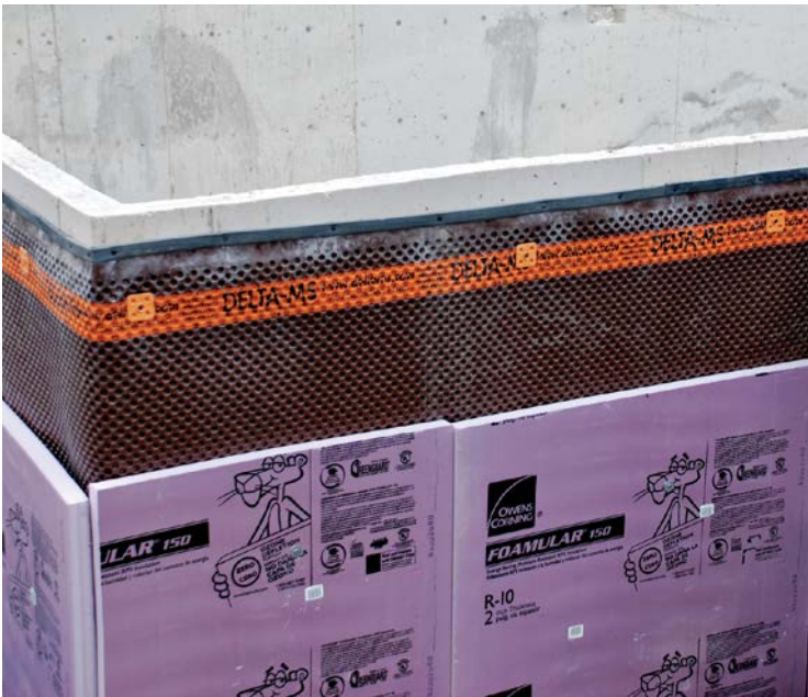
Rigid insulation is fairly expensive, but will ensure against condensation inside the basement and will cut down on heating costs as well.
