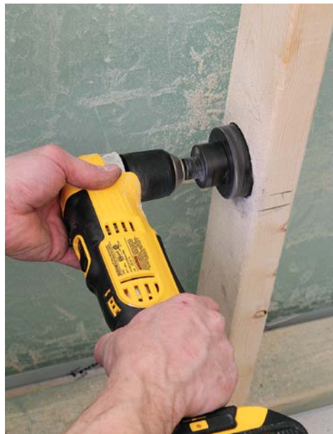
8 Drill holes through the studs.
