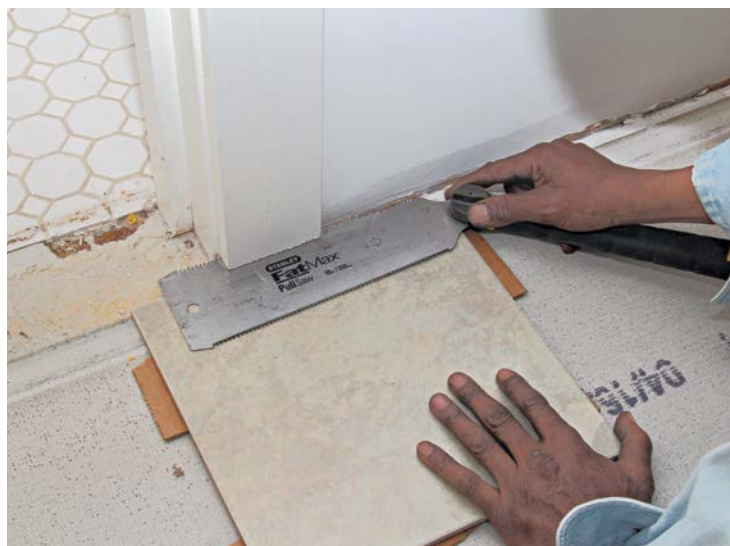
Cut the bottom of door casings so that the substrate and the finish flooring can slip underneath. Here, for example, the height guide is made with a sheet of backerboard, thin shims to represent the thickness of the mortar in which the tiles will be installed, and a tile. Cut with a special saw made for the purpose, or as shown here, with a Japanese pull saw.
