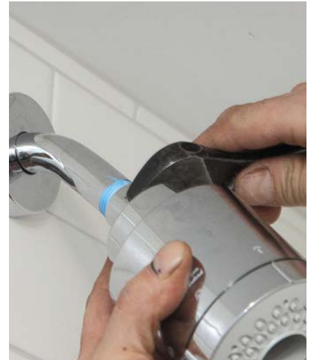
2 Tighten the shower arm, then the showerhead.
