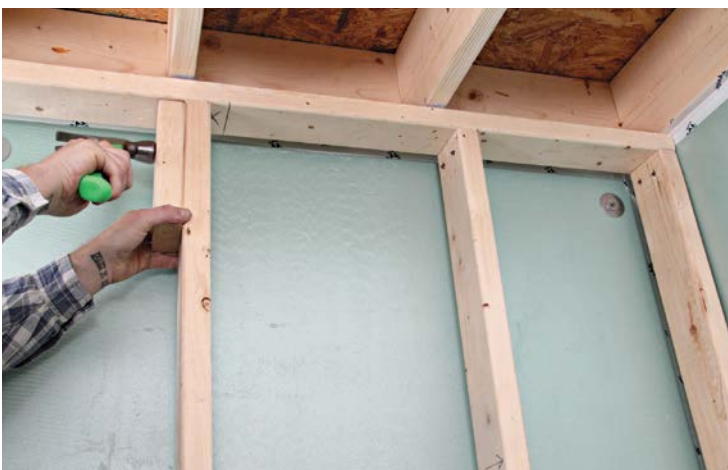
7 Tap studs into position; aim for a snug but not tight fit.
