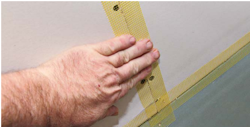
1 Apply self-sticking fiberglass mesh to tapered and butt joints.
