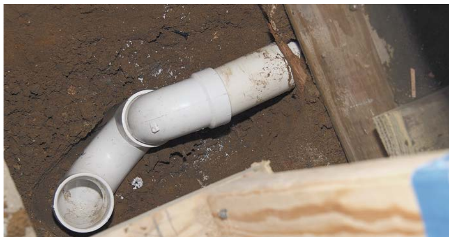
2 Connect the drainpipe to a P trap and position it according to the manufacturer's instructions.
