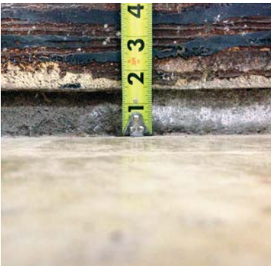
A floor that is 1 1/2 in. below the bottom of the wall (left) has sunk and needs to be raised and reinforced. After raising the foundation with a foundation pier and supporting it by pumping in concrete, as shown on p. 46, the floor is brought up to meet the wall and will not sink any farther (right).
