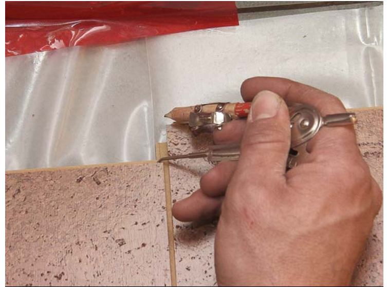
12 To cut around a pipe, position the board against the obstacle and adjust a compass for the depth of the cut.
