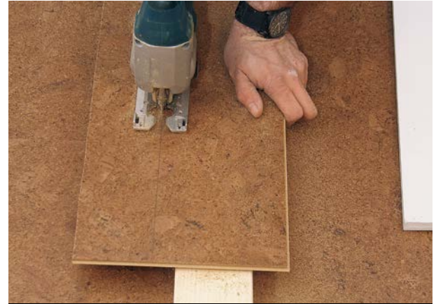
8 Where you meet the wall lengthwise, cut planks \frac{3}{8} in. short of the wall.
