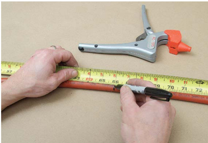
1 Measure for cutting and mark with a felt-tipped pen.
