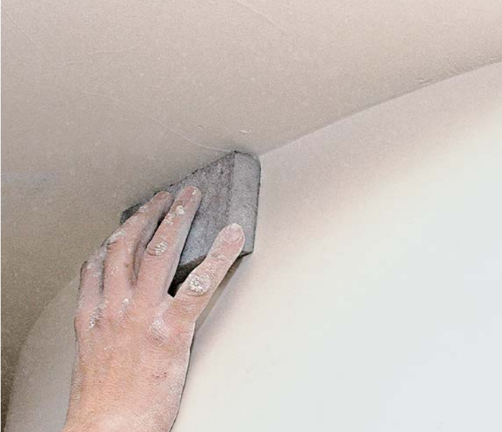
3 A foam sanding block works well in unusual places.
