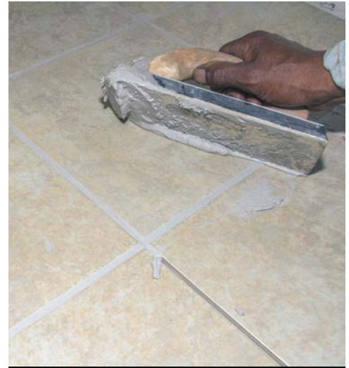
12 Tilt the float up and squeegee away most of the excess grout.
