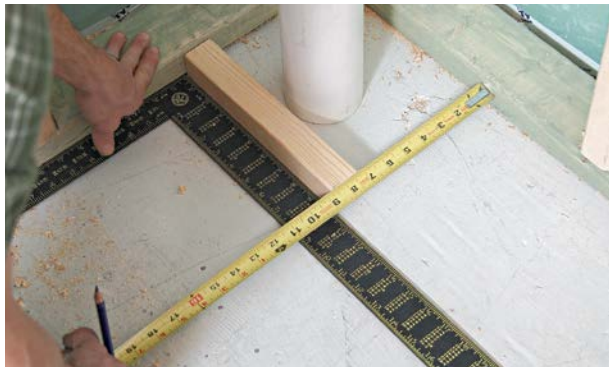
3 Install blocking on the floor to outline the chase.
