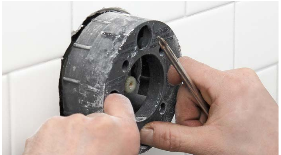
3 Remove the faucet's plastic guide.
