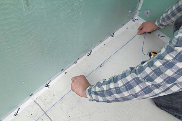
3 Snap chalklines on the floor and on the framing above indicating the positions of the plates.
