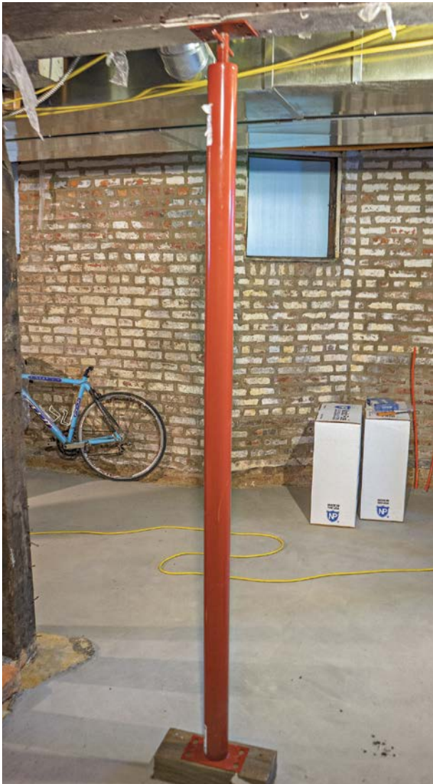
1 Use adjustable posts to raise the beam, then insert pieces of wood between the top of the post and the underside of the beam.
