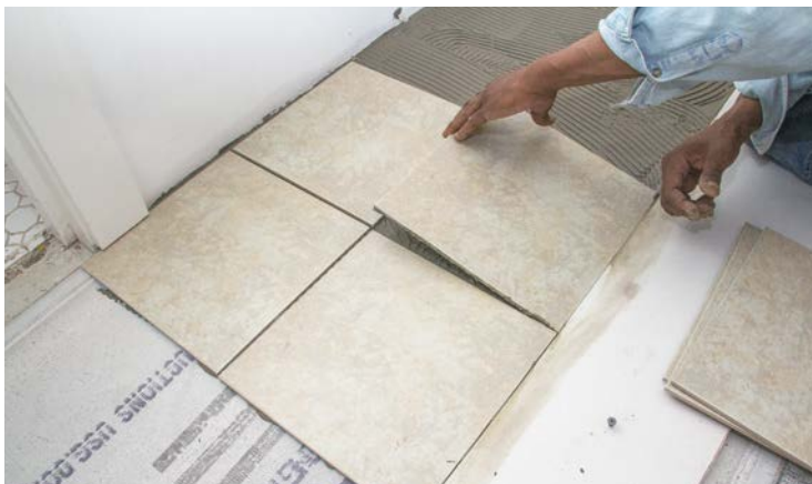
5 Lower tiles onto the thinset so you don't need to slide them very much.
