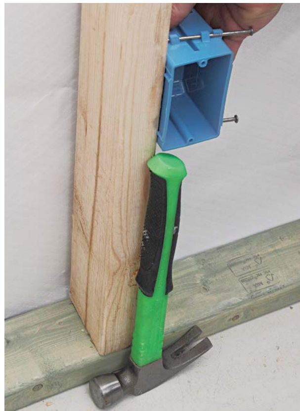
A hammer makes for an easy and convenient height gauge for receptacle boxes.
