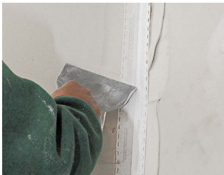
5 Scrape with a knife to fully embed the tape.
