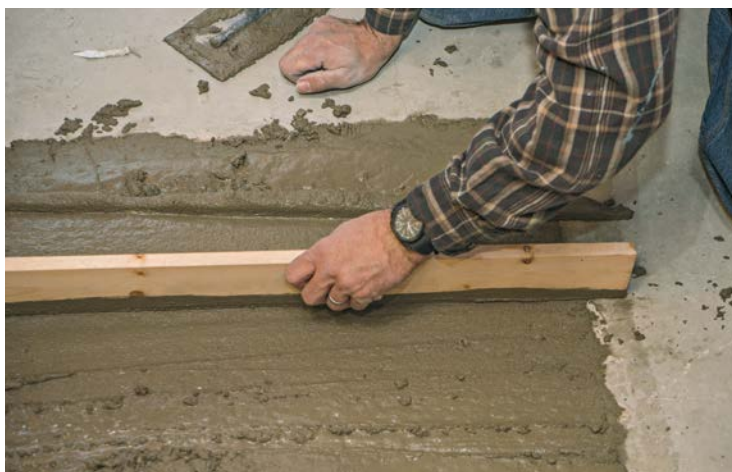
3 Roughly screed the patch with a 2x4.
