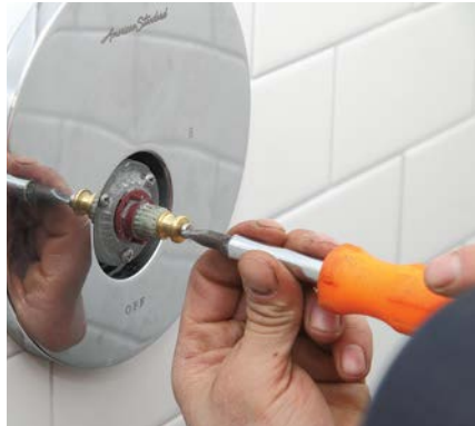
5a Install the faucet's handle assembly . . .
