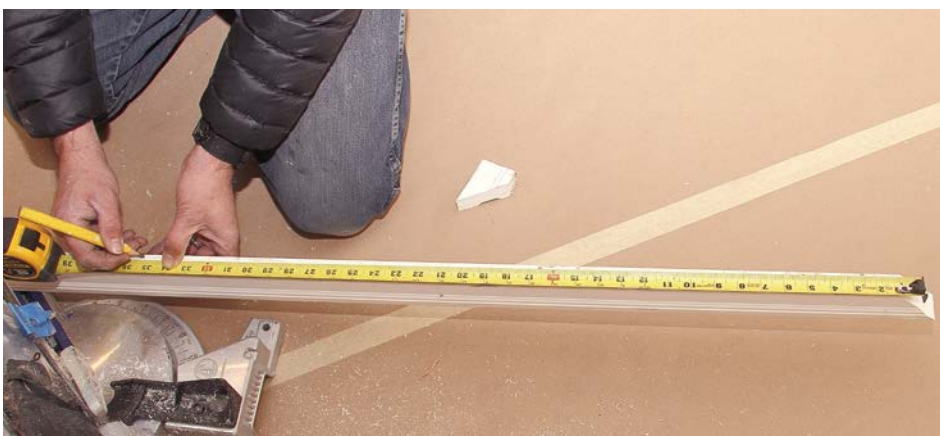
3a Measure for miter cuts on each end by burning an inch . . .
