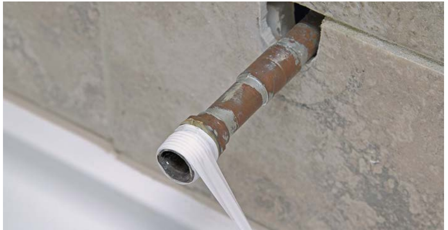
6 Wrap both ends of a pipe with Teflon tape and screw into the outlet in the wall.
