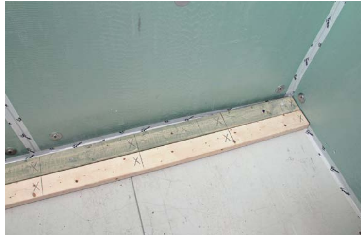
4 Mark both plates with stud locations.
