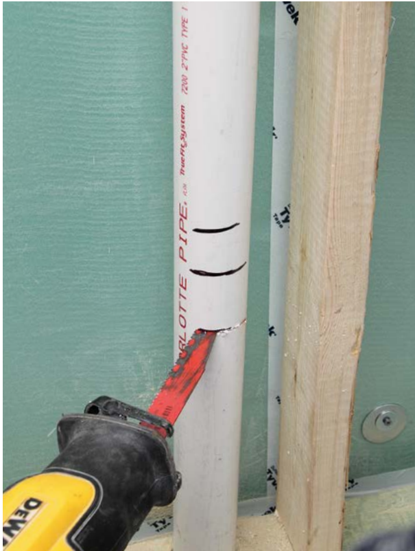
3 Cut with a fine-toothed blade.
