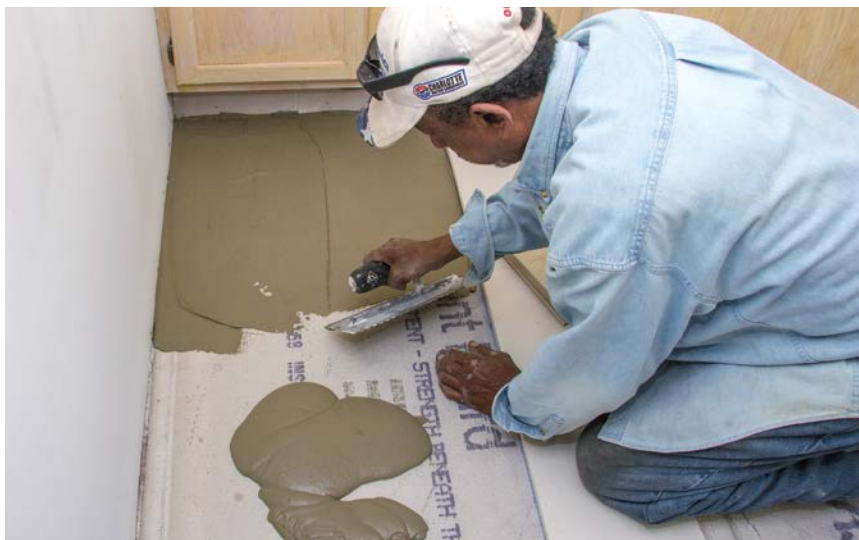
3 With the flat side of the trowel, push and spread the thinset.
