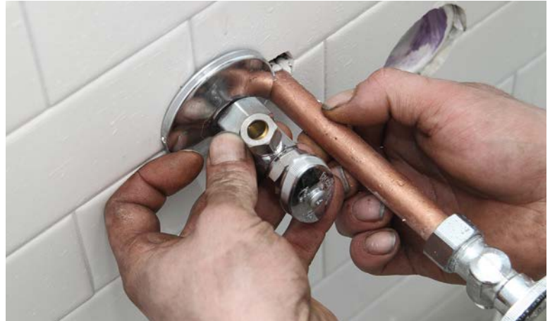
1 Measure for cutting the pipe so the valve will hide it.
