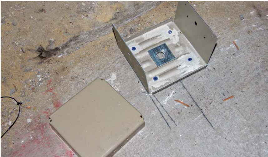
2 Find a level spot under the beam for the post anchor, then secure it to the concrete floor with a masonry screw.
