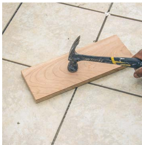
8 Use a flat board to check that the surface is even, and tap where needed.
