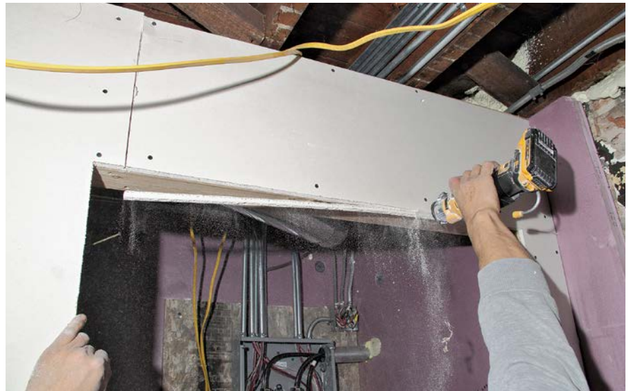
At a doorway or other opening, pros often attach drywall so it overhangs the opening. Then they use a router with a cutting bit to cut around the opening.
