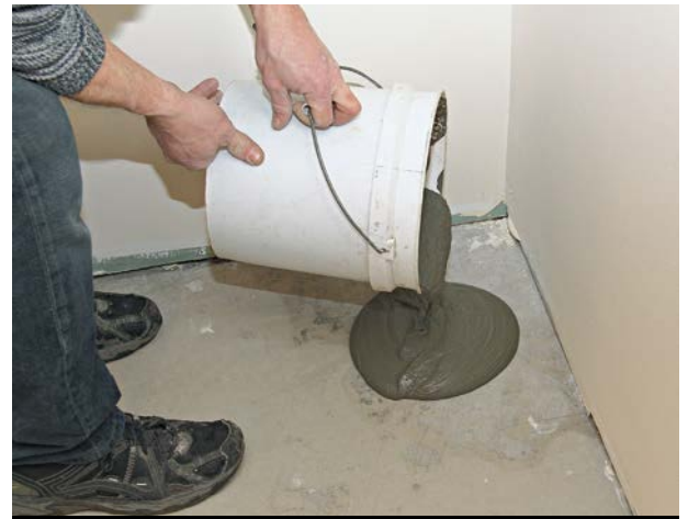
2 Mix a soupy batch of self-leveling compound and pour into the area.
