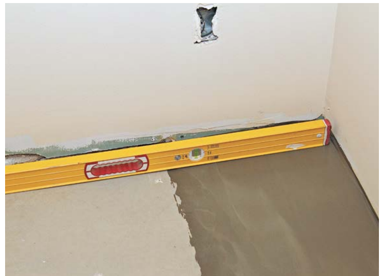
4 Check that the new patch is level with the surrounding surface.
