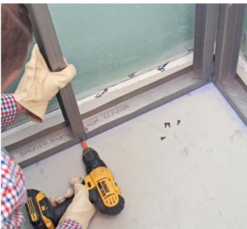
6 Attach studs with self-tapping screws.
