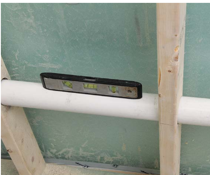
10 Recheck for slope.
