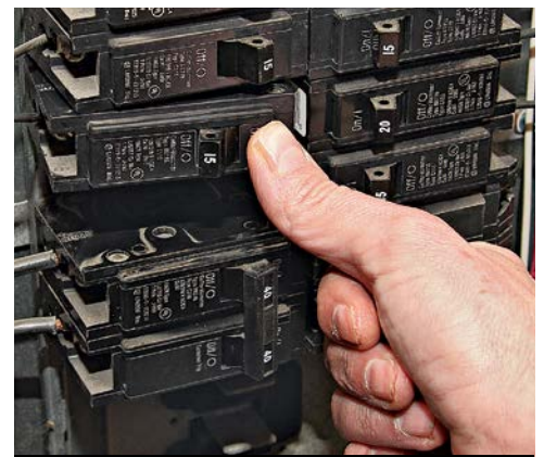
5 Snap the breaker into place. Restore power at the main breaker, and test.
