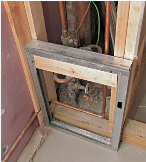
Always frame out for an access panel for the plumbing behind a shower.
