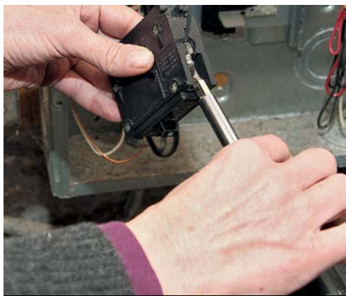
4b . . . then tighten the setscrew.
