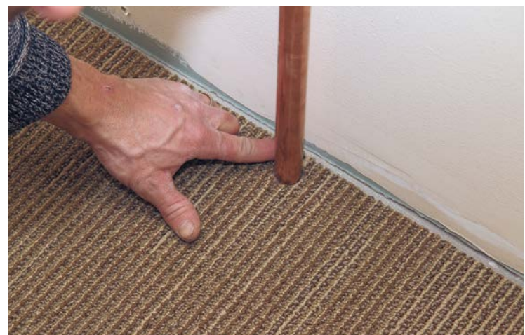
9 See that the fit is just snug, and not too tight.
