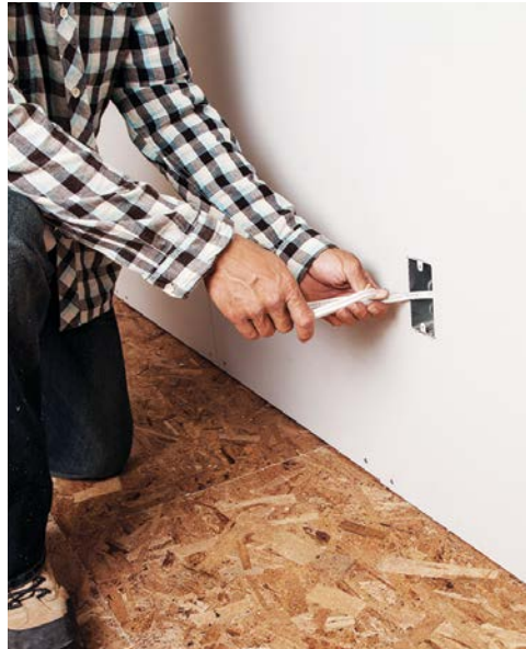
5b . . . then install into boxes.
