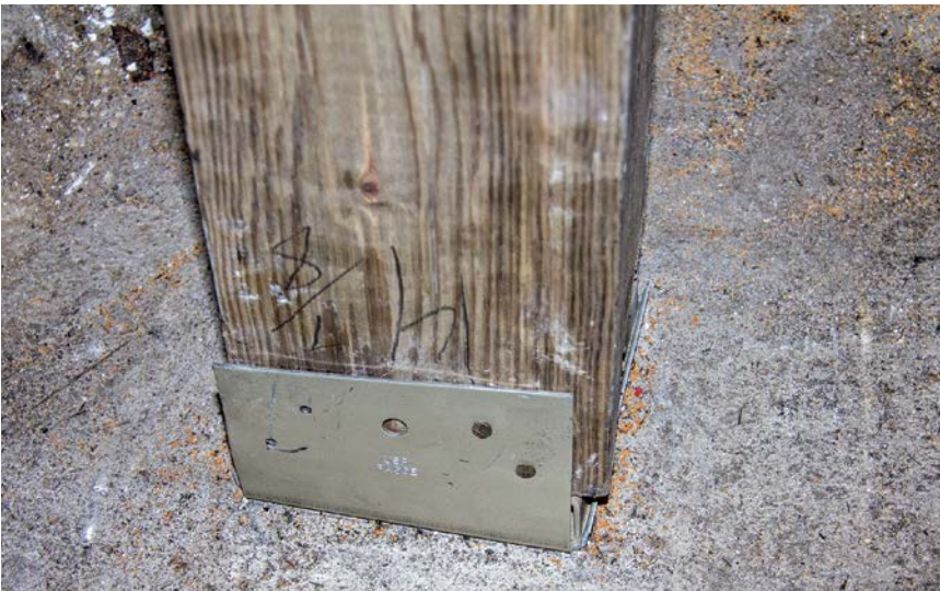
3 With the post set firmly and level in the anchor, secure the two together with screws or nails.
