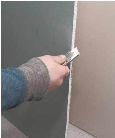
6 Scrape the ragged cut until smooth.
