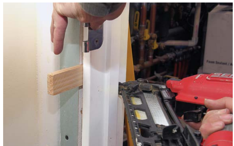
9 Drive pairs of finish nails near the shims.
