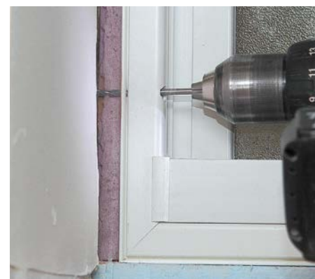
When installing a window, check for square and plumb or level. Drive mounting screws into the wood buck. Or, if there is no buck, drill holes into the concrete or masonry, and drive masonry screws that penetrate at least 1\frac{1}{2} in.
