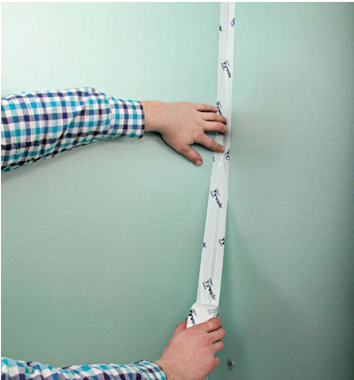
5 Building-paper tape can be used to seal joints between sheets.
