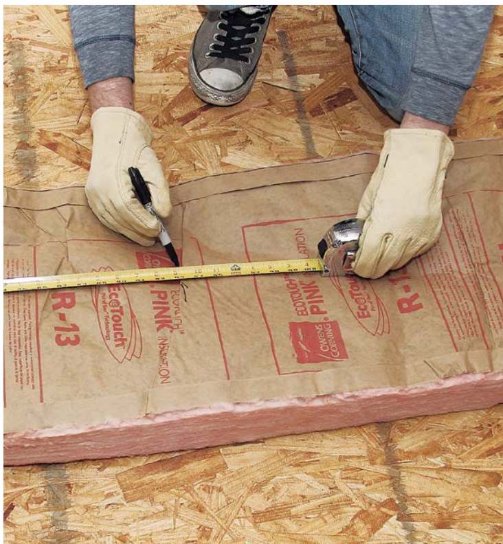
1 Precisely measure and mark for cutting a fiberglass blanket.
