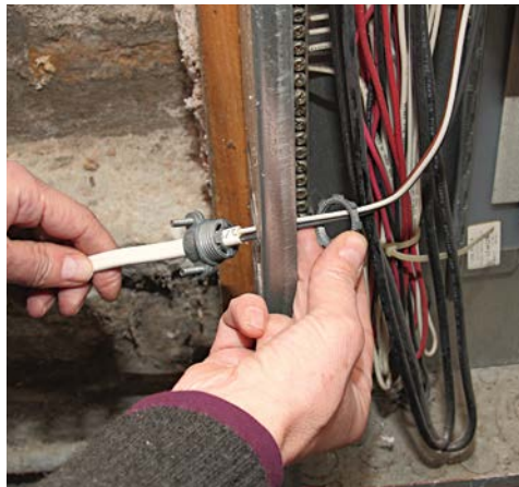
2 Install a cable clamp and run an ample length of cable into the panel.
