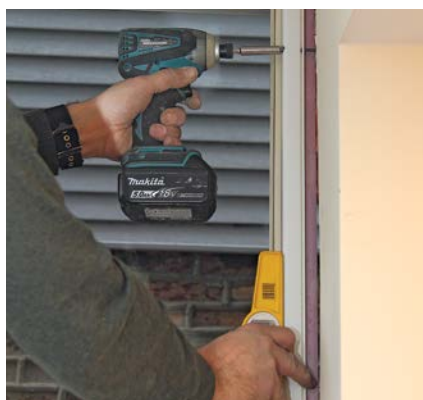
When installing a window, check for square and plumb or level. Drive mounting screws into the wood buck. Or, if there is no buck, drill holes into the concrete or masonry, and drive masonry screws that penetrate at least 1\frac{1}{2} in.
