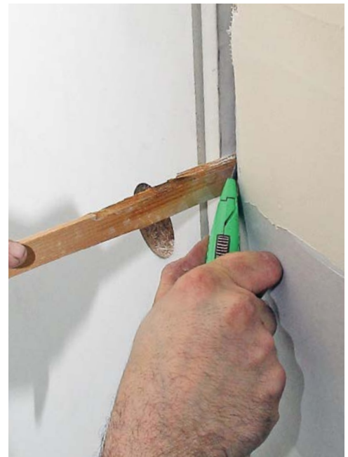
14 Cut away the exposed parts of the shims.
