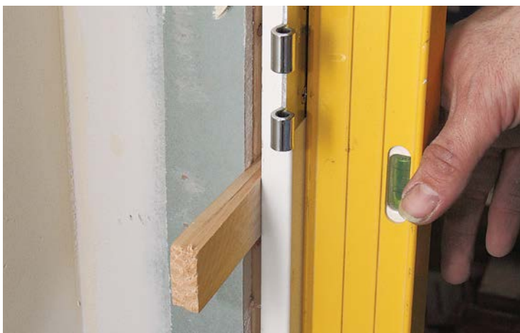
8 Shim the hinge-side jamb with pairs of shims.
