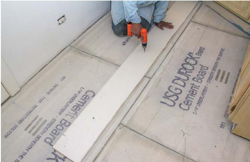
1 Fasten a temporary straightedge to guide your first row of tiles.
