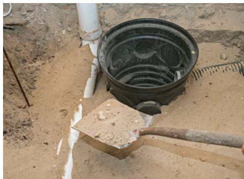
A basin is buried in the basement floor, with its top just above the floor level. Here, drain tile runs into the basin.
