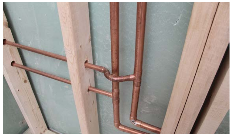
6 Assemble in a dry run, then disassemble and solder.
