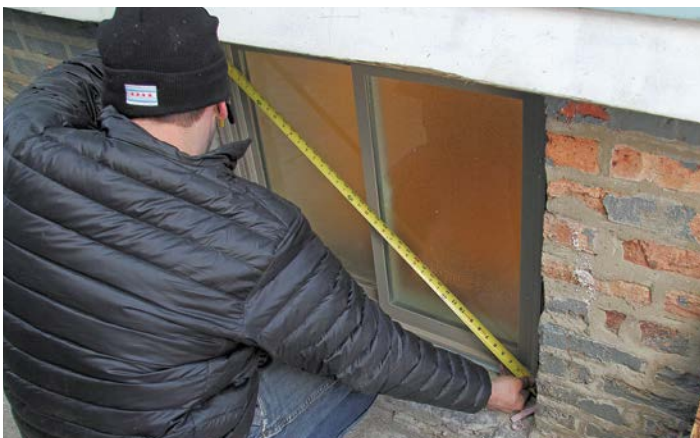
1 Check that the window is square and make adjustments if needed.
