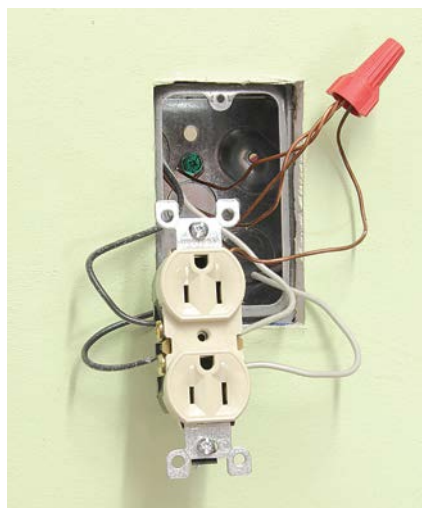
To wire a receptacle, connect grounds together, then to the ground terminal. Connect hots to the brass terminals and neutrals to the silver terminals.
