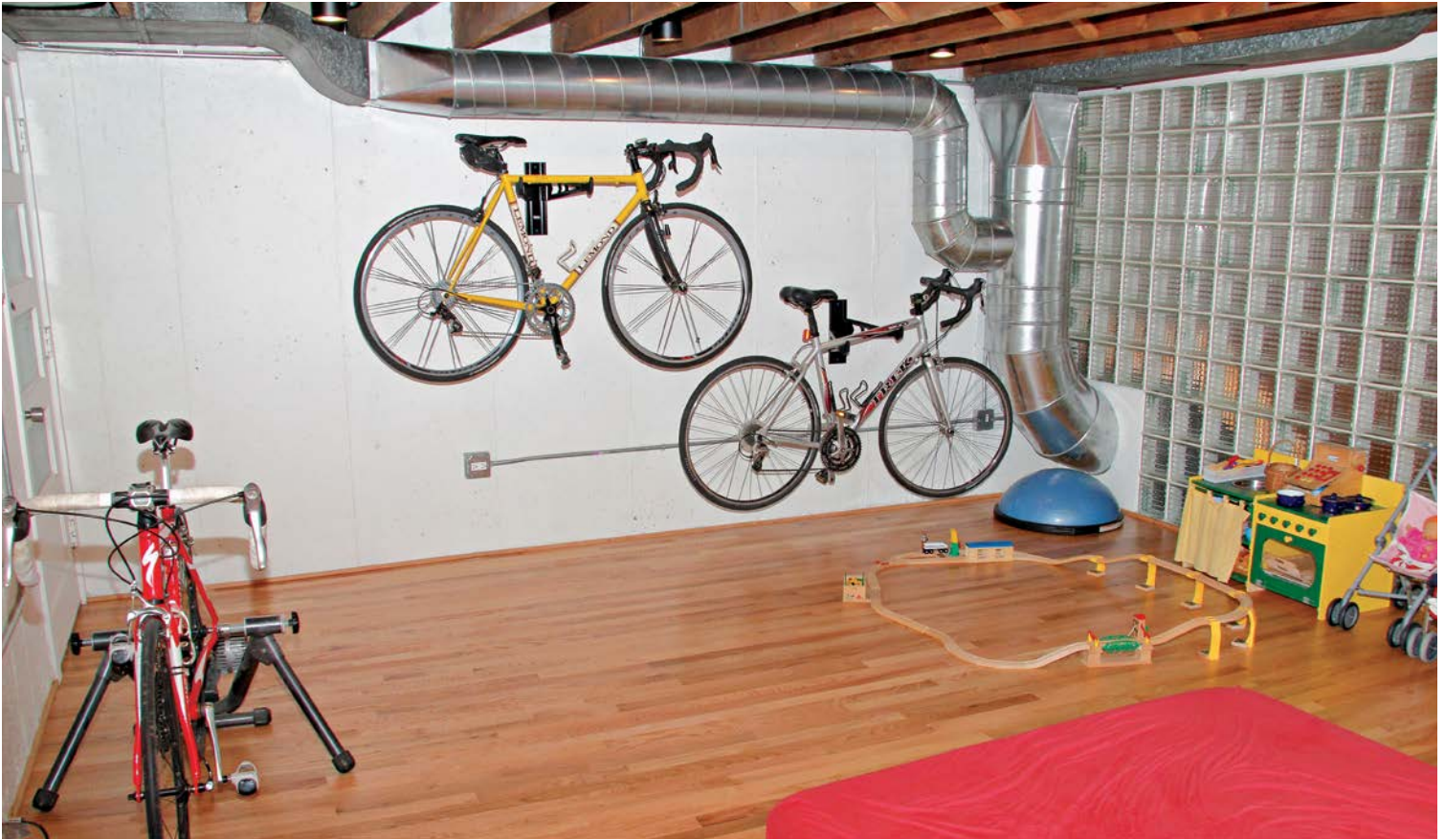
In this basement, a hardwood floor was laid, but the walls were simply spray painted; ceiling joists are left exposed, and electrical supplies are on display. Rather than hiding large ducts, they are celebrated for their shininess. Overhead canister lights are also left exposed, as is the wiring leading to them. A wall of glass block adds to a Euro style.
