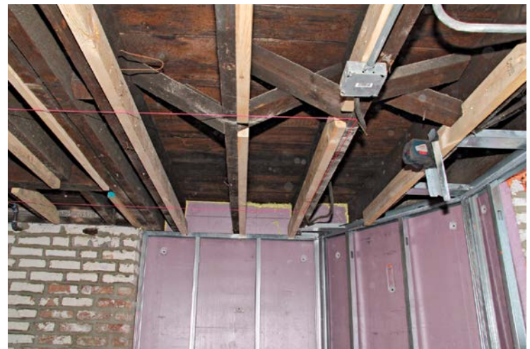
Here, the laser level shines on string lines and bottoms of sister boards to keep the new ceiling perfectly level.
