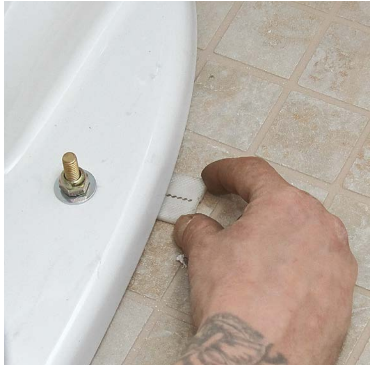
8 Push to see that the bowl rests firmly. Install plastic shims if needed.
