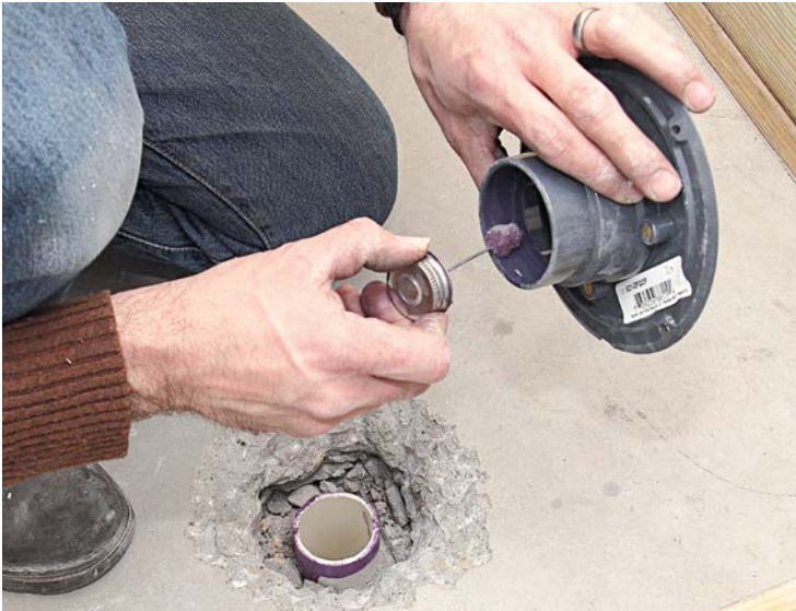
2a Prime the drain flange, ...
