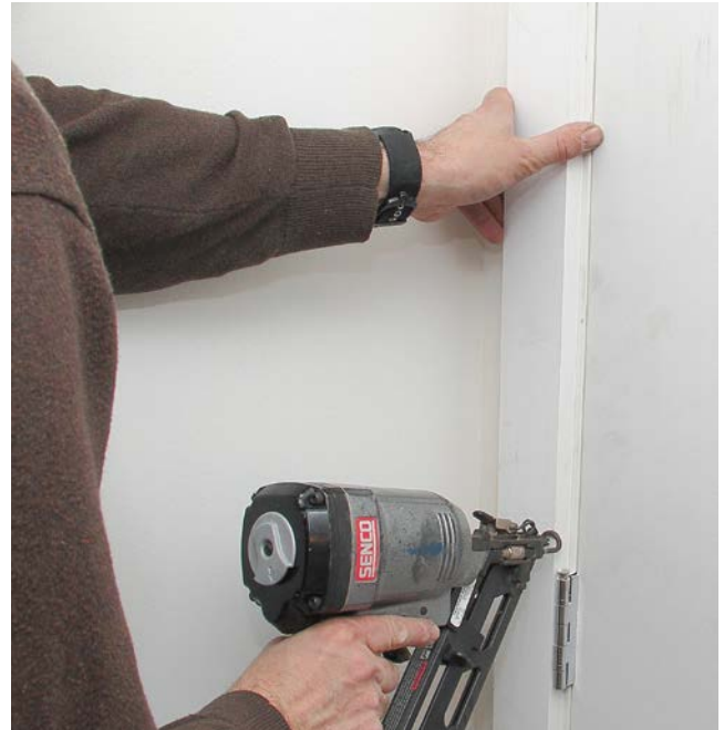
4 Cut side casing to height and install with pairs of nails along the reveal line.
