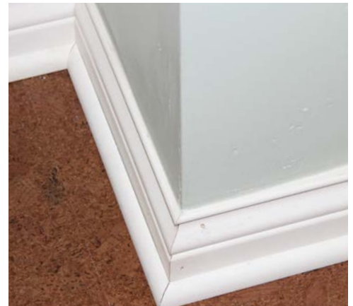
6 Base shoe can be simply cut at 45° bevels.
