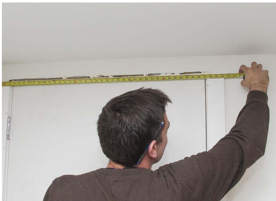
5 Measure and cut the head casing.
