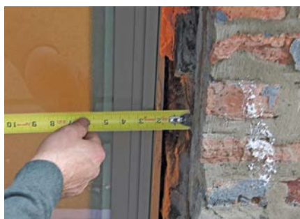
Measure to learn the thickness of the window buck pieces. Here, the window will rest on a piece of rigid insulation, for a bit less heat loss. Install to produce an opening that is square at the corners and about \frac{3}{8} in. narrower and shorter than the window.
