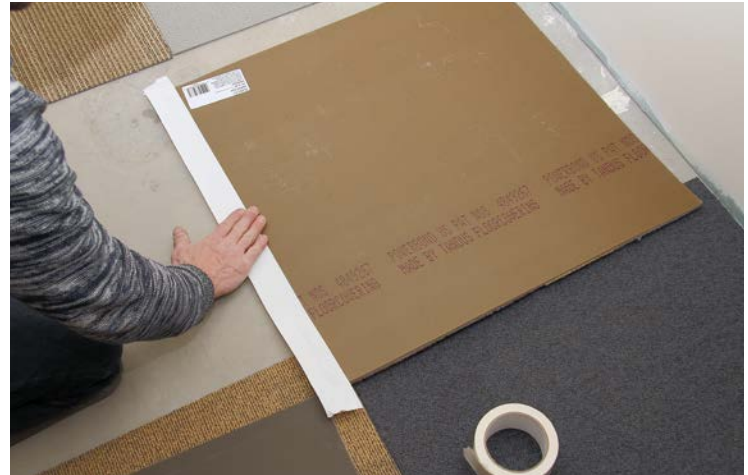
3 To adhere with double-sided tape, press the sticky side onto the underside of a tile, allowing it to overhang.
