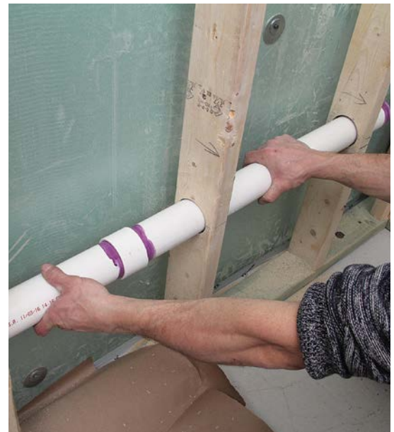
9 Slip sections of pipe through the holes.
