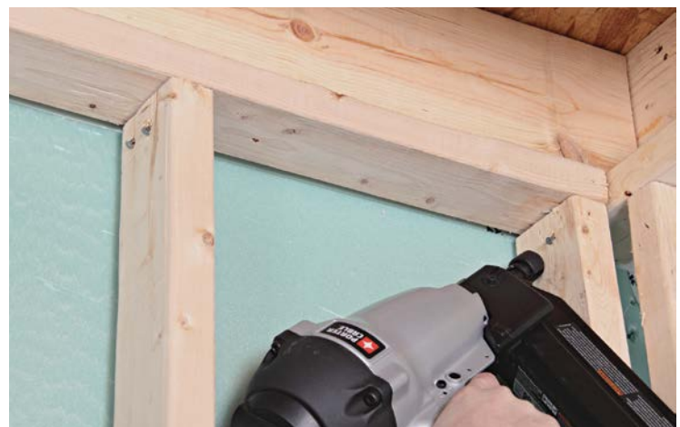
8 Drive nails or screws at angles to attach the studs to the plates.
