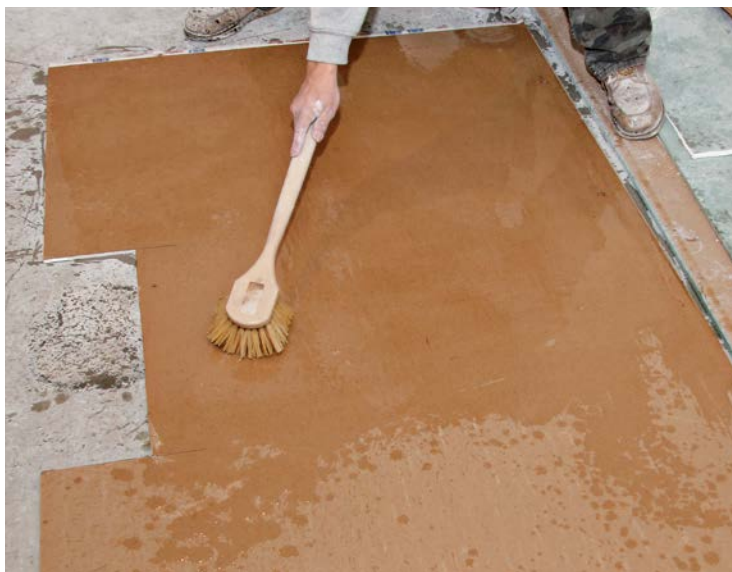
3 Wet the backside of sheets of \frac{1}{4} -in. drywall to make them pliable.
