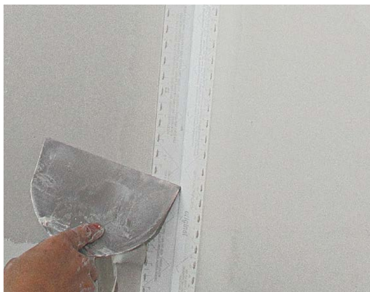
6 Apply another coat of compound on top of the tape.
