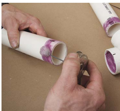
5 Apply a generous amount of PVC glue to the pipe ends and insides of fittings.
