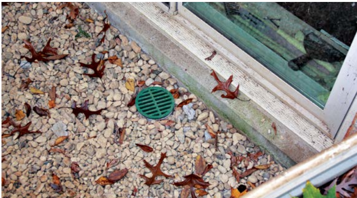
The drainpipe's grate is placed at a low spot at the bottom of the window well. The grate, and the surrounding gravel, should be a couple of inches below the masonry window opening. It's important to keep the grate clear of leaves and other debris that could clog it.
