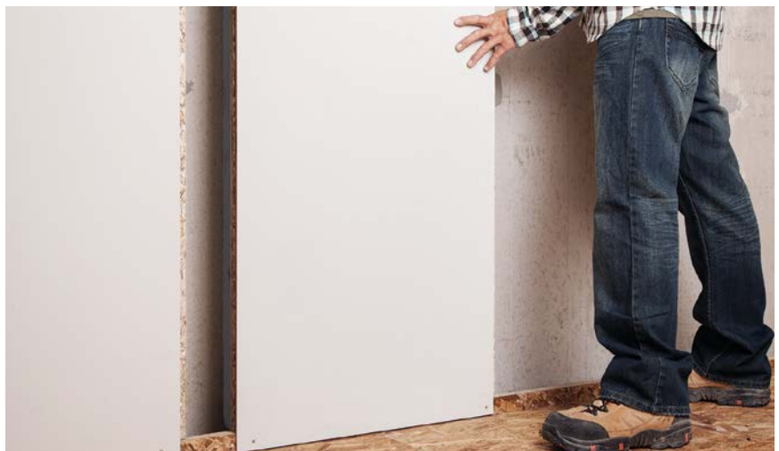
4 Slide the next panels so the tongues and grooves nest firmly, and screw to the tracks.
