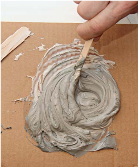
3 Mix a batch of two-part epoxy.
