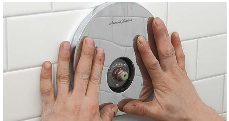
4b . . . then the escutcheon is snapped into place.
