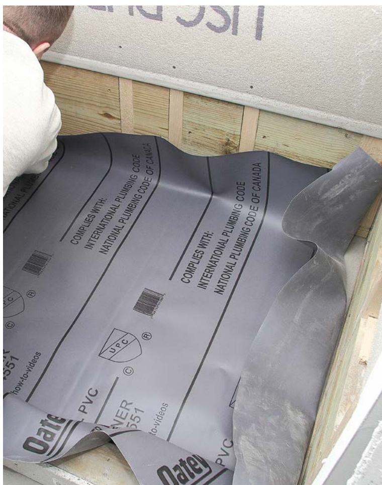
3 Set the liner on the floor and smooth it out.
