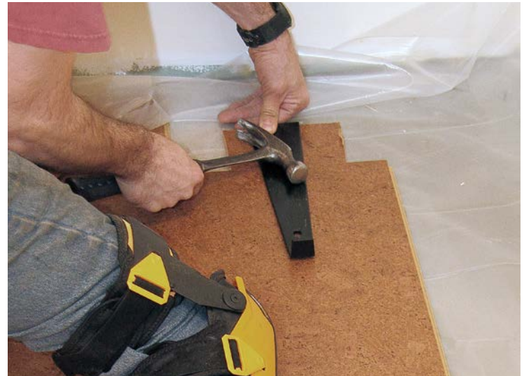
10 Near an end wall, use a pulling tool and press down on the other end.
