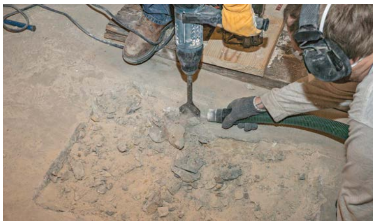
1 Chip out the damaged area to a depth of at least 1½ in.
