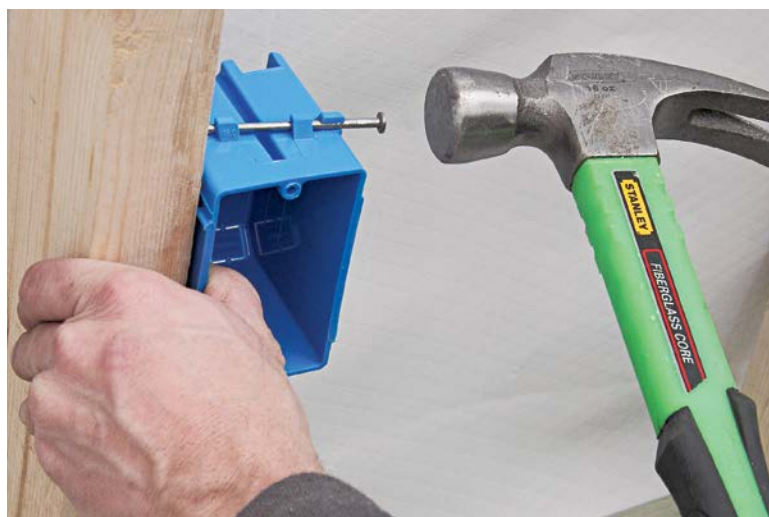
To attach this plastic box, simply position it using the guide, so it extends \frac{1}{2} in. out from the stud, and drive the nails.
