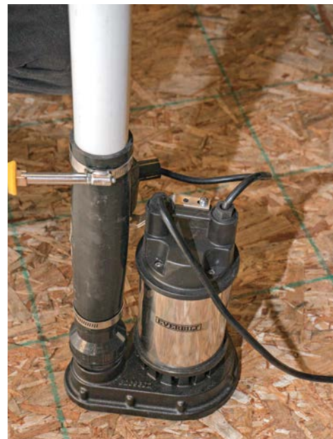
This submersible pump is attached to a check valve (just below the rubber fitting), which keeps water from backing up into your home. A discharge pipe rises out of the pump. The pump gets plugged into a standard 120-volt electrical receptacle.
