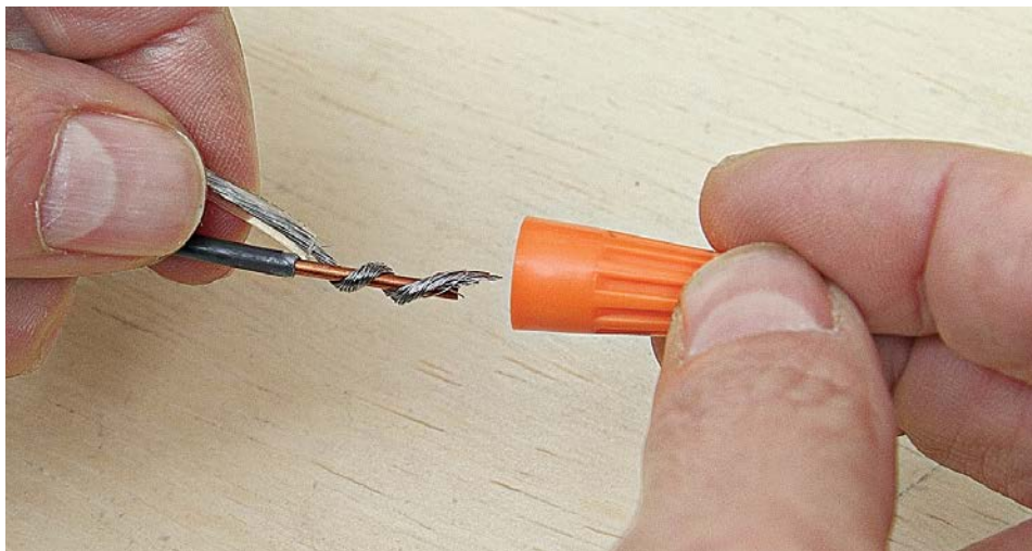
Wrap a stranded wire around one or more solid wires and tighten with a wire nut.
