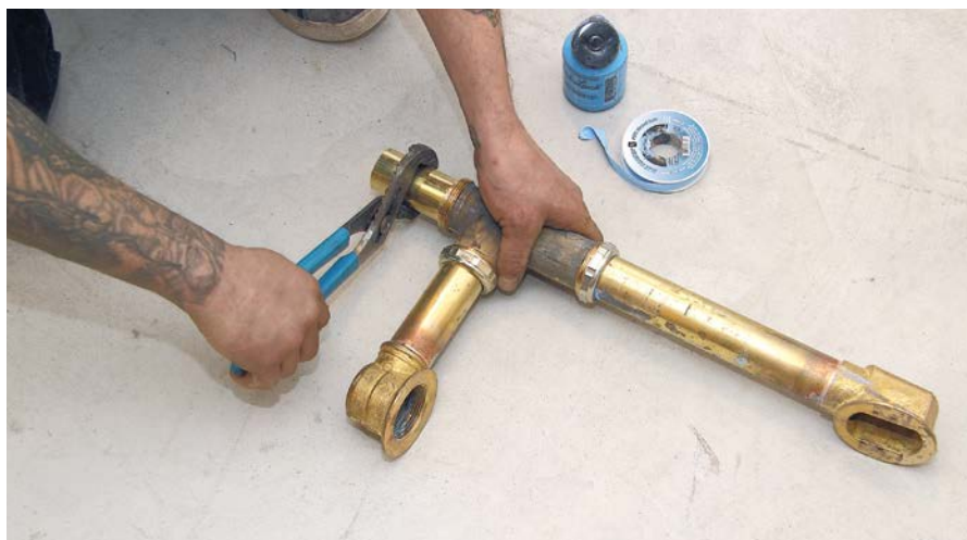
3 Put together a waste-and-overflow assembly and test that it fits on the tub.
