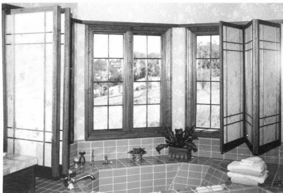
Hinged shoji screens can be used on bay windows or other nonlinear planes unsuited to sliding screens. Here, fiberglass on the window side provides insulation. The inside panels are fitted with hand-batiked fiber to match the wallpaper design. Shoji in a bathroom offer privacy without blocking off natural light. Designed by Max Perlman, Wiseman Lighting and Design. U.S.A.
