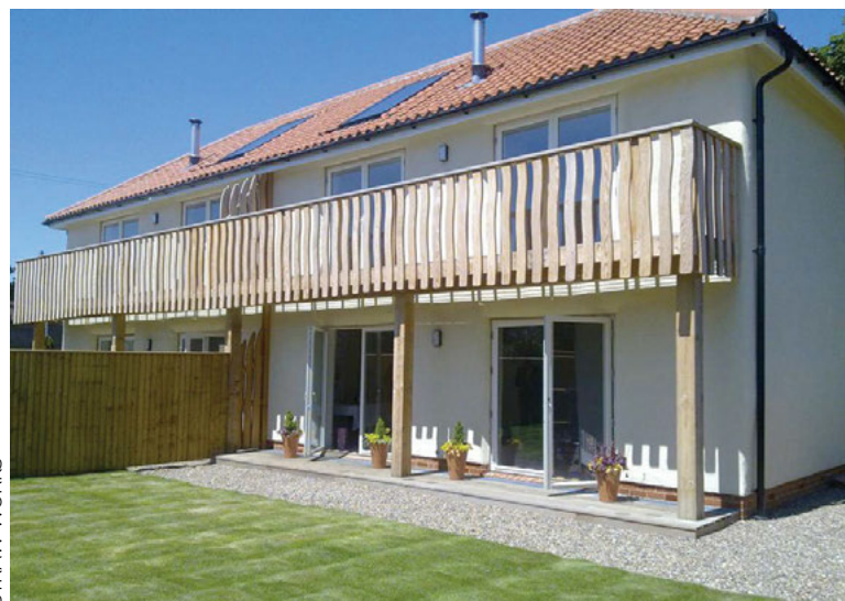
Below: Council houses designed and built by Straw Works.
