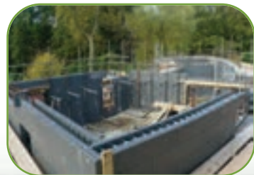
Curved Thermowall Construction.
