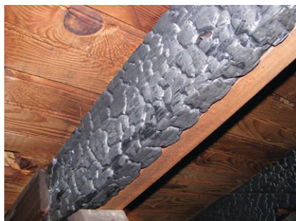
"Sistering" alongside a charred beam can help with stability.
