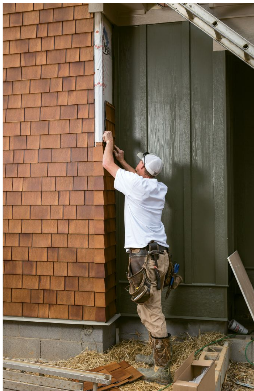
TANDO Beach House Shake is fabricated from a polypropylene material and designed to be almost indistinguishable from traditional cedar shake. The siding can be installed by a single worker and is available in shades of fresh cedar, weathered grays and a redwood-stained look (shown here). Circle 5 on inquiry card
