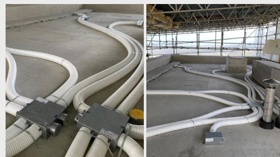
(above) Installation of the MVHR system at the first passive house in the Channel Islands.
