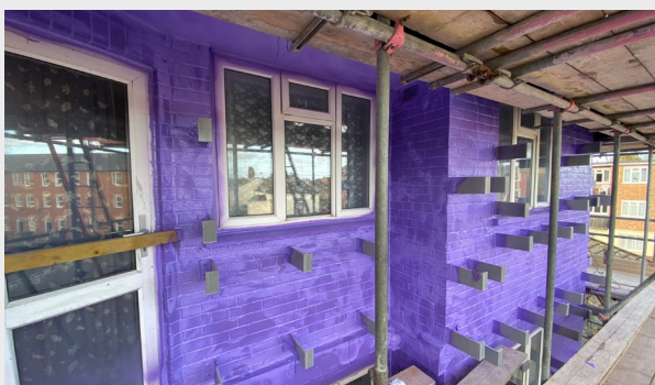
(above) The external airtight layer and void-forming brackets in place at Beattie Passive's Enerphit project for Great Yarmouth Borough Council; and (right) a rendering of the finished scheme.
