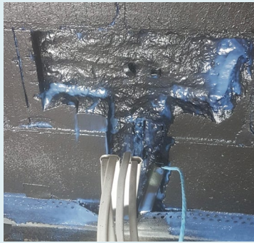
(above) Blowerproof applied to the inner face of blockwork at a wall chase before dotting and dabbing plasterboard, in architect Mel Reynolds' project in Sandycove, Co. Dublin. The project is aiming for the passive house plus standard.
