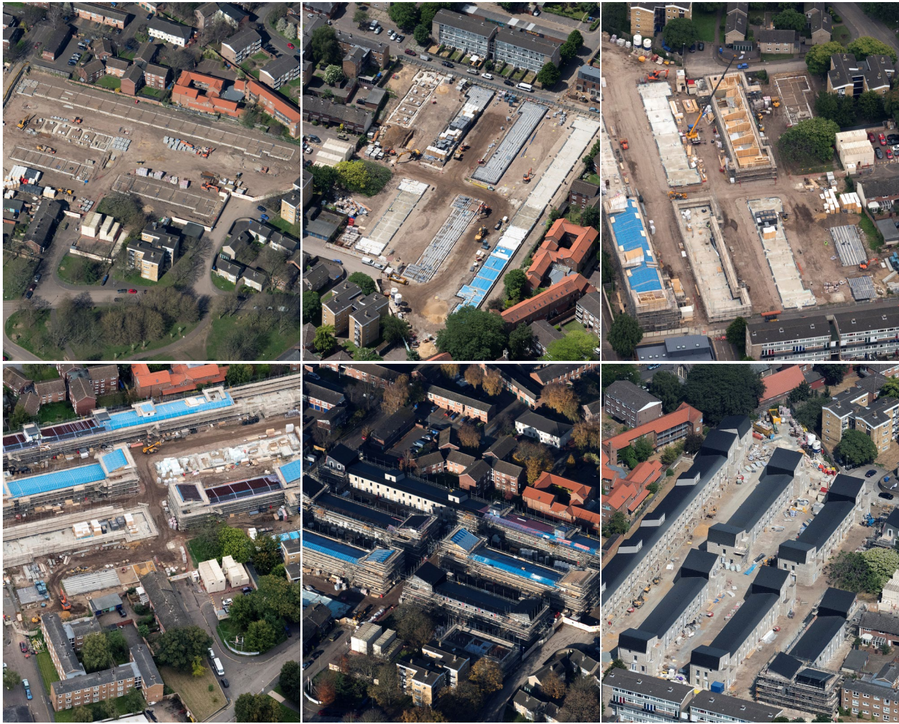
above Drone shots of the site on the west side of Norwich city, showing progress from the beginning of works to the completion of the build.
