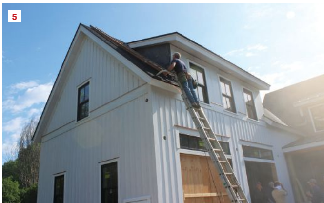
Co-author Jim Bradley points to smoke leaking from double-hung windows in living space above the garage (4). After checking the window openings and dormer framing, workers determined that the window units themselves were leaking (5).
