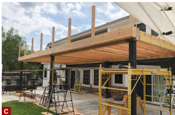
Figure 3. Instead of a ledger, a 7x14 PSL flush carrying beam (one was also installed at the outside edge of the deck) provided support for the freestanding deck at the house (A). To complete the seismic design, the inside and outside carrying beams were connected to each other with 6x12 Doug fir beams, which were fastened with \frac{3}{4} -inch-diameter through-bolts to brackets welded to the steel columns (B). 2x12 Doug fir joists were hung from the carrying beams, which were blocked out with 2x12s sandwiched around the 4x4 deck posts bolted to the framing (C). Because the entire deck would be protected by a waterproofing system, non-PT-treated material and engineered lumber was used in its construction.
