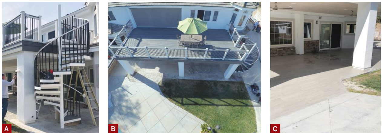
Figure 8. The new stucco finish on the columns and soffit was painted to match the existing house (A, B). To wrap up the project, the old concrete patio was prepped to receive new plank-style patio tiles patterned to match the deck's wood ceiling (C). Though not shown in the photos, a new door that provides access to the upper level was installed in a follow-up project.
