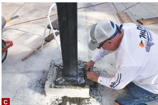
Figure 2. Fabricated by a certified welding shop, each of the engineered steel columns weighed about 250 pounds; a portable contractor's lift was used to hoist them into position on top of the concrete piers (A). The lift would also be used to hoist heavy 7x14 PSL beams into place on top of the columns once the columns had been bolted to the piers (B). Workers turned the nuts supporting the columns with a box wrench to adjust the columns' height and plumb, then packed the voids between the column base plates and piers with non-shrinking grout (C).
