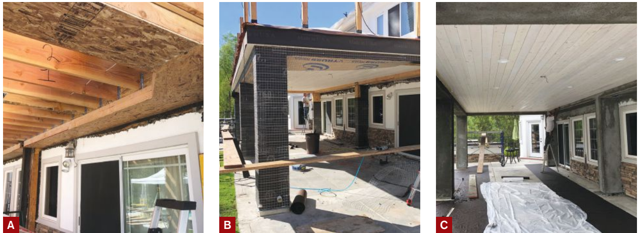
Figure 5. Underneath the perimeter of the deck, workers framed a soffit and covered it with OSB in preparation for a stucco finish (A). After covering the soffit and boxed columns with building paper and wire lath for the stucco (B), workers installed the tongue-and-groove wood plank ceiling (C). J trim was installed at the corners where the ceiling would meet the stucco to give the installation a clean look.
