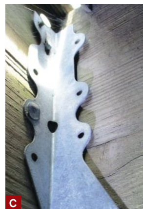
Figure 3. White rust is already forming on this joist hanger, which is only approved for interior use (A). Metal-roofing screws aren't approved joist-hanger fasteners (B), nor are roofing nails (C). All of the holes in metal hardware should be filled with approved hanger nails or structural screws, and the hanger flanges should fit snugly against the joist (D). Metal hardware shouldn't be field-modified; with its seat removed, this hanger provides minimal joist support (E).
