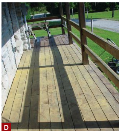
Figure 2. Sometimes a light sanding with a random-orbit sander (A) is enough to prep decking for a new finish. On large decks, you may want to rent a walk-behind drum or orbital sander (B). If fastener heads are flush with the surface, aggressive sanding (C) can remove their protective coating. After scuff sanding (D), be sure to clean up all dust before recoating.
