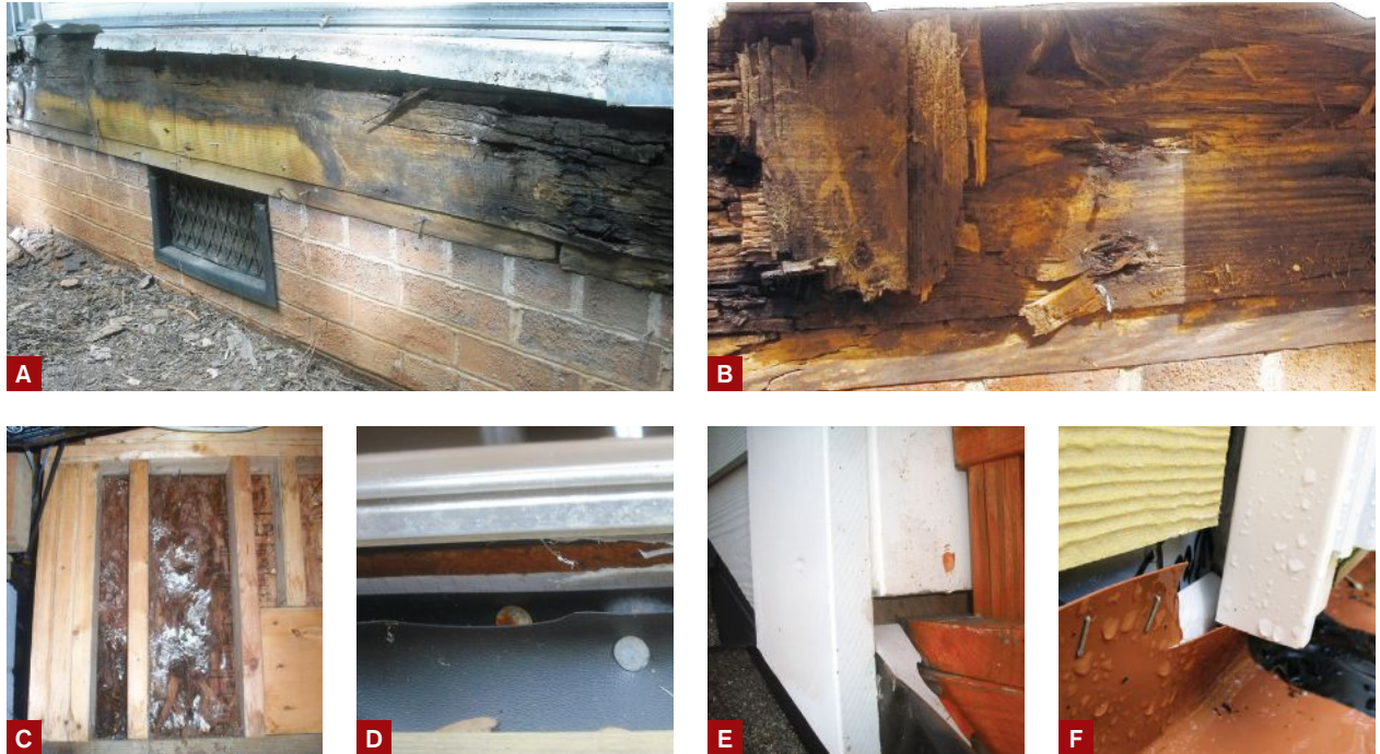
Figure 5. The sheathing and band joists on these homes (A, B) are in rough shape, thanks to moisture intrusion from their decks, and require replacement. Improperly installed ledger flashing on a one-year-old deck was the cause of this water damage (C). Flashing is often improperly installed underneath door thresholds (D) and where ledgers intersect with other building components, such as a roof (E). During a new-home inspection, the author discovered flashing that hadn't been integrated with the water-resistant barrier underneath the home's siding (F).
