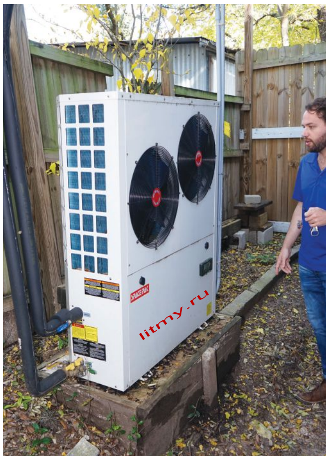
Outside the building, a 3-ton SpacePak Solstice air-to-water heat pump dumps excess heat from the building to the outdoor air—just one of many possible solutions that are possible with radiant cooling.
