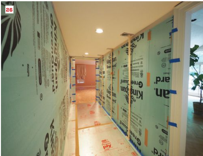
Hardwood stairs can be protected using hardboard or plywood tread covers (24), secured to skirtboards using cleats. For stair railings, the author recommends wrapping the railing in sill sealer and tape (25). Foam board works well for protecting walls (26).
