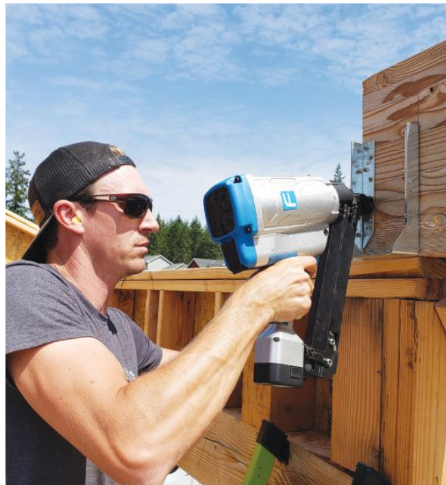
Kyle Davis installs a joist hanger using a Fasco America F70G gas-powered hoseless positive placement nailer.
