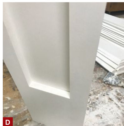
Figure 2. On most frames, the author cut a \frac{3}{8} -inch-deep rabbet with a router around the inside back edge, then glued the \frac{3}{8} -inch-thick PVC panel to the frame. Clipping the panel edges at a 45-degree angle allowed the panels to fit the rounded corners of the rabbet (A, B). For a deeper, \frac{3}{4} -inch panel reveal, the panels could simply be glued and stapled to the back of the frame (C, D). The edges of each frame were ripped to 45 degrees so that they could be glued together to form the post sleeves (E).
