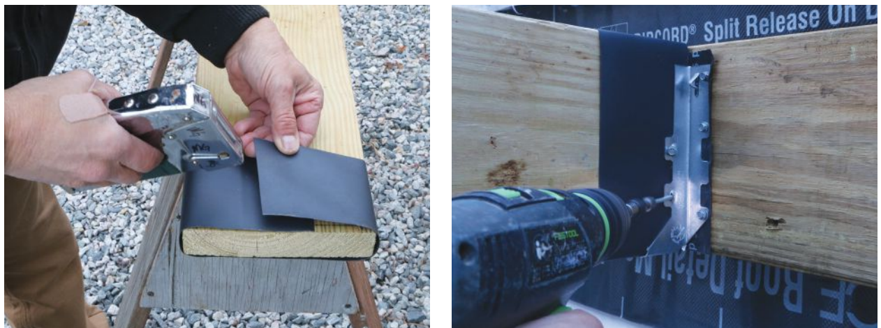
Figure 3. Applying a staple-on isolation membrane or a self-adhering membrane to joist ends (above left) and the ledger (above right) reduces the rate of galvanic reaction between the treated lumber and the metal hanger.
