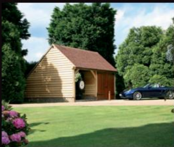
OAK FRAMED BUILDINGS
